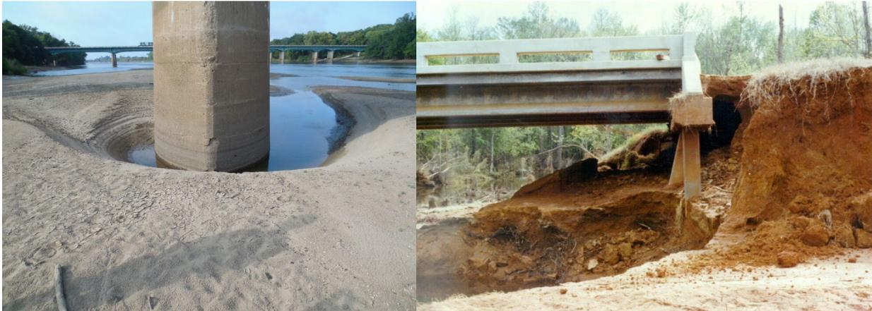
**Figure 1:** Examples of the damages scour causes around bridge piers (left) and abutments (right). Source: US Geological Survey (USGS).
