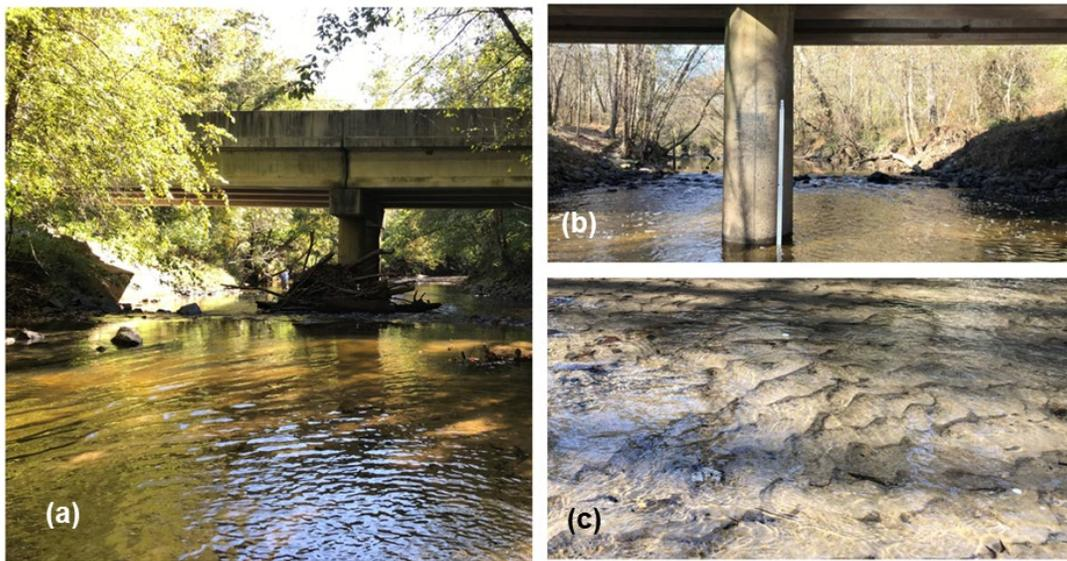
**Figure 13:** The Glenn Rd bridge crossing over Ellerbe Creek in Durham, NC, USA viewed from upstream (a) and downstream (b). The channel-bed material is characterized as medium sand with less than 5% fines (c).
