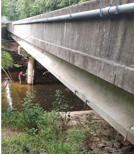
**Figure 11:** The electrical PVC conduit used to secure the electrical and FO cables along the side barrier of the bridge.
