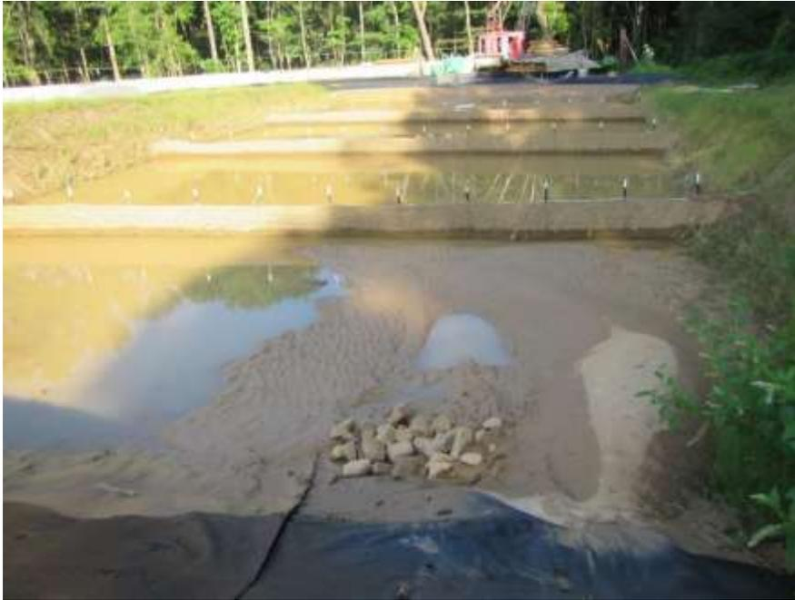
**Figure 3.3.** Picture of Basin 3 at one of the two inlets. Sampler tubing can be seen along the top of the first baffle.
