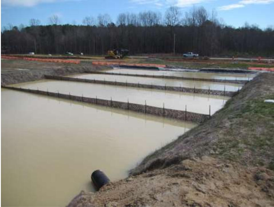
**Figure 3.5.** Picture of Borrow Pit Basin during skimmer discharge period.
