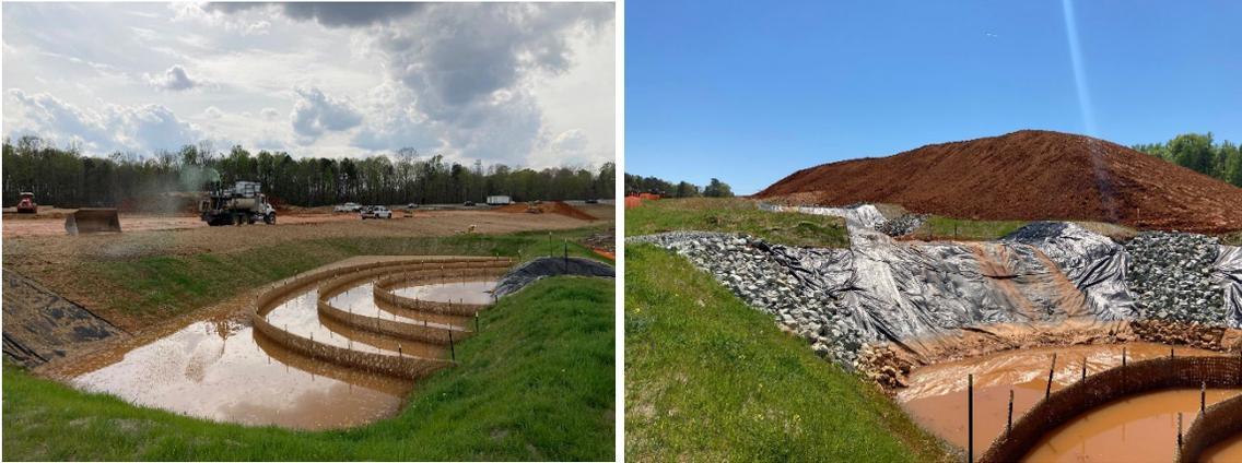
**Figure 19.** Basin A and Basin C-3 (tiered) at the I-40/NC86 site.
