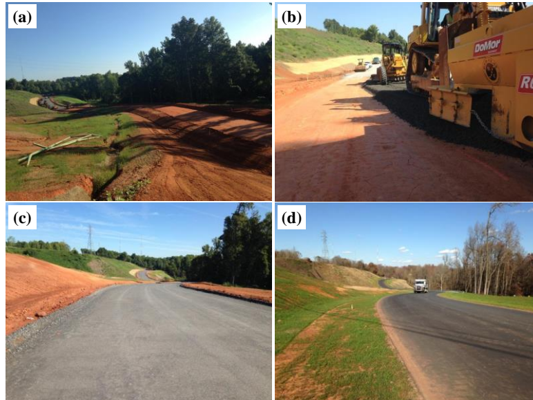
Figure 4. Images of Pineville quarry site during construction; (a) compacted subgrade, (b) placing cement treated base, (c) compacted base, and (d) finished surface.
