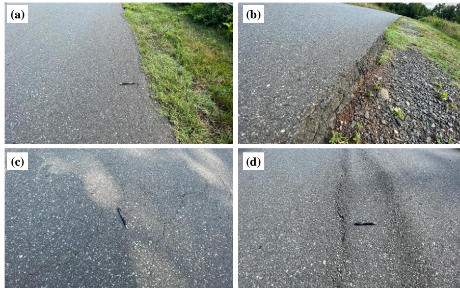
Figure 8. Select photographs from July 2022 condition survey on conventional test site; (a) edge cracking at northbound 10+00, (b) shoulder deterioration at northbound 11+00, (c) fatigue cracking at northbound 14+59, and (d) slippage cracking at northbound 14+25.
