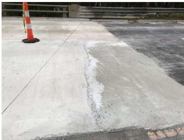
Figure 6-6: Substandard LMC-VES Concrete (Ripped out Later).
