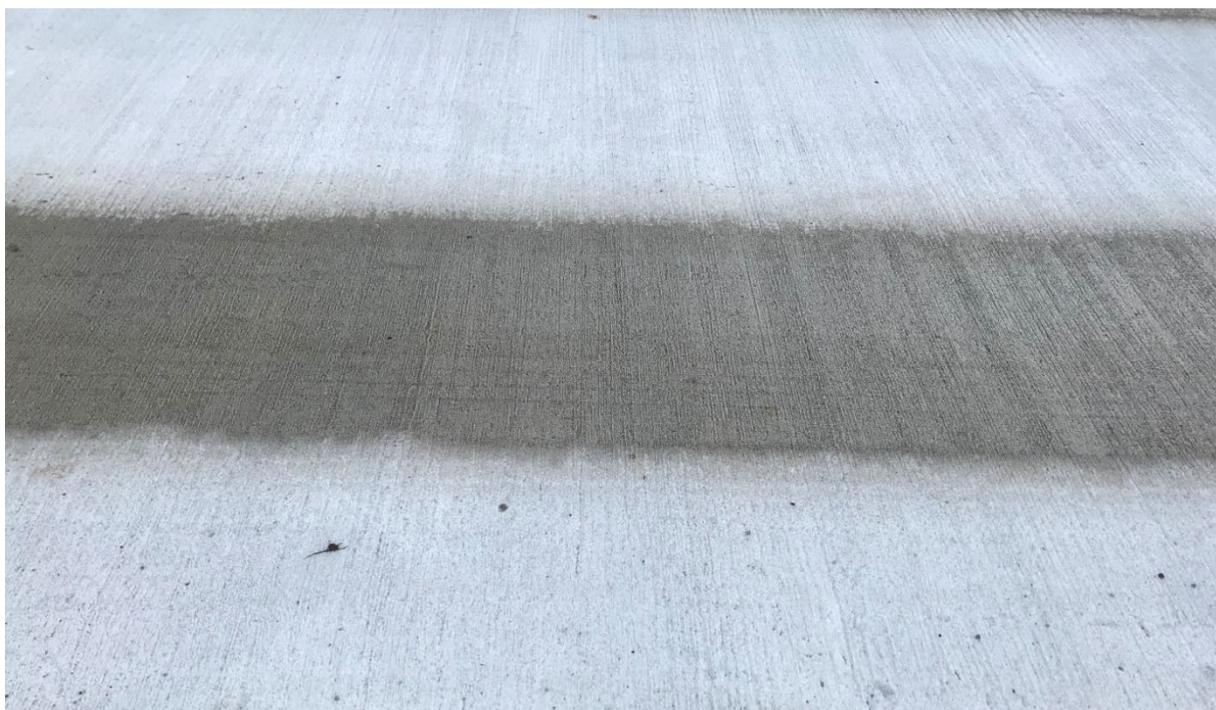
Figure 6-14: Lane 1 Surface (Water Applied to Look for Cracks).
