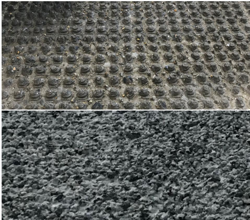
Figure 5-7: Comparison of Simulated Base Slab Surface (above) and Typical Scarified Bridge Deck Surface (below).
