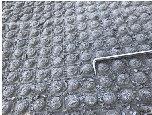
Figure 5-5: Intermediate Base Slab Surface (after removing mat, prior to pressure washing).
