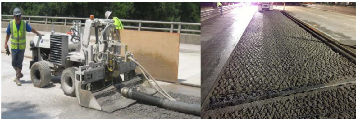
Figure C-1: Hydro Demo and Resulting Surface.
