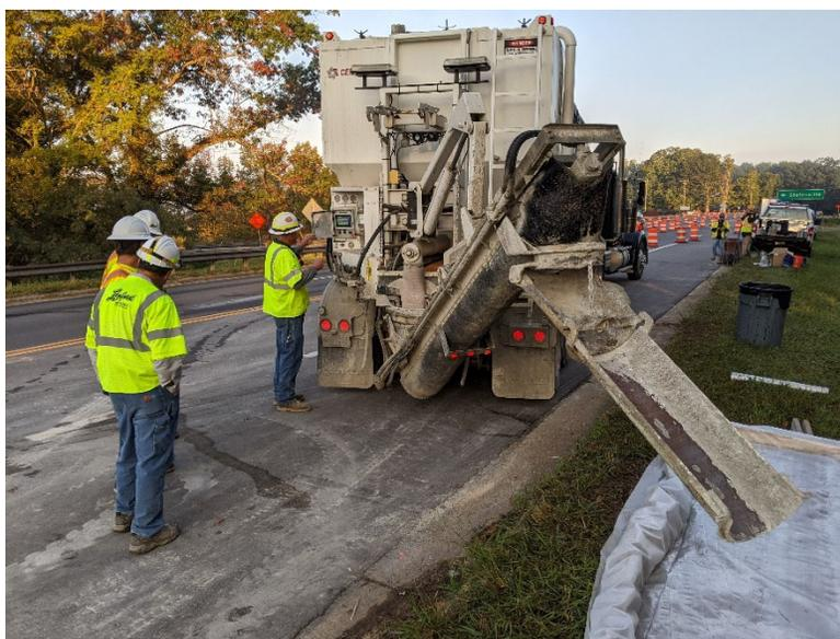
Figure 6-5: Preparing to Discharge Initial LMC-VES in the Inspection Area.
