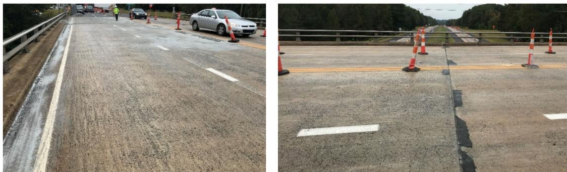
Figure 6-1: Bridge Prior to Overlay.
