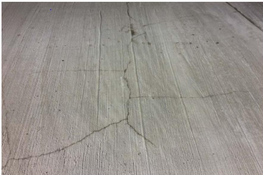
Figure 1-1: Overlay Cracking.
