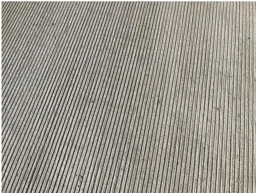
Figure 6-16: Final Grooved Surface, Typical of All Lanes.
