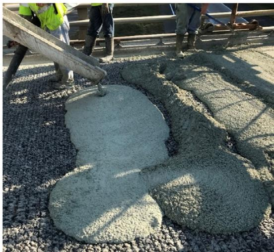
Figure 6-7: Transition to Retarder (citric acid at left, no citric acid at right).
