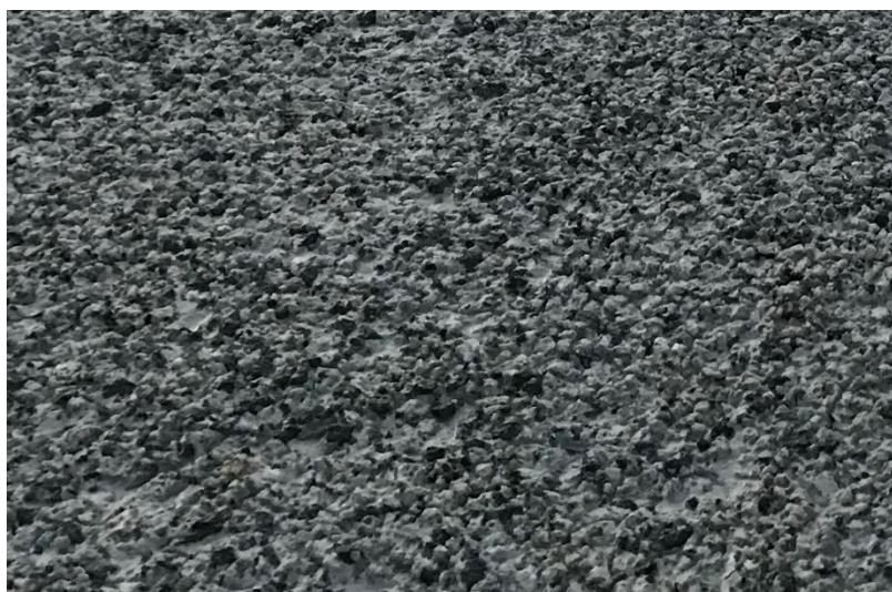
Figure 5-2: Typical Bridge Deck Surface after Hydro Demo.
