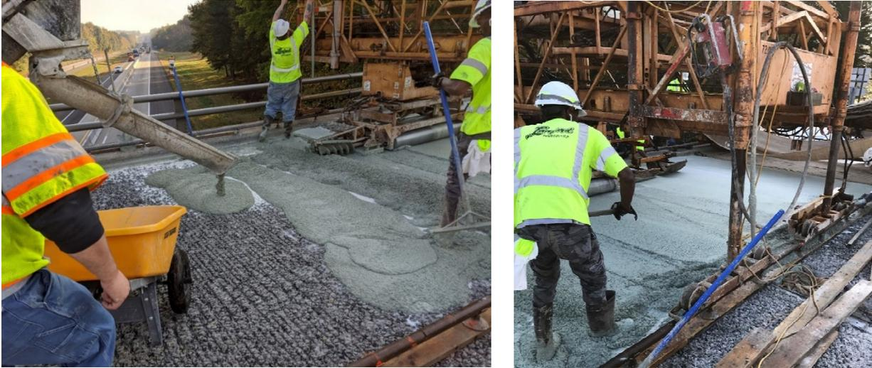
Figure 6-3: Concrete Placement (left) and Bidwell Screed (right).
