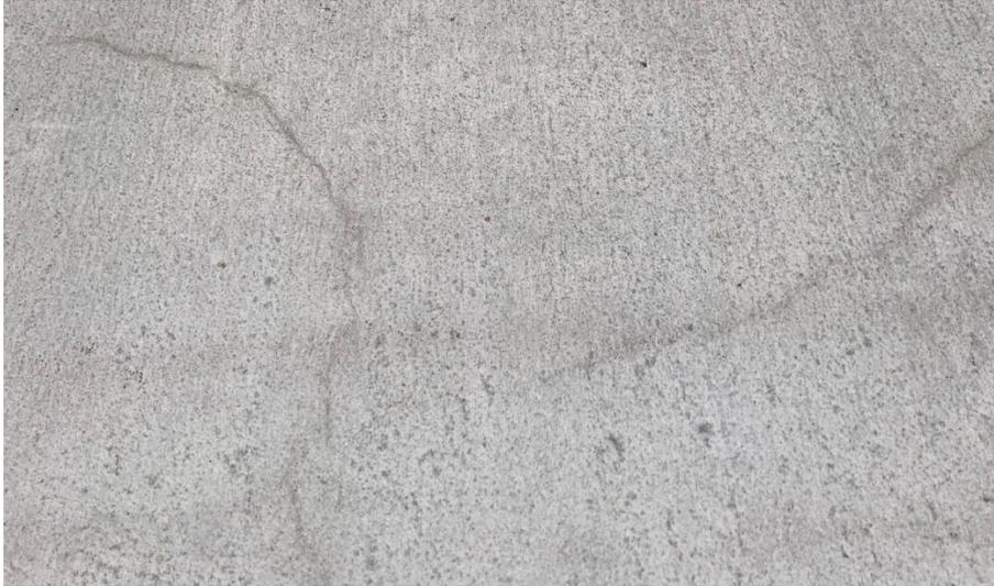
Figure 6-15: Lane 2 Cracking Near Cold Joint.
