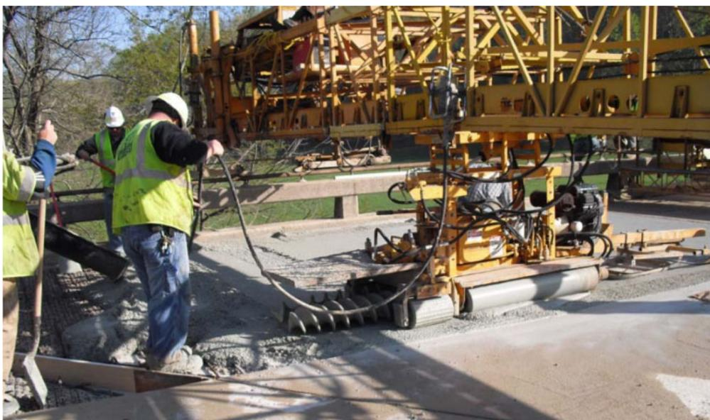
Figure C-2: Placing, Vibrating, Screeding, and Finishing.
