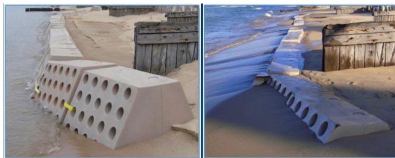
Figure A.7. A type of sandsaver (Sniffen, 2021).
