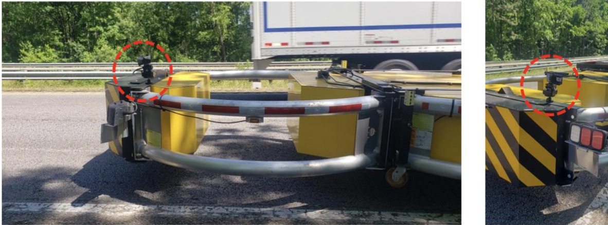
Figure 6 Mounting the sensor on crash attenuator
