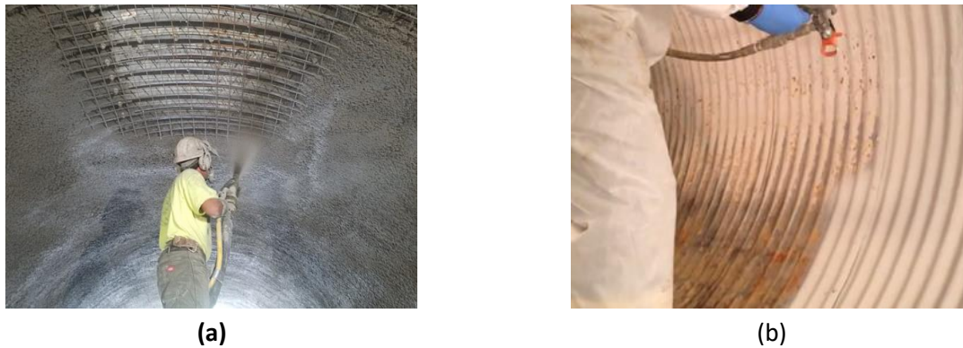
Figure 12. Examples of sprayed-on liners: (a) cementitious liners (Courtesy of Curtis Concrete Pumping), and (b) polymer-based coatings and liners (Courtesy of Epoxytec Intl, Inc.)
