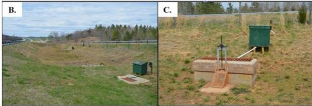
Figure 5. DDB is long and narrow (B) with an outlet structure in the center (C)
