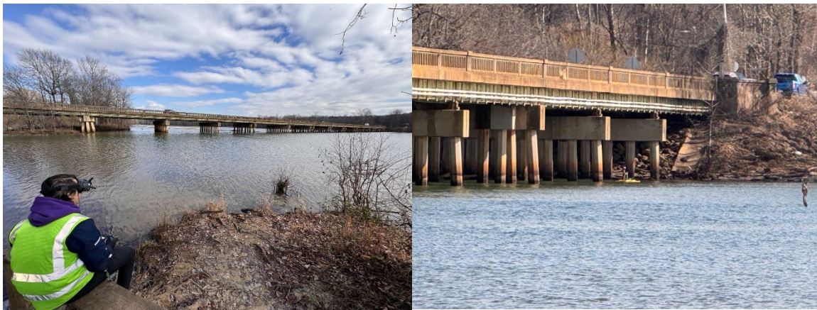
Figure 88: Left: Student piloting drone using first-person-view (FPV) goggles. Right HyDrone on the east side of the bridge near Bent 16.
