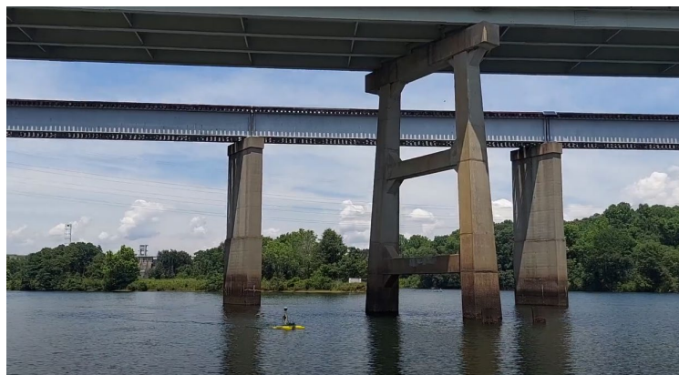
Figure 35: HyDrone performing a survey under a bridge during Test #10
