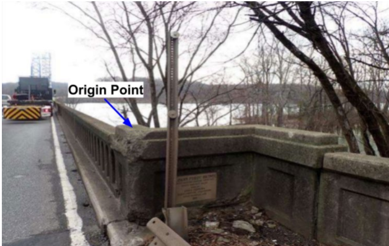
Figure 83: Location of origin point used for streambed profile measurements.
