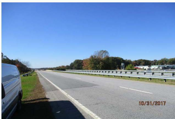
Looking Westbound From West Leg
