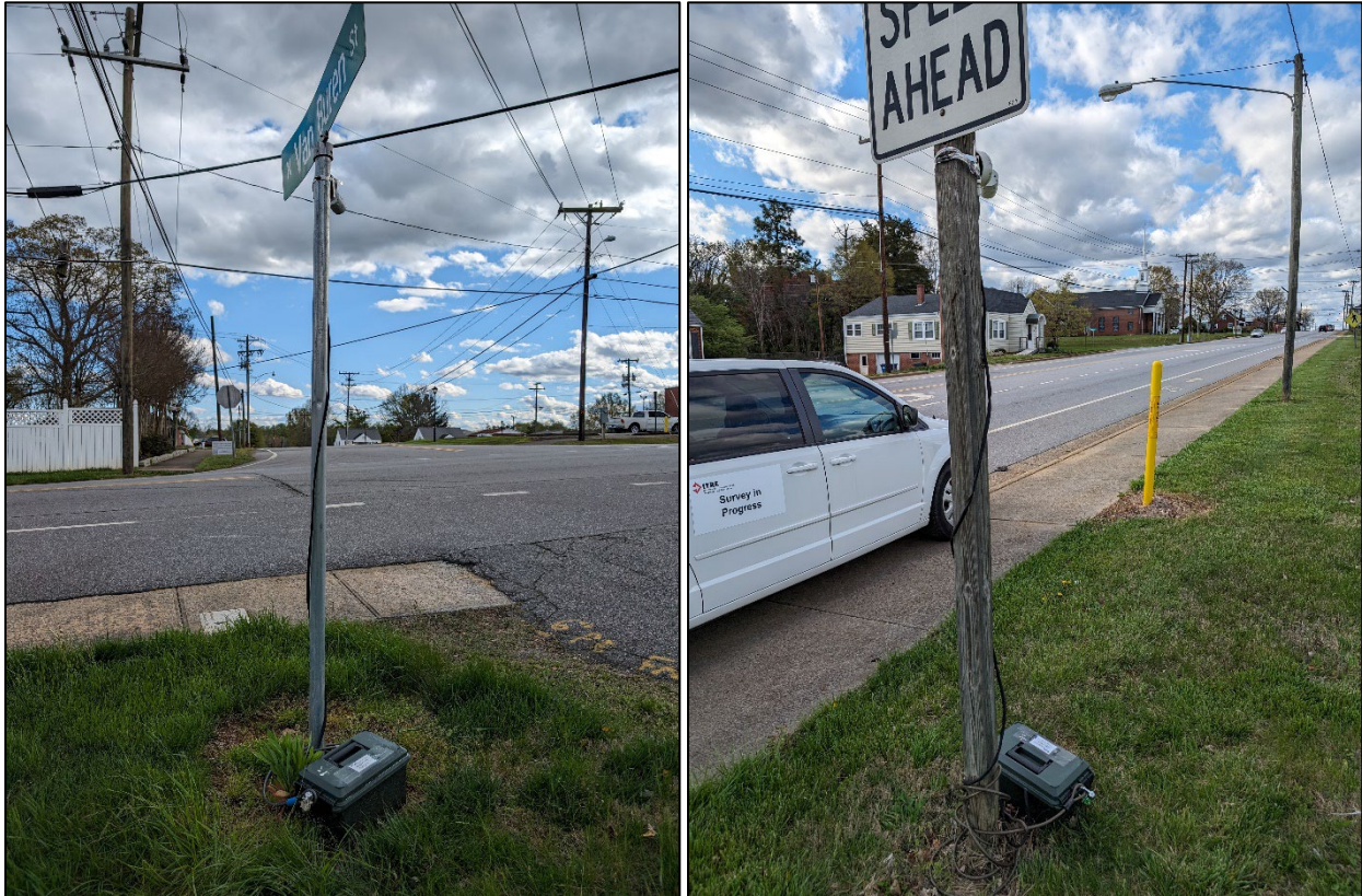
Example field install of data collection cameras
