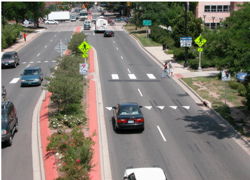
Figure 15. Package of potential midblock pedestrian crossing treatments to address multiple threat crash risk, crossing distance, and lack of gaps (pedestrian activated flashing signal) on higher volume, multi-lane street.
