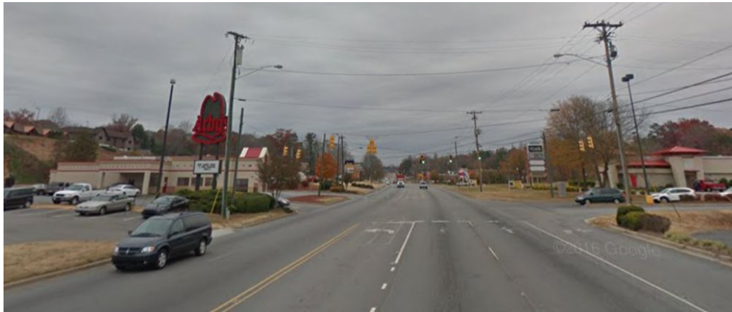
Figure 11 Signalized junction, left/right turn lanes and no pedestrian signals or crosswalks on US 321 junction with Eastwood Village. A visitor was killed when trying to cross near the intersection during early morning hours.
