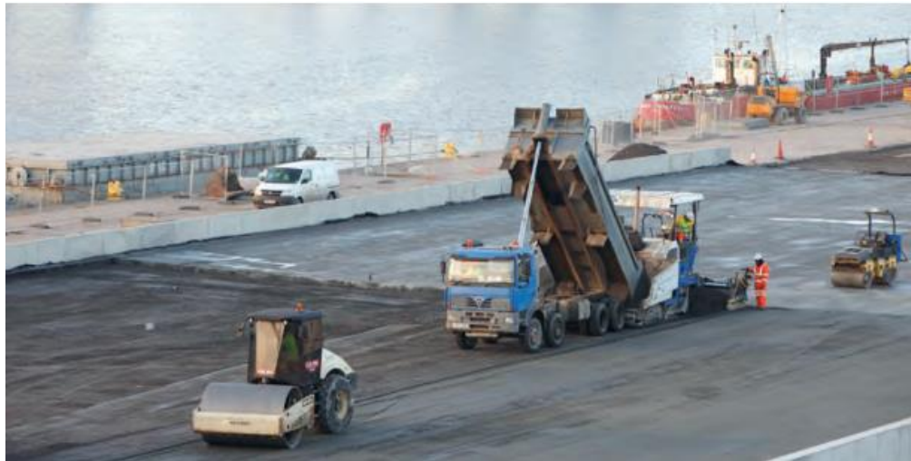
Figure 1.3. RCC roadway construction in the UK
