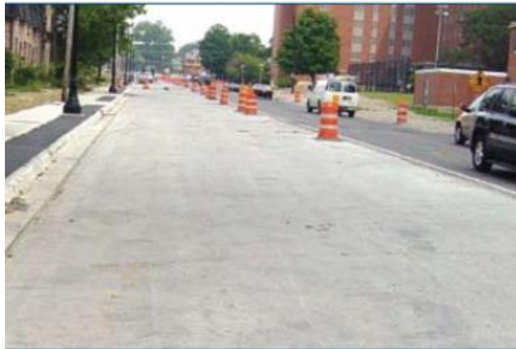
Figure 3.1. RCC pavement constructed in arterial street in Columbus, Ohio
