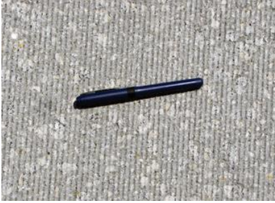
Figure 3.3. US-78 RCC pavement roughness in Aiken, SC
