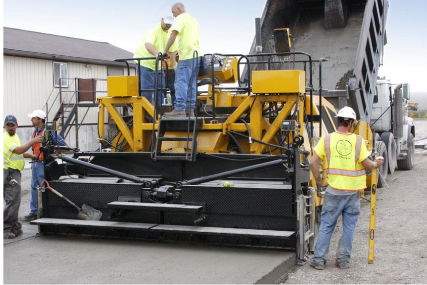
Figure 1.2. Roller-compacted concrete (RCC) placement
