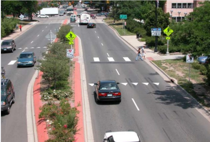
Photo: Potential safety countermeasures including midblock pedestrian crossing treatments to address multiple threat crash risk
