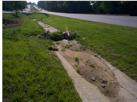
**Figure 3.3 – Lateral Ditches Blocked**
