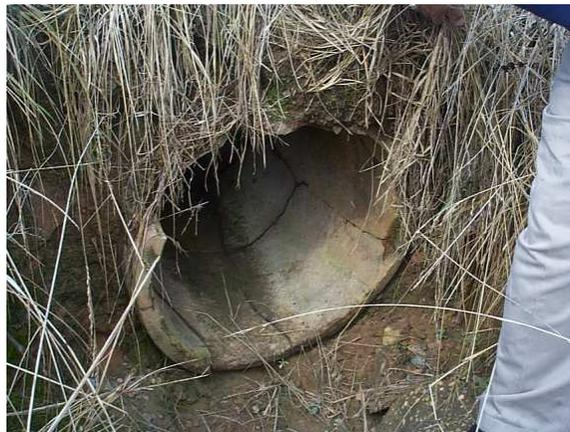
**Figure 3.7 – Crossline Pipes Damaged**
