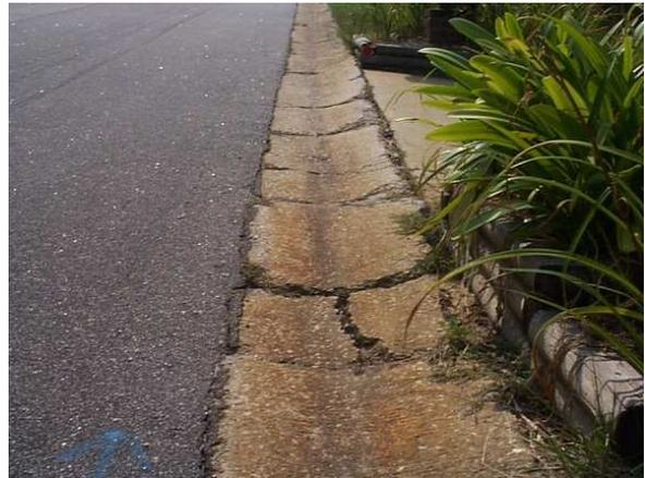
**Figure 3.9 – Gutters Damaged**
