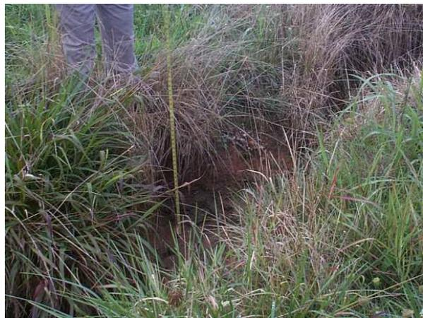
**Figure 3.4 – Lateral Ditches Eroded**
