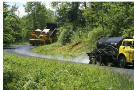
Preservation Bituminous Surface Treatment
