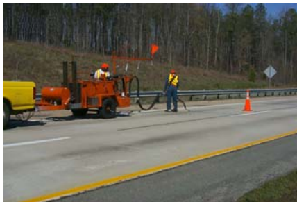
Preservation Crack Sealing
