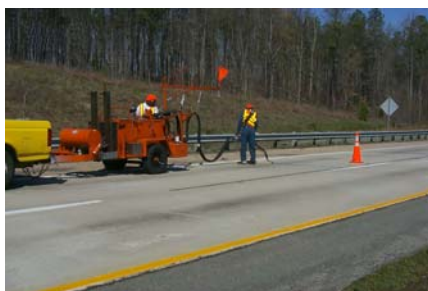
Preservation Crack Sealing
