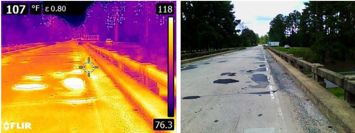
Figure 39: Example 1 of Known Damage, Left E4 thermal, Right E4 RGB image.
