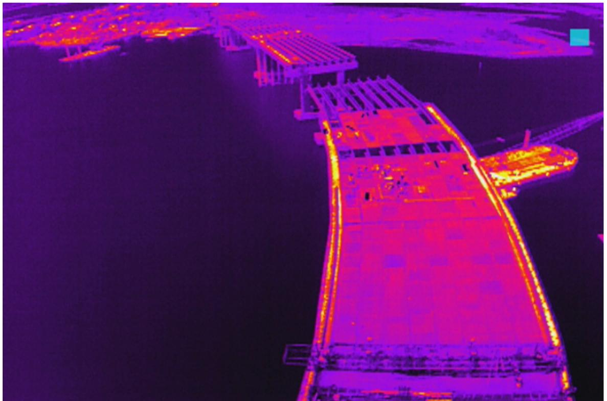
*Figure 50: Thermal Imagery of Gallants Bridge from NGAT Inspire UAS*
