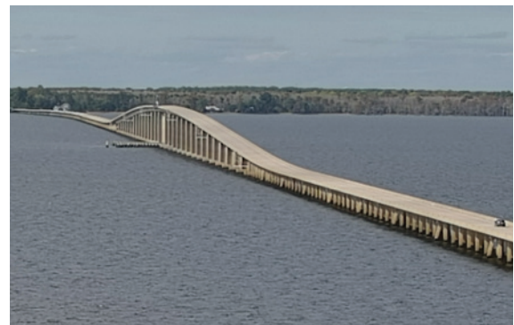
Albermarle Sound Bridge
