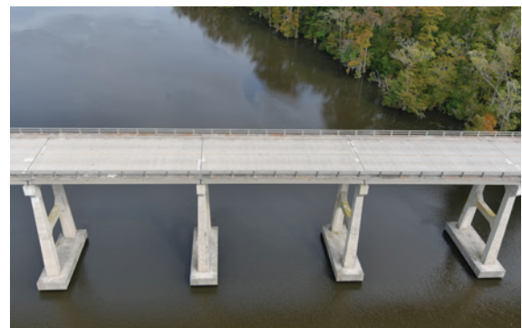
Three Rivers Bridge
