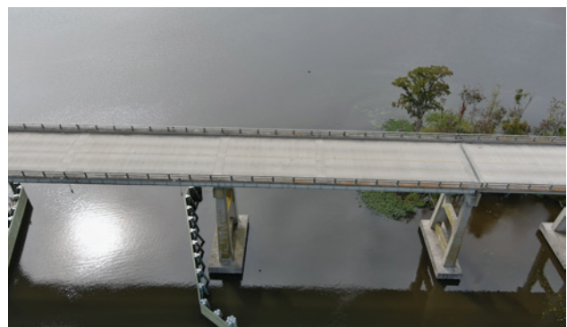
Existing Conditions at the BRITE Bridges
