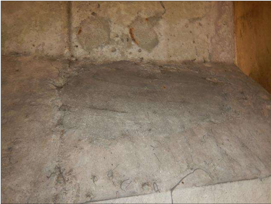
Span 31 Beam 8: [NEW REPAIR-PATCHING] FORMERLY --> spall with exposed rebar on the bottom left flange chamfer at 0.5ft from Bent 28 (14" x 8" x 1")
