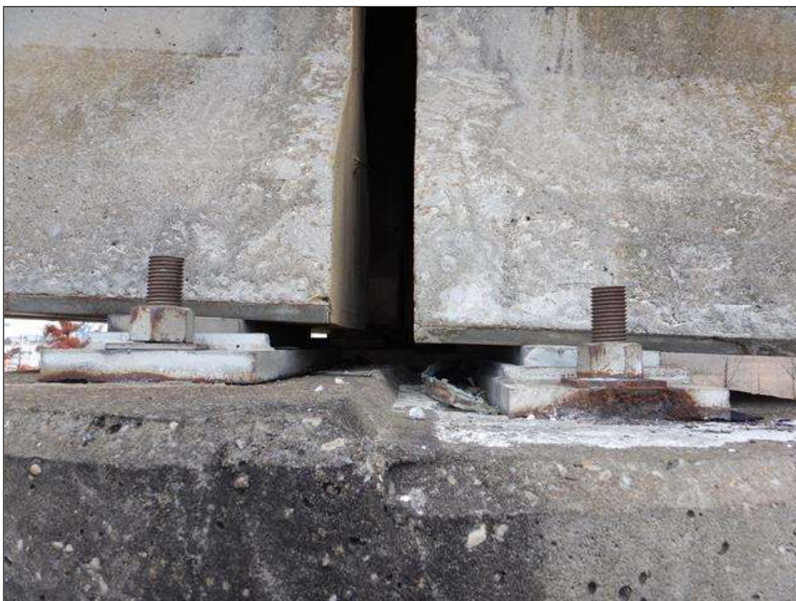
GIRDERS 1 BEARINGS AT BENT 10 [TYPICAL BEARING AT BENTS 1-10]
