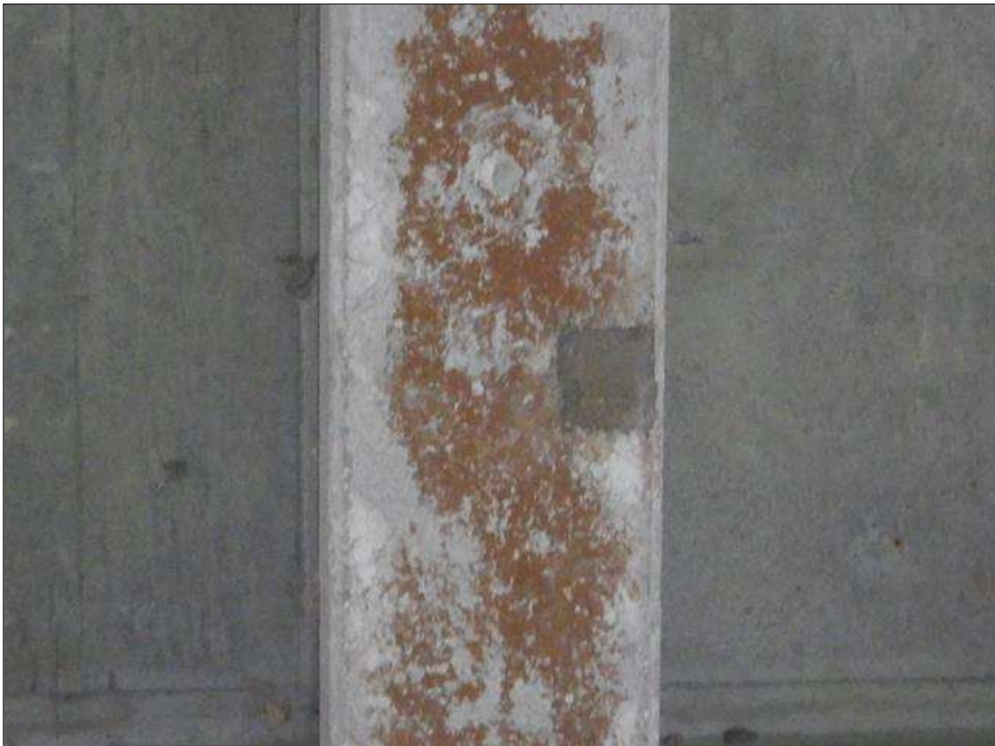
Span 8 Beam 2: [NEW REPAIR - PATCHING] FORMERLY --> (6" x 6" x 1/4") spall with exposed rebar on the bottom face at 24ft from bent 7
