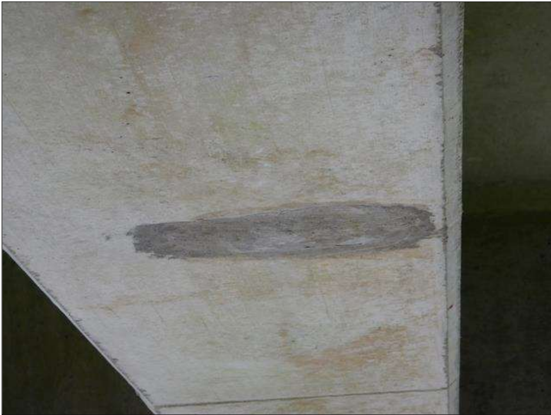
Span 11 Beam 4: [NEW REPAIR - PATCHING] FORMERLY --> (7" x 6" x 1/2") spall with exposed rebar on the bottom face at 27ft from bent 11
