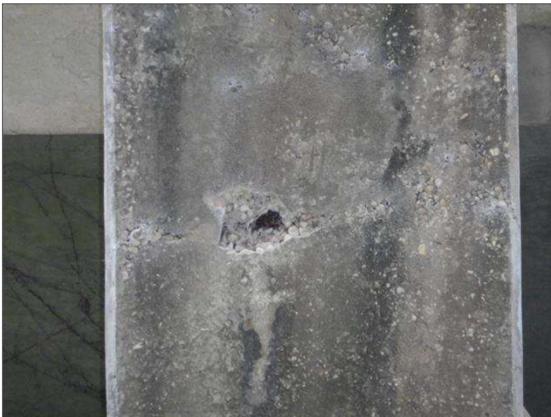
Bent 5 Cap 1: spall with exposed rebar on the bottom face under the left overhang (10" x 8" x 2")
