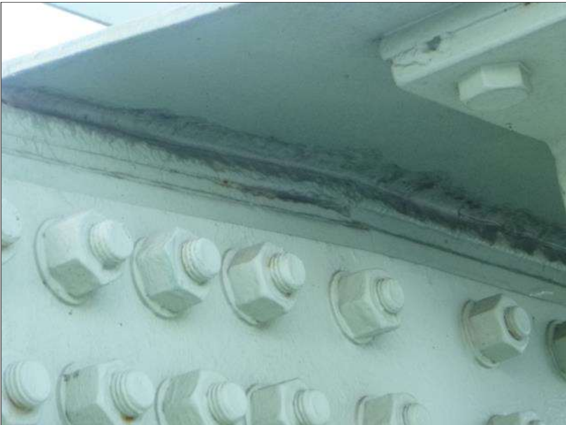
Span 18 Lift Span U7 SOUTH: 40" LONG X 1 1/2" WIDE AREA OF CLEANED AND PAINTED SECTION LOSS TO UNDERSIDE OF GUSSET PLATE SOUTH SIDE. (3/8" REMAINING)
