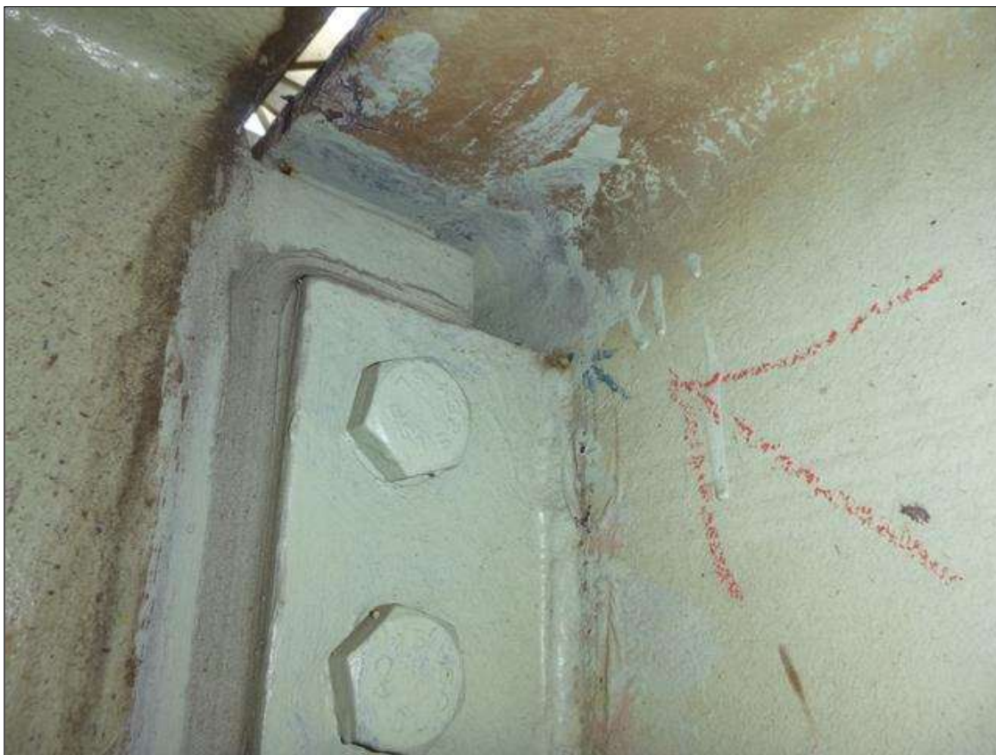
Span 18 Lift Span Stringer 8: REPAIR OBSERVED IN 2020 INSP: CRACKS NOT VISIBLE, AREA HAS BEEN PAINTED OVER. 2018 REPORT HAD BETWEEN FB's 8-9 - 1" CRACK IN WEB ACROSS TOP OF DIAPHRAGM CONNECTION, WIDE/ (2) 3/4" CRACKS IN CONNECTION WELD AT TOP
