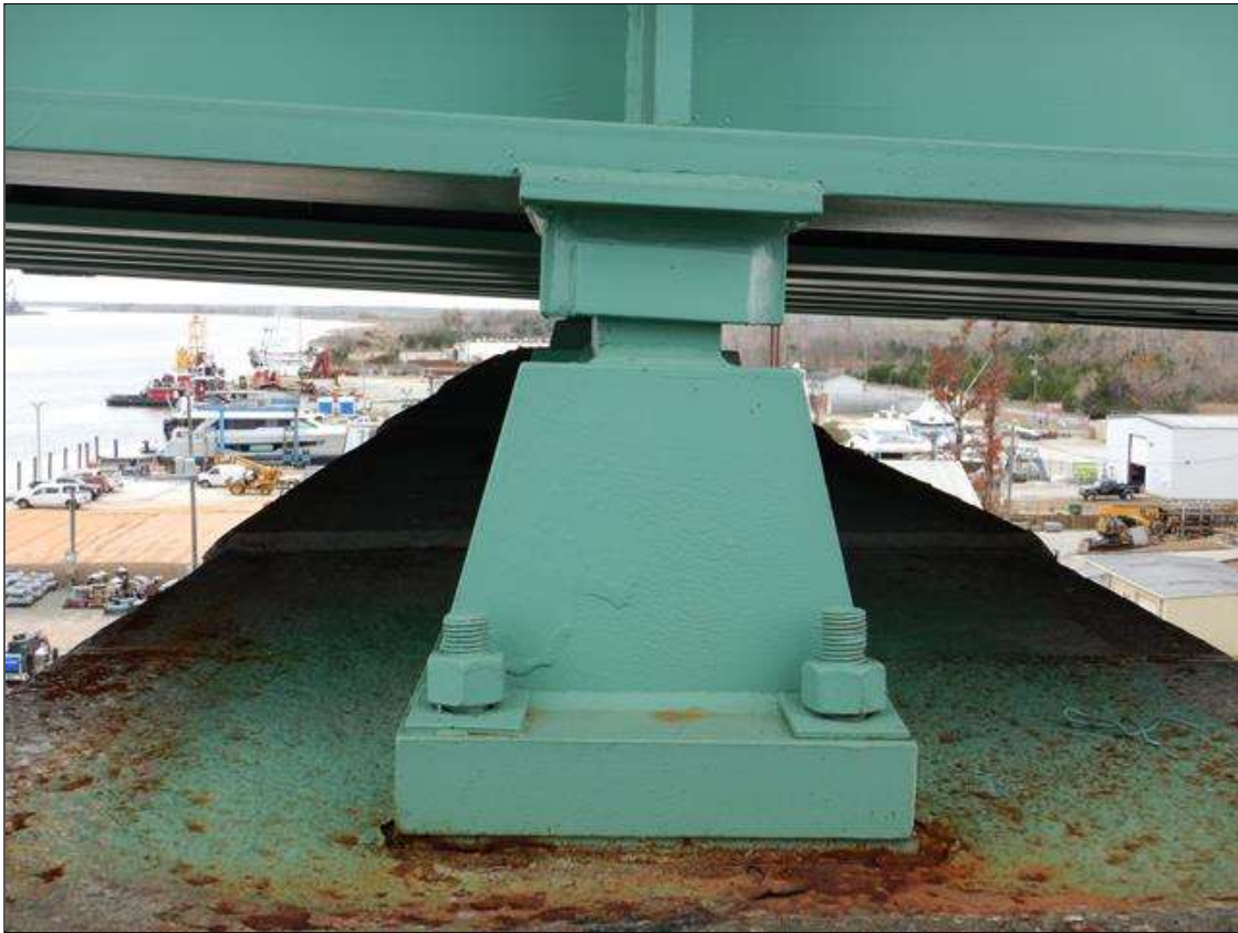
GIRDER 1 BEARING AT BENT 13 [TYPICAL BEARING AT BENT 13]
