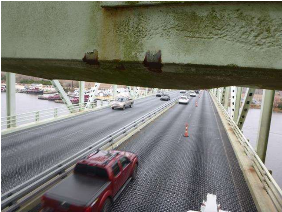
Span 19 EAST TOWER NORTH: 6/2020 - IMPACT DAMAGE - BOTTOM WEST HORIZONTAL TRUSS MEMBER - DEFORMATION IN TOP AND BOTTOM PLATES OF MEMBER BEGINING AT NORTHWEST TOWER LEG AND CONTINUING SOUTH 16'. MOST SEVERE DEFORMATION IN BOTTOM PLATE AT POINT OF IMPACT (11'-3" FROM NORTHWEST TOWER LEG), WITH AREAS BENT UPWARD AND DOWNWARD UP TO 1-1/2" x 3'L (PAR)
