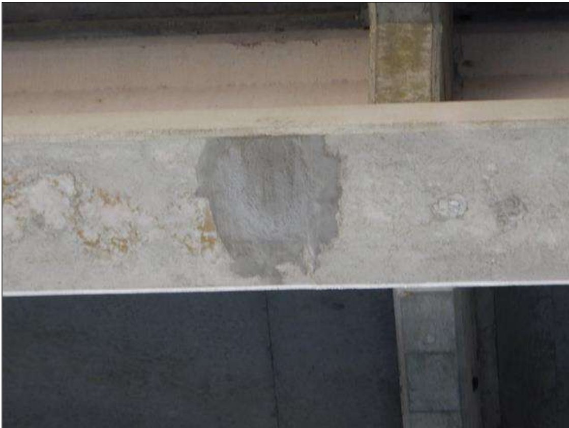
Span 28 Beam 3: [NEW REPAIR-PATCHING] FORMERLY --> multiple spalls with exposed rebar on the bottom face near mid span up to (9" x 4" x 1/2")
