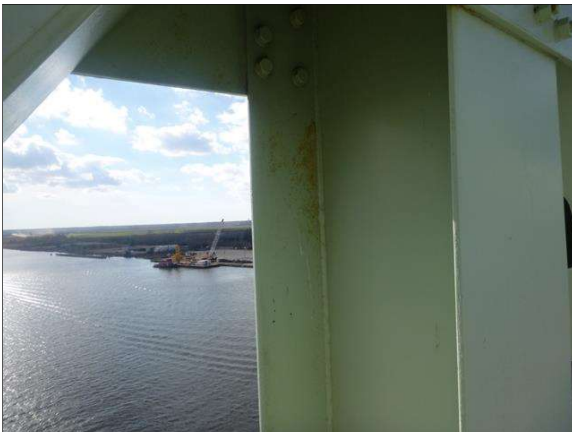
Span 18 Lift Span L9U9 SOUTH: SOUTH FLANGE EAST SIDE NEAR U8 FRECKLED RUST 18" X 6" AREA.
