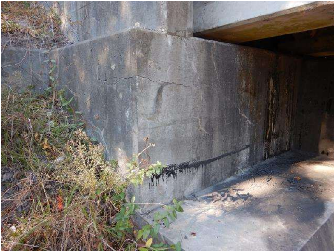
End Bent 1 Cap 1: horizontal cracking on the front and right faces up to (1/4") wide (2.5ft on each face)
