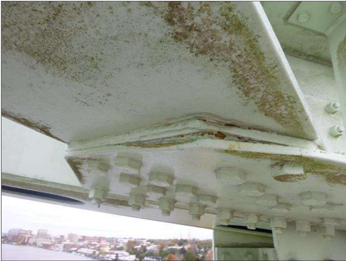
Span 18 Lift Span U10 NORTH: OUT OF PLANE BENDING 3/8" GAP TO BOTTOM OF GUSSET PLATE @ U10 NORTH SIDE.
