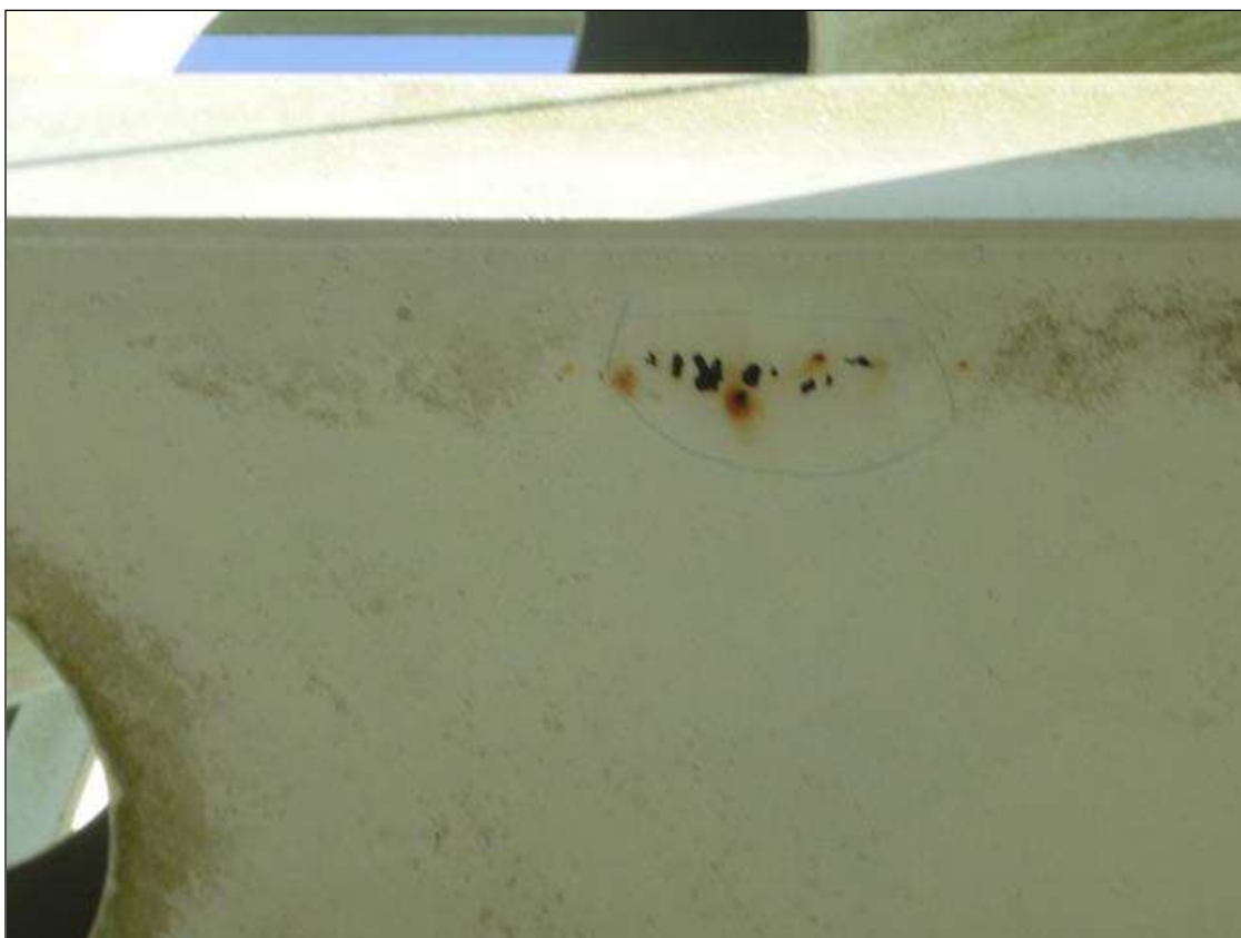
Span 17 WEST TOWER SOUTH: [PROMPT ACTION REQUEST] IN BOTTOM OF FIRST HORIZONTAL AT SOUTH EAST LEG CORROSION WITH HOLES UP TO 1/2" DIAMETER.
