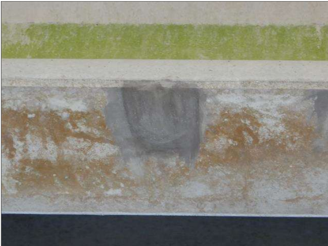
Span 28 Beam 5: [NEW REPAIR-PATCHING] FORMERLY --> spall with exposed steel on the bottom face at 24ft from bent 26 (12" x 5" x 1/2")
