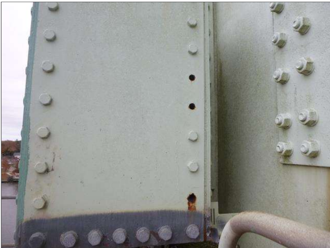
Span 18 Lift Span L0 NORTH: [PROMPT ACTION REQUEST] WHEEL GUIDE WEST PLATE 3 MISSING BOLTS WITH CORROSION AT BOLT HOLES.
