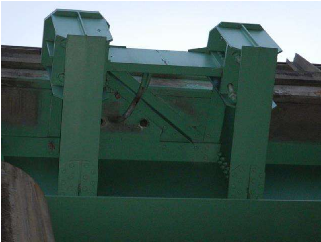
Span 26 Beam 1: [PROMPT ACTION REQUEST] West brace for removed overhead sign: southeastern bolt is loose and over the roadway (bolt could not be removed by hand), bolt has no top nut holding it in place.
