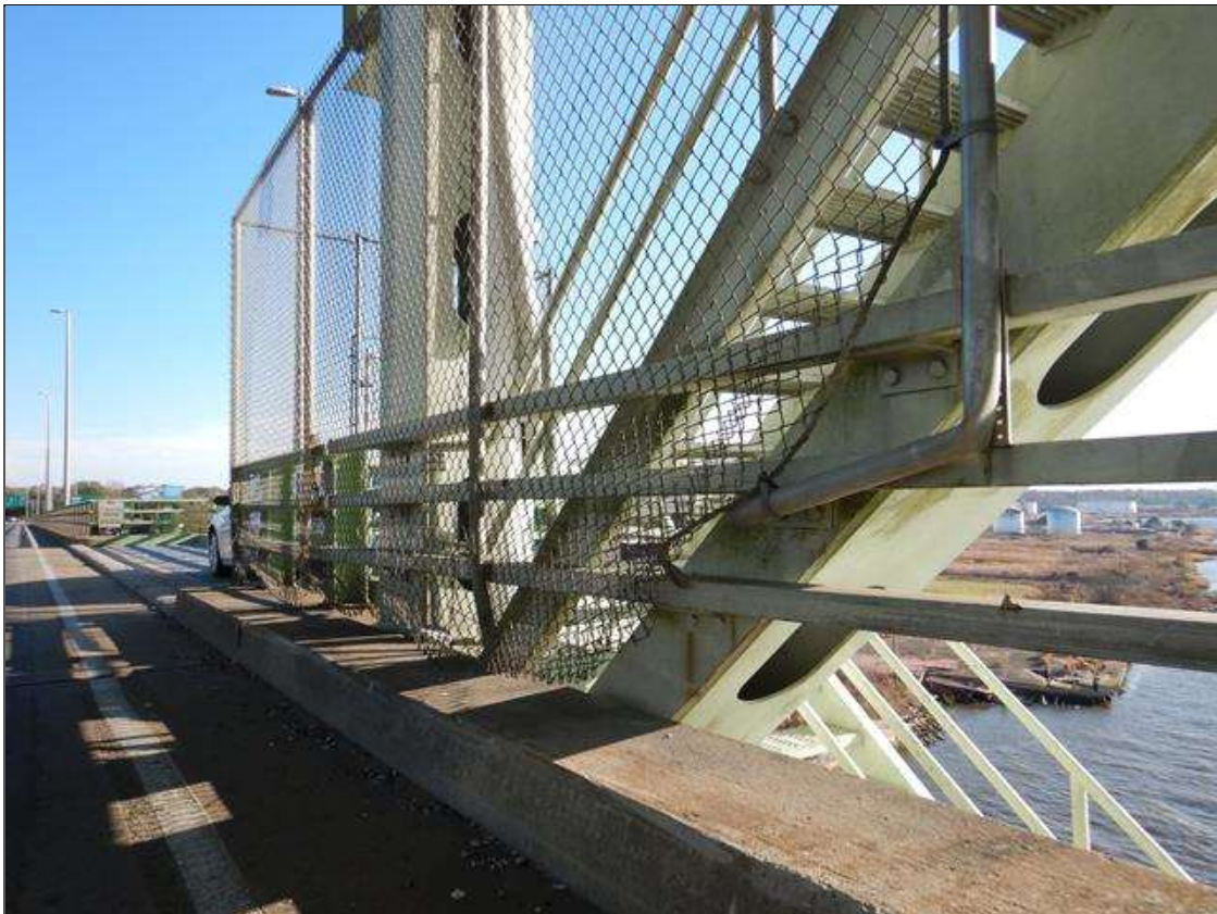
EAST TOWER AT THE RIGHT LANES, THERE IS IMPACT DAMAGE TO THE CHAIN LINK FENCING AT THE STAIRWAY [APPROXIMATELY 24' LONG]
