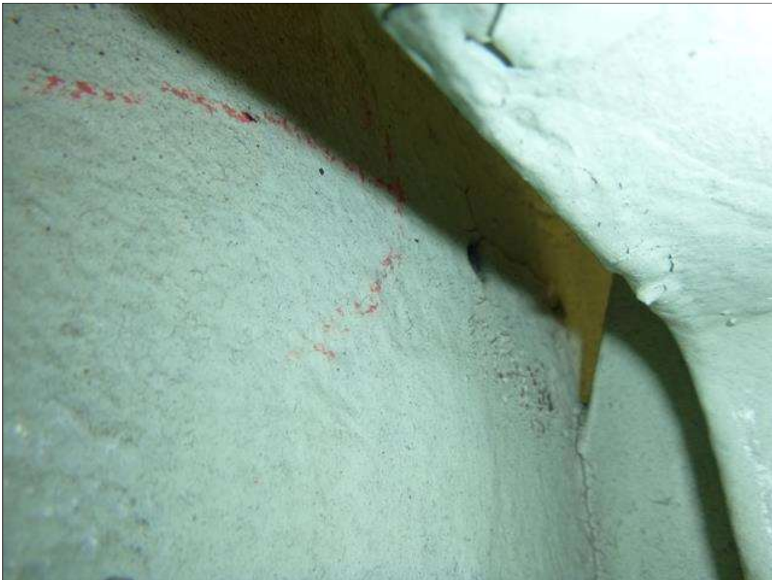
Span 18 Lift Span Stringer 7: OBSERVED IN 2020 INSP: BETWEEN FB's 6-7 - (1) CRACK PROPAGATED UP TO 1/4" PAST EAST ARREST HOLE, PAR ISSUED.
