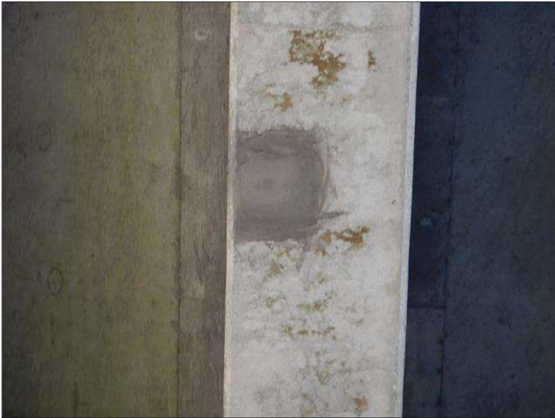
Span 27 Beam 2: [NEW REPAIR-PATCHING] FORMERLY --> DELAMINATION area on the bottom face at 10ft from bent 24 (4" x 2")
