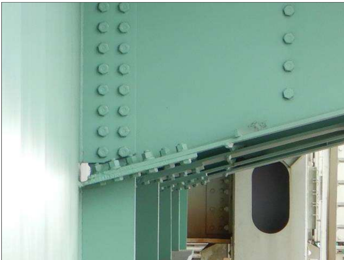
Span 16 Beam 8: [PROMPT ACTION REQUEST] Brace Beam 1 at EB Parking Area angle at bottom of railing, section loss on plate up to (1/16") into the angle and 100% section loss on (x2) nuts
