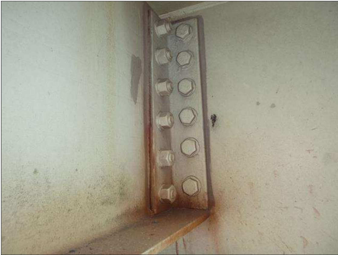
Span 18 Lift Span Stringer 9: BETWEEN FB's 9-10 - SLIGHT MOVEMENT UNDER LIVE LOAD AT FLOOR BEAM 10 - LOWER BOLTS AT STRINGER WEB CONNECTION ARE SECURE BUT NOT FULLY TIGHTENED - PROMPT ACTION REQUEST
