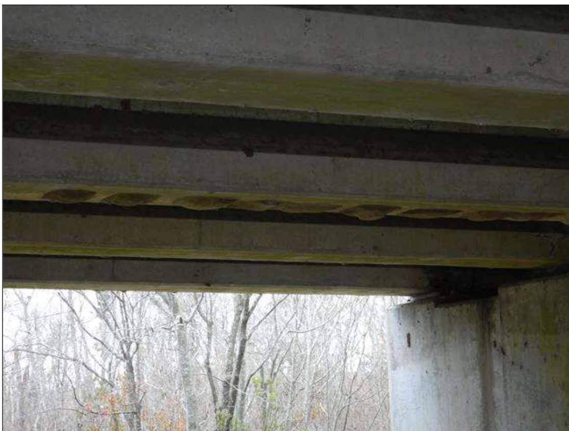
Span 2 Beam 7: [NEW REPAIR - PATCHING] FORMERLY --> 10ft section of 10 spalls with exposed rebar up to (6" x 6" x 1/2") on the bottom face starting 2ft from bent 1
