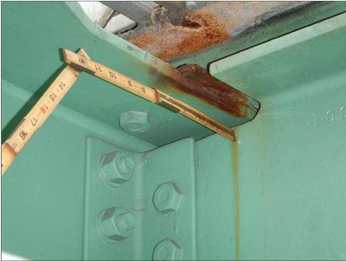
Span 16 Beam 1: [PROMPT ACTION REQUEST] BRACE BEAM 2 AT STRINGER 3 AT THE WESTBOUND PARKING AREA ON THE TOP FLANGE, SECTION LOSS [AVERAGE 1/2" REMAINING] IN A 2" X 2" AREA ON BOTH SIDES OF THE FLANGE.
