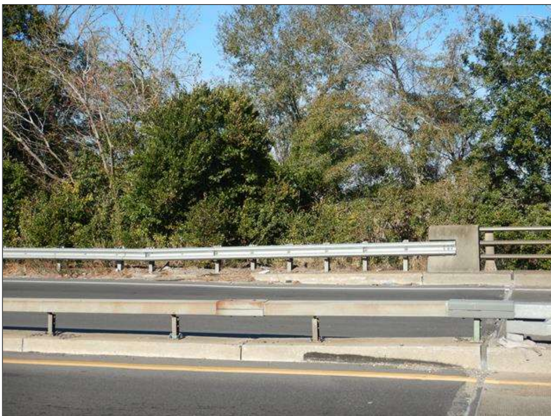
NORTHWEST CORNER, GUARDRAIL TRANSITION AND CONNECTION [SOUTHWEST CORNER SIMILAR]
