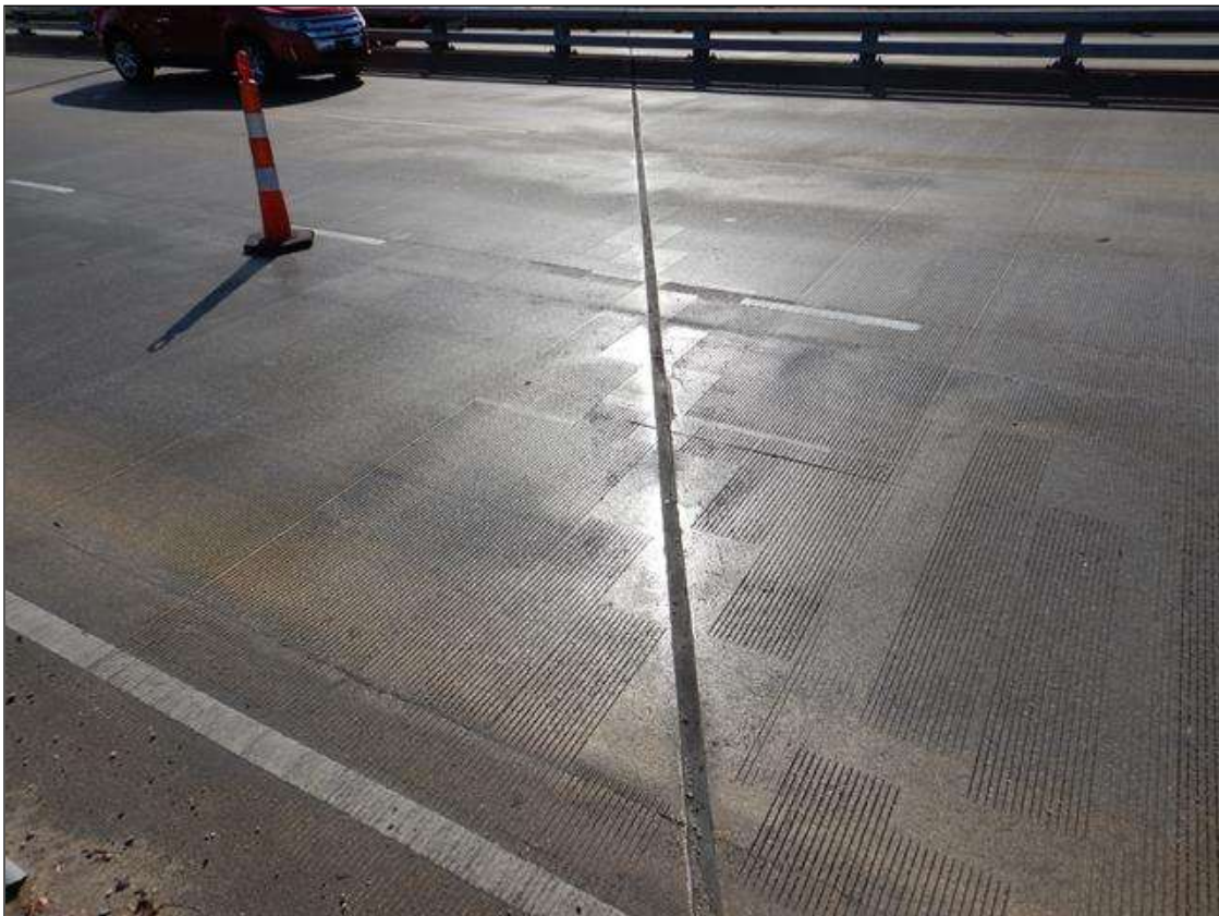
Span 31 Joint at Bent 28: LEFT LANES, THERE IS A TEAR IN THE TOP OF THE SEAL [APPROXIMATELY 2" DIAMETER]
