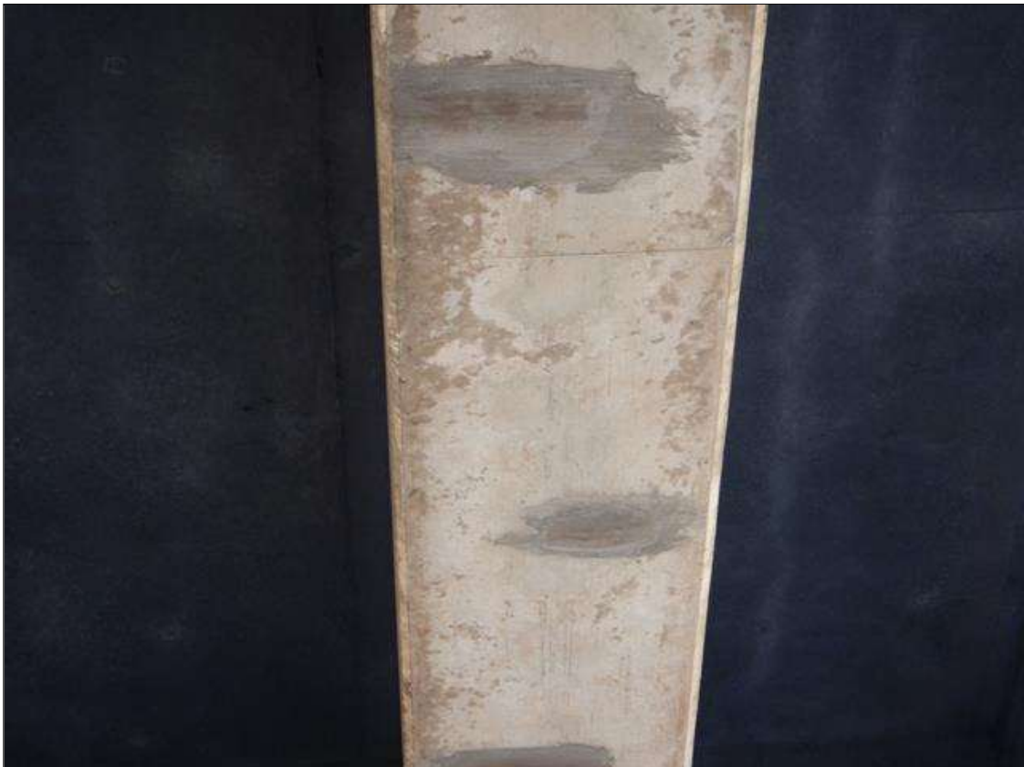
Span 31 Beam 2: [NEW REPAIR-PATCHING] FORMERLY --> (x2) spalls with exposed rebar on the bottom face at 14ft and 21ft from Bent 29 up to (10" x 4")
