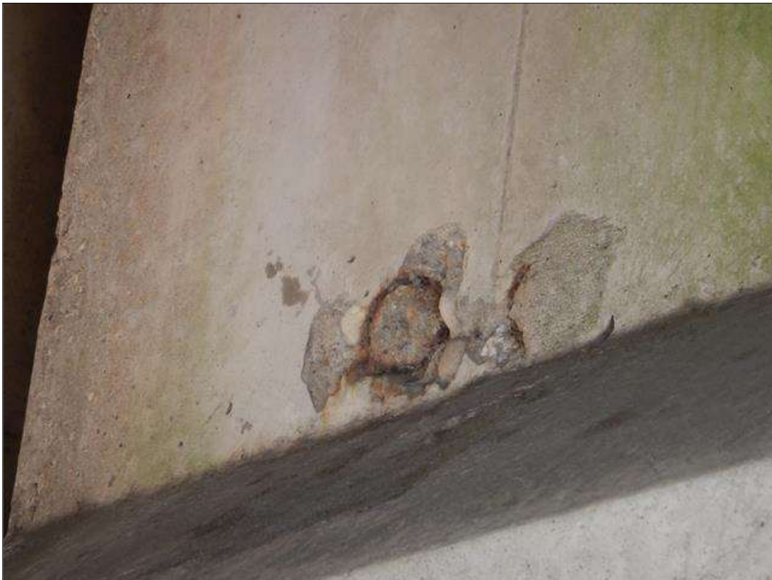
Span 31 Beam 7: [PROMPT ACTION REQUEST] spall with exposed rebar on the right web at 1ft from Bent 28 (7" x 3" x 1/2")
