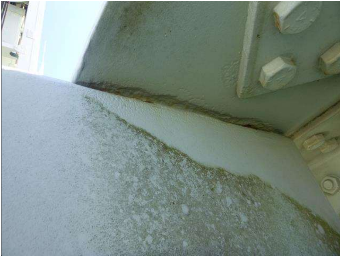
Span 18 Lift Span U11 SOUTH: BOTTOM OF TOP GUSSET PLATE AT LB11 EAST SIDE 15" X 1/2" AREA OF PITTING UP 1/16" DEEP.
