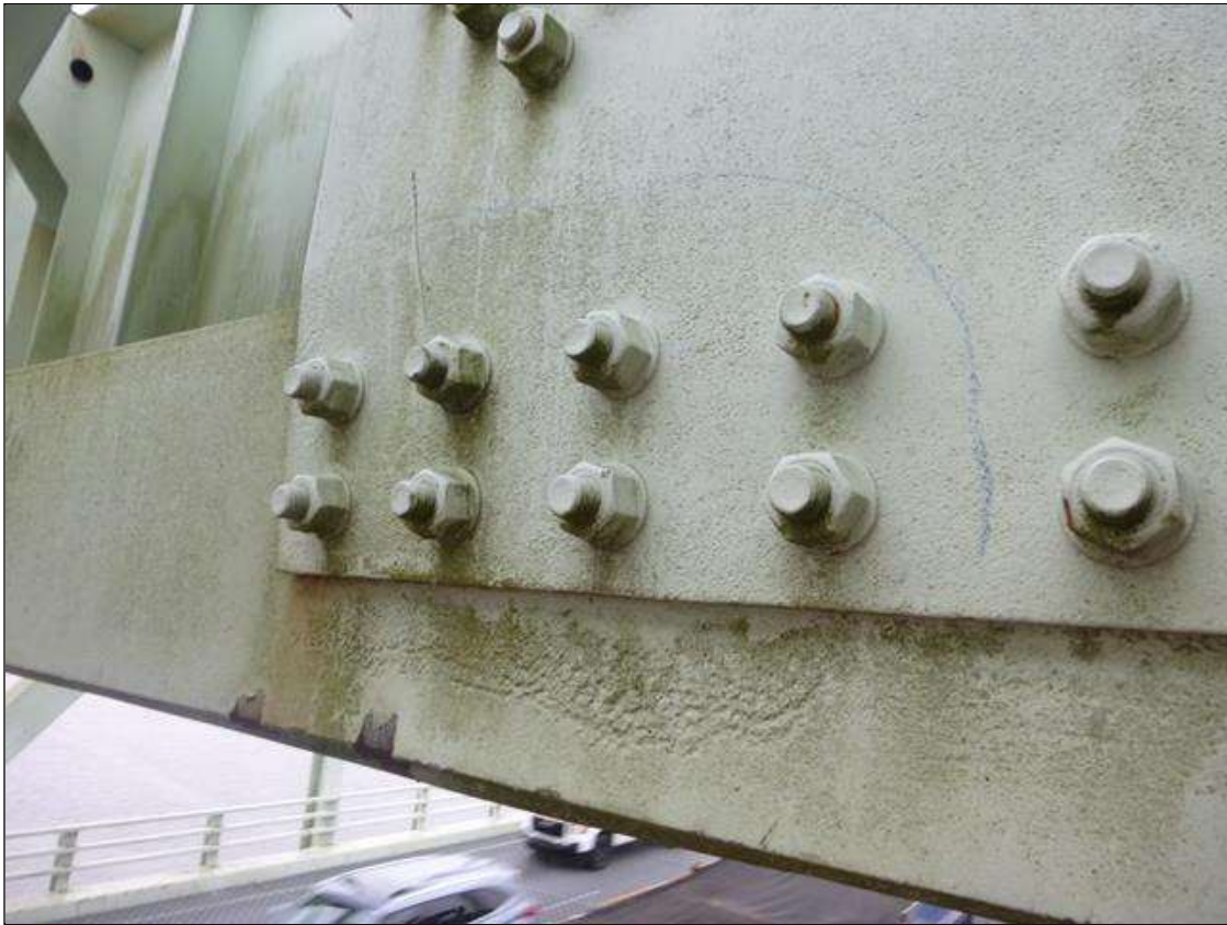
Span 19 EAST TOWER NORTH: 6/2020 - IMPACT DAMAGE - BOTTOM WEST HORIZONTAL TRUSS MEMBER - DIAGONAL CONNECTION GUSSET PLATE - 18"LONG x 8"HIGH SECTION AT BOTTOM SOUTH CORNER BENT 1/2" TO THE WEST - LOCATED AT 11'-3" FROM NORTHWEST TOWER LEG (PAR)
