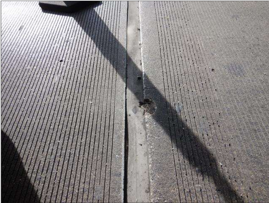
Span 20 Joint at Bent 17: SCATTERED ALONG THE LENGTH, SCATTERED EDGE CHIPPING IN THE ADJACENT DECK HEADERS UP TO 3" WIDE X 1" DEEP
