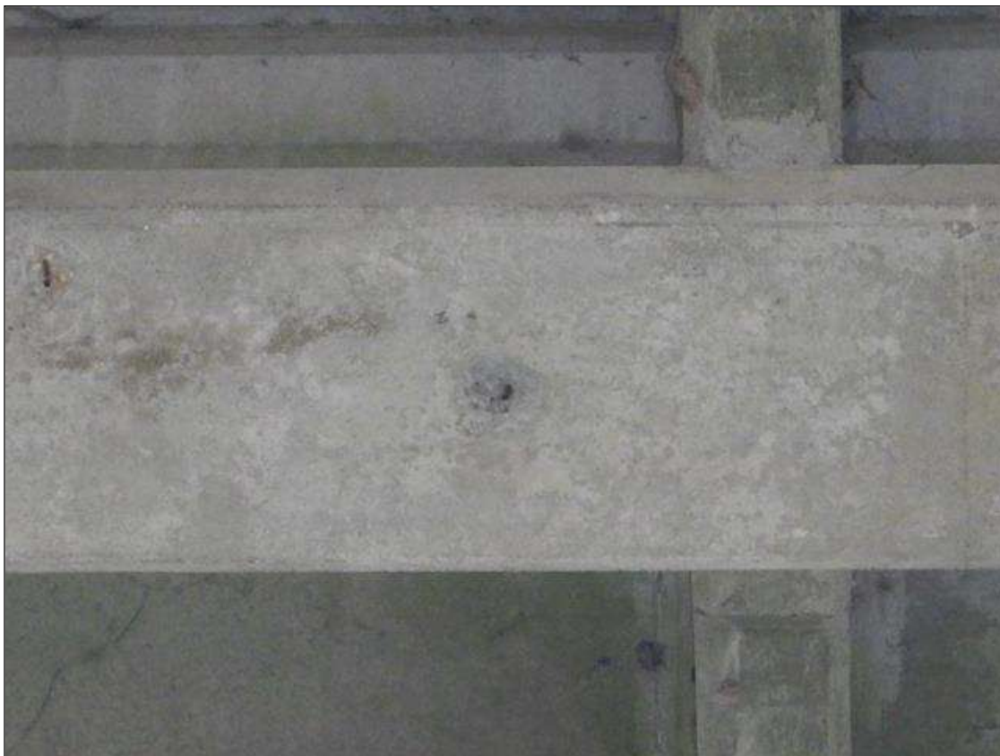
Span 6 Beam 8: spall on the bottom face, 20 FOOT. from bent 6 cap, 2" in diameter x 1/4" deep with exposed rebar
