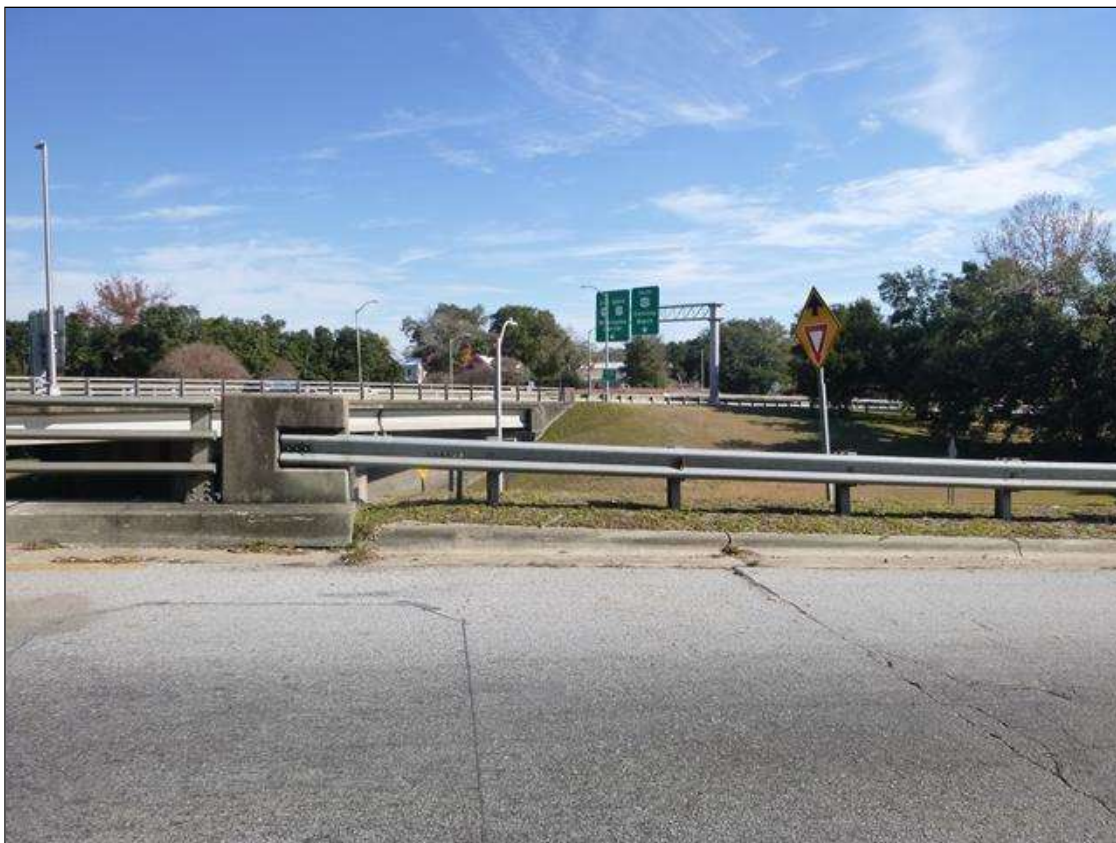
RAMP ABUTMENT NORTHEAST CORNER, GUARDRAIL TRANSITION AND CONNECTION [RAMP ABUTMENT SOUTHEAST CORNER SIMILAR]
