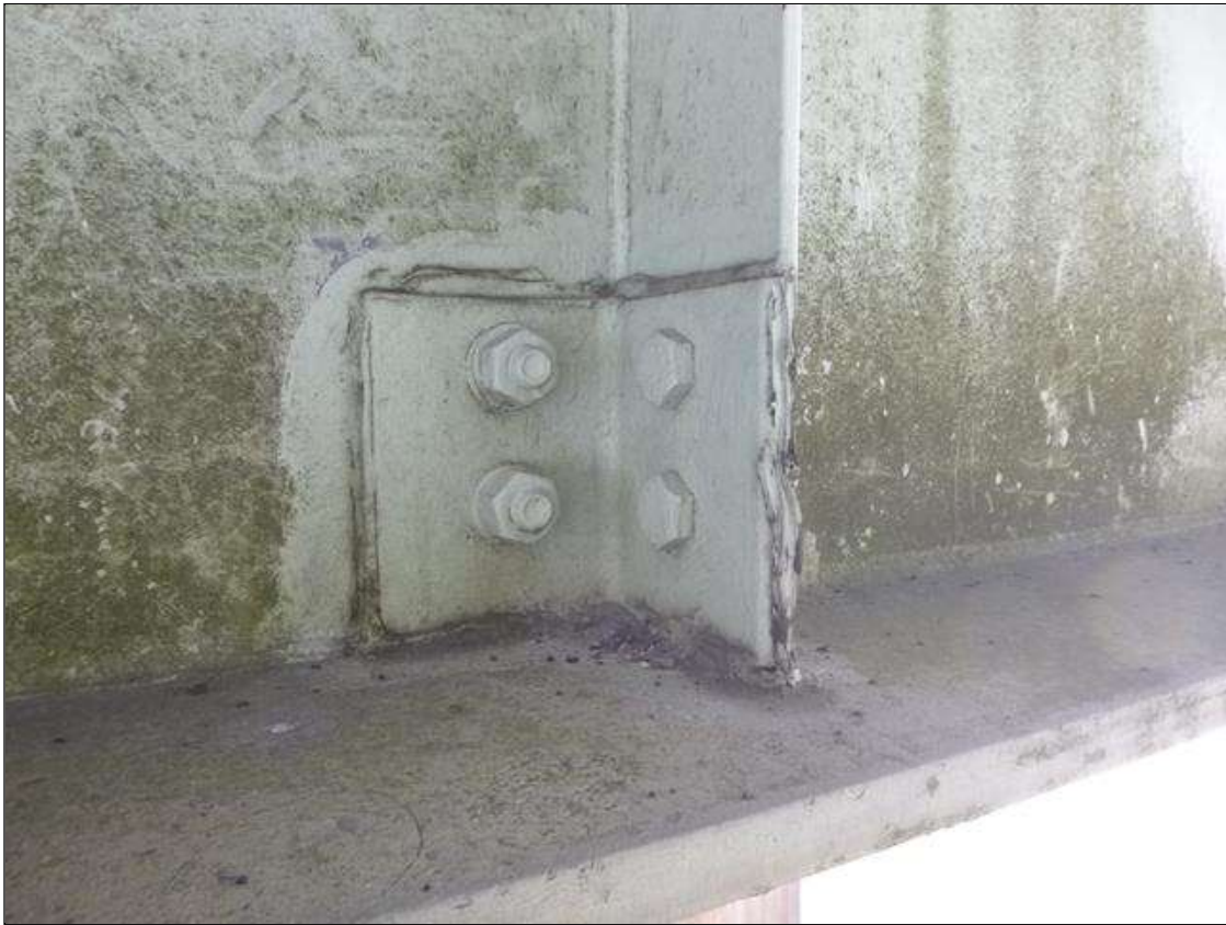
Span 18 Lift Span Floor Beam 11: FB 11, WEST SIDE, STIFFENER 11 HAS BEEN REPAIRED ADJACENT TO THE BOTTOM FLANGE, WITH A 6" X 6" X 7" HIGH X 1/2" THICK ANGLE BOLTED TO THE STIFFENER AND WEB ON THE NORTH SIDE EAST AND WEST FACES. 2018 REPORT HAD 3" LONG x 1" HIGH PITTED AREA IN WEB WIDE/ 1/4" DIAMETER HOLE - AT BOTTOM FLANGE ADJACENT TO VERTICAL STIFFENER 11 - AREA CLEANED AND PAINTED - PROMPT ACTION REQUEST.
