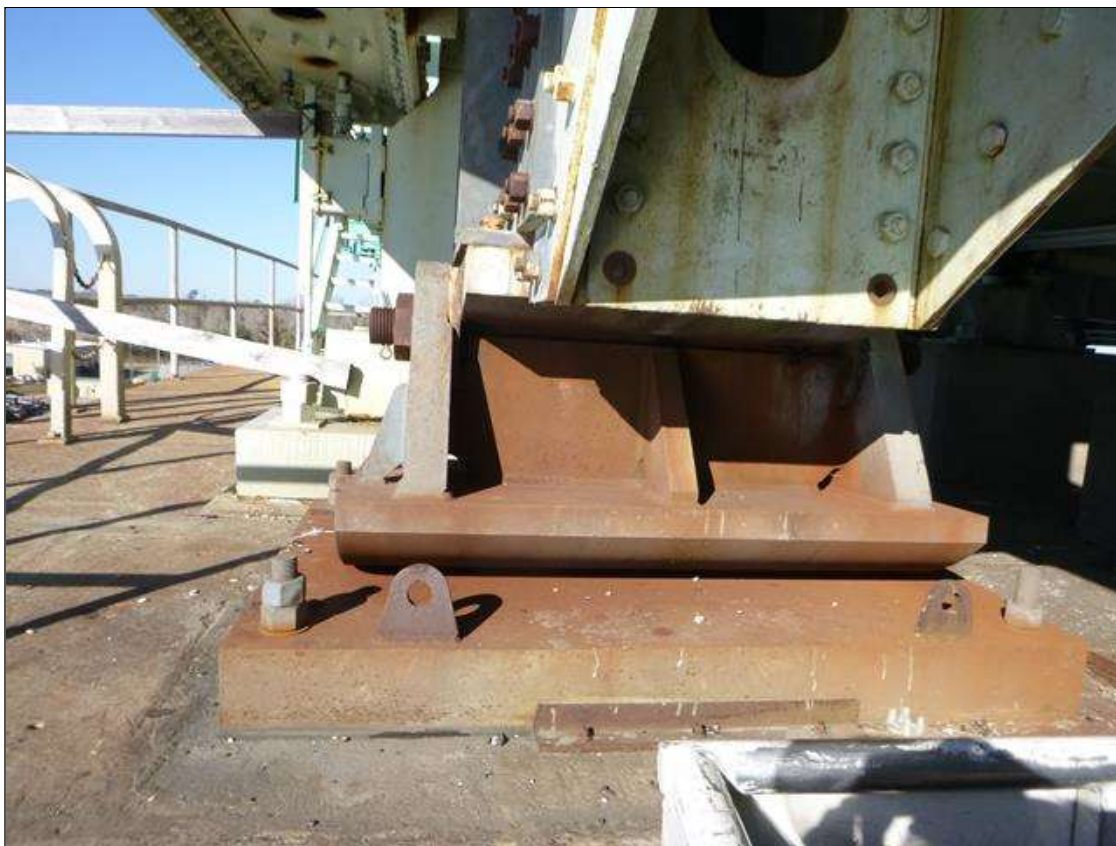
SOUTH TRUSS BEARING AT BENT 16, NORTH TRUSS BEARING SIMILAR
