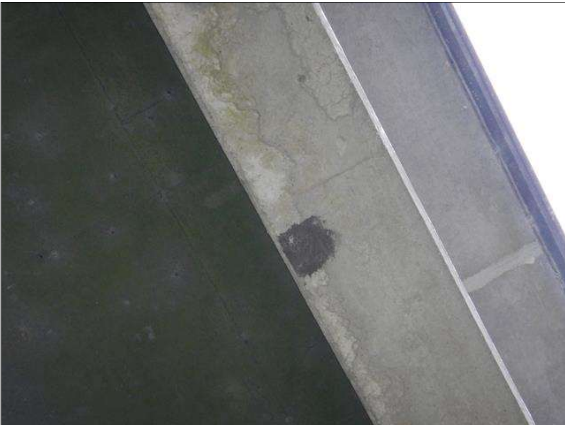
Span 4 Beam 1: [NEW REPAIR - PATCHING] FORMERLY --> (4" x 3" x 1/4") spall with exposed rebar on the bottom face at 13ft from bent 4
