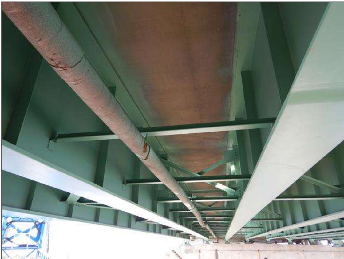
SPAN 20 BAY 6, A 3" INSULATED STEEL PIPE HANGS FROM STEEL SUPPORTS, FULL SPAN LENGTH
