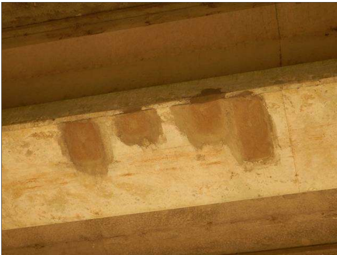
Span 30 Beam 9: [NEW REPAIR-PATCHING] FORMERLY --> (x4) spalls with exposed rebar on the bottom face starting at 30ft from bent 27 up to (13" x 3" x 1/4")
