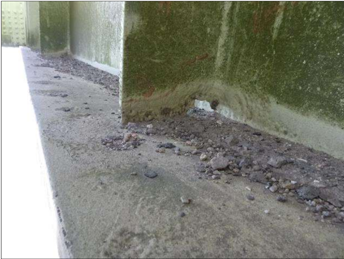
Span 18 Lift Span Floor Beam 10: OBSERVED IN 2020 INSP: VERTICAL STIFFENER 11 EAST SIDE - 4" HIGH PITTED AREA AT BOTTOM FLANGE WIDE/ 1-1/2" DIAMETER HOLE AT WEB - 1/16" TO 1/8" REMAINING SECTION IN LOWER 1" OF AREA, PAR ISSUED.
