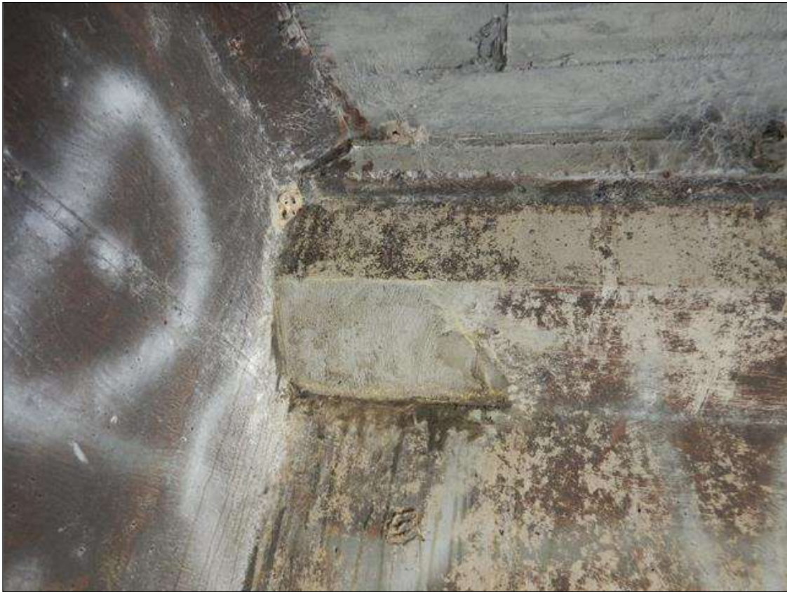
Span 35 - Ramp Span Beam 2: [NEW REPAIR-PATCHING] FORMERLY --> spall with exposed rebar in the top left flange at Ramp End Bent (7" x 1 1/2" x 1/4")
