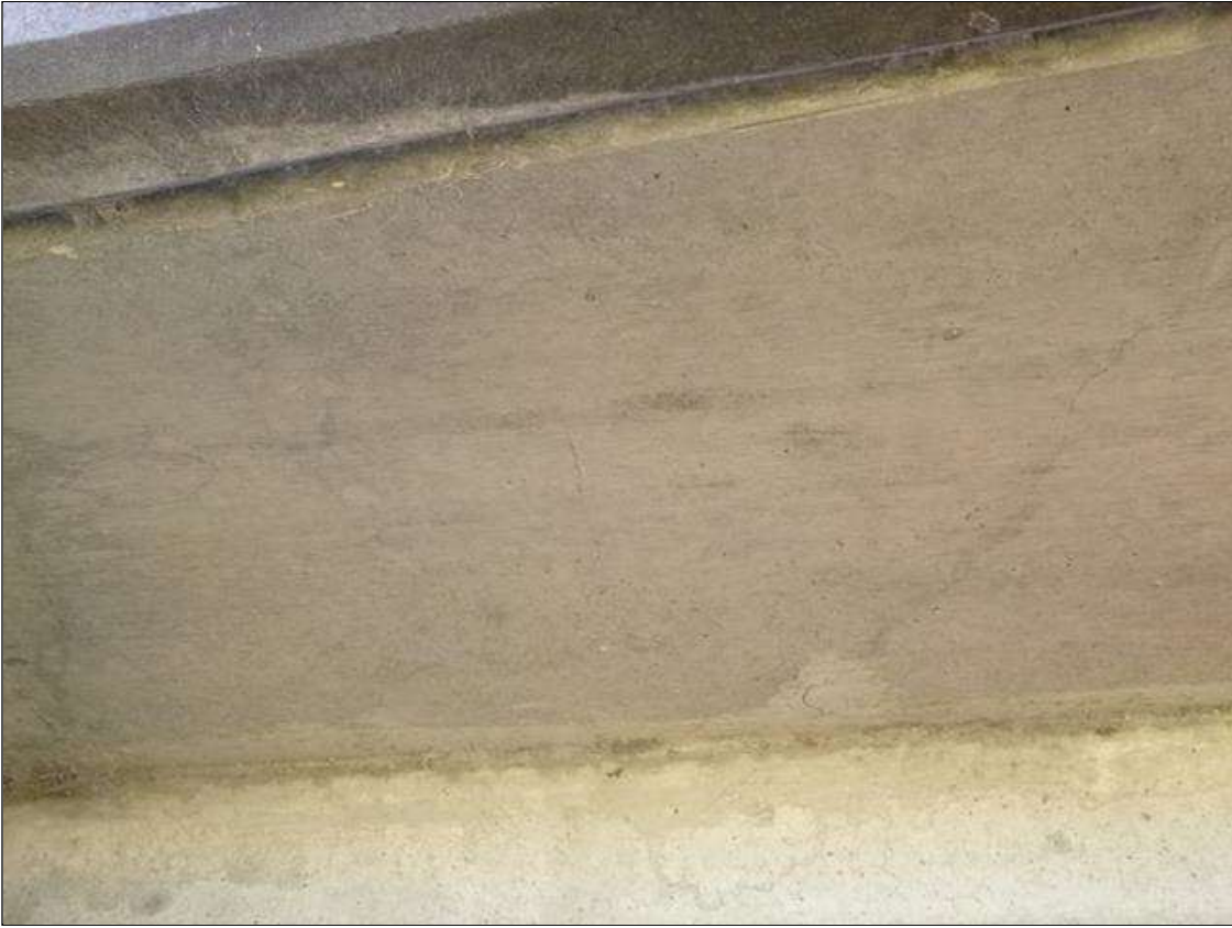
Span 35 - Ramp Span Deck: [NEW REPAIR - PATCHING] FORMERLY --> spall with exposed rebar on the left overhang at Ramp End Bent (20" x 24" x 6")
