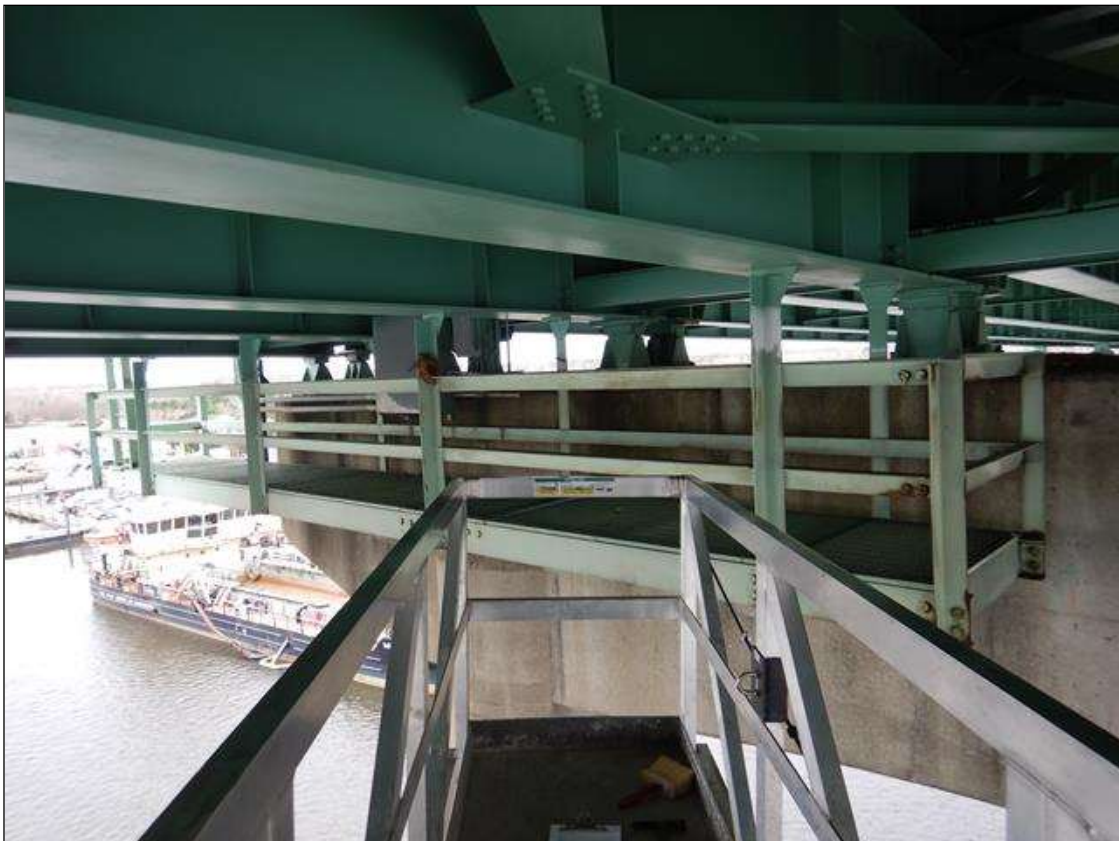
SPAN 20, A STEEL CATWALK [APPROXIMATELY 30' LONG X 50" WIDE X 46" HIGH] HANGS FROM GIRDERS 1-4 ADJACENT TO BENT 18. A SIMILAR CATWALK HANGS FROM SPAN 16 GIRDERS 5-8 ADJACENT TO BENT 15.
