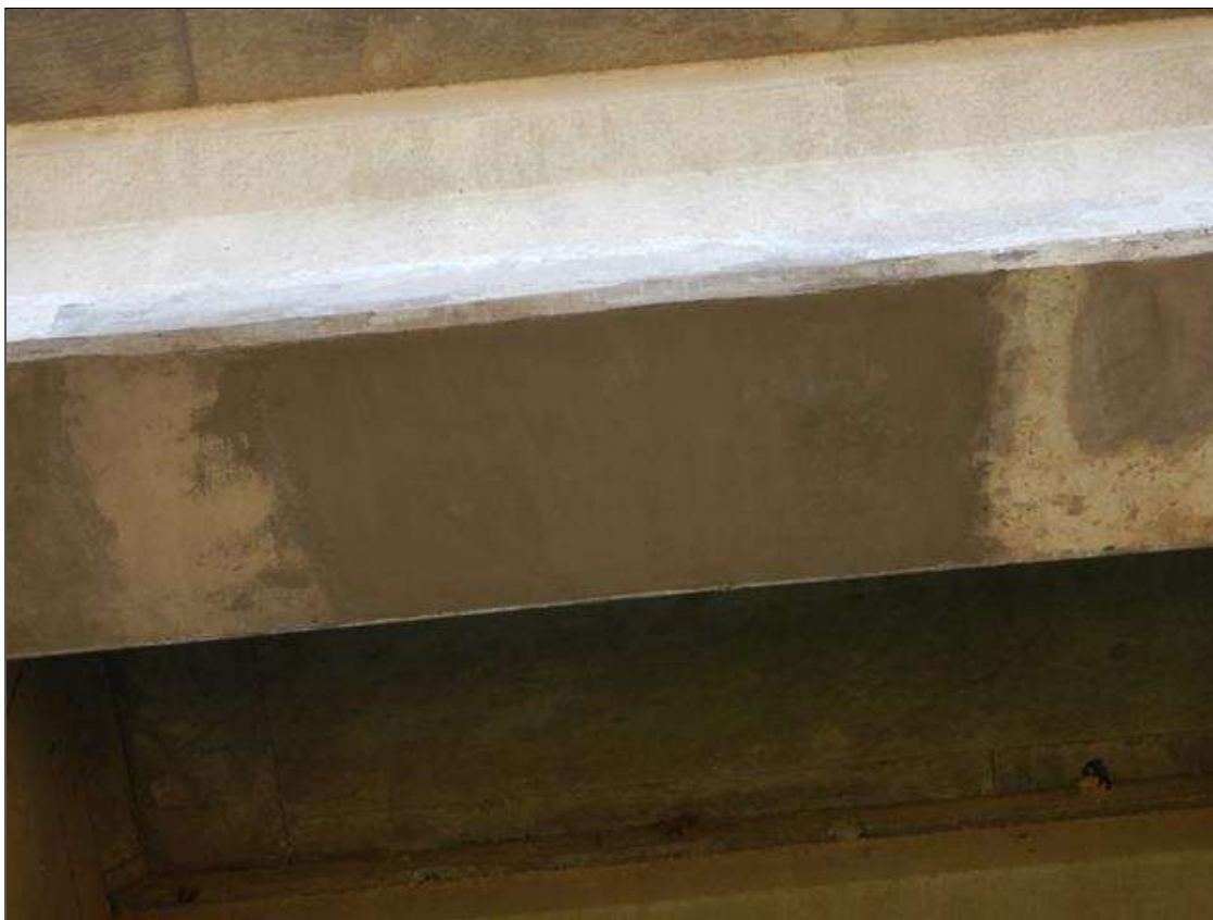
Span 34 - Ramp Span Beam 1: [NEW REPAIR-PATCHING] FORMERLY --> spall with exposed rebar (45" x 7" x 2") and (1) exposed strand 16ft from Bent 30, strand exposed for (24") long, active corrosion with section loss less than (1/16") on strand
