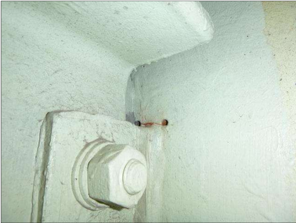
Span 18 Lift Span Stringer 11: (PAR) BETWEEN FB's 10-11 - TOTAL OF (5) 1/16" TO 1/8" CRACKS PROPAGATING PAST ARREST HOLES AT TOP OF DIAPHRAGM CONNECTION
