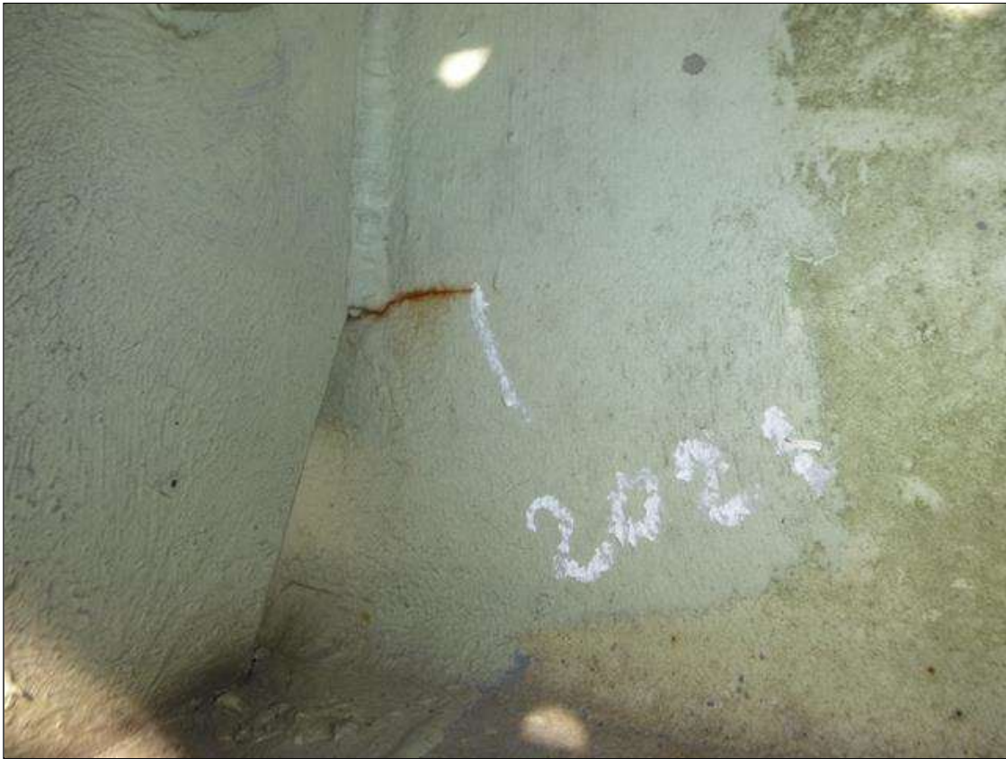
Span 18 Lift Span Stringer 13: (PAR) BETWEEN FB's 2-3 - 1 1/4" LONG CRACK IN WEB ACROSS BOTTOM OF WELD AT DIAPHRAGM CONNECTION ON SOUTH SIDE.
