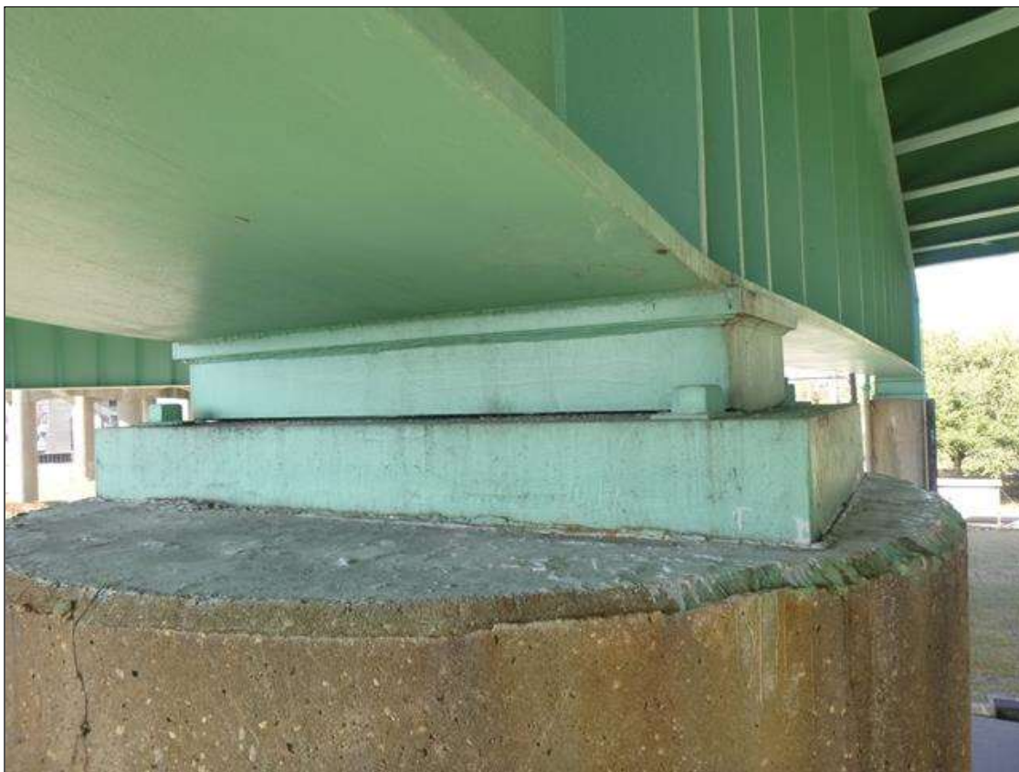
BENT 23 RIGHT END FIXED BEARING [BENT 22 LEFT END SIMILAR]
