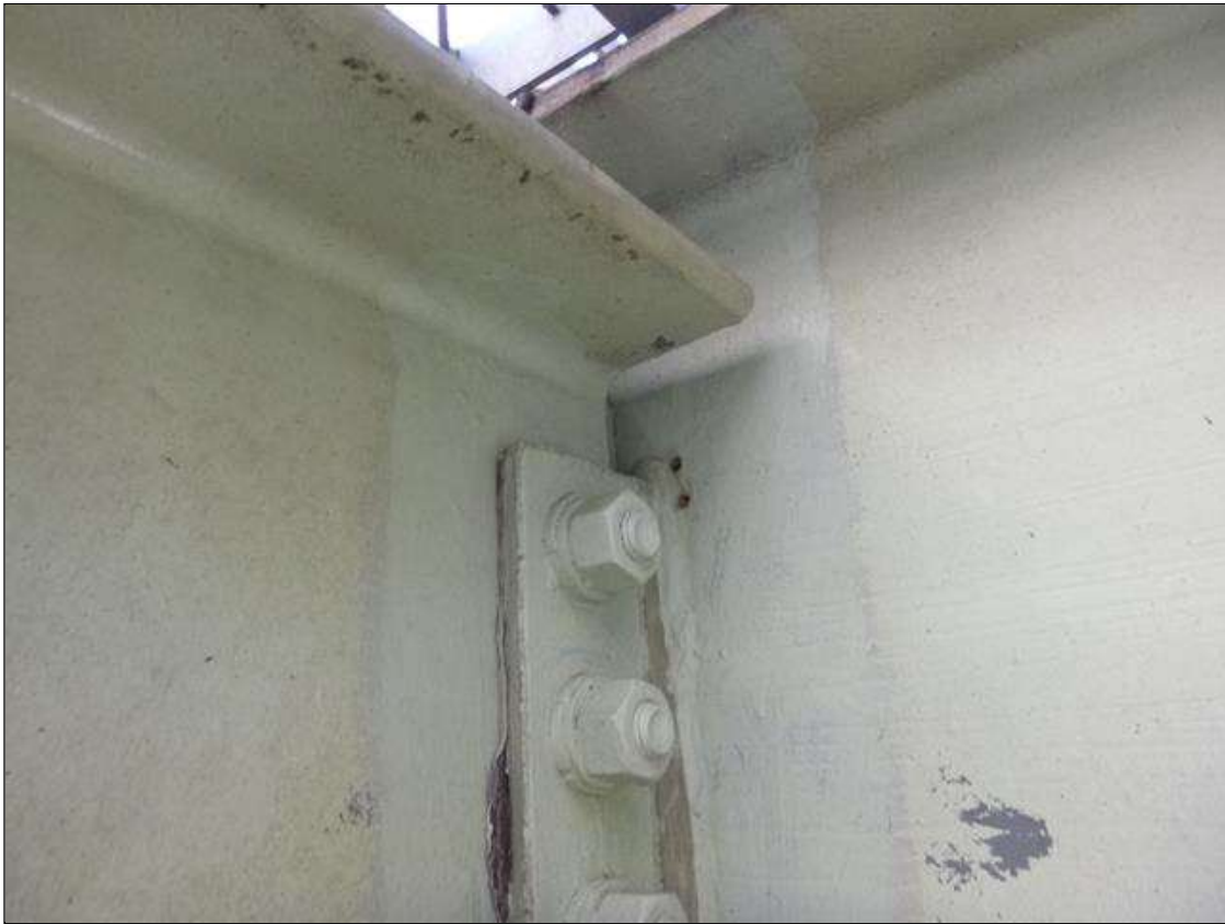
Span 18 Lift Span Stringer 11: BETWEEN FB's 5-6 - ARRESTED CRACK IN WEB AT TOP OF DIAPHRAGM CONNECTION
