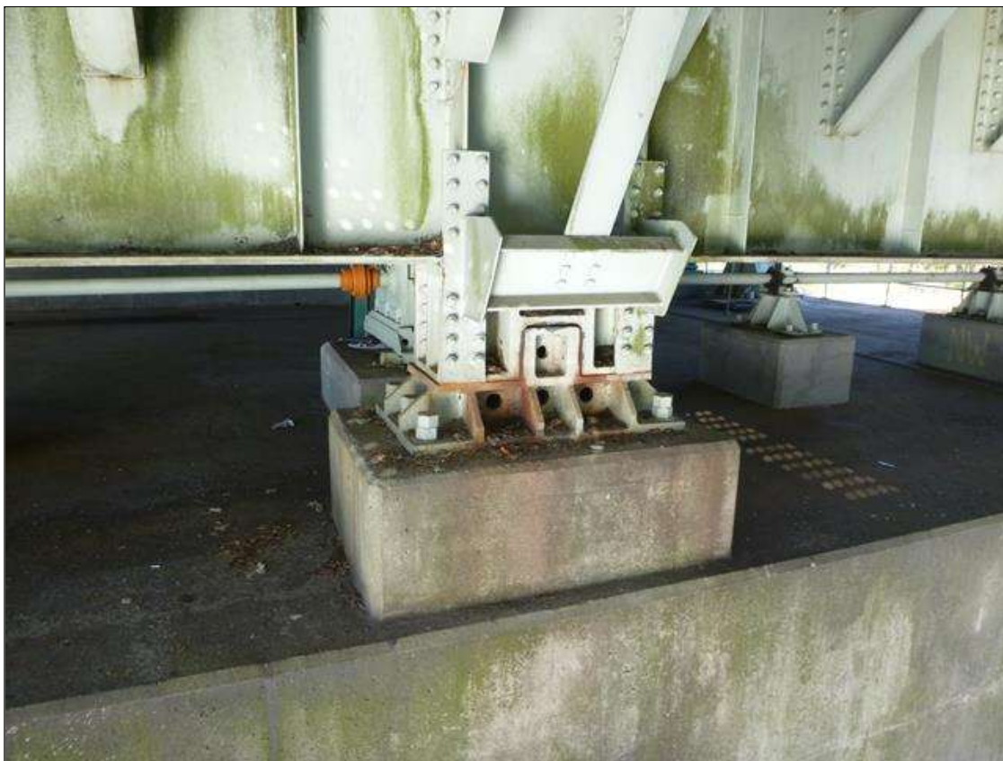
BRIDGE GUIDE AT FLOORBEAM 0
