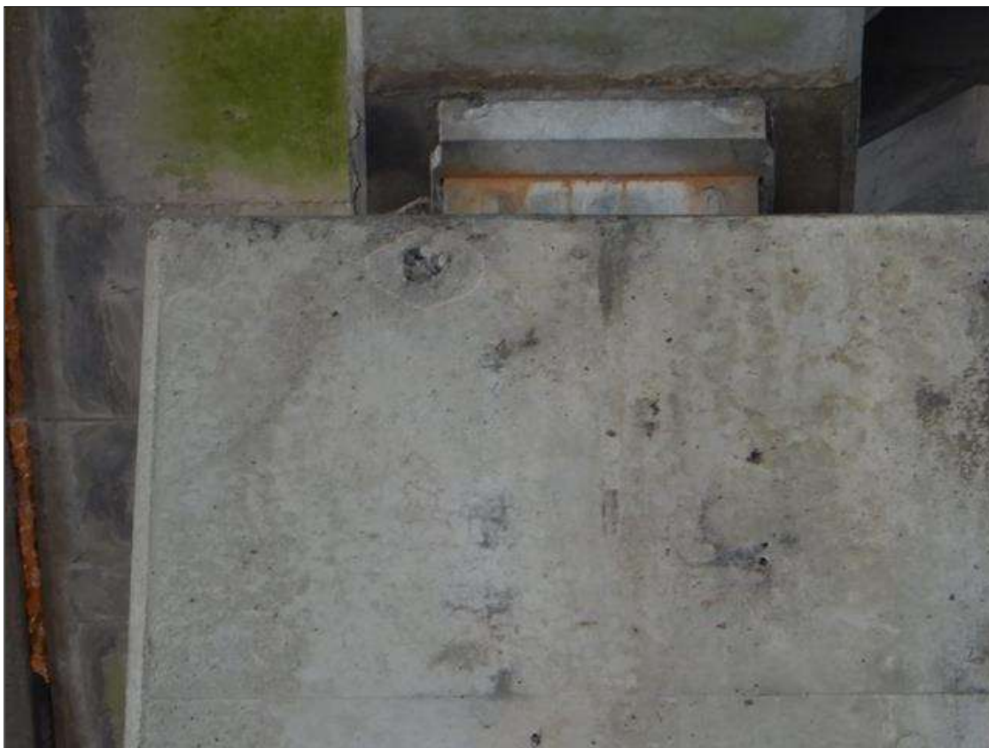
Bent 26 Cap 1: (2 1/4" x 1 1/4" x 2" deep) spall on the east face under girder 6 near top edge
