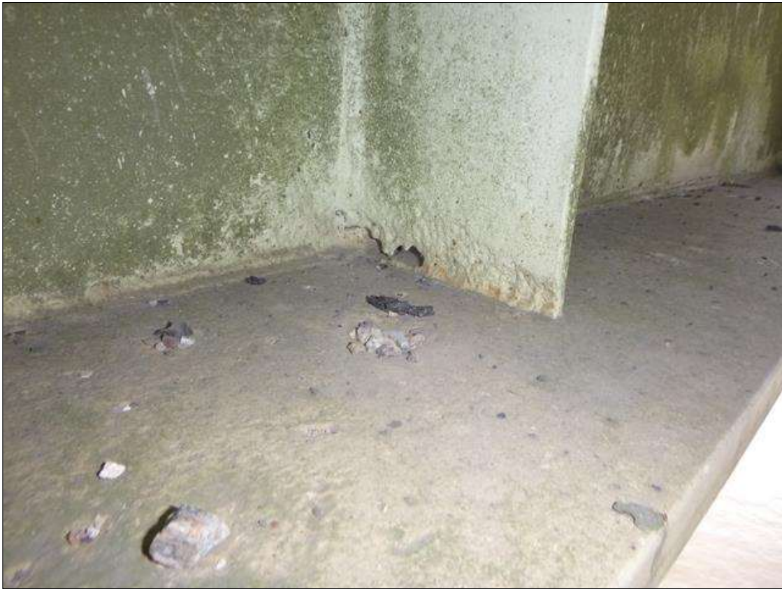
Span 18 Lift Span Floor Beam 11: VERTICAL STIFFENER 12 WEST - PITTED AREA AT BOTTOM FLANGE OF FLOOR BEAM UP TO 3" HIGH WIDE/ 2" LONG x 1/2" HIGH HOLE AT WEB - 1/16" TO 1/8" REMAINING SECTION IN LOWER 1/2" OF AREA - CLEANED AND PAINTED - PROMPT ACTION REQUEST
