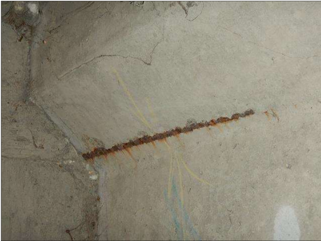
Span 35 - Ramp Span Beam 5: [PROMPT ACTION REQUEST] spall with exposed steel on the top left flange at the Ramp End Bent (13" x 1" x 1/4")
