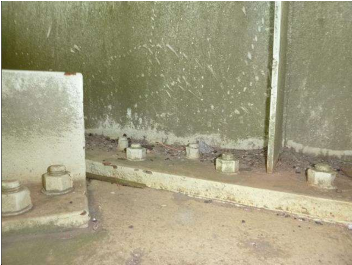
Span 18 Lift Span Floor Beam 5: 50-80% LOSS TO (5) CENTER BOTTOM LATERAL GUSSET FASTENERS AT BOTTOM FLANGE ON WEST SIDE
