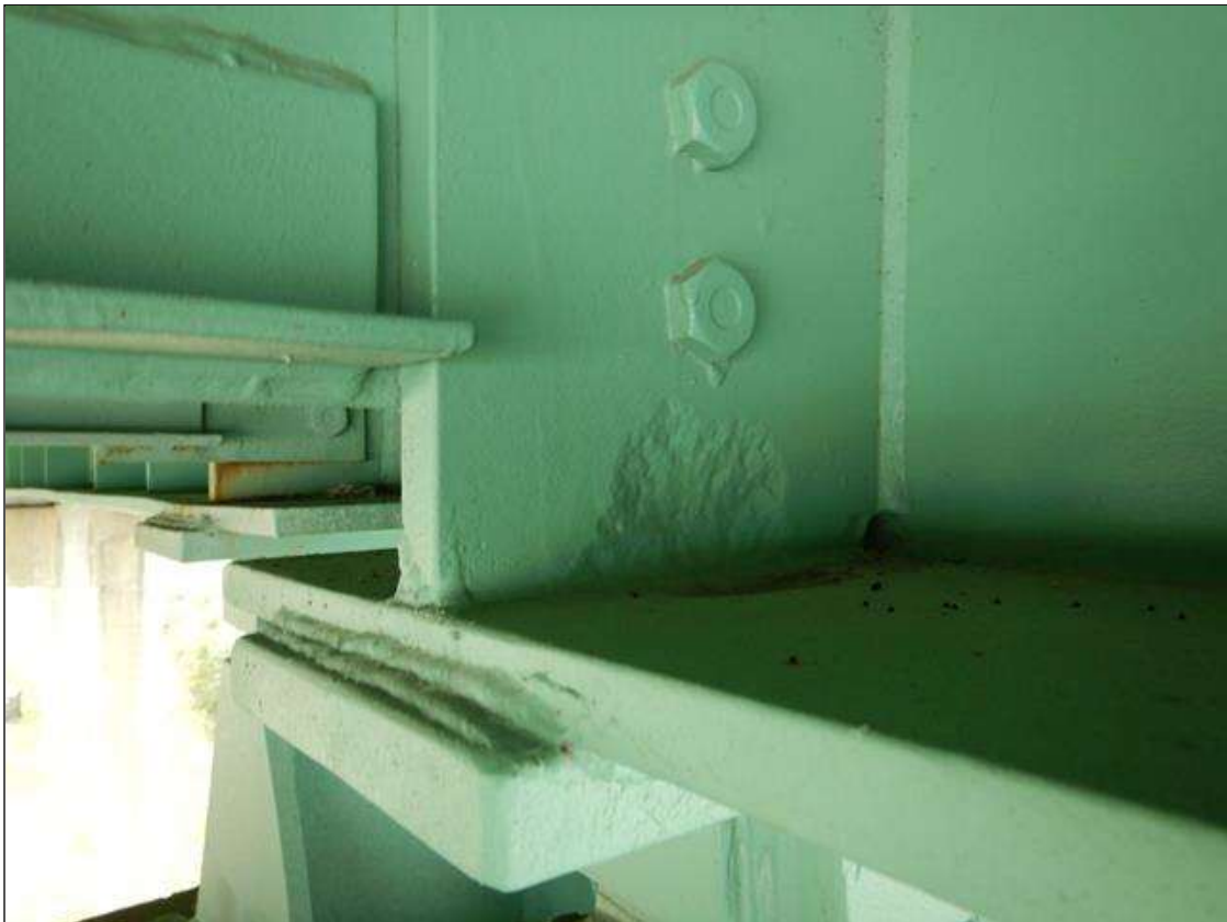
Span 12 Beam 4: Section loss on the bottom right web stiffener at bent 12 (6" x 5") by less than (1/16") into the stiffener and greater than 75% section loss on bottom gusset connection nut
