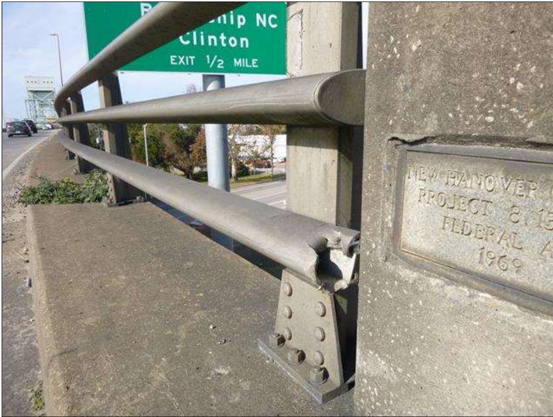
Span 32 Left Bridge Rail: damage to the bottom rail at End Bent 2
