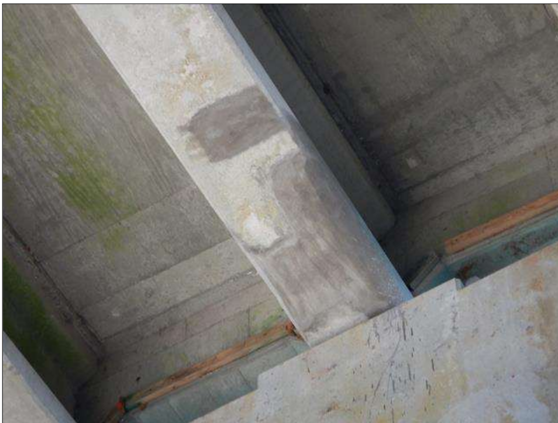
Span 27 Beam 6: [NEW REPAIR-PATCHING] FORMERLY --> spall with exposed rebar (32" x 22" x 3") and (1) exposed strand on the bottom and left faces at Bent 24, strand exposed for (20") long, active corrosion with no measureable section loss on strand
