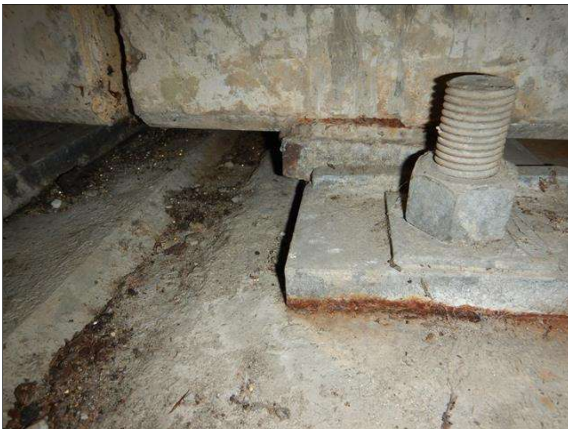
Span 1 Beam 5 - Beam 5 Far Bearing: Up to (1/2") movement of bearing to east beyond masonry plate with 8% loss in bearing
