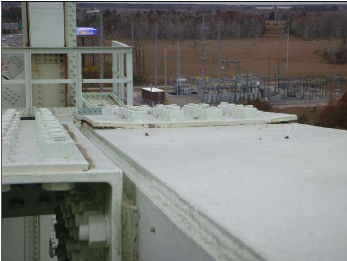
Span 18 Lift Span U1 NORTH: TOP GUSSET CONNECTION HAS 1/4" OUT OF PLANE BENDING WITH PACK RUST BETWEEN PLATES.
