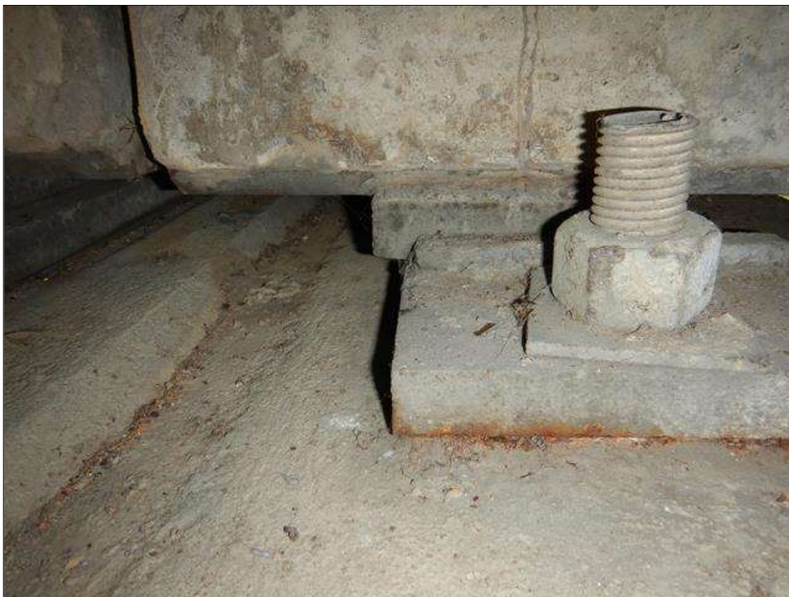
Span 1 Beam 4 - Beam 4 Far Bearing: Up to (1/2") movement of bearing to east beyond masonry plate with 8% loss in bearing
