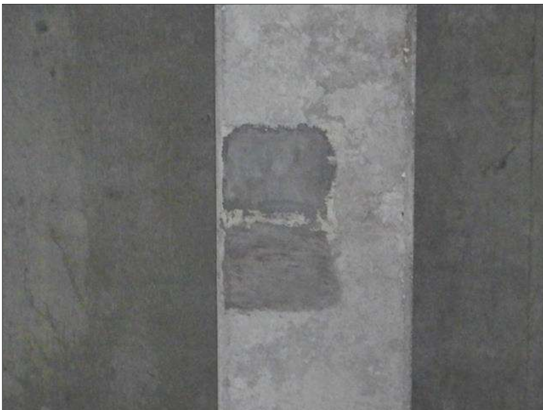
Span 8 Beam 2: [NEW REPAIR - PATCHING] FORMERLY --> (9" x 7" x 1/2") spall with exposed rebar on the bottom face at 13ft from bent 8
