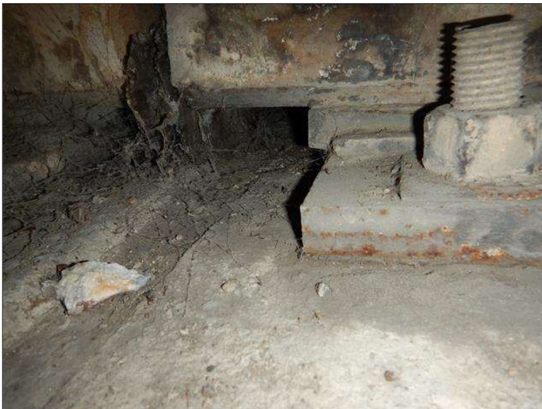
Span 1 Beam 7 - Beam 7 Far Bearing: Up to (1/2") movement of bearing to east beyond masonry plate with 8% loss of bearing
