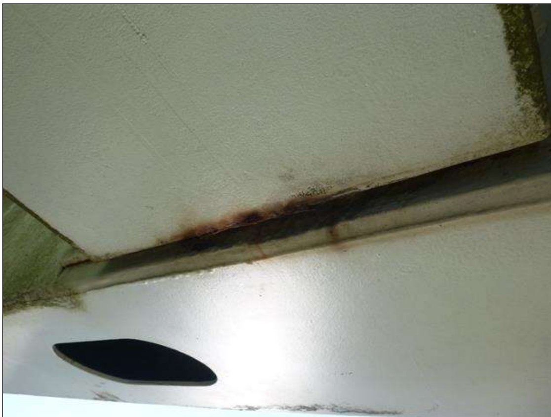
PITTED AREA UP TO 2"W x 5/16"D ACROSS BOTTOM OF BOTTOM FLANGE AT L1 SOUTH LATERAL GUSSET CONNECTION
