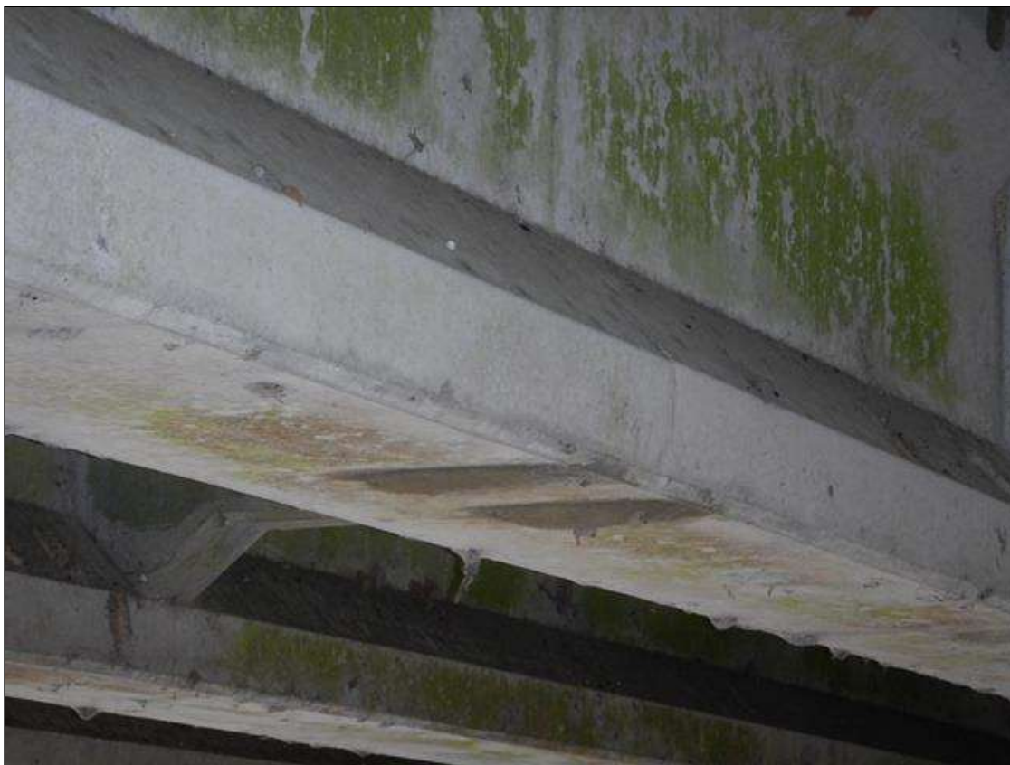
Span 1 Beam 7: spall with exposed rebar on the bottom face at 28ft from bent 1 (7 1/2" x 4 1/2" x 1/8")
