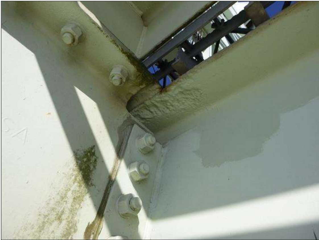
Span 18 Lift Span Stringer 14: BETWEEN FB's 0-1 - AREAS ALONG EDGES OF TOP FLANGE UP TO 8" LONG x 2" WIDE / 5/16" REMAINING - CLEANED AND PAINTED
