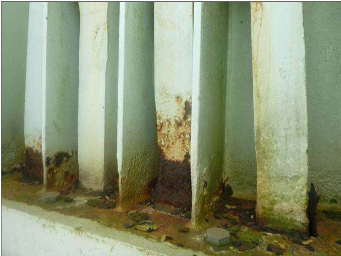
WEST TOWER: NORTHWEST CABLE BANK EAST BOUND LANE, LOSS OF SECTION .258" WITH 3.49" REMAINING
