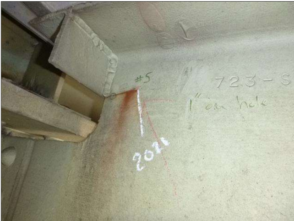
Span 18 Lift Span Stringer 12: LONGITUDINAL CRACK, 2.5" LONG IN THE TOP OF THE WEB AT FB 12, PAR ISSUED.
