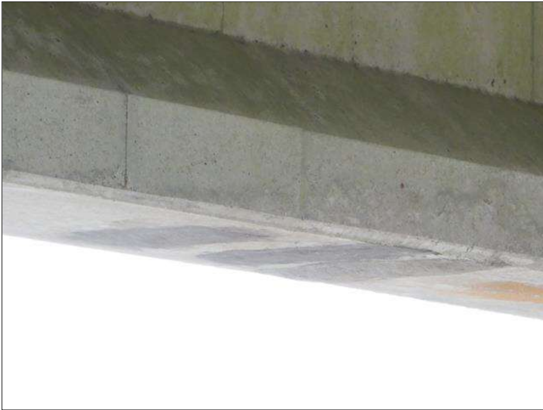
Span 11 Beam 9: [NEW REPAIR - PATCHING] FORMERLY --> (x6) spalls in a 2ft section up to (7" 1/2" x 2 1/2" x 1/4") at 14ft from bent 10
