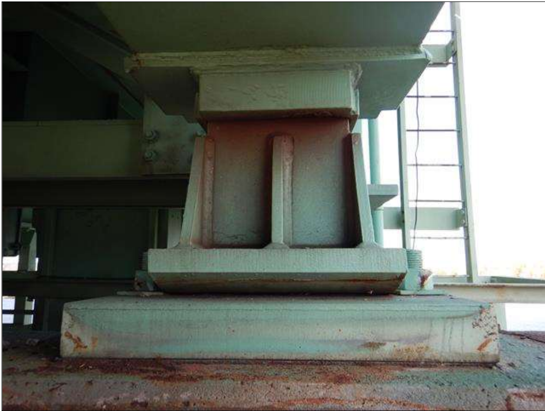
Span 21 Beam 1 - Beam 1 Near Bearing: SCATTERED SURFACE CORROSION
