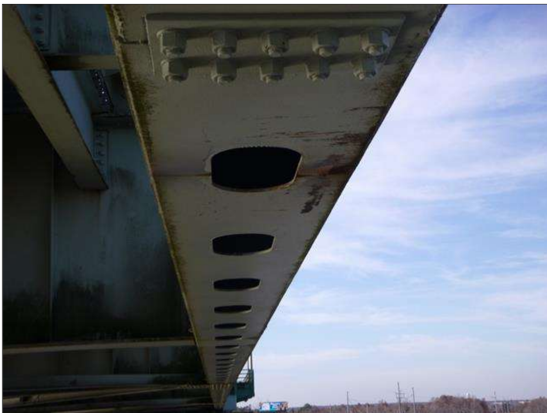
Span 18 Lift Span L5L6 NORTH: IN BOTTOM AT MID-LENGTH SURFACE RUST.
