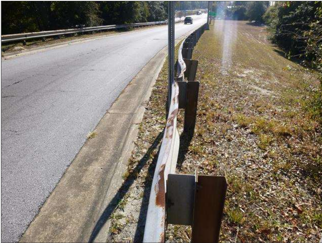
AT THE RAMP ABUTMENT SOUTHEAST CORNER GUARDRAIL, APPROXIMATELY 10' OUT FROM THE BRIDGE RAIL, DAMAGE WITH FLATTENED RAIL AND POSTS DEFLECTED UP TO 6" AT THE TOP [APPROXIMATELY 20' LONG AFFECTED]
