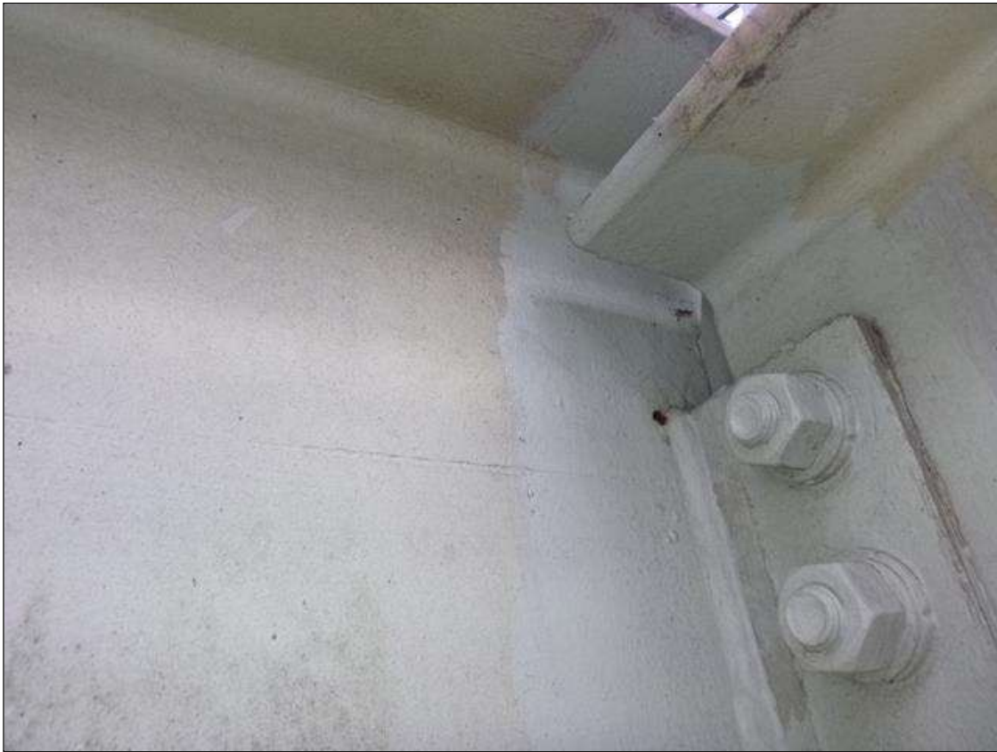
Span 18 Lift Span Stringer 11: OBSERVED IN 2020 INSP: CRACK NOT VISIBLE, AREA HAS BEEN PAINTED OVER. 2018 REPORT HAD BETWEEN FB's 6-7 - CRACK PROPAGATED 3/16" PAST ARREST HOLE AT TOP OF DIAPHRAGM CONNECTION
