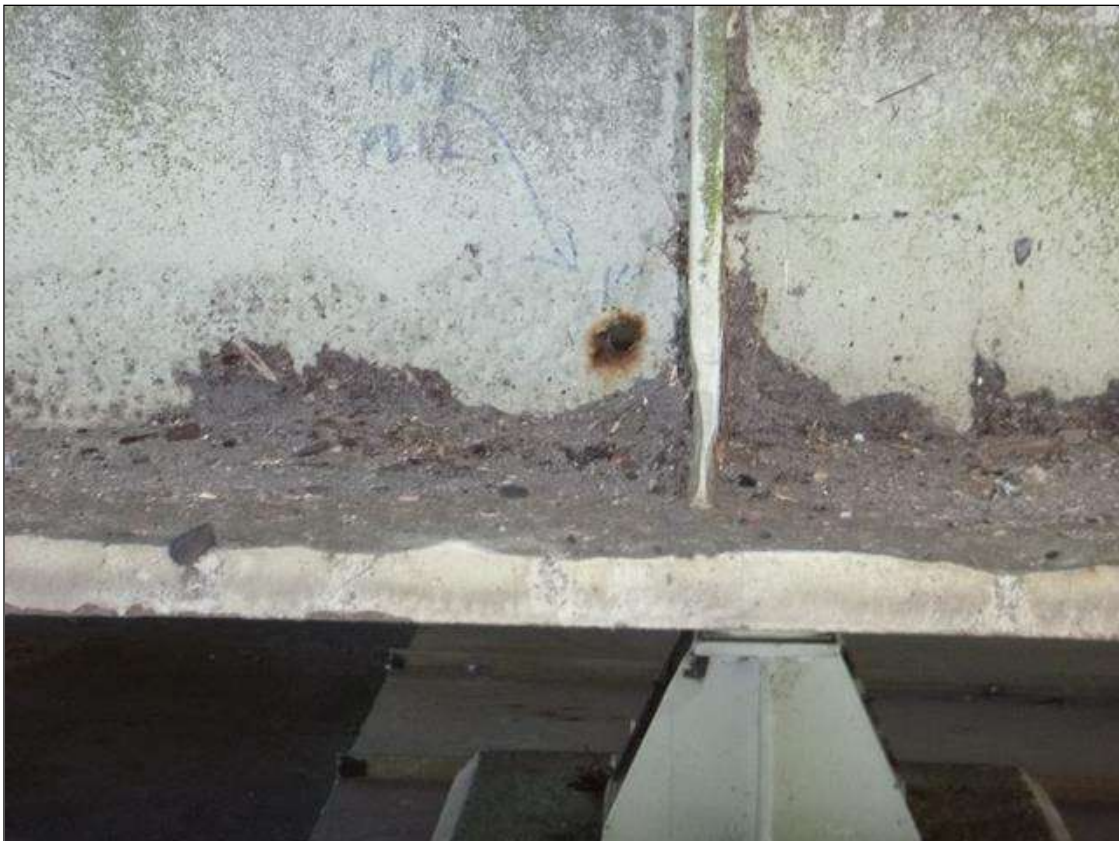
Span 18 Lift Span Floor Beam 12: 1" HOLE IN WEB AT BOTTOM FLANGE BETWEEN STRINGERS 4 & 5 - PROMPT ACTION REQUEST
