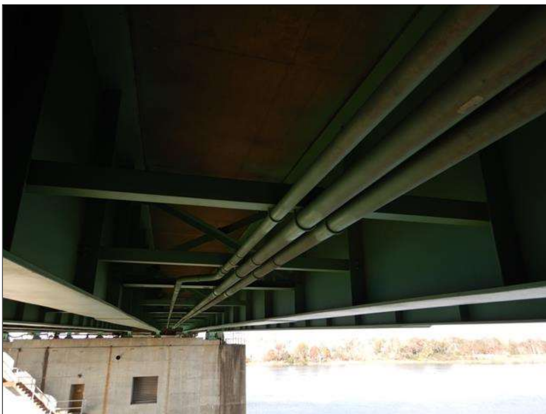
SPAN 20 BAY 2, (3) UP TO 4" DIAMETER STEEL CONDUITS HANG FROM STEEL SUPPORTS, FULL SPAN LENGTH
