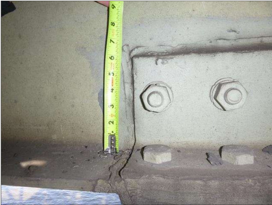
Span 18 Lift Span Stringer 3: REPAIR OBSERVED IN 2020 INSP: BETWEEN FB 10 - 11, REPAIR TO THE BOTTOM FLANGE AND LOWER WEB, 9 FOOT. LONG. 6" X 4" X 3/8" THICK ANGLE HAS BEEN BOLTED TO BOTH SIDES OF THE WEB. A 9" WIDE X 1/2" THICK PLATE HAS BEEN BOLTED TO THE BOTTOM FLANGE IN THE SAME AREA STARTING AT FB 11.
