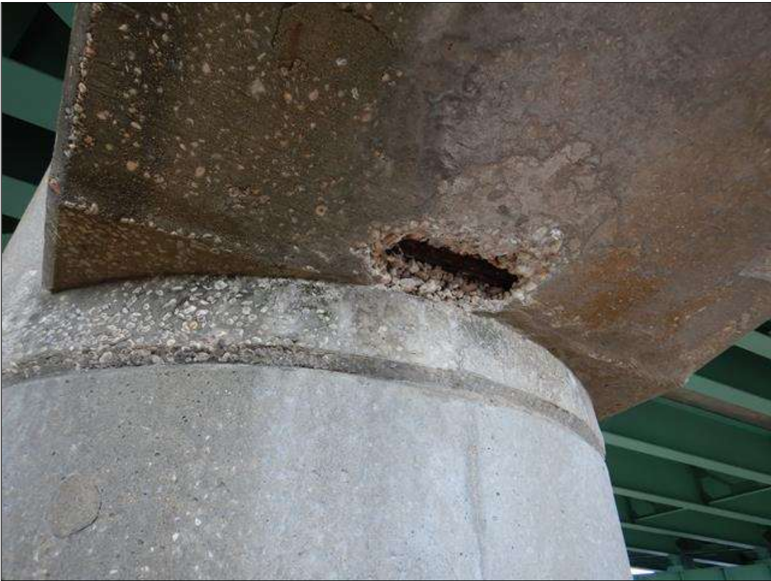
Bent 21 Cap 2: RIGHT SIDE OF COLUMN 3, BOTTOM OF CAP, SPALLING WITH EXPOSED REBAR [1' LONG X 6" WIDE X 2" DEEP] WITH LAYERED RUST ON THE REBAR
