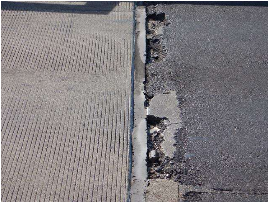
Span 1 Joint at Abutment 1: SCATTERED ALONG THE LENGTH OF THE ADJACENT DECK HEADERS IN THE RIGHT AN LEFT LANES, SPALLING WITH LOSS OF THE HEADER CONCRETE [UP TO 3" DEEP X 5" LONG] WITH LOSS OF ADHESION IN THE AFFECTED AREAS. THE BALANCE OF THE JOINT HEADERS HAVE SCATTERED MAP CRACKING TO 1/4" WIDE.
