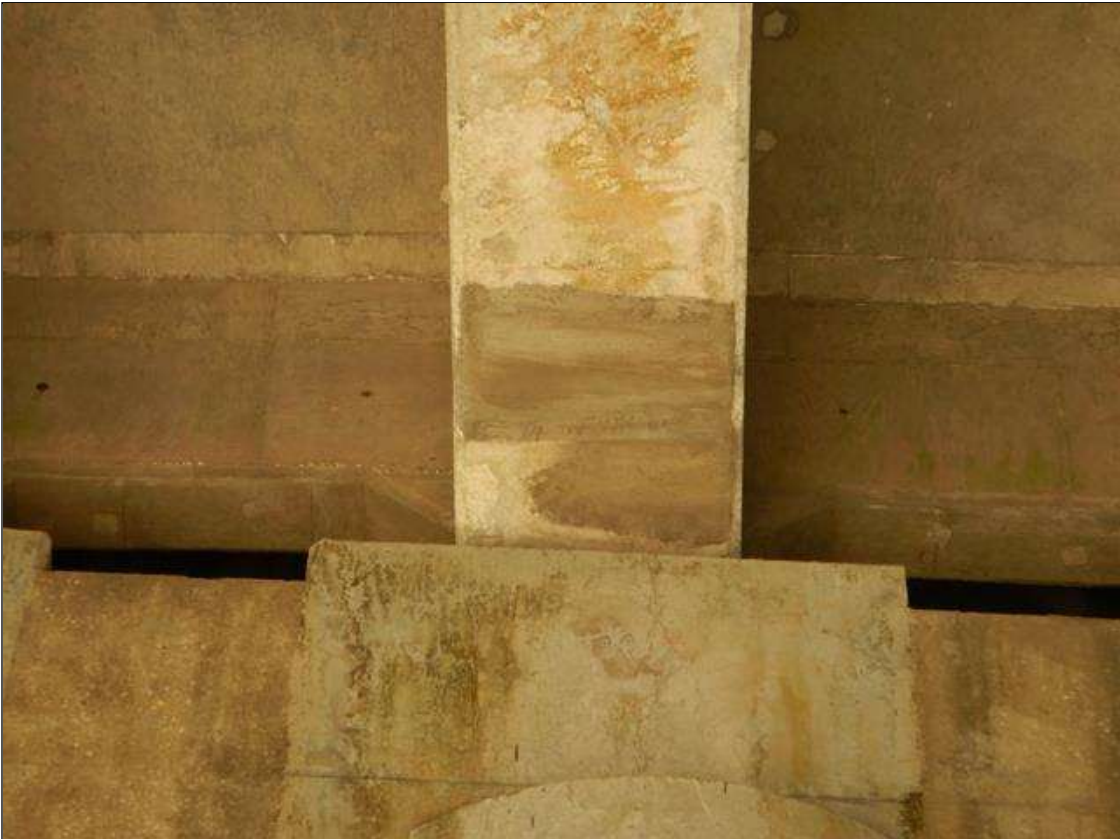
Span 28 Beam 10: [NEW REPAIR-PATCHING] FORMERLY --> spall with exposed rebar on the bottom face at bent 25 (6" x 4" x 1/2")
