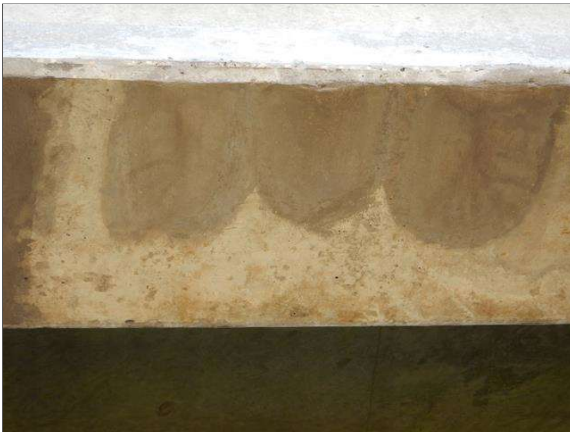
Span 34 - Ramp Span Beam 1: [NEW REPAIR-PATCHING] FORMERLY --> (x2) spalls with exposed rebar on the bottom face at 14ft and 18ft from Bent 30 up to (6" x 6" x 1/2")
