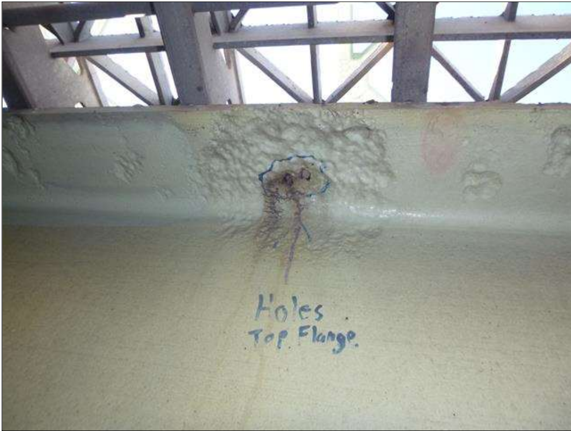
Span 18 Lift Span Stringer 4: BETWEEN FB's 3 & 4 - (2) 1/2" HOLES WIDE/ 6"LONG x 4"WIDE PITTED AREA ON NORTH SIDE OF TOP FLANGE AT 3' FROM FROM FB 4 CONNECTION - AREA CLEANED AND PAINTED, PAR ISSUED.
