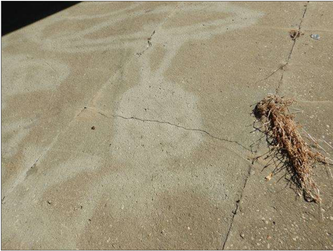
AT ABUTMENT 2, RIGHT SIDE OF THE CONCRETE SLOPE PROTECTION ON THE SLOPE, TWO AREAS OF HORIZONTAL CRACKING TO 1/8" WIDE [APPROXIMATELY 8' TOTAL]
