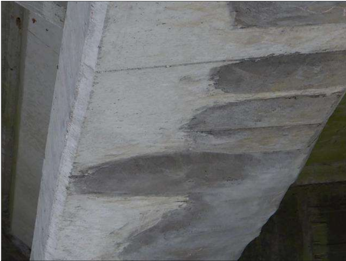
Span 11 Beam 6: [NEW REPAIR - PATCHING] FORMERLY --> (5" x 4" x 1/2") spall with exposed rebar on the bottom face at 13ft from bent 10
