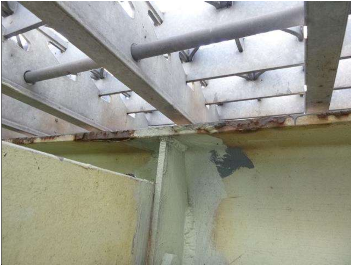
Span 18 Lift Span Stringer 9: BETWEEN FB's 9-10 - ACTIVE CORROSION ALONG TOP OF TOP FLANGE - NO MEASURABLE SECTION LOSS
