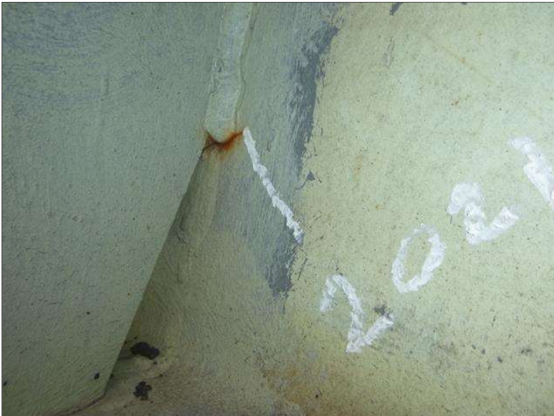
Span 18 Lift Span Stringer 6: BETWEEN FB's 8-9 - 1/2" LONG CRACK AT BOTTOM OF DIAPHRAGM CONNECTION - PROMPT ACTION REQUEST
