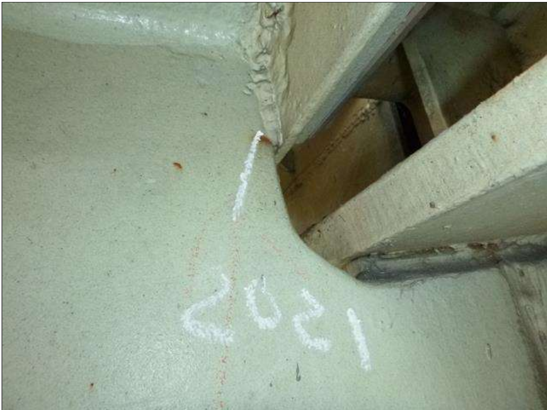
Span 18 Lift Span Stringer 8: LONGITUDINAL CRACK, 1/2" LONG IN THE TOP OF THE WEB AT FB 12, PAR ISSUED.
