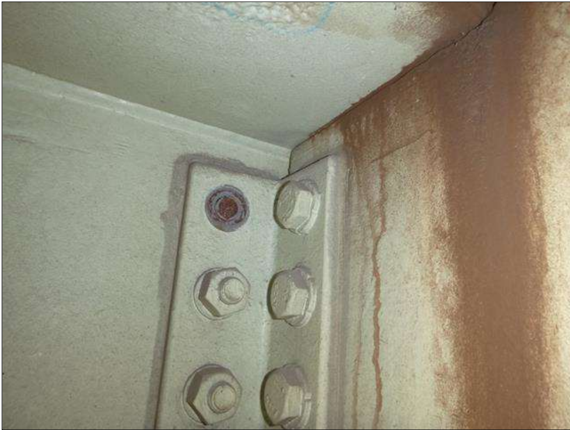
Span 18 Lift Span Stringer 4: BETWEEN FB 6-7, CONNECTION TO FB 7, TOP BOLT AT NORTH SIDE OF STRINGER IS SHEARED, PAR ISSUED.
