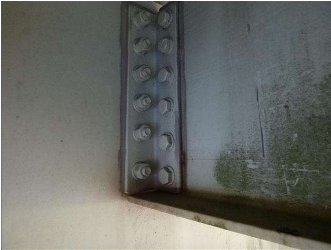
Span 18 Lift Span Stringer 10: BETWEEN FB's 9-10 - SLIGHT MOVEMENT UNDER LIVE LOAD AT FLOOR BEAM 10 - LOWER BOLTS AT STRINGER WEB CONNECTION ARE SECURE BUT NOT FULLY TIGHTENED - PROMPT ACTION REQUEST
