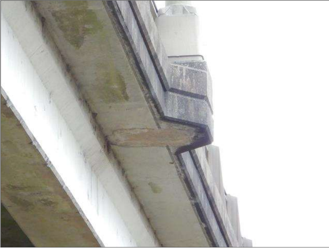
Span 2 Deck: [NEW REPAIR - PATCHING] FORMERLY --> spall with exposed rebar in the right overhang under light pole (27" x 20") DELAMINATION area and (19" x 12" x 2") spall
