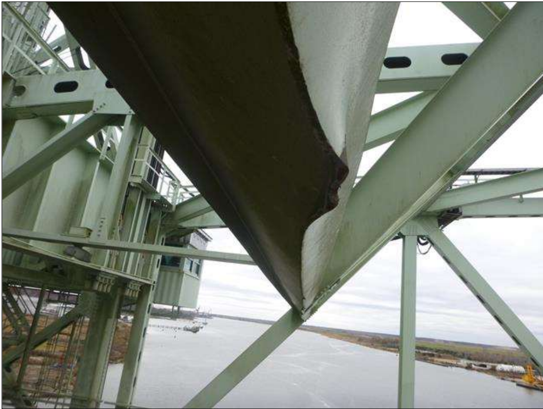
Span 18 Lift Span LB11: BOTTOM SWAY BRACE END PORTAL DAMAGE 30" WIDE X 2-1/4" DEFORMATION OVER RIGHT WEST BOUND LANE.
