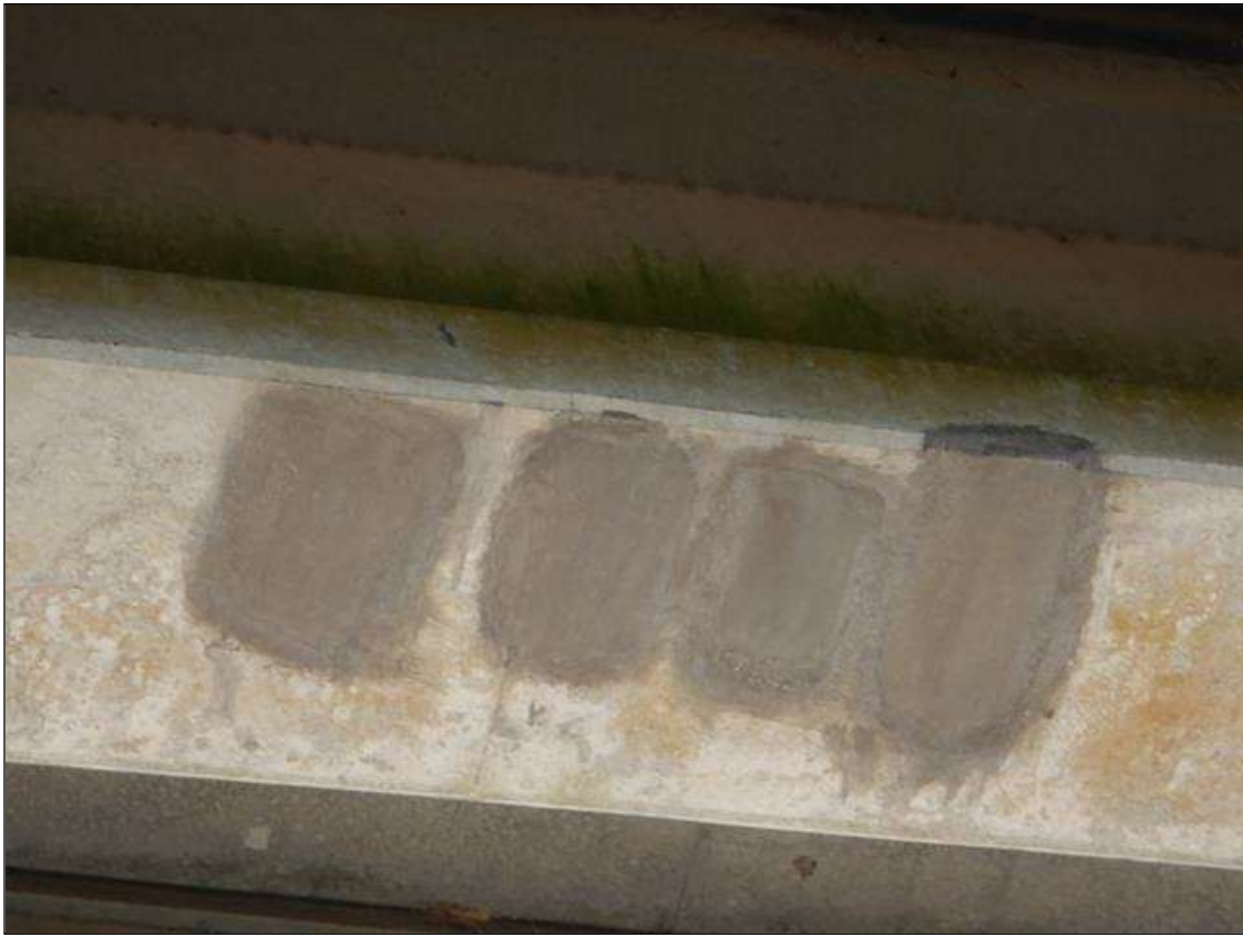
Span 29 Beam 7: [NEW REPAIR-PATCHING] FORMERLY --> (x4) spalls with exposed rebar on the bottom face at 26ft from Bent 27 up to (13" x 7" x 1/2")
