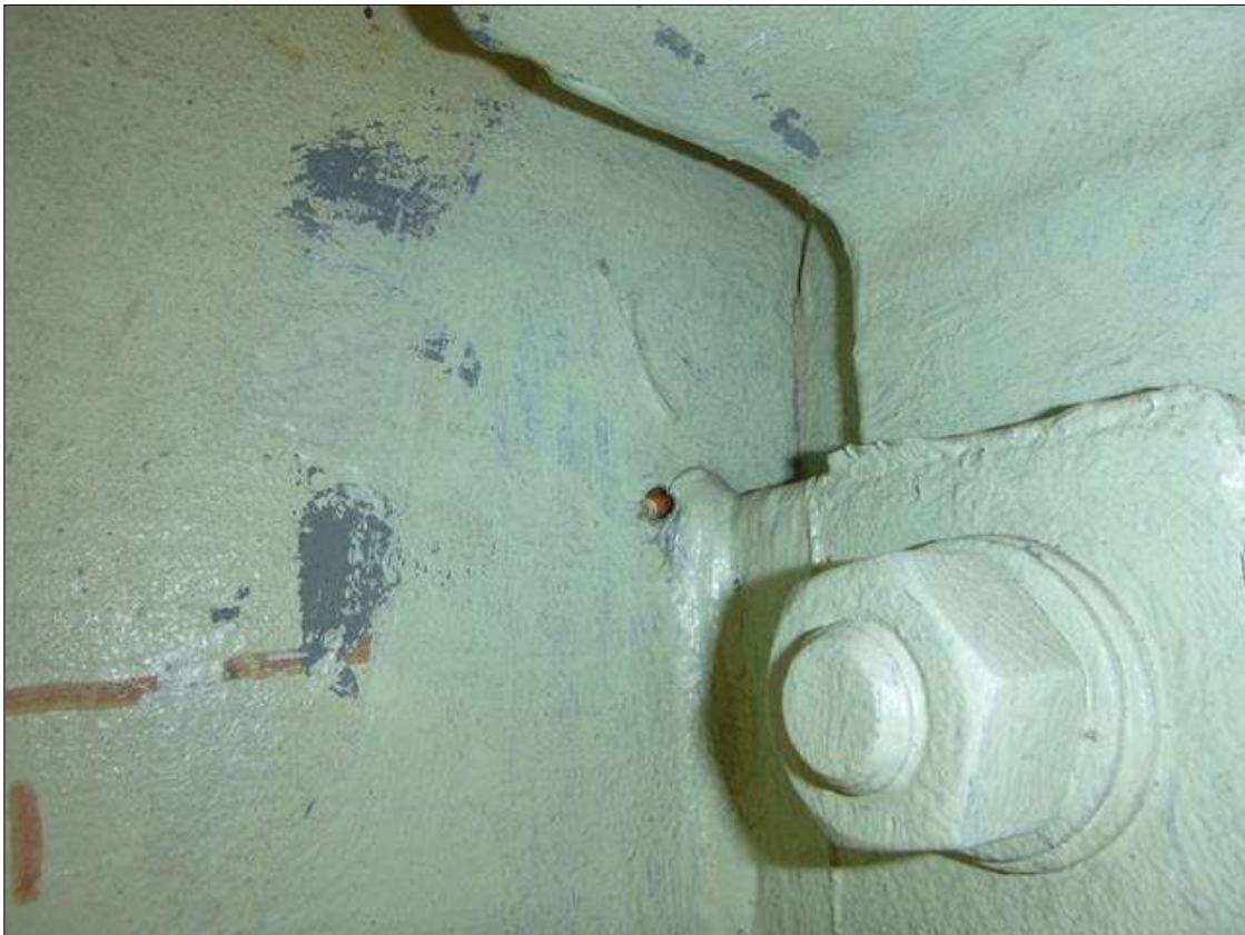
Span 18 Lift Span Stringer 11: OBSERVED IN 2020 INSP; BETWEEN FB's 9-10 - (1) 1/2" LONG CRACK PROPAGATING PAST ARREST HOLE AT TOP OF DIAPHRAGM CONNECTION, PAR ISSUED.
