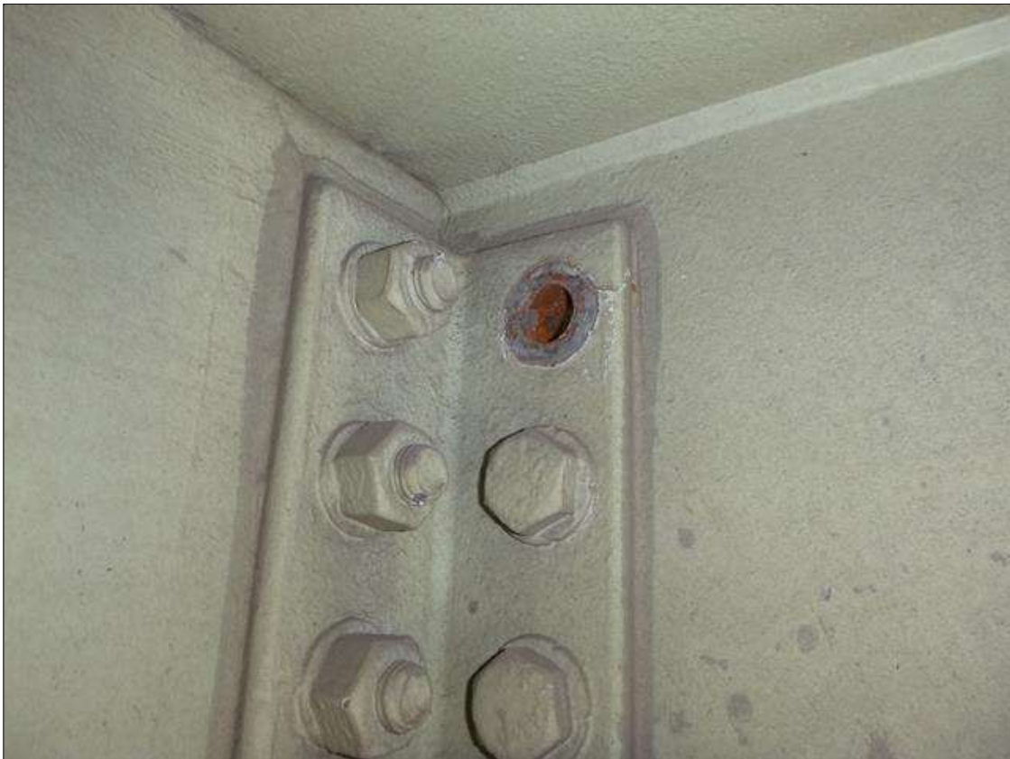
Span 18 Lift Span Stringer 3: BETWEEN FB 7-8, TOP BOLT HAS SHEARED AT SOUTH SIDE OF STRINGER CONNECTION TO FB. 8, PAR ISSUED.
