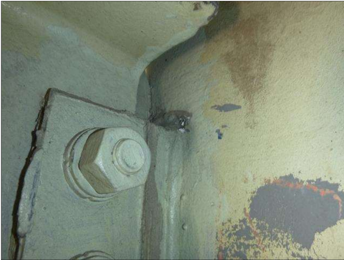
Span 18 Lift Span Stringer 4: BETWEEN FB's 7-8 - CRACK PROPAGATED 1/4" PAST ARREST HOLE AT TOP OF DIAPHRAGM CONNECTION - PROMPT ACTION REQUEST
