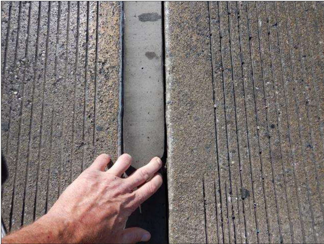
Span 21 Joint at Bent 18: SCATTERED ALONG THE LENGTH, LOSS OF ADHESION UP TO FULL DEPTH
