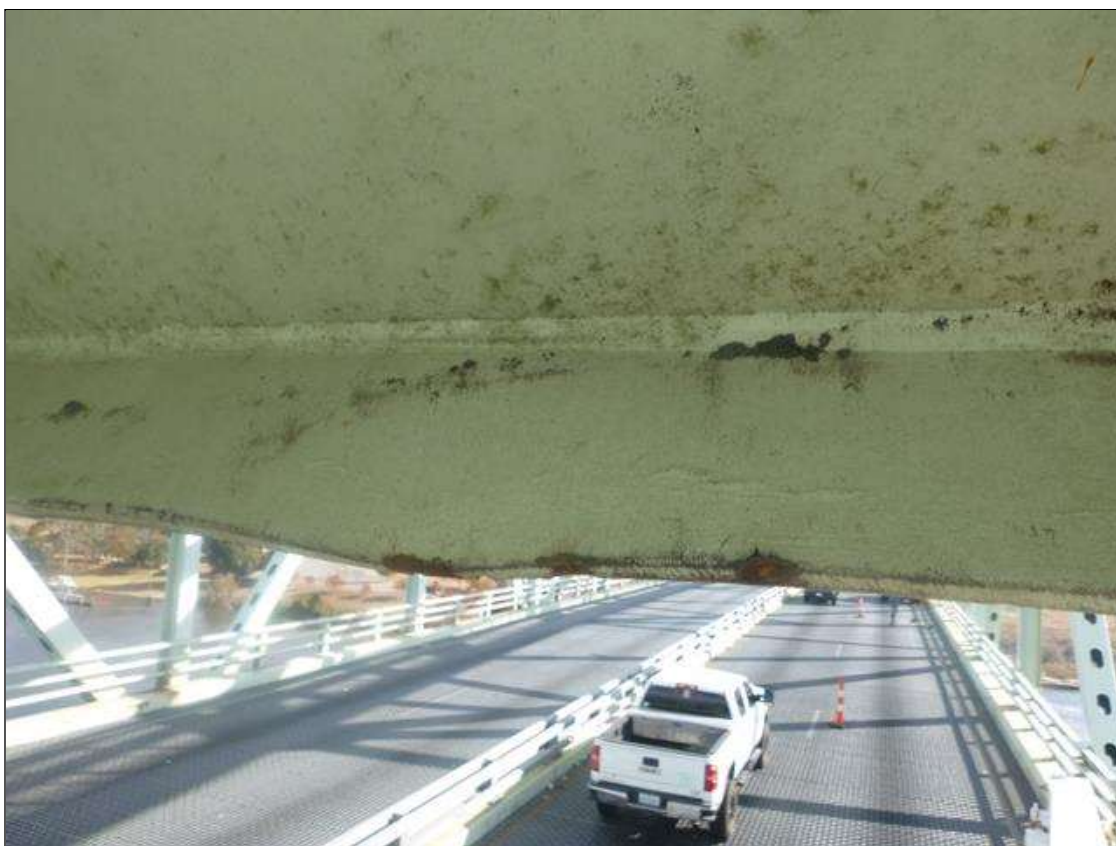
Span 18 Lift Span LB0: IMPACT DAMAGE 9" WIDE X 1" DEFORMATION IN WEST FLANGE OVER RIGHT EAST BOUND LANE.
