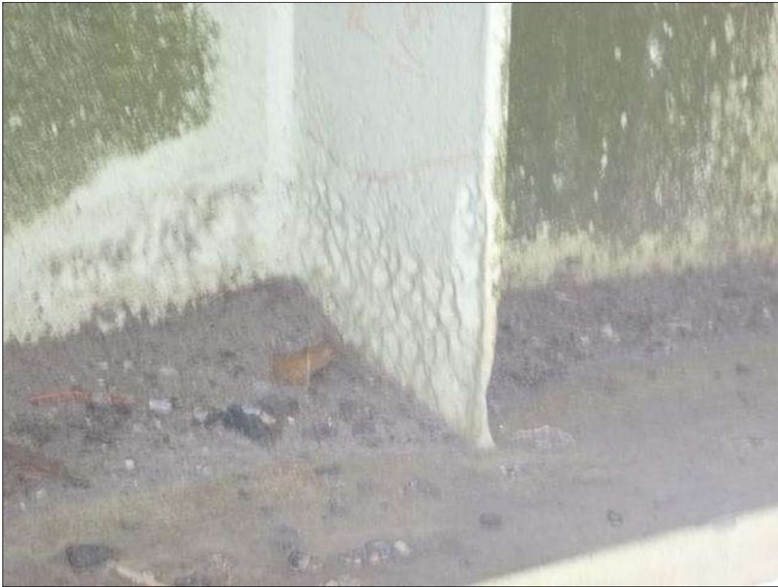
Span 18 Lift Span Floor Beam 10: VERTICAL STIFFENER 6 ON WEST SIDE - 2-1/2" HIGH PITTED AREA AT BOTTOM FLANGE - LOWER 1" OF AREA REDUCED TO 1/16" - CLEANED AND PAINTED
