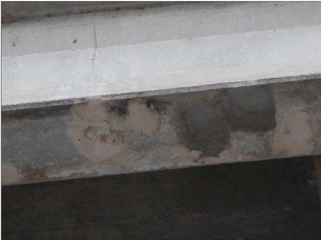
Span 9 Beam 9: [NEW REPAIR - PATCHING] FORMERLY --> (5" x 4" x 1/4") spall with exposed rebar on the bottom face at 10ft from bent 8
