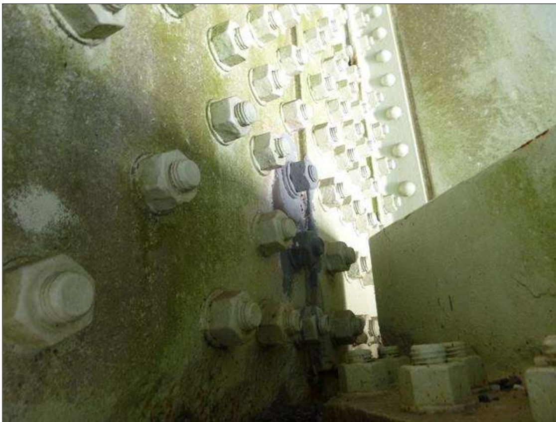
Span 18 Lift Span L6 NORTH: REPAIR OBSERVED IN 2020 INSP: 2 BOLTS HAVE BEEN REPLACED AREA HAS BEEN PAINTED OVER. 2018 REPORT HAD SHEARED BOLT ON INSIDE PLATE - WEST SIDE OF L6.
