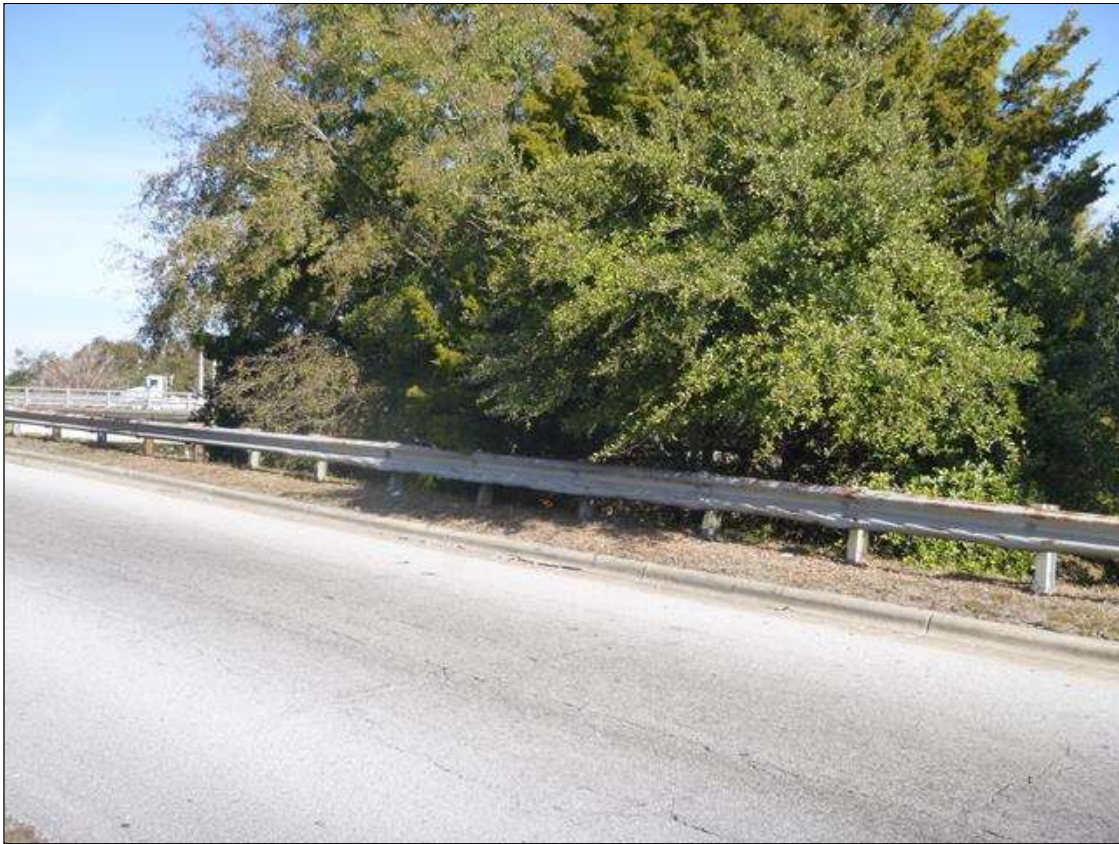
AT THE RAMP ABUTMENT NORTHEAST CORNER GUARDRAIL, SCATTERED ALONG THE LENGTH AND CONCENTRATED NEAR THE MIDDLE, DAMAGE WITH FLATTENED RAIL AND POSTS DEFLECTED UP TO 6" AT THE TOP [APPROXIMATELY 75' LONG AFFECTED]
