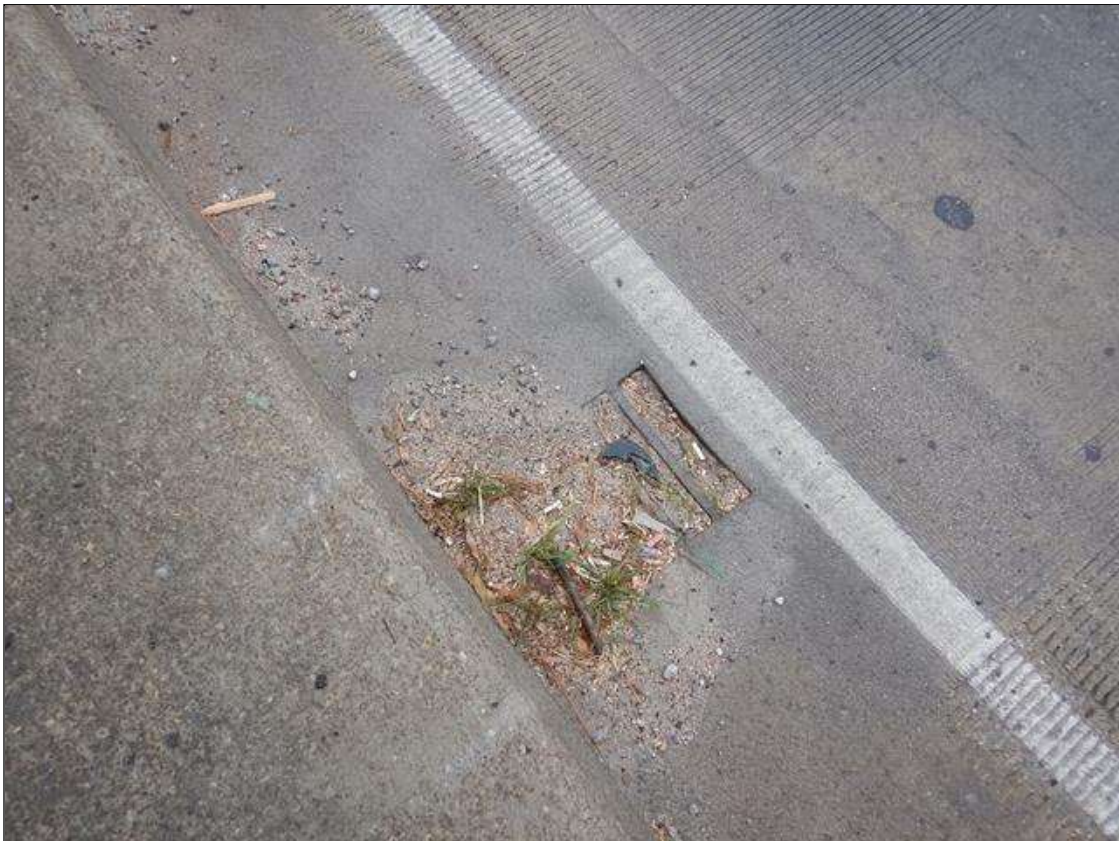
ALONG THE RIGHT & LEFT GUTTERLINES, THE DRAINAGE SYSTEM INLETS ARE IMPACTED WITH DEBRIS IN SCATTERED LOCATIONS.
