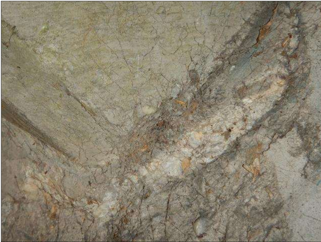
Span 35 - Ramp Span Beam 5: spall with no exposed steel on the bottom left flange under the end diaphragm at the Ramp End Bent (10" x 7" x 1/2" deep), DELAMINATION area at the back of the beam on the bottom left face at the same location (9" x 6")
