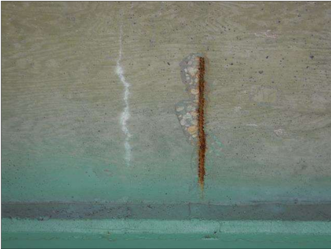
Span 14 Deck: spall with exposed rebar in bay 7 at 6ft from bent 13 (18" x 4" x 1/4")
