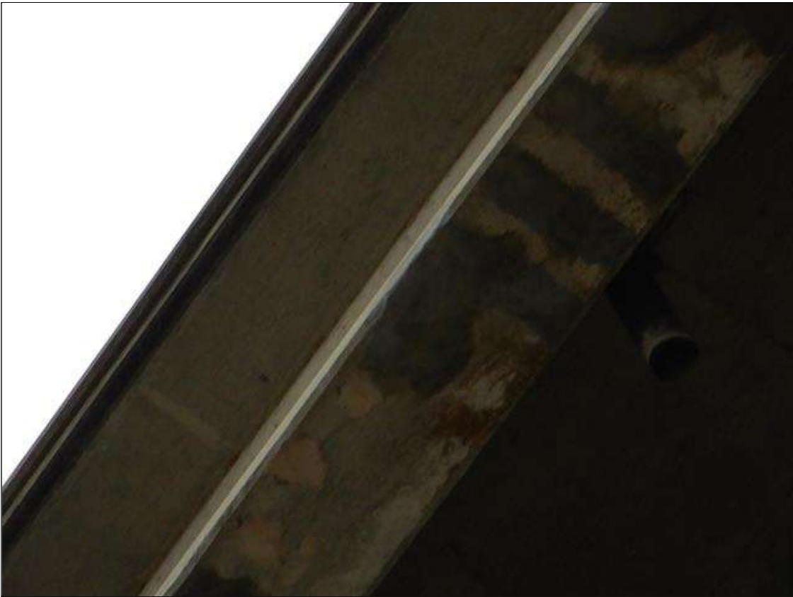
Span 10 Beam 9: [NEW REPAIR - PATCHING] FORMERLY --> (x4) spoalls with exposed rebar on the bottom face at 14ft from bent 9 up to (9" x 2" x 1/4")
