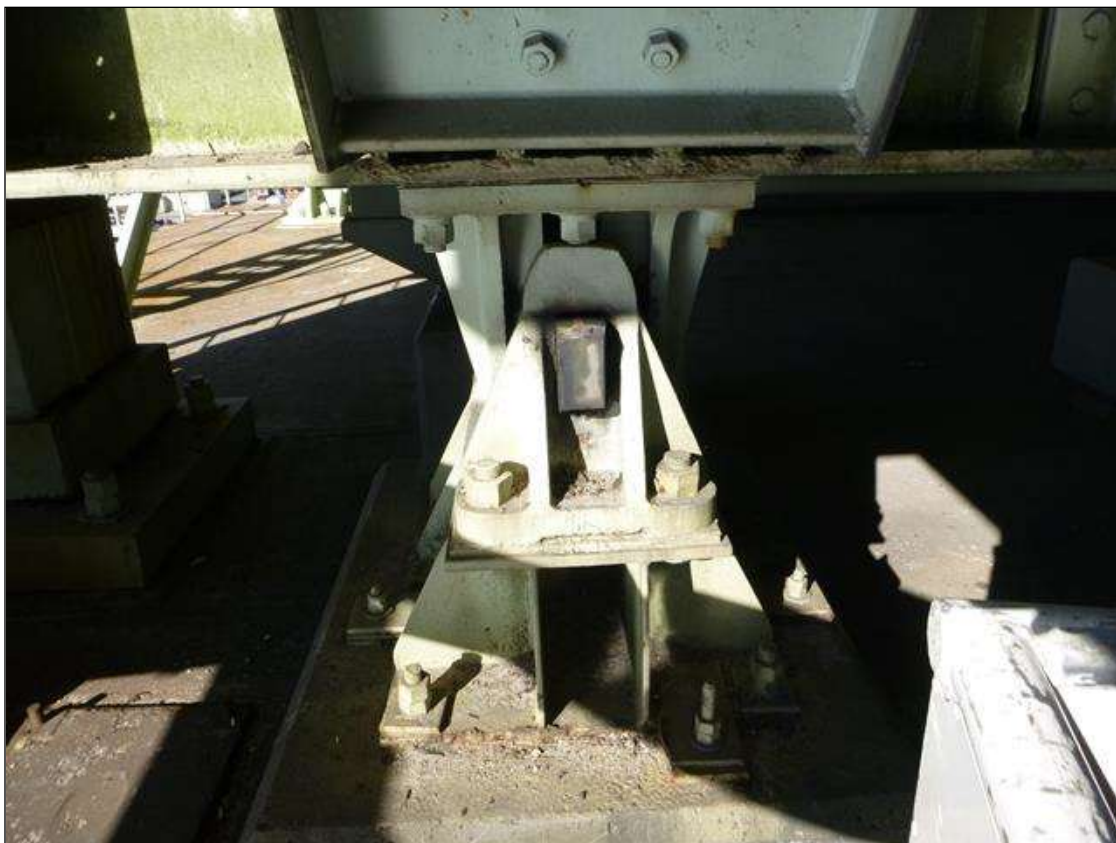
BRIDGE LOCK AT FLOORBEAM 0
