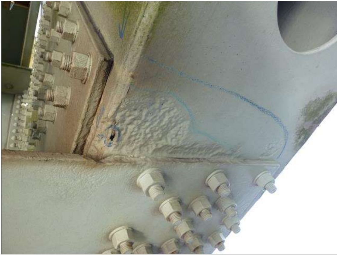
Span 18 Lift Span L10L11 NORTH: OBSERVED IN 2020 INSP: BOTTOM OF CHORD AT L10 - 4"LONG x 12"WIDE PITTED AREA UP TO 1/4"DEEP (APPROX. 3/16" REMAINING SECTION) WIDE/ 1-1/2"LONG x 3/16"WIDE HOLE AND 1-1/2"LONG CRACK PROPAGATING FROM WEST SIDE OF HOLE, PAR ISSUED.
