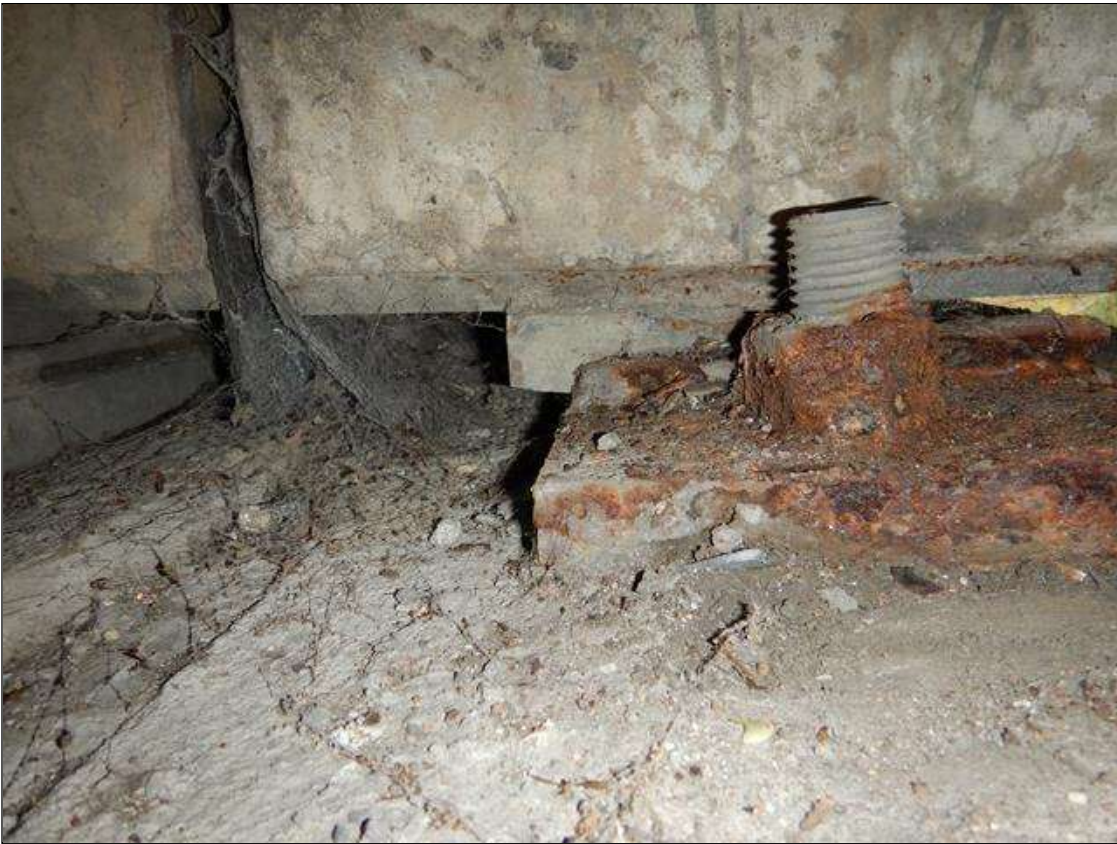
Span 1 Beam 2 - Beam 2 Far Bearing: Up to (3/4") movement of bearing to east beyond masonry plate with 13% loss of bearing.
