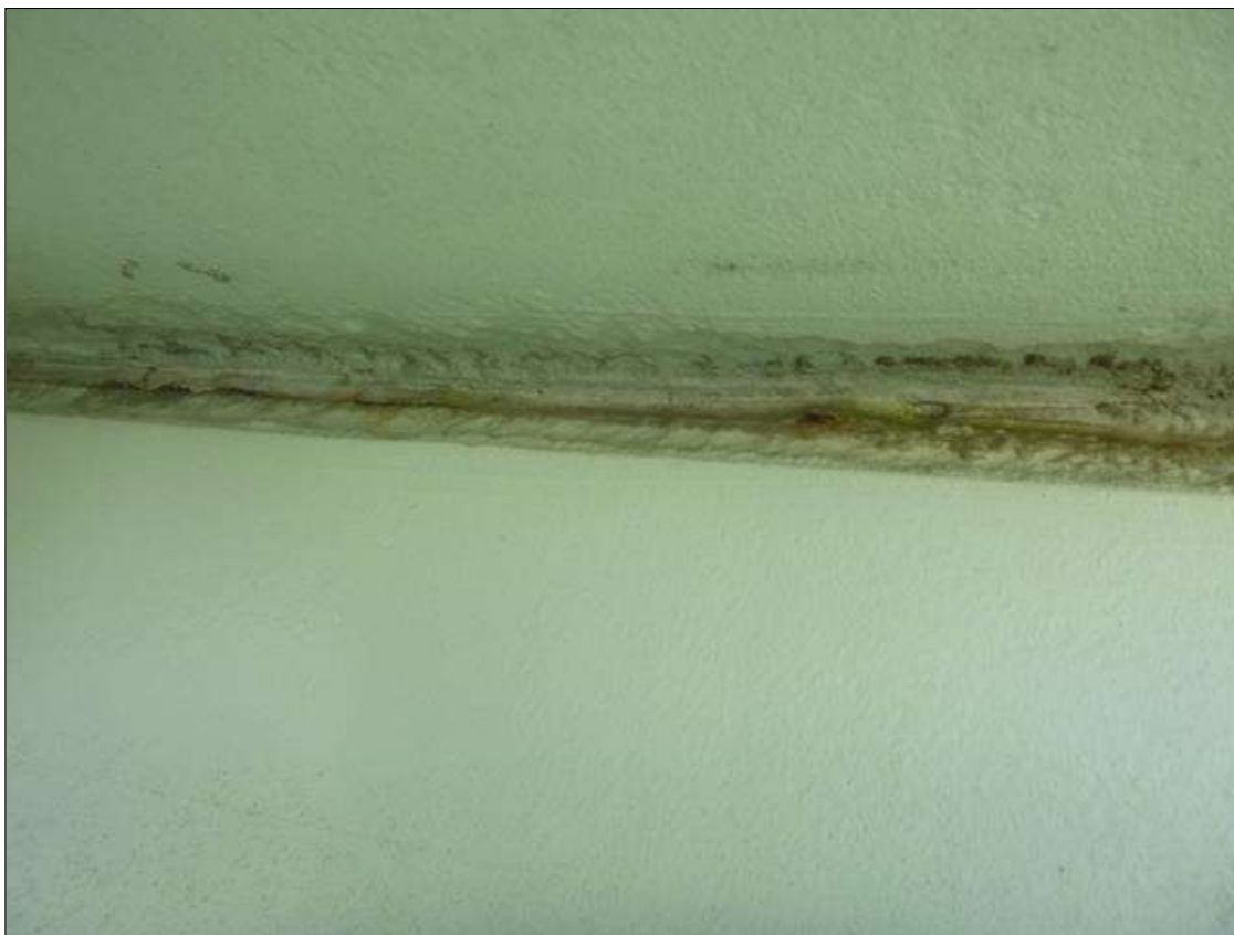
Span 18 Lift Span U2 SOUTH: 1/8" - 3/16" PITTING & SECTION LOSS TO TOP LATERAL BETWEEN U2 FOR A LENGTH OF 15FT (BOTTOM FLANGE)
