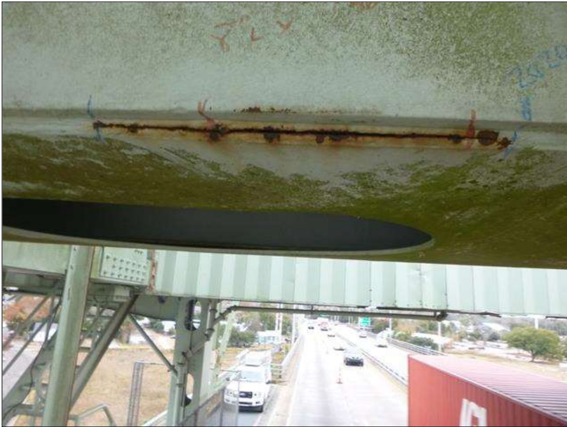
Span 19 EAST TOWER NORTH: 6/2020 - IMPACT DAMAGE - BOTTOM WEST HORIZONTAL TRUSS MEMBER - CRACK ALONG WELD AT BOTTOM WEST CORNER 14" LONG - LOCATED 6' FROM NORTHWEST TOWER LEG (PAR)
