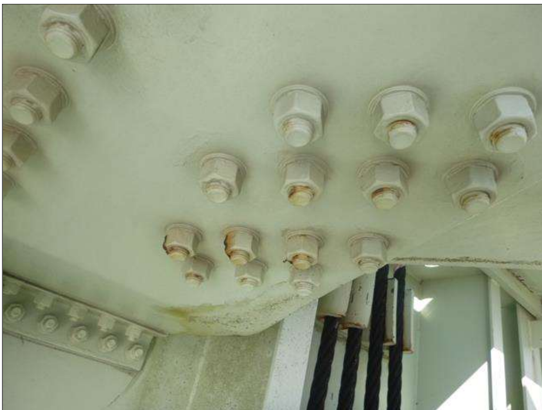
Span 18 Lift Span U0 SOUTH: AT LATERAL BRACING CONNECTION SURFACE RUST ON BOLTS
