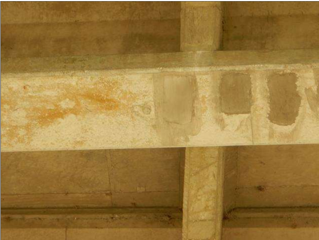
Span 27 Beam 11: [NEW REPAIR-PATCHING] FORMERLY --> (8" x 3" x 1/2") spall with exposed rebar on the bottom face at 21ft from bent 24
