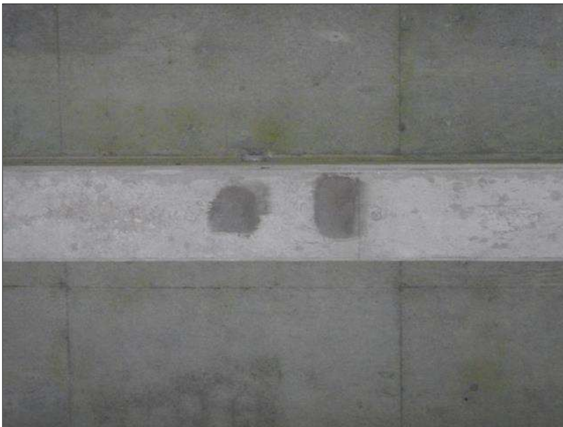
Span 8 Beam 3: [NEW REPAIR - PATCHING] FORMERLY --> (x2) spalls with exposed rebar at mid span on the bottom face up to (8" x 4" x 1/2")
