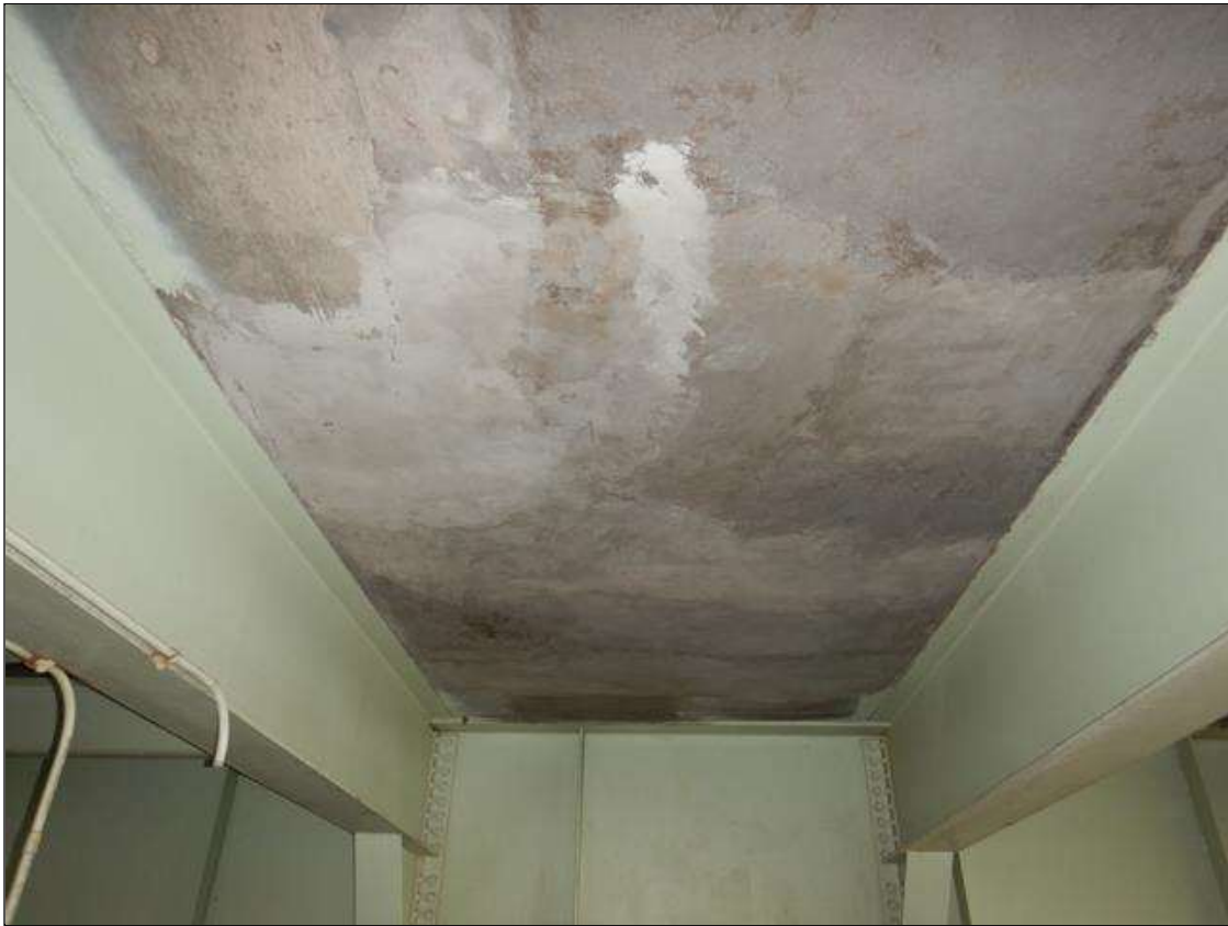
Span 19 Deck: [NEW REPAIR- PATCHING] FORMERLY --> PRIORITY MAINTENANCE - large spall with exposed rebar on the deck bottom between stringer 5 and 6 (16ft x 8ft x 2in)
