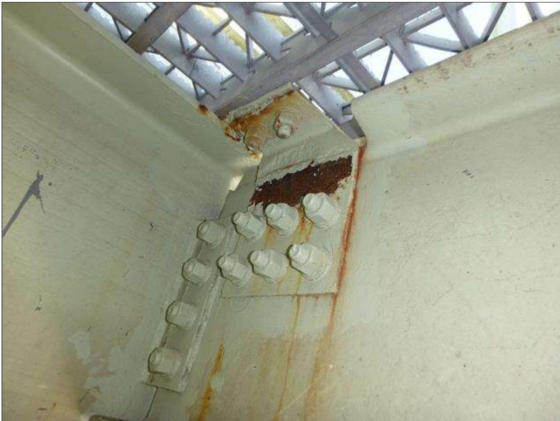
Span 18 Lift Span Stringer 1: BETWEEN FB's 0-12 - DIAPHRAGM CONNECTION TO STRINGER HAS SURFACE RUST.
