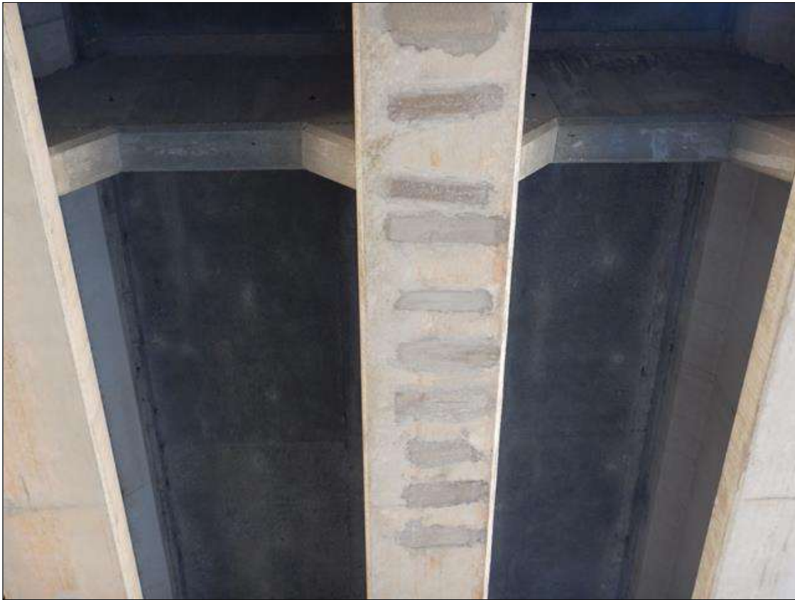
Span 31 Beam 2: [NEW REPAIR-PATCHING] FORMERLY --> spall with exposed rebar on the bottom face at 30ft from Bent 28 (8" x 5" x 1/2")
