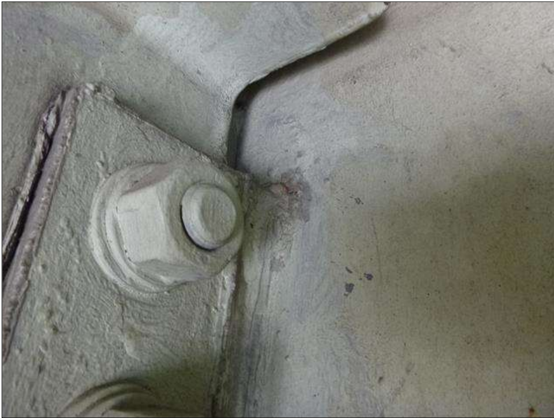
Span 18 Lift Span Stringer 5: BETWEEN FB's 9-10 - CRACK PROPAGATED 1/2" PAST ARREST HOLE AT TOP OF DIAPHRAGM CONNECTION – PROMPT ACTION REQUEST
