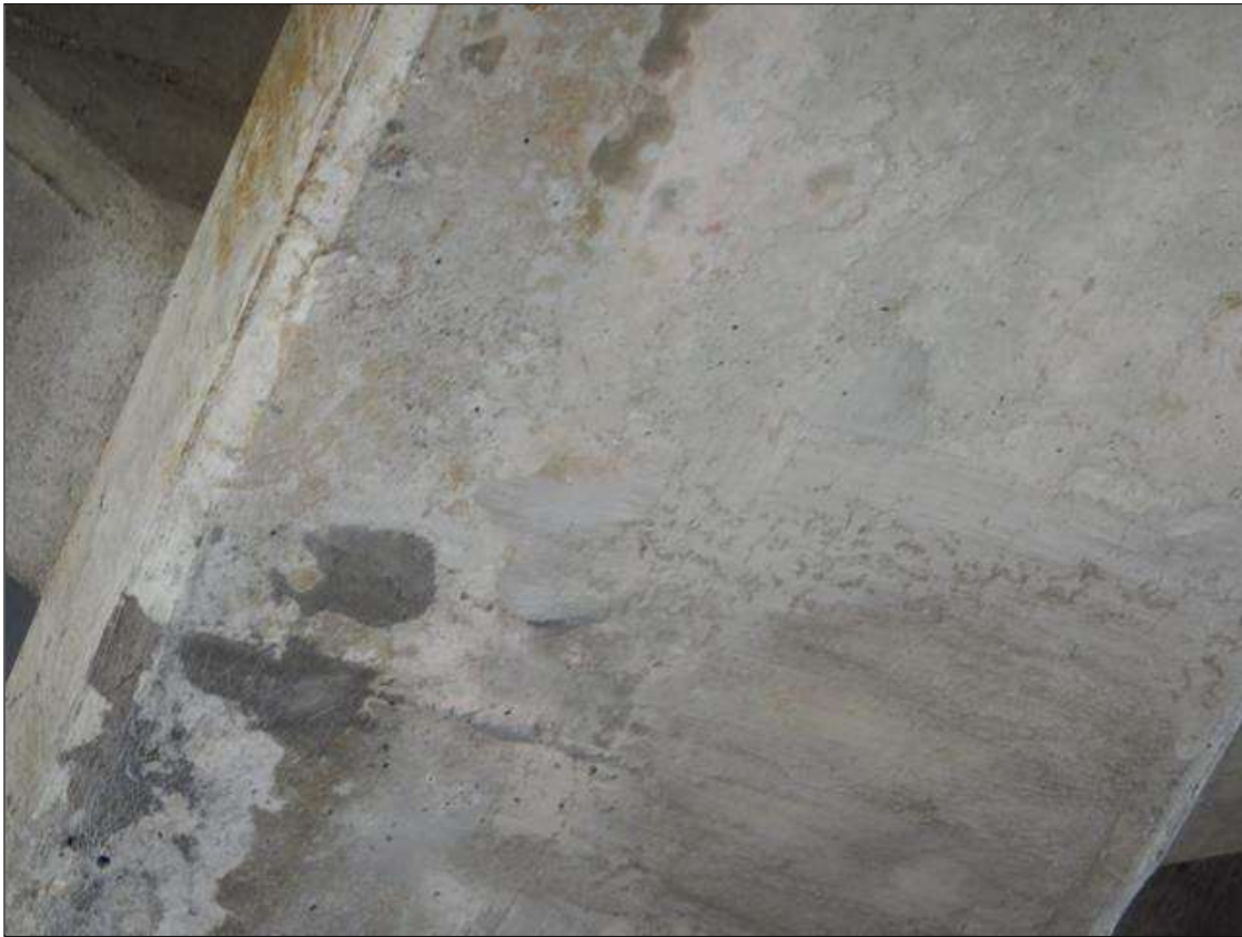
Span 35 - Ramp Span Beam 4: [NEW REPAIR-PATCHING] FORMERLY --> spall with exposed rebar on the bottom face at 19ft from Bent 31 (10" x 7" x 1/2")
