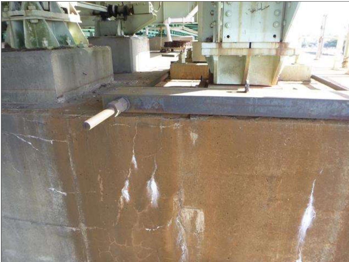
Bent 17 - Lift Span Bent Cap 1: 1/2" WIDE HORIZONTAL CRACK ALONG TOP EDGE OF WEST FACE AT SOUTH END - VISIBLE FROM TRUSS PANEL 2 BEARING
