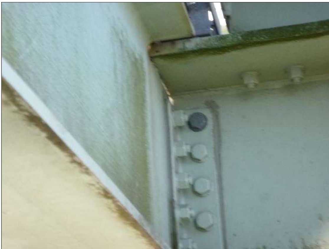
Span 18 Lift Span Stringer 1: NEW REPAIR 2021 INSPECTION: BETWEEN FB's 4-5 (1) NEW BOLT AT TOP NORTH SIDE AT FLOORBEAM 4.
