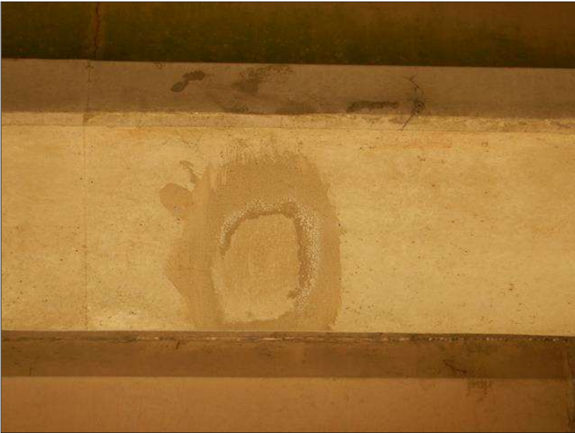
Span 30 Beam 10: [NEW REPAIR-PATCHING] FORMERLY --> (x3) spalls with exposed rebar on the bottom face at 20ft from bent 28 up to (10" x 3" x 1/4")
