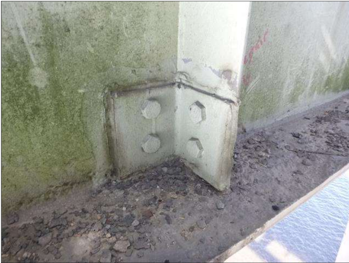
Span 18 Lift Span Floor Beam 9: REPAIR OBSERVED 2021 INSPECTION 7" HIGH 6" X 6" X 3/8" ANGLE BOLTED TO EAST AND WEST FACES ON SOUTH SIDE OF STIFFENER 4, 2020 INSPECTION HAD 7" x 7" PITTED AREA IN WEB AT BOTTOM FLANGE WIDE/ 3/16" DIAMETER HOLE - AREA ADJACENT TO VERTICAL STIFFENER 4 - CLEANED AND PAINTED
