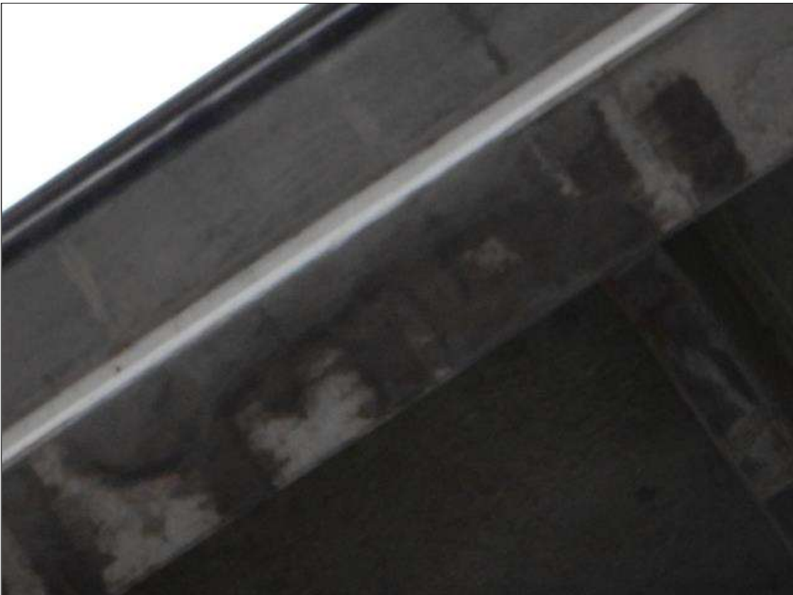
Span 10 Beam 9: [NEW REPAIR - PATCHING] FORMERLY --> (x5) spalls with exposed rebar on the bottom face at 21.5ft from bent 10 up to (9" x 3 1/2" x 1/4")
