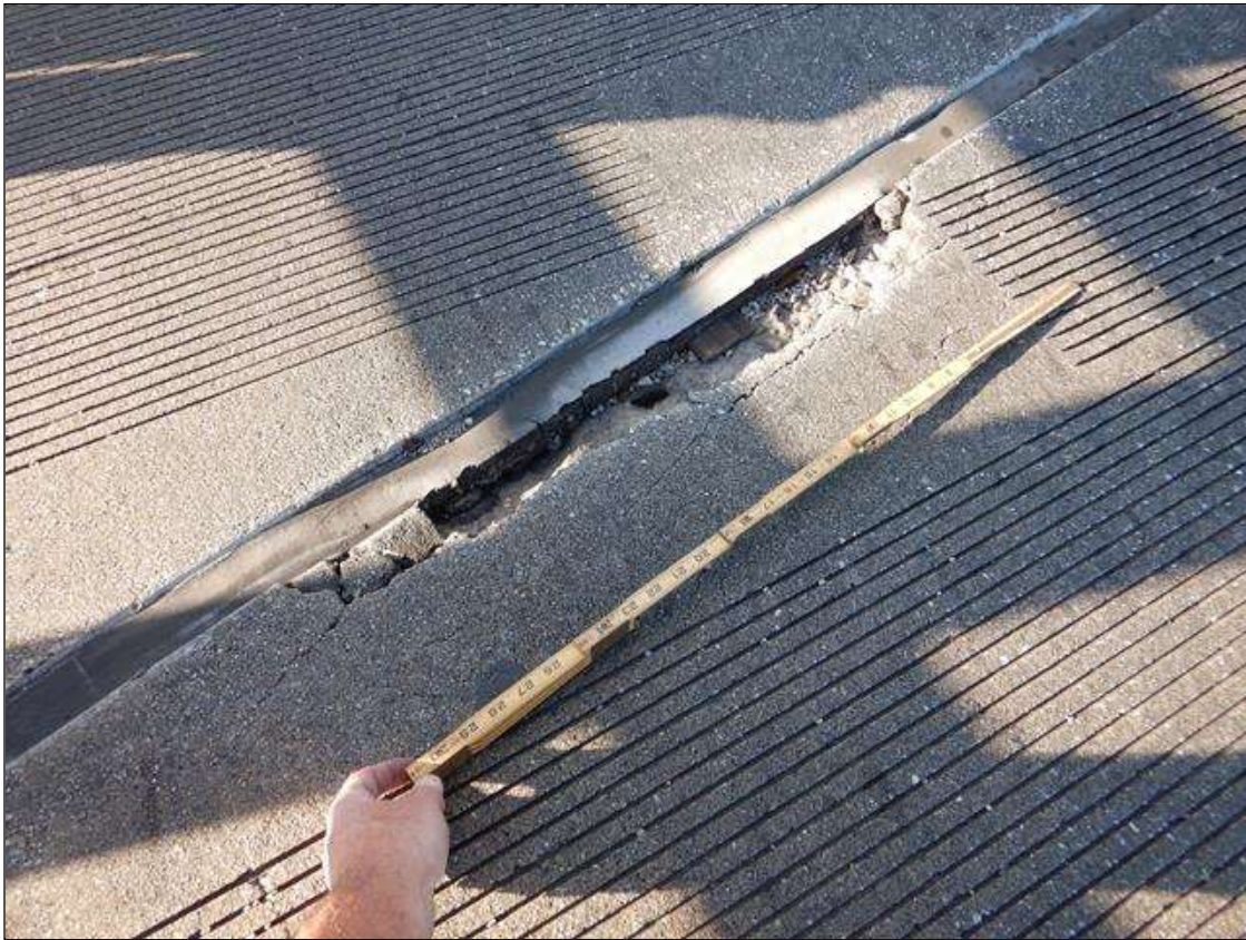
Span 8 Deck: [PROMPT ACTION REQUEST] RIGHT LANES AT BENT 7, SPALL (36" LONG x 3" WIDE x 1.5" DEEP AT 4' FROM RIGHT CURB)
