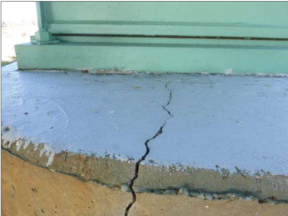
Bent 23 Pile 1: SCATTERED THROUGHOUT THE COLUMN, VERTICAL & MAP CRACKING TO 1/4" WIDE. THIS CRACKING CROSSES THE TOP OF THE COLUMN UNDER THE BEARING AREA.
