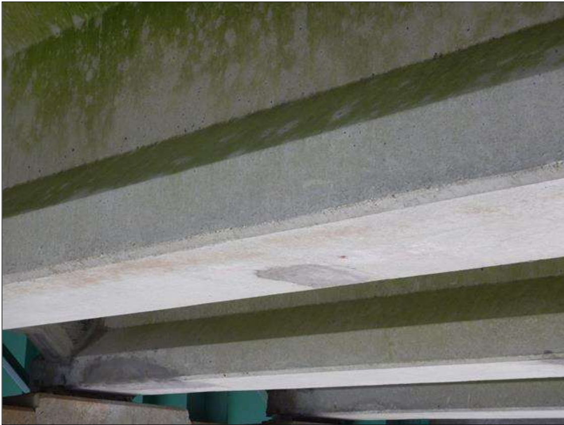
Span 11 Beam 5: [NEW REPAIR - PATCHING] FORMERLY --> (5" x 5" x 1/2") spall with exposed rebar on the bottom face at 12ft from bent 11
