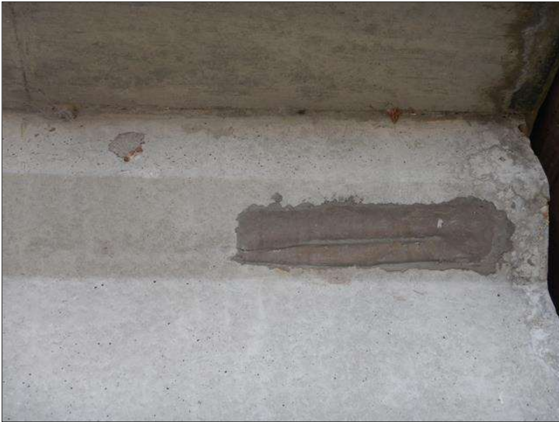
Span 8 Beam 1: [NEW REPAIR - PATCHING] FORMERLY --> (13" x 2 1/2") area of exposed rebar without section loss in the top left chamfer at bent 7
