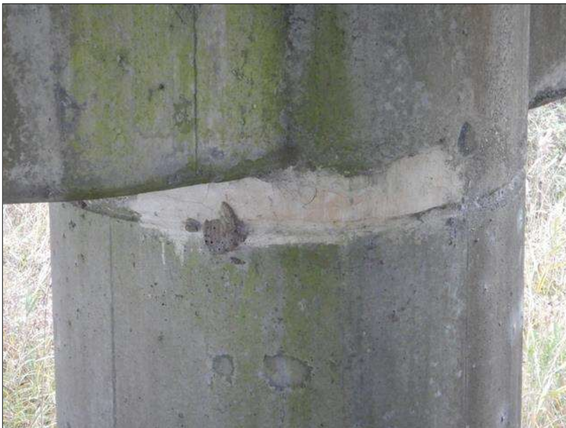
Bent 1 Pile 2: (40" x 8") sound patch on the southwest face at the cap, 0.009" wide horizontal cracks observed
