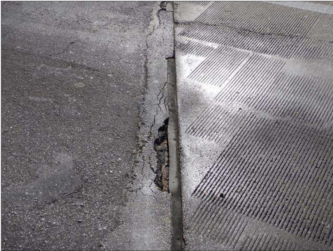
Span 32 Joint at Abutment 2: SCATTERED ALONG THE LENGTHS OF THE ADJACENT DECK HEADERS, SPALLING [UP TO 18" LONG X 3" WIDE X 2" DEEP]
