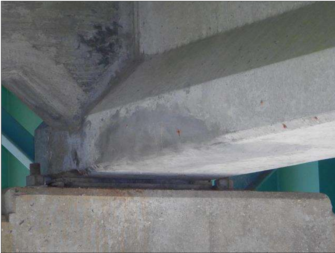
Span 11 Beam 6: [NEW REPAIR - PATCHING] FORMERLY --> PRIORITY MAINTENANCE - (x2) spalls with exposed strands on the bottom face starting at 5in from Bent 11 (8" x 7" x 1") and (7 1/2" x 6 1/2" x 2"), strands exposed for up to (1") long each, cracking up to 0.013" wide at this location for 28" long
