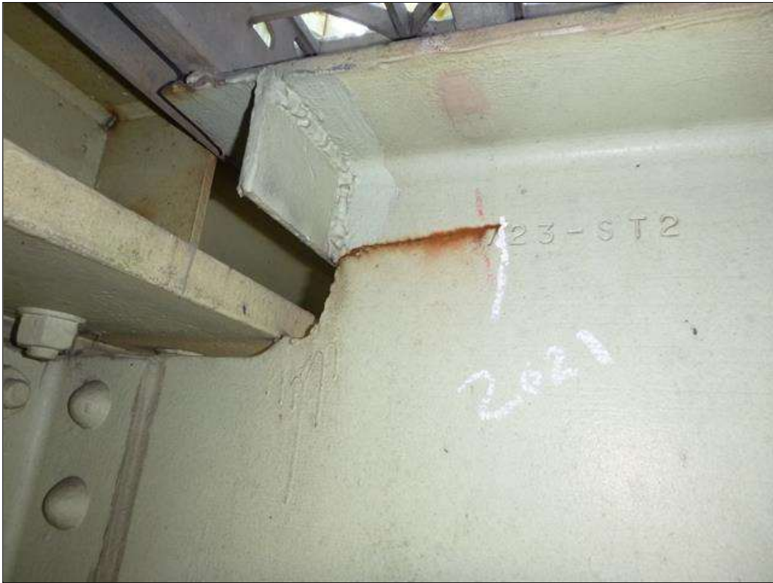
Span 18 Lift Span Stringer 9: LONGITUDINAL CRACK, 5" LONG IN THE TOP OF THE WEB AT FB 12, PAR ISSUED.
