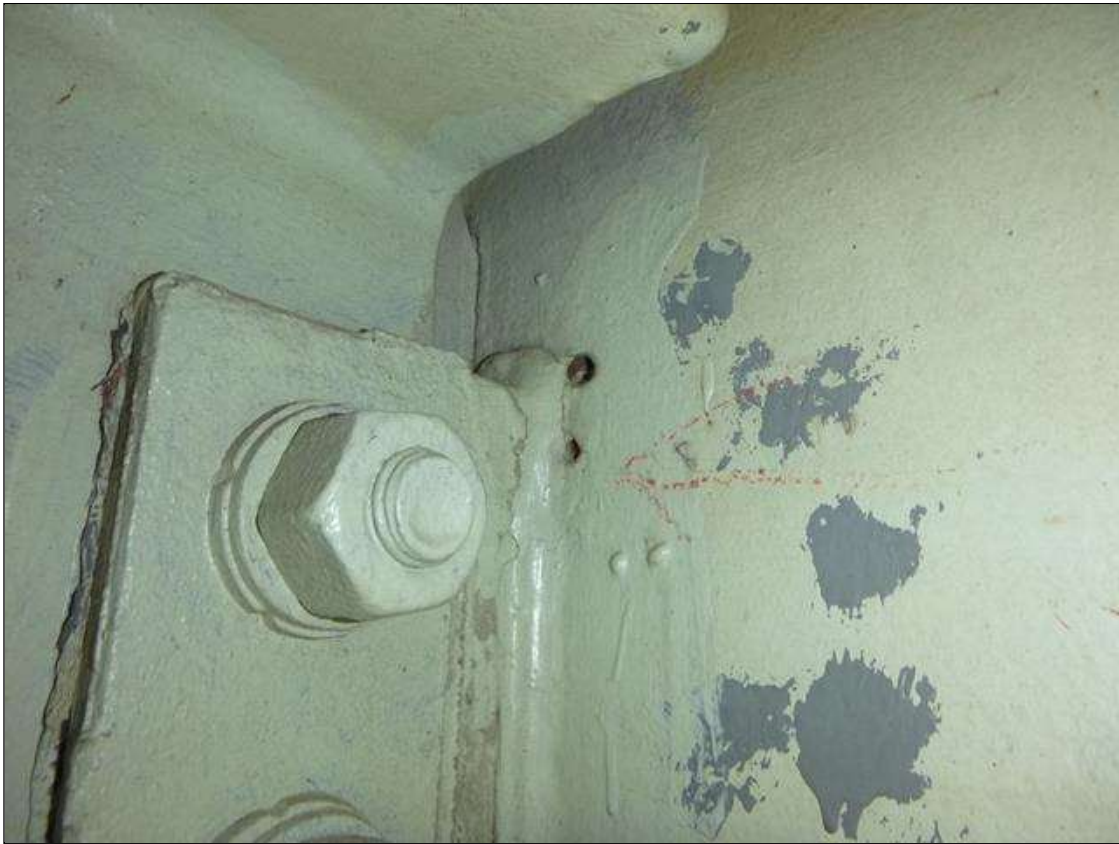
Span 18 Lift Span Stringer 11: BETWEEN FB's 4-5 - CRACK PROPAGATED 3/16" PAST ARREST HOLE AT TOP OF DIAPHRAGM CONNECTION - PROMPT ACTION REQUEST
