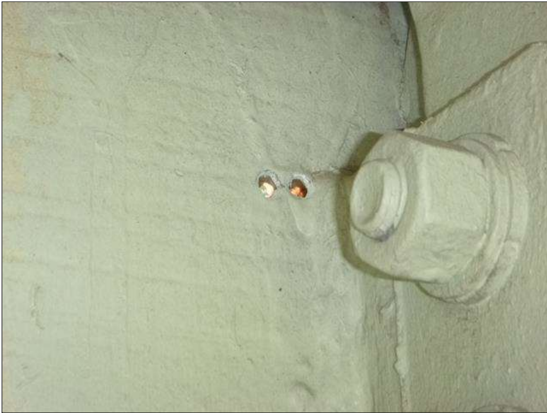
Span 18 Lift Span Stringer 11: BETWEEN FB's 8-9 - ARRESTED CRACK IN WEB AT TOP OF DIAPHRAGM CONNECTION
