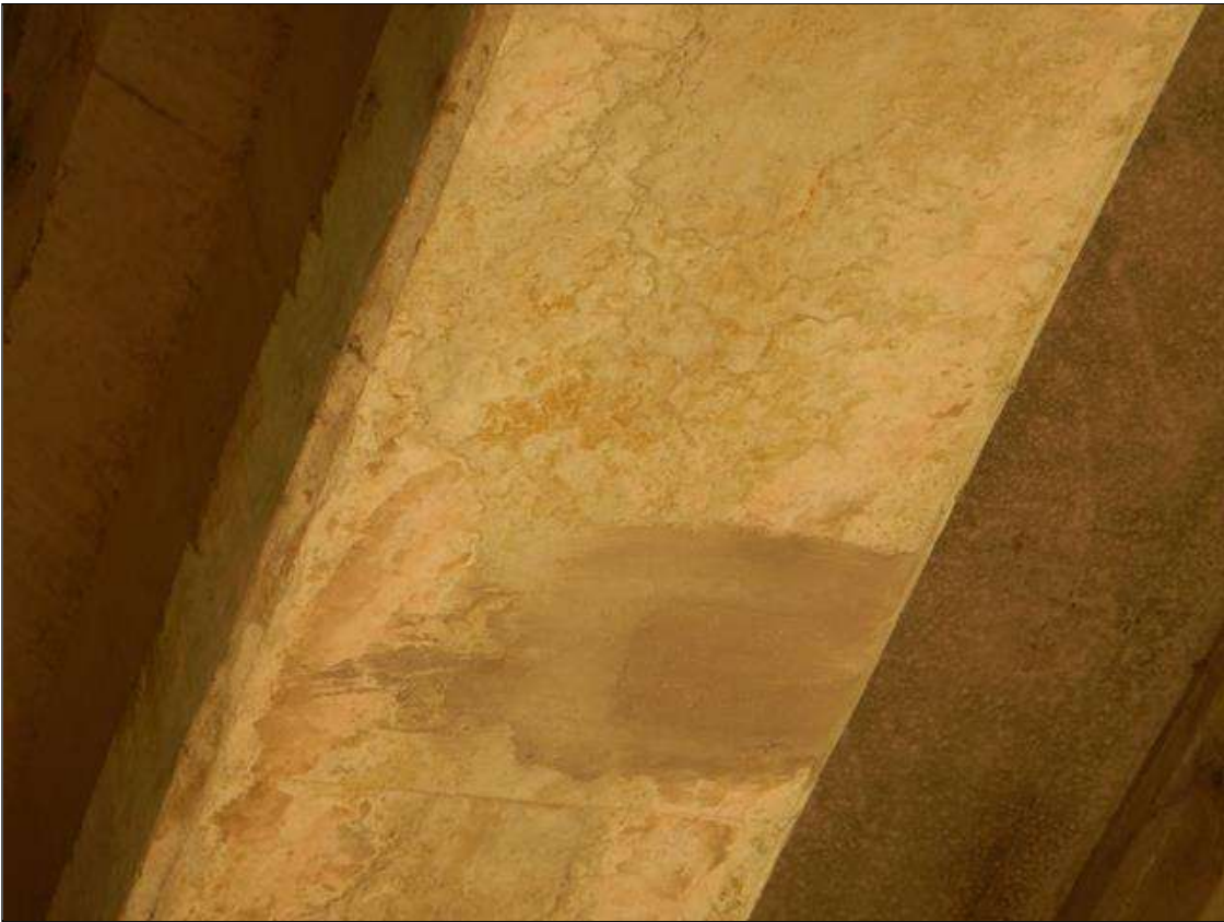
Span 30 Beam 9: [NEW REPAIR-PATCHING] FORMERLY --> DELAMINATION on the bottom face at 7ft from bent 28 (6" x 6")
