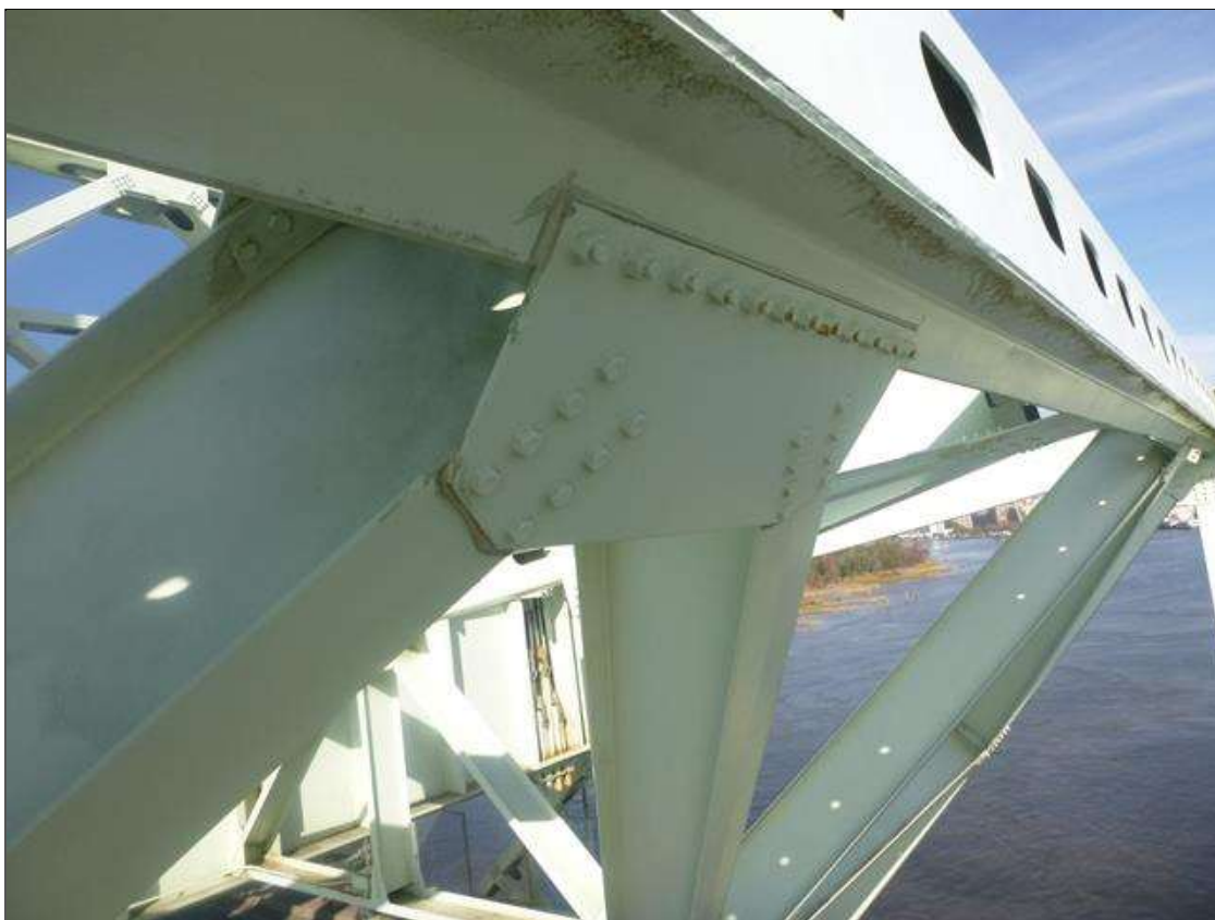
Span 18 Lift Span LB1: SURFACE RUST ON BOLTS AT RANDOM.
