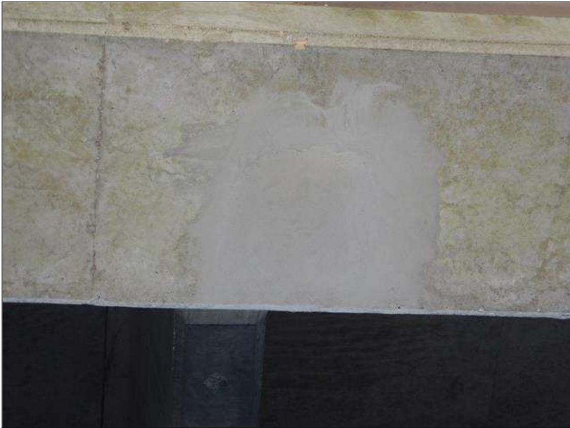
Span 30 Beam 4: [NEW REPAIR-PATCHING] FORMERLY --> (x4) spalls with exposed rebar on the bottom face at mid span up to (10" x 9" x 1/4")
