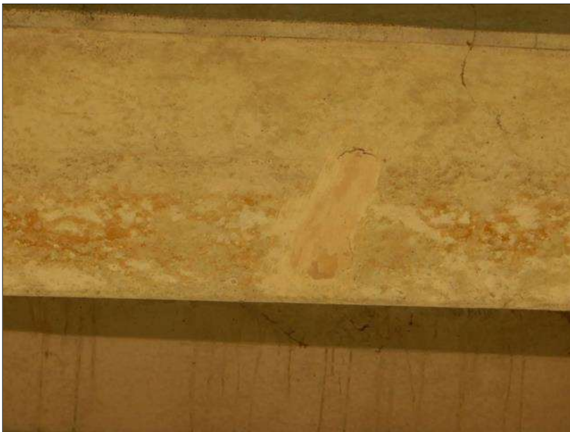
Span 29 Beam 10: (11" x 5") unsound patch on the bottom face near mid span
