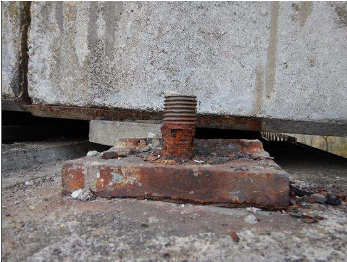
Span 1 Beam 1 - Beam 1 Far Bearing: Up to 100% section loss on the left anchor rod nut
