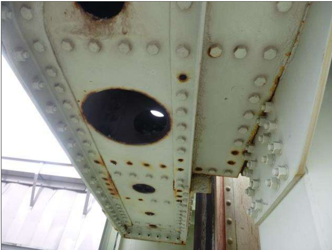
Span 18 Lift Span U12 NORTH: WHEEL GUIDE BOTTOM PLATE 20 MISSING BOLTS WITH CORROSION AT BOLT HOLES.
