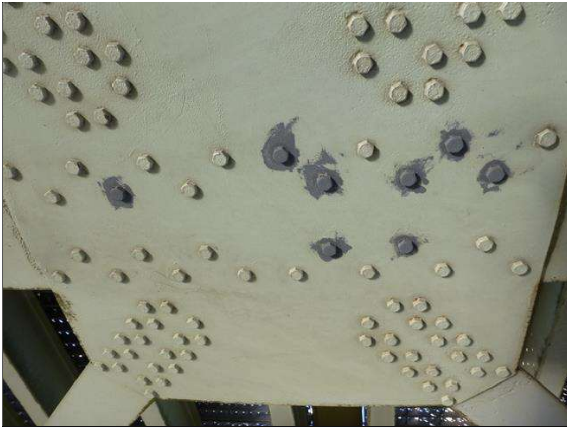
Span 18 Lift Span Floor Beam 9: NEW REPAIR OBSERVED IN 2021 INSPECTION (6) NEW BOLTS AT CENTER BOTTOM LATERAL CONNECTION, 2020 INSPECTION REPORT - CENTER BOTTOM LATERAL GUSSET - 30% - 90% LOSS TO (8) FASTENERS AT BOTTOM FLANGE ON EAST SIDE - CLEANED AND PAINTED
