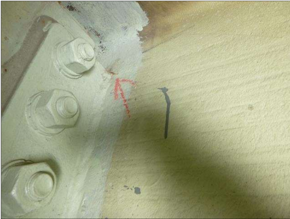
Span 18 Lift Span Stringer 7: BETWEEN FB's 5-6 - 1" CRACK IN WEB ACROSS TOP OF WELD AT DIAPHRAGM CONNECTION - SOUTH SIDE - PROMPT ACTION REQUEST
