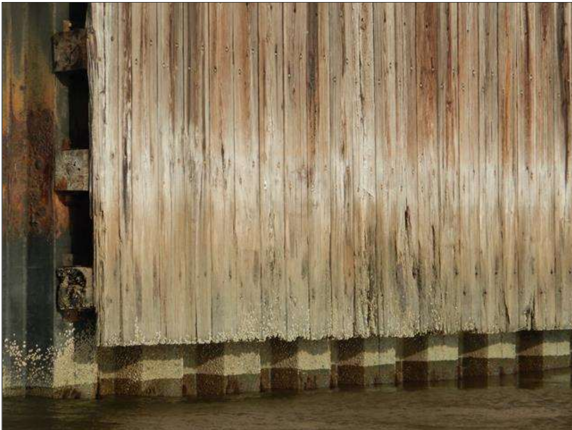
Bent 16 - Lift Span Bent Footing: EAST FACE: TIMBER SHEETING BUFFER BOARDS ARE DECAYED 6' HIGH X UP TO 2" DEEP ALONG TIDAL ZONE.
