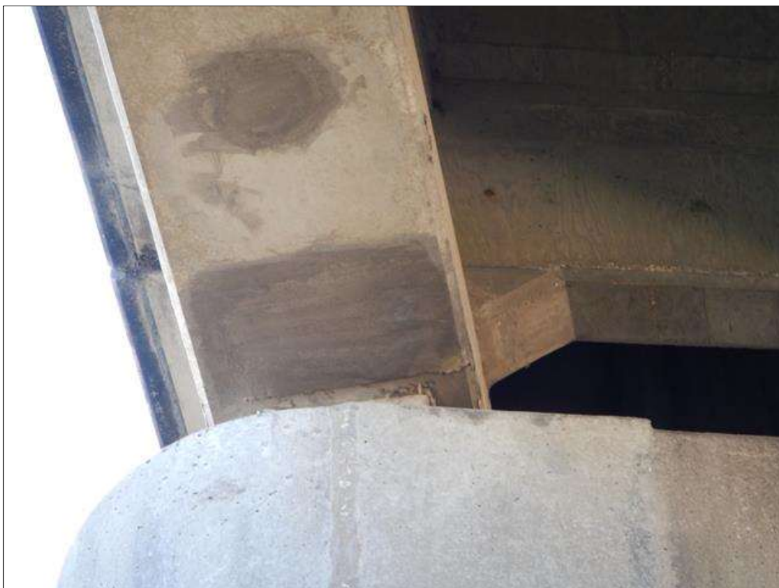
Span 29 Beam 1: [NEW REPAIR-PATCHING] FORMERLY --> spall with exposed rebar on the bottom face at bent 26 (11" x 6" x 1/2')
