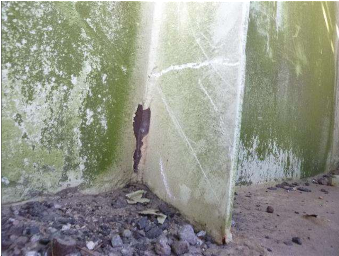
Span 18 Lift Span Floor Beam 10: REPAIR OBSERVED IN 2021 INSP: STIFFENER 1 HAS BEEN REPAIRED FROM THE BOTTOM UP 7" HIGH. 2020 REPORT HAD VERTICAL STIFFENER 1 EAST - 3" HIGH PITTED AREA AT BOTTOM FLANGE WIDE/ ~1/2" DIAMETER HOLES AT EDGES - 1/16" TO 1/8" REMAINING SECTION IN LOWER 1" OF AREA - PROMPT ACTION REQUEST
