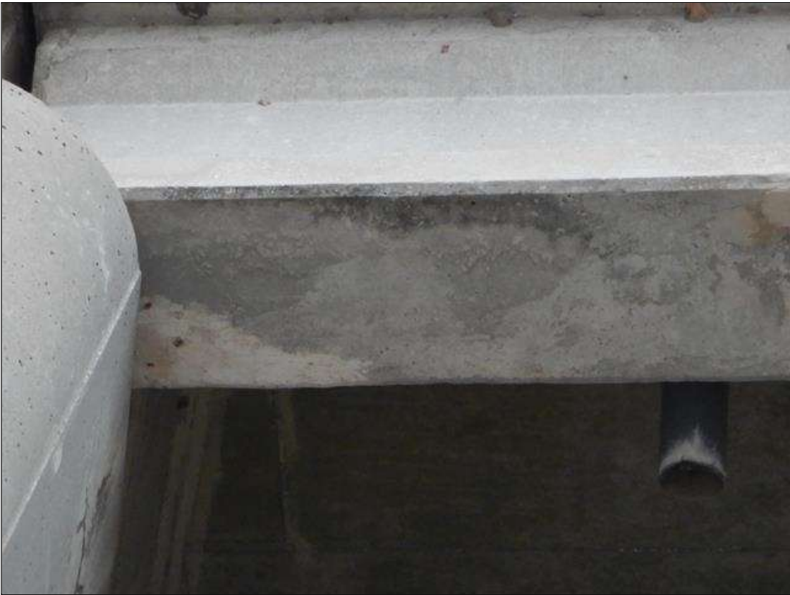
Span 9 Beam 9: [NEW REPAIR - PATCHING] FORMERLY --> (20" x 20") area of failed repair, DELAMINATION and up to 0.025" longitudinal cracking on the bottom face at 4ft from bent 8
