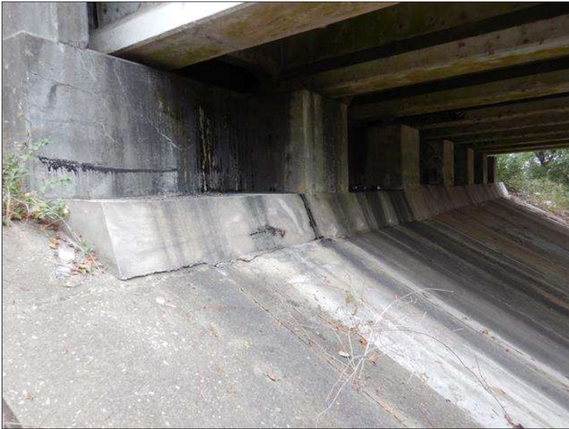
End Bent 1 Cap 1: [NEW REPAIR - CONCRETE PLACED] FORMERLY --> PRIORITY MAINTENANCE - undermining of the cap for its full length and up to its full width, fill has been lost from underneath the cap, no obvious fill has been lost from behind the End Bent
