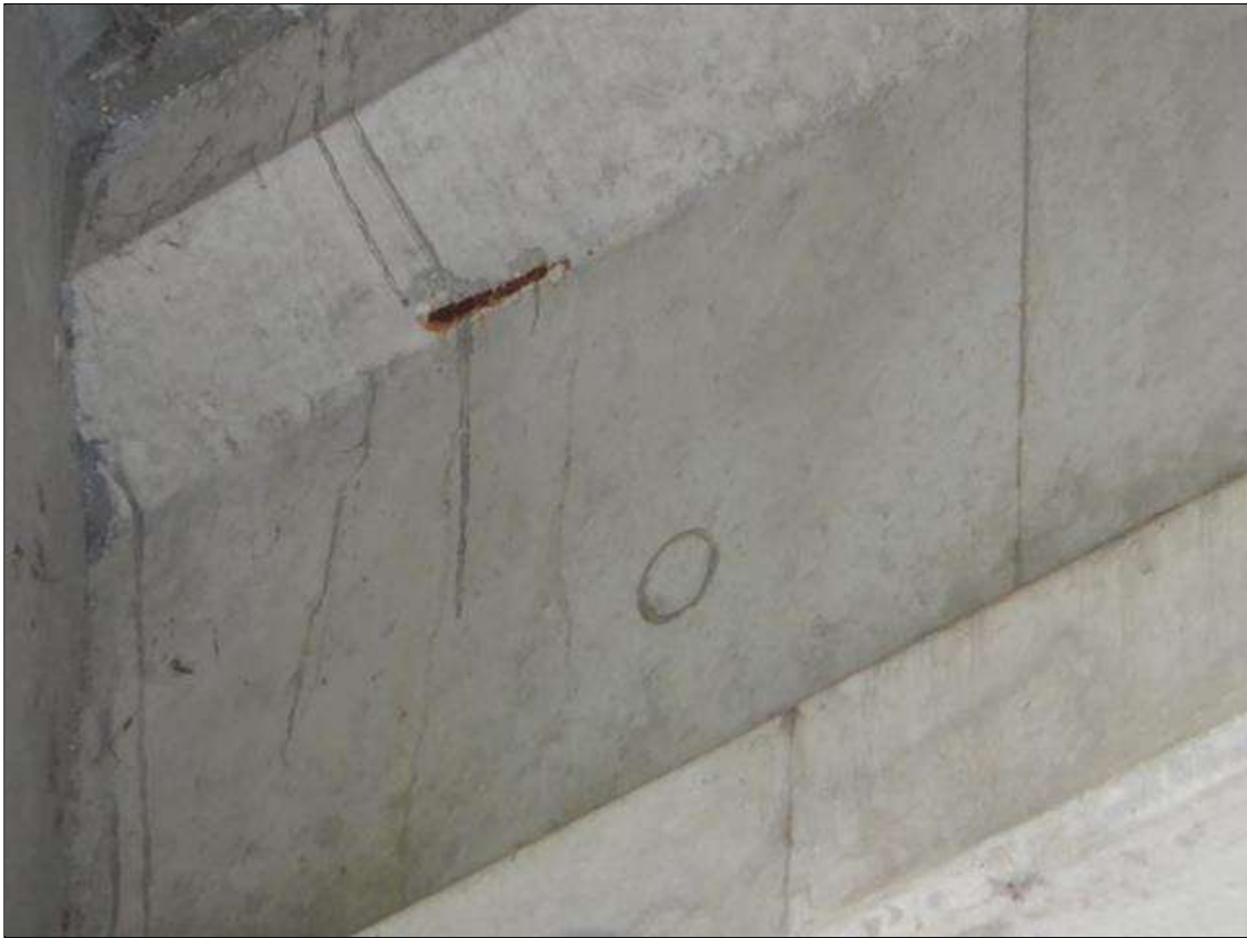
Span 32 Beam 10: [PROMPT ACTION REQUEST] spall with exposed rebar on the top right flange at 3ft from Bent 29 (4" x 1 1/2" x 1/8")
