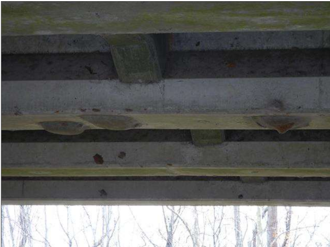
Span 2 Beam 7: [NEW REPAIR - PATCHING] FORMERLY --> (x3) spalls with exposed rebar on the bottom face at 18ft from bent 1 up to (6" X 5" X 1/2")
