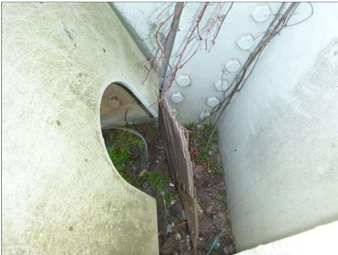
Span 18 Lift Span L6 NORTH: DIRT AND DEBRIS BUILDUP ON TOP OF BOTTOM CHORD.
