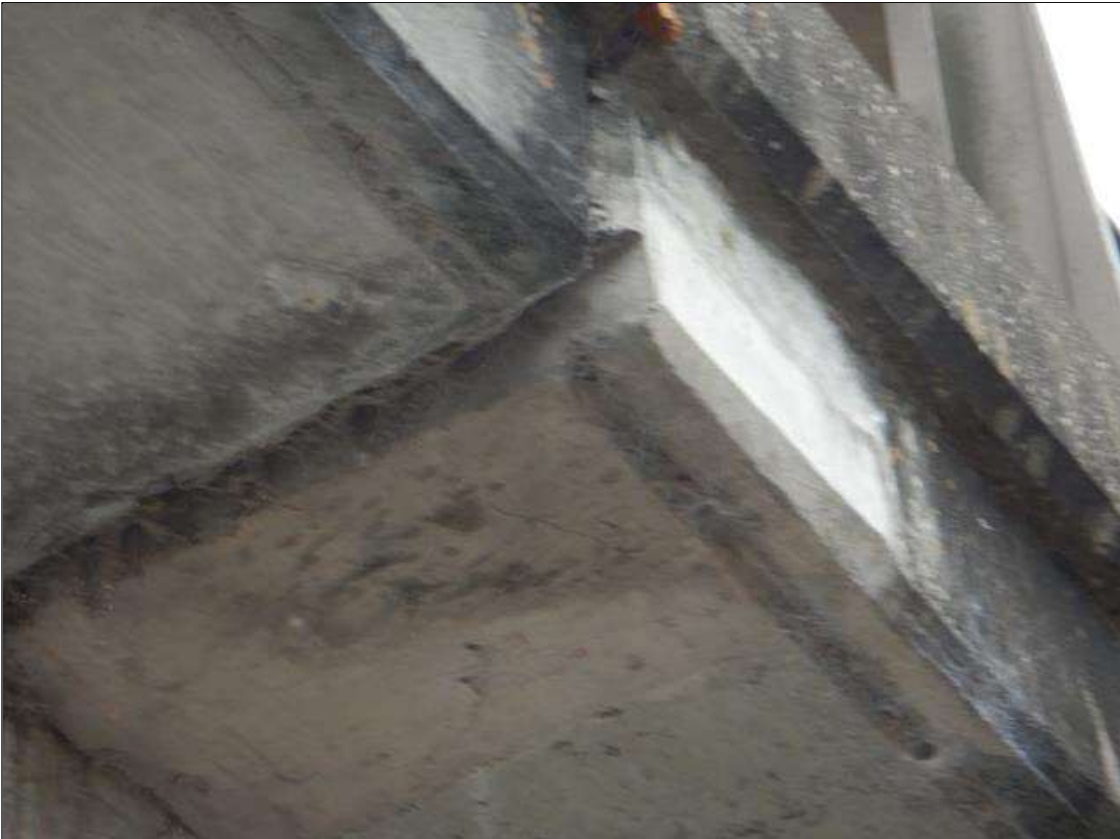
Span 1 Deck: [NEW REPAIR - PATCHING] FORMERLY --> spall with exposed rebar on the bottom of the left overhang at bent 1 (23" x 14" x 4 1/2")
