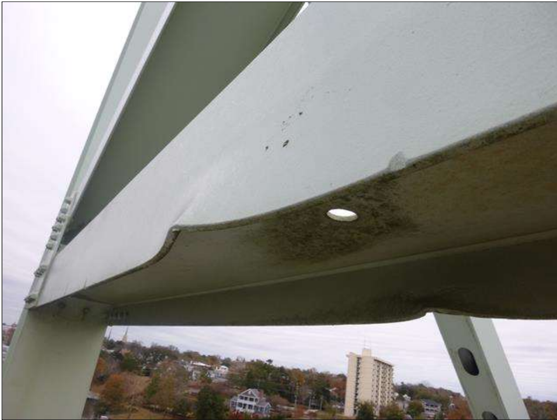
Span 18 Lift Span LB9: 1 3/4" DEEP X 9" LONG IMPACT DAMAGE TO EAST AND WEST FLANGE OVER RIGHT EAST BOUND LANE, LOCATED 7.67' FROM L9-U9 NORTH VERTICAL.
