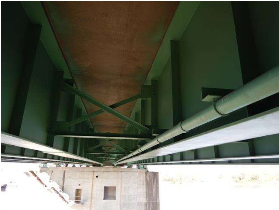
SPAN 20 BAY 3, A 4" STEEL PIPE HANGS FROM STEEL SUPPORTS, FULL SPAN LENGTH
