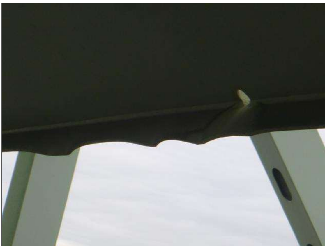
Span 18 Lift Span LB11: BOTTOM SWAY BRACE END PORTAL DAMAGE 3' WIDE X 1-1/2" DEFORMATION OVER LEFT WEST BOUND LANE.
