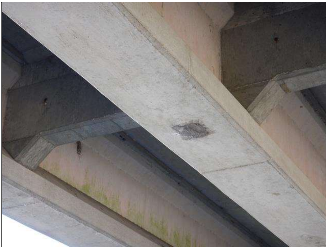
Span 28 Beam 2: sound patch on the bottom face, 10" x 10", at 1/3 point
