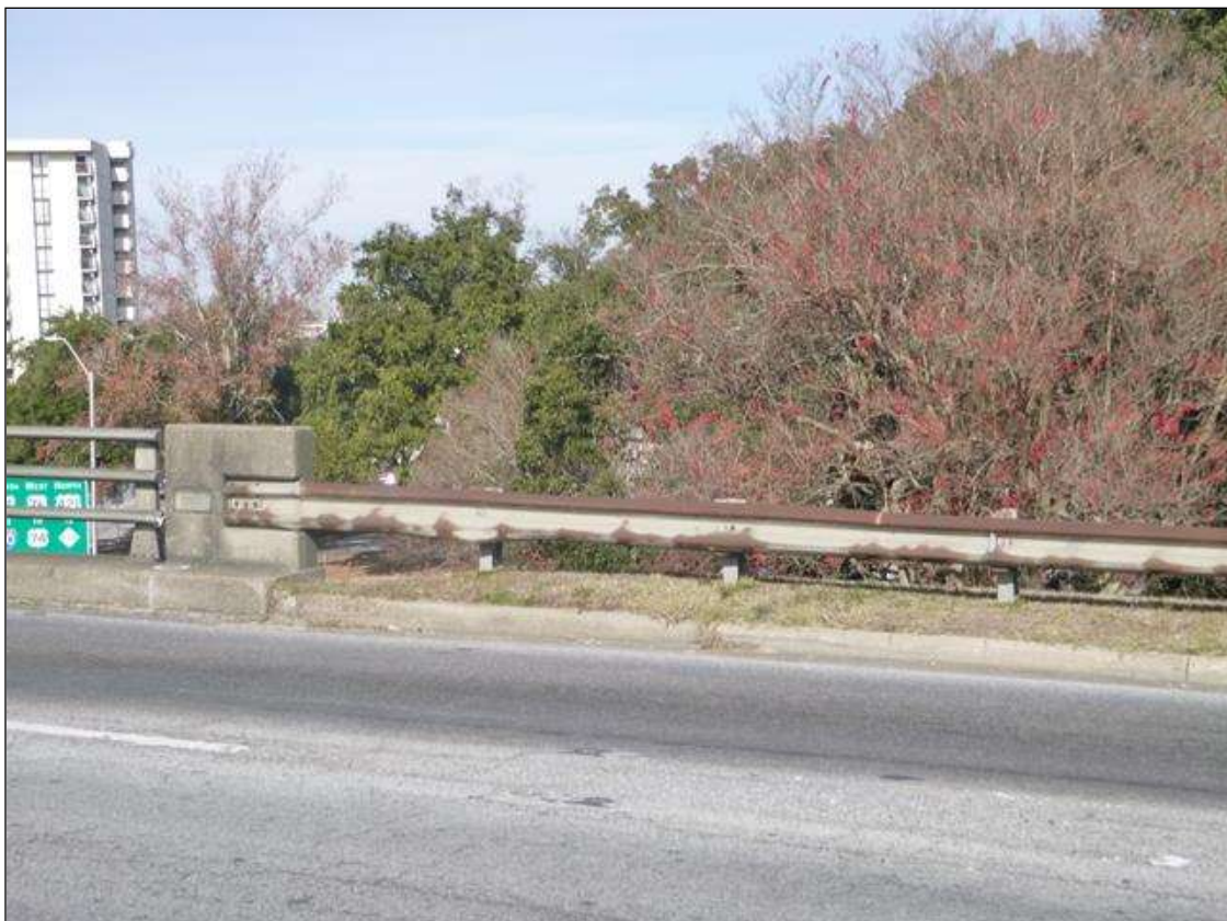
NORTHEAST CORNER, GUARDRAIL TRANSITION AND CONNECTION
