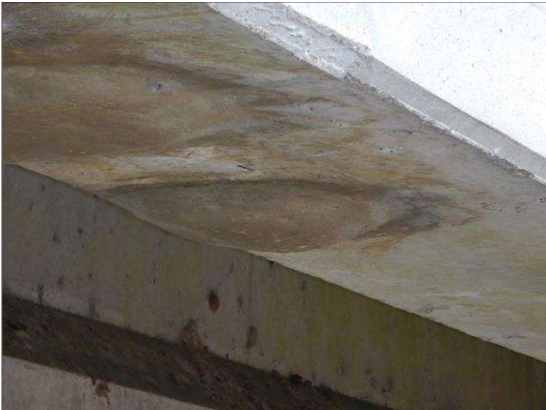
Span 2 Beam 1: [NEW REPAIR - PATCHING] FORMERLY --> spall with exposed rebar on the bottom face at 26ft from bent 1 (10" x 6 1/2" x 1/2")
