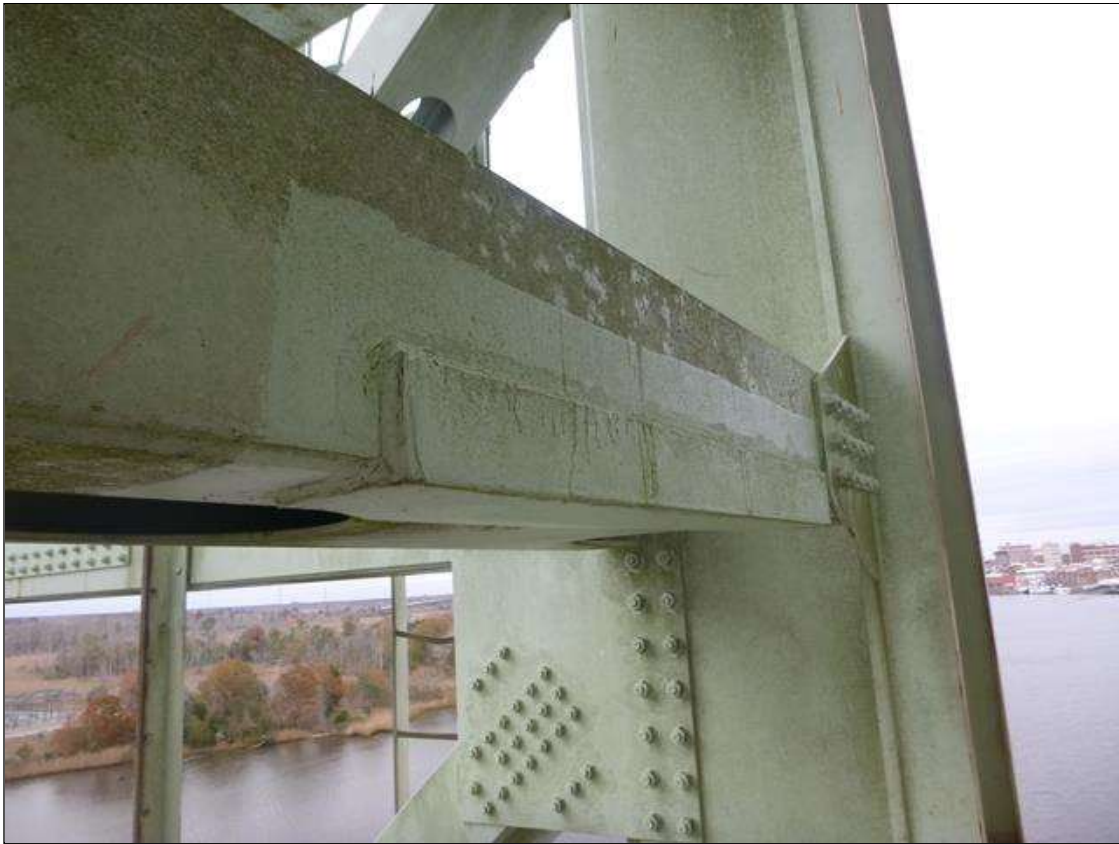
Span 17 WEST TOWER NORTH: HORIZONTAL AT NORTH EAST TOWER LEG 46" LONG 6" X 4" X 3/8" ANGLE REPAIR TO EAST FACE AND BOTTOM BEGINNING 1' FROM NORTHEAST TOWER LEG
