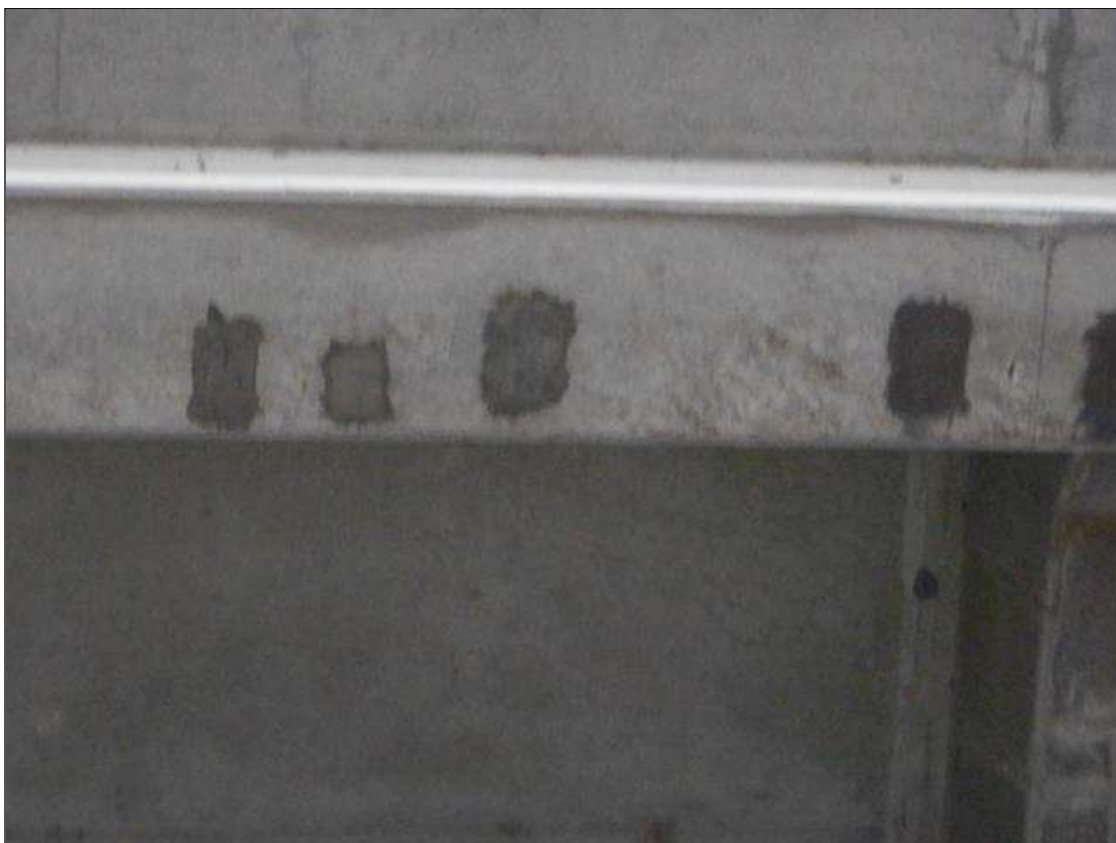
Span 10 Beam 9: [NEW REPAIR - PATCHING] FORMERLY --> (x4) spalls with exposed rebar on the bottom face at mid span up to (12" x 2" x 1/4")
