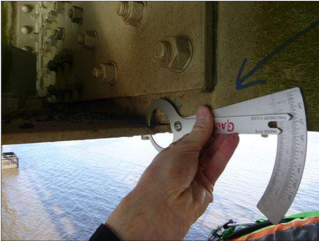
Span 18 Lift Span L10 NORTH: BOTTOM LATERAL GUSSET AT L10 NORTH- 1" WIDE X 4" LONG AREA ON EAST SIDE AT BOTTOM CHORD HAS 1/4" SECTION LOSS WITH 1/4" REMAINING, PAR ISSUED.
