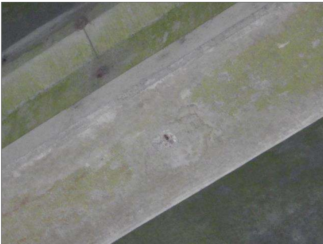
Span 4 Beam 3: (4" x 3" x 1/8") spall with exposed rebar on the bottom face 28ft from bent 3
