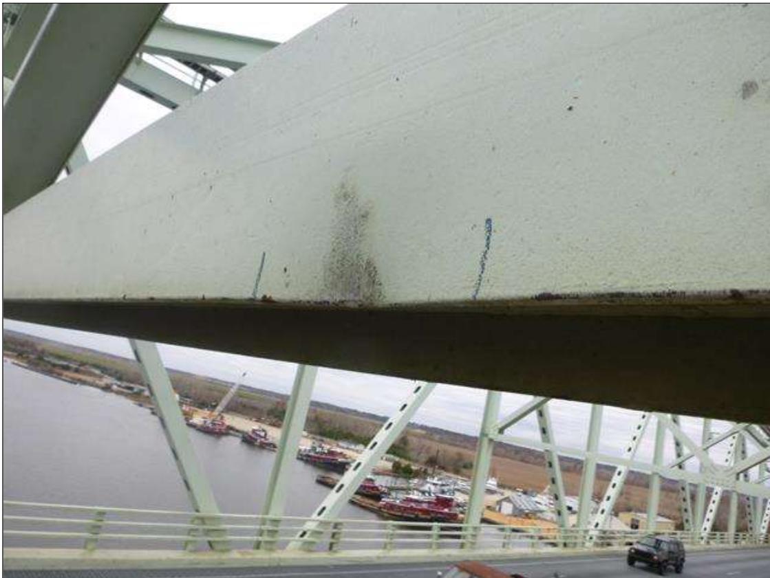
Span 18 Lift Span LB9: IMPACT DAMAGE 8" WIDE X 3/4" DEFORMATION ON EAST BOTTOM FLANGE OVER RIGHT EAST BOUND LANE 12.5 FEET FROM L9-U9 NORTH.
