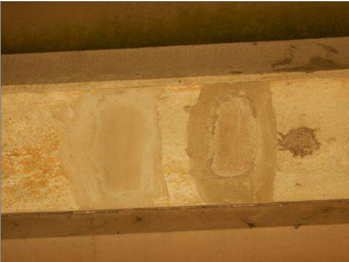
Span 30 Beam 10: [NEW REPAIR-PATCHING] FORMERLY --> (x3) spalls with exposed rebar on the bottom face at 20ft from ben 28 up to (10" x 3" x 1/4")
