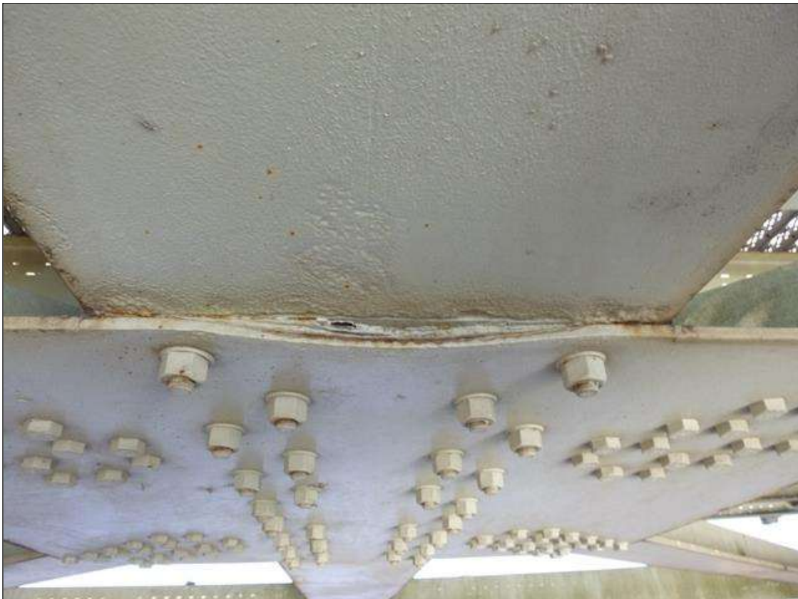
Span 18 Lift Span Floor Beam 3: 3/4" PACK RUST BETWEEN BOTTOM FLANGE AND CENTER BOTTOM LATERAL GUSSET - SOUTH SIDE
