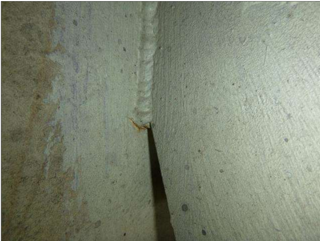
Span 18 Lift Span Stringer 3: BETWEEN FB's 1-2 - 1" CRACK IN WEB ACROSS BOTTOM OF WELD AT DIAPHRAGM CONNECTION - PROMPT ACTION REQUEST
