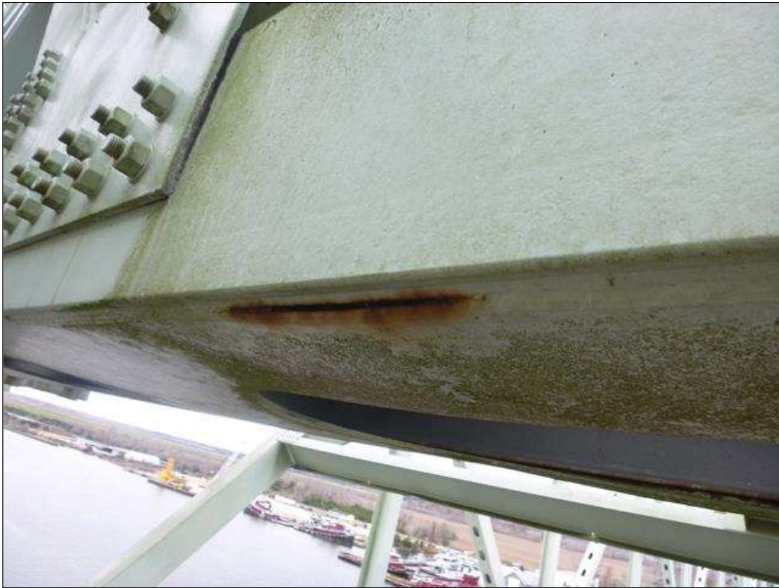
Span 19 EAST TOWER NORTH: CRACK - BOTTOM WEST HORIZONTAL TRUSS MEMBER - CRACK ALONG WELD AT BOTTOM EAST CORNER 9" LONG LOCATED 24' FROM NORTHWEST TOWER LEG (PAR)
