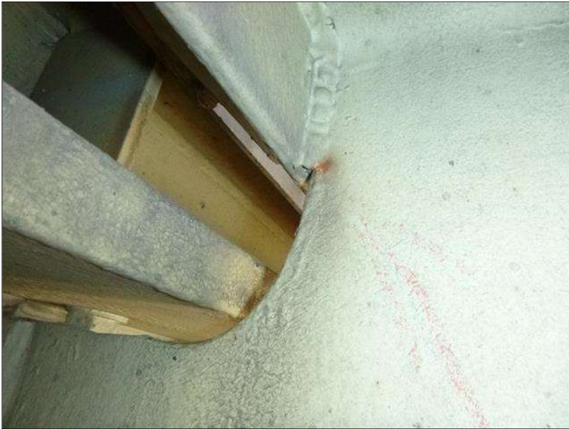
Span 18 Lift Span Stringer 13: LONGITUDINAL CRACK, 1/4" LONG IN THE TOP OF THE WEB AT THE WELD AT FE 12, PAR ISSUED.
