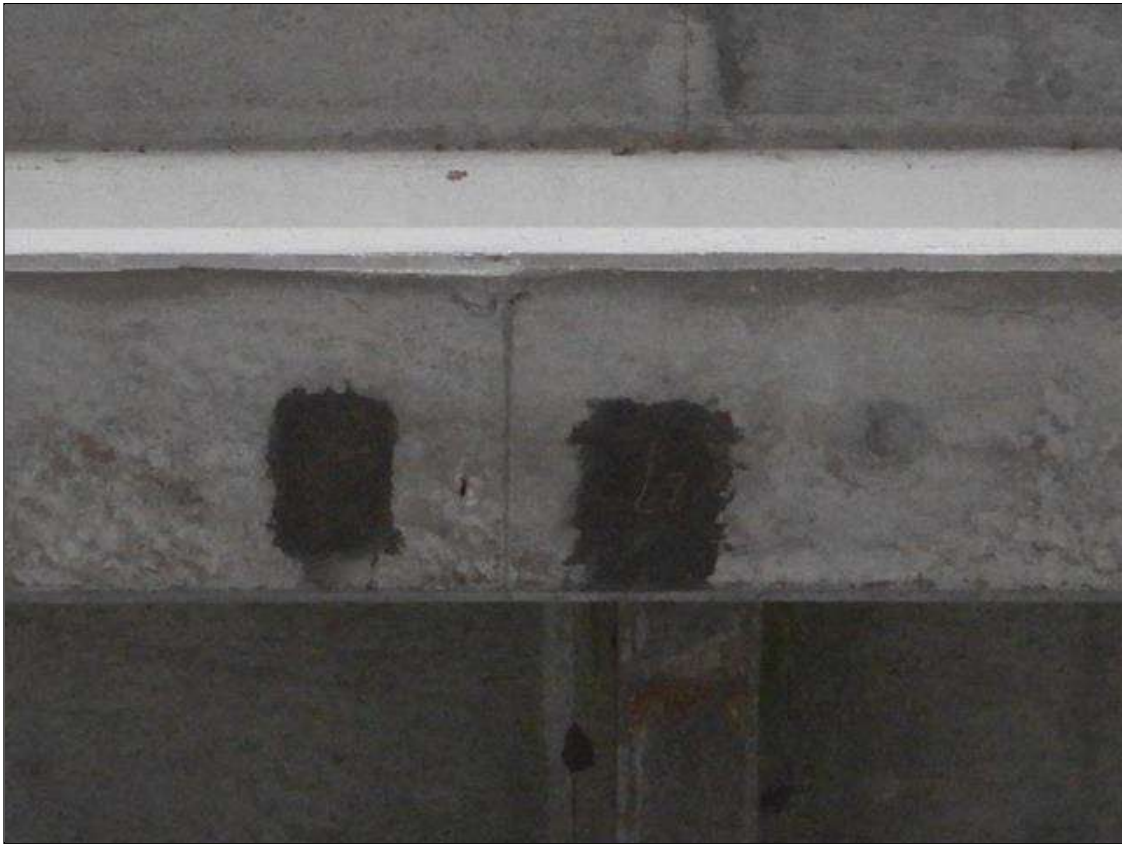
Span 10 Beam 9: [NEW REPAIR - PATCHING] FORMERLY --> (4" x 4" x 1/4") spall with exposed rebar on the bottom face at 11ft from bent 10
