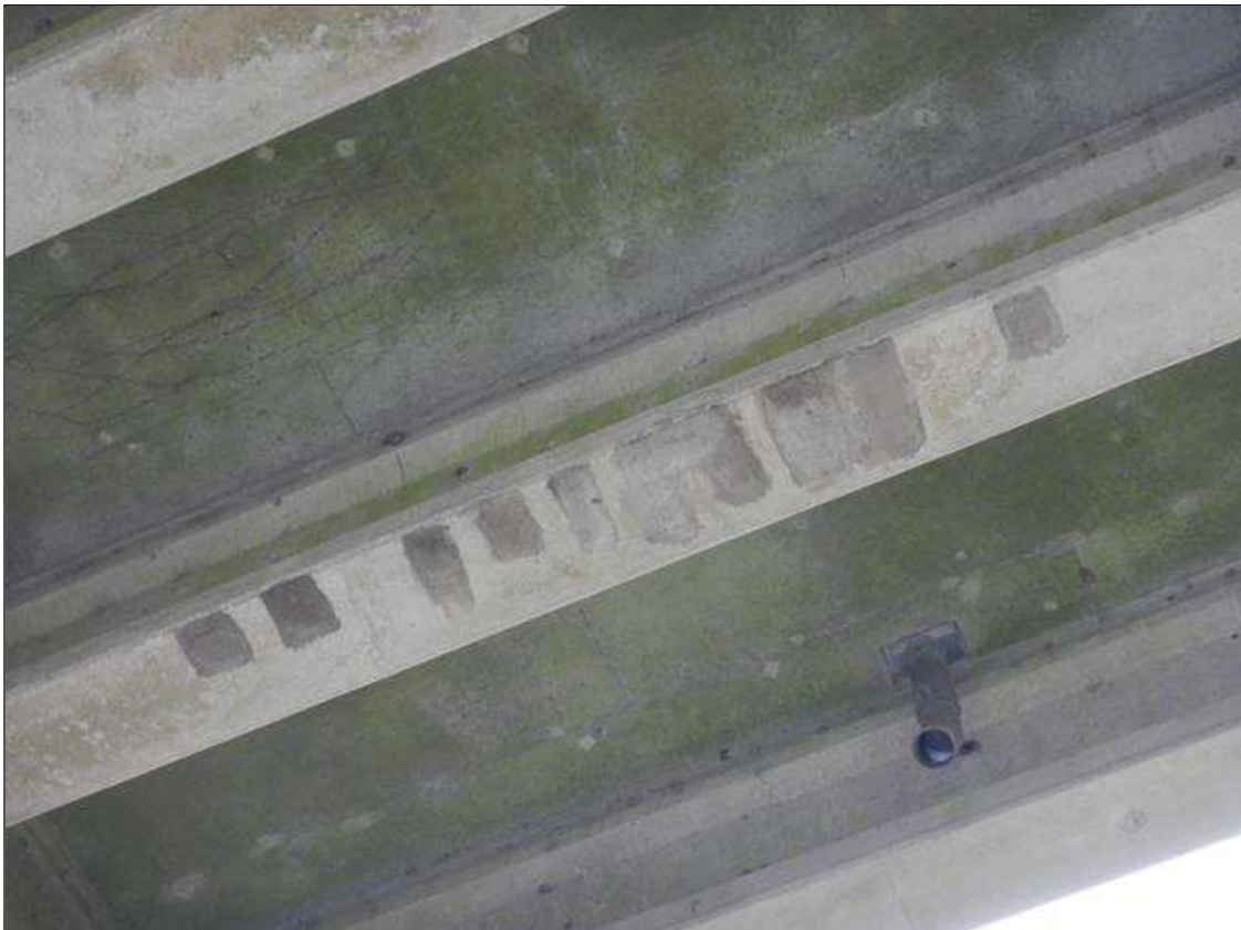
Span 5 Beam 2: [NEW REPAIR - PATCHING] FORMERLY --> (x9) spalls with exposed rebar on the bottom face at mid span up to (12" x 2" x 1/2")
