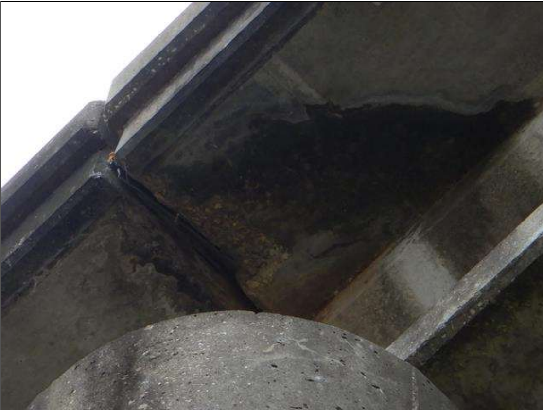
Span 4 Deck: [NEW REPAIR - PATCHING] FORMERLY --> spall with exposed rebar on the left overhang at bent 4 (17' x 6" x 3")
