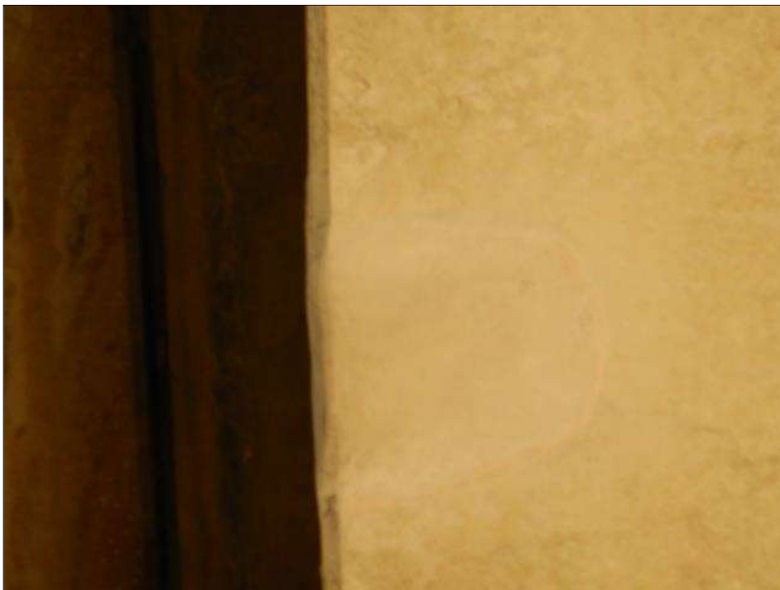
Span 30 Beam 7: [NEW REPAIR-PATCHING] FORMERLY --> failed patch on the bottom face at 25ft from Bent 27 exposing steel (6" x 6" x 1/2")
