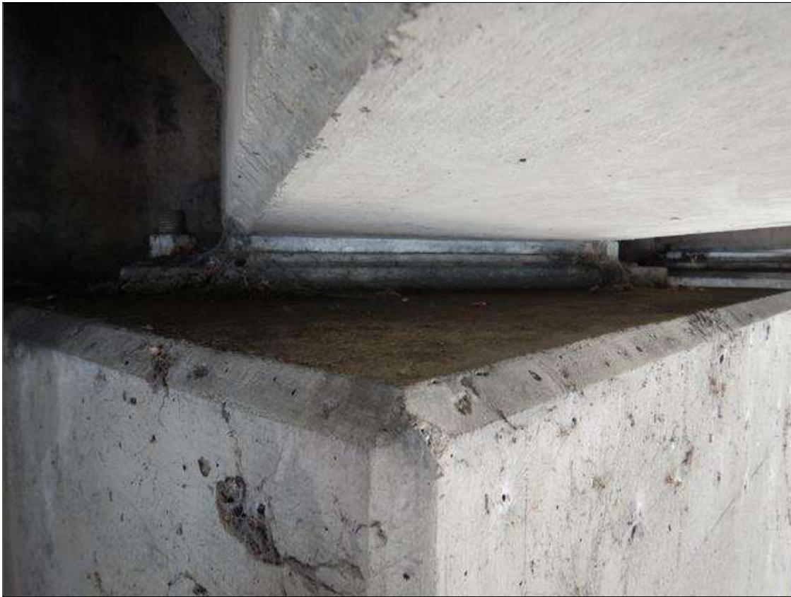
SPAN 32 GIRDER 6 FAR BEARING [SIMILAR FOR ALL SPAN 32 NEAR AND FAR BEARINGS FROM GIRDERS 2-11]
