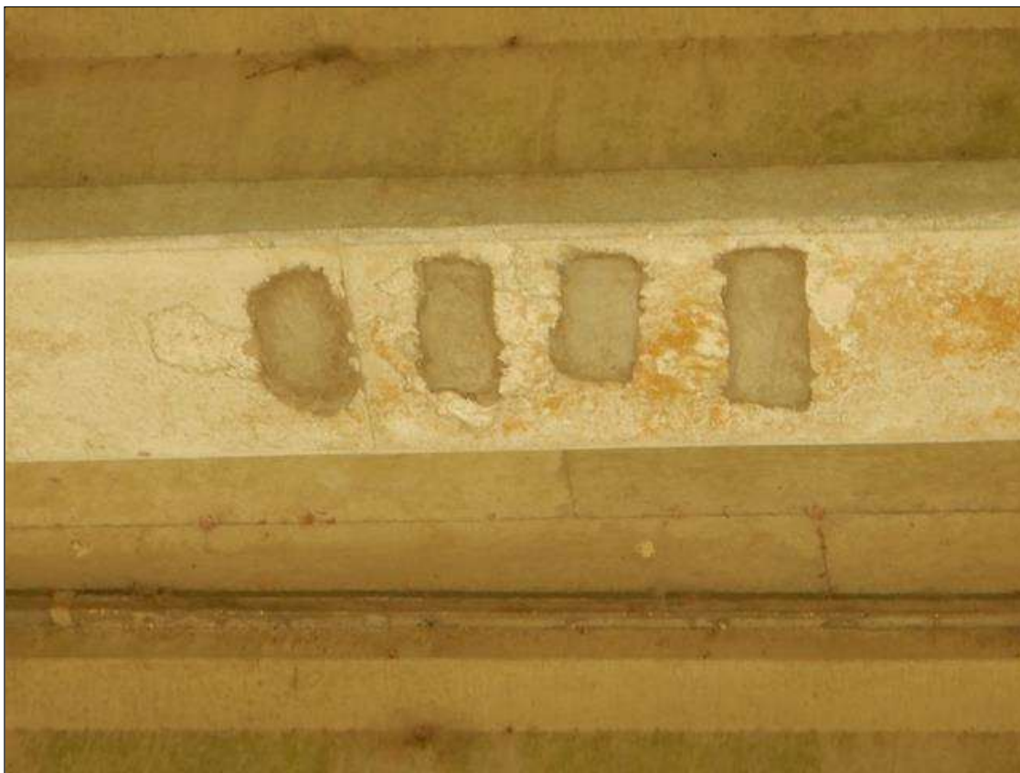
Span 27 Beam 11: [NEW REPAIR-PATCHING] FORMERLY --> (x4) DELAMINATION areas on the bottom face at mid span up to (6" x 6")
