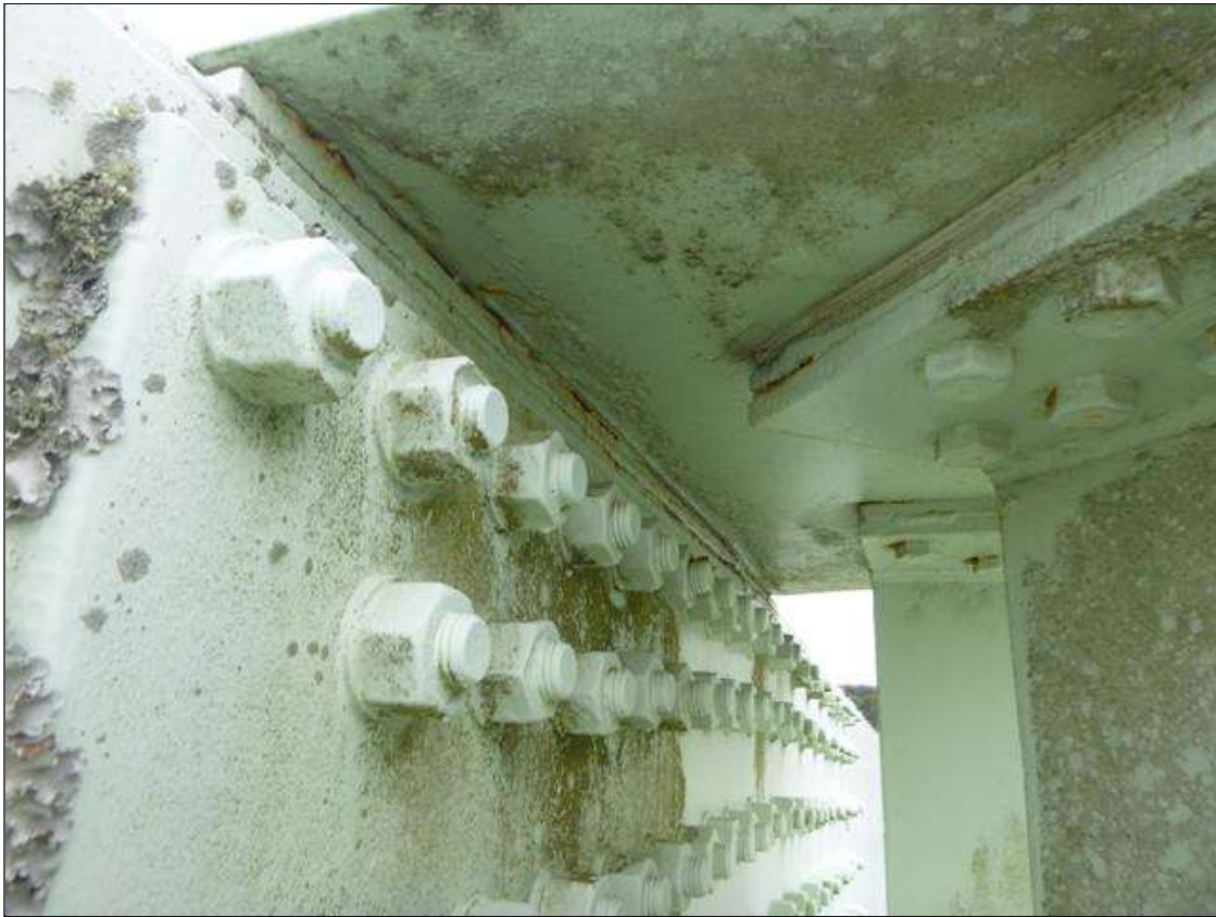
Span 18 Lift Span U9 NORTH: 35" LONG X 1-1/2" WIDE AREA 3/16" SECTION LOSS TO UNDERSIDE OF TOP GUSSET PLATE U9. (AREA IS CLEANED AND PAINTED.)
