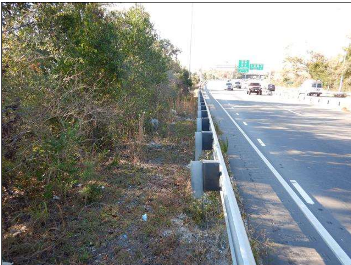
SOUTHWEST CORNER, GUARDRAIL TIED TO EXTENDED RUN [NORTHWEST CORNER SIMILAR]
