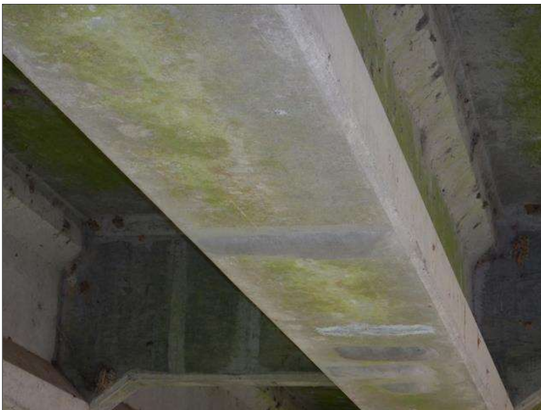
Span 3 Beam 2: [NEW REPAIR - PATCHING] FORMERLY --> (8" x 6" x 1/2") spall with exposed rebar on the bottom face at mid span
