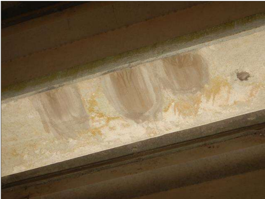
Span 29 Beam 7: [NEW REPAIR-PATCHING] FORMERLY --> (x3) spalls with exposed rebar on the bottom face at 17ft from Bent 27 up to (5" x 3" x 1/4")
