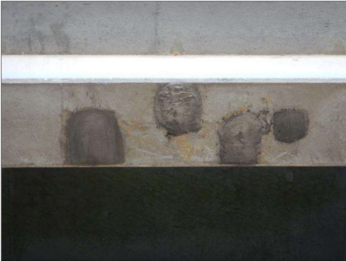
Span 28 Beam 1: [NEW REPAIR-PATCHING] FORMERLY --> (x4) spalls with exposed rebar on the bottom face near mid span up to (4" x 2 1/2" x 1/2")
