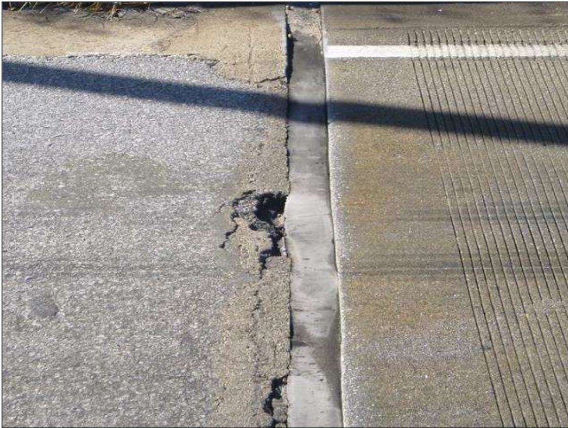
Span 35 - Ramp Span Expansion Joint: SCATTERED ALONG THE ADJACENT DECK HEADER, MAP CRACKING TO 1/4" WIDE WITH POPOFFS UP TO 8" LONG X 2" WIDE X UP TO 1.5" DEEP
