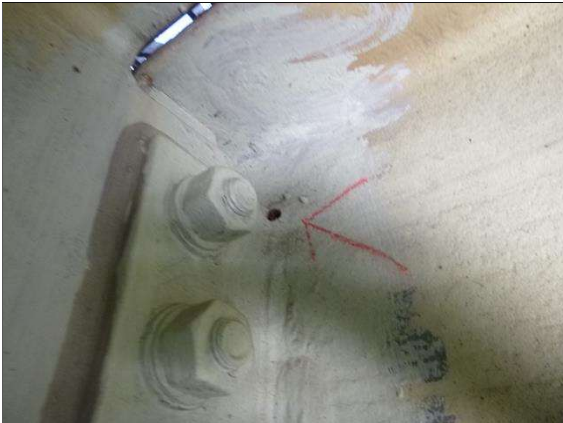
Span 18 Lift Span Stringer 7: OBSERVED IN 2020 INSP: BETWEEN FB's 4-5 - CRACK PROPAGATED 1/4" PAST ARREST HOLE ON EAST SIDE AT TOP OF DIAPHRAGM CONNECTION - PAR ISSUED.
