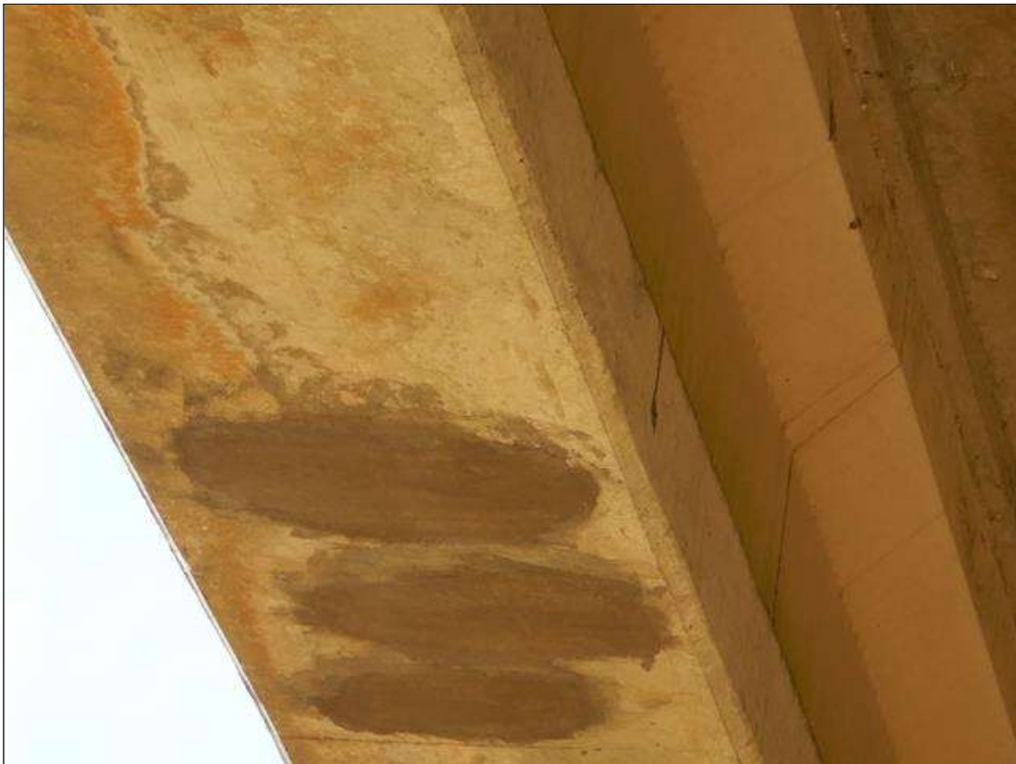
Span 30 Beam 11: [NEW REPAIR-PATCHING] FORMERLY --> spall with exposed rebar on the bottom face at 22ft from Bent 28 (12" x 6" x 1/2")
