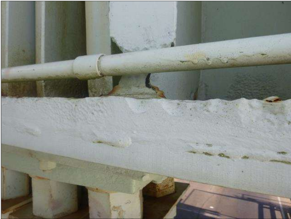
Span 18 Lift Span LB12: [PROMPT ACTION REQUEST] EASTBOUND LANE NORTHWEST CABLE BANK, RIGHT STIFFNER, COMPLETE LOSS OF SECTION 1-1/4" WIDE ON BOTH FLANGE ALONG BOTTOM 4" HIGH.
