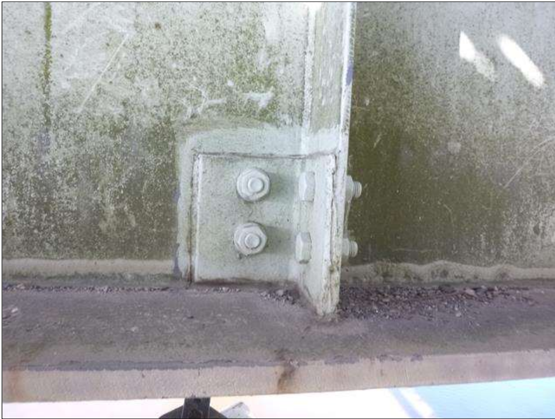
Span 18 Lift Span Floor Beam 10: FB 10, EAST SIDE, STIFFENER 9 HAS BEEN REPAIRED ADJACENT TO THE BOTTOM FLANGE, WITH A 6" X 6" X 7" HIGH X 1/2" THICK ANGLE BOLTED TO THE STIFFENER AND WEB ON THE SOUTH SIDE OF THE WEST AND EAST FACES.
