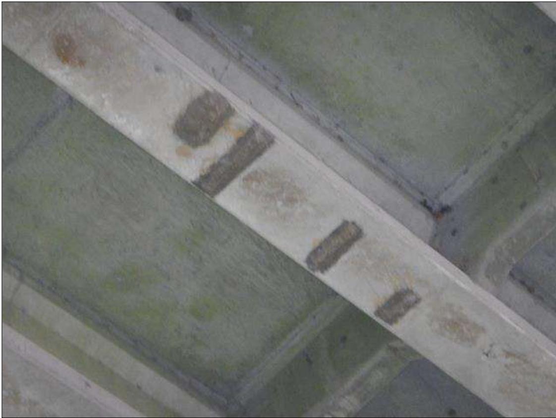
Span 6 Beam 2: [NEW REPAIR - PATCHING] FORMERLY --> (x4) spalls with exposed rebar on the bottom face starting at 22ft from bent 5 up to (16" x 5" x 1/2")
