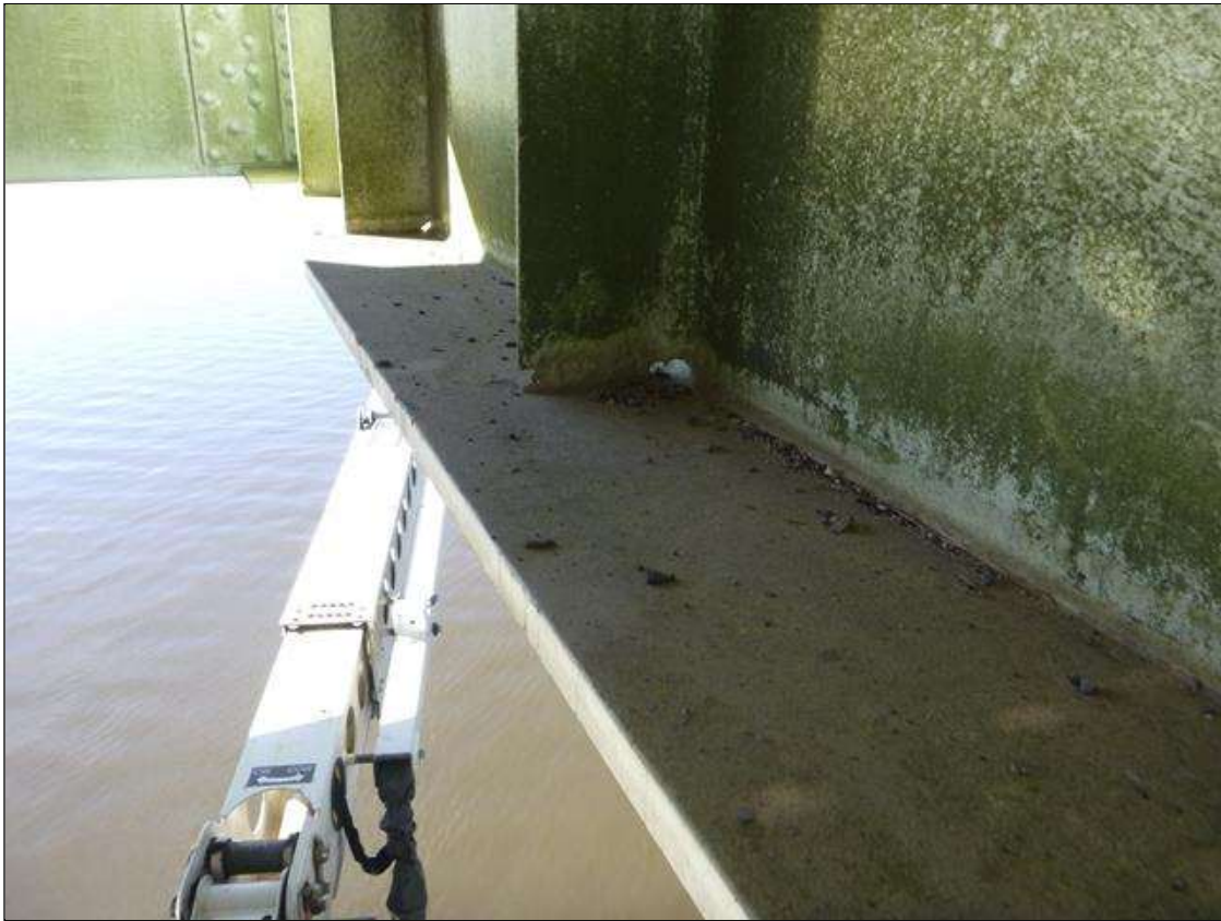
Span 18 Lift Span Floor Beam 9: VERTICAL STIFFENER 12 AND 13 ON EAST SIDE - 4" HIGH PITTED AREA AT BOTTOM FLANGE - LOWER 1" OF AREA REDUCED TO 1/16" WIDE/ ~3/4" HOLES AT EDGES - AREA CLEANED AND PAINTED
