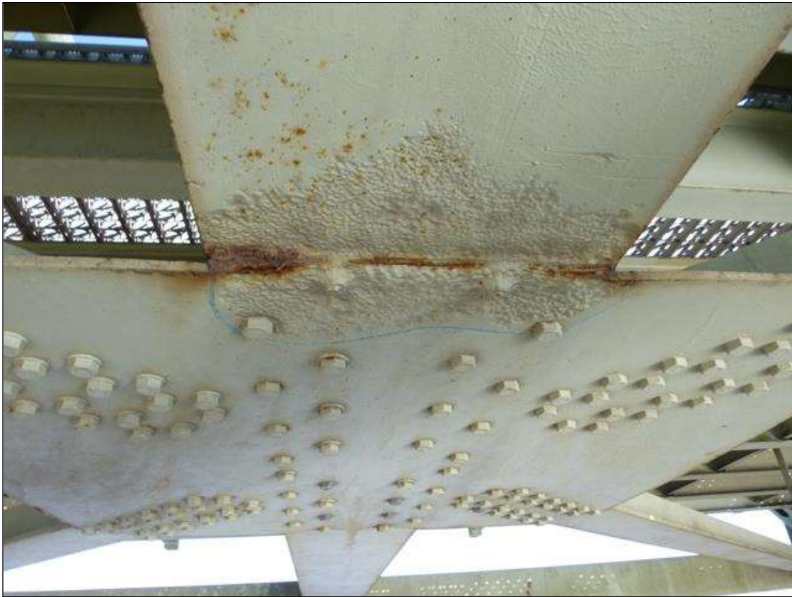
CENTER BOTTOM LATERAL GUSSET - SOUTH SIDE - UP TO 1/2" PACK RUST BETWEEN GUSSET AND BOTTOM FLANGE ON EAST AND WEST SIDES - 10"L x 4" AREA OF GUSSET AT BOTTOM FLANGE REDUCED TO 3/8" - 60% LOSS TO (2) FASTENERS.
