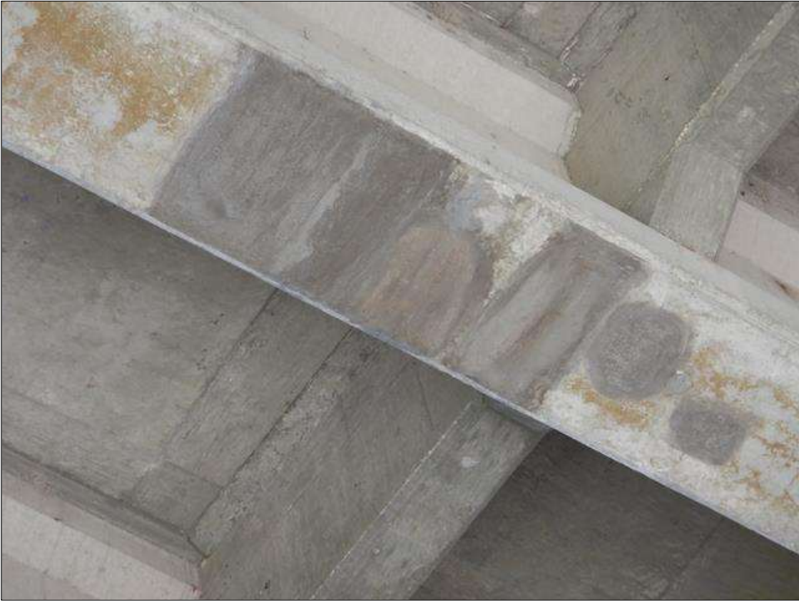
Span 28 Beam 9: [NEW REPAIR-PATCHING] FORMERLY --> multiple spalls with exposed rebar and sound patches on the bottom face up to (13" x 6" x 1/2")
