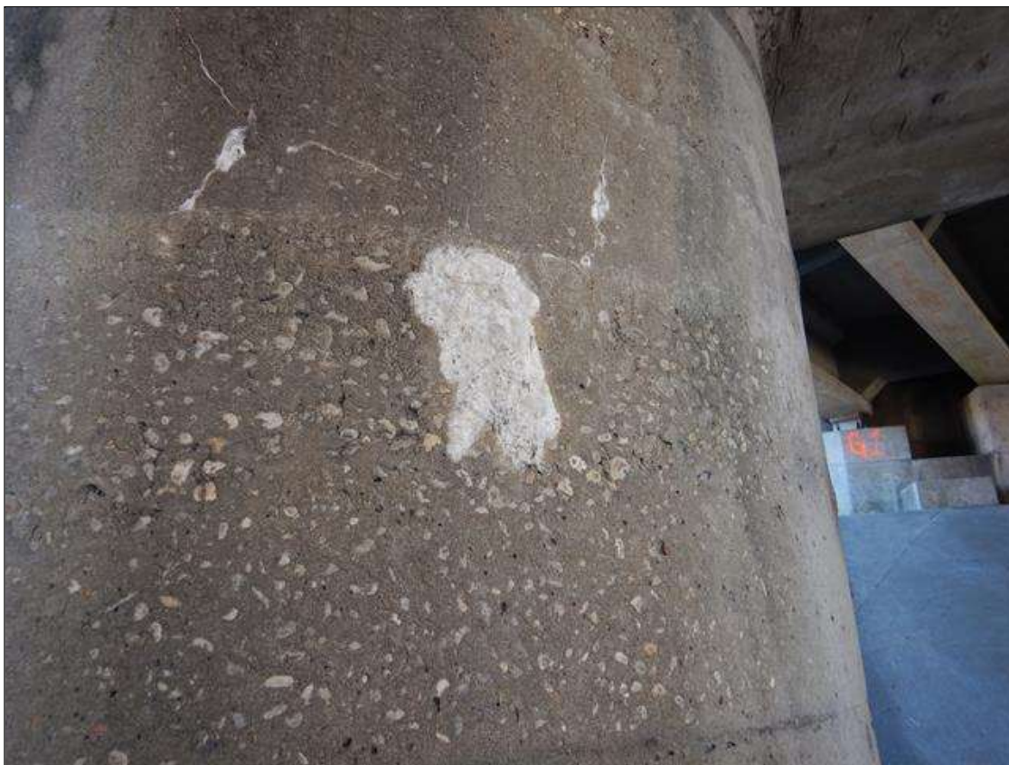
Bent 29 Pile 1: efflorescence build-up at 2ft below the cap
