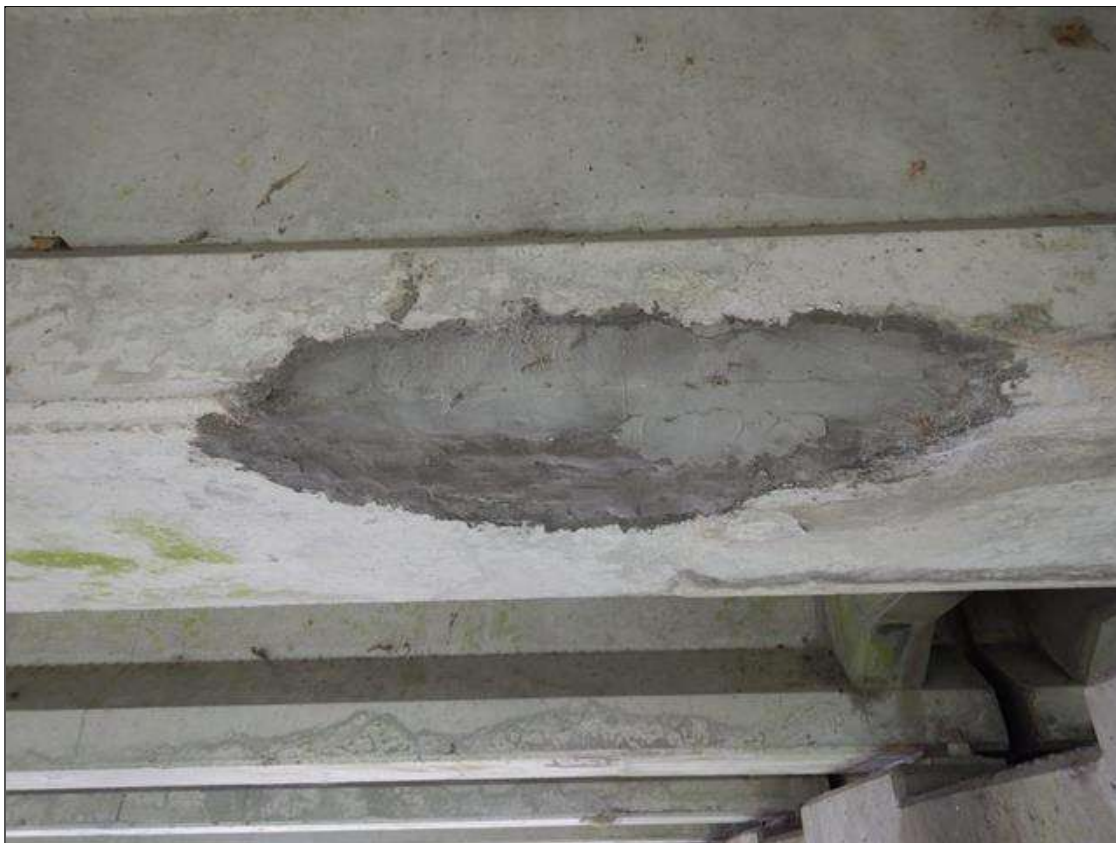
Span 3 Beam 5: sound patch on the bottom right face at 21" from bent 3, 10" wide x 30" long
