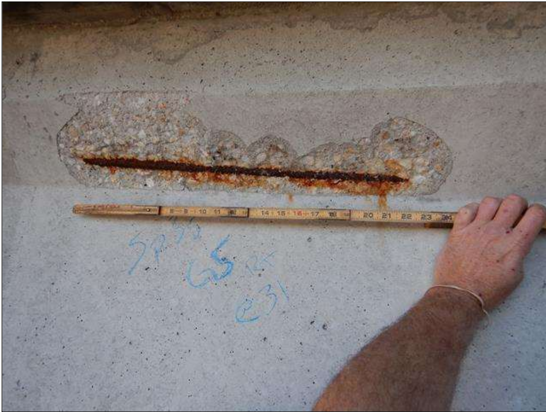
Span 35 - Ramp Span Beam 5: [PROMPT ACTION REQUEST] APPROXIMATELY 1.5' OUT FROM BENT 31, UPPER RIGHT FLANGE, SPALLING WITH EXPOSED REBAR [APPROXIMATELY 2' LONG X UP TO 5" WIDE X UP TO 1/2" DEEP]; NO MEASURABLE SECTION LOSS
