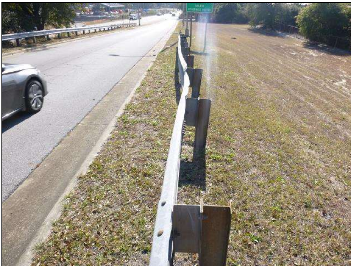
AT THE RAMP ABUTMENT SOUTHEAST CORNER GUARDRAIL, APPROXIMATELY 30' OUT FROM THE GUARDRAIL END, DAMAGE WITH FLATTENED RAIL AND POSTS DEFLECTED UP TO 6" AT THE TOP [APPROXIMATELY 18' LONG AFFECTED]
