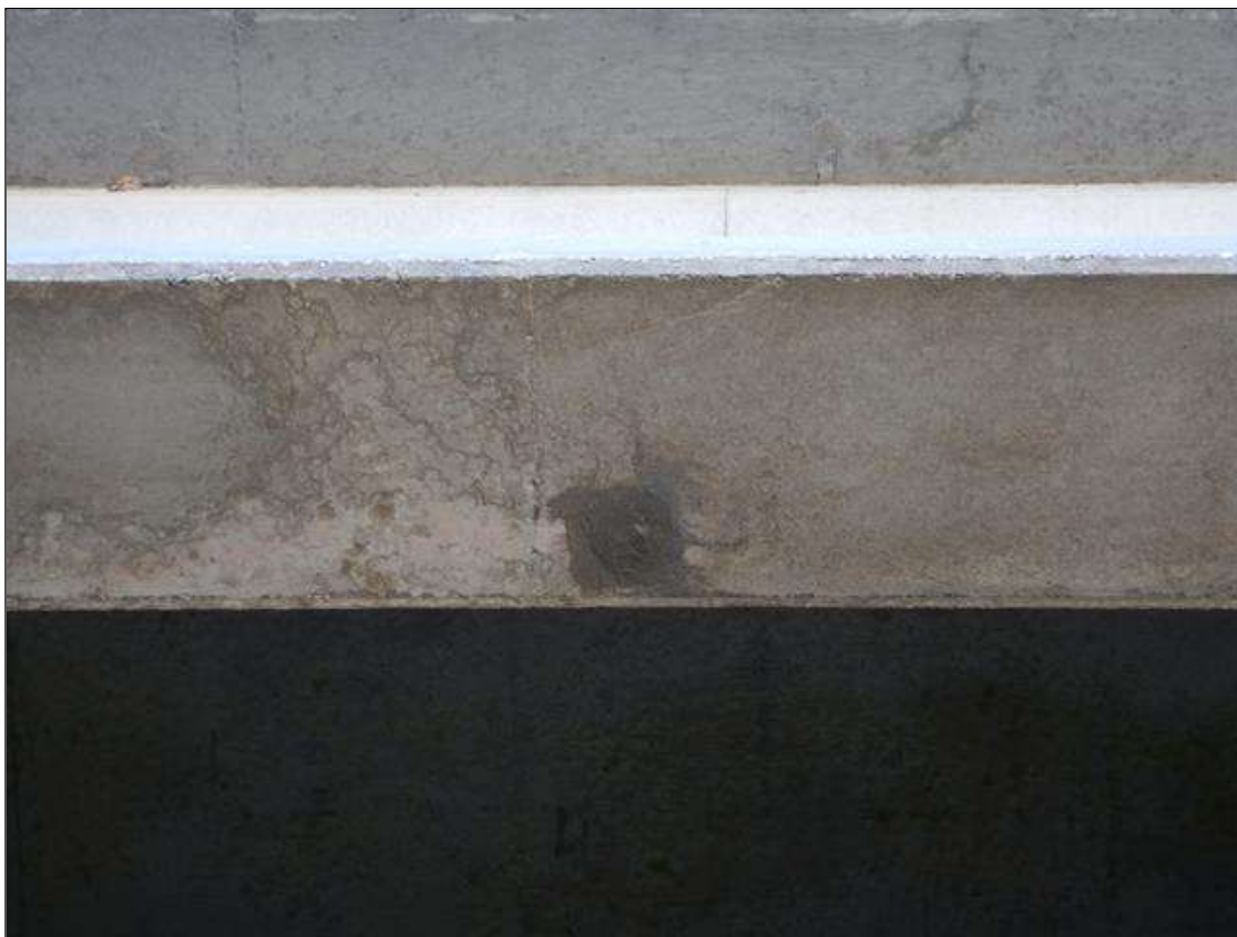
Span 28 Beam 1: sound patch on the bottom face at 12.5ft from bent 26 (7" x 6")
