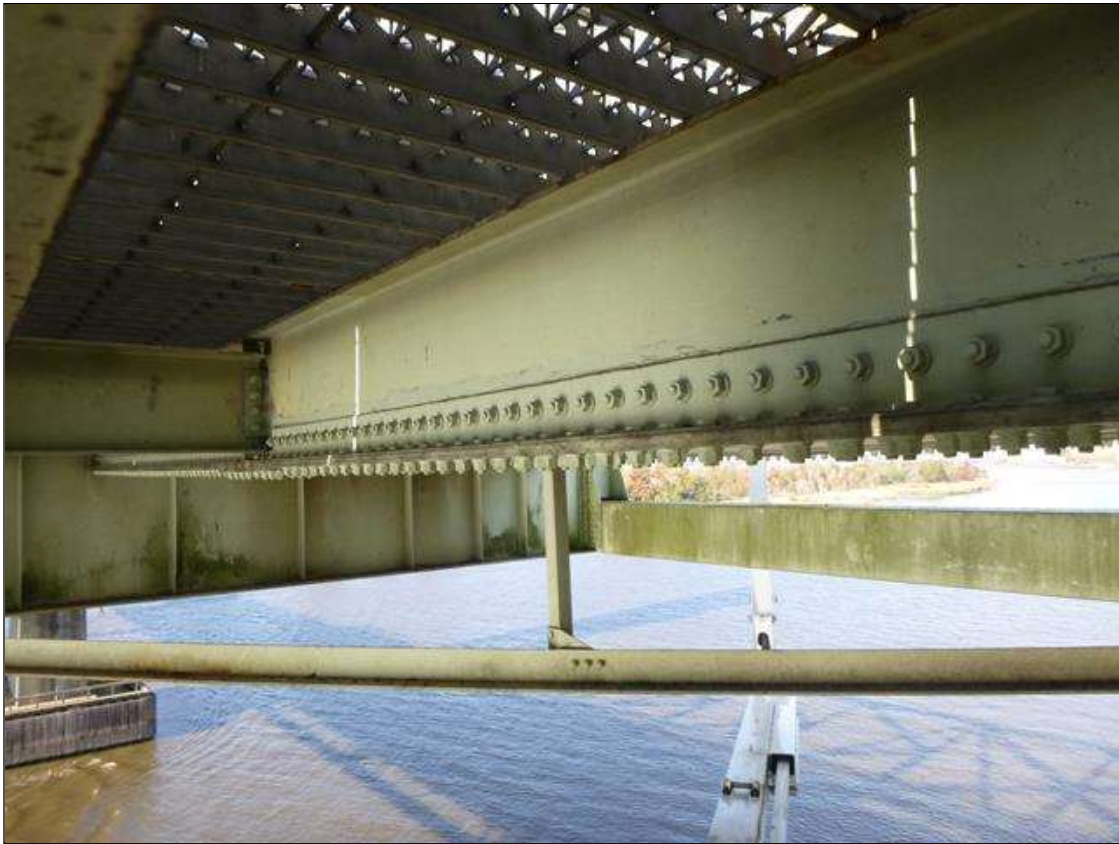
Span 18 Lift Span Stringer 5: REPAIR OBSERVED IN 2021 INSPECTION: 6" X 4" X 3/8" THICK ANGLE AND 9" WIDE X 1/2" THICK PLATE HAS BEEN BOLTED TO BOTH SIDES OF THE WEB AND BOTTOM FLANGE, FULL LENGTH 2020 REPORT HAD BETWEEN FB's 7-8 - PITTED AREAS ON WEB AT BOTTOM FLANGE ON NORTH SIDE UP TO 3"HIGH x 1/8"DEEP SCATTERED ACROSS FULL LENGTH - CLEANED AND PAINTED
