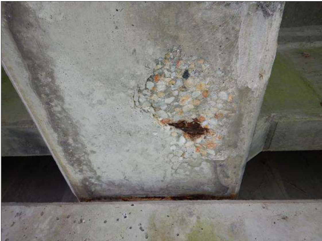
Span 3 Beam 5: [PROMPT ACTION REQUEST] GIRDER END AT BENT 3, LOWER SIDE, SPALLING WITH EXPOSED REBAR [APPROXIMATELY 8" X 10" X UP TO 1" DEEP]
