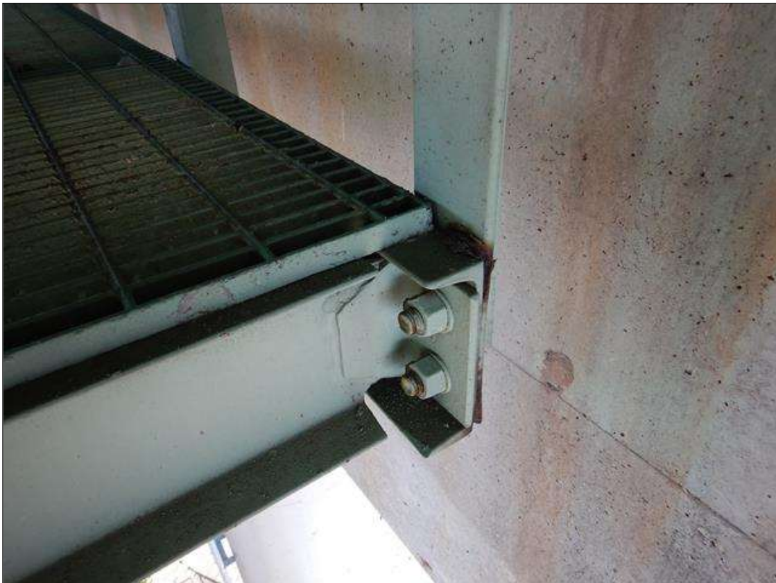
Span 16 Beam 8: Surface corrosion and with pack rust between members of the platform attached to the beams at the east face of bent 15.
