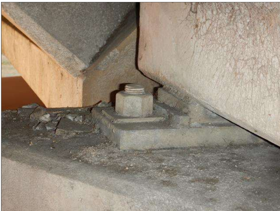
Span 32 Beam 9 - Beam 9 Far Bearing: [NEW REPAIR-NUT INSTALLED] FORMERLY --> missing right anchor rod nut
