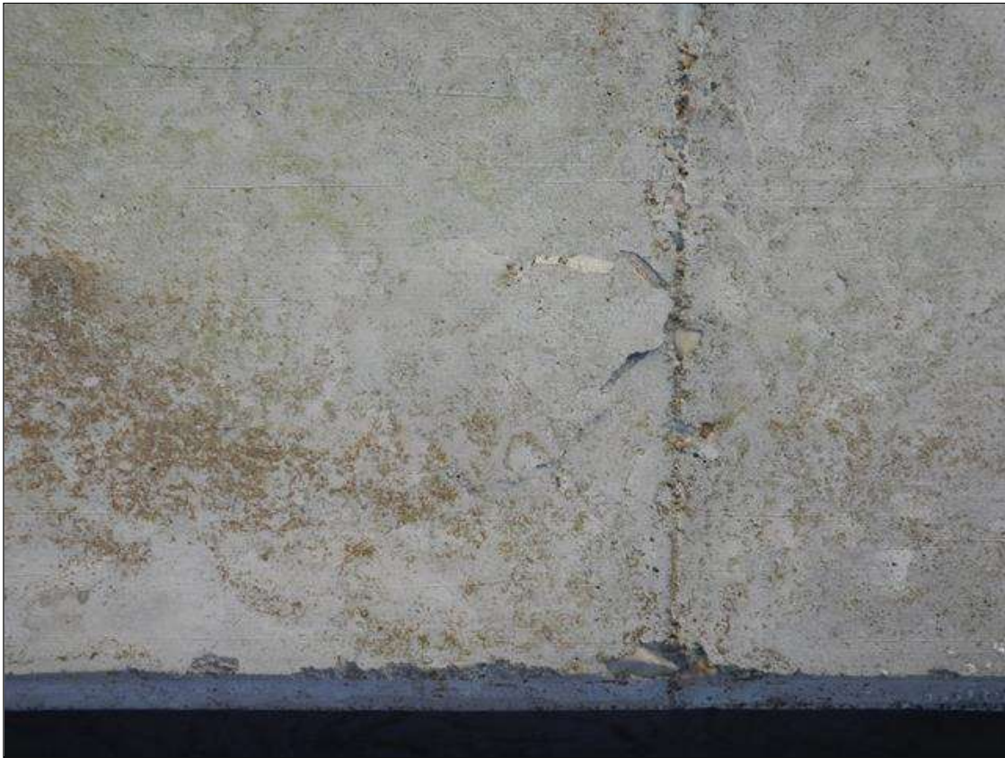
Span 35 - Ramp Span Beam 1: APPROXIMATELY 14' OUT FROM THE RAMP ABUTMENT, LOWER SIDE, DELAMINATION WITH ASSOCIATED CRACKING TO 1/8" WIDE [APPROXIMATELY 5"]
