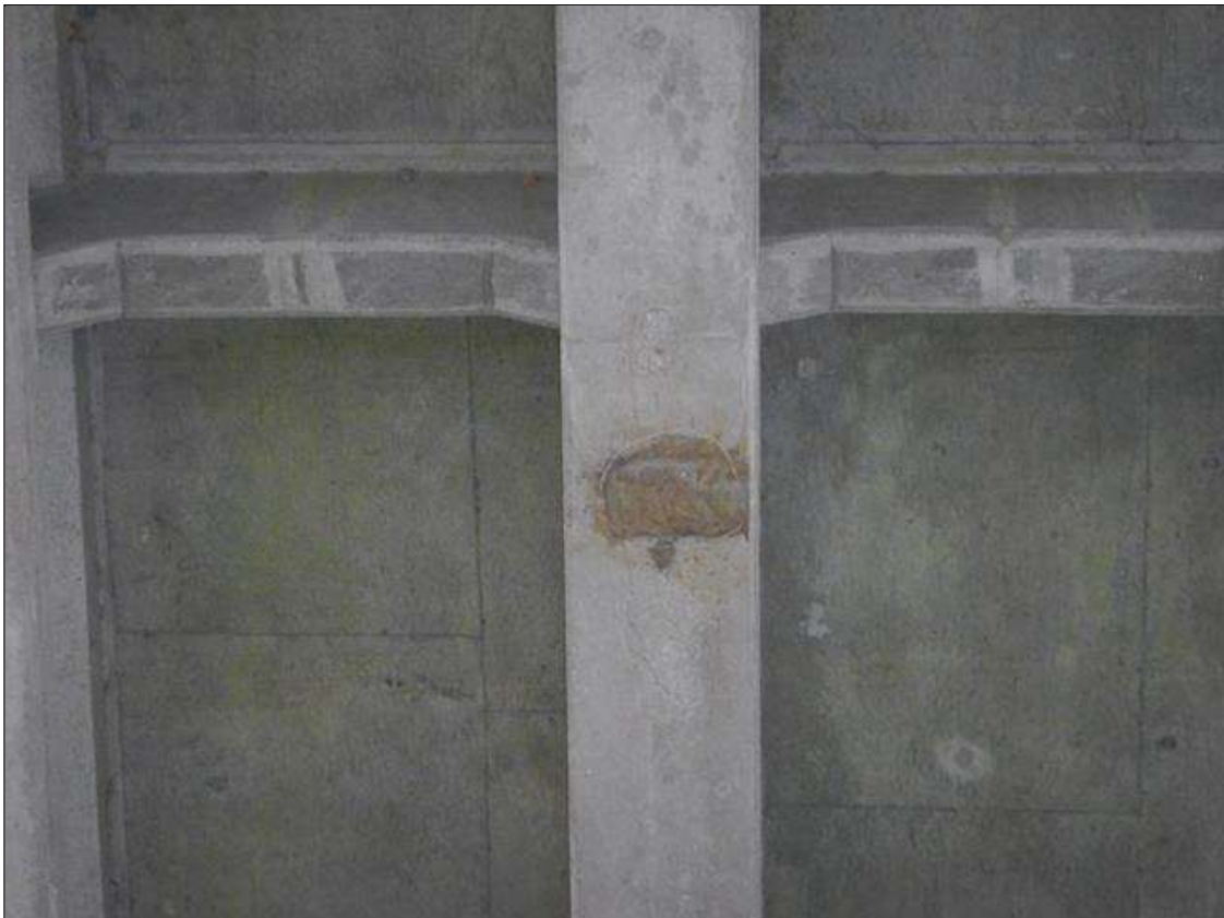
Span 8 Beam 3: [NEW REPAIR - PATCHING] FORMERLY --> (8" x 5" x 1/2") spall with exposed rebar on the bottom face at 21ft from bent 7
