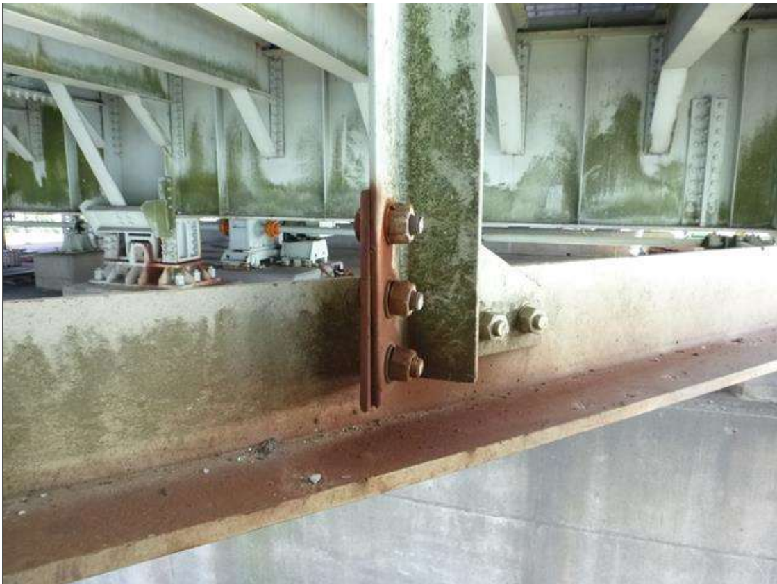
Span 18 Lift Span Floor Beam 12: LATERAL BRACING FROM FLOORBEAM 11 TO L12 AT MID LENGTH LOOSE BOLTS IN CONNECTION TO VERTICAL BRACE.
