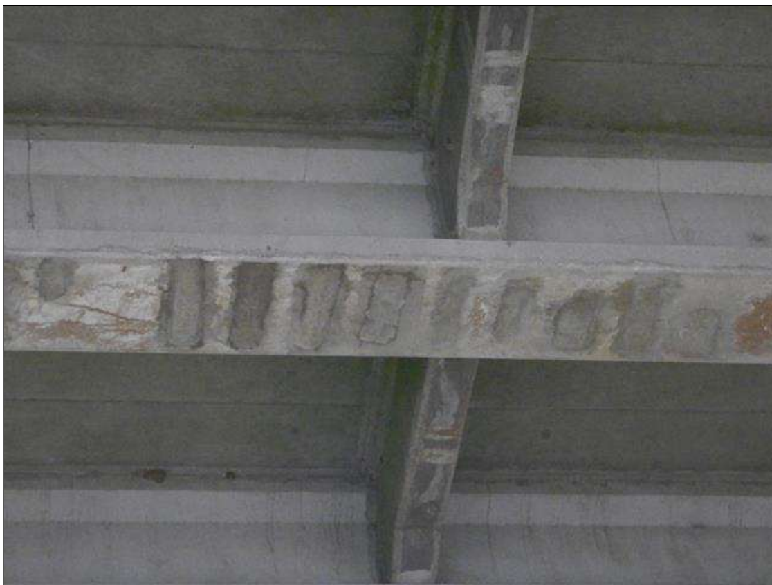
Span 10 Beam 3: [NEW REPAIR - PATCHING] FORMERLY --> multiple spalls with exposed rebar on the bottom face beginning at 17ft from bent 10 up to (12" x 2" x 1/4")
