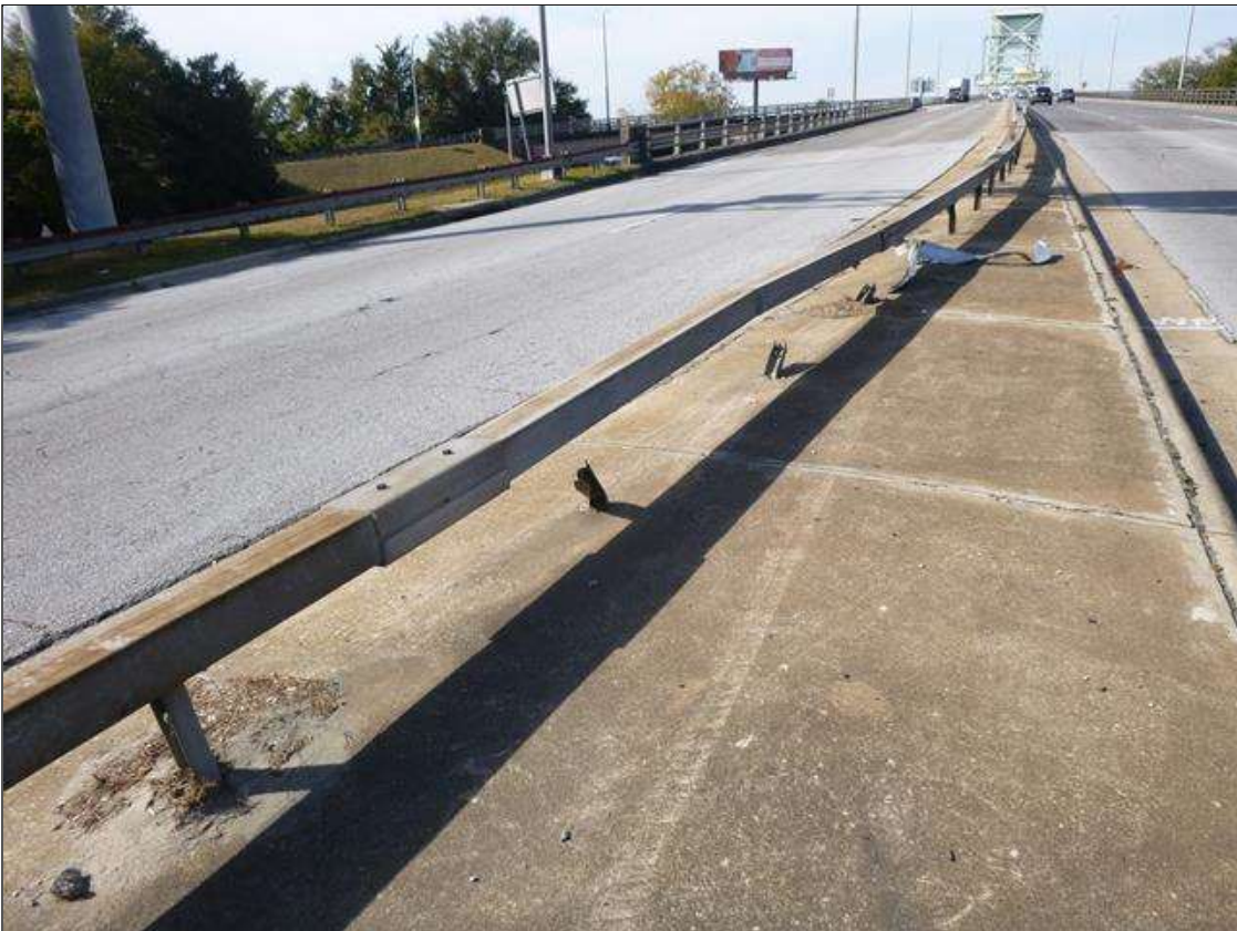
[PROMPT ACTION REQUEST] AT THE ABUTMENT 2 APPROACH, THE MEDIAN RAIL HAS IMPACT DAMAGE WITH FIVE BROKEN POSTS
