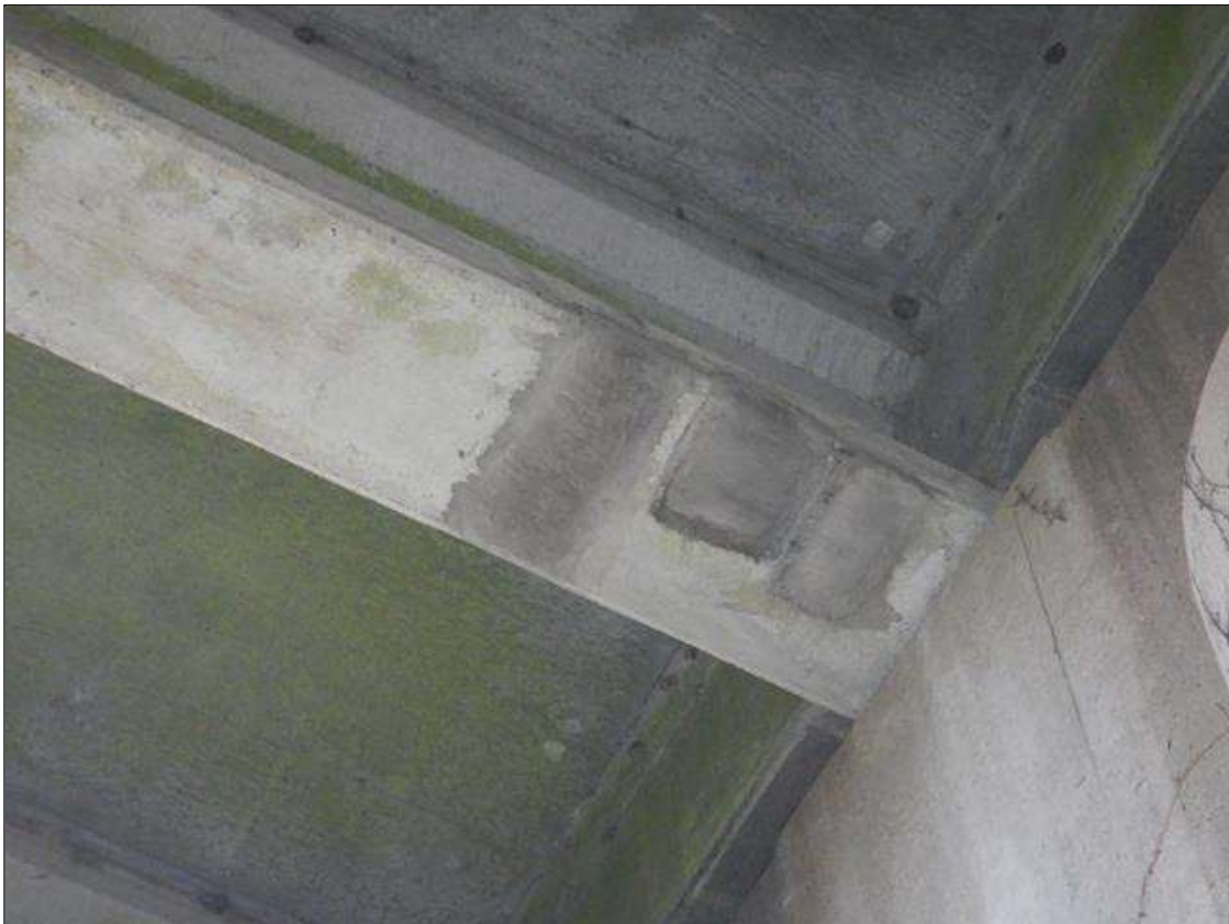
Span 5 Beam 2: [NEW REPAIR - PATCHING] FORMERLY --> (x3) spalls with exposed rebar on the bottom face at bent 5 up to (9" x 7" x 1")
