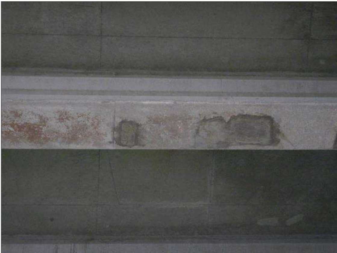
Span 10 Beam 3: [NEW REPAIR - PATCHING] FORMERLY --> (x3) spalls with exposed rebar on the bottom face at 78in from bent 10 up to (10" x 6" x 1/2")
