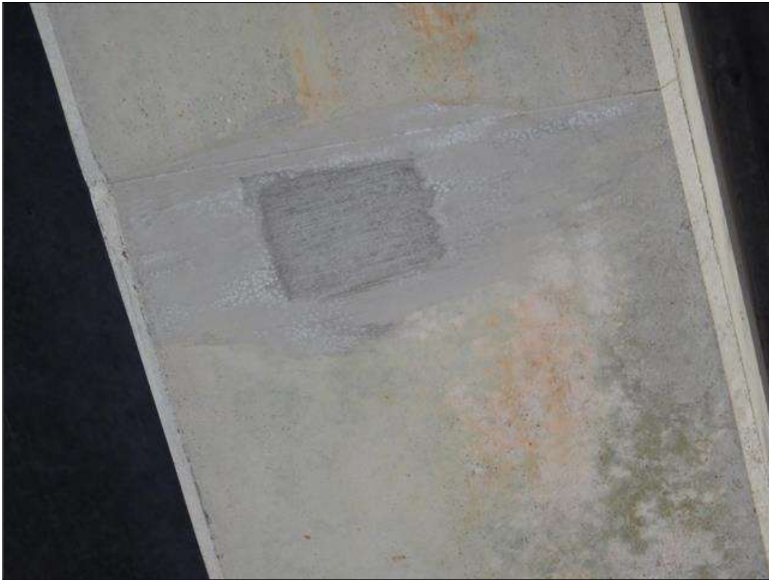
Span 31 Beam 5: [NEW REPAIR-PATCHING] FORMERLY --> spall with exposed rebar on the bottom face at 16ft from Bent 28 (5" x 4" x 1/4")
