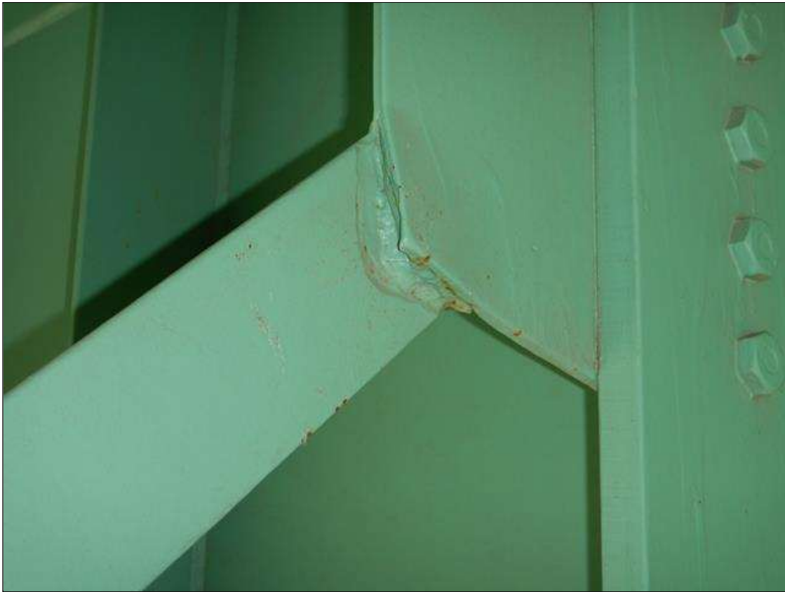
Span 13 Beam 2: corrosion and on the end diaphragm at Bent 13 and pack rust in the gusset plates
