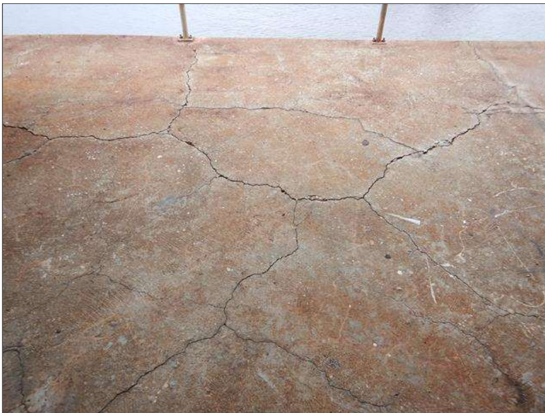
Bent 16 - Lift Span Bent Cap 1: cracking up to (1/8") wide on the top face at the southwest corner
