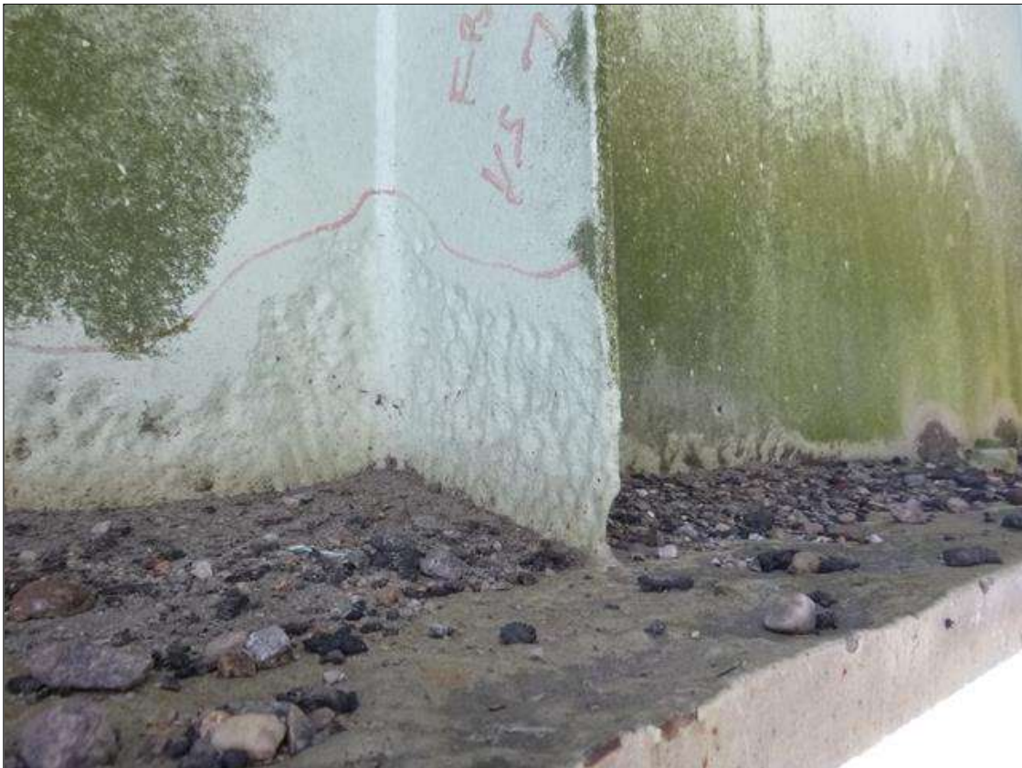
Span 18 Lift Span Floor Beam 9: VERTICAL STIFFENER 7 ON WEST SIDE - 4" HIGH PITTED AREA AT BOTTOM FLANGE WIDE/ 1/8" REMAINING SECTION IN LOWER 1-1/2" OF AREA - CLEANED AND PAINTED
