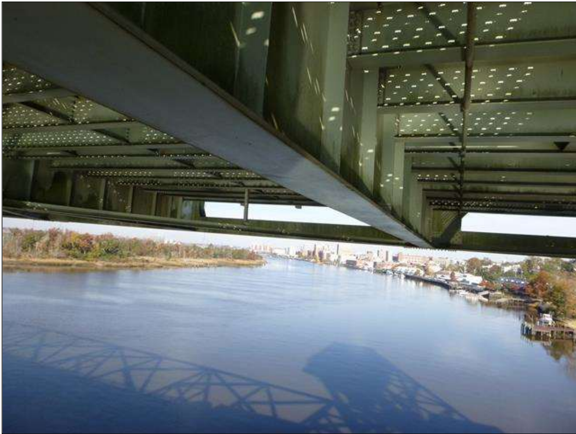
Span 18 Lift Span Floor Beam 10: 2021 INSPECTION THERE IS NO CENTER GUSSET PLATE 2020 INSPECTION HAD BOTTOM FLANGE HAS PITTED AREAS AROUND BOTH SIDES OF CENTER GUSSET PLATE, .25"DEEP X 2"WIDE X FULL WIDTH OF BOTTOM FLANGE.
