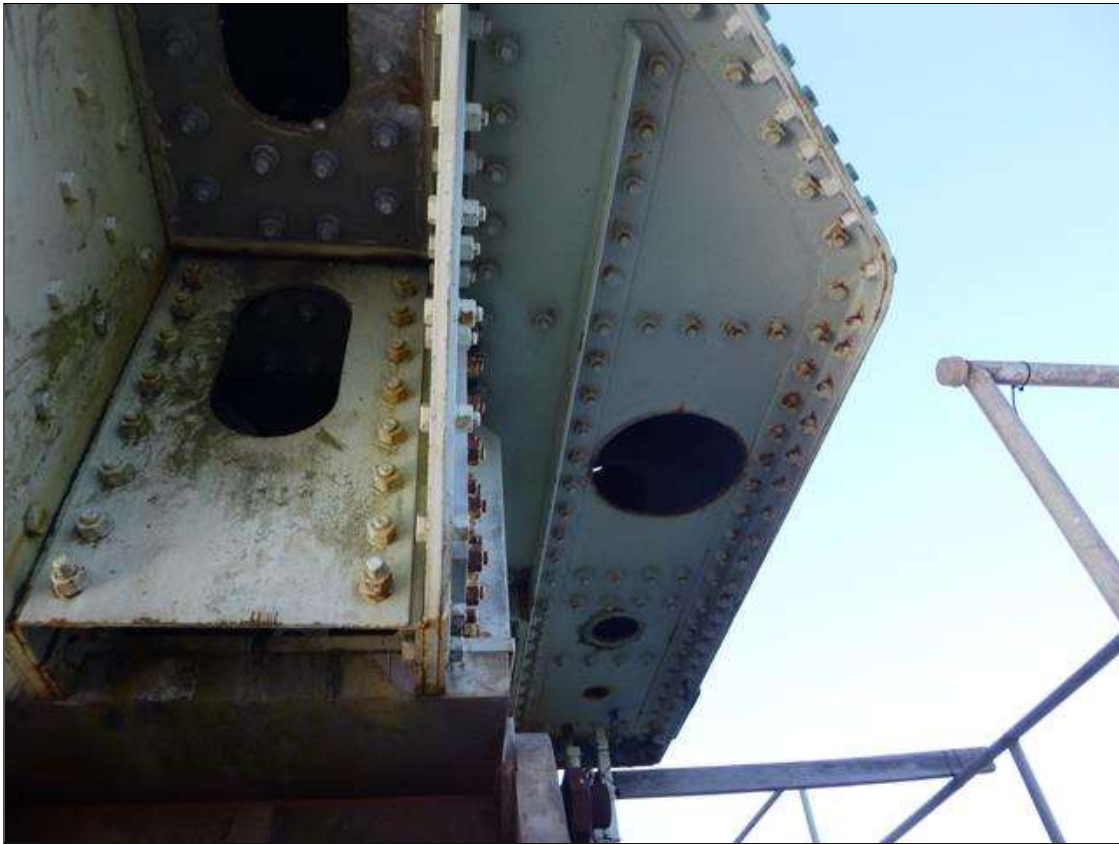
Span 18 Lift Span L0 NORTH: SURFACE RUST ON BOLTS.
