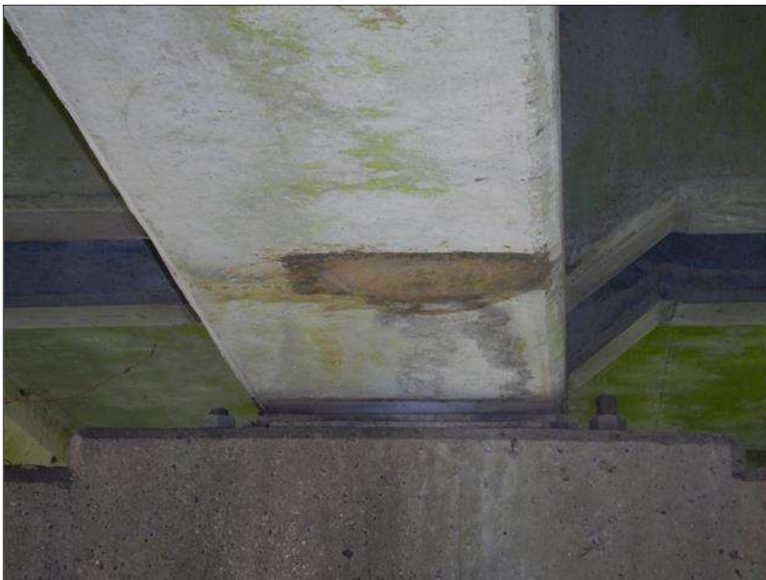
Span 3 Beam 3: [NEW REPAIR - PATCHING] FORMERLY --> spall with exposed rebar on the bottom face at 31in from bent 3 (9" x 3" x 1/2")
