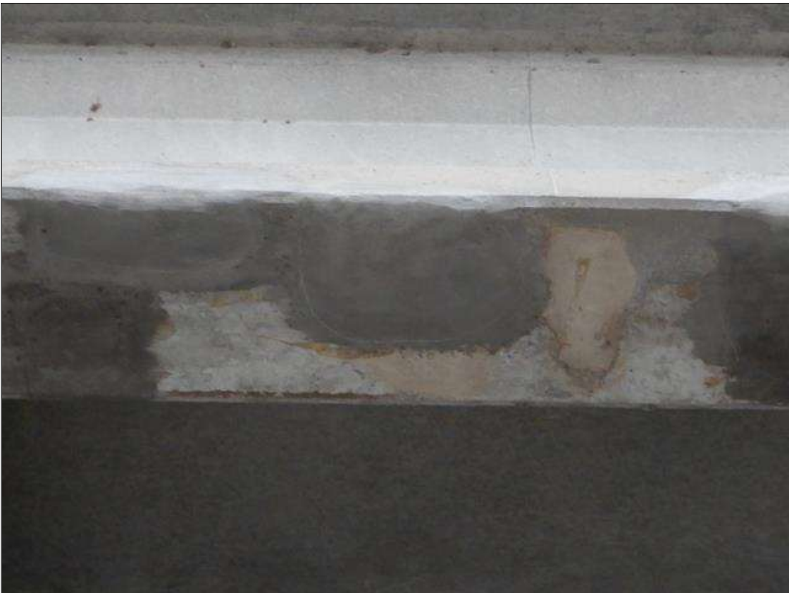
Span 9 Beam 9: [NEW REPAIR - PATCHING] FORMERLY --> (14" x 12" x 1/2") spall with exposed rebar on the bottom face at 20ft from bent 9
