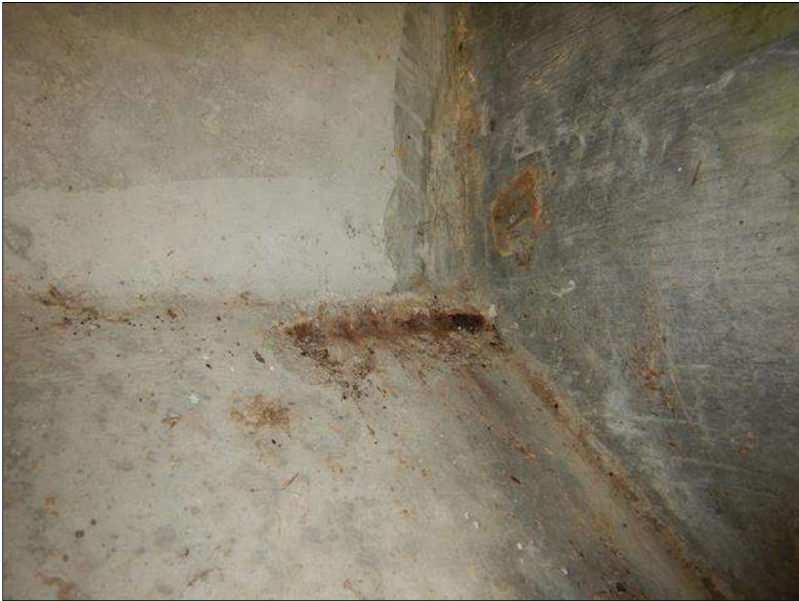
Span 3 Beam 5: [PROMPT ACTION REQUEST] (6" x 2" x 1/4") spall with exposed rebar in the bottom right chamfer at bent 3
