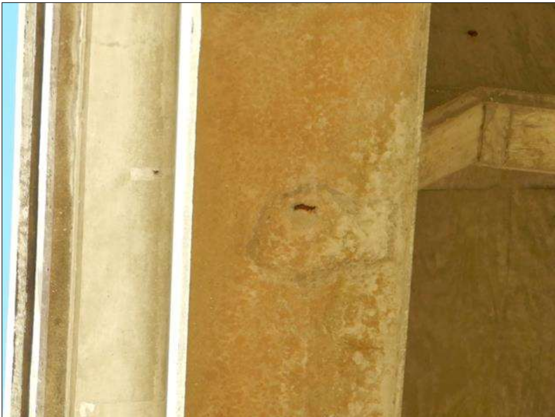
Span 27 Beam 15: [PROMPT ACTION REQUEST] (3" x 3" x 1/4") spall with exposed rebar on the bottom face at 21ft from bent 24
