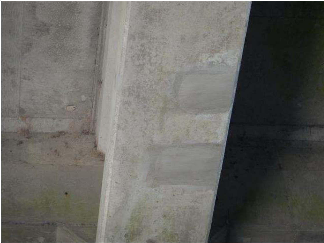
Span 29 Beam 5: [NEW REPAIR-PATCHING] FORMERLY --> (x2) spalls with exposed rebar on the bottom face at 3ft from Bent 26 up to (9" x 4")
