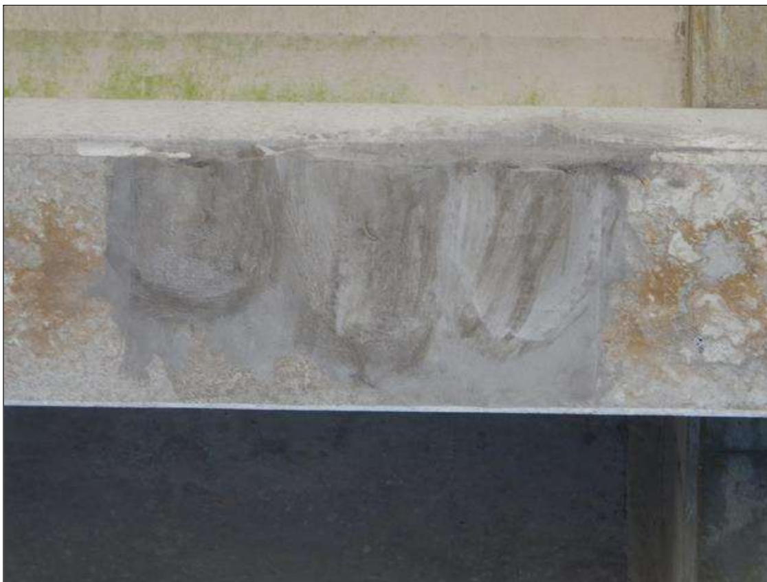
Span 28 Beam 5: [NEW REPAIR-PATCHING] FORMERLY --> spall with exposed rebar (13" x 9" x 1") and (2) exposed strands on the bottom face at 22ft from Bent 25, strands exposed for up to (9.5") long, active corrosion with less than (1/16") section loss on the strands
