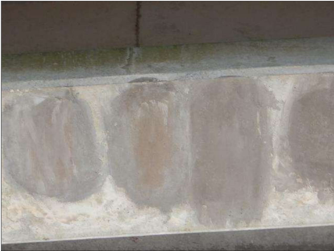
Span 29 Beam 7: [NEW REPAIR-PATCHING] FORMERLY --> spall with exposed rebar on the bottom face at 22ft from bent 27 (5" x 4" x 1/2")
