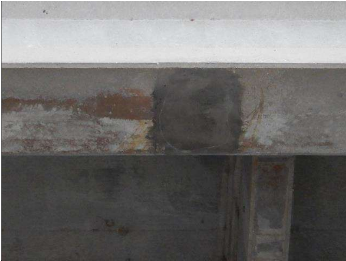
Span 9 Beam 9: [NEW REPAIR - PATCHING] FORMERLY --> PRIORITY MAINTENANCE - spall with exposed strands on the bottom face at 16ft from bent 8 (16" x 13" x 1 1/2"), (x2) strands exposed for (4") long
