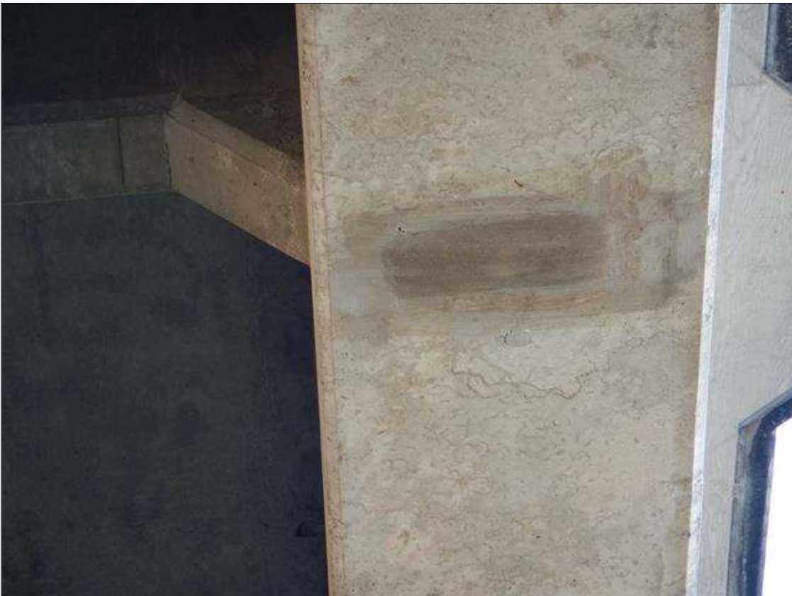
Span 30 Beam 1: [NEW REPAIR-PATCHING] FORMERLY --> spall with exposed rebar on the bottom face at 22ft from bent 28 (9" x 4" x 1/2")
