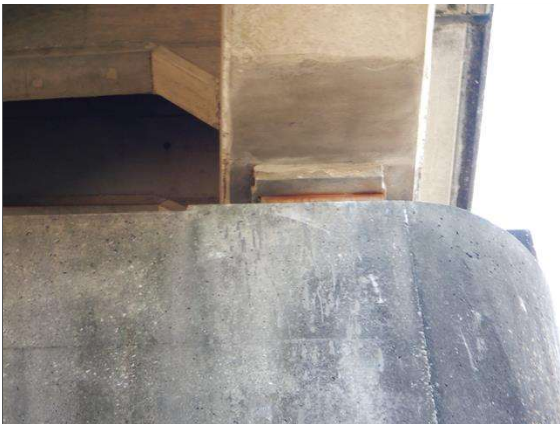
Span 29 Beam 1: [NEW REPAIR-PATCHING] FORMERLY --> spall with exposed rebar on the bottom face at bent 27 (3" x 3" x 1/8")
