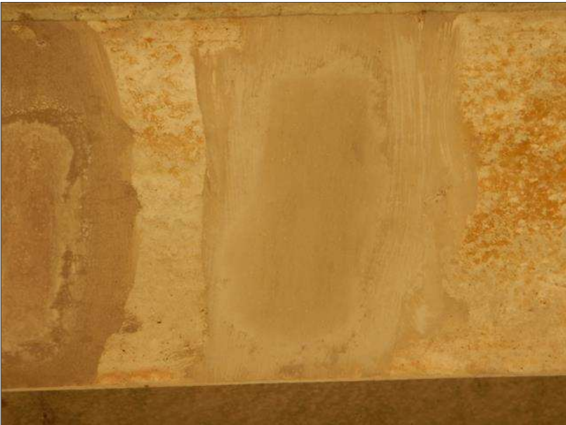
Span 30 Beam 10: [NEW REPAIR-PATCHING] FORMERLY --> area of delamination on the bottom face, 5" in diameter, 15' from bent 28, with 3/16" separation
