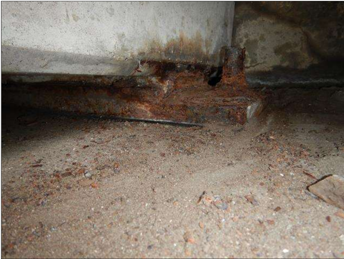
Span 1 Beam 1 - Beam 1 Near Bearing: Active corrosion and 100% section loss on the left anchor rod nut (up to 50% section loss on the right nut) section loss on the masonry plate at the front left corner up to (3/16") into the plate into the top of the plate (3" wide x 2 1/2" long
