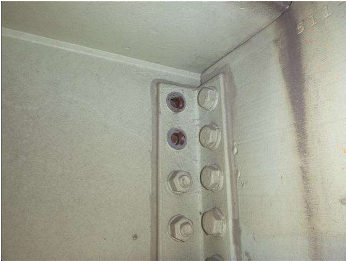
Span 18 Lift Span Stringer 4: BETWEEN FB 7-8, TOP (2) BOLTS HAVE SHEARED AT NORTH SIDE OF STRINGER CONNECTION TO FB. 8, PAR ISSUED.
