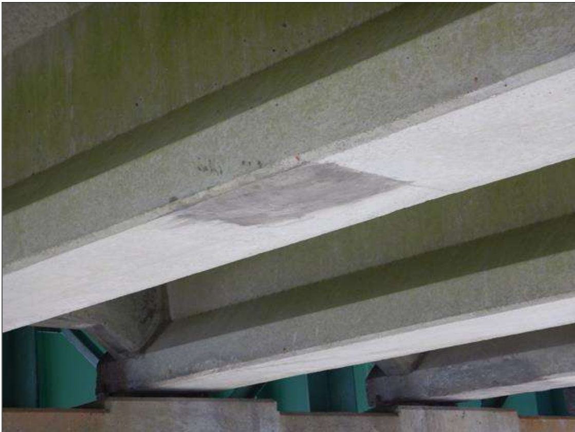
Span 11 Beam 6: [NEW REPAIR - PATCHING] FORMERLY --> (x2) spalls with exposed rebar on the bottom face up to (8" x 7" x 1/2") at 11ft from bent 11
