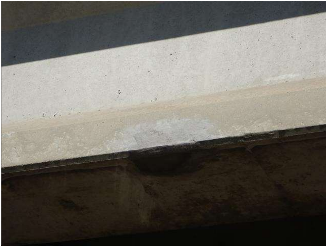
Span 31 Beam 12: [NEW REPAIR-PATCHING] FORMERLY --> Impact Damage (apparent) on the bottom right flange over exit ramp, spall with no exposed steel (8" x 3" x 1/2") - Clearance 16.25ft at this location
