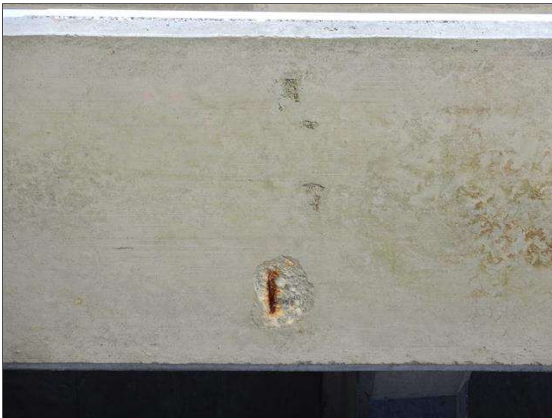
Span 35 - Ramp Span Beam 1: [PROMPT ACTION REQUEST] APPROXIMATELY 18' OUT FROM THE RAMP ABUTMENT, LOWER SIDE, SPALLING WITH EXPOSED REBAR [APPROXIMATELY 5" DIAMETER X UP TO 1/2" DEEP]; NO MEASURABLE SECTION LOSS
