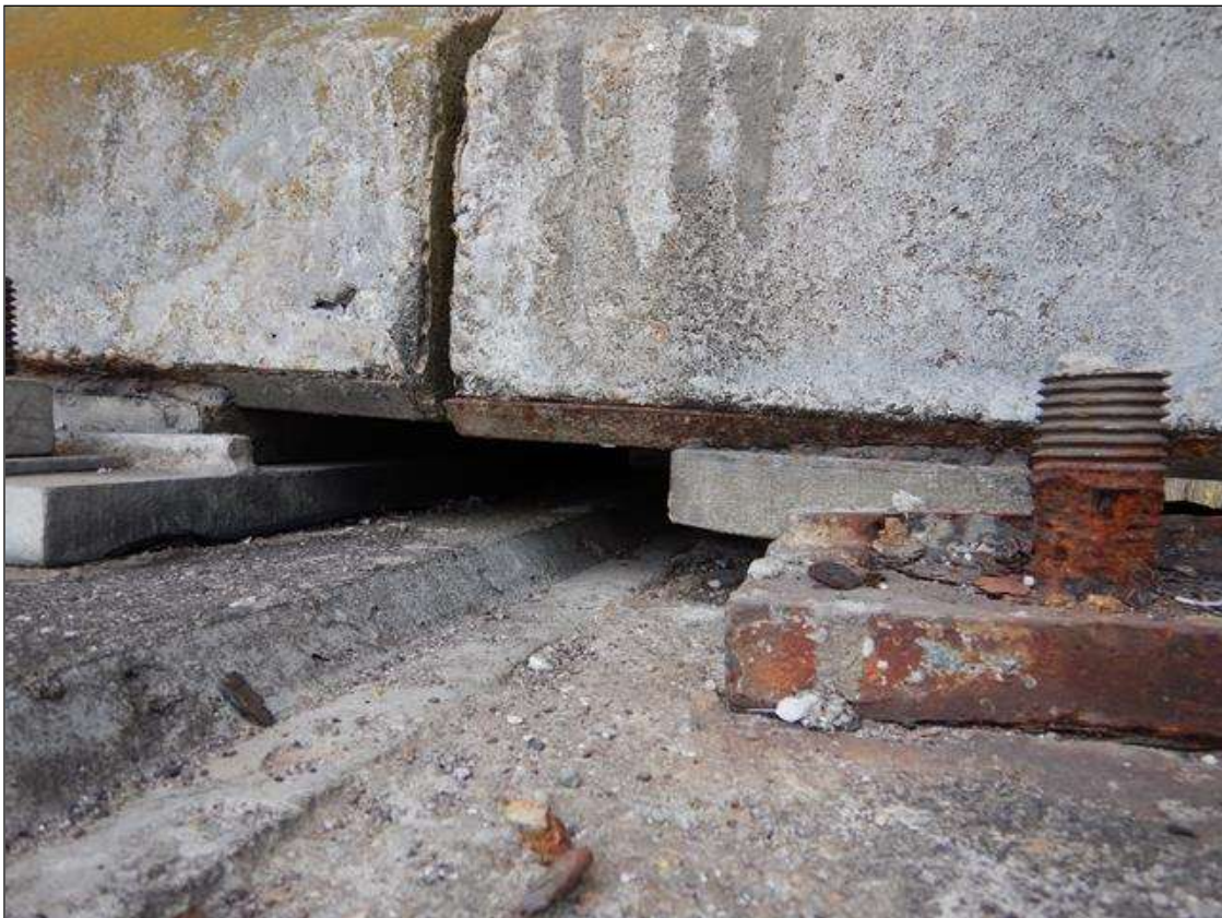
Span 1 Beam 1 - Beam 1 Far Bearing: up to (1-9/16") movement of bearing east beyond masonry plate with 26% loss of bearing
