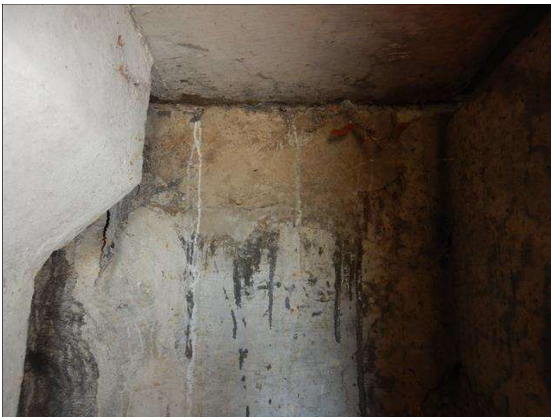
Ramp End Bent Abutment: [NEW REPAIR-PATCHING] FORMERLY --> spall with no exposed rebar behind girder 5 (16" x 6" x 2")
