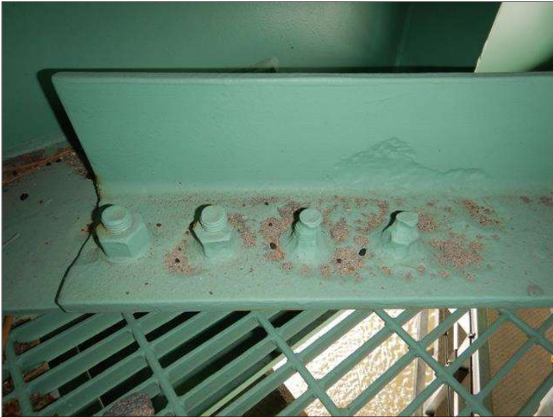
Span 16 Beam 4: [PROMPT ACTION REQUEST] 5/16" section loss on end diaphragm gusset in the right web at bent 15 due to previous rust. (3" x 3") with (1/16") remaining, section loss on 3 nuts up to 60%. area has been cleaned and repainted. section loss in more than 25% of the gusset plate thickness
