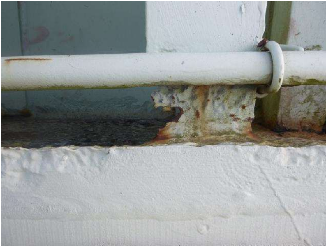
Span 18 Lift Span LB12: [PROMPT ACTION REQUEST] EASTBOUND LANE: 3RD STIFFNER RIGHT OF NORTHWEST CABLE BANK LOSS OF SETION .392" WITH .134" REMAINING ALONG BOTTOM 4" HIGH ON WEB AND FLANGES.
