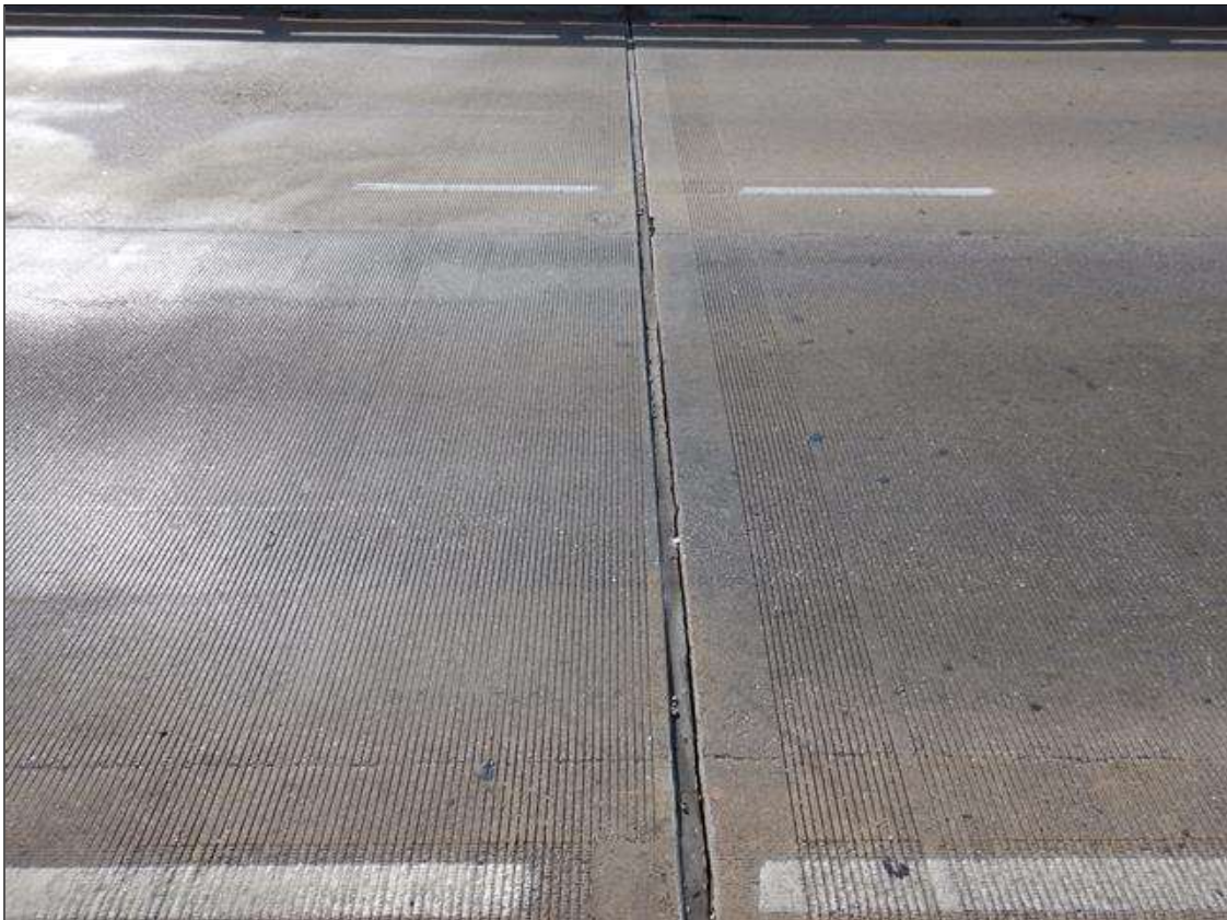
Span 13 Joint at Bent 12: SCATTERED ALONG THE LENGTH, LOSS OF SEAL ADHESION UP TO FULL DEPTH AND SCATTERED EDGE CHIPPING IN THE ADJACENT DECK HEADERS UP TO 1" WIDE
