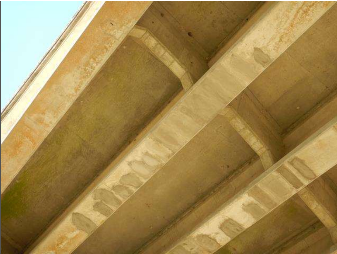
Span 27 Beam 14: [NEW REPAIR-PATCHING] FORMERLY --> (x13) DELAMINATION areas on the bottom face at 10f from bent 24 up to (10" x 2 1/2" x 1/4")
