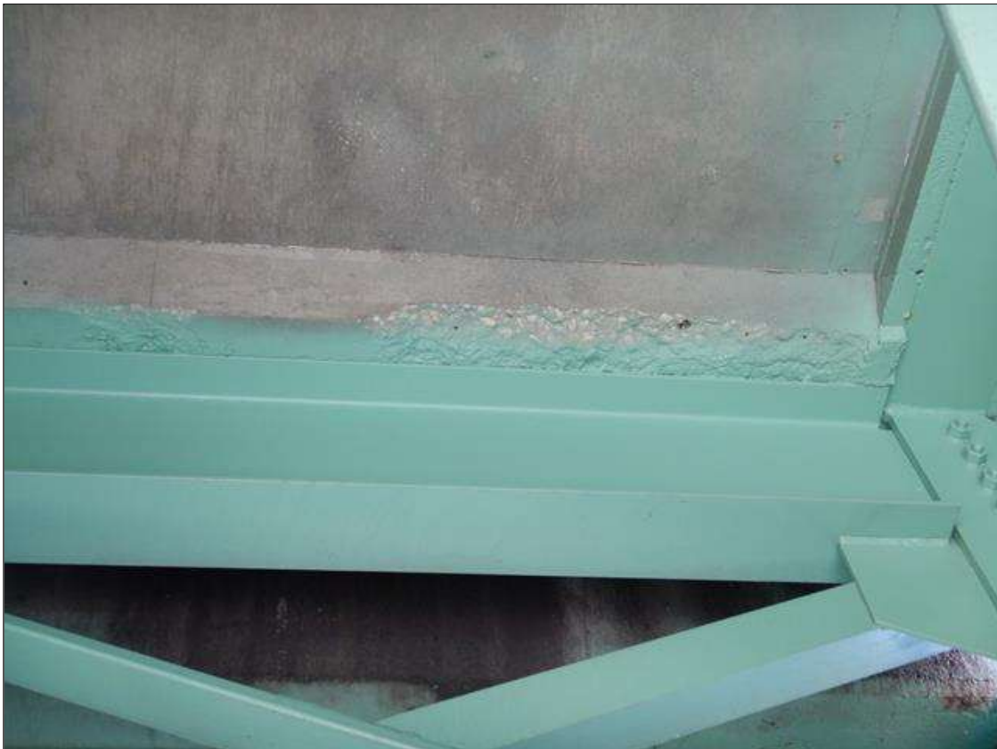
Span 21 Deck: (x2) spalls with no exposed steel on the deck bottom in bay 1 at bent 18 up to (30" x 4" x 1").
