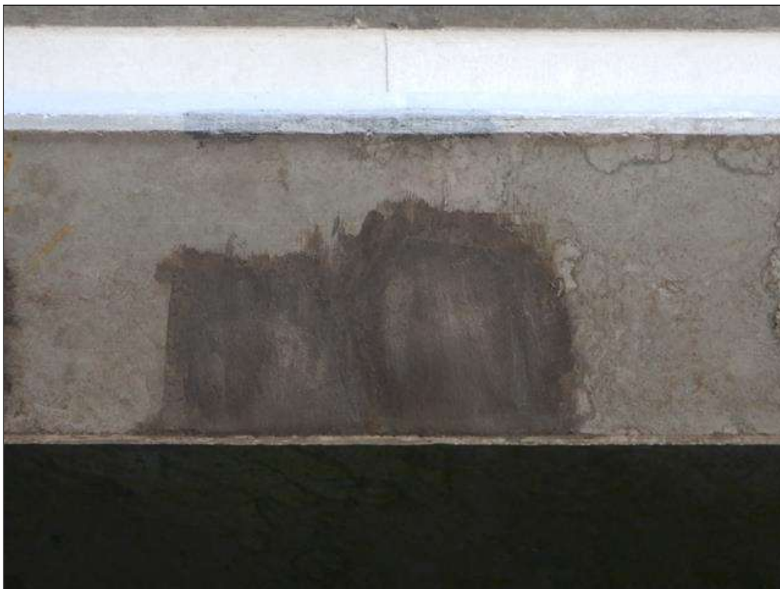
Span 28 Beam 1: (x2) sound patches on the bottom face at mid span up to (8" x 7")
