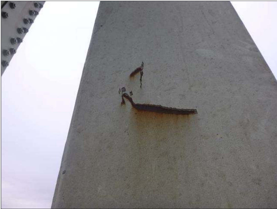
Span 18 Lift Span L0U1 NORTH: SCRAPES ON NORTH FACE 6' ABOVE BRIDGE DECK WITH SURFACE RUST.
