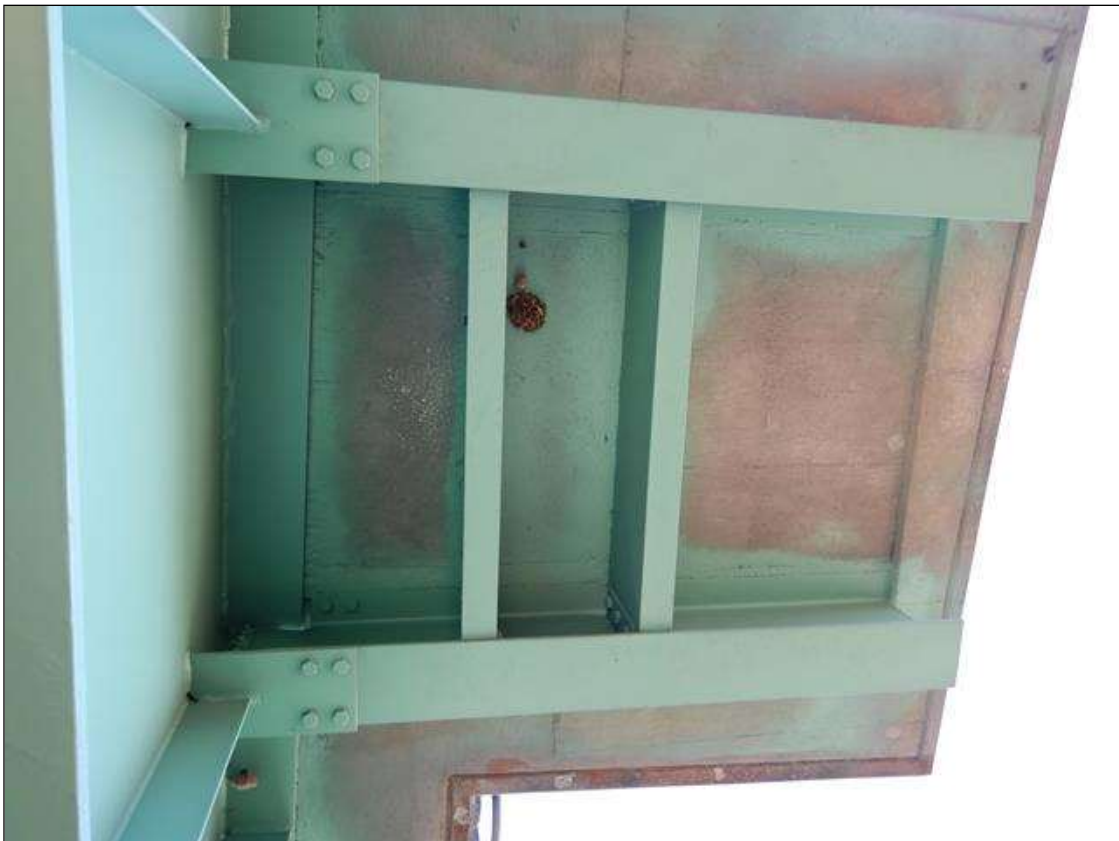
SPAN 23, LEFT SIDE, FRAMING FOR THE TRAFFIC SIGNAL OVERHANG [SIMILAR AT SPAN 13 RIGHT SIDE]
