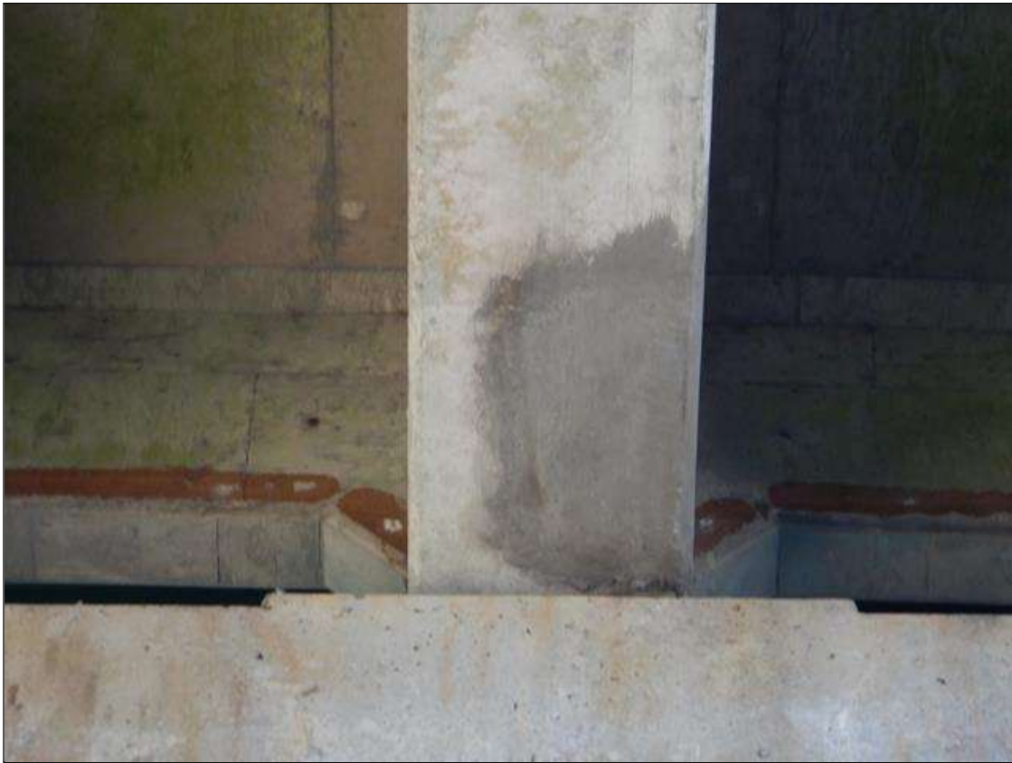
Span 27 Beam 2: [NEW REPAIR-PATCHING] FORMERLY --> spall with exposed rebar (27" x 4" x 2 1/2") and (1) strand exposed on the bottom left flange at Bent 24, strand exposed for (16") long, active corrosion on strand with no measureable section loss
