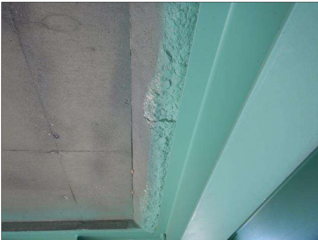
Span 22 Deck: spall with no exposed steel on the deck bottom at bent 20 in bay 1 (7.5ft x 3" x 3").
