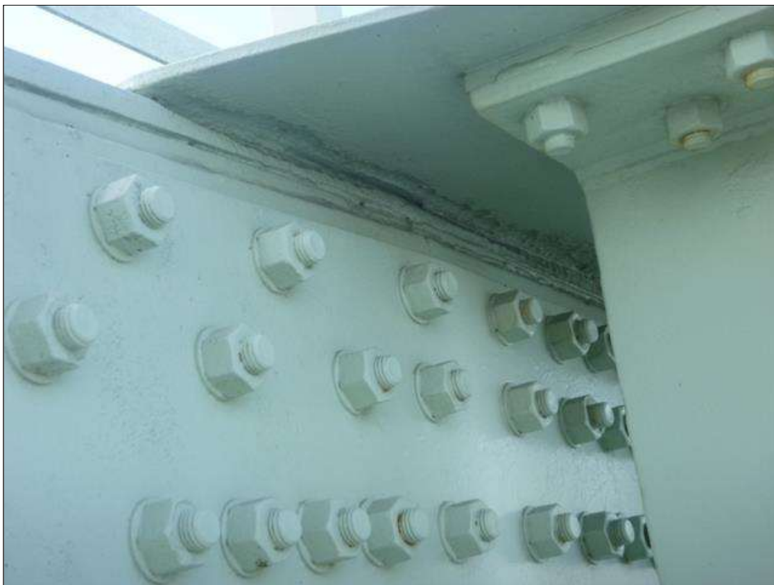
Span 18 Lift Span U9 SOUTH: 32" LONG X 1 1/2" WIDE AREA OF CLEANED AND PAINTED SECTION LOSS TO UNDERSIDE OF GUSSET PLATE @ U9 SOUTH SIDE.
