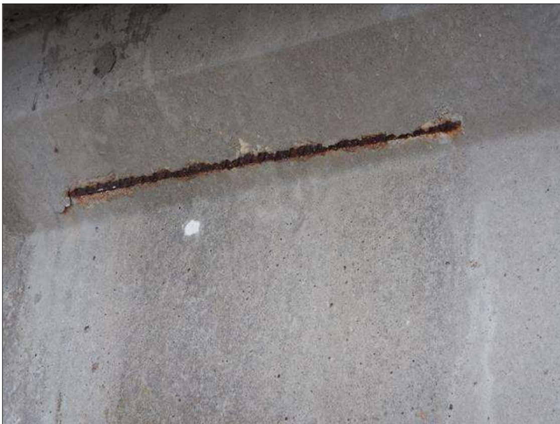
Span 10 Beam 9: [NEW REPAIR - PATCHING] FORMERLY --> (26" x 1") area of exposed rebar in the top left chamfer at bent 10
