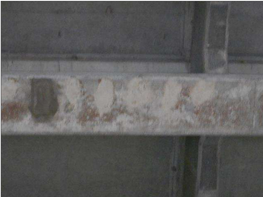
Span 10 Beam 8: [NEW REPAIR - PATCHING] FORMERLY --> (X3) spalls with exposed rebar on the bottom face at 14ft from bent 9 at failed repairs up to (10" x 6" x 1/2")
