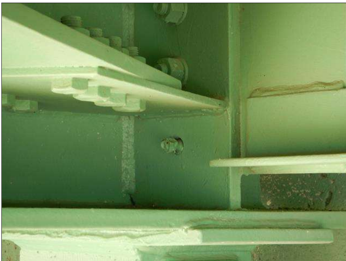
Span 23 Beam 7: Bent 21, bent daphragm attachment at the right side of beam 7, bottom nut is missing
