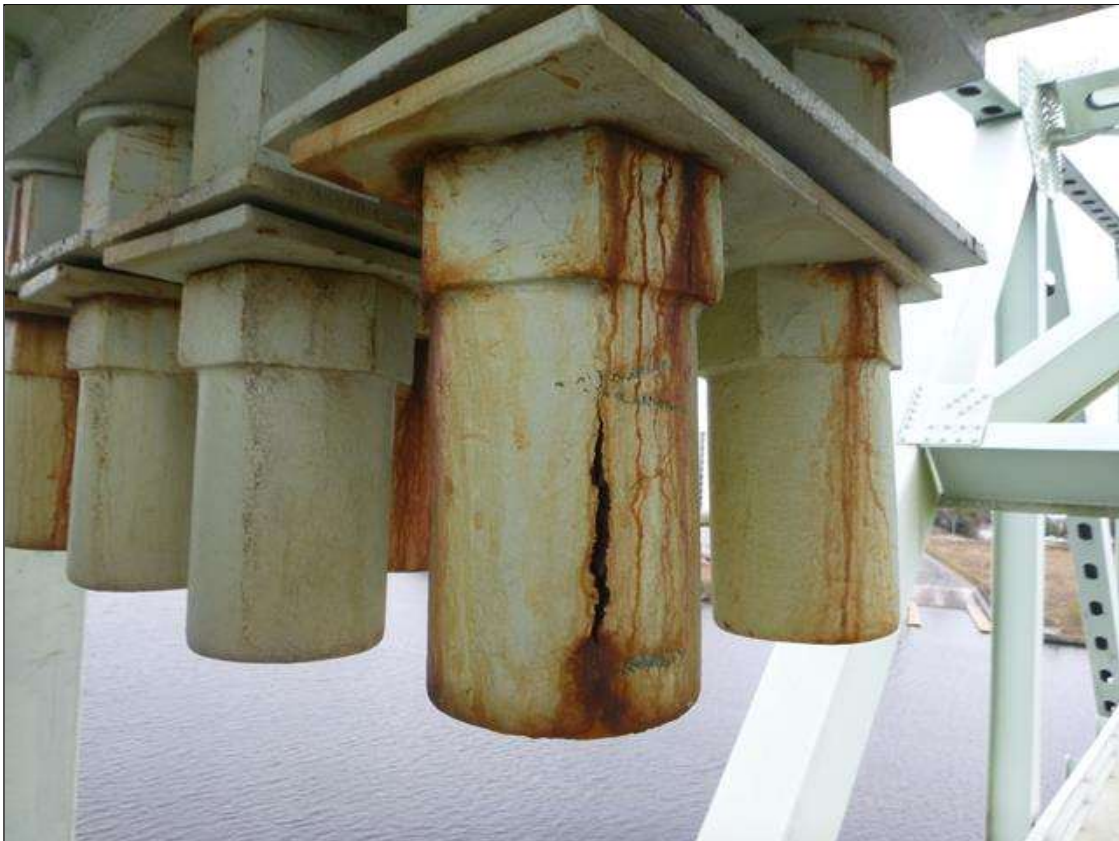
Span 18 Lift Span LB0: WEST TOWER NORTHWEST CABLE BANK, NORTH BANK WEST FACE, 4TH CABLE ROD PROTECTION CAP HAS 3/16" CRACK
