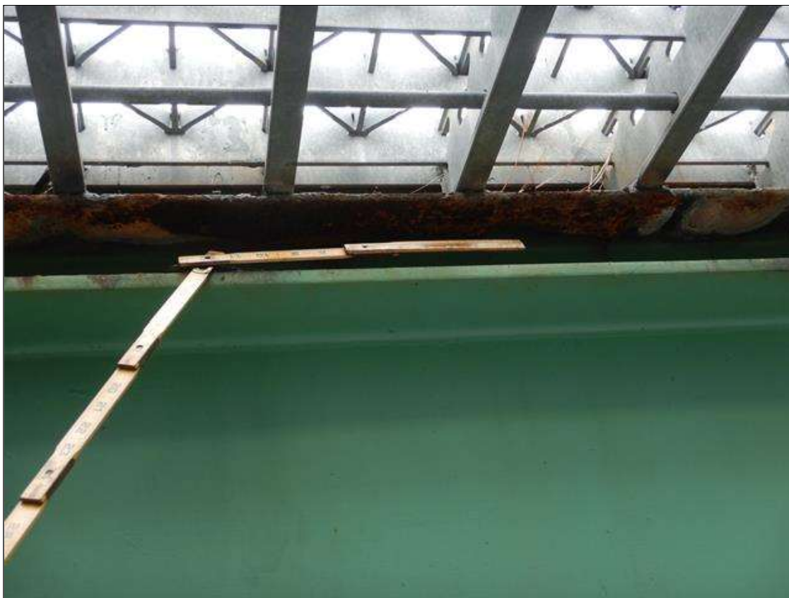
Span 20 Beam 1: PRIORITY MAINTENANCE - "nailer" beam on top of stringer 3 between brace 3 and 4 on the top flange: active corrosion and section loss with (11/32") remaining for the full length and width of the top flange (PROMPT ACTION REQUEST)
