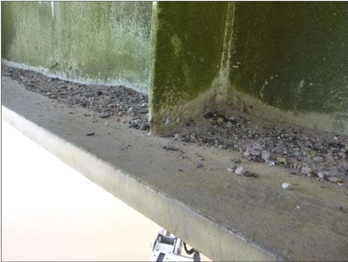
Span 18 Lift Span Floor Beam 10: (PAR) VERTICAL STIFFENER 12 EAST SIDE - 4" HIGH PITTED AREA AT BOTTOM FLANGE WIDE/ (3) HOLES FROM 1/4" TO 1/2" IN DIAMETER - 1/16" TO 1/8" REMAINING SECTION IN LOWER 1" OF AREA
