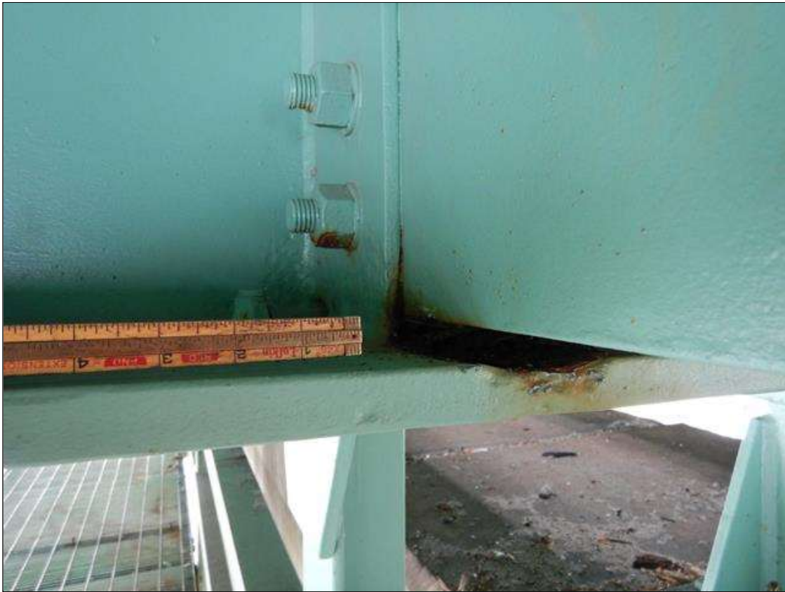
Span 16 Beam 5: [PROMPT ACTION REQUEST] - bottom left web stiffener and platform connection at bent 15: up to 100% section loss on platform nut on the bottom flange; active corrosion on the stiffener, web, flange and diaphragm gusset with no measureable section loss
