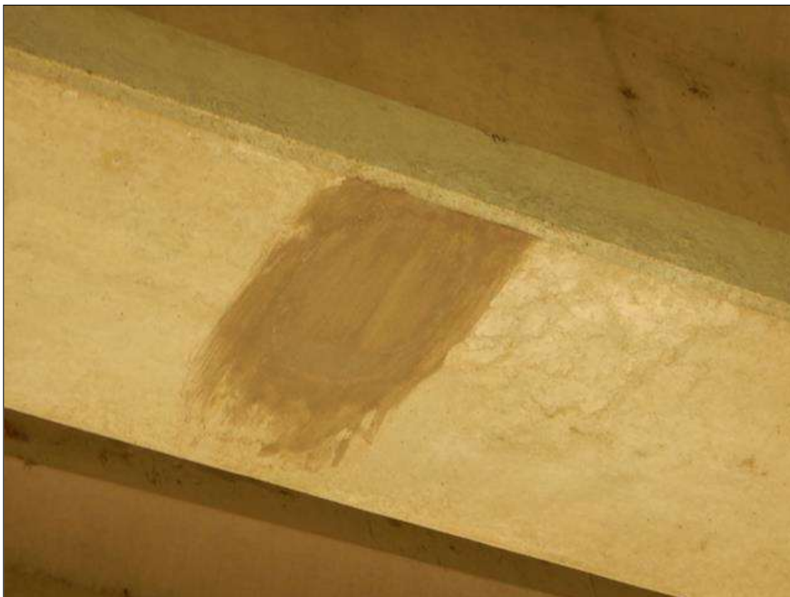
Span 29 Beam 11: [NEW REPAIR-PATCHING] FORMERLY --> spall with exposed rebar on the bottom face at 30ft from bent 27 (10" x 6" x 1/4")
