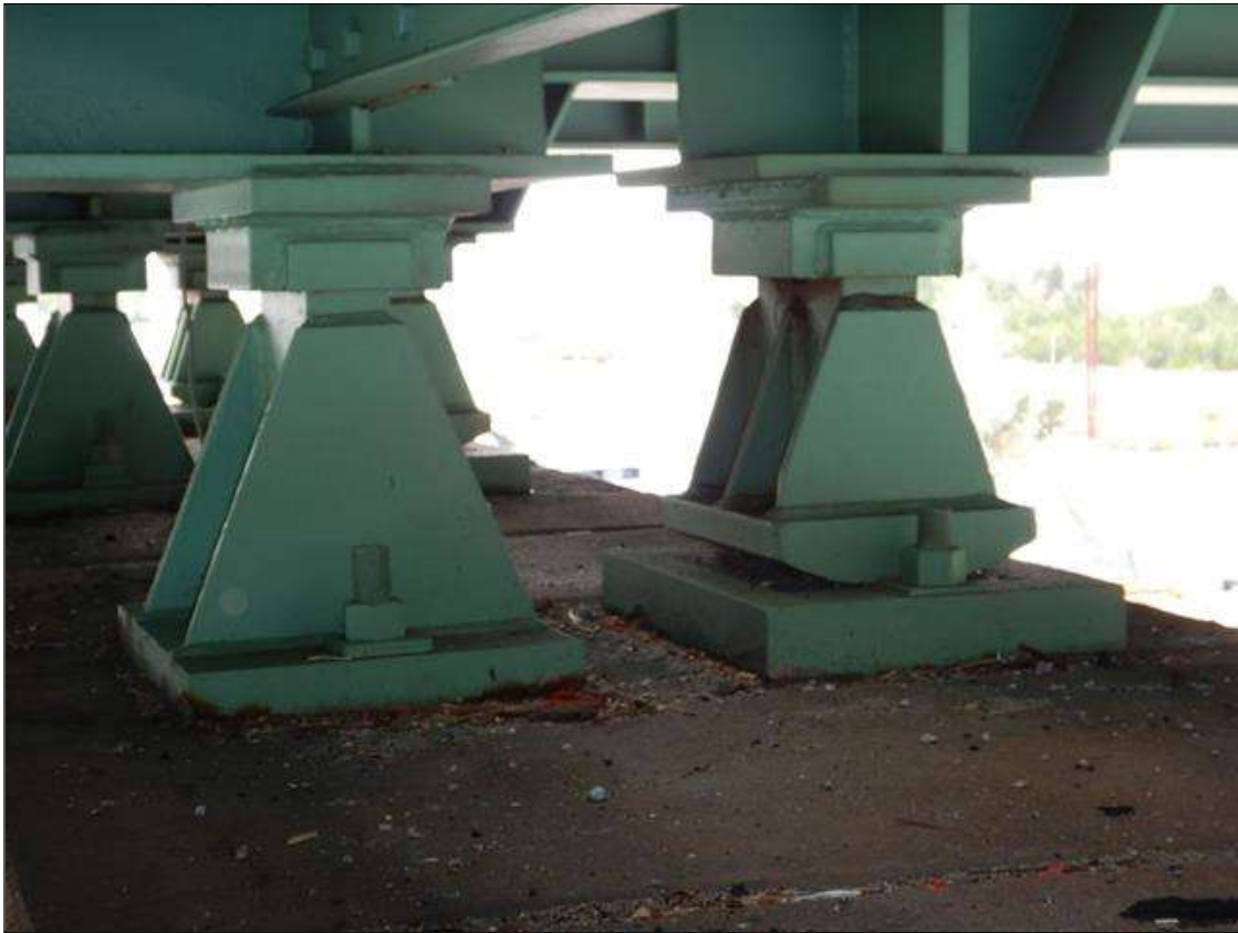
GIRDERS 6 BEARINGS AT BENT 15 [TYPICAL FOR ALL BEARINGS AT BENT 15]
