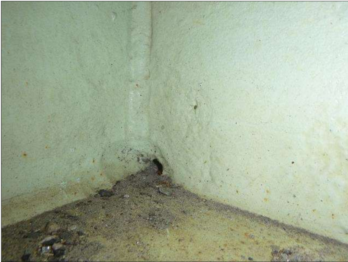
Span 18 Lift Span Floor Beam 12: STIFFNER 11 AND 12 EAST SIDE HAS 3/4" HOLE AT WEB THAT HAVE BEEN CLEANED, PAINTED AND ARRESTED.
