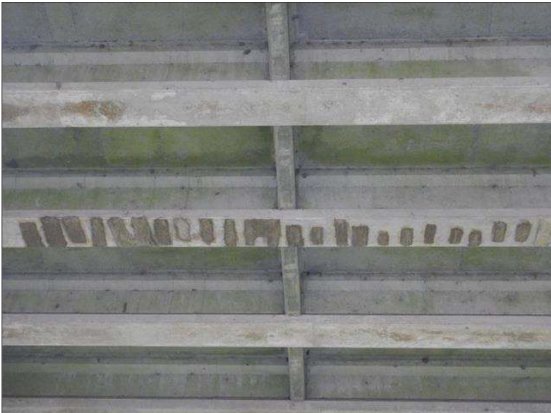
Span 6 Beam 5: [NEW REPAIR - PATCHING] FORMERLY --> 36 feet of spalling with exposed rebar on the bottom face starting at 26ft from bent 5 up to (13" x 4" x 1/2")
