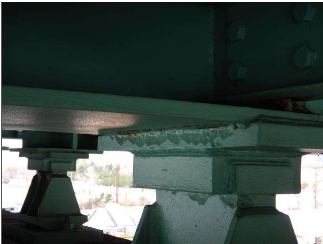
Span 16 Beam 5 - Beam 5 Near Bearing: Section loss in the top plate (18" x 1" x 1/16" into the plate)
