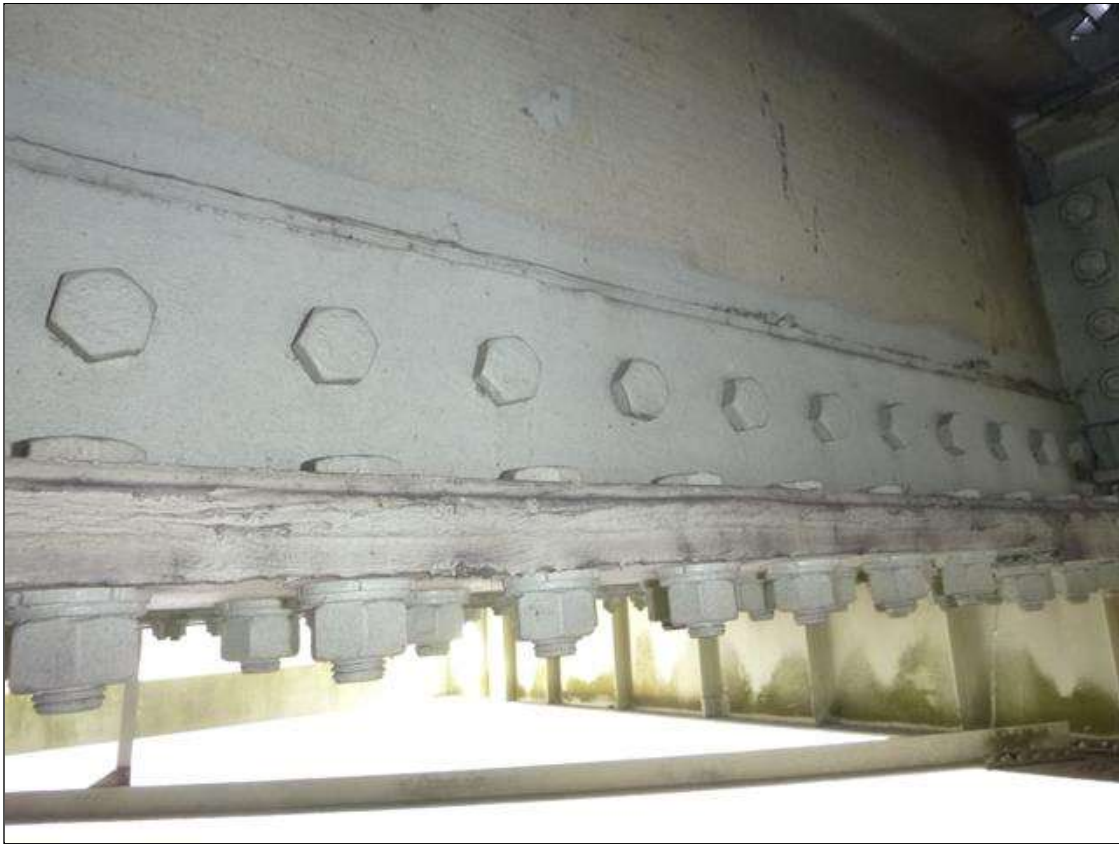
Span 18 Lift Span Stringer 7: REPAIR OBSERVED IN 2021 INSPECTION 6" X 4" X 3/8" THICK ANGLE AND 9" WIDE X 1/2" THICK PLATE HAS BEEN BOLTED TO BOTH SIDES OF THE WEB AND BOTTOM FLANGE, FULL LENGTH, 2020 INSPECTION REPORT HAD BETWEEN FB's 11-12 - PITTED AREA IN WEB ON SOUTH SIDE AT BOTTOM FLANGE AT FB 11 CONNECTION UP TO 3"LONG x 4"HIGH x 3/16"DEEP- CLEANED AND PAINTED
