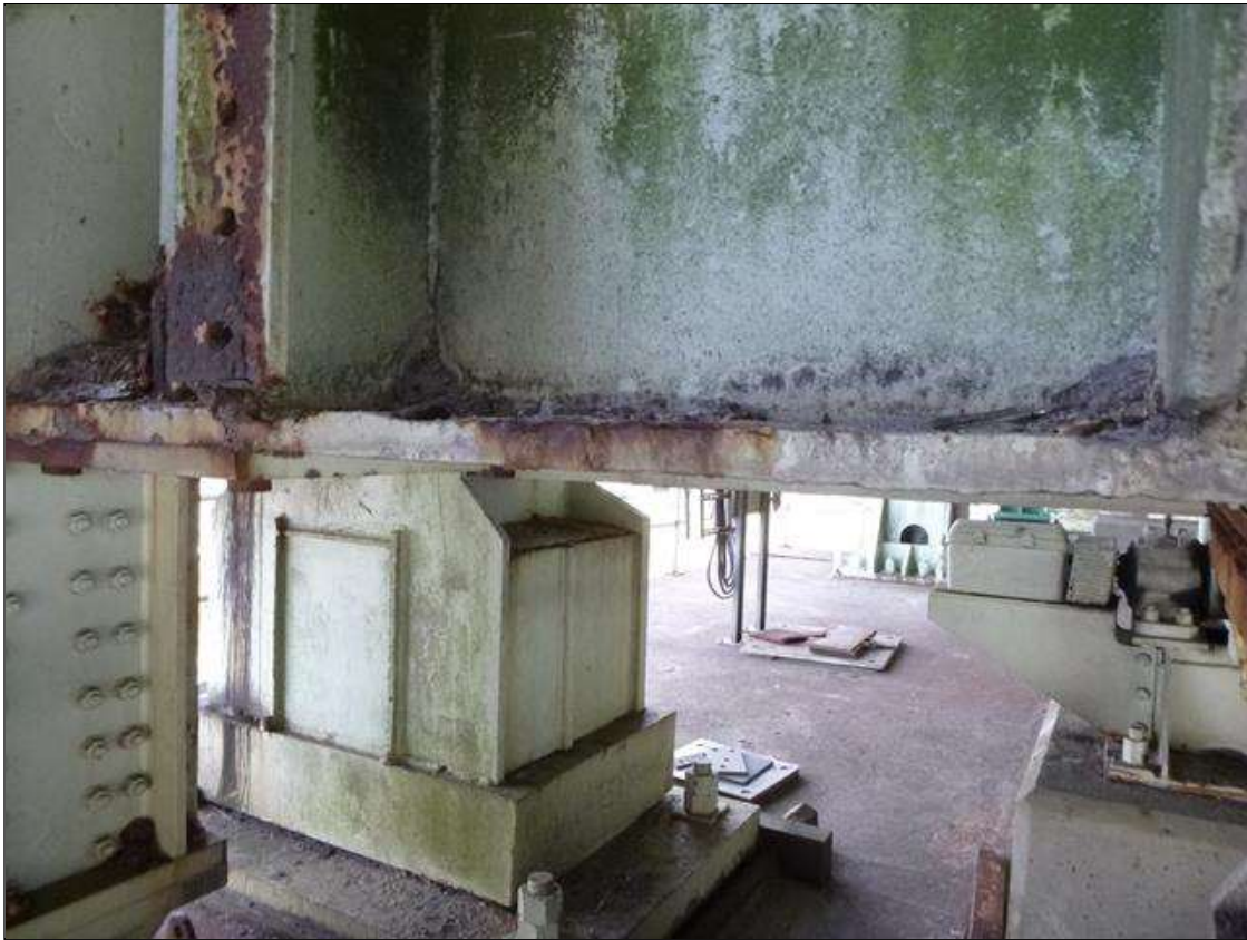
Span 18 Lift Span Floor Beam 12: (PAR) LOSS OF SECTION .341" WITH .967" REMAINING BOTTOM WEST FLANGE, 4' LONG X 2.5" WIDE BEGINING 2' LEFT OF NORTHEAST BEARING.
