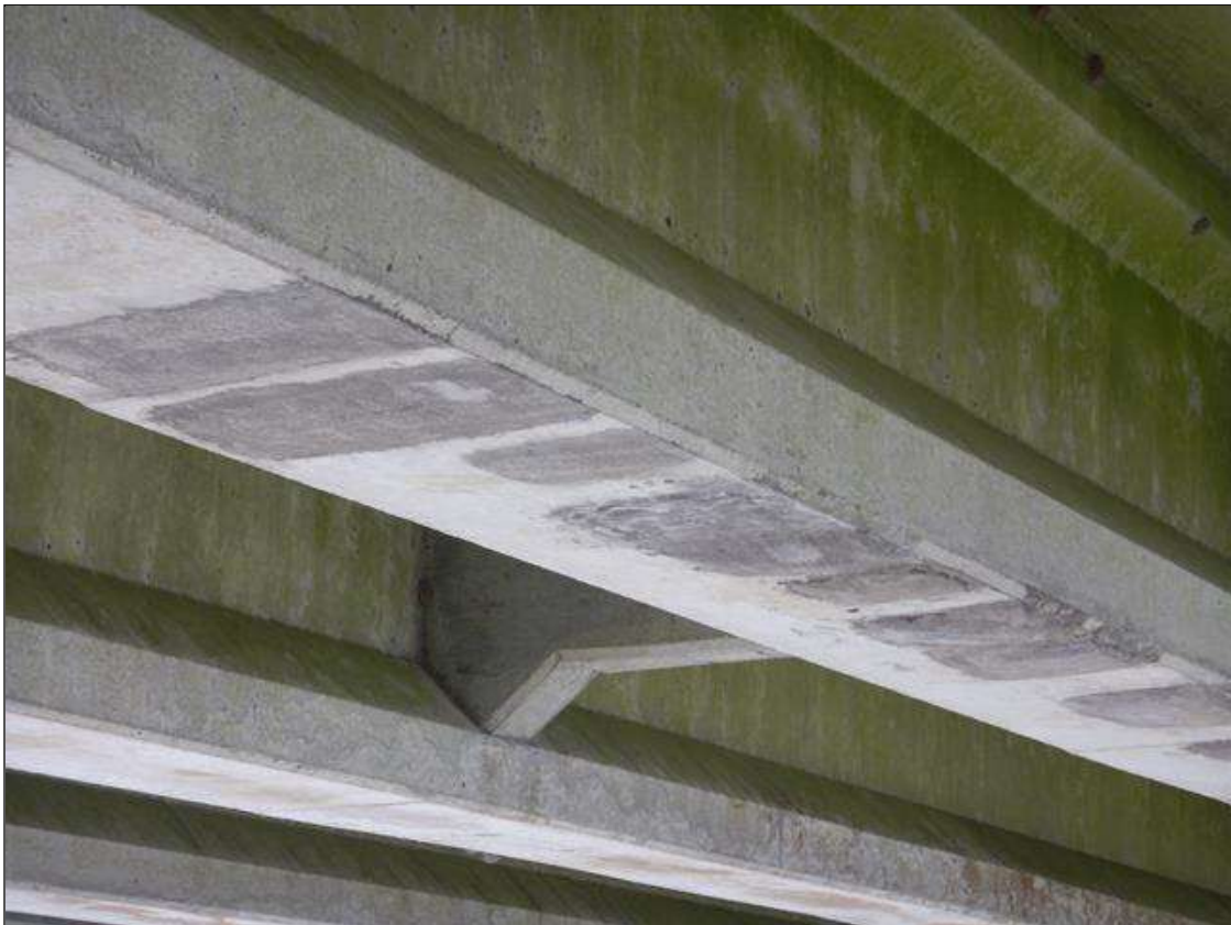
Span 11 Beam 6: [NEW REPAIR - PATCHING] FORMERLY --> multiple spalls with exposed rebar on the bottom face at 18ft from bent 10 up to (16" x 6" x 1/2")
