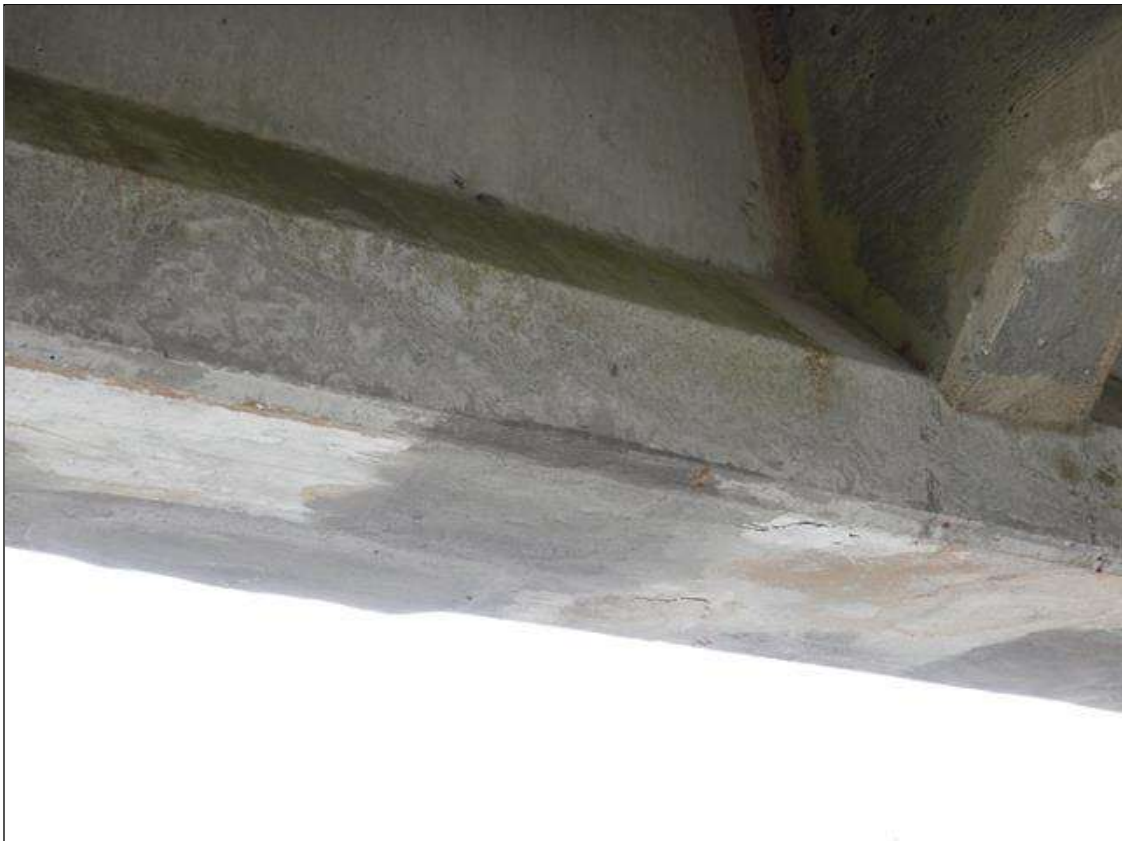
Span 9 Beam 9: (16" x 9") unsound patch with (8" x 7") DELAMINATION area on the bottom face at 17ft from bent 8
