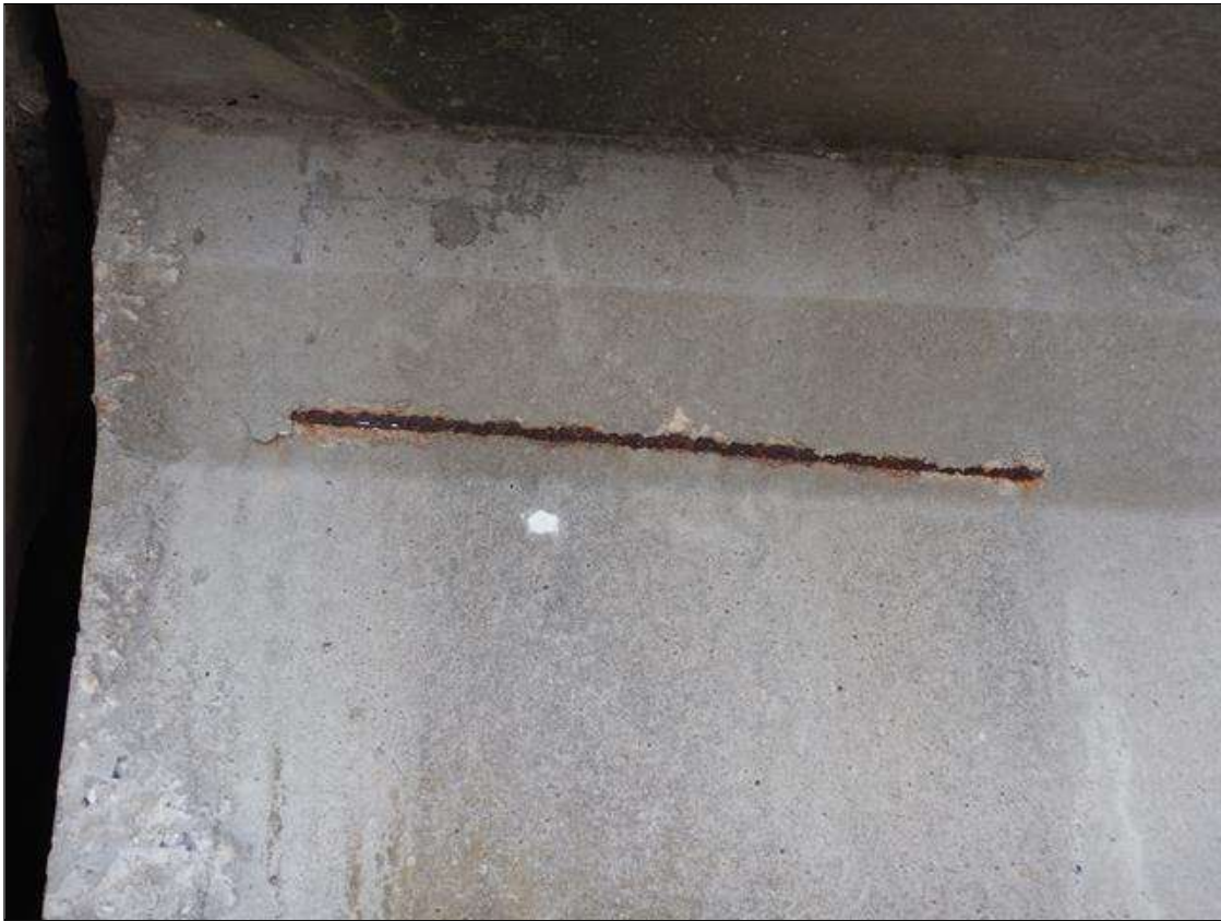
Span 10 Beam 1: [PROMPT ACTION REQUEST] spall with exposed rebar on the top left chamfer at bent 10 (24" x 1").
