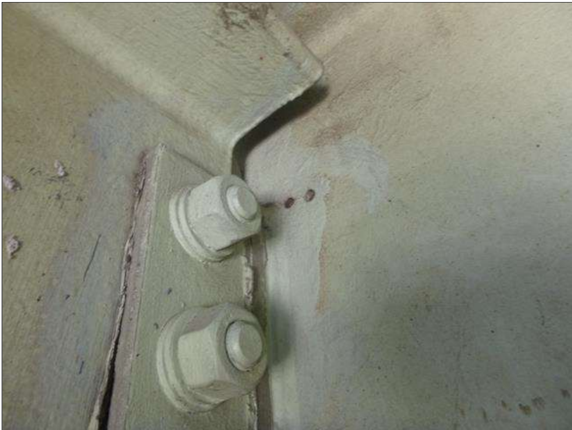
Span 18 Lift Span Stringer 4: BETWEEN FB's 9-10 - ARRESTED CRACK IN WEB AT TOP OF DIAPHRAGM CONNECTION
