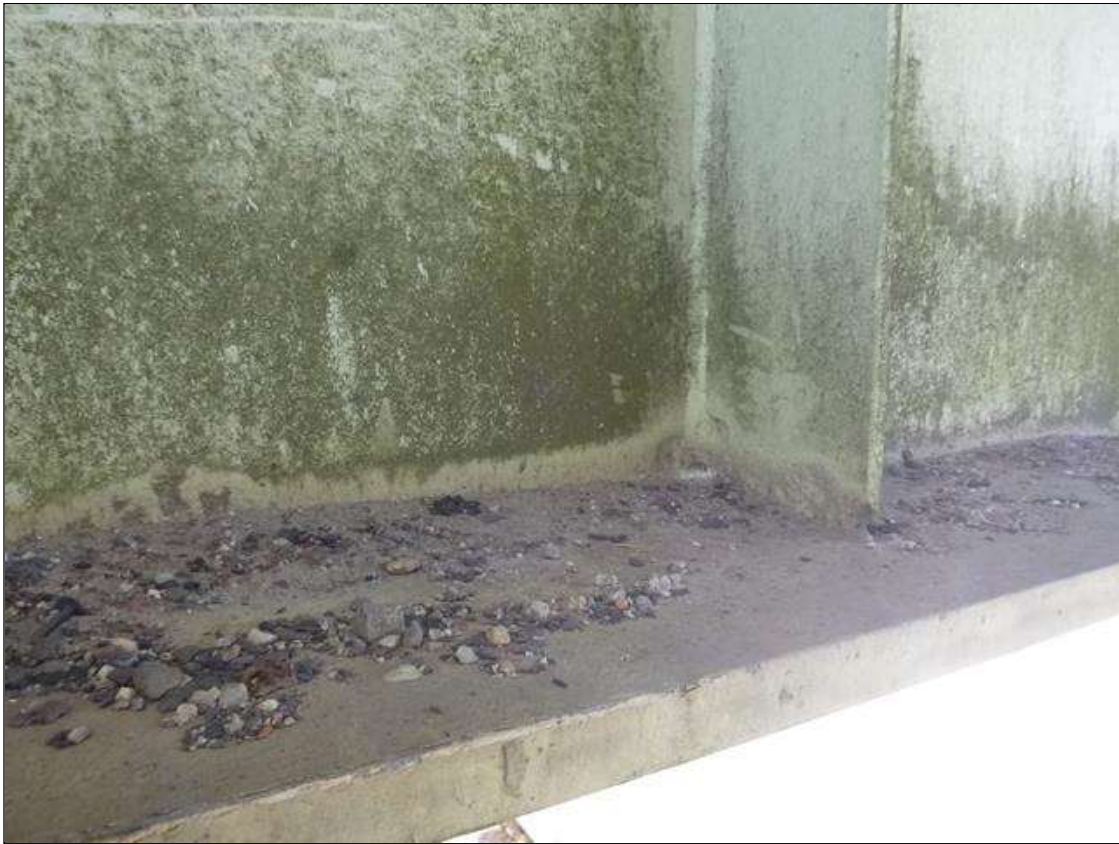
Span 18 Lift Span Floor Beam 10: VERTICAL STIFFENER 12 WEST SIDE - 2" HIGH PITTED AREA AT BOTTOM FLANGE WIDE/ 1/2" DIAMETER HOLES AT EDGES - 1/16" TO 1/8" REMAINING SECTION IN LOWER 1" OF AREA - PROMPT ACTION REQUEST
