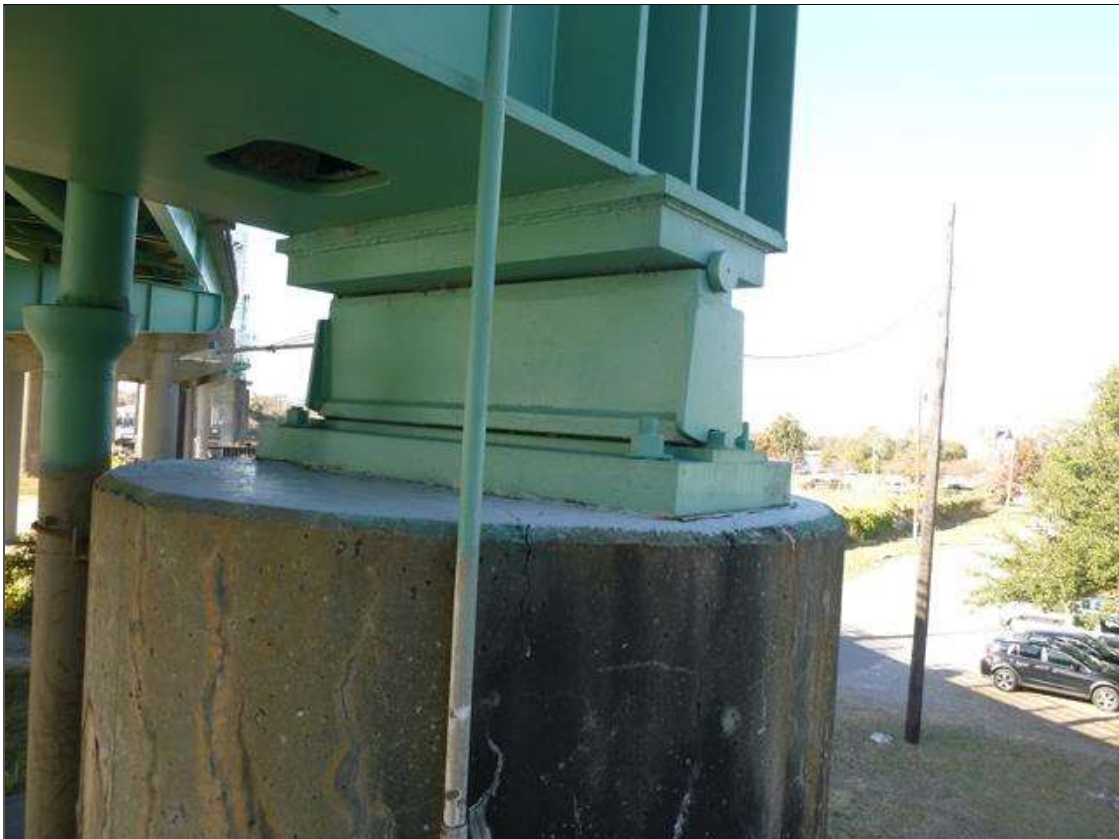
BENT 23 LEFT END MOVABLE BEARING [BENT 22 RIGHT END SIMILAR]
