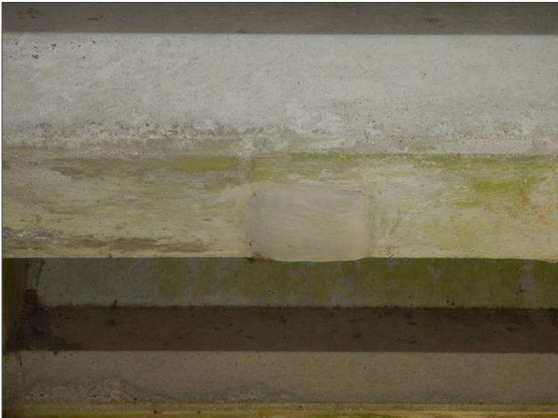
Span 3 Beam 7: [NEW REPAIR - PATCHING] FORMERLY --> (13" x 5" x 3/4") spall with exposed rebar on the bottom face at 32in from bent 3
