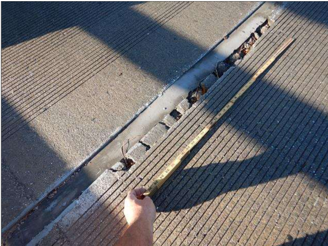
Span 21 Deck: [PROMPT ACTION REQUEST] RIGHT LANES AT BENT 18, SPALL (42" LONG x 2" WIDE x 3.5" DEEP AT 4' FROM RIGHT CURB)
