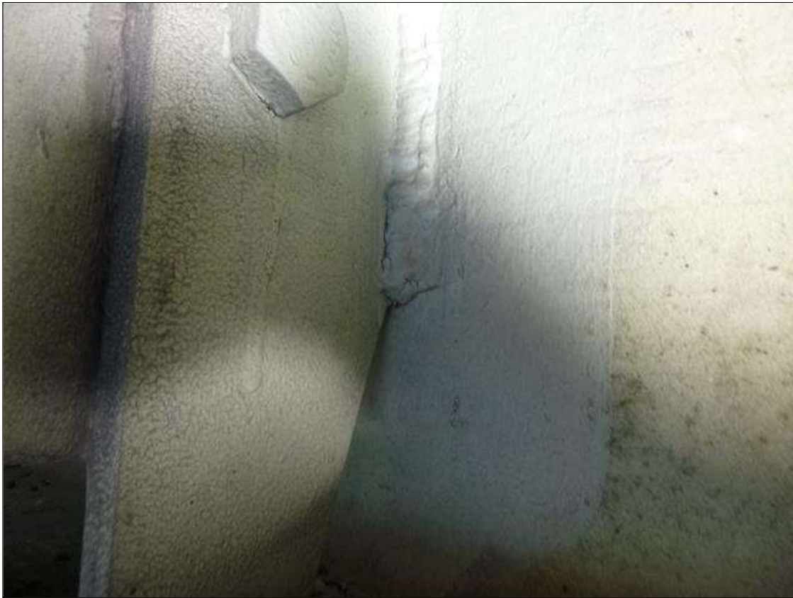
Span 18 Lift Span Stringer 5: BETWEEN FB's 5-6 - 1" LONG CRACK IN WEB ACROSS BOTTOM OF DIAPHRAGM CONNECTION
