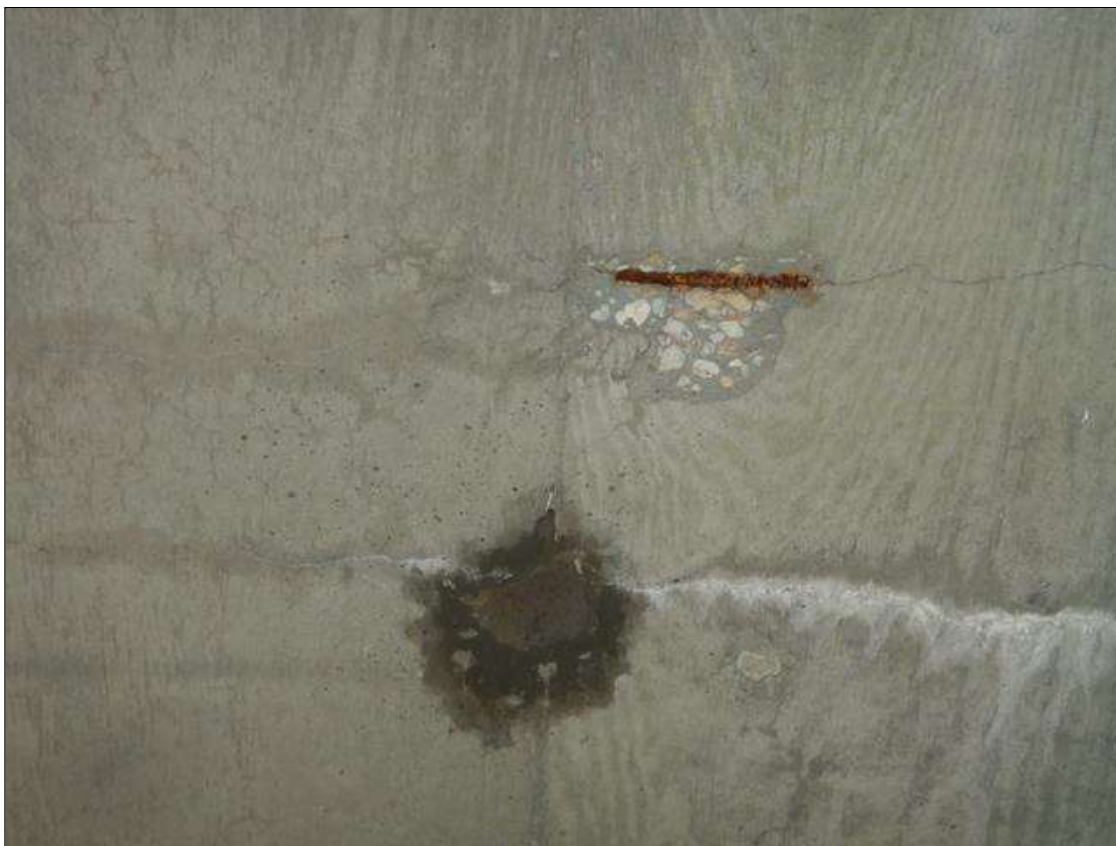
Span 14 Deck: (x2) spalls exposed rebar on the deck bottom in bay 4 at 60ft from Bent 13 up to (7" x 4" x 1/2").
