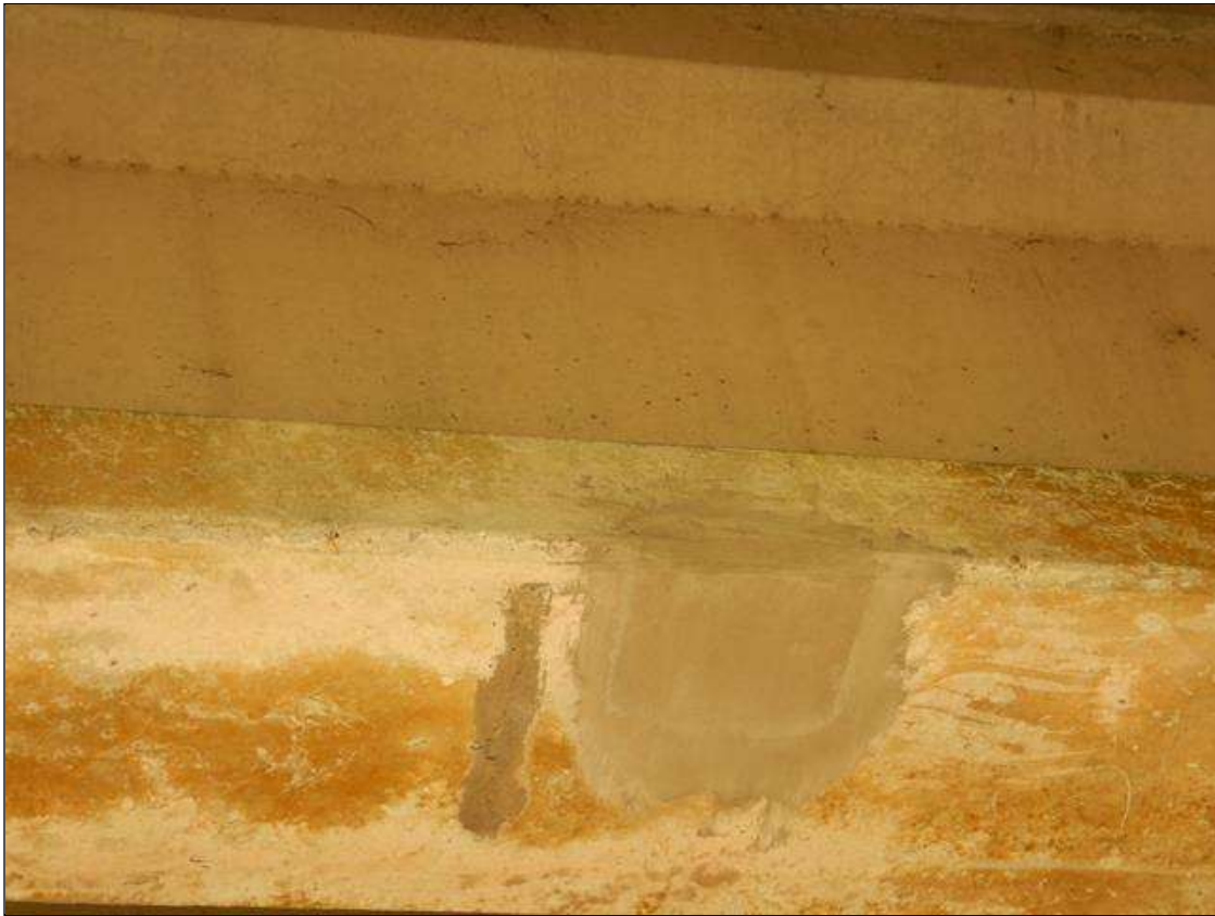
Span 30 Beam 10: [NEW REPAIR-PATCHING] FORMERLY --> spall with exposed rebar on the bottom right flange with exposed strand (11" x 7" x 1") at 6ft from bent 28, strand exposed for 6" long
