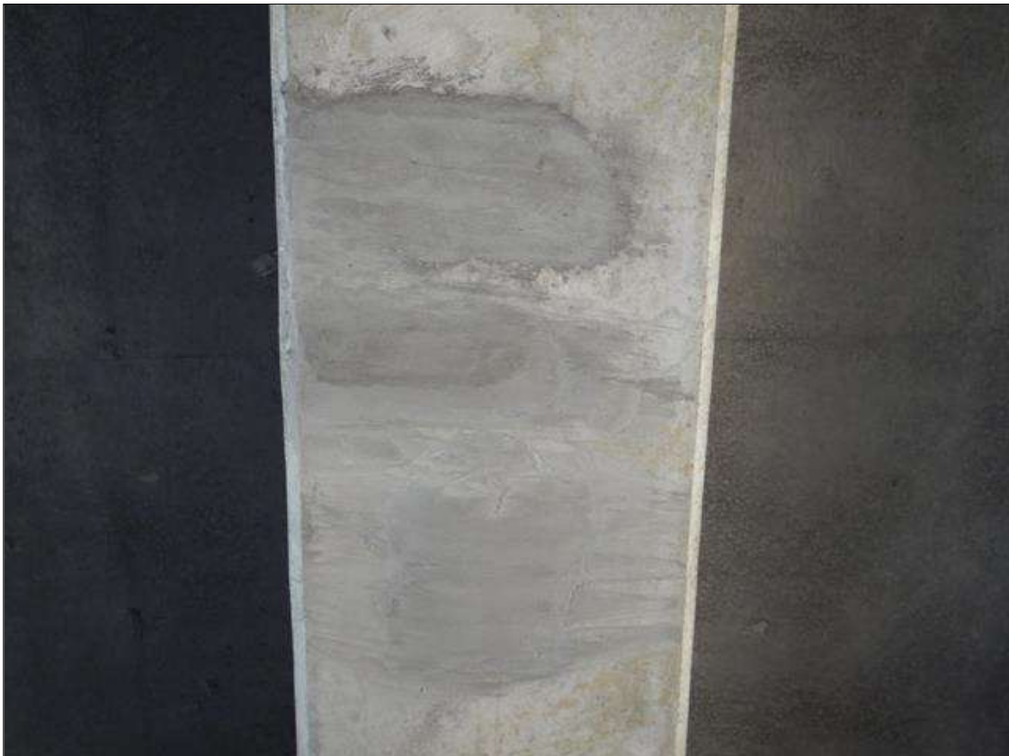
Span 30 Beam 4: [NEW REPAIR-PATCHING] FORMERLY --> Spall with exposed rebar in bottom of girder, approximately 32' from face of Bent 27 Cap
