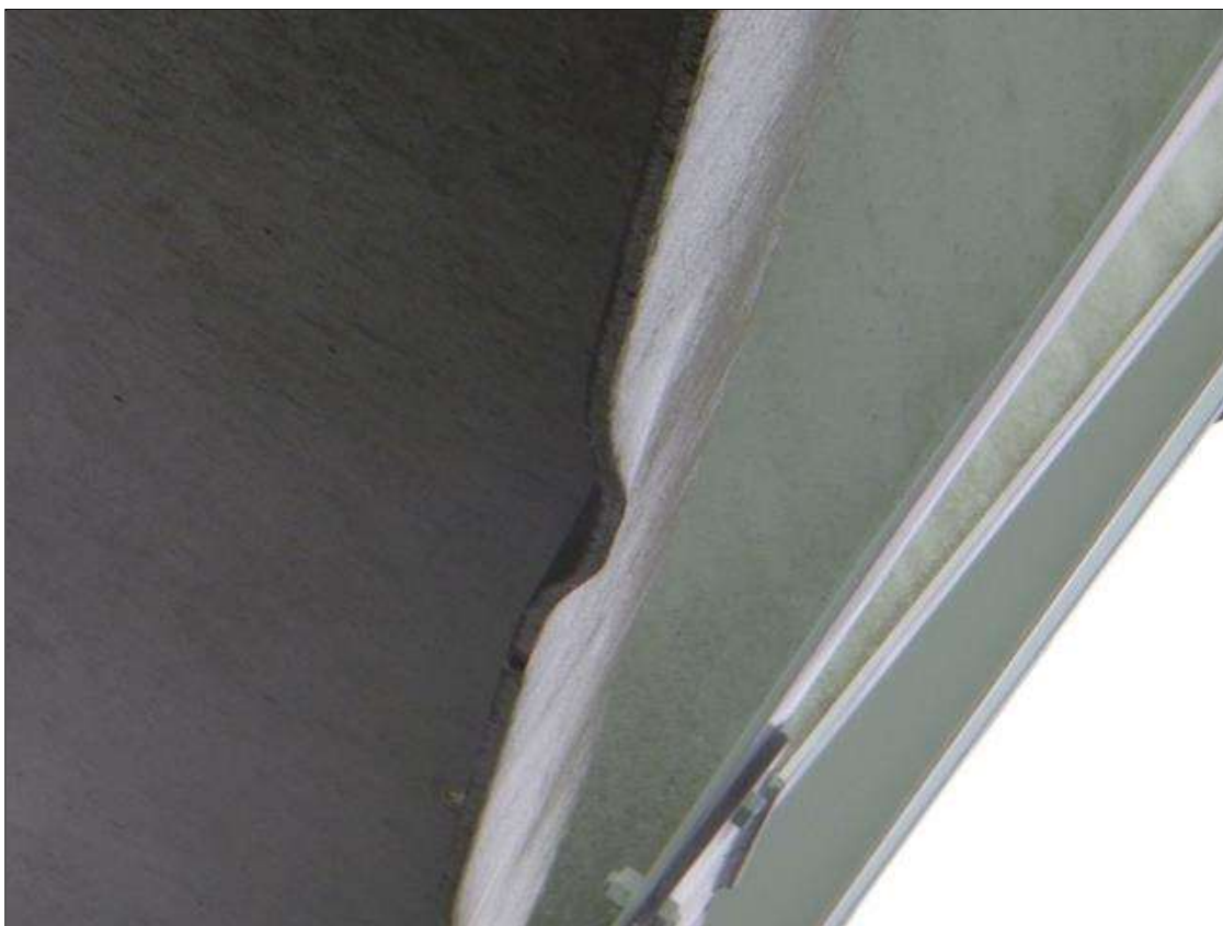
Span 18 Lift Span LB11: BOTTOM SWAY BRACE END PORTAL DAMAGE 1' WIDE X 1/2" DEFORMATION OVER LEFT WEST BOUND LANE.
