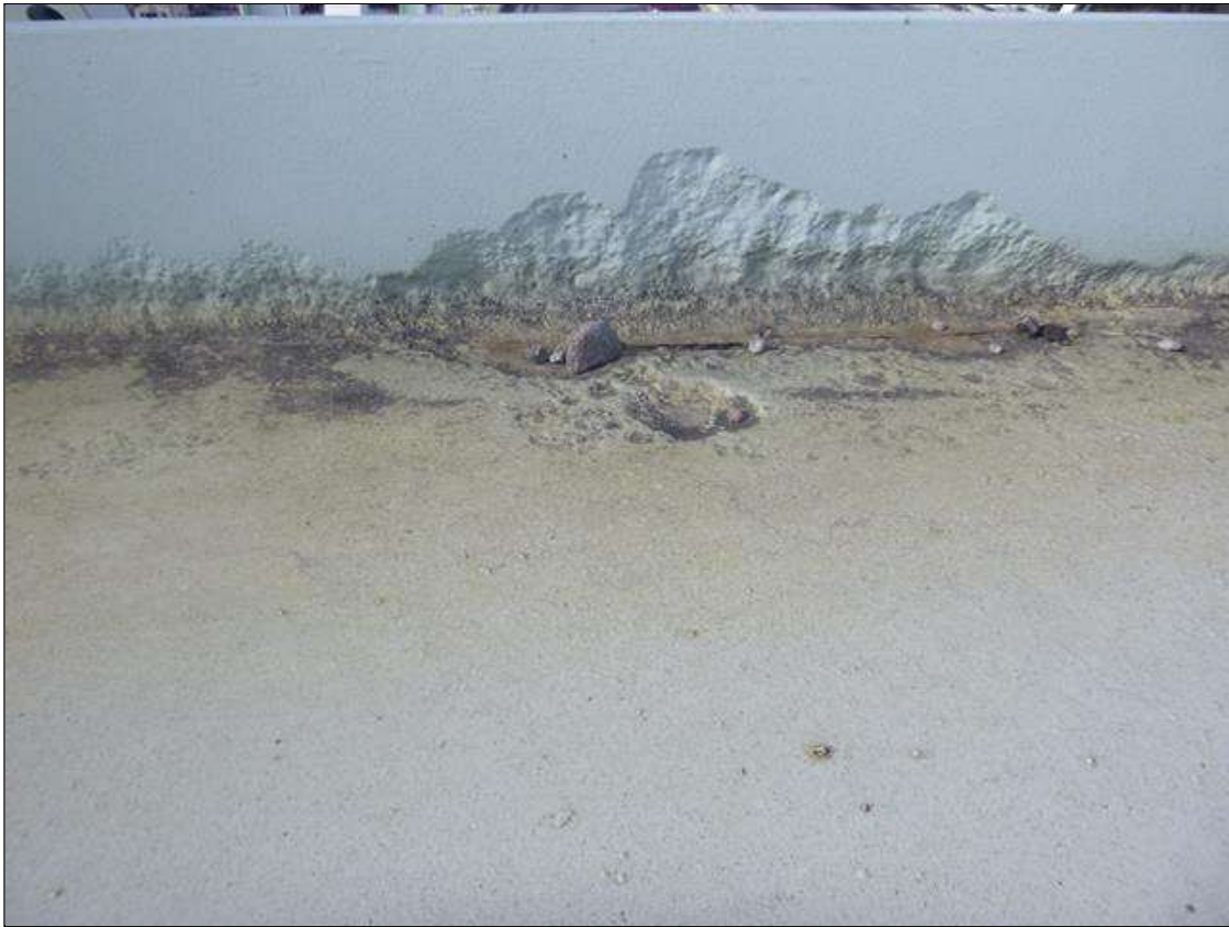
Span 18 Lift Span LB5: LOWER HORIZONTAL CHORD BEGINNING AT SOUTH TRUSS FOR 11' PITTING UP TO 3" WIDE X 1/16" DEEP IN WEB AND WEST FLANGE.
