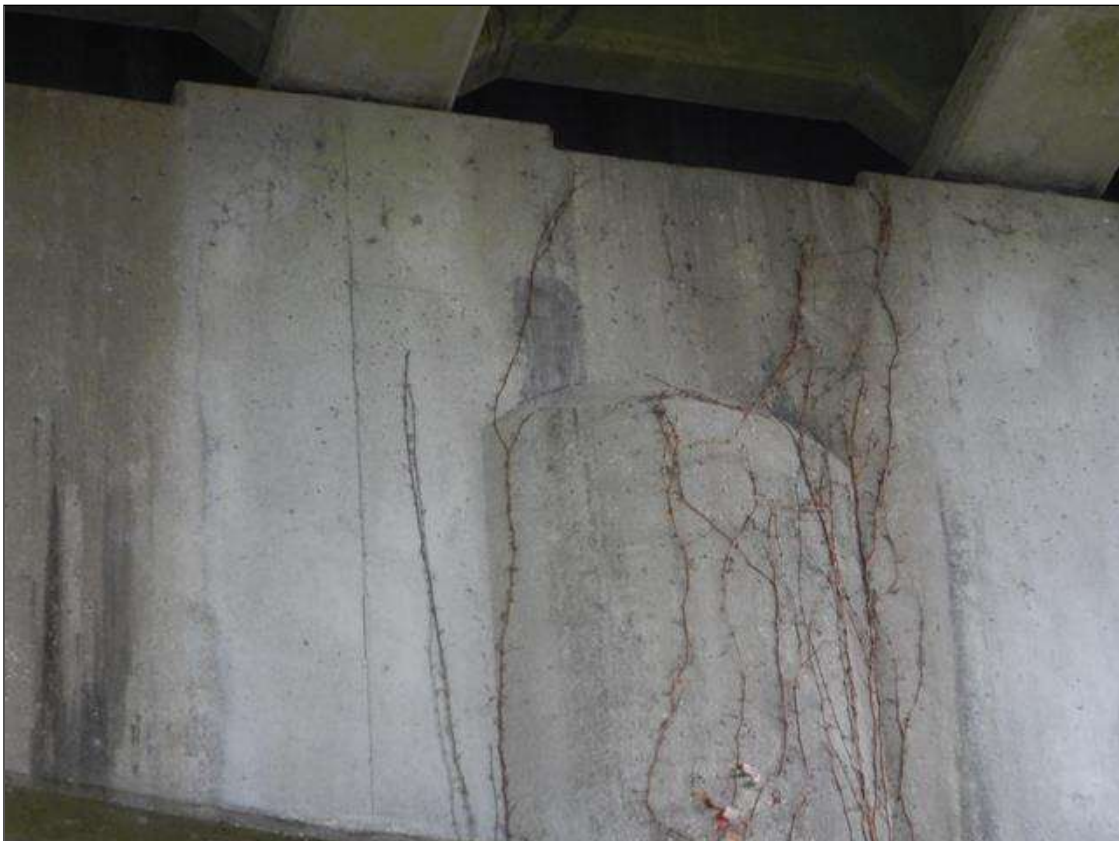
Bent 4 Cap 1: [NEW REPAIR - PATCHING] FORMERLY --> spall with exposed rebar on the east face under girder 3 (16" x 6" x 1")
