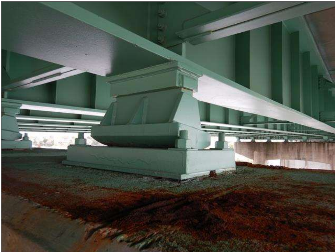
GIRDER 7 BEARING AT BENT 14 [TYPICAL BEARING AT BENT 14]
