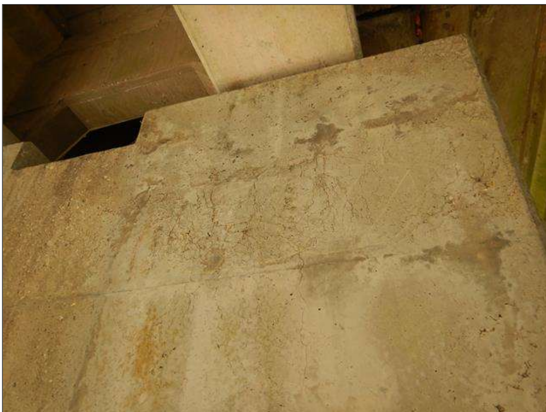
Bent 25 Cap 2: area of delamination on the west face of the cap under girder 8, 20" long x 15" high with hairline map cracking.
