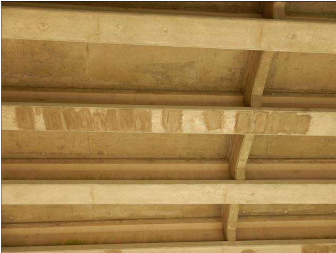
Span 28 Beam 12: [NEW REPAIR-PATCHING] FORMERLY --> 20ft area of DELAMINATION and repairs on the bottom face at mid span up to (18" x 4")
