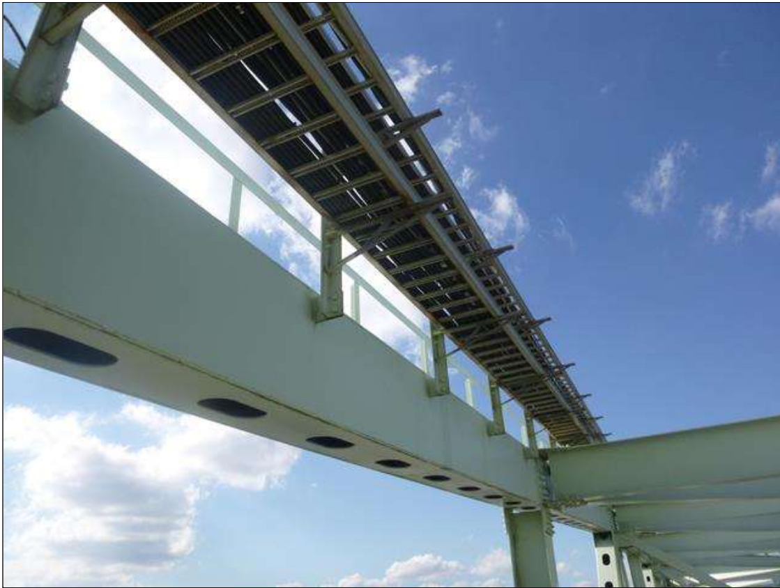
UTILITIES ALONG TOP CHORD SOUTH TRUSS
