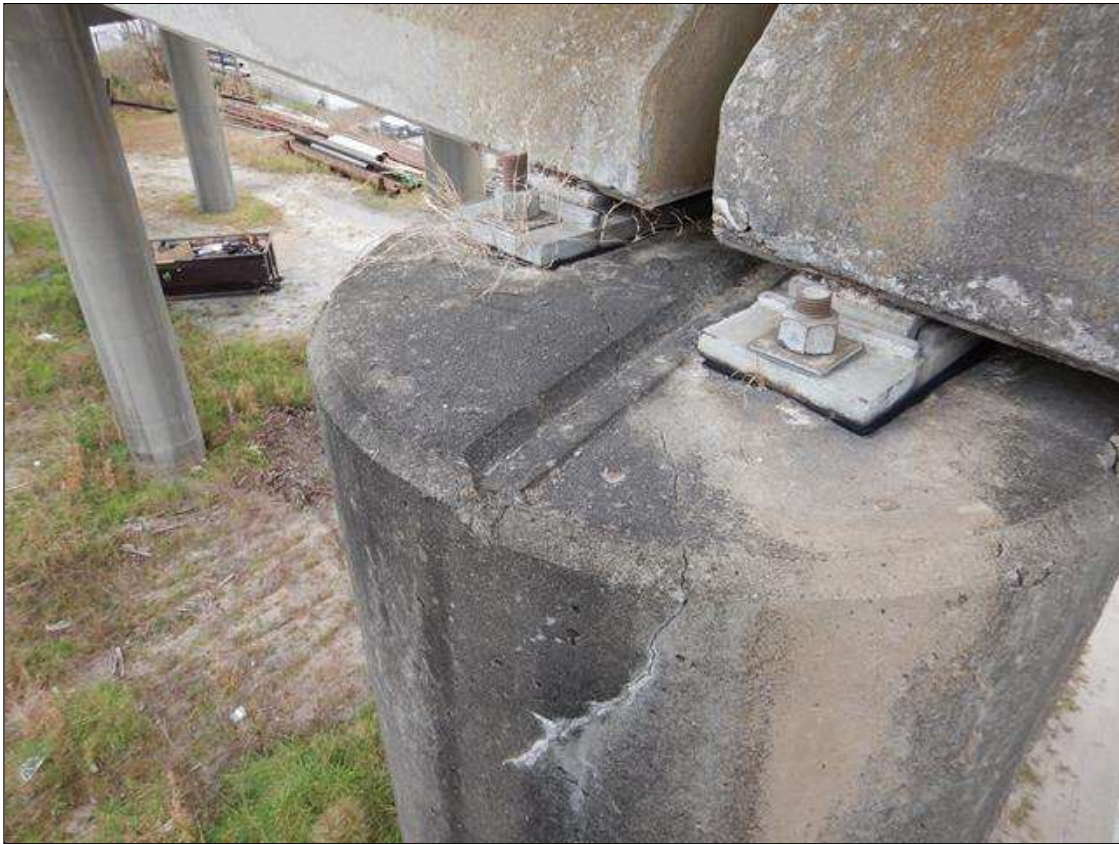
Bent 8 Cap 1: [PROMPT ACTION REQUEST] AT THE SPAN 9 GIRDER 1 NEAR BEARING, OPEN CRACKING TO 3/16" WIDE EMANATES FROM THE LEFT ANCHOR BOLT EXTENDING DOWN THE EAST FACE APPROXIMATELY 4.5', AND THE WEST APPROXIMATELY 1.5'.
