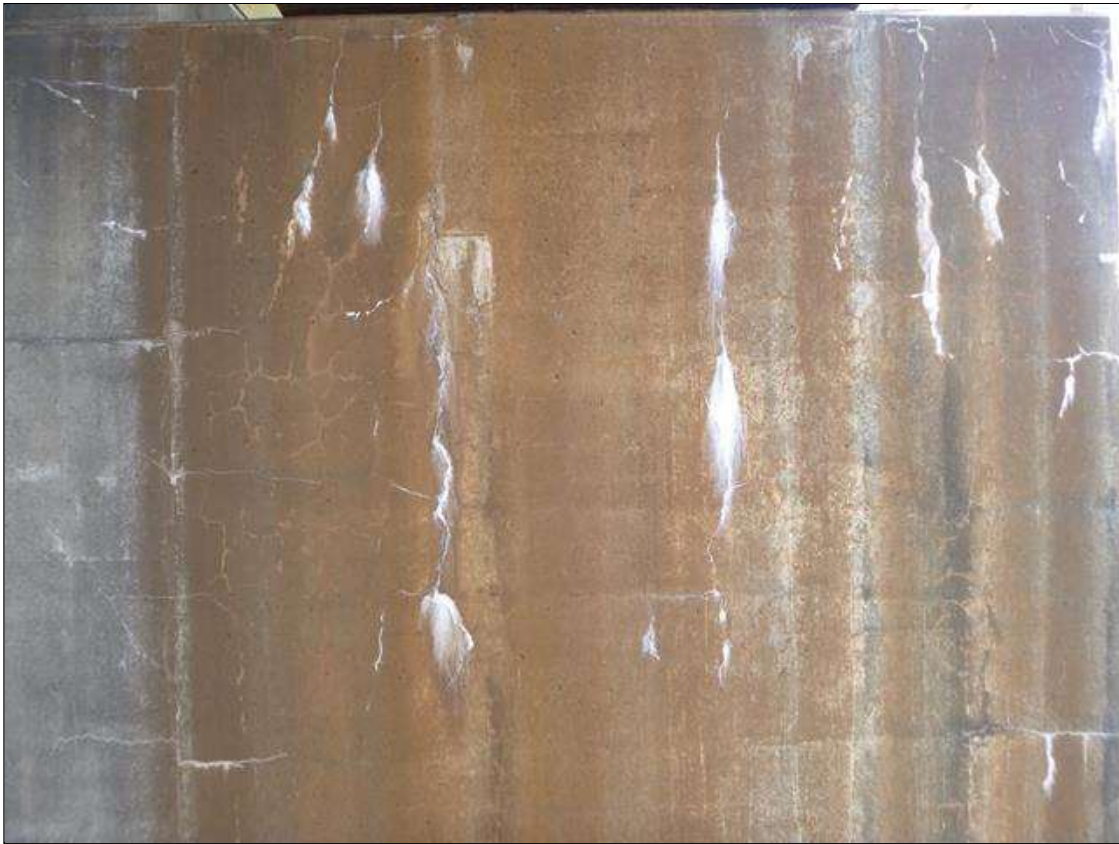
Bent 17 - Lift Span Bent Cap 1: efflorescence build-up on all faces for the full height and width.
