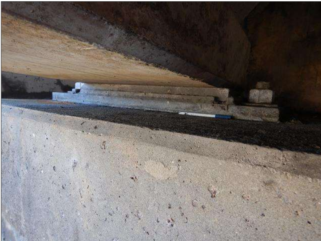
SPAN 35 GIRDER 1 FAR BEARING [TYPICAL BEARING AT THE RAMP ABUTMENT]
