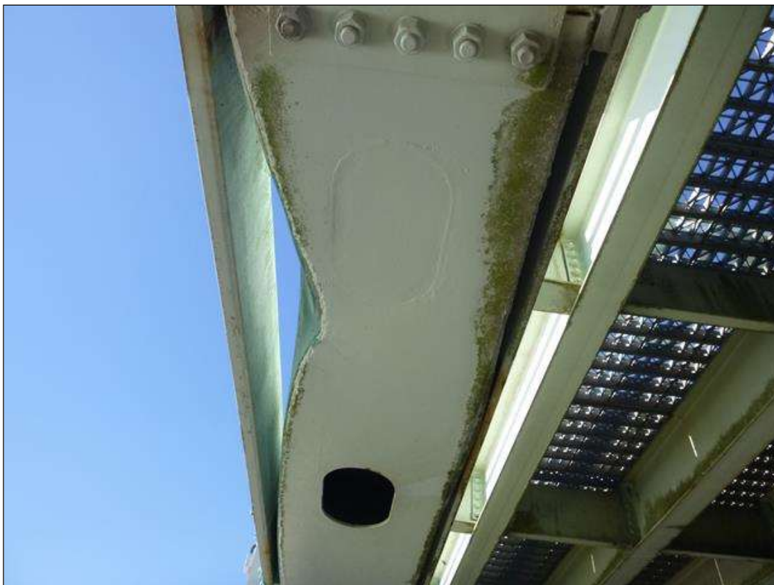
Span 18 Lift Span L5L6 SOUTH: IMPACT DAMAGE REPAIR TO CHORD AT L6
