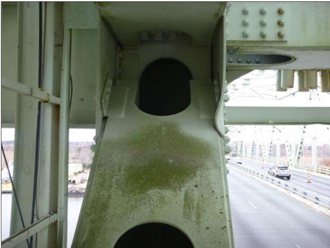
Span 19 EAST TOWER SOUTH: SOUTHWEST TOWER LEG NORTH FACE GUSSET PLATE EAST END 12" X 4" X 1" DISTORTION.
