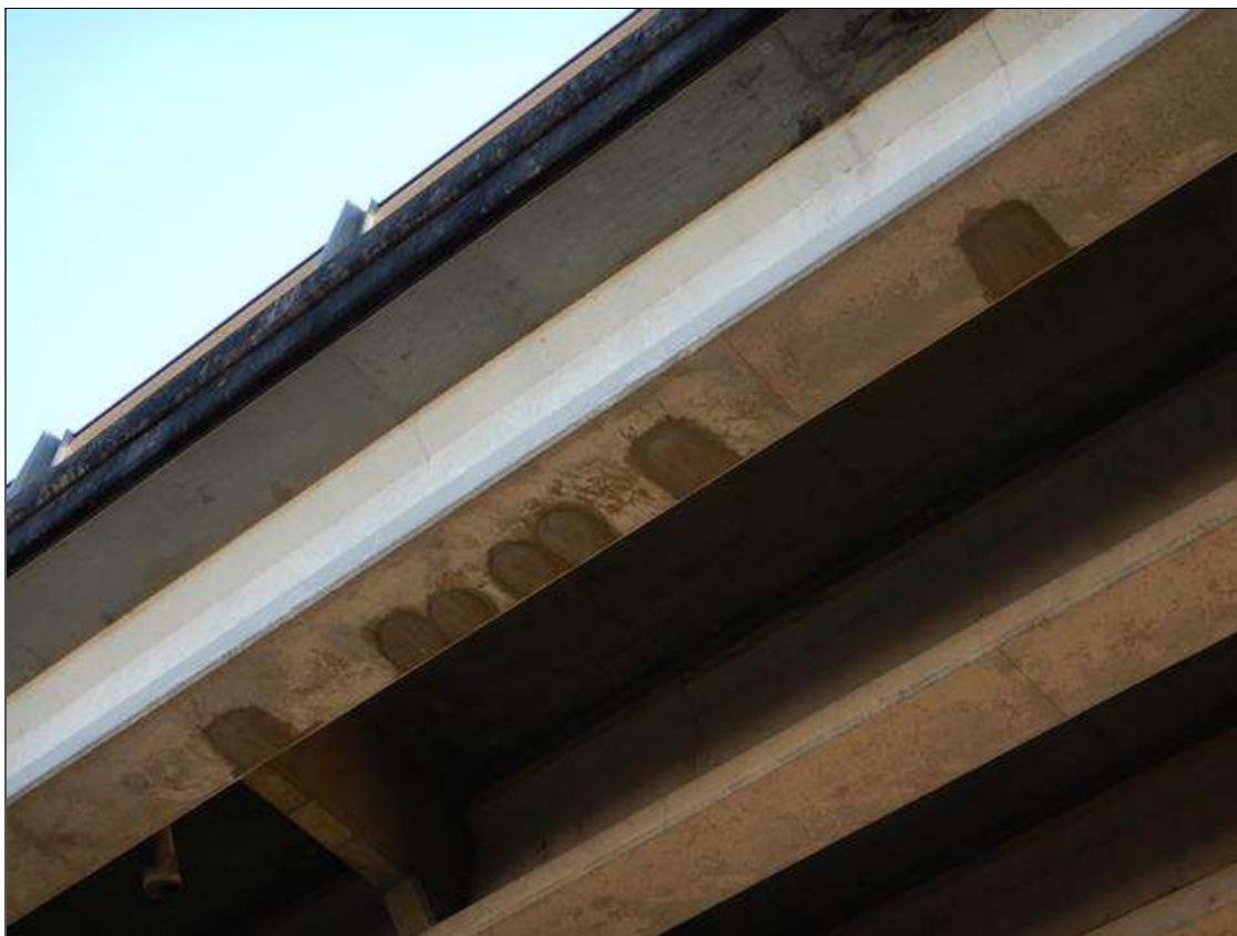
Span 27 Beam 1: [NEW REPAIR-PATCHING] FORMERLY --> (x7) spalls with exposed rebar on the bottom face at mid span up to (7" x 4" x 1/2")
