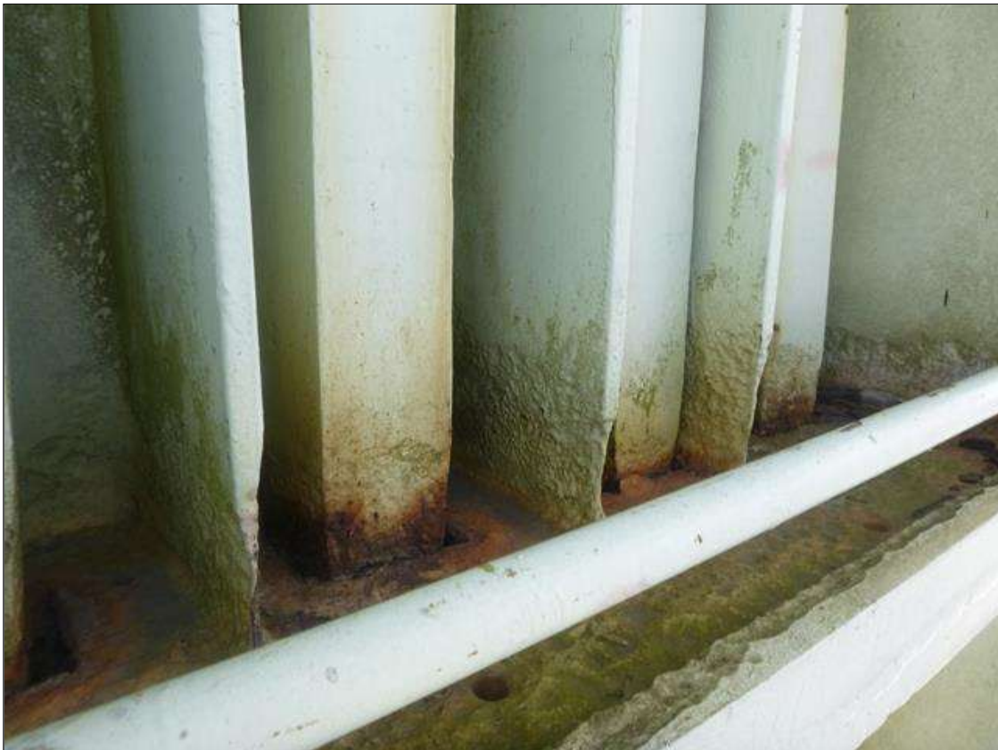
Span 18 Lift Span LB12: [PROMPT ACTION REQUEST] EASTBOUND LANE SOUTHWEST CABLE EYE BAR GUIDE PLATES HAVE LOSS OF SETION .234" WITH .406" REMAINING ALONG BOTTOM 4" HIGH.
