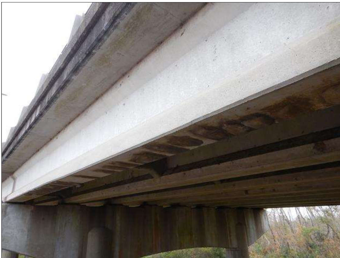
Span 2 Beam 1: [NEW REPAIR - PATCHING] FORMERLY --> multiple spalls with exposed rebar on the bottom face starting at 20.5ft from bent 1 up to (10" x 2 1/2" x 1/2")
