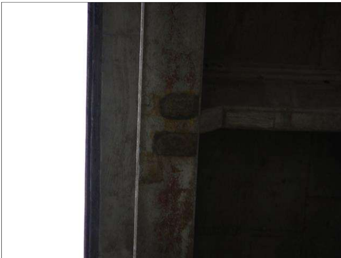
Span 8 Beam 9: [NEW REPAIR - PATCHING] FORMERLY --> 2ft area of (x3) spalls with exposed rebar on the bottom face at 13ft from bent 7 up to (7" x 3" x 1/4")
