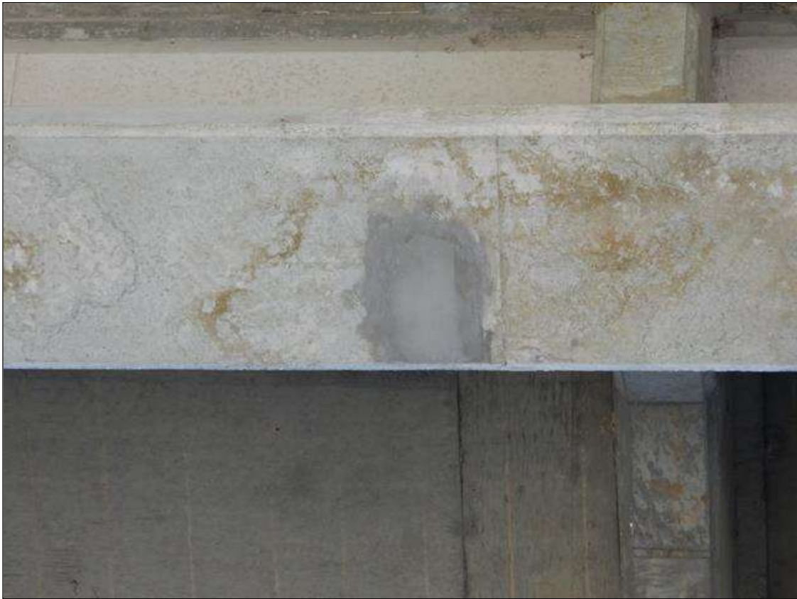
Span 27 Beam 5: [NEW REPAIR-PATCHING] FORMERLY --> spall with exposed rebar on the bottom face at 23ft from Bent 25 (7" x 5" x 1/2")
