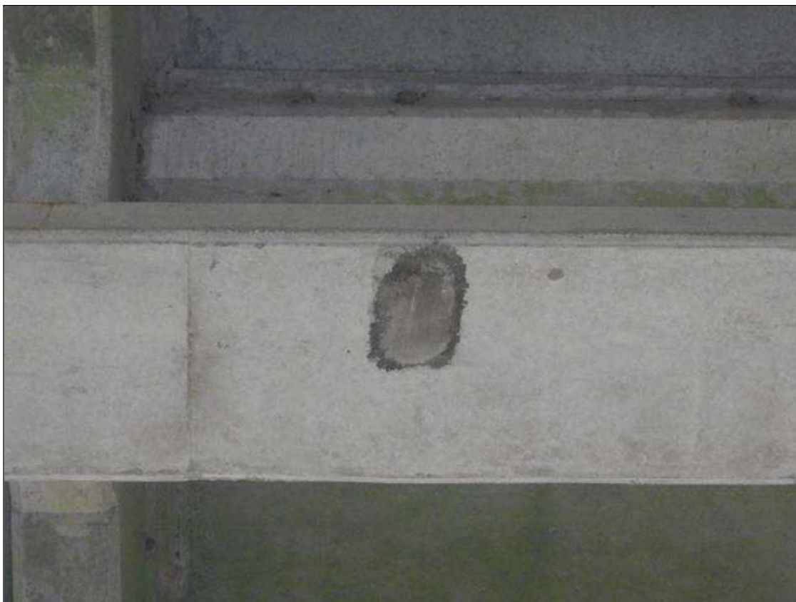
Span 5 Beam 2: [NEW REPAIR - PATCHING] FORMERLY --> (6" x 2" x 1/8") spall with exposed rebar on the bottom face at 24ft from bent 4
