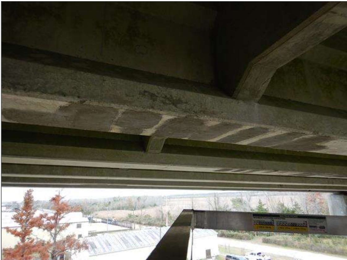
Span 11 Beam 5: [NEW REPAIR - PATCHING] FORMERLY --> (x13) spalls with exposed rebar on the bottom face up to (17" x 5" x 1/2") starting at 16.5ft from bent 11
