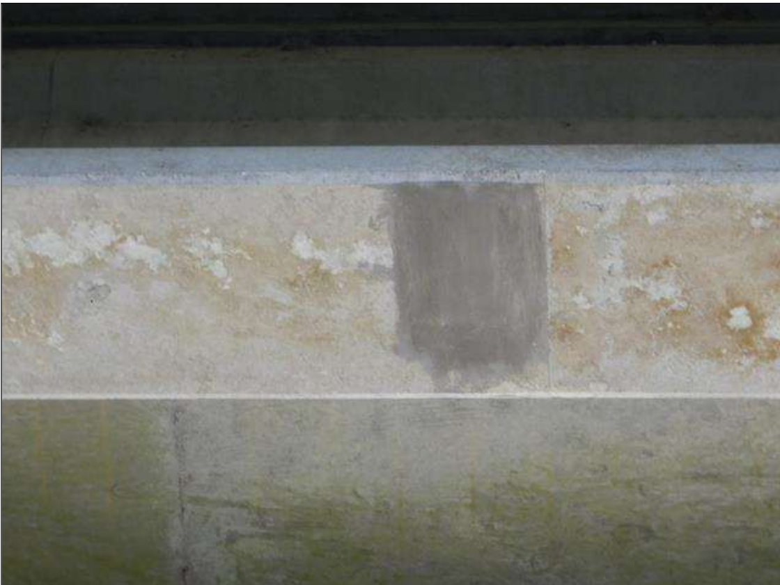
Span 27 Beam 6: [NEW REPAIR-PATCHING] FORMERLY --> spall with exposed rebar on the bottom face at 16ft from bent 25 (4" x 3" x 1/4")
