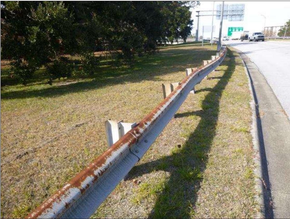
SOUTHEAST CORNER, THE GUARDRAIL HAS SCATTERED MINIMAL IMPACT DAMAGE ALONG THE LENGTH [APPROXIMATELY 80' LONG AFFECTED]
