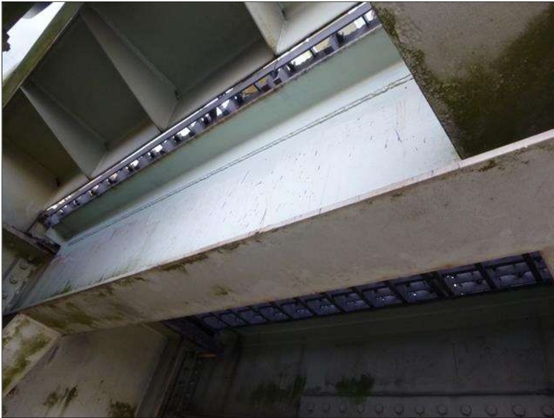
Span 18 Lift Span Stringer 1: REPAIR OBSERVED IN 2021 INSPECTION BETWEEN FB 11 - 12, BEGINNING AT FLOORBEAM 12 FOR 7.5' A 5" X 3.5" X 3/8" THICK ANGLE HAS BEEN WELDED TO BOTH SIDES OF THE TOP FLANGE AND WEB, 2018 REPORT HAD BETWEEN FB's 11-12 - SECTION LOSS TO KNIFE EDGE IN AREAS UP TO 2-1/2"WIDE x 6"LONG SCATTERED ALONG NORTH AND SOUTH SIDES OF TOP FLANGE - UP TO 1" REDUCTION IN FLANGE WIDTH AT SOME LOCATIONS - CLEANED AND PAINTED
