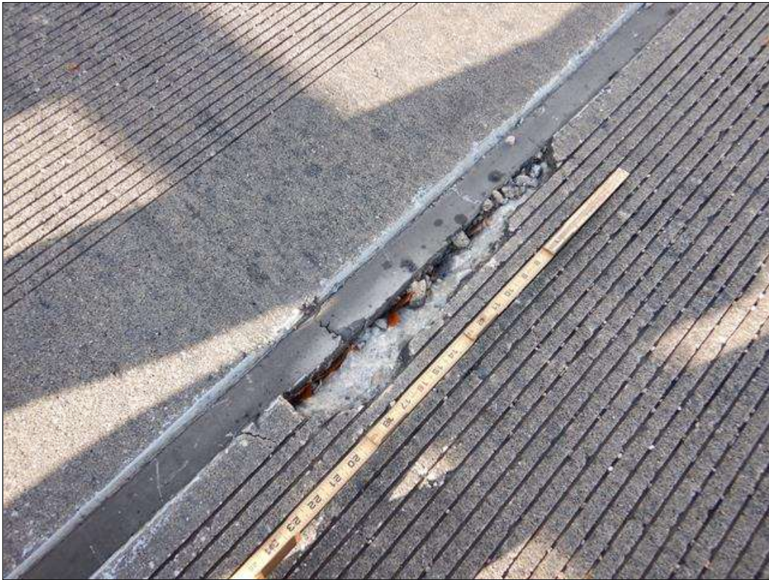
Span 5 Deck: [PROMPT ACTION REQUEST] RIGHT LANES AT BENT 4, TWO SPALLS (18" LONG x 3" WIDE x 1.5" DEEP AT 8' FROM RIGHT CURB) & (8" LONG x 2" WIDE x 3" DEEP AT 2' FROM CENTERLINE)
