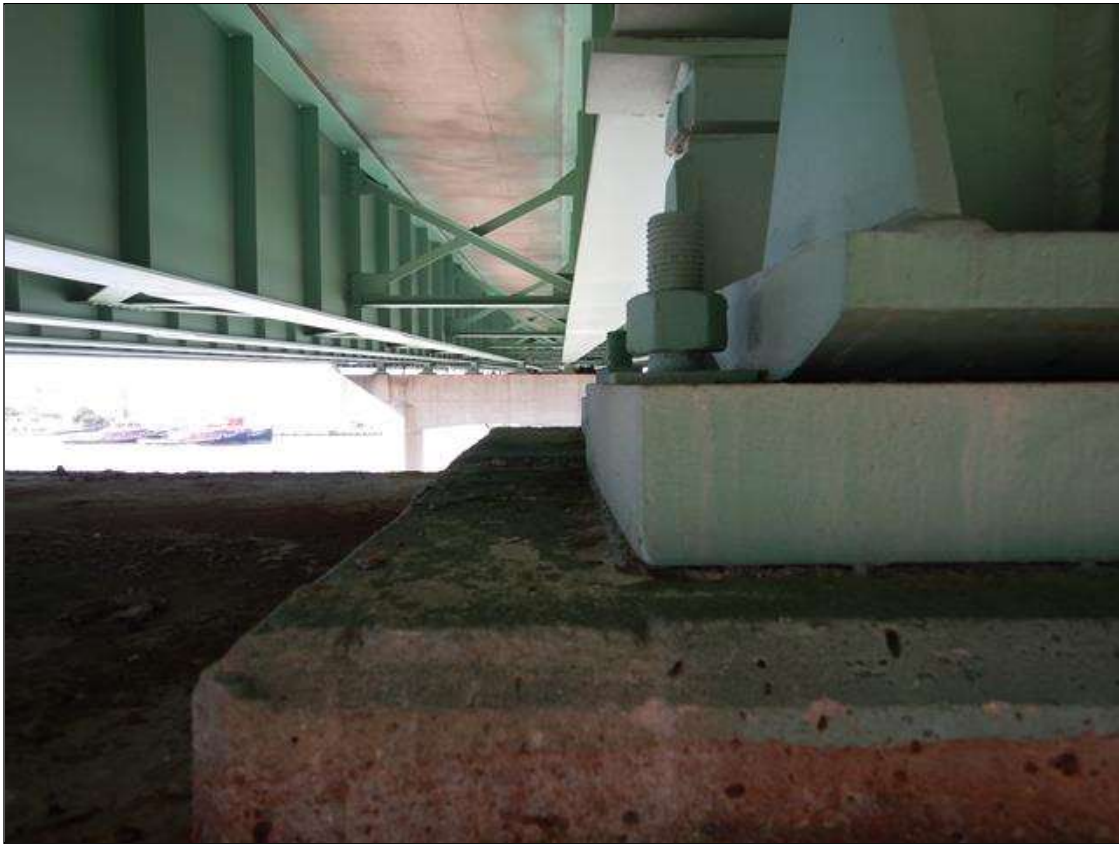
Span 22 Beam 3 - Beam 3 Near Bearing: [PROMPT ACTION REQUEST] RIGHT ANCHOR BOLT LIFTED 3/4"
