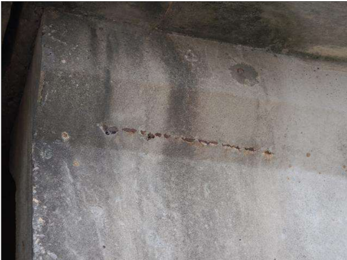
Span 8 Beam 1: [PROMPT ACTION REQUEST] (16" x 1") area of exposed rebar in the top left chamfer at bent 8
