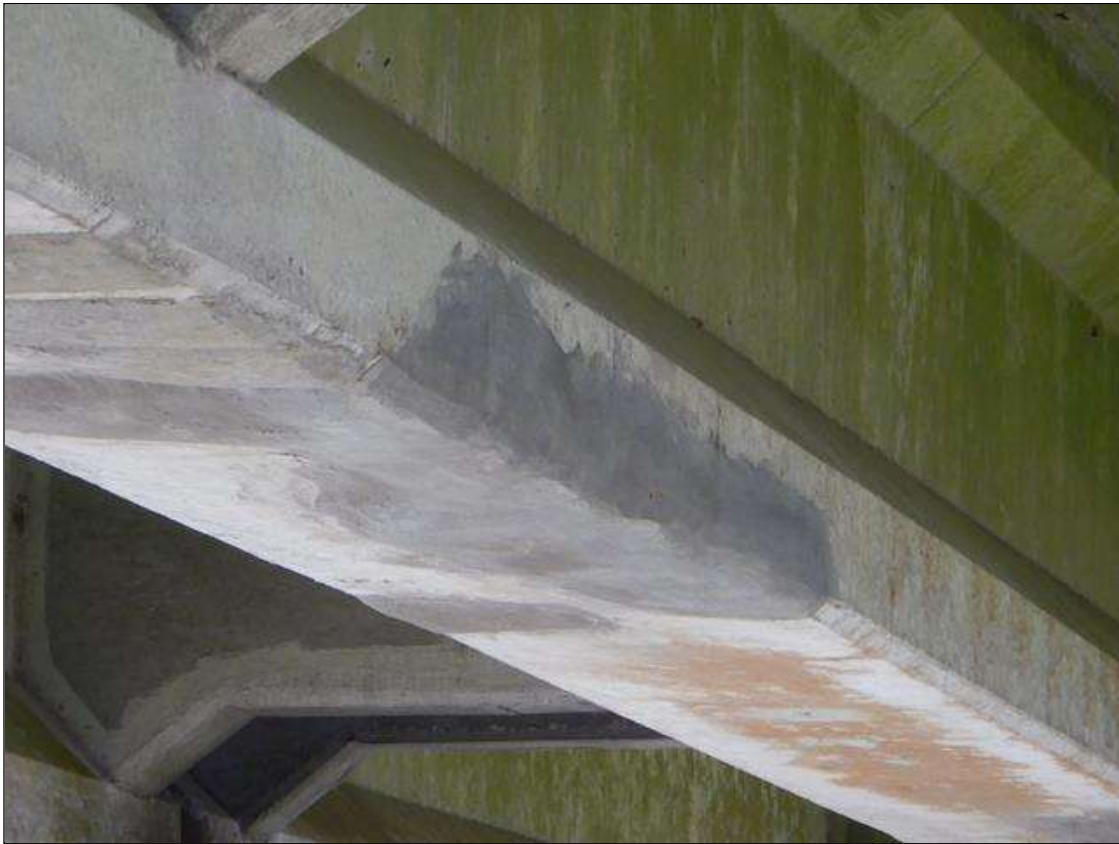
Span 11 Beam 6: [NEW REPAIR - PATCHING] FORMERLY --> (16" x 5" x 1") area of DELAMINATION and cracking up to 0.02" wide on the bottom and left faces at 14ft from bent 10
