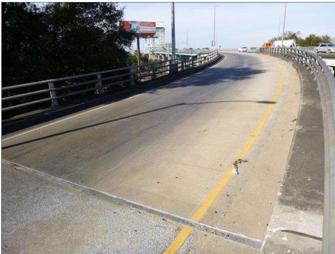
SPAN 35 EPOXY OVERLAY WEARING SURFACE [SPANS 33 & 34 SIMILAR]
