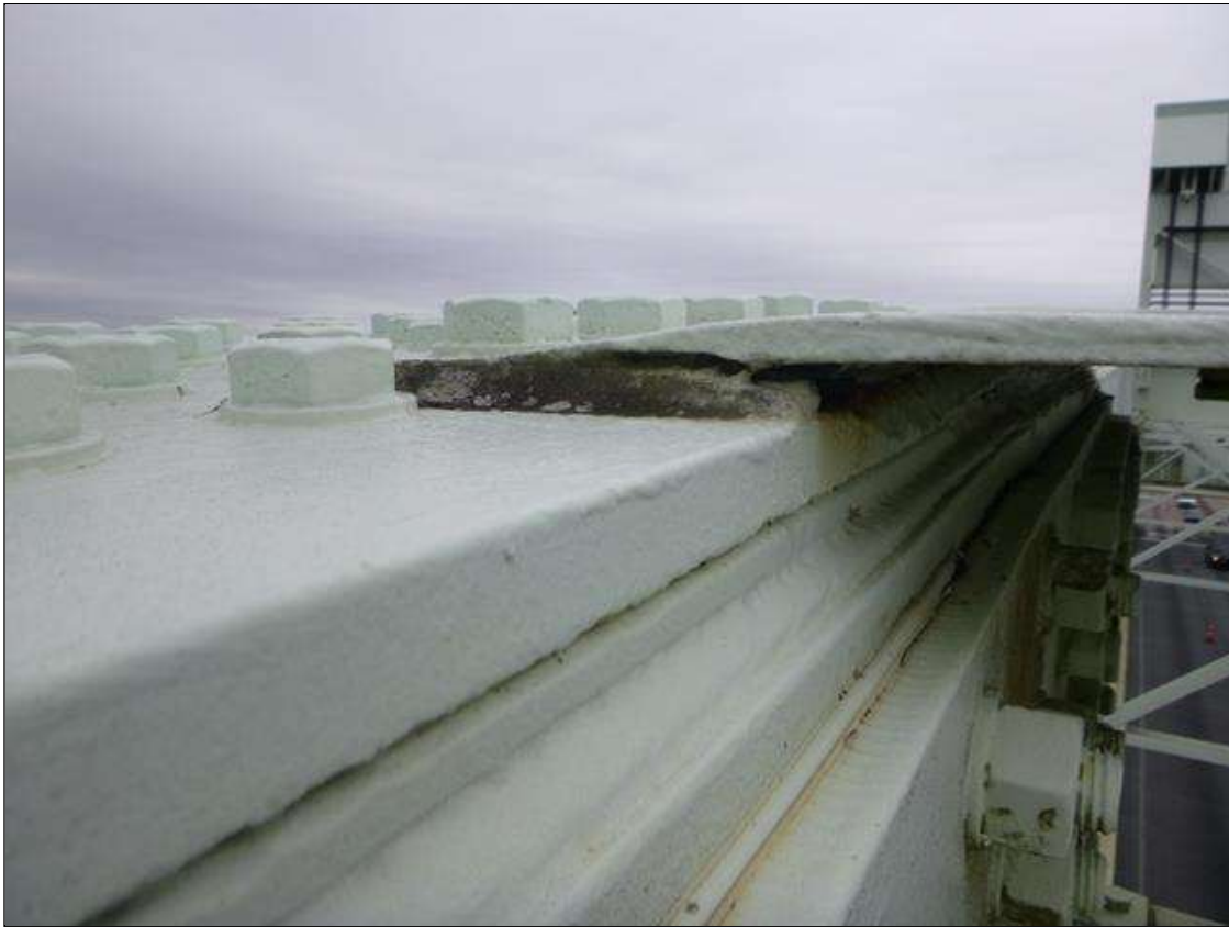
Span 18 Lift Span Truss Panel 1 - U3 NORTH: TOP GUSSET PLATE: OUT OF PLANE BENDING \frac{1}{2} " DUE PACK RUST WITH \frac{1}{8} " LOSS OF SECTION AND \frac{1}{4} " REMAINING ALONG PLATE EDGES. (PAR)
