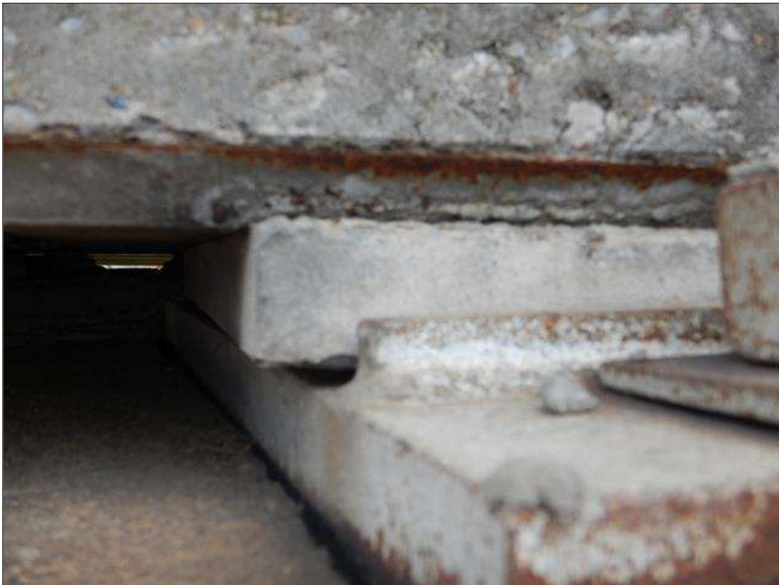
Span 8 Beam 1 - Beam 1 Near Bearing: up to (9/16") movement of bearing to the east beyond the masonry plate with up to 9% bearing loss.
