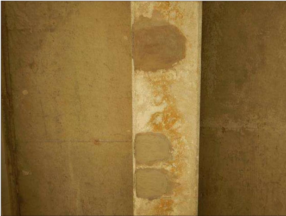
Span 28 Beam 10: [NEW REPAIR-PATCHING] FORMERLY --> (x3) spalls with exposed rebar on the bottom face at 12ft from Bent 25 up to (5" x 5" x 1/2")
