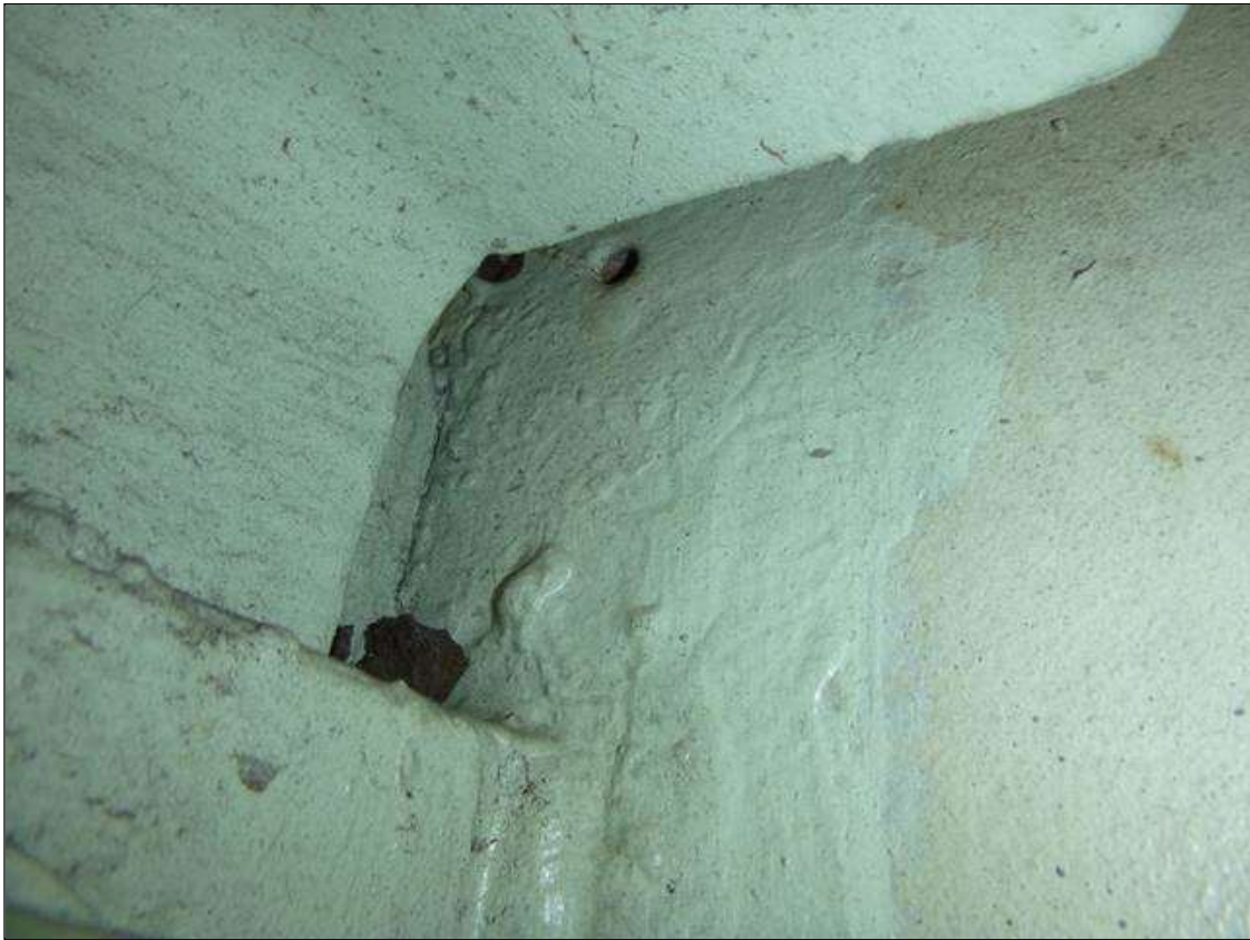
Span 18 Lift Span Stringer 8: BETWEEN FB's 11-12 - CRACK PROPAGATED 1/4" PAST EAST ARREST HOLE AT TOP OF DIAPHRAGM CONNECTION – PROMPT ACTION REQUEST
