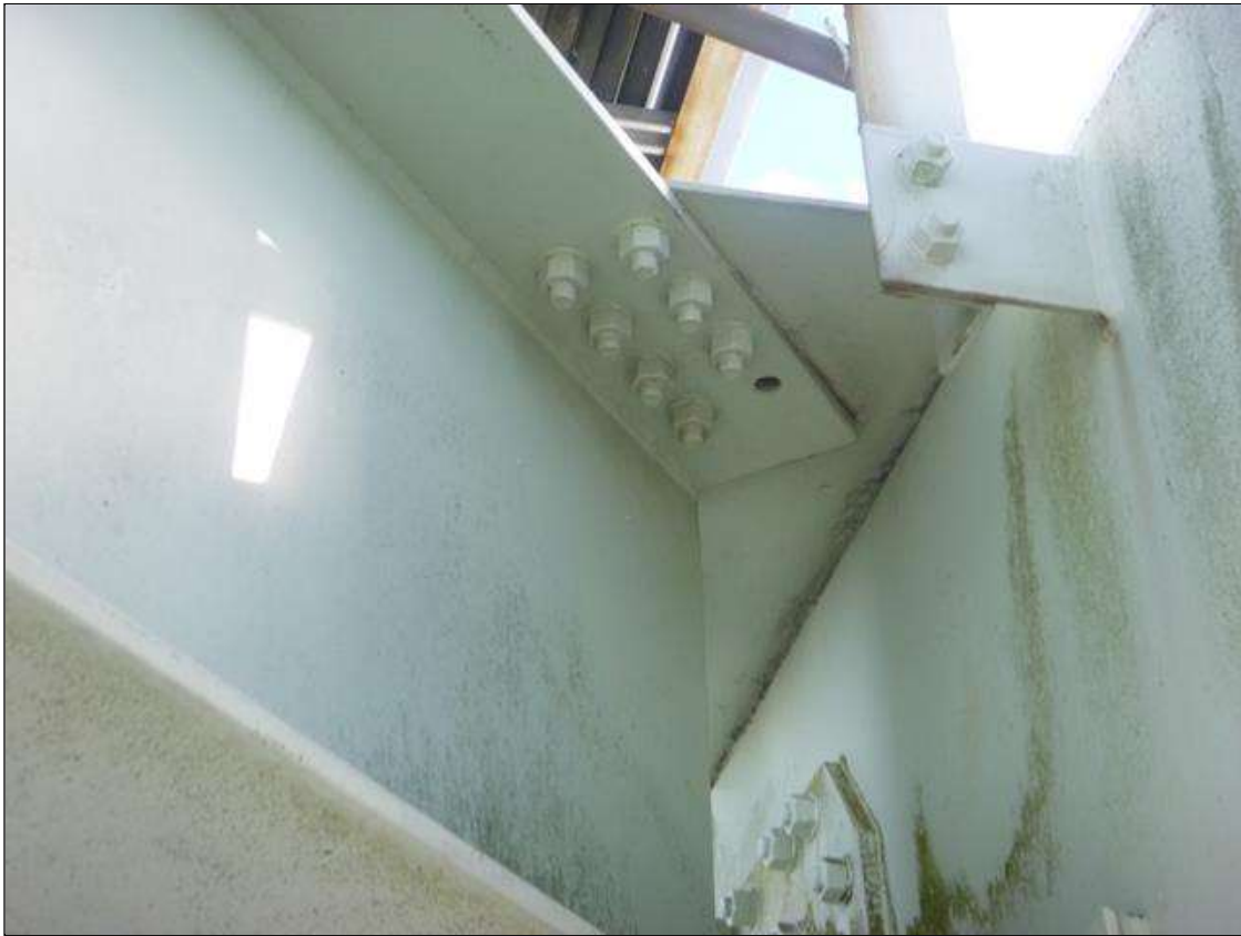
Span 18 Lift Span U8 SOUTH: EAST SIDE TOP CONNECTION TO LATERAL BRACING MISSING (1) BOLT
