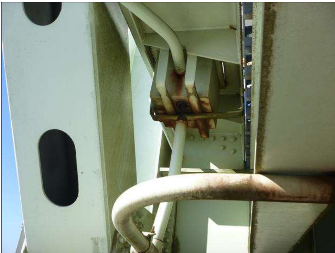
AT L2 SOUTH SIDE BROKEN CONDUIT.
