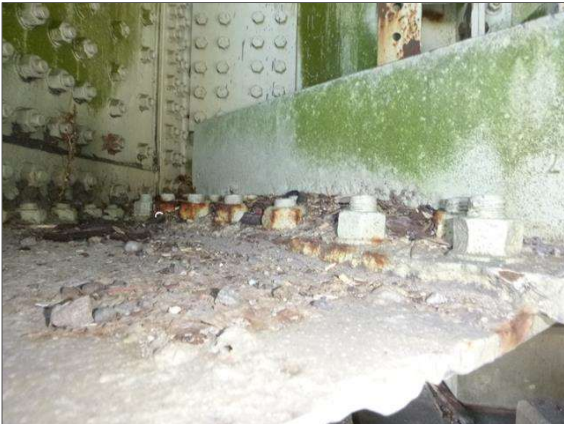
Span 18 Lift Span Floor Beam 12: LATERAL BRACING FROM FLOORBEAM 11 TO U12 AT U12 SURFACE RUST ON BOLTS.
