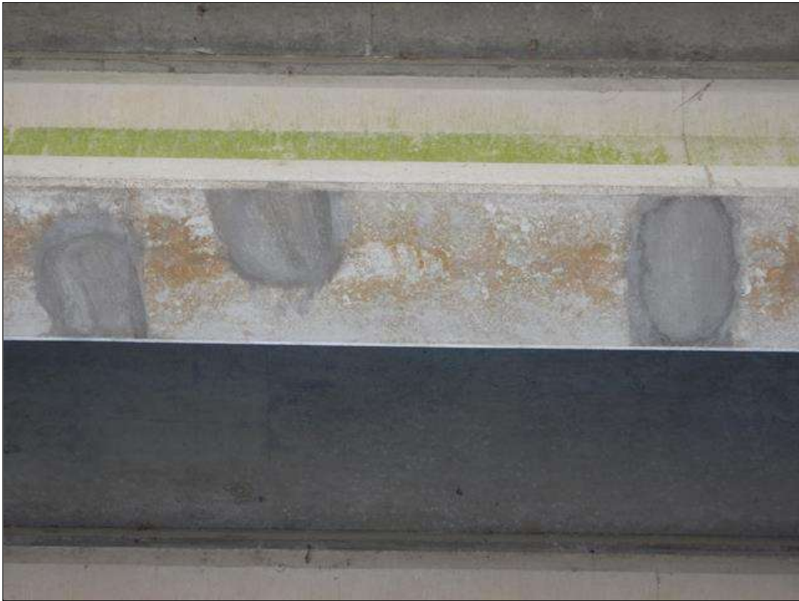
Span 28 Beam 5: [NEW REPAIR-PATCHING] FORMERLY --> (x3) spalls with exposed rebar on the bottom face starting at 22.5ft from Bent 26 up to (6" x 4" x 1/2")
