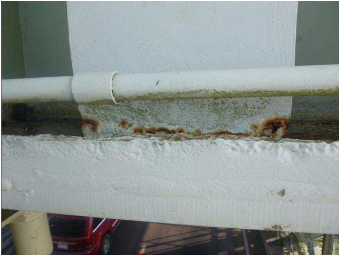
Span 18 Lift Span LB12: [PROMPT ACTION REQUEST] EASTBOUND LANE: 2ND STIFFNER RIGHT OF NORTHWEST CABLE BANK LOSS OF SECTION .334" WITH .321" REMAINING ALONG BOTTOM 4-1/2" HIGH ON WEST FLANGE.
