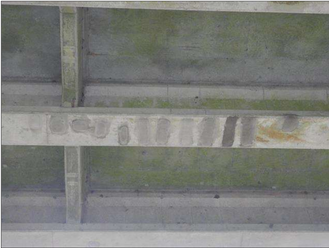
Span 5 Beam 2: [NEW REPAIR - PATCHING] FORMERLY --> mutiple (x13) spalls with exposed rebar on the bottom face starting at 11ft from bent 5 up to (14" x 2" x 1/4")
