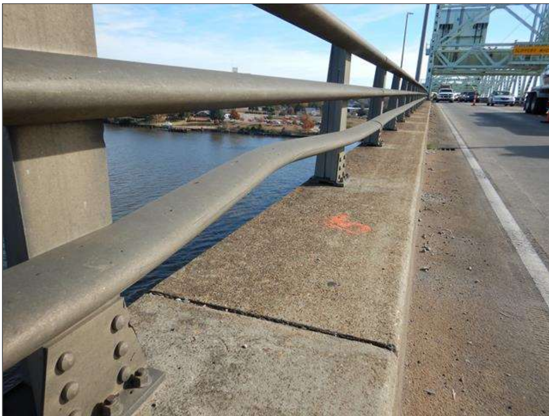
Span 15 Left Bridge Rail: (84" x 3 1/2") impact damage to the bottom rail at 38ft from bent 14
