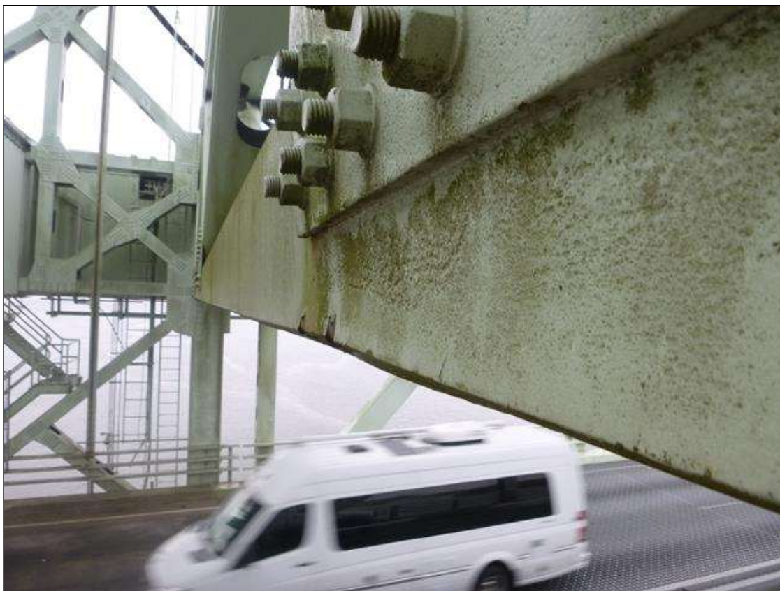
Span 19 EAST TOWER NORTH: 6/2020 - IMPACT DAMAGE - BOTTOM WEST HORIZONTAL TRUSS MEMBER - 3'L SECTION ON EAST SIDE BENT 1/2" TO THE WEST - LOCATED 11'-3" FROM NORTHWEST TOWER LEG (PAR)
