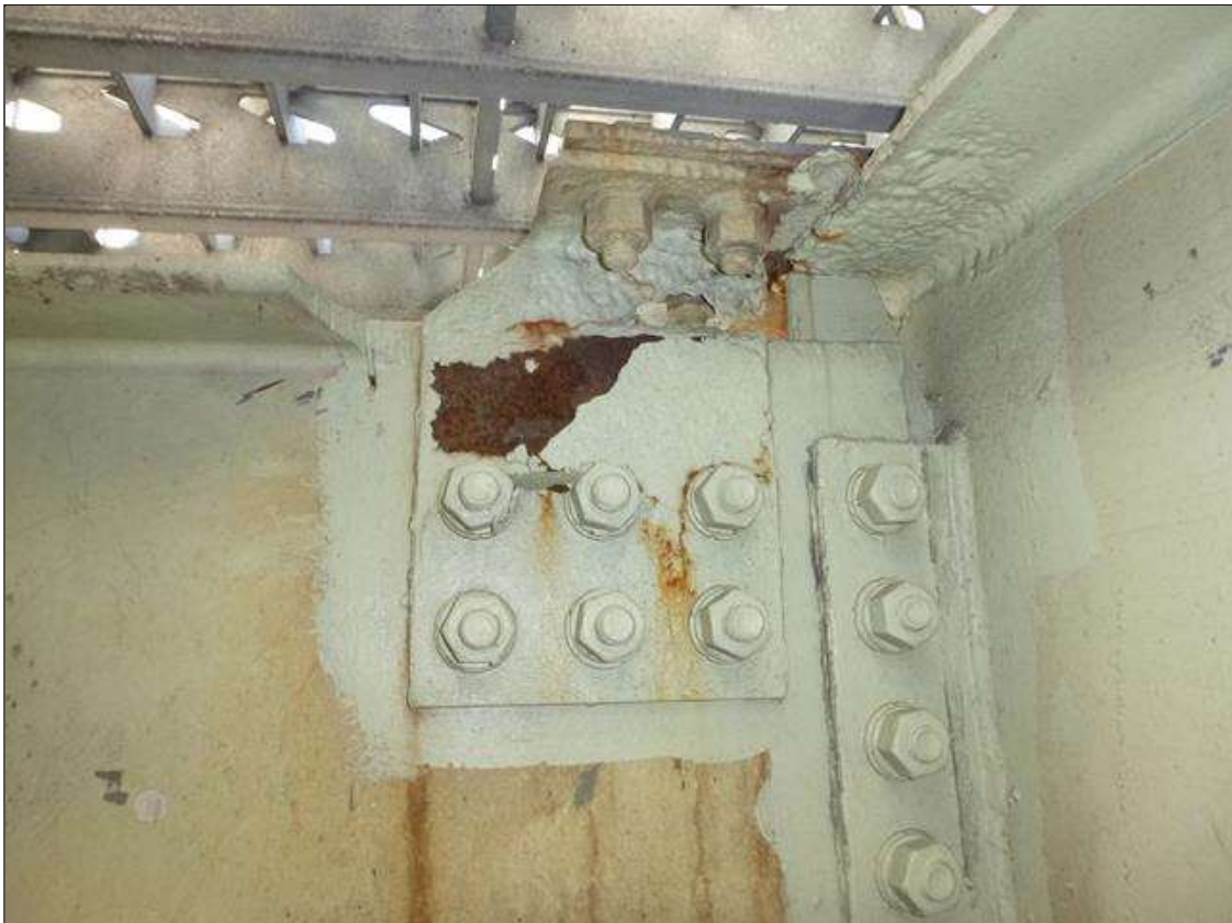
Span 18 Lift Span Stringer 14: (PAR) BETWEEN FB's 0-1 INTERMEDIATE DIAPHRAGM CONNECTOR PLATE CORROSION HOLE 5" X 1.5"
