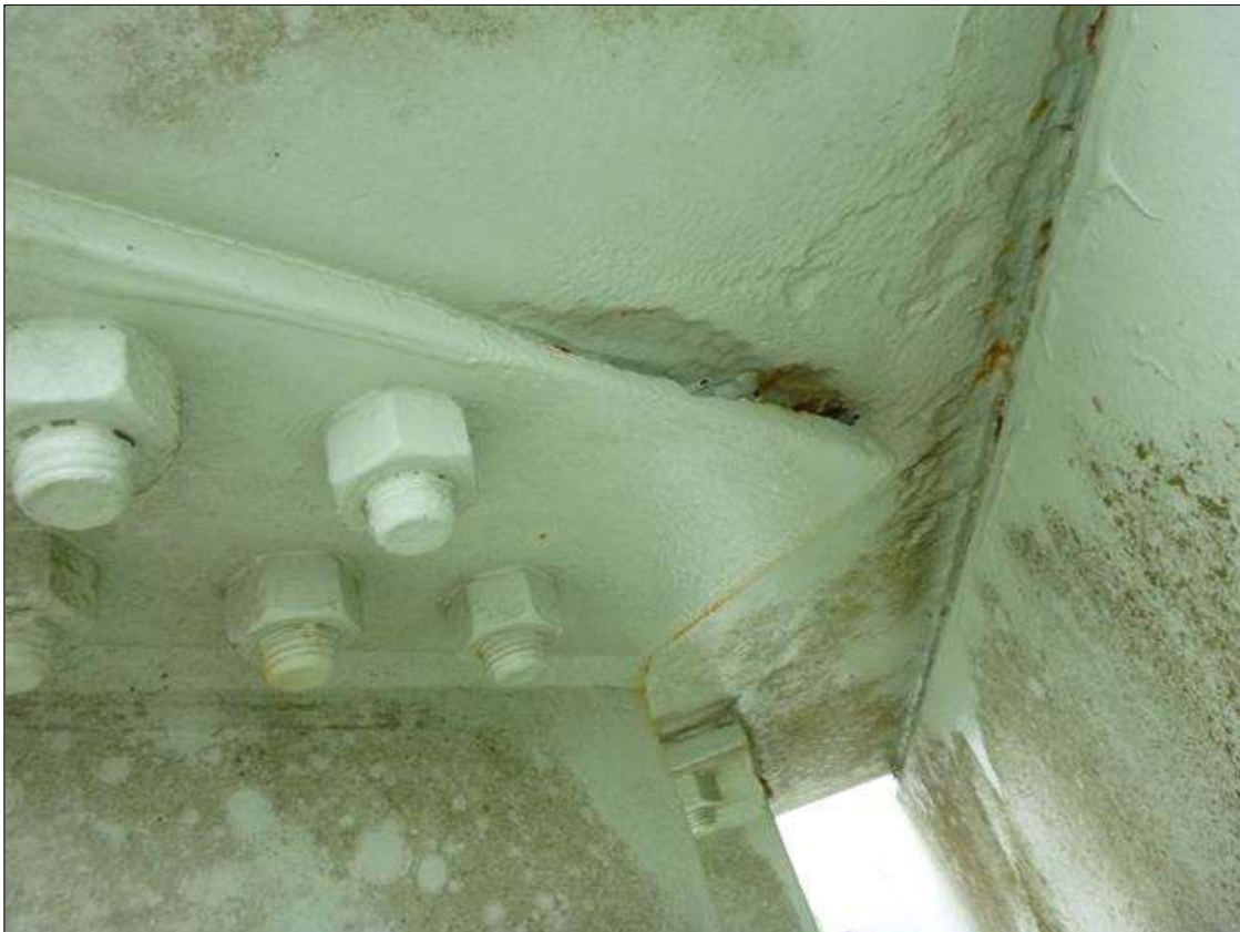
Span 18 Lift Span U4 NORTH: BOTTOM OF TOP GUSSET PLATE AT EAST DIAGONAL BRACE 7" X 1" X 3/16" DEEP PITTING CLEANED AND PAINTED.
