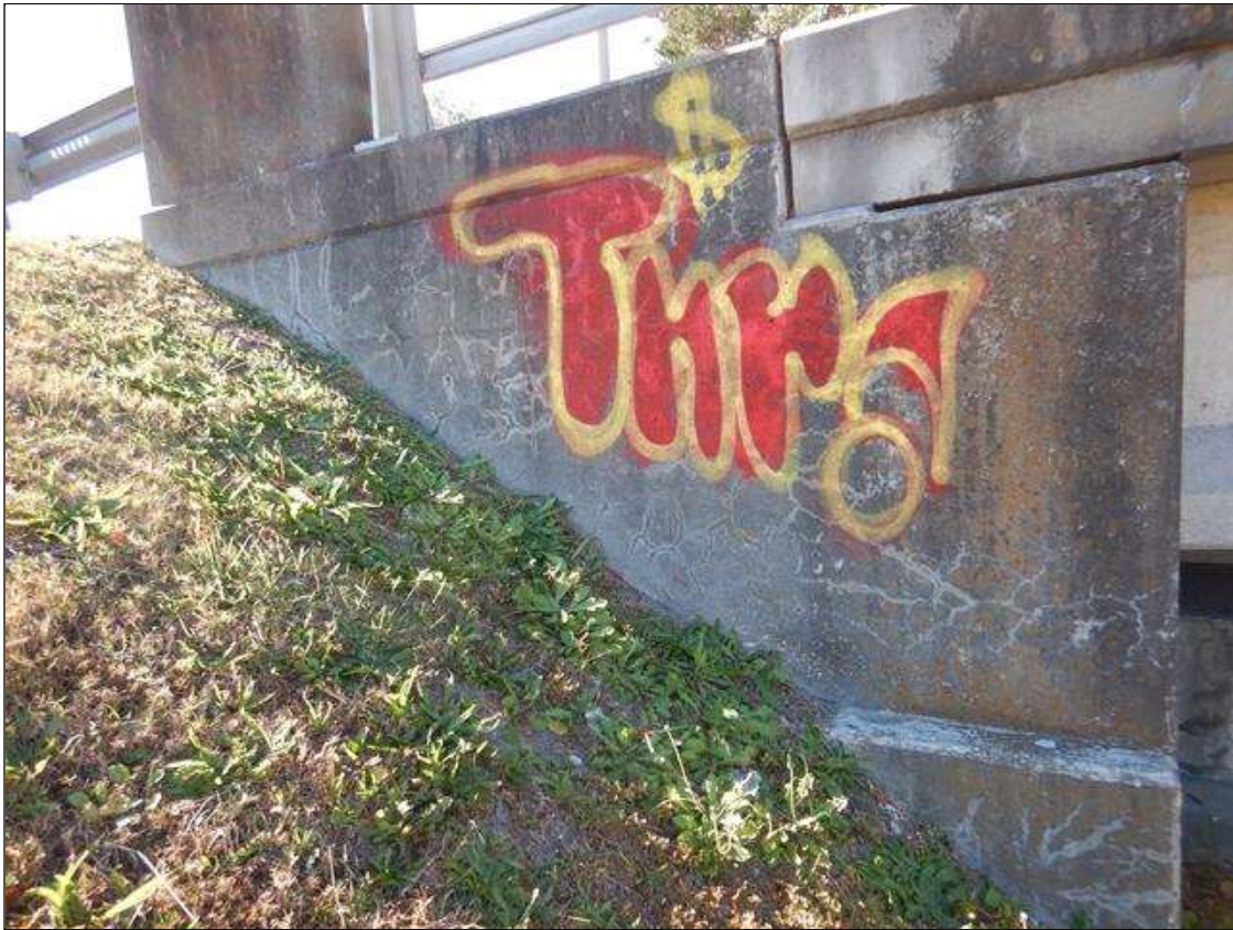
Ramp End Bent Abutment: area of hairline map cracking on the left side of ramp bridge abutment, 10 FOOT. long with EFFLORESCENCE.
