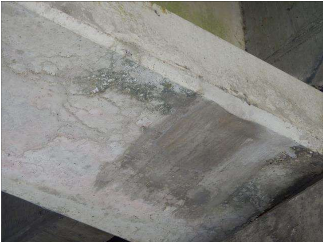
Span 35 - Ramp Span Beam 4: [NEW REPAIR-PATCHING] FORMERLY --> spall with exposed rebar on the bottom face at 1ft from bent 31 (7" x 6" x 1/2")
