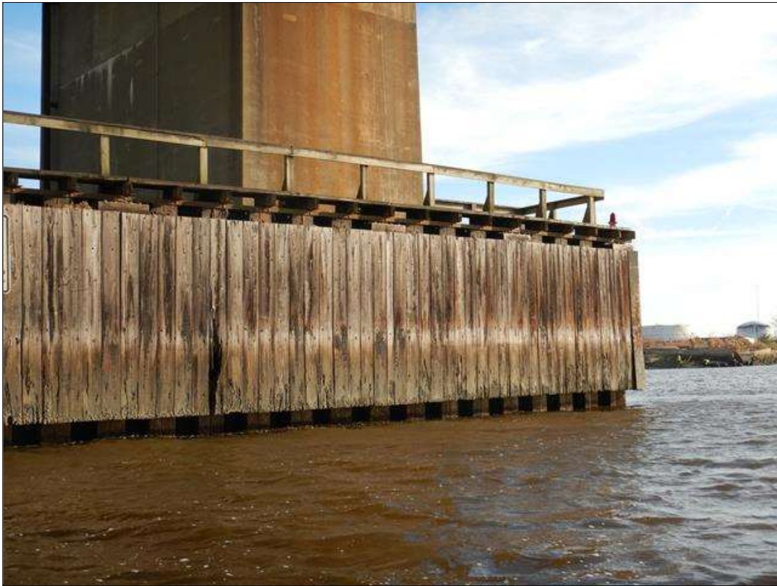
Bent 17 - Lift Span Bent Footing: TIMBER SHEETING BUFFER BOARD IS BROKEN AND MISSING NEAR CENTERLINE ON WEST FACE.
