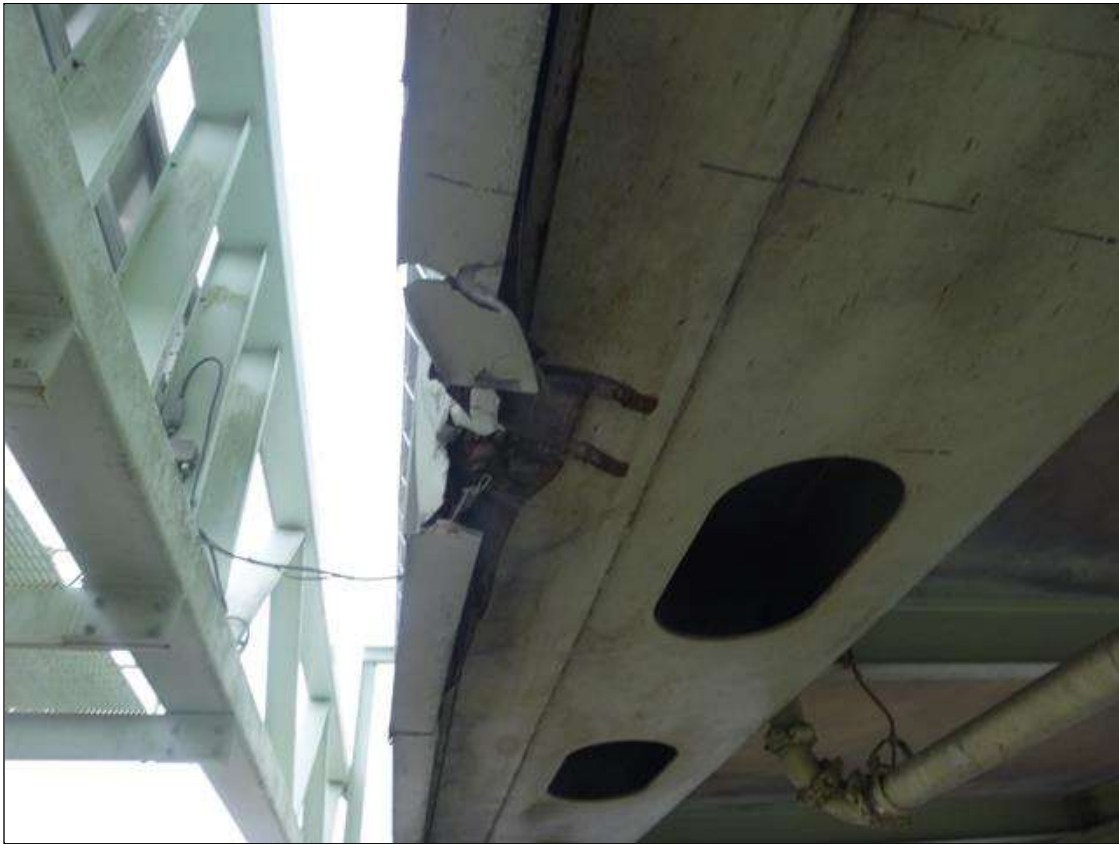
Span 19 EAST TOWER NORTH: 6/2020 - IMPACT DAMAGE - BOTTOM EAST HORIZONTAL TRUSS MEMBER - 32" LONG SECTION OF COVER PLATE ON EAST SIDE BENT UPWARD 1-1/4" WIDE/ (2) 6-1/2" LONG GOUGES UP TO 1/16" DEEP - LOCATED 11' FROM NORTHEAST TOWER LEG - NO DAMAGE TO ACTUAL TRUSS MEMBER (COVER PLATE ONLY)
