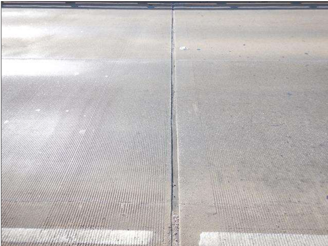
Span 4 Joint at Bent 3: SCATTERED ALONG THE LENGTH, PUNCTURES UP TO 1" DIAMETER IN THE LEFT LANES AND SCATTERED LOSS OF ADHESION IN THE RIGHT.
