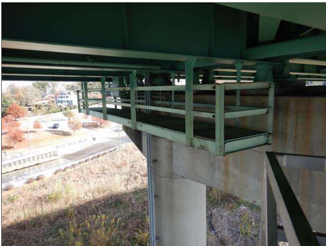
SPAN 20, A STEEL CATWALK HANGS FROM GIRDERS 1-4 [APPROXIMATELY 30' LONG X 3' WIDE X 3' HIGH]
