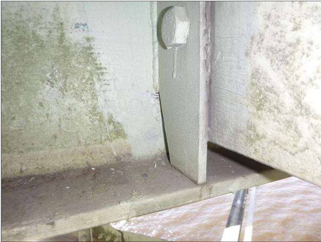
Span 18 Lift Span Stringer 10: REPAIR OBSERVED IN 2021 INSP: CRACK NOT VISIBLE AREA HAS BEEN PAINTED OVER. 2020 REPORT BETWEEN FB's 5-6 - 1-1/2" LONG CRACK IN DIAPHRAGM CONNECTION WELD AT BOTTOM ON NORTH SIDE.
