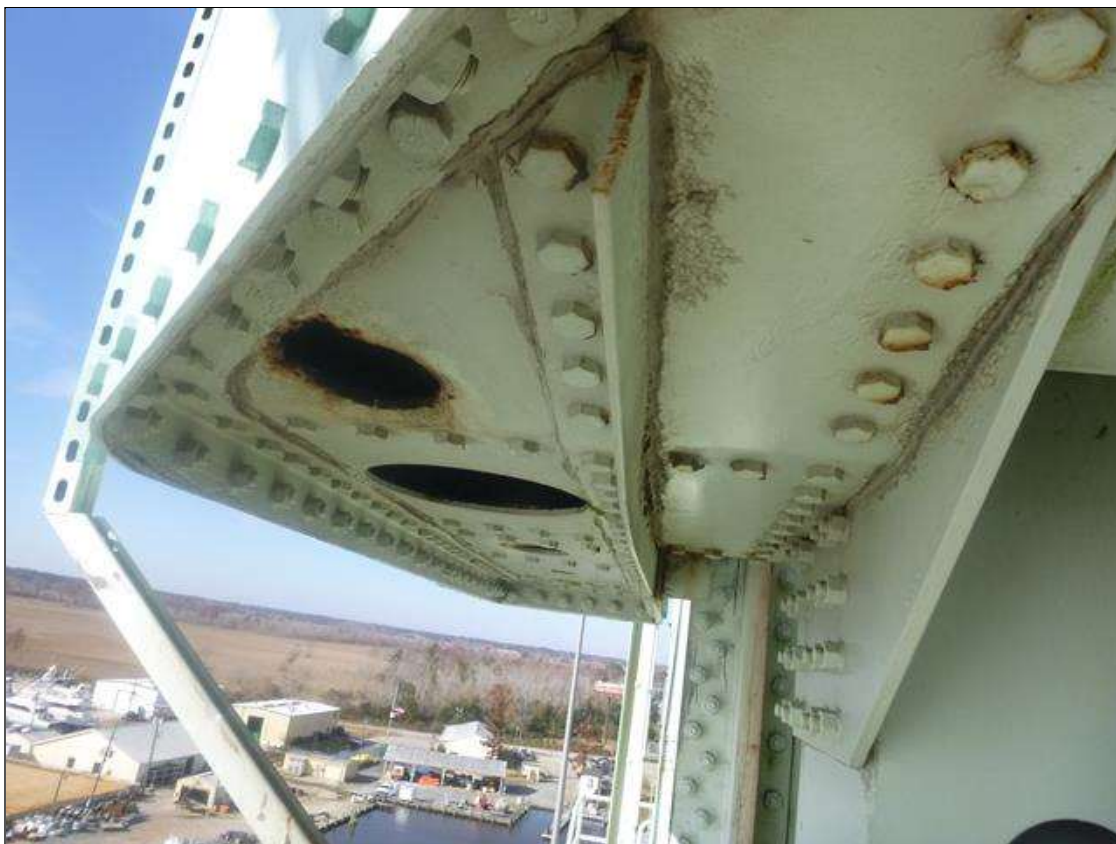
Span 18 Lift Span U0 SOUTH: (PROMPT ACTION REQUEST) BOTTOM PLATE AT ACCESS HOLE CORROSION WITH HOLE 5" X 2" HOLE.
