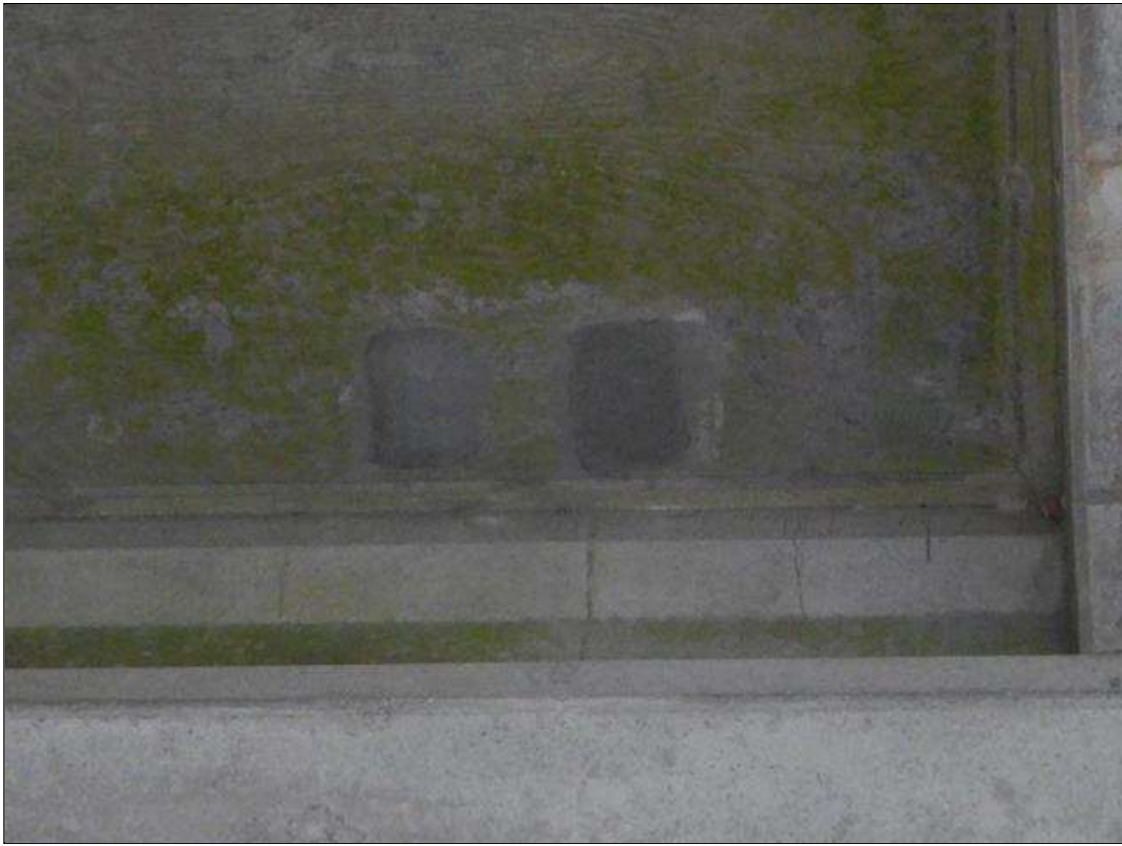
Span 8 Deck: [NEW REPAIR - PATCHING] FORMERLY --> (20" x 9") area of (x2) spalls with exposed rebar on the deck bottom in bay 4, 15.5ft from bent 8 up to (9" x 4" x 1/2')
