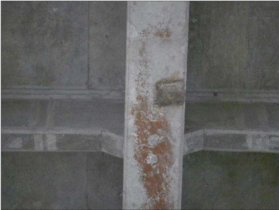
Span 8 Beam 6: [NEW REPAIR - PATCHING] FORMERLY --> (7" x 4" x 1/2") spall with exposed rebar on the bottom face at 20ft from bent 7
