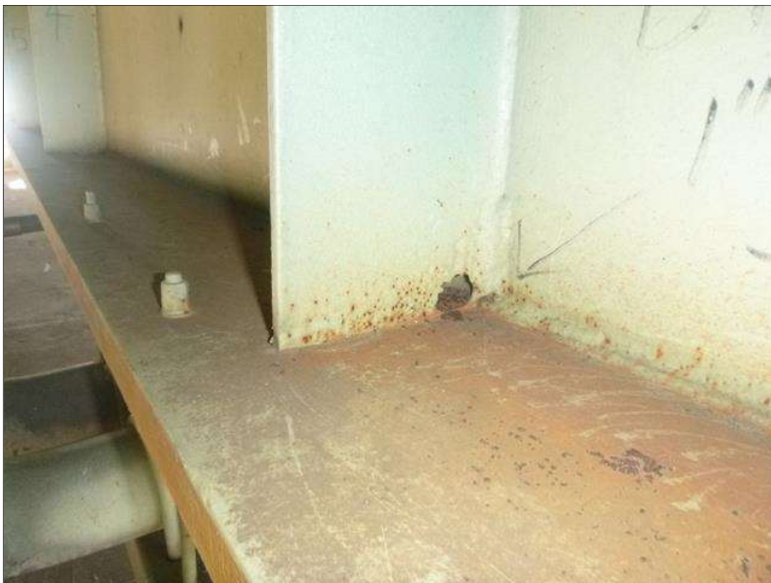
Span 19 Floor Beam 2: HOLE 1" DIAMETER IN BOTTOM OF STIFFNER 3 ON EAST SIDE.
