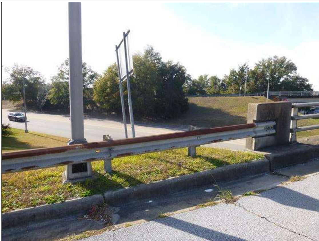
SOUTHEAST CORNER, GUARDRAIL TRANSITION AND CONNECTION
