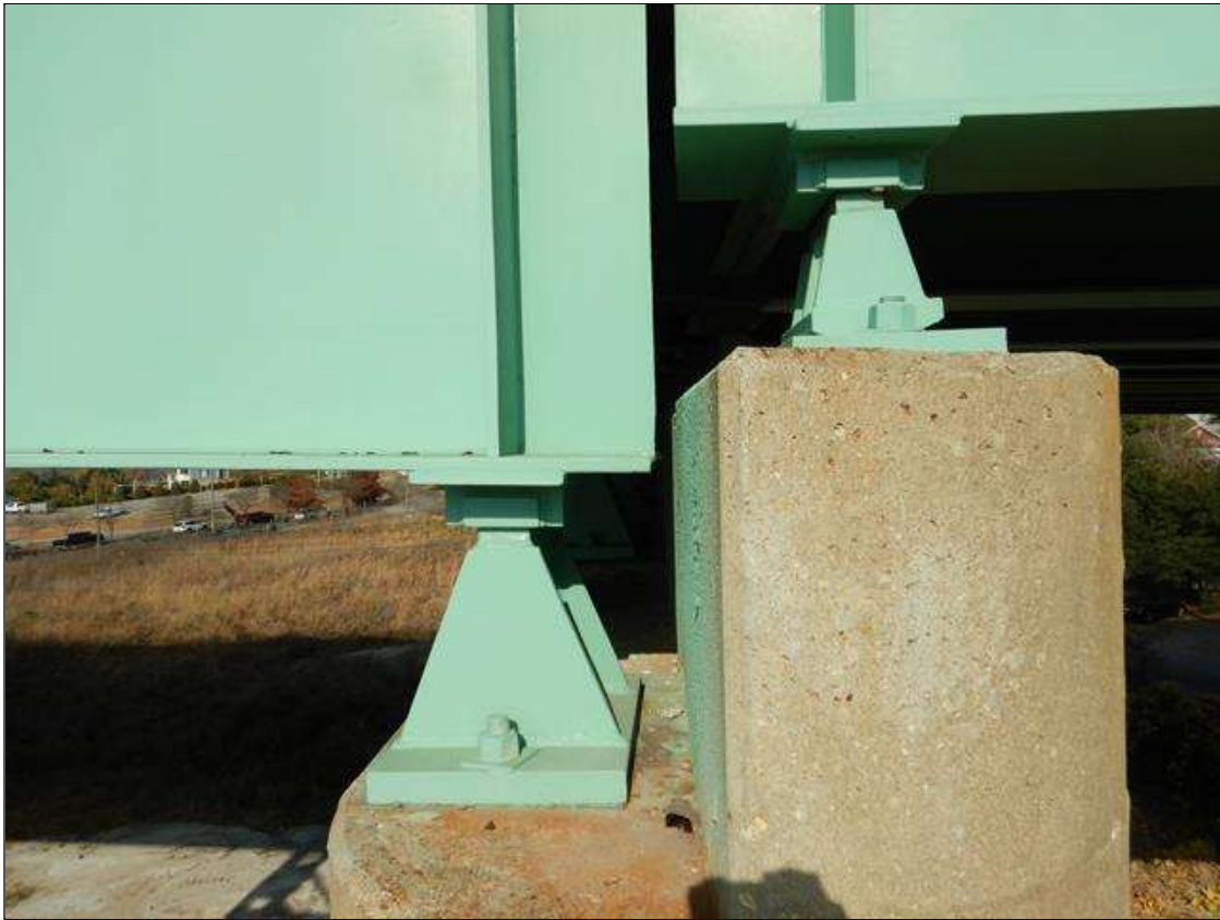
GIRDERS 8 BEARINGS AT BENT 21, TYPICAL BEARINGS AT BENT 21
