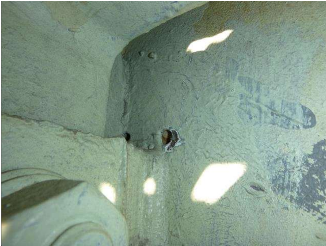
Span 18 Lift Span Stringer 10: BETWEEN FB's 9-10 - (2) CRACKS PROPAGATED PAST ARREST HOLE AT TOP OF DIAPHRAGM CONNECTION - (1) 1/8" AND (1) 1/4" – PROMPT ACTION REQUEST
