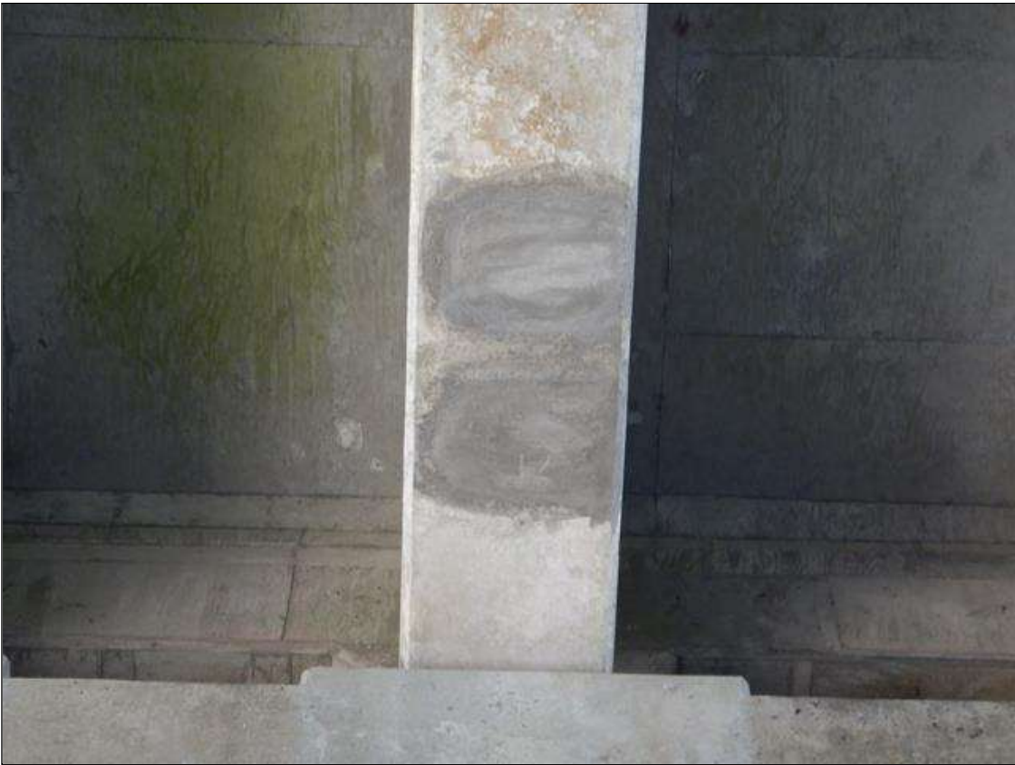
Span 28 Beam 5: [NEW REPAIR-PATCHING] FORMERLY --> (x2) spalls with exposed rebar on the bottom face at bent 25 up to (7" x 7" x 1/2")
