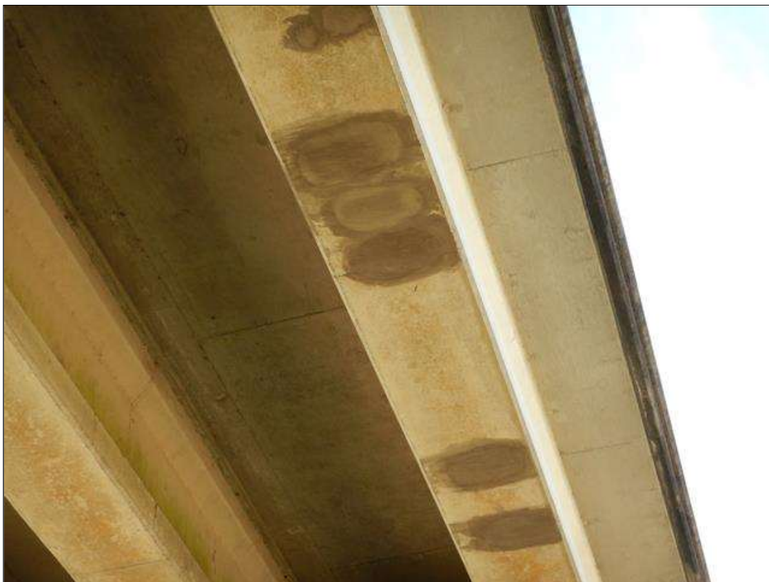
Span 33 - Ramp Span Beam 1: [NEW REPAIR-PATCHING] FORMERLY --> (x4) spalls with exposed rebar on the bottom face up to (5" x 5" x 1/2") at several locations
