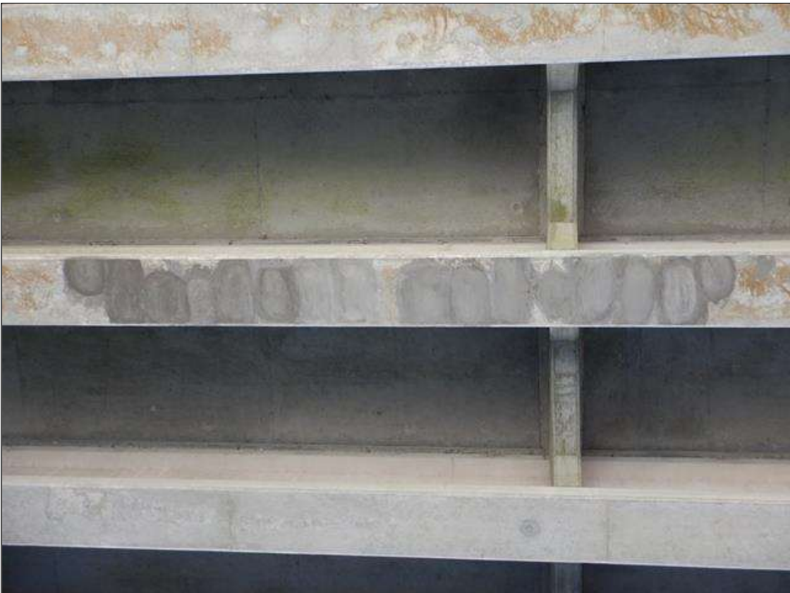
Span 28 Beam 5: [NEW REPAIR-PATCHING] FORMERLY --> multiple spalls with exposed rebar on the bottom face starting at 9ft from bent 25 up to (18" x 6" x 1/2")
