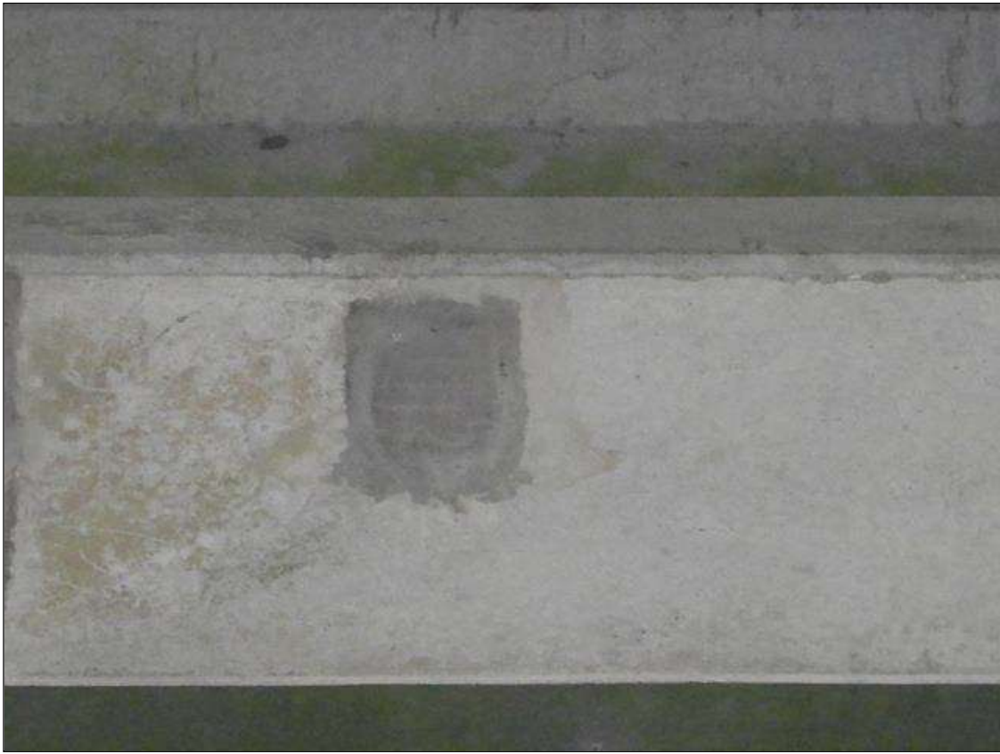
Span 5 Beam 2: [NEW REPAIR - PATCHING] FORMERLY --> (8" x 4" x 1/2") spall with exposed rebar on the bottom face at 14ft from bent 4
