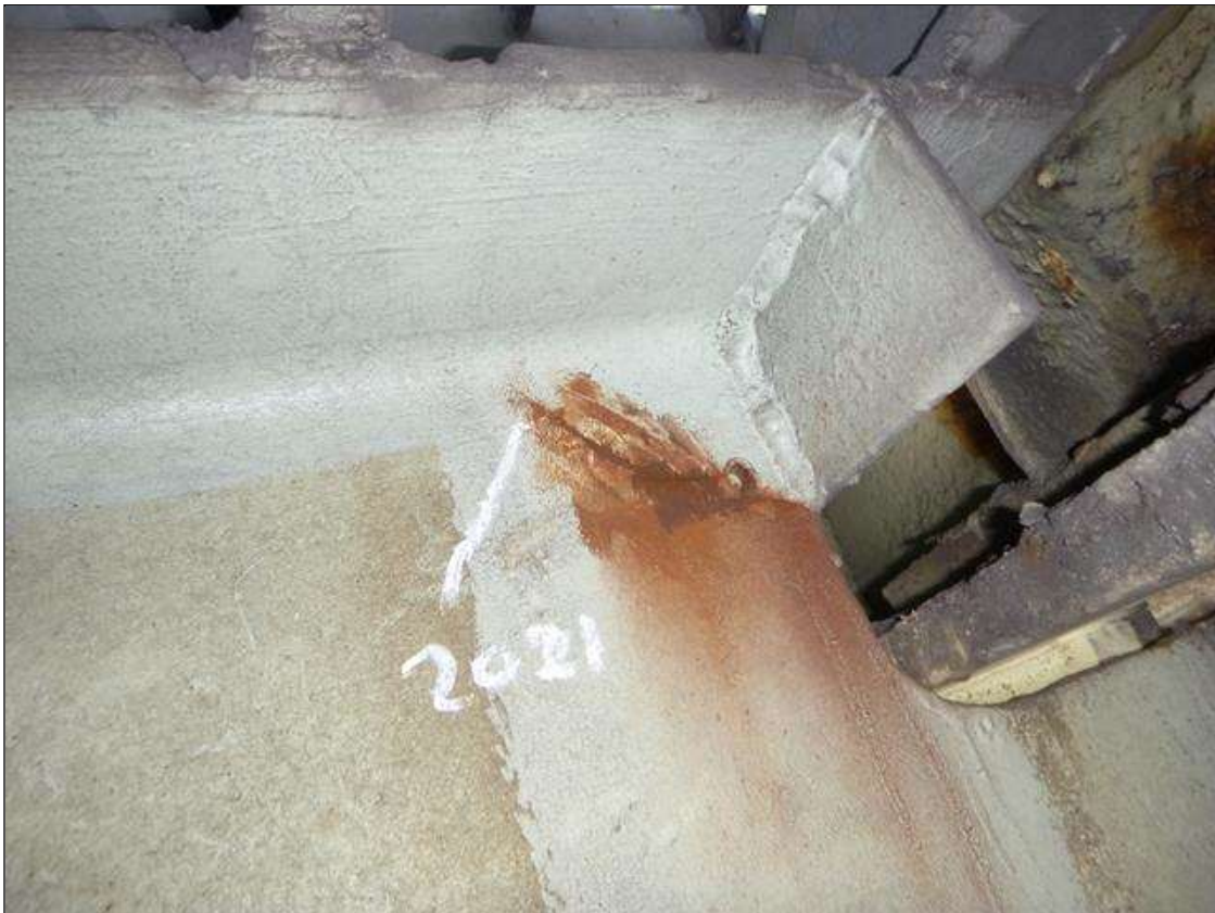
Span 18 Lift Span Stringer 12: (PAR) BETWEEN FB's 0-1 - CRACK EXTENDING 3" PAST ARRESTING HOLE IN COPING AT FB 0 CONNECTION
