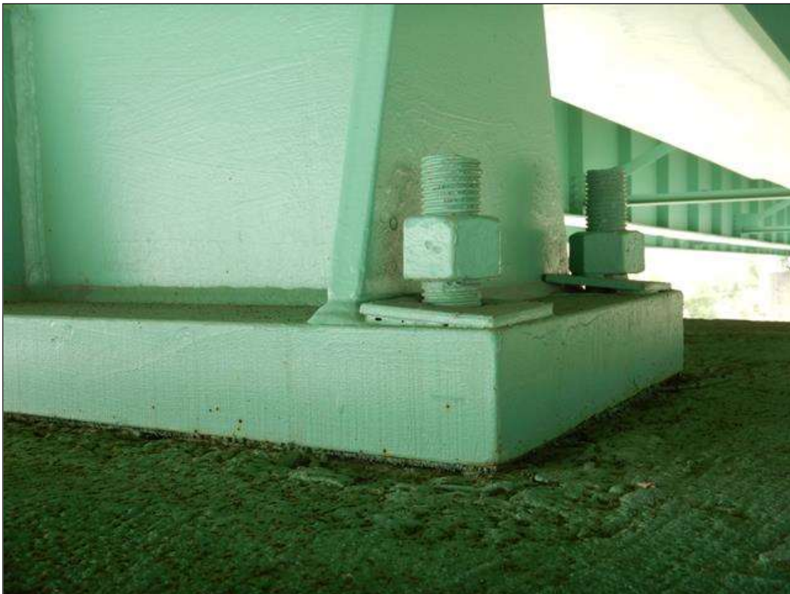
Span 13 Beam 6 - Beam 6 Intermediate Bearing 1: LEFT FAR ANCHOR NUT IS NOT TIGHTENED, APPROXIMATELY 3/4" ABOVE THE PLATE.
