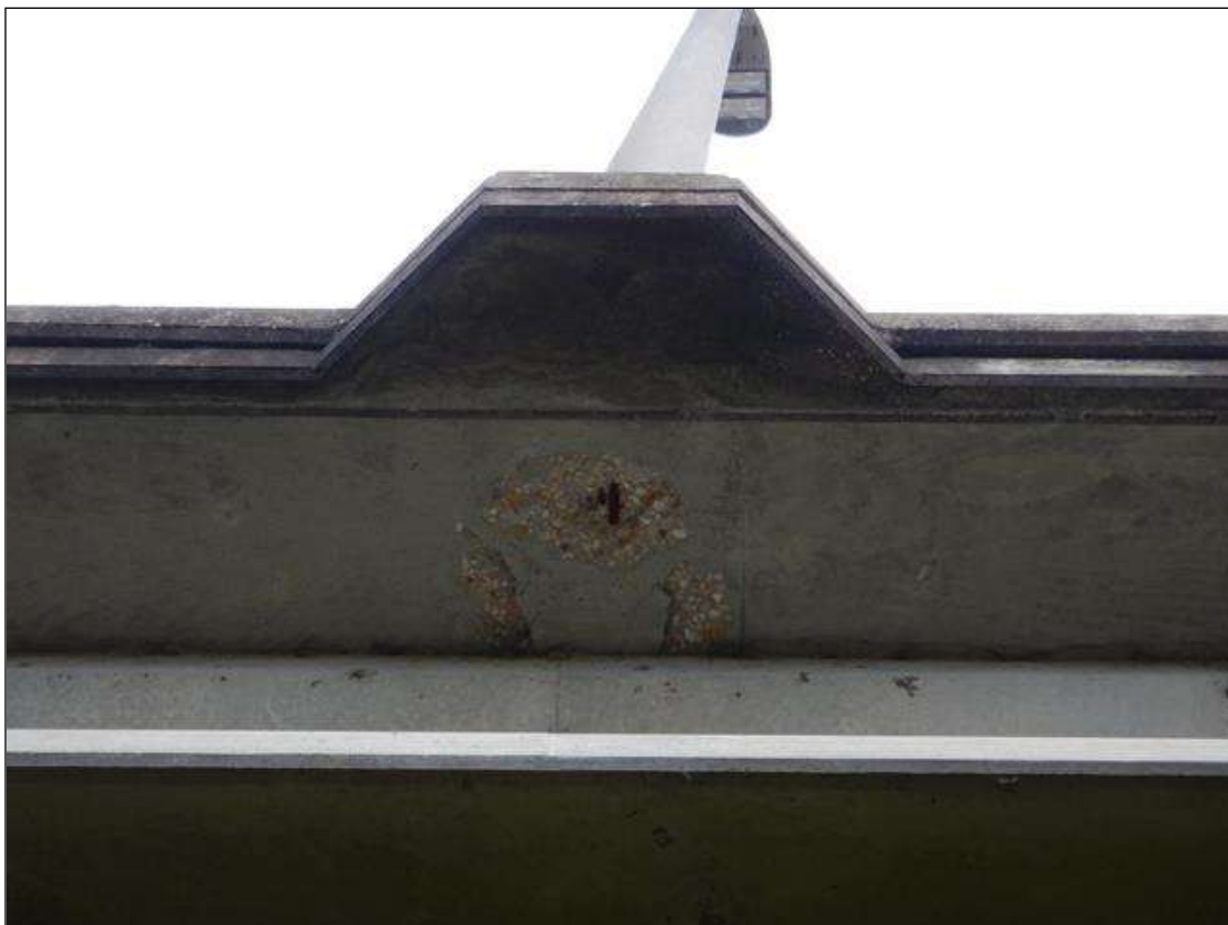
Span 5 Deck: bottom right overhang at light pole: spall, 16" wide x 24" long x 1.5" deep with exposed rebar with adjacent delaminated area, near mid-span
