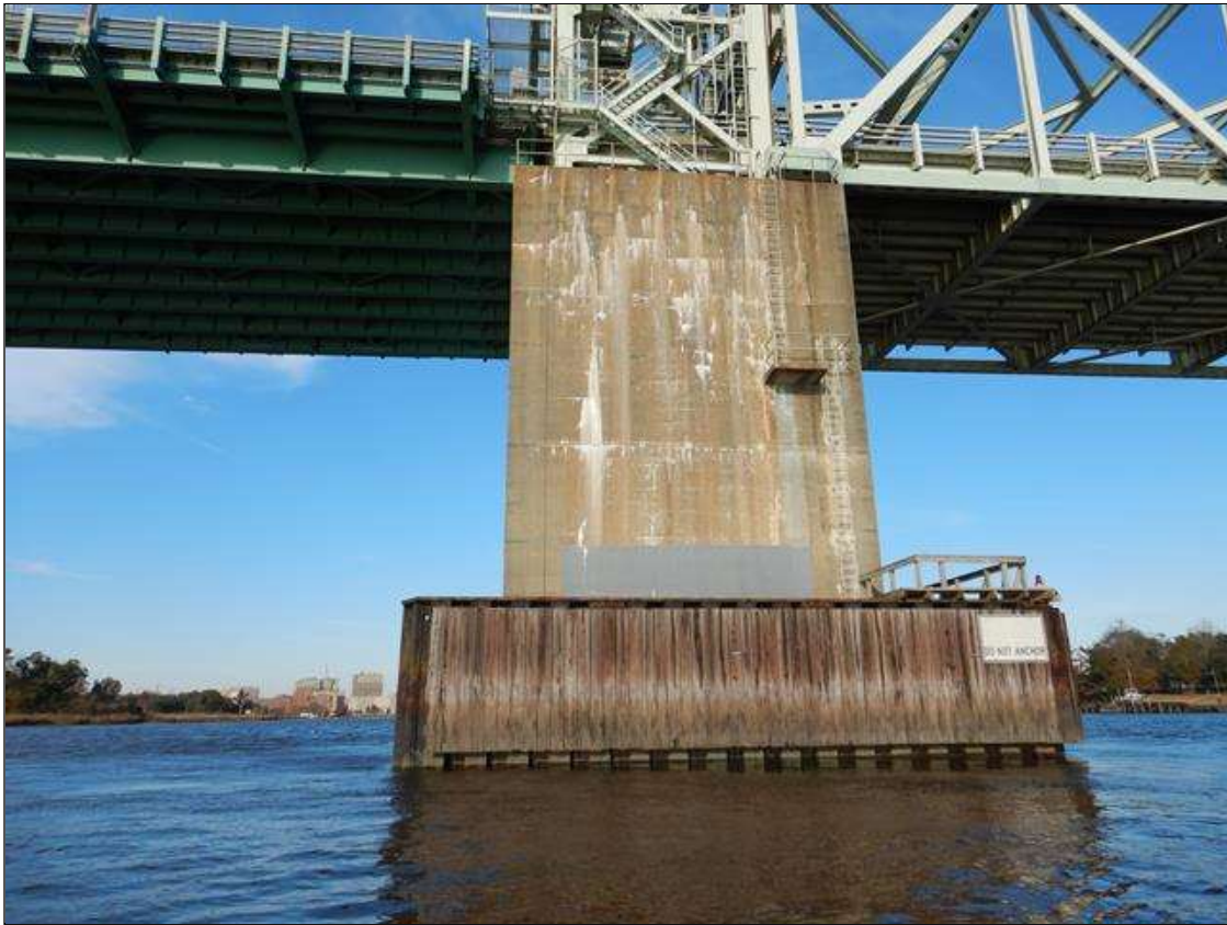
Bent 16 - Lift Span Bent Pile 1: HAIRLINE TO 1/16" WIDE CRACKING WIDE/ EFFLORESCENCE SCATTERED THROUGHOUT 25% OF ALL FACES
