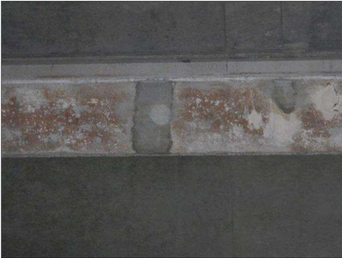
Span 10 Beam 8: [NEW REPAIR - PATCHING] FORMERLY --> 1ft area of (x2) spalls with exposed rebar on the bottom face at 7ft from bent 9 up to (8" x 7" x 1/2")
