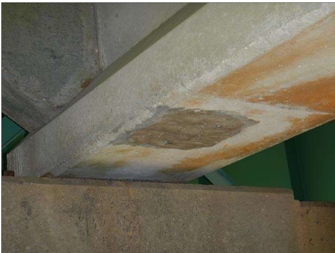
Span 11 Beam 2: [NEW REPAIR - PATCHING] FORMERLY --> spall with exposed rebar on the bottom face at 9in from bent 11 (11" x 10" x 1/2")
