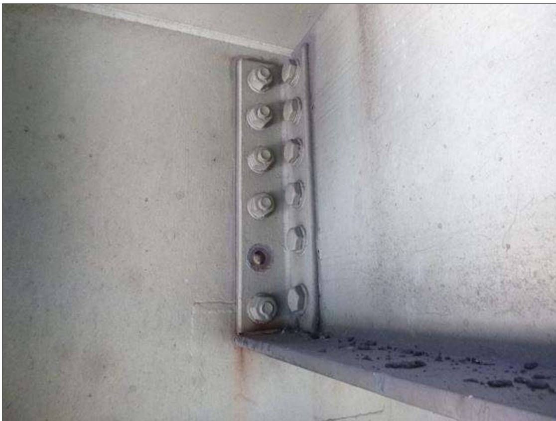
Span 18 Lift Span Stringer 3: ONE BOLT MISSING ON THE SOUTH SIDE OF STRINGER CONNECTION TO FLOOR BEAM 1, PAR ISSUED.
