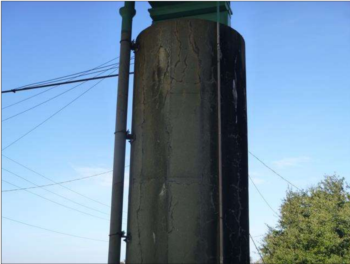
Bent 23 Pile 1: surface efflorescence for 30 square feet
