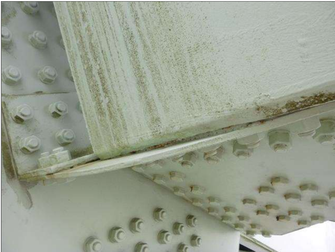
Span 18 Lift Span U1 NORTH: BOTTOM GUSSET CONNECTION AT LATERAL CONNECTION HAS 1/4" OUT OF PLANE BENDING WITH PACK RUST BETWEEN PLATES. AREA HAS BEEN CLEANED AND PAINTED
