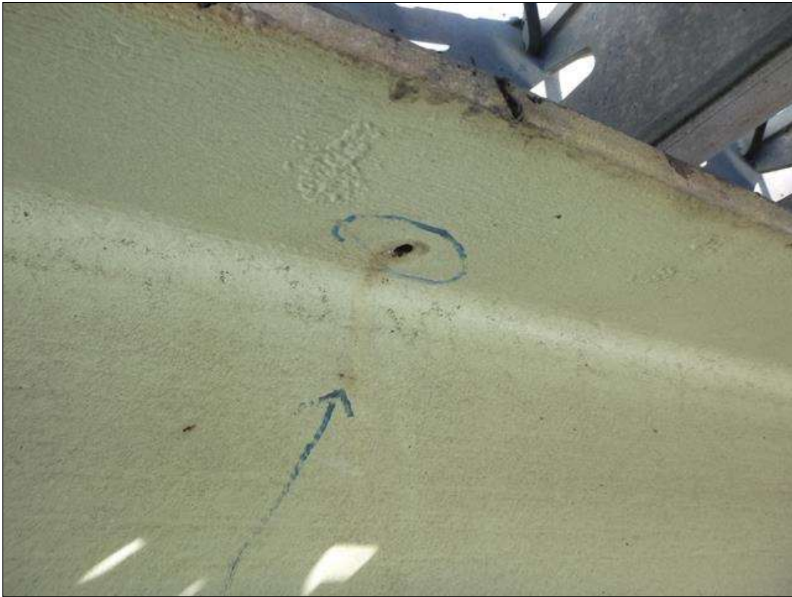
Span 18 Lift Span Stringer 4: BETWEEN FB"s 4-5 - SOUTH SIDE TOP FLANGE 10' FROM FLOORBEAM 4, 3/8" DIAMETER HOLE.
