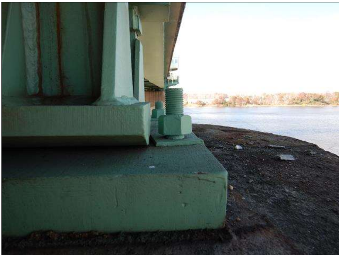
Span 22 Beam 1 - Beam 1 Near Bearing: [PROMPT ACTION REQUEST] LEFT ANCHOR BOLT LIFTED 1/2"
