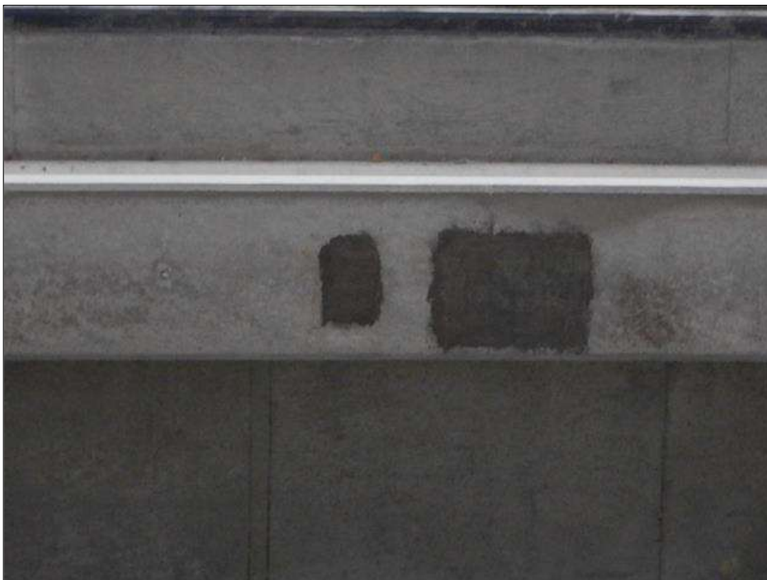
Span 10 Beam 9: [NEW REPAIR - PATCHING] FORMERLY --> (10" x 5" x 1/4") spall with exposed rebar on the bottom face at 25ft from bent 9
