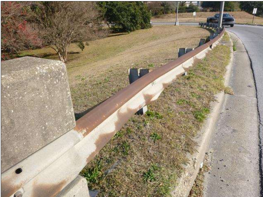
NORTHEAST CORNER GUARDRAIL, IMPACT DAMAGE WITH POSTS DEFLECTED UP TO 6" AT THE TOP [APPROXIMATELY 10' LONG]
