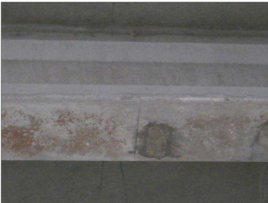
Span 10 Beam 3: [NEW REPAIR - PATCHING] FORMERLY --> (4" x 4" x 1/2") spall with exposed rebar on the bottom face at 12ft from bent 10
