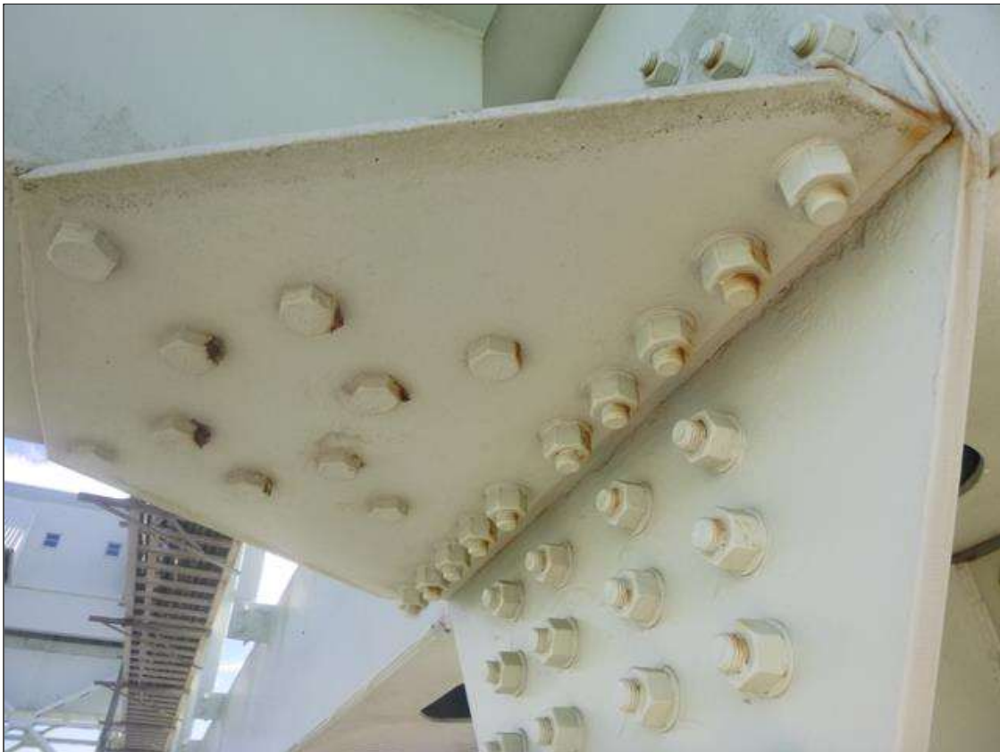
Span 18 Lift Span U6 SOUTH: NORTH FACE SURFACE RUST ON BOLTS.
