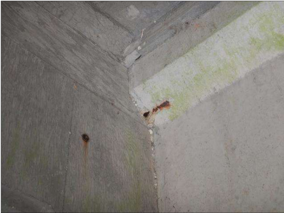
Span 28 Beam 8: [PROMPT ACTION REQUEST] spall with exposed rebar on the top right flange at bent 25 (5" x 1 1/2" x 1/4")
