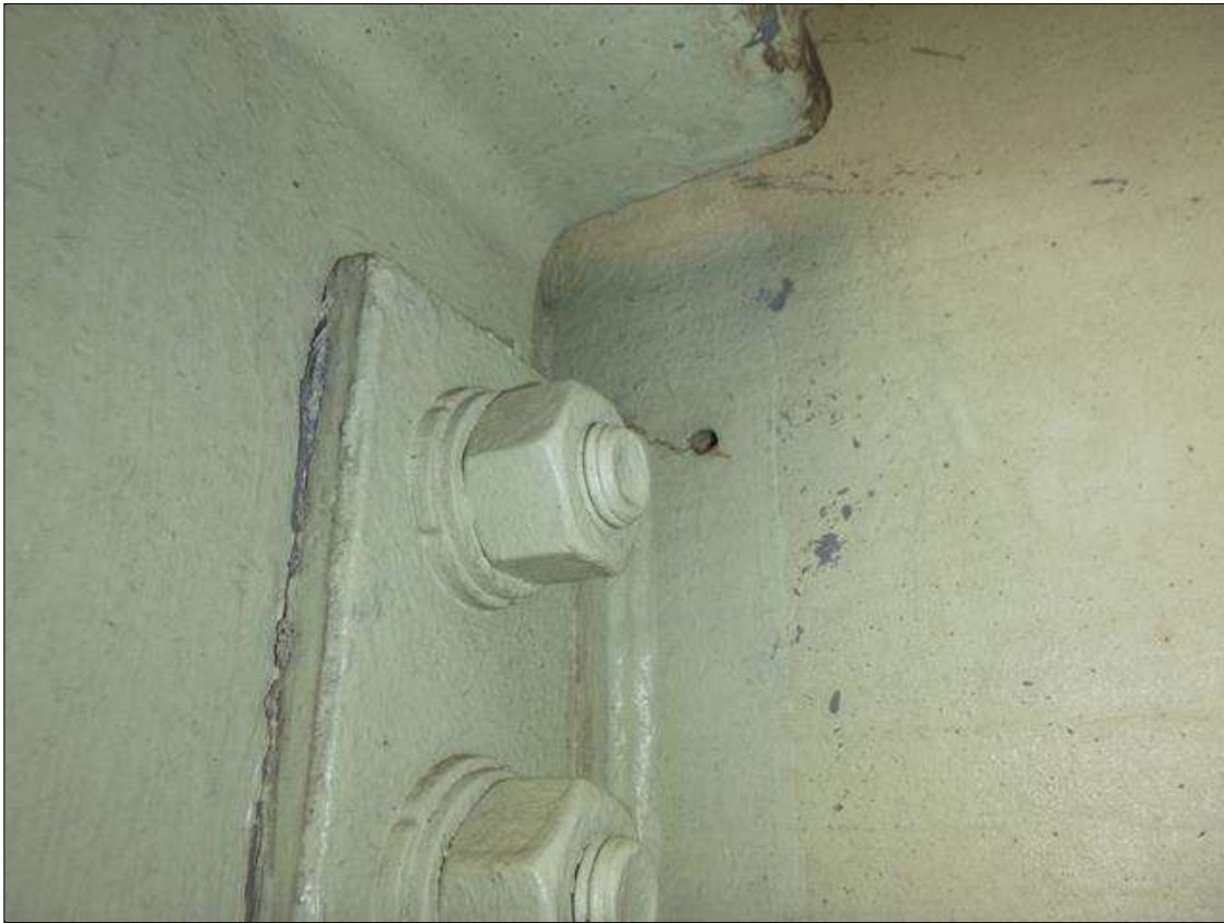
Span 18 Lift Span Stringer 11: OBSERVED IN 2020 INSP.; AREA HAS BEEN PAINTED OVER, NO CHANGE, PROPAGATED CRACK STILL VISIBLE. PAR ISSUED. 2018 REPORT HAD BETWEEN FB's 3-4 - CRACKS PROPAGATED UP TO 3/16" PAST EAST AND WEST ARREST HOLES AT TOP OF DIAPHRAGM CONNECTION - PAR ISSUED
