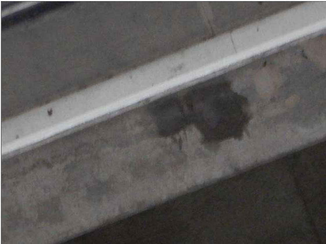
Span 10 Beam 9: [NEW REPAIR - PATCHING] FORMERLY --> 1ft area of (x2) spalls with exposed rebar on the bottom face at 7ft from bent 9 up to (5" x 5" x 1/2")
