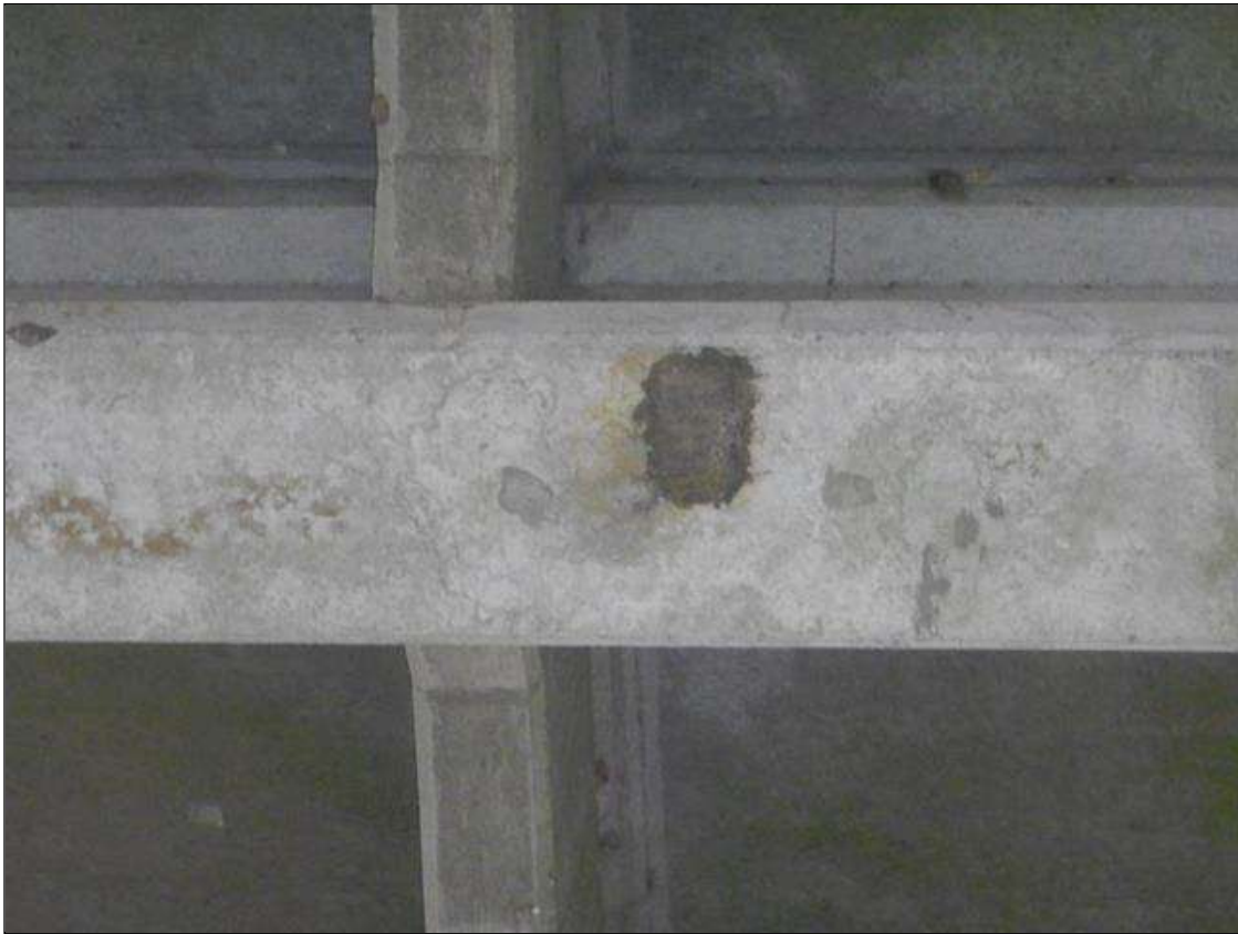
Span 7 Beam 6: [NEW REPAIR - PATCHING] FORMERLY --> area of delamination on the bottom face, 20 FOOT. from bent 7, 8" wide x 12" long with 1/8" separation
