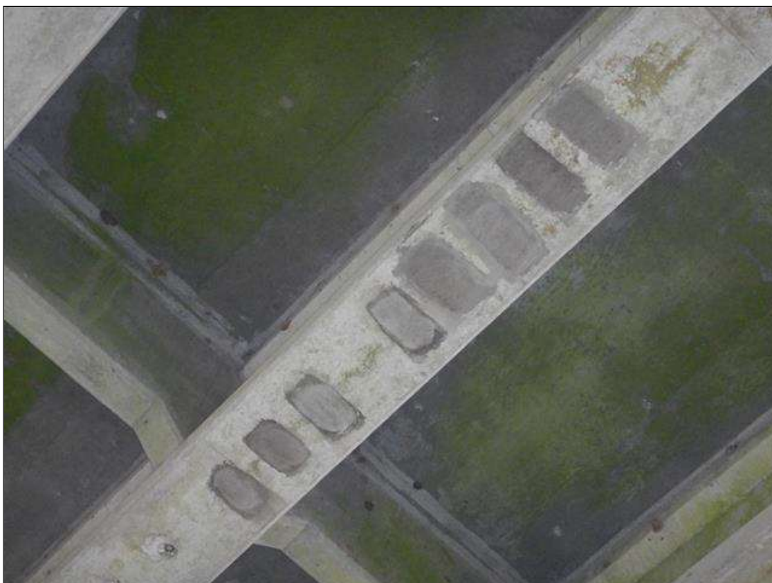
Span 4 Beam 4: [NEW REPAIR - PATCHING] FORMERLY --> (x8) spalls with exposed rebar on the bottom face starting at 21in from bent 3 up to (7" x 4" x 1/2')
