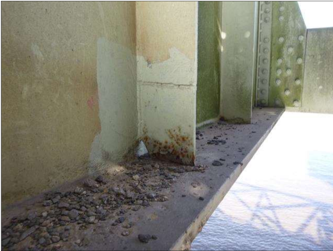
Span 18 Lift Span Floor Beam 9: REPAIR OBSERVED 2021 INSPECTION 7" HIGH REPAIR FROM TOP OF BOTTOM FLANGE WITH SURFACE RUST, 2020 INSPECTION HAD VERTICAL STIFFENER 2 ON EAST SIDE - 3" HIGH PITTED AREA AT BOTTOM FLANGE - LOWER 2" OF AREA REDUCED TO KNIFE EDGE WIDE/ (2) 1/2" TO 1-1/2" DIAMETER HOLES - CLEANED AND PAINTED
