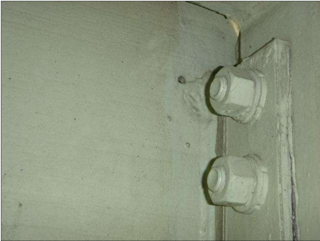
Span 18 Lift Span Stringer 4: REPAIR OBSERVED IN 2021 INSPECTION CRACK NOT VISIBLE, AREA HAS BEEN PAINTED OVER. 2020 REPORT HAD BETWEEN FB's 5-6 - CRACK PROPAGATED 3/16" PAST ARREST HOLE AT TOP OF DIAPHRAGM CONNECTION
