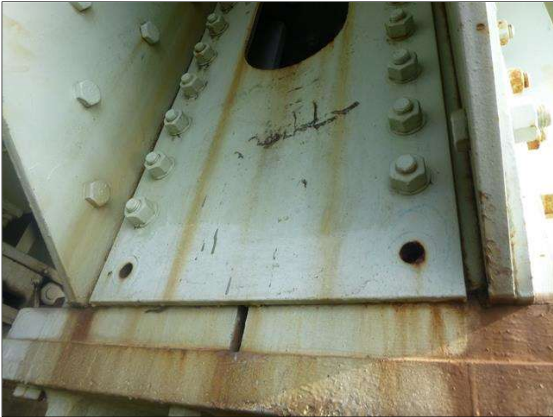
Span 18 Lift Span Truss Panel 2 - L12U12 SOUTH: 2 MISSING BOLTS AT THE BOTTOM OF THE WEST GUSSET AT BEARING. (PAR)
