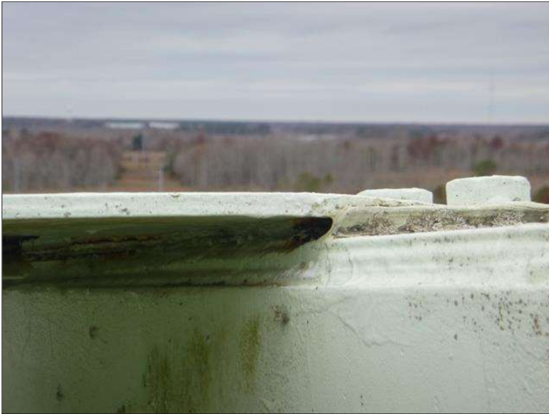
Span 18 Lift Span U2 NORTH: U2 TOP GUSSET PLATE HAS 1/8" OUT OF PLANE BENDING DUE TO PACK RUST BUILD UP BETWEEN MEMBERS. (PAR)
