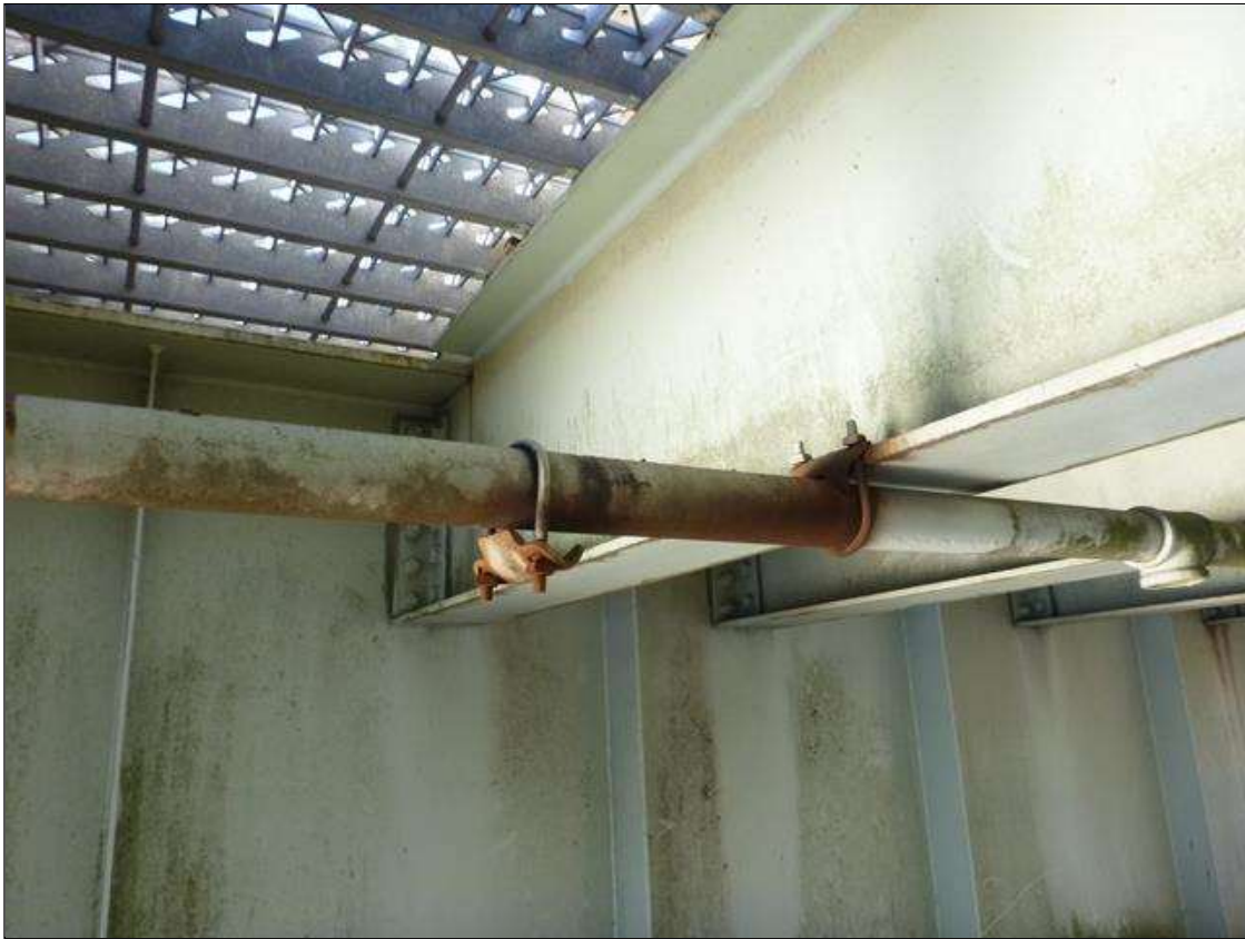
BETWEEN FLOOR BEAMS 6 AND 7 THERE ARE 5 OF 9 UTILITY BRACKETS DISCONNECTED..
