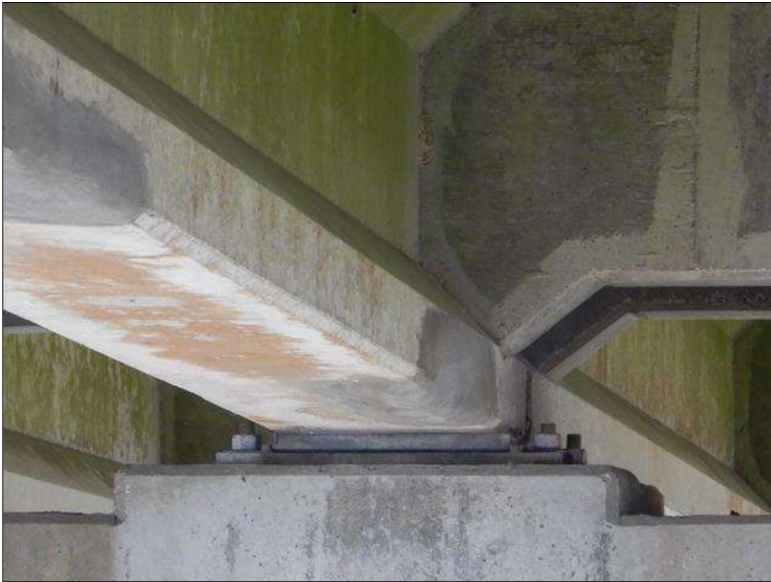
Span 11 Beam 6: ([NEW REPAIR - PATCHING] FORMERLY --> 4" x 4" x 1/2") spall with exposed rebar on the bottom face at bent 10
