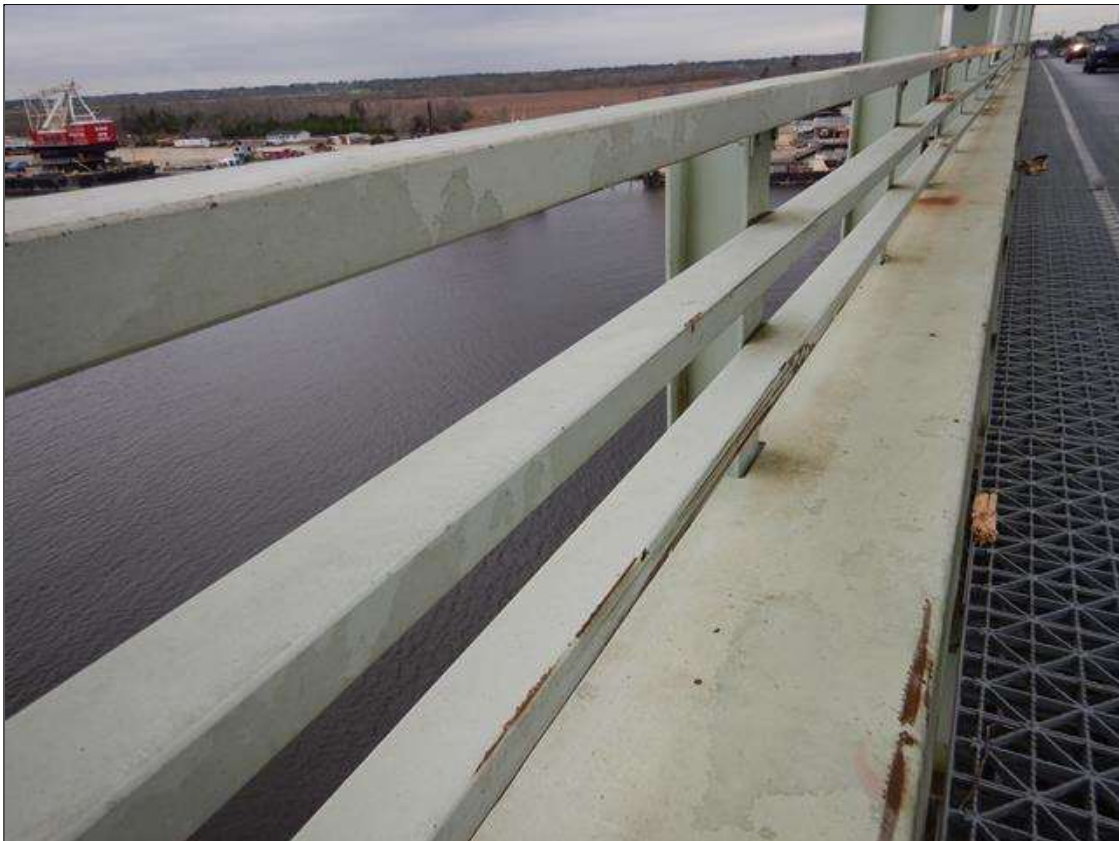
Span 18 Lift Span Left Bridge Rail: IMPACT DAMAGE/SCRAPES ON LEFT CURB WITH ASSOCIATED SURFACE CORROSION.
