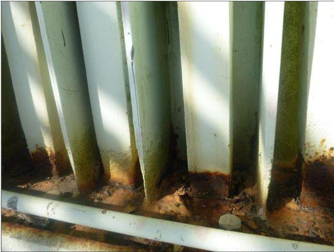
Span 18 Lift Span LB1: [PROMPT ACTION REQUEST] (3) ROD GUIDE PLATES HAVE LOSS OF SECTION UP TO .296" WITH .347" REMAINING ALONG
