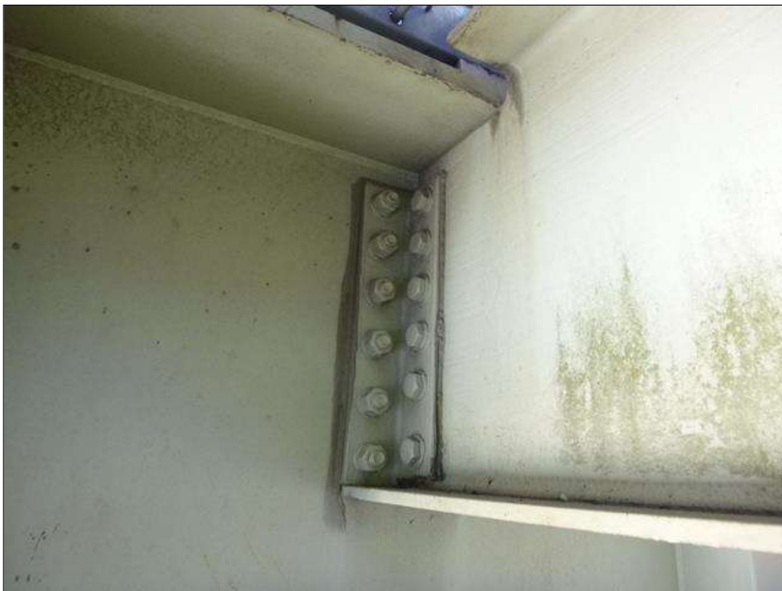
STRINGER TO FLOORBEAM CONNECTION
