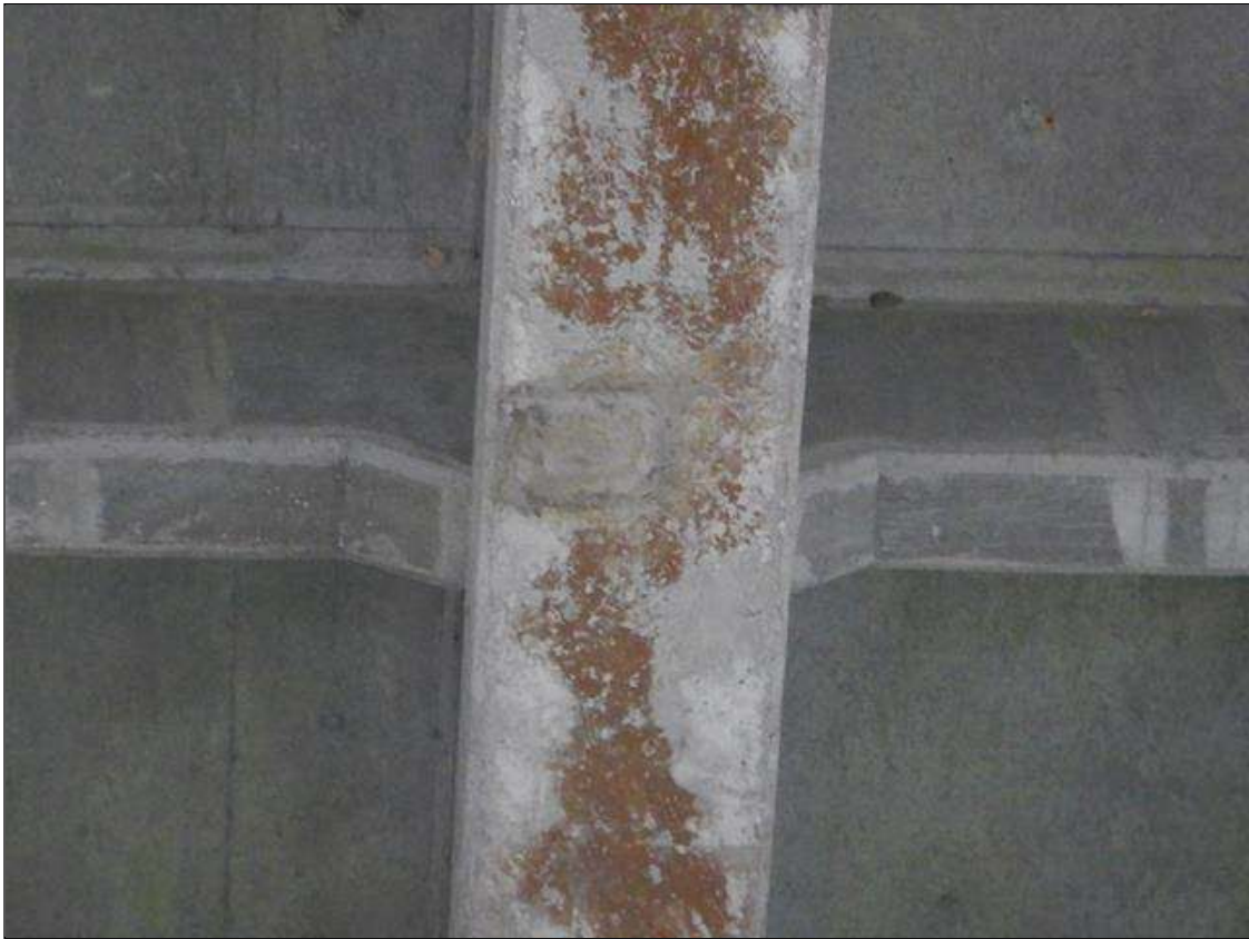
Span 8 Beam 2: [NEW REPAIR - PATCHING] FORMERLY --> (8" x 5" x 1/2") spall with exposed rebar on the bottom face at 28ft from bent 8
