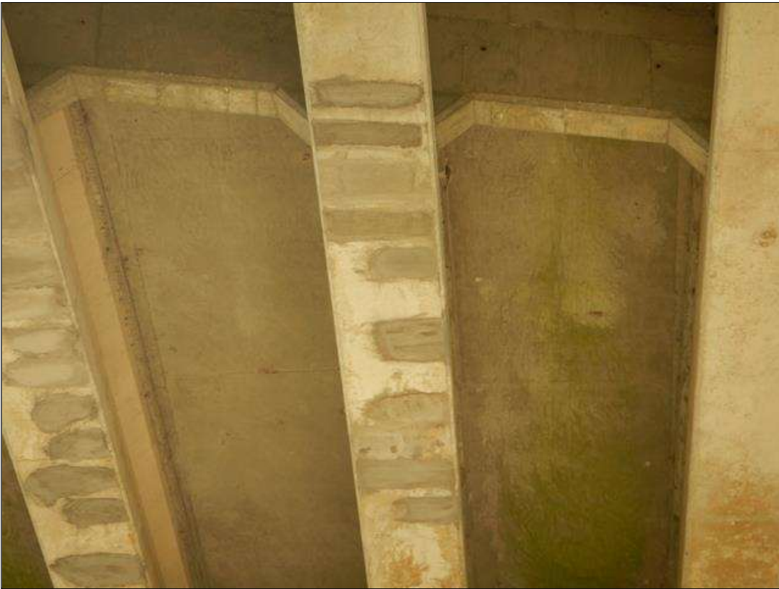
Span 27 Beam 13: [NEW REPAIR-PATCHING] FORMERLY --> (x12) DELAMINATION areas on the bottom face at 10f from bent 24 up to (18" x 1 1/2" x 1/4")
