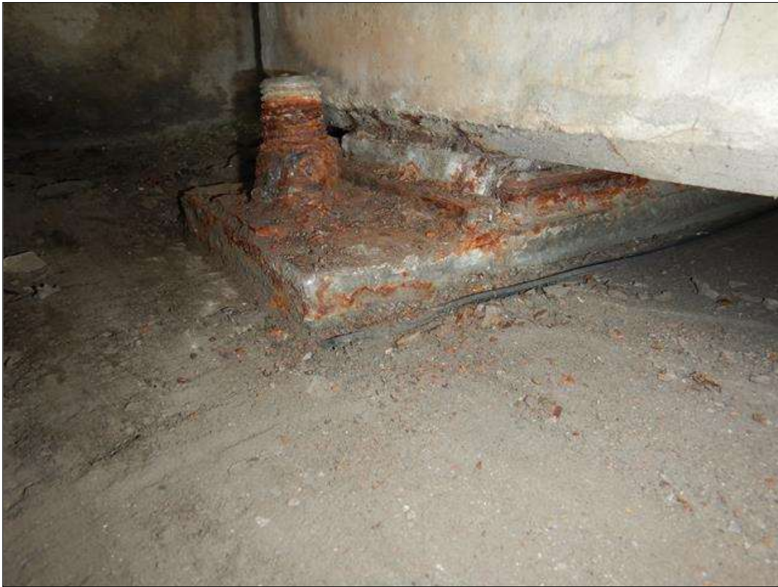
Span 1 Beam 9 - Beam 9 Near Bearing: corrosion and scale with no measureable section loss on the left anchor rod, nut and plate
