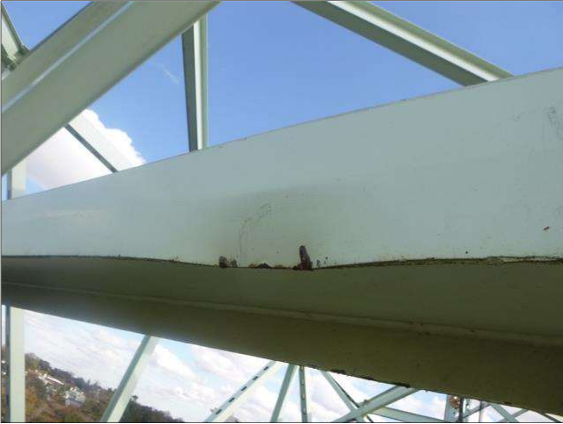
Span 18 Lift Span LB7: IMPACT DAMAGE 20" WIDE X 1-1/2" DEFORMATION IN WEST FLANGE OVER RIGHT EAST BOUND LANE.
