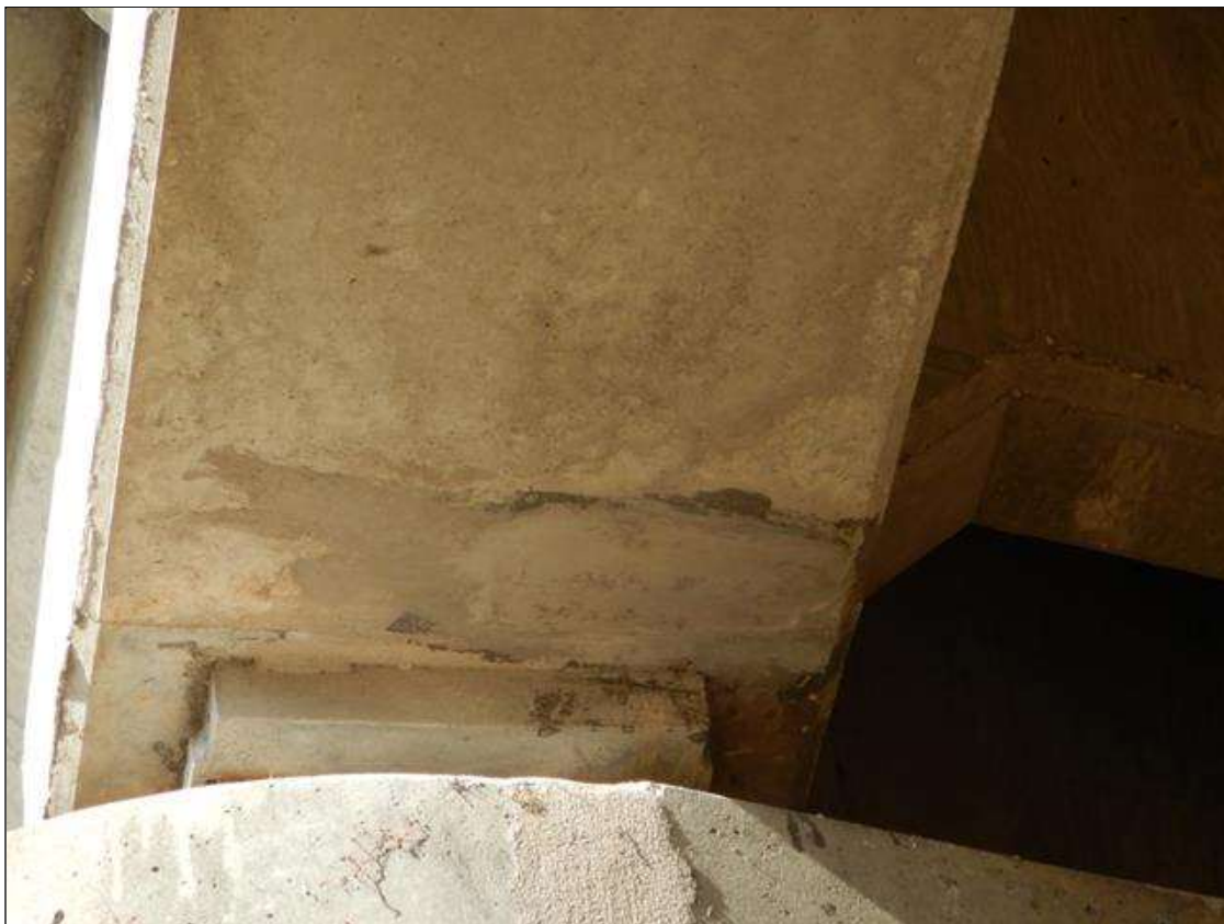
Span 30 Beam 11: [NEW REPAIR-PATCHING] FORMERLY --> spall with exposed rebar on the bottom face at bent 27 (11" x 4" x 1/2")
