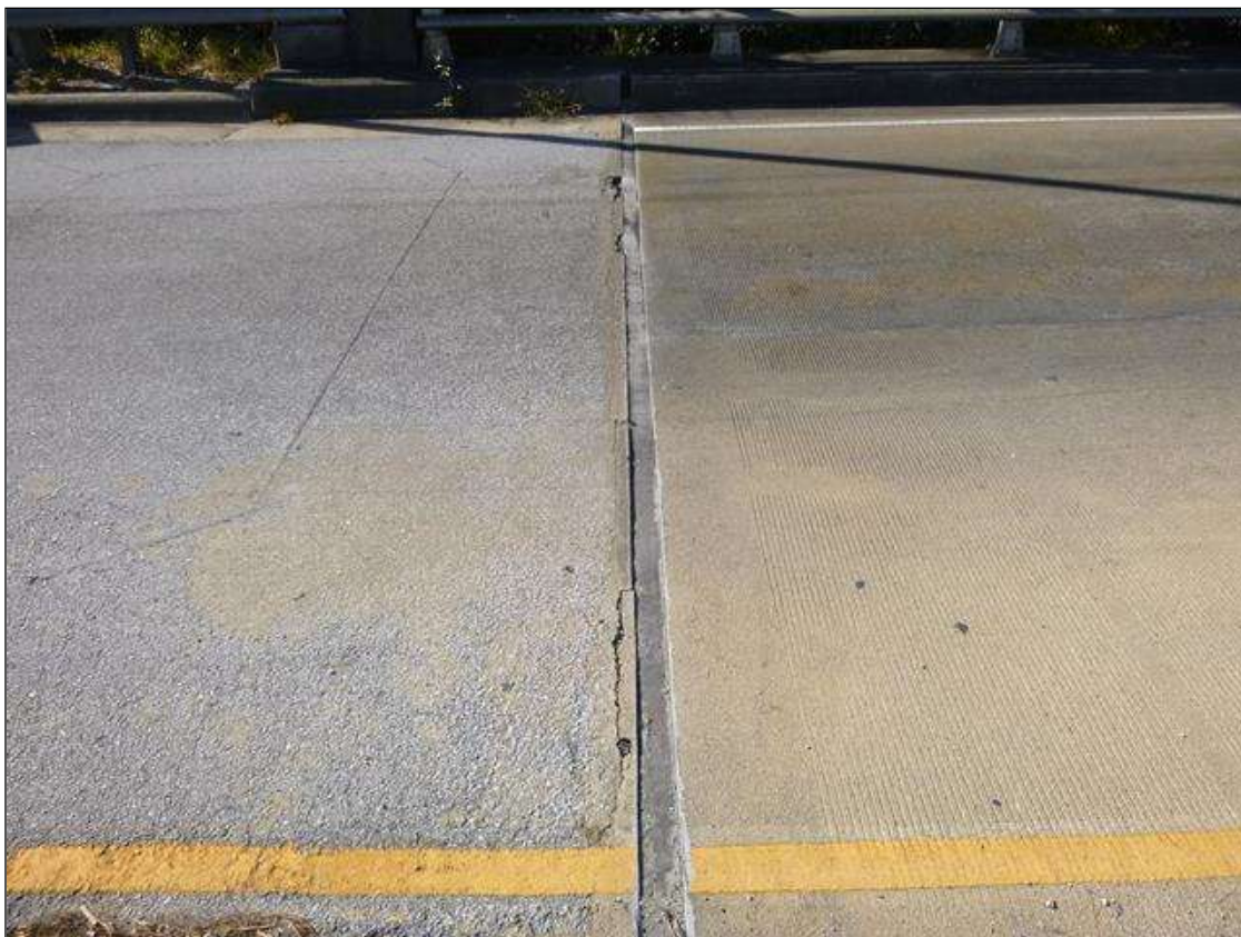
JOINT AT ABUTMENT 2
