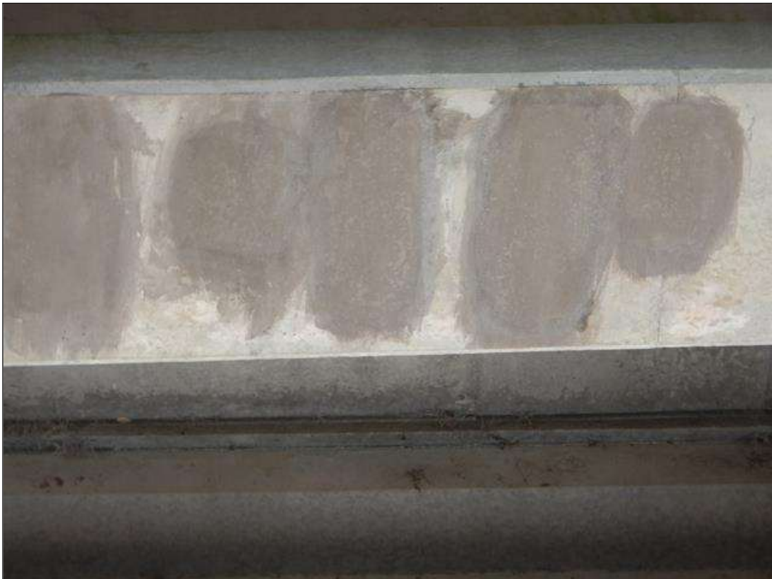
Span 29 Beam 7: [NEW REPAIR-PATCHING] FORMERLY --> (x2) spalls with exposed rebar on the bottom face at 23ft from Bent 27, (10" x 7") and (18" x 6")
