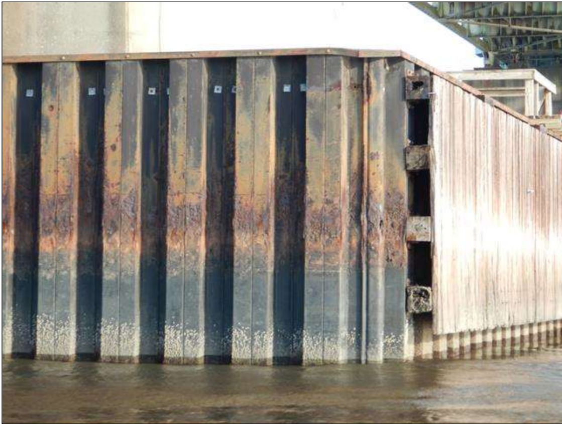
Bent 16 - Lift Span Bent Footing: WEST FACE: STEEL SHEETING HAS SURFACE LOSS OF SECTION UP TO 3/16" IN TIDAL ZONE 5' HIGH.
