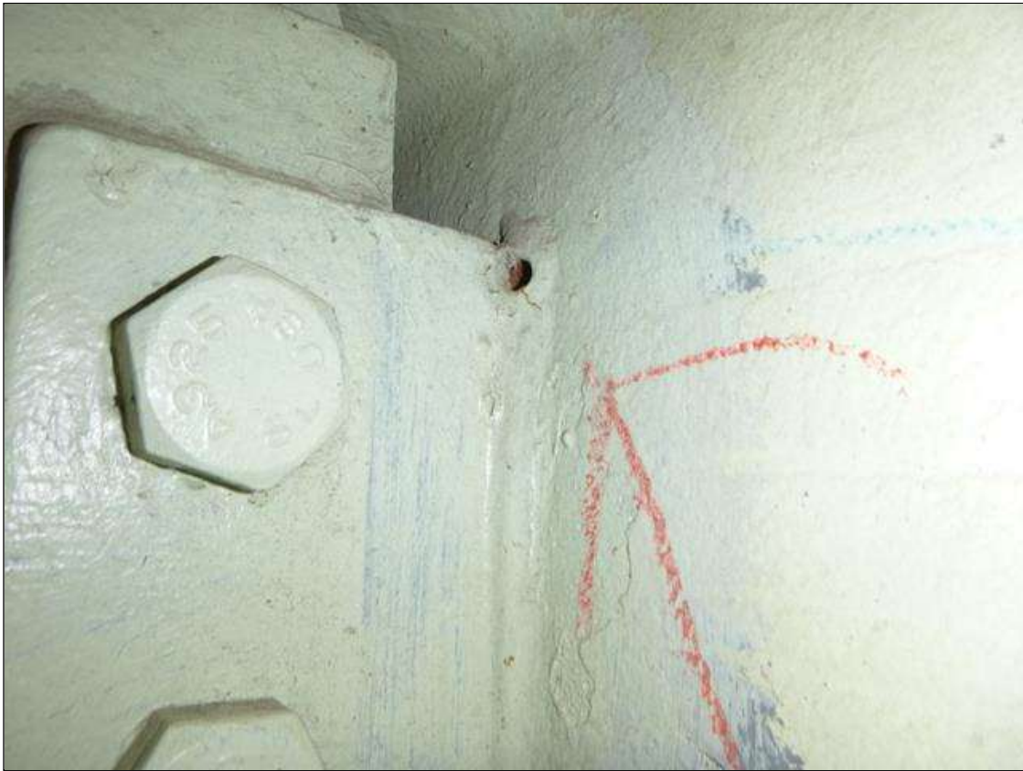
Span 18 Lift Span Stringer 8: BETWEEN FB's 7-8 - (2) CRACKS PROPAGATED 3/16" PAST ARREST HOLE AT TOP OF DIAPHRAGM CONNECTION - PROMPT ACTION REQUEST
