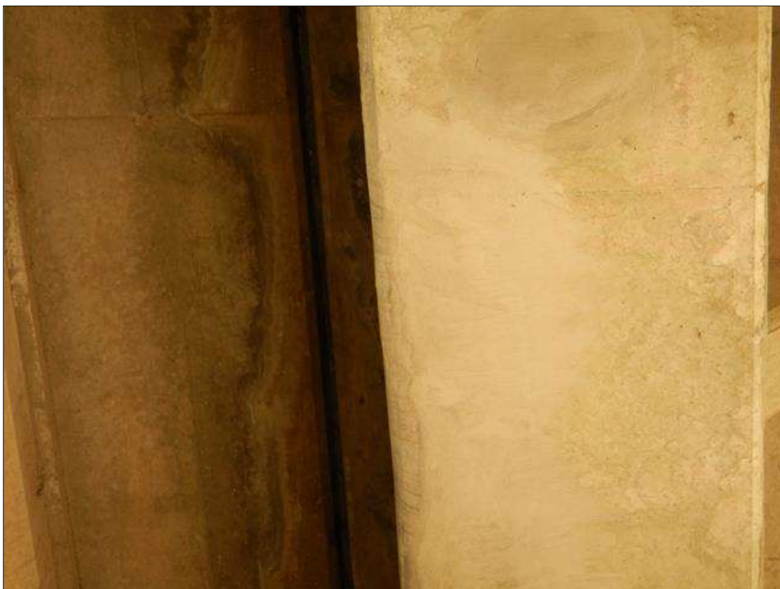
Span 30 Beam 7: [NEW REPAIR-PATCHING] FORMERLY --> spall with no exposed steel on the bottom face at 23.5ft from Bent 27 (6" x 6" x 1/2")
