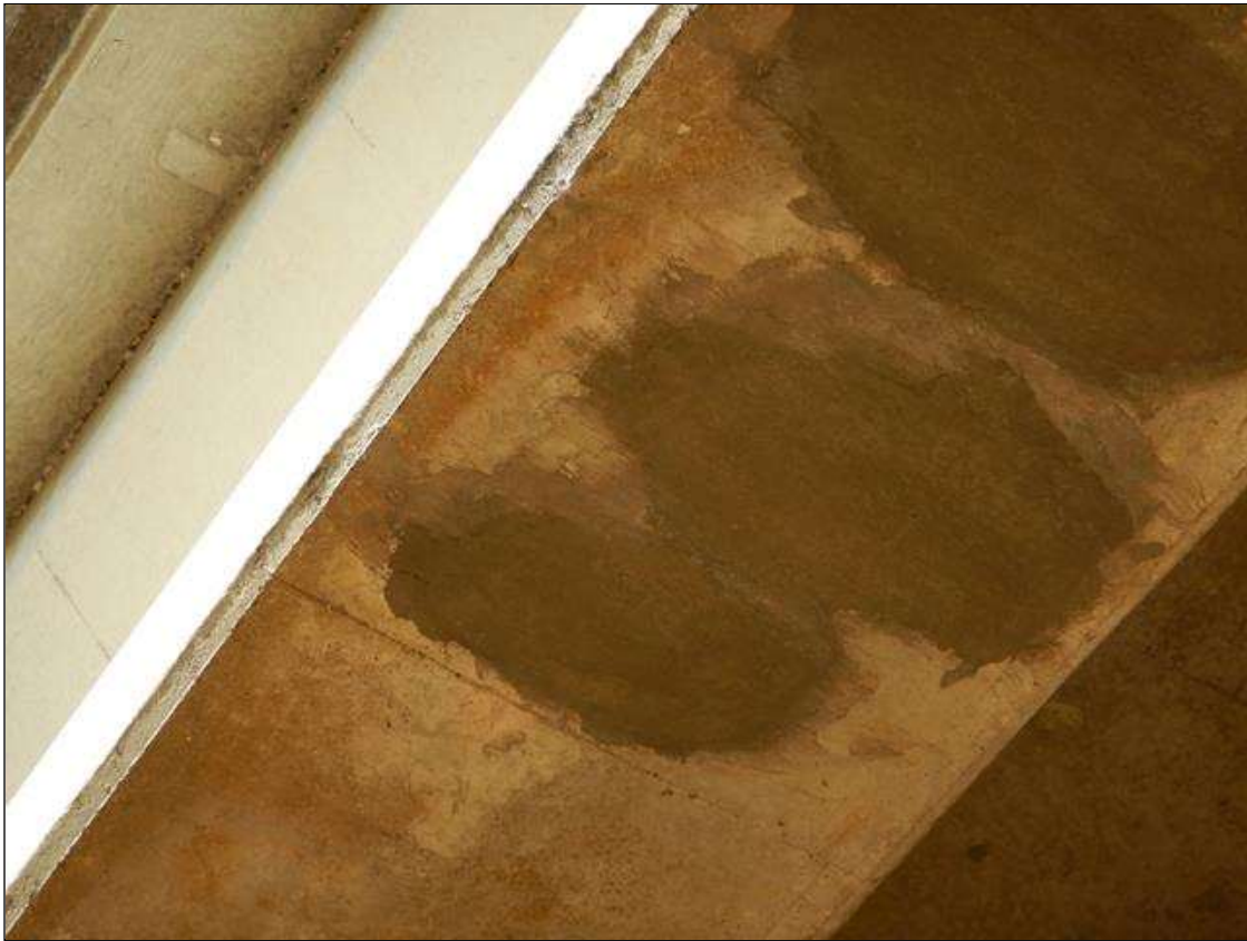
Span 30 Beam 11: [NEW REPAIR-PATCHING] FORMERLY --> spall with exposed rebar on the bottom face at 24ft from bent 28 (6" x 1" x 1/4")
