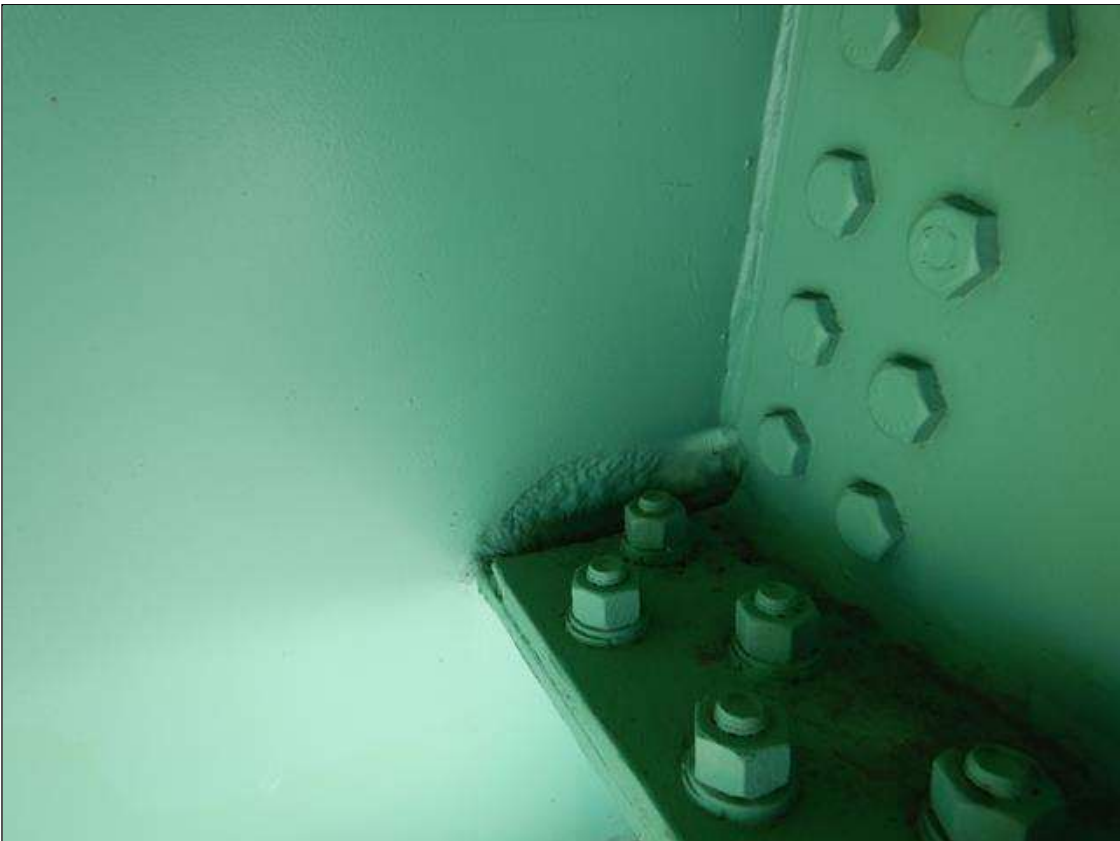
Span 20 Beam 8: [NEW REPAIR - NUT REPLACED] FORMERLY --> Bracket 3 at EB Parking Area West Face: section loss up to 75% section loss on (x1) nut; section loss in the web (6" x 2 1/2") by up to (1/16") into the web
