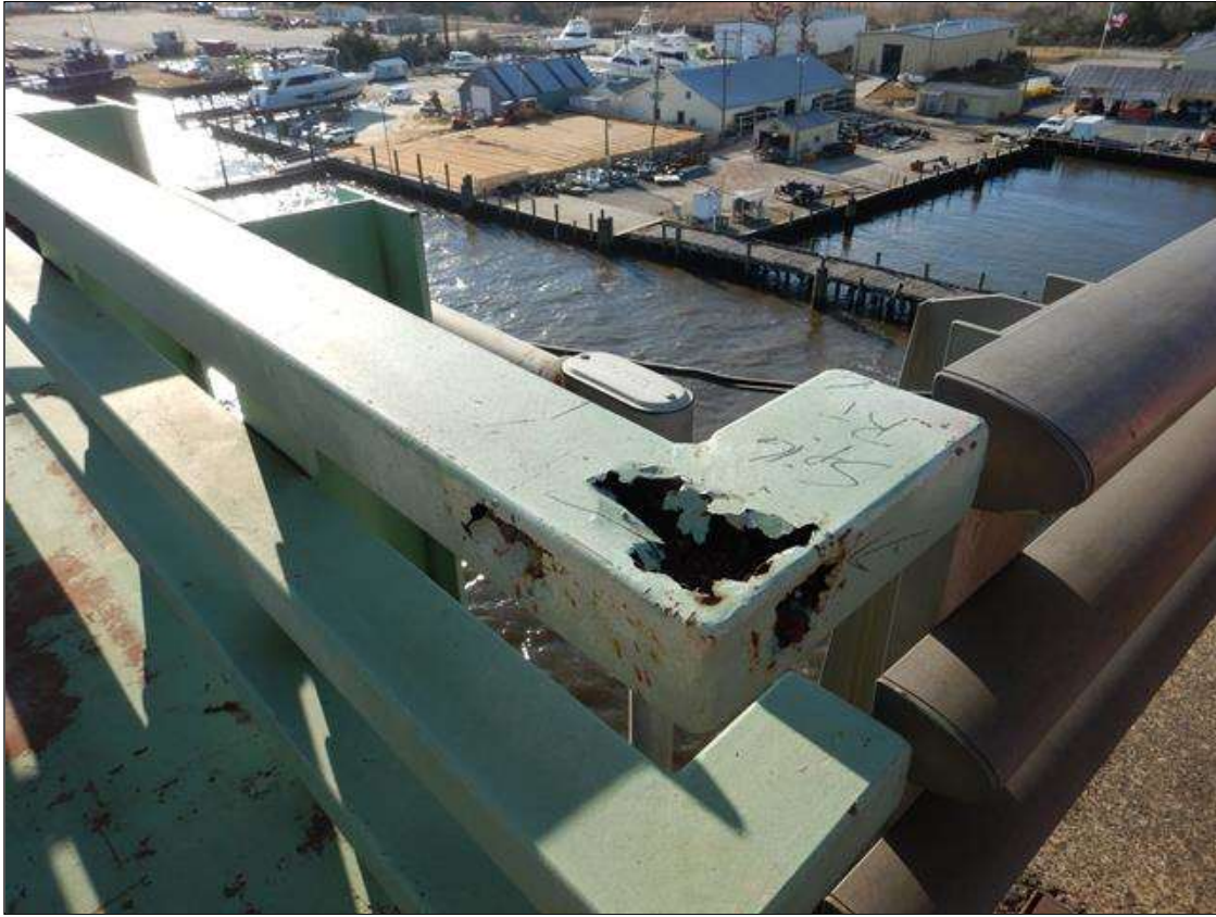
Span 16 Right Bridge Rail: [PROMPT ACTION REQUEST] AT THE PARKING AREA, THE TOP RAIL AT THE WEST END HAS CORROSION HOLES IN THE TOP AND SIDE AT THE CORNER UP TO 5" WIDE X 4" LONG IN THE TOP AND UP TO 3" DIAMETER ON THE SIDES
