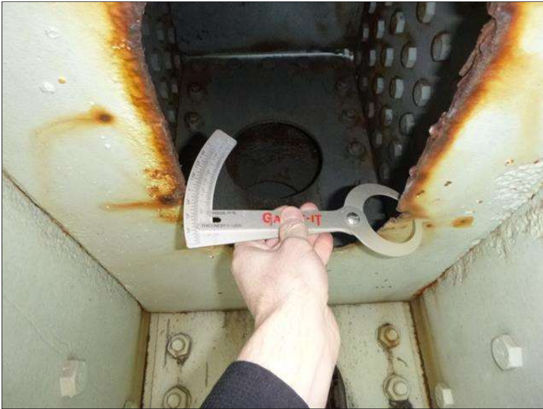
Span 18 Lift Span L11L12 NORTH: OBSERVED IN 2020 INSP: 2" WIDE SECTION AROUND BOTTOM PORTAL AT L12 REDUCED TO 1/16" WIDE/ 100% LOSS TO 1" AREAS AT EDGE - ACTIVE CORROSION PRESENT, PAR ISSUED.
