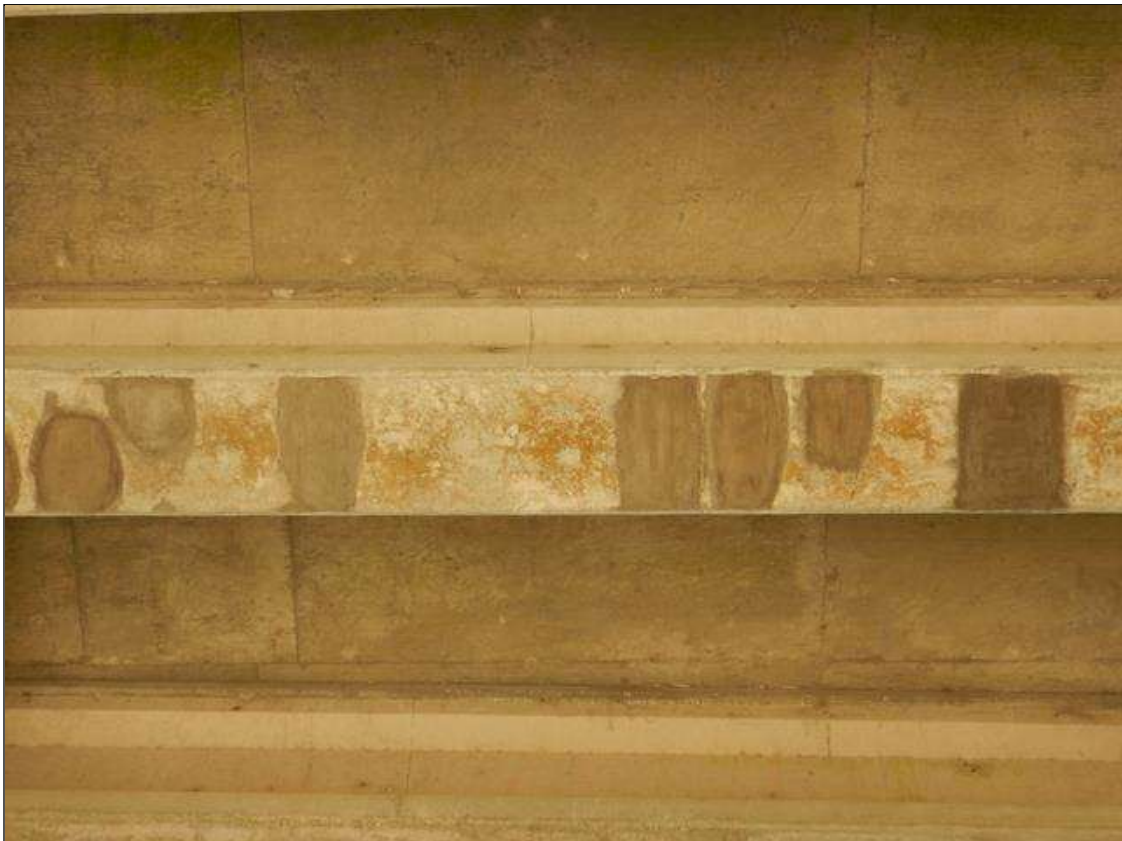
Span 28 Beam 9: [NEW REPAIR-PATCHING] FORMERLY --> (x5) spalls with exposed rebar on the bottom face up to (18" x 6" x 1") and unsound patches up to (18" x 9") near mid span
