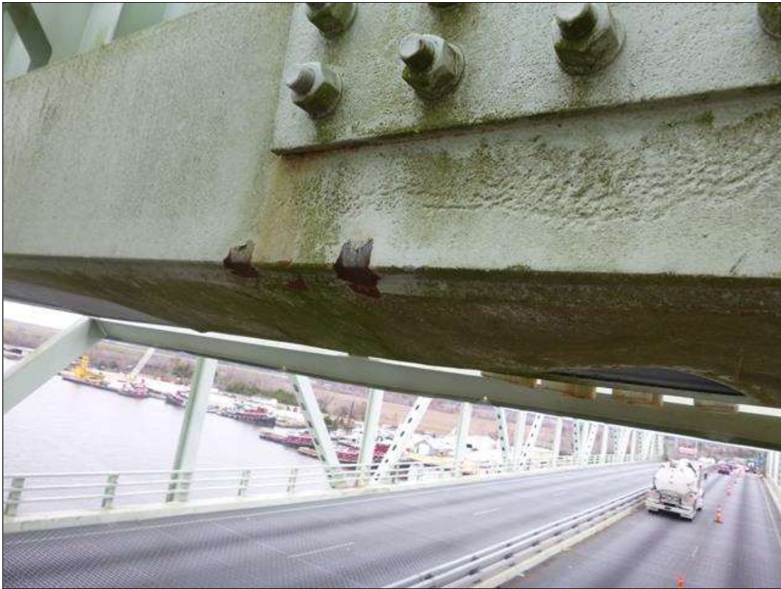
Span 19 EAST TOWER NORTH: 6/2020 - IMPACT DAMAGE - BOTTOM WEST HORIZONTAL TRUSS MEMBER - (2) 1"WIDE x 3/4"LONG x 3/16"DEEP GOUGES, AND (1) ~1/2" DIAMETER x 1/16"DEEP INDENTION ON BOTTOM EAST CORNER AT 11'-3" FROM NORTHWEST TOWER LEG
