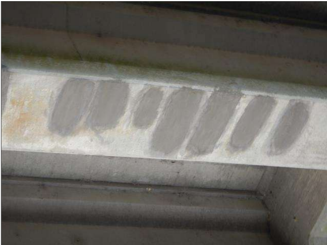
Span 29 Beam 7: [NEW REPAIR-PATCHING] FORMERLY --> spall with exposed rebar near large patched area near mid span (8" x 4" x 1/2")
