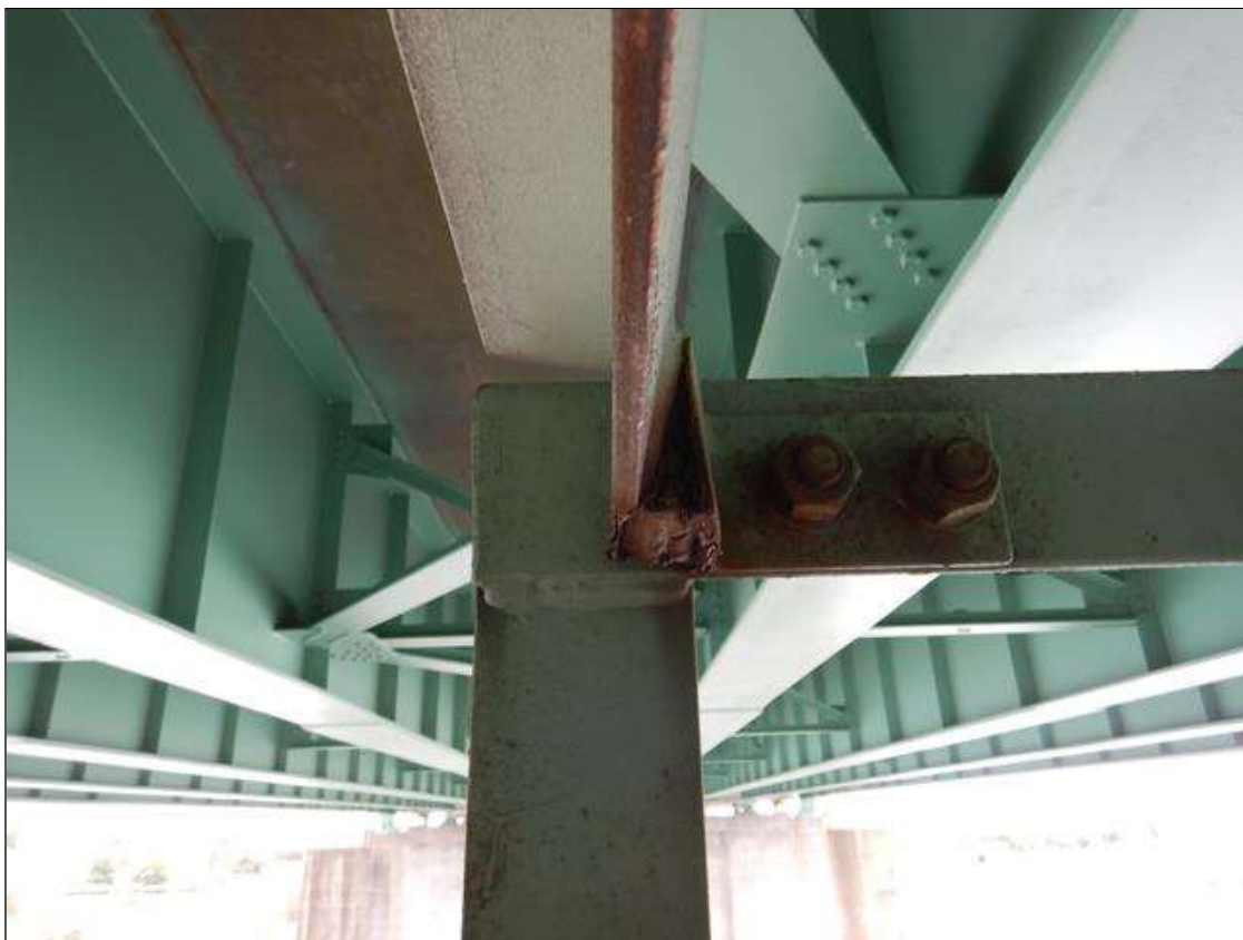
Span 20 Beam 1: surface corrosion and with pack rust between members of the platform attached to the beams at the west face of bent 18
