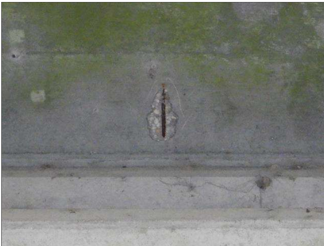
Span 5 Deck: bottom of the deck has a spall in bay 5 at mid-span, 5" long x 9" wide x 3/4" deep with exposed rebar
