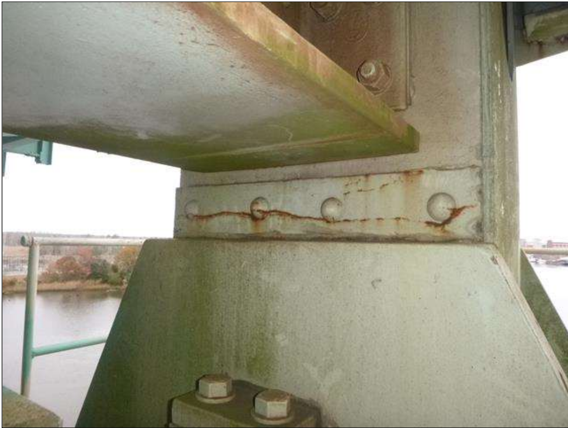
Span 17 WEST TOWER NORTH: WEST TOWER: RUST LEACHING ALONG HAIRLINE CRACK SOUTH FACE IN BRACE PLATE. ULTRASONIC INSPECTION REQUESTED.
