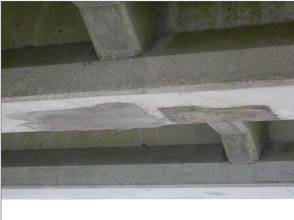
Span 11 Beam 8: [NEW REPAIR - PATCHING] FORMERLY --> (x3) spalls in a 2ft area up to (5" x 5" x 1/2") at 21ft from bent 11
