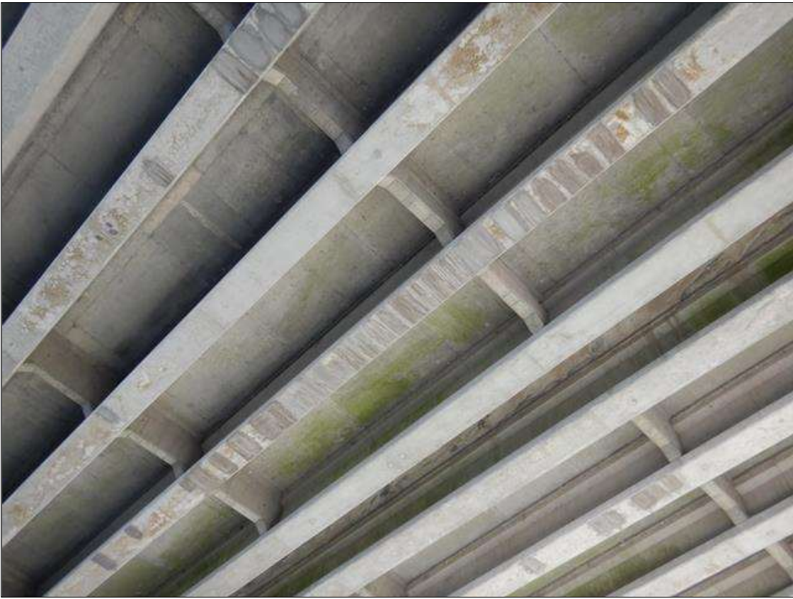
Span 27 Beam 6: [NEW REPAIR-PATCHING] FORMERLY --> (x23) spalls with exposed rebar on the bottom face up to (18" x 5" x 1/2")
