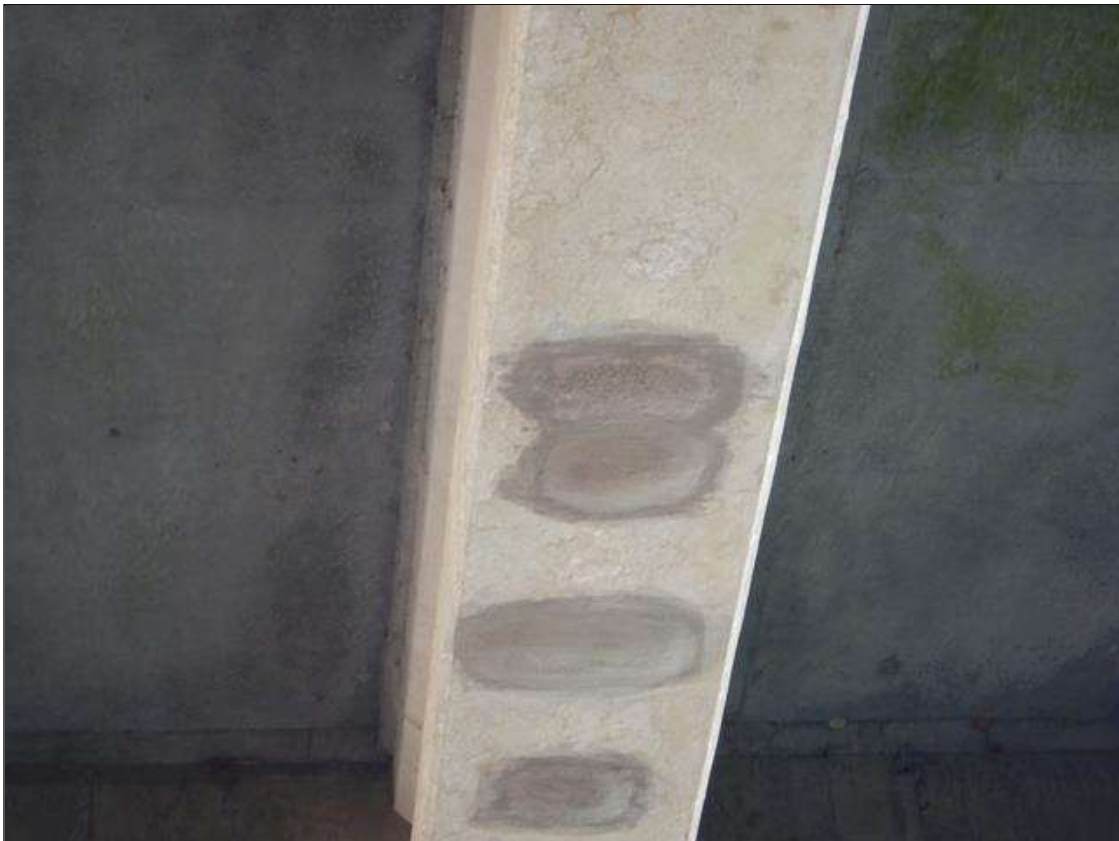
Span 29 Beam 2: [NEW REPAIR-PATCHING] FORMERLY --> (x2) spalls with exposed rebar on the bottom face at mid span up to (6" x 5" x 1/2")
