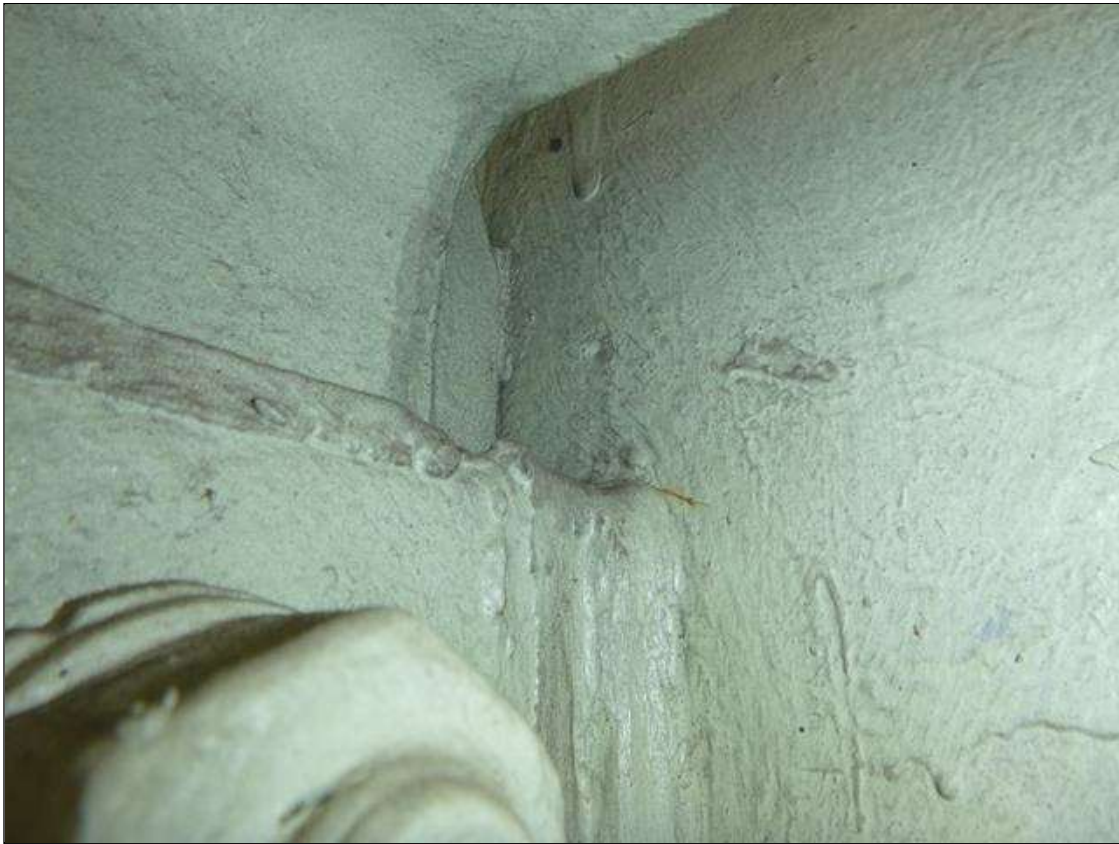
Span 18 Lift Span Stringer 5: BETWEEN FB'S 1- 2 - 1-1/2" LONG CRACK IN WEB ACROSS TOP OF WELD AT DIAPHRAGM CONNECTION
