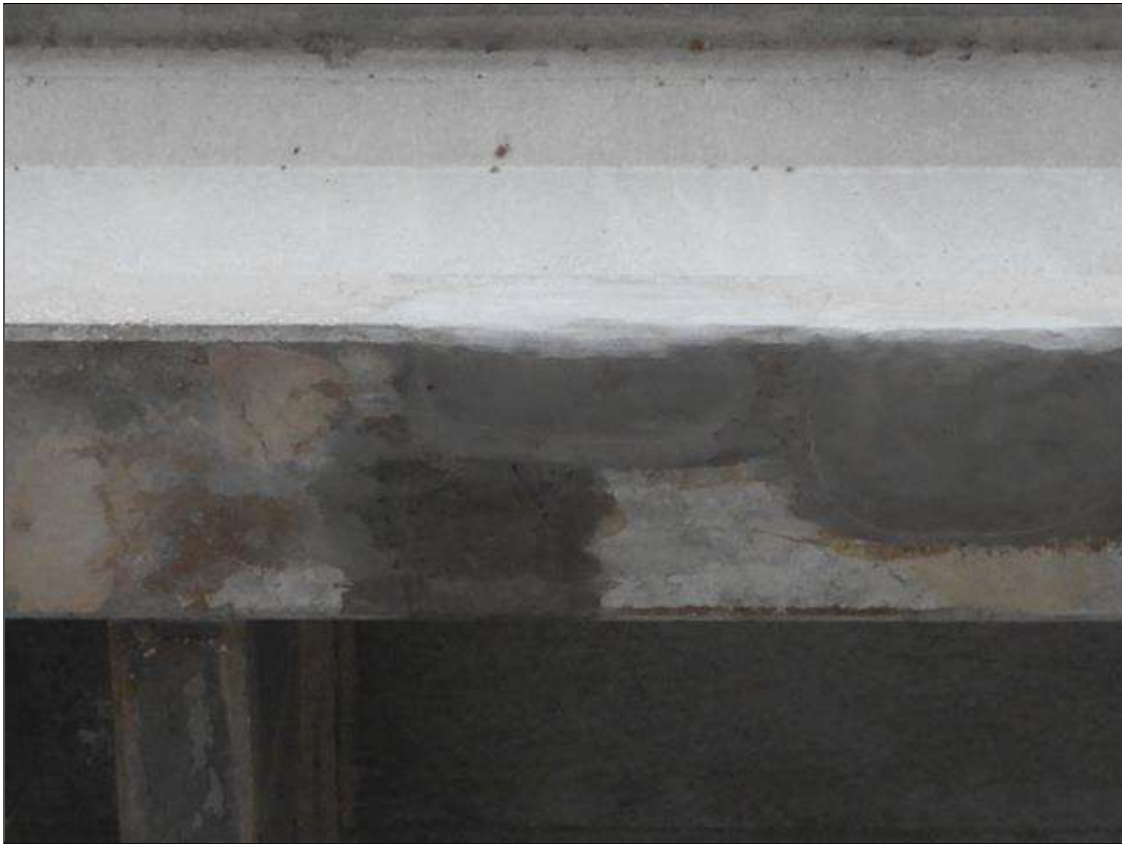
Span 9 Beam 9: [NEW REPAIR - PATCHING] FORMERLY --> PRIORITY MAINTENANCE - spall with exposed strands on the bottom face at 14ft from bent 9 (18" x 7" x 2"), strand exposed for (10") long
