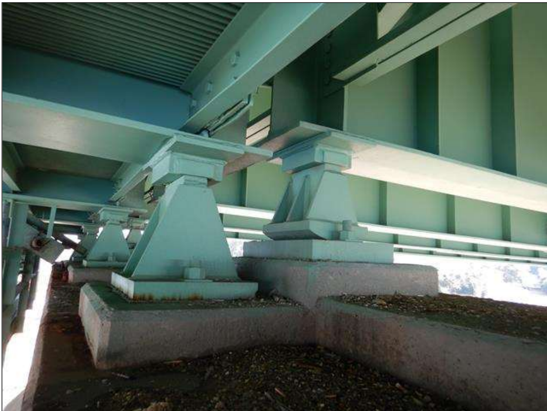
GIRDERS 4 BEARINGS AT BENT 18, TYPICAL BEARINGS AT BENT 18 [SIMILAR AT BENT 19 & BENT 20]
