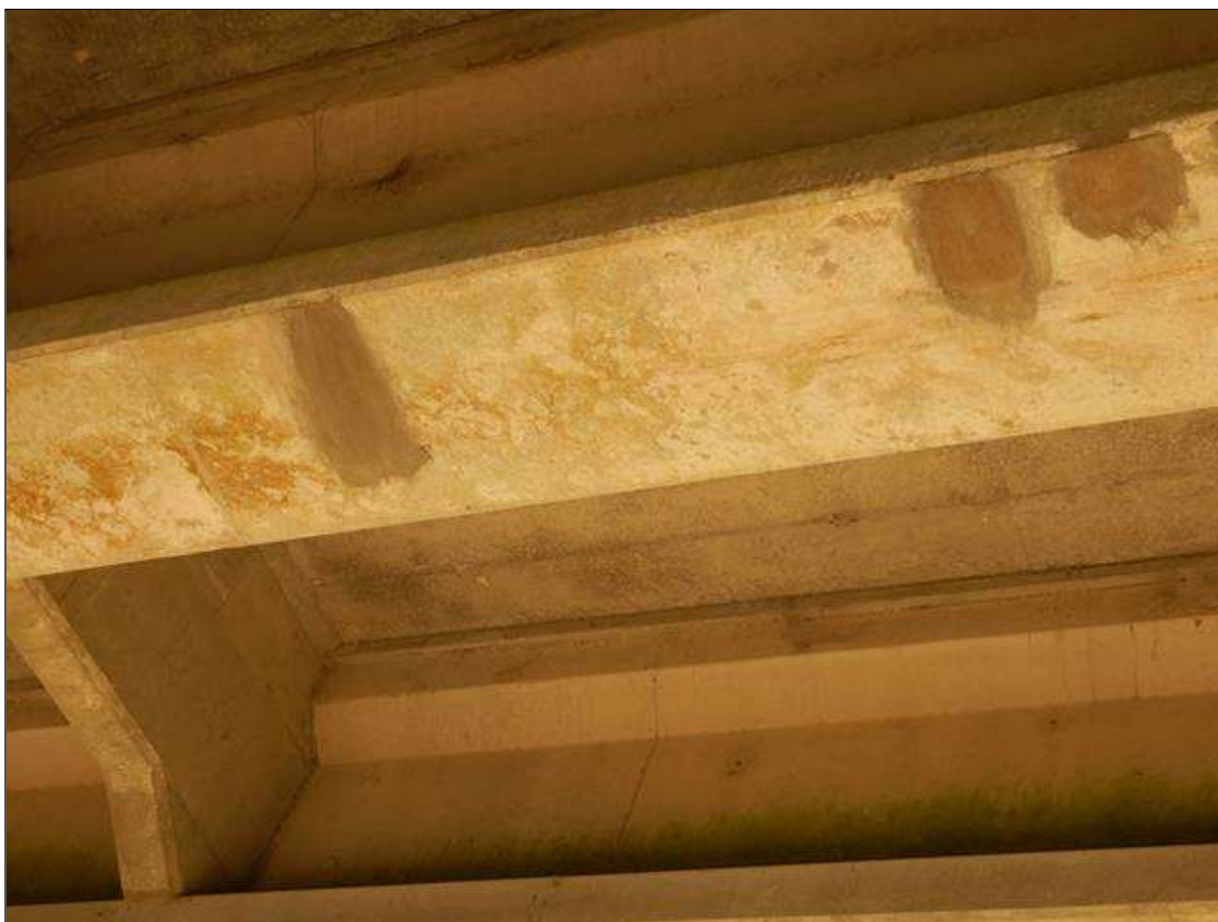
Span 30 Beam 9: [NEW REPAIR-PATCHING] FORMERLY --> spall with exposed rebar on the bottom face at mid span (11" x 5" x 1/4")
