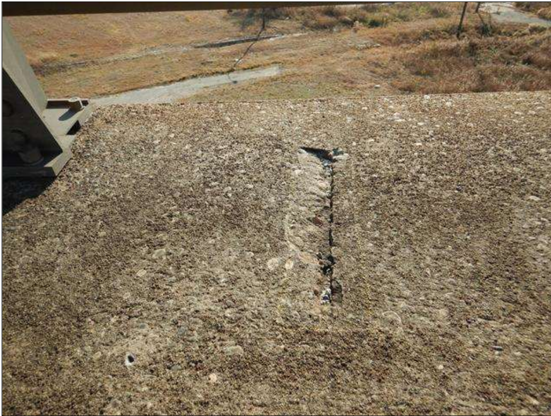
Span 22 Right Bridge Rail: TOP OF THE REINFORCED CONCRETE CURB, SPALLING WITH EXPOSED REBAR [APPROXIMATELY 16" X 2" X 3/4"], NO MEASURABLE SECTION LOSS
