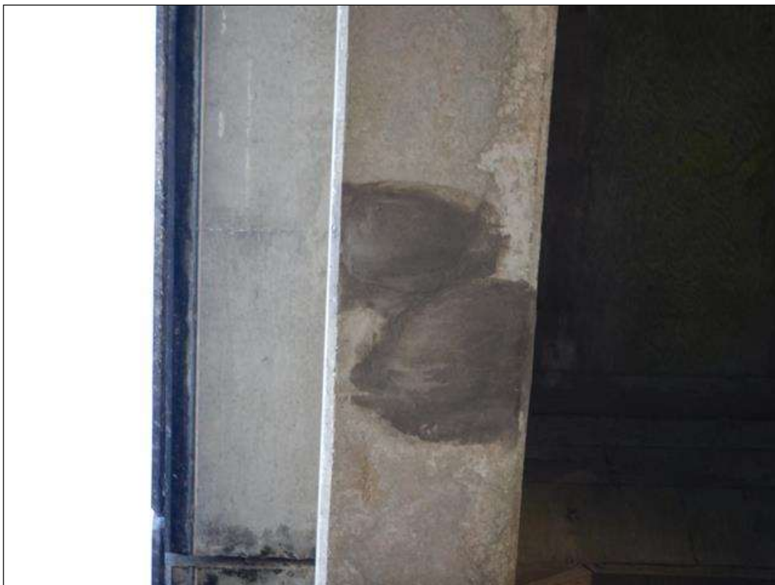
Span 28 Beam 1: [NEW REPAIR-PATCHING] FORMERLY --> (x2) spalls with exposed rebar on the bottom face at 3ft from bent 26 up to (8" x 6" x 3/4")
