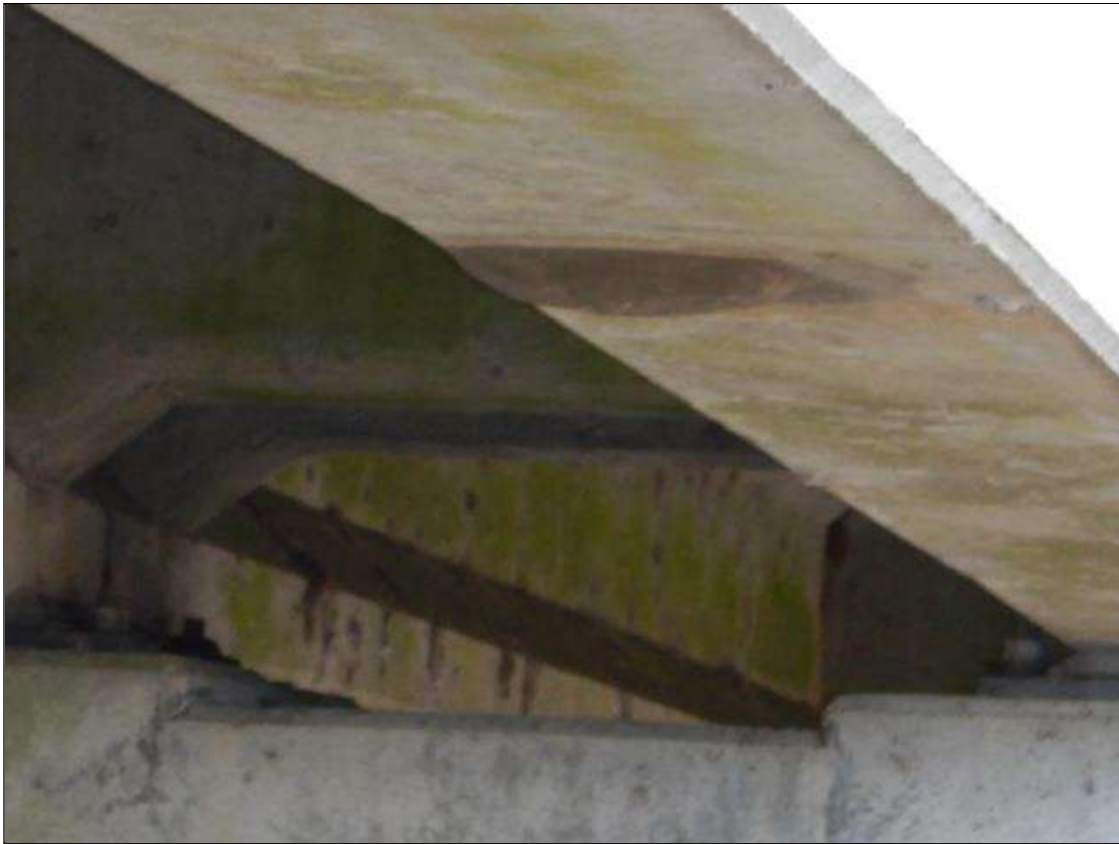
Span 2 Beam 1: [NEW REPAIR - PATCHING] FORMERLY --> spall with exposed rebar on the bottom face at 22.5ft from bent 1 (10" x 6" x 1/2")
