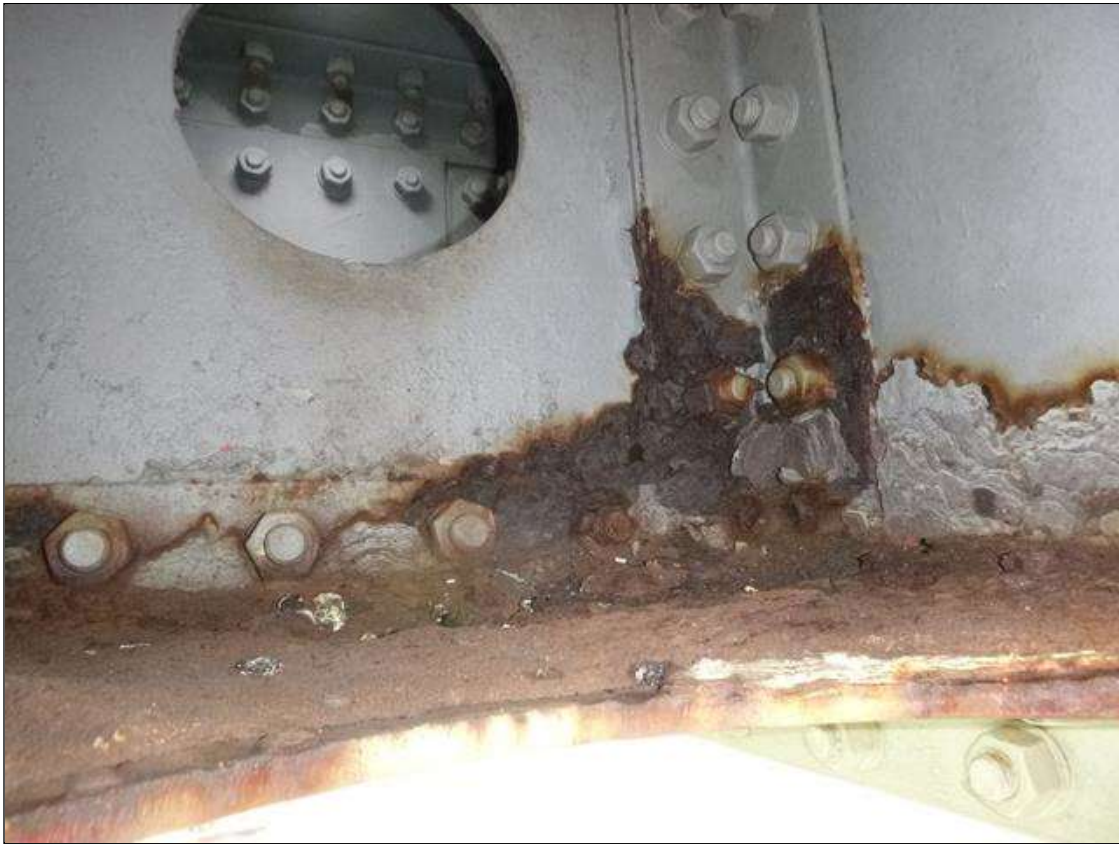
Span 18 Lift Span U0 NORTH: [PROMPT ACTION REQUEST] WHEEL GUIDE TOP OF BOTTOM PLATE AND INTERNAL BRACING HAS RUST SCALE AND 1" DIAMETER CORROSION HOLE IN INTERNAL BRACING.
