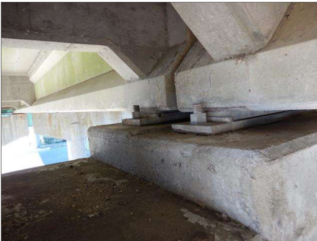
GIRDERS 8 BEARINGS AT BENT 25 [SIMILAR AT SPAN 28 FAR BEARINGS AND SPAN 27 NEAR BEARINGS]
