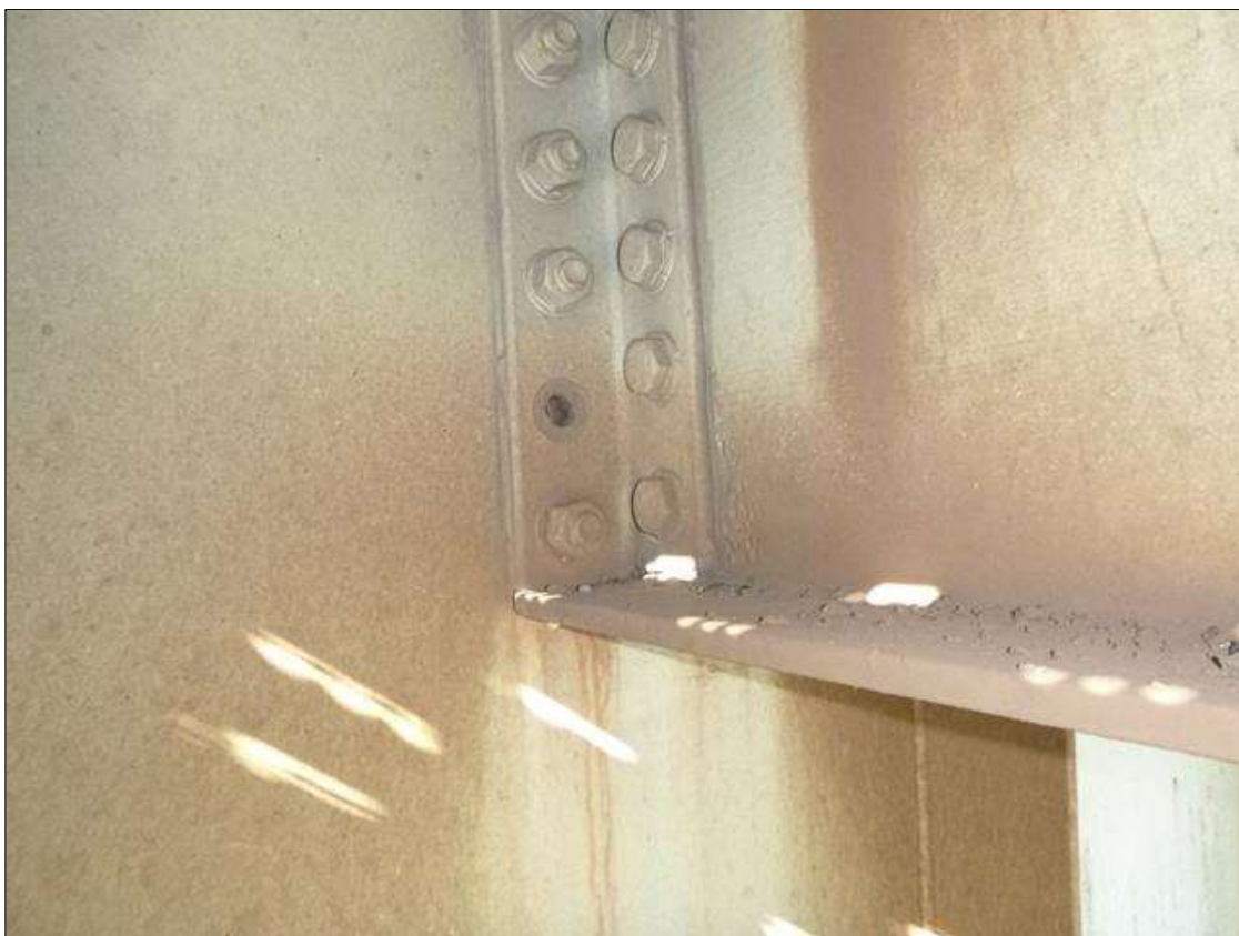
Span 18 Lift Span Stringer 2: ONE BOLT MISSING ON EACH SIDE OF THE STRINGER CONNECTION TO FB 1, PAR ISSUED.
