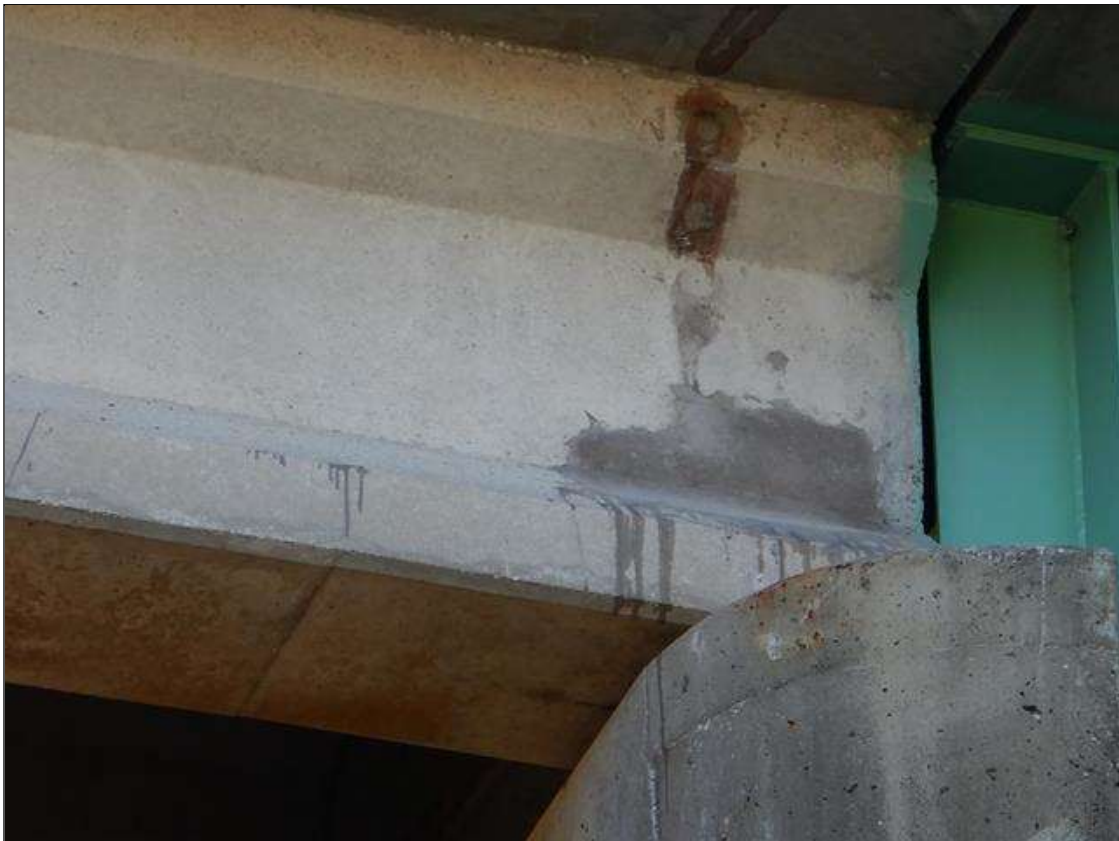
Span 27 Beam 1: [NEW REPAIR-PATCHING] FORMERLY --> spall with exposed rebar on the left web at bent 24 (20" x 2" x 1/4")
