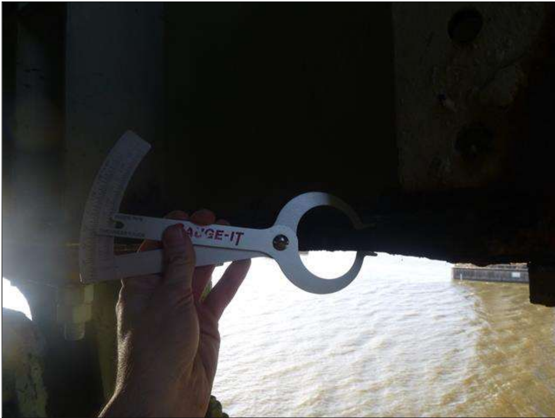
Span 18 Lift Span Floor Beam 12: LOSS OF SECTION .625" WITH .683" REMAINING BOTTOM EAST FLANGE 4' LONG X 3.25" WIDE OVER OLD ANCHOR POINT BEGINNING 2' LEFT OF NORTHEAST BEARING. PAINT HAS FAILED. (PAR)
