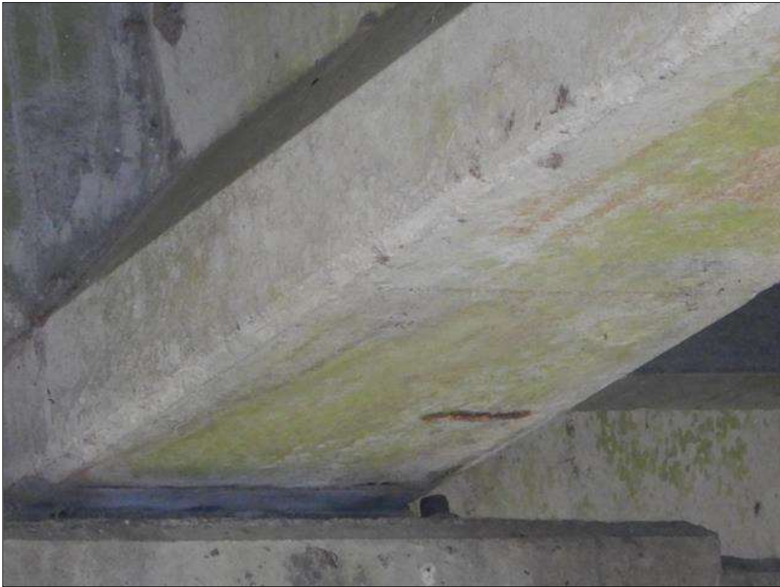
Span 2 Beam 2: [PROMPT ACTION REQUEST] 14" section of 2 areas of exposed rebar in the bottom face at bent 2 up to (6" x 2")
