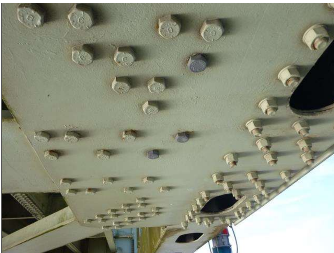
Span 18 Lift Span L6 NORTH: (3) NEW BOLTS IN BOTTOM GUSSET AT FLOORBEAM AND LATERAL BRACING CONNECTION ON EAST SIDE
