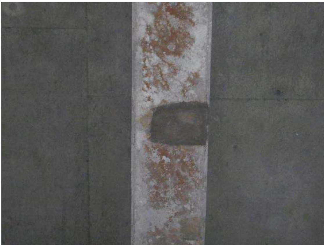
Span 8 Beam 2: [NEW REPAIR - PATCHING] FORMERLY --> (9" x 7" x 1/2") spall with exposed rebar on the bottom face at 17ft from bent 7
