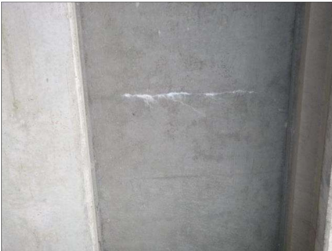
Span 32 Deck: hairline transverse surface cracking with EFFLORESCENCE. in bays 11, 10 and 9
