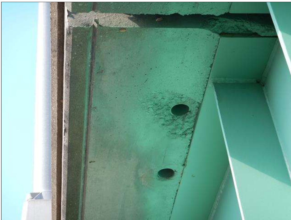
Span 21 Deck: spall with no exposed steel at deck drain on the right overhang at bent 19 (14" x 12" x 1 1/2")
