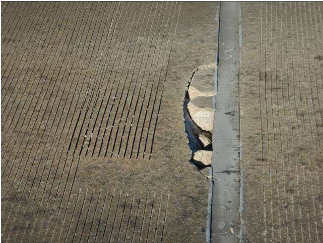
Span 22 Deck: [PROMPT ACTION REQUEST] RIGHT LANES AT BENT 20, SPALL (30" LONG x 3" WIDE x 4" DEEP AT 8' FROM MEDIAN RAIL)
