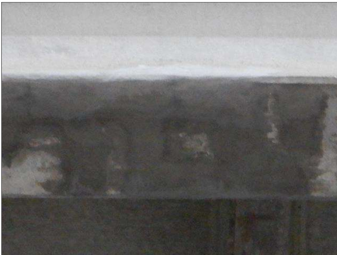
Span 10 Beam 9: [NEW REPAIR - PATCHING] FORMERLY --> PRIORITY MAINTENANCE - (x2) spalls with exposed strands on the bottom face starting at 18ft from bent 9 (23" x 9" x 1 1/2") & (14" x 10" x 1") in a failed repair with total area of (60" x 20"), (x4) strands exposed up to (19") long
