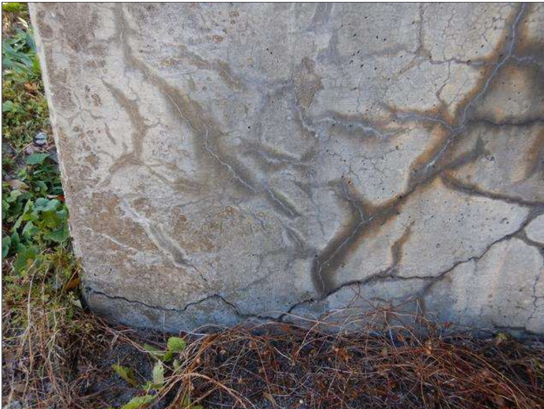
Ramp End Bent Ramp End Bent Cap: horizontal cracking on the west face under girder 1 up to (1/2") wide for 5.5ft long (surface efflorescence present)
