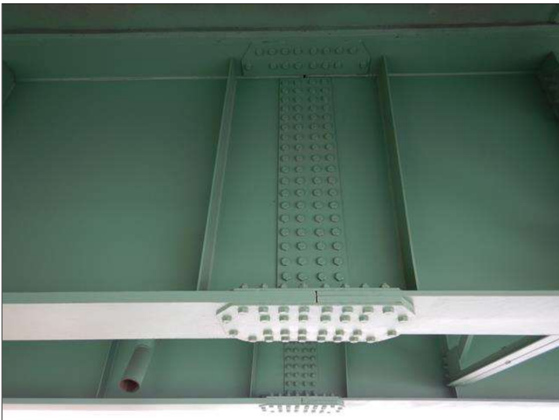
SPAN 14 GIRDER 2 SPLICE [TYPICAL FOR ALL CONTINUOUS SPAN SPLICES]
