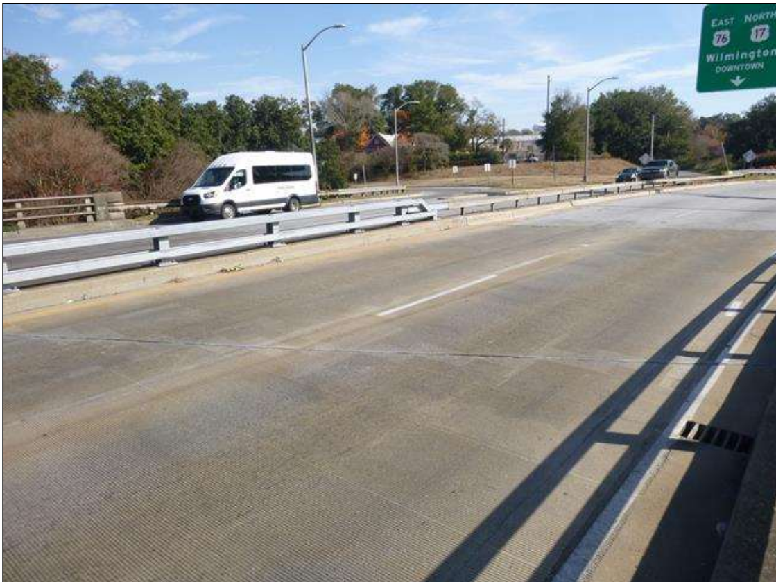
SPAN 32 EPOXY OVERLAY [ ALL SPANS SIMILAR EXCEPT THE LIFT SPAN XXXXXXXXXXXXXXXXXXXX
