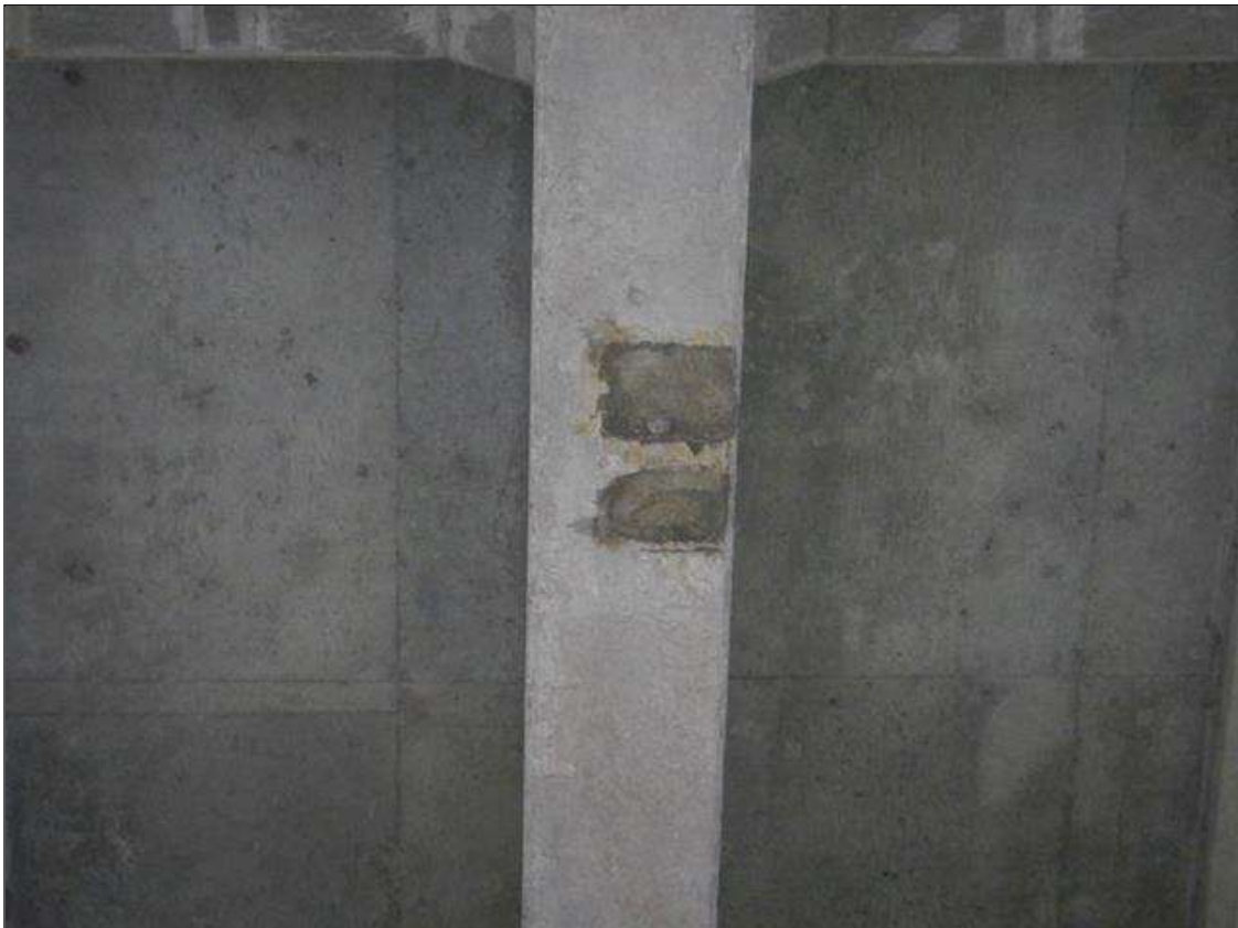
Span 8 Beam 7: [NEW REPAIR - PATCHING] FORMERLY --> (x2) spalls with exposed rebar on the bottom face at 13ft from bent 7 up to (6" x 3" x 1/4")
