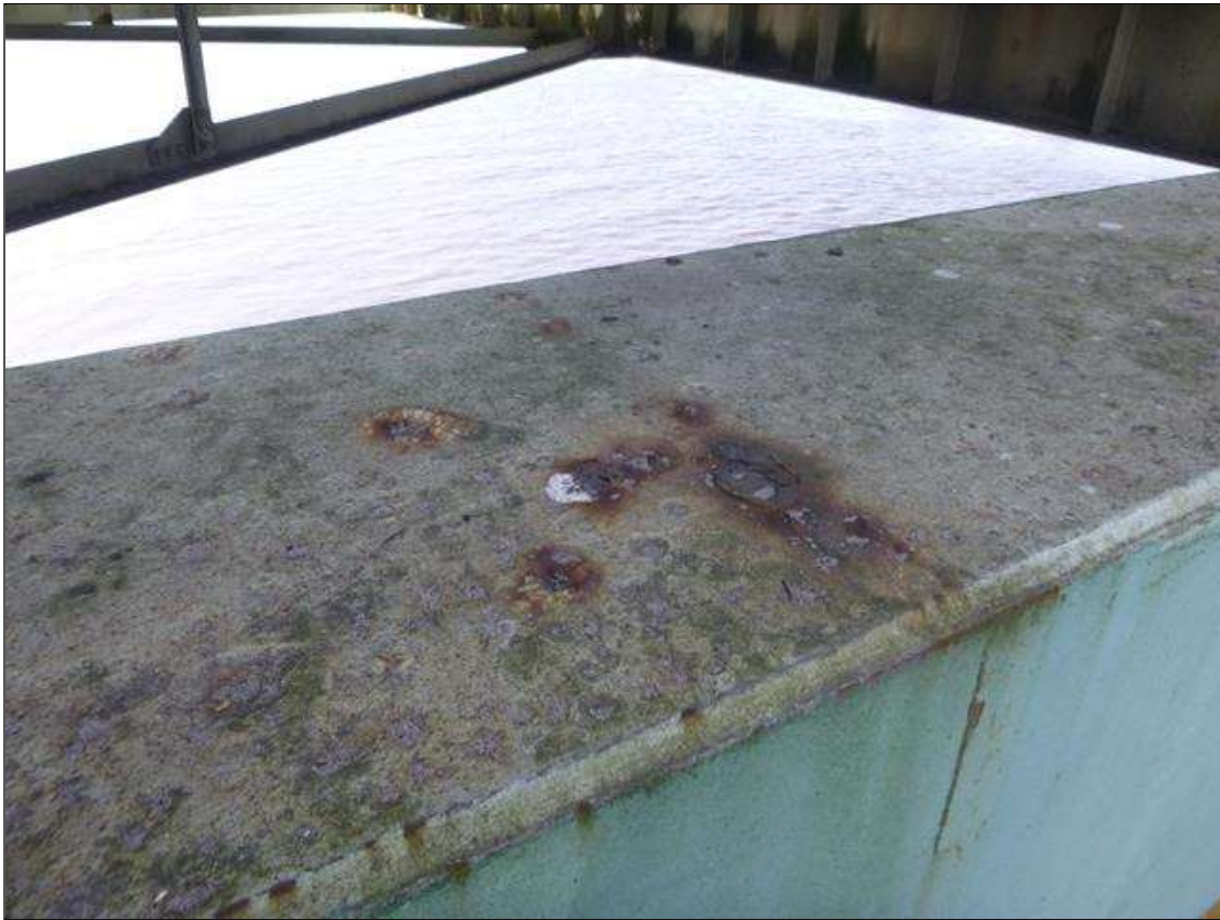
Span 18 Lift Span L11L12 NORTH: OBSERVED IN 2020 INSP: PITTED AREAS UP TO 2" IN DIAMETER x 1/4" DEEP SCATTERED THROUGHOUT TOP OF CHORD - ACTIVE CORROSION PRESENT IN SOME OF THESE AREAS, PAR ISSUED.
