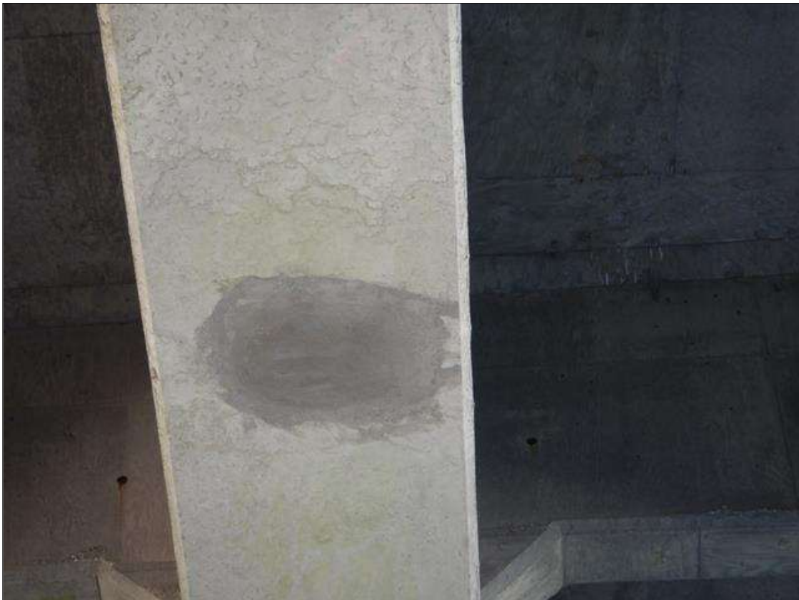
Span 30 Beam 3: [NEW REPAIR-PATCHING] FORMERLY --> spall with exposed rebar on the bottom face at 18ft from bent 27 (11" x 10" x 1/4")
