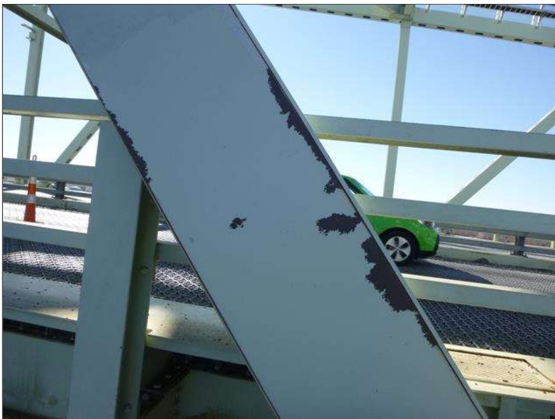
Span 18 Lift Span L2U3 NORTH - Protective System: NORTH FACE 5' FROM L2 PEELING OF TOP COAT
