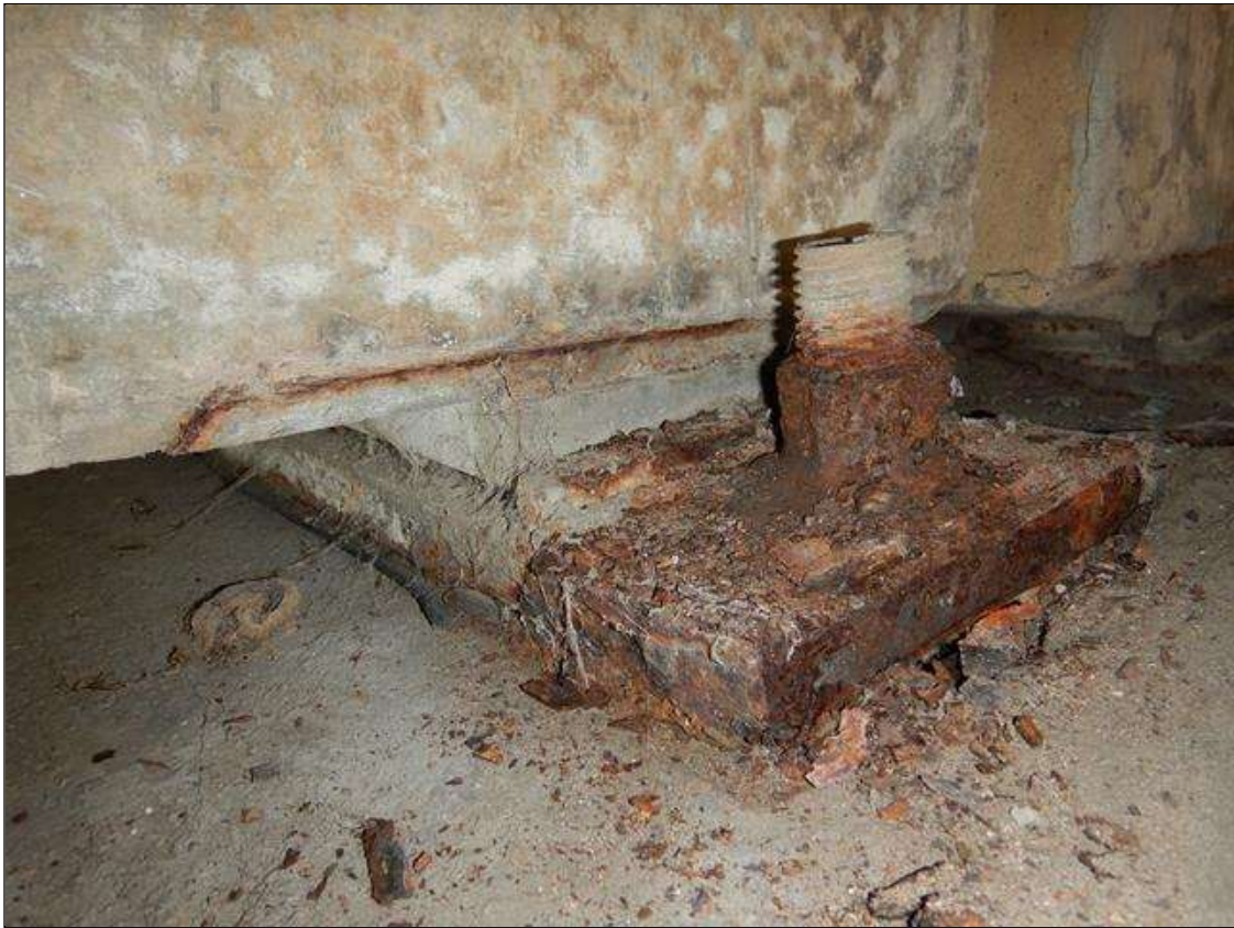
Span 3 Beam 5 - Beam 5 Near Bearing: LEFT ANCHOR NUT HAS CORROSION WITH APPROXIMATELY 50% SECTION LOSS
