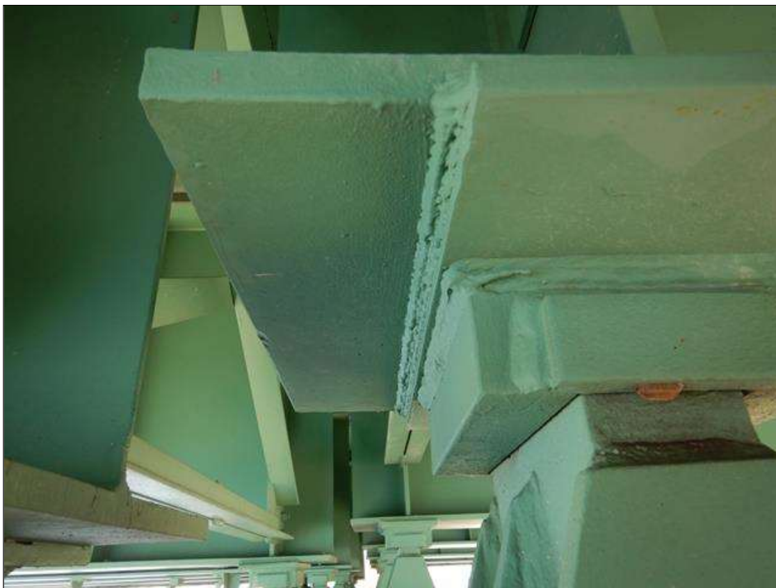
Span 21 Beam 6 - Beam 6 Near Bearing: REPAINTED
