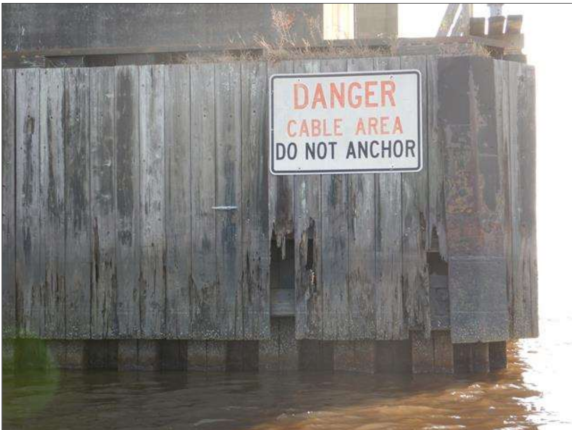
Bent 17 - Lift Span Bent Footing: (5) TIMBER SHEETING BUFFER BOARDS ARE DECAYED/BROKEN ON NORTHWEST SIDE WITH SECTION MISSING.
