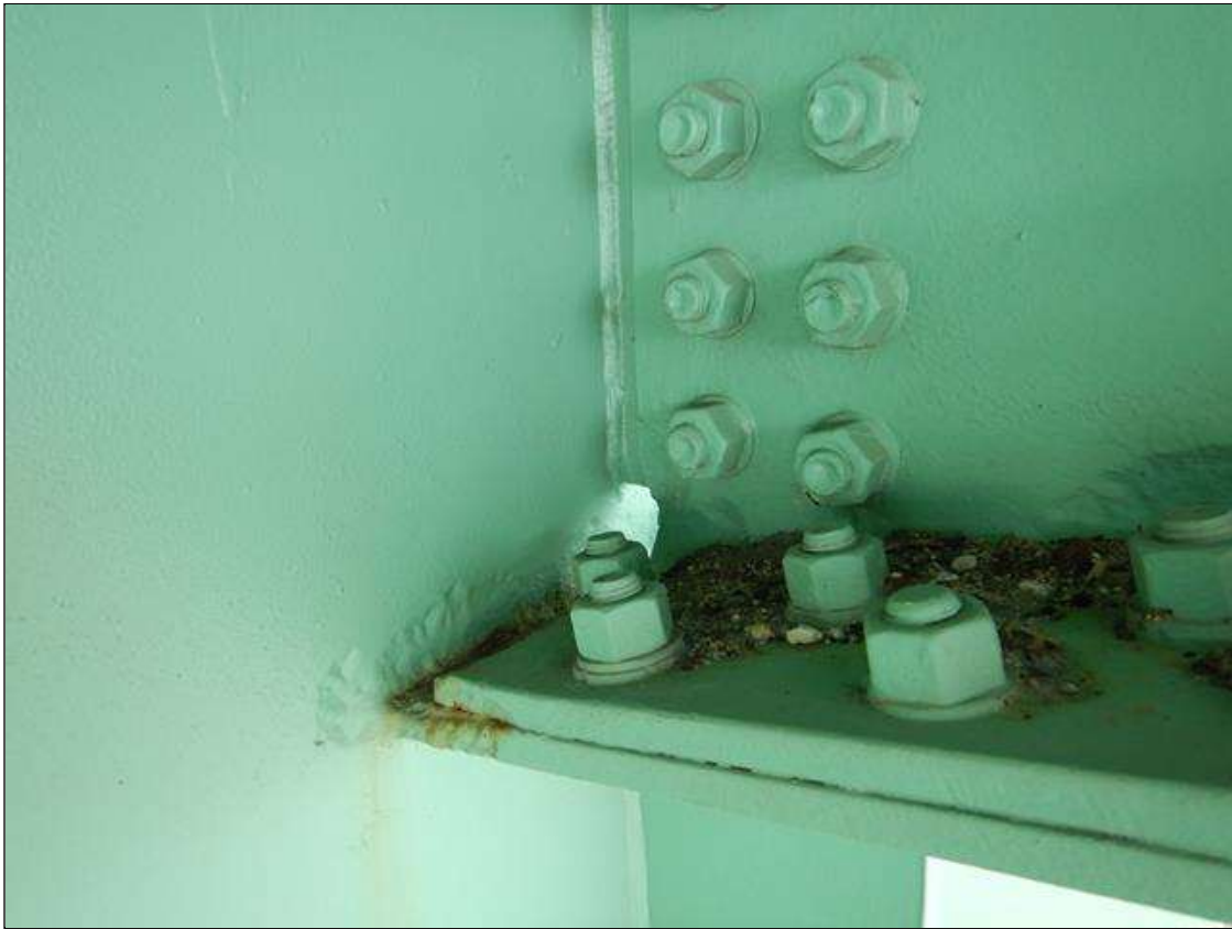
Span 16 Beam 1: [NEW REPAIR - NUTS REPLACED] FORMERLY --> PRIORITY MAINTENANCE - Bracket 1 at WB Parking Area both faces: section loss on the bottom flange/plate of the brace beam at the web (7" x 1 3/4") with (11/16") remaining; up to 100% section loss on (x2) nut on the bottom plate on both faces; active corrosion with no measureable section loss web on both faces (PROMPT ACTION REQUEST)
