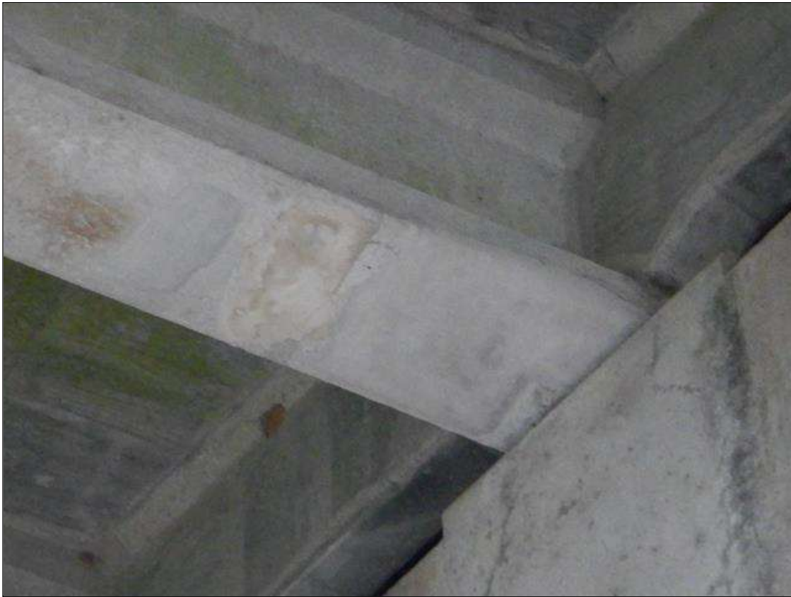
Span 8 Beam 5: [NEW REPAIR - PATCHING] FORMERLY --> PRIORITY MAINTENANCE - spall with exposed strand on the bottom right face at bent 8 (27" x 20" x 3"), up to 100% section loss of strand for 10in long (PROMPT ACTION REQUEST).
