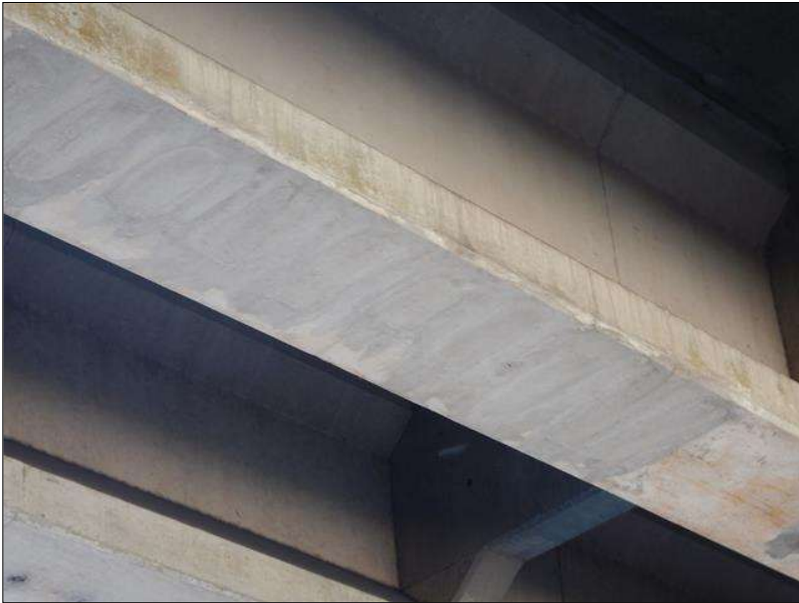
Span 31 Beam 2: [NEW REPAIR-PATCHING] FORMERLY --> (x25) spalls with exposed rebar on the bottom face at mid span up to (20" x 5" x 1/2")
