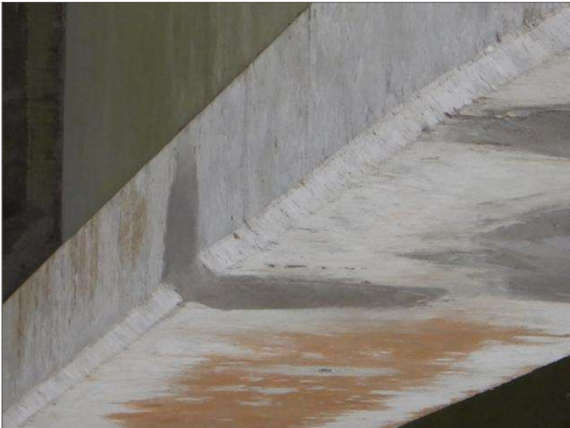
Span 11 Beam 6: [NEW REPAIR - PATCHING] FORMERLY --> PRIORITY MAINTENANCE - spall with exposed strands on the bottom right face at 12ft from bent 10 (34" x 7" x 2"), strand exposed for 20" long
