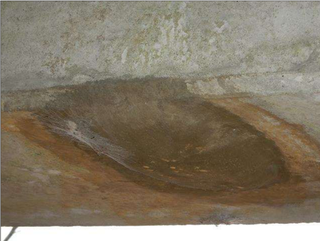
Span 2 Beam 1: [NEW REPAIR - PATCHING] FORMERLY --> spall with exposed rebar on the bottom face at 11ft from bent 1 (5" x 3" x 1/4")
