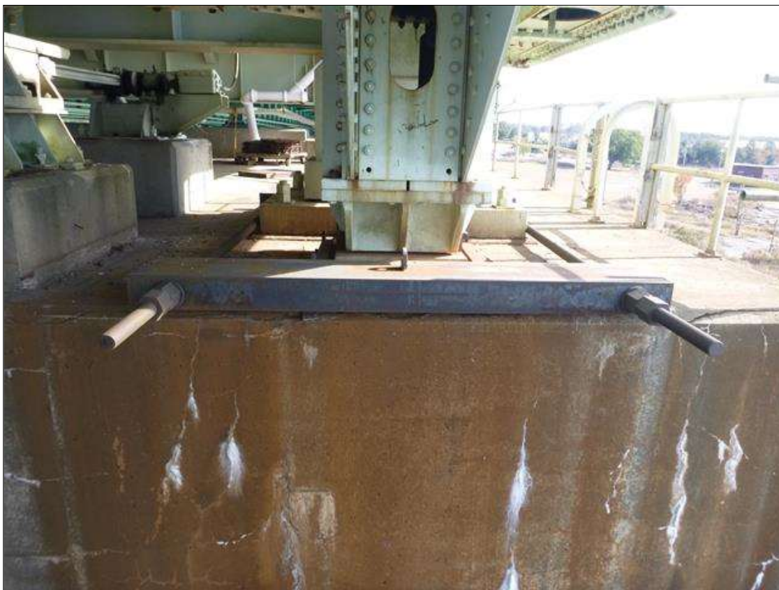
SOUTH TRUSS BEARING AT BENT 17, NORTH TRUSS BEARING SIMILAR
