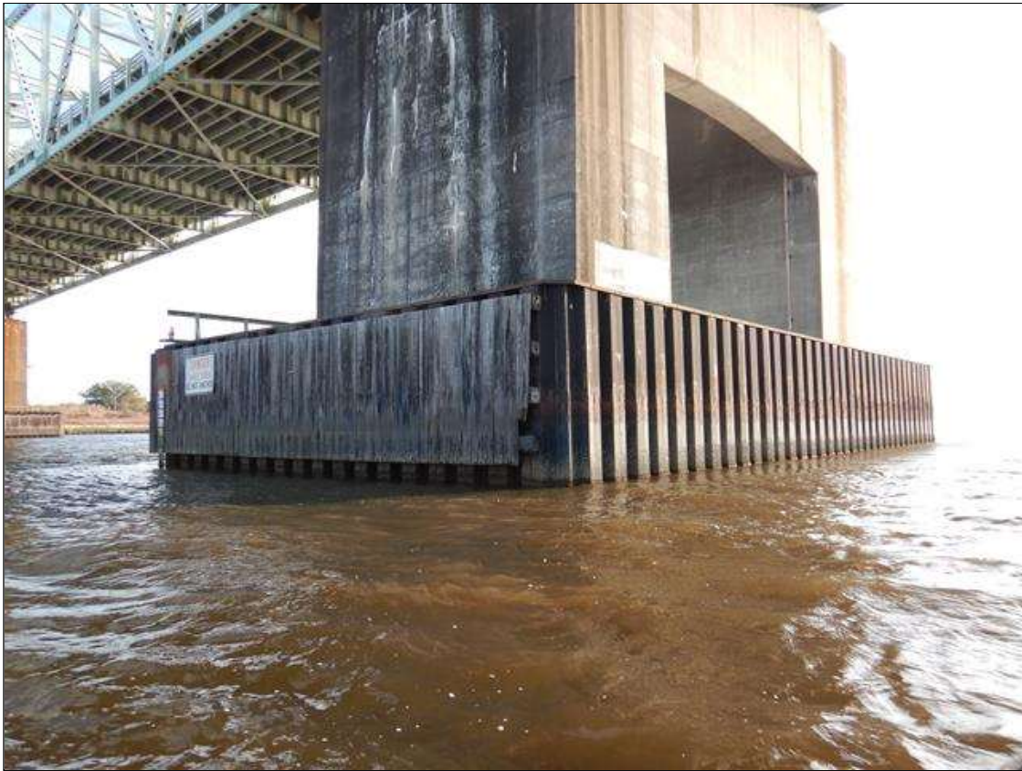
WEST TOWER PROTECTION AT THE WATERLINE, ALL SIDES [PROTECTION AT THE EAST TOWER SIMILAR]
