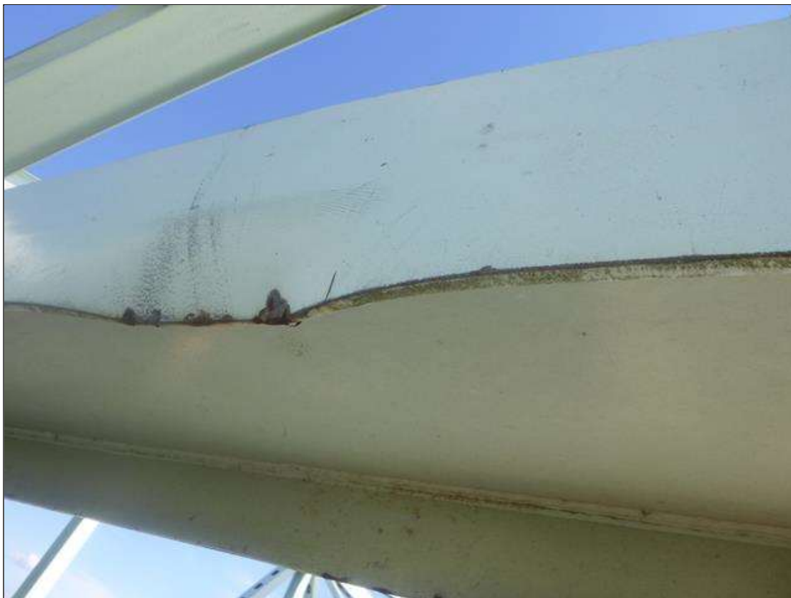
Span 18 Lift Span LB3: IMPACT DAMAGE 16" WIDE X 1-1/2" DEFORMATION IN BOTH FLANGES OVER RIGHT EAST BOUND LANE.
