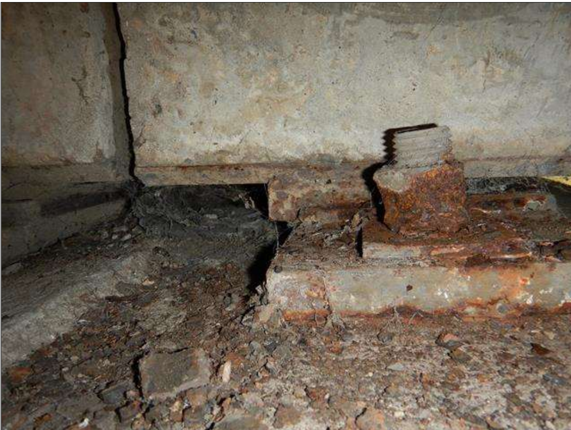
Span 1 Beam 3 - Beam 3 Far Bearing: Up to (3/4") movement of bearing to east beyond masonry plate with 13% loss in bearing
