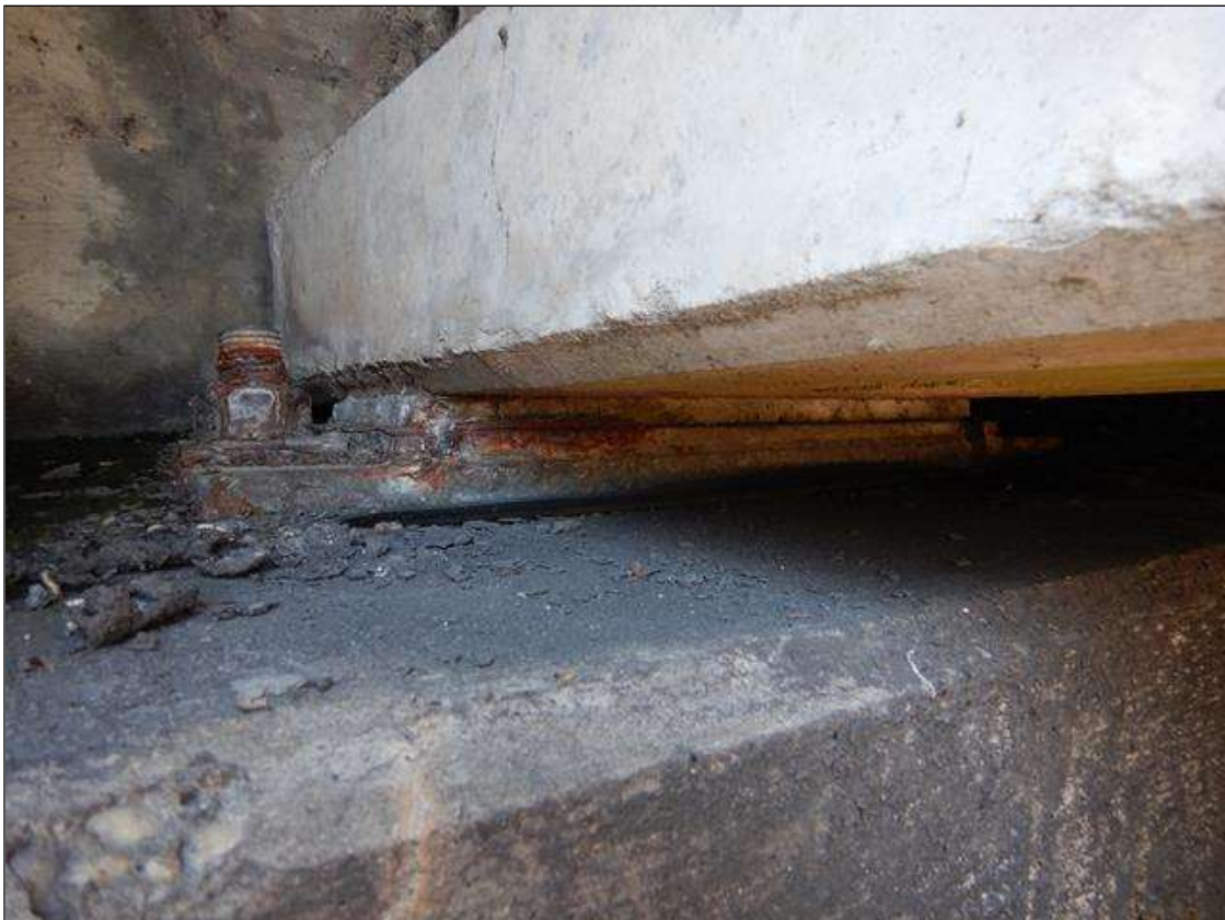
SPAN 1 GIRDER 9 NEAR BEARING [TYPICAL BEARING AT ABUTMENT 1]
