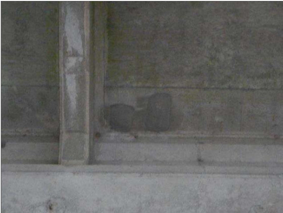
Span 8 Deck: [NEW REPAIR - PATCHING] FORMERLY --> (15" x 9") area of (x2) spalls with exposed rebar on the deck bottom in bay 5 at 17.5ft from bent 8 up to (9" x 2")
