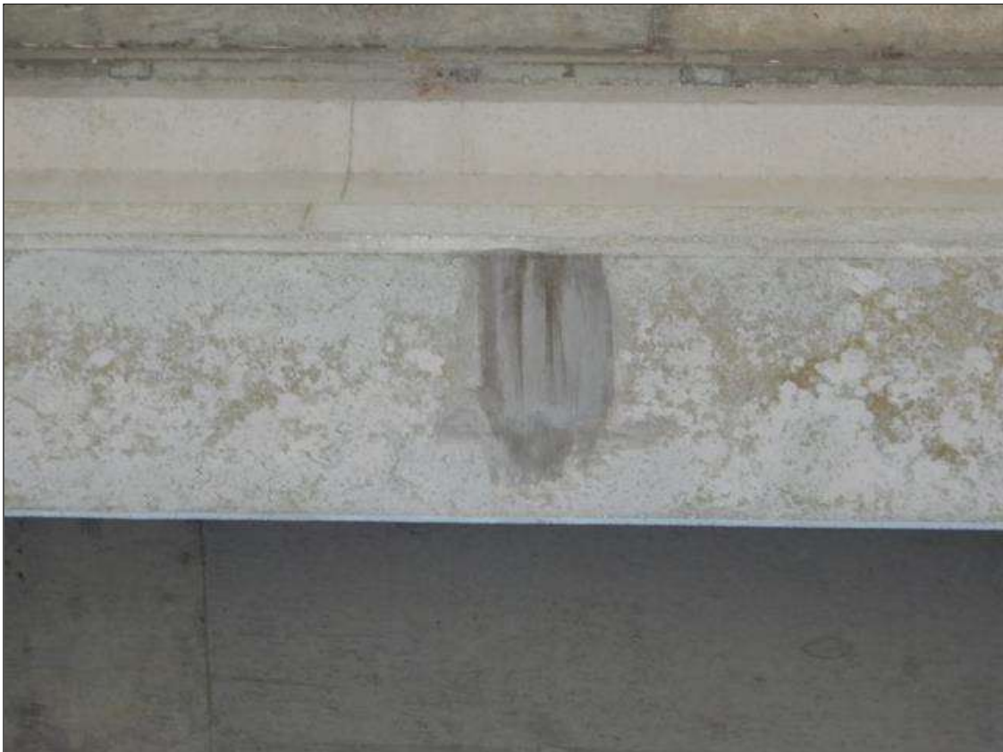
Span 27 Beam 4: [NEW REPAIR-PATCHING] FORMERLY --> spall with exposed rebar on the bottom face at 28ft from bent 24 (5" x 3" x 1/2")
