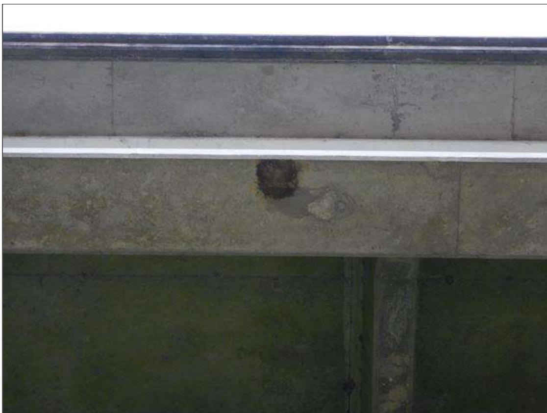
Span 6 Beam 1: [NEW REPAIR - PATCHING] FORMERLY --> (4" x 3" x 1/8") spall with exposed rebar on the bottom face at 19ft from bent 6
