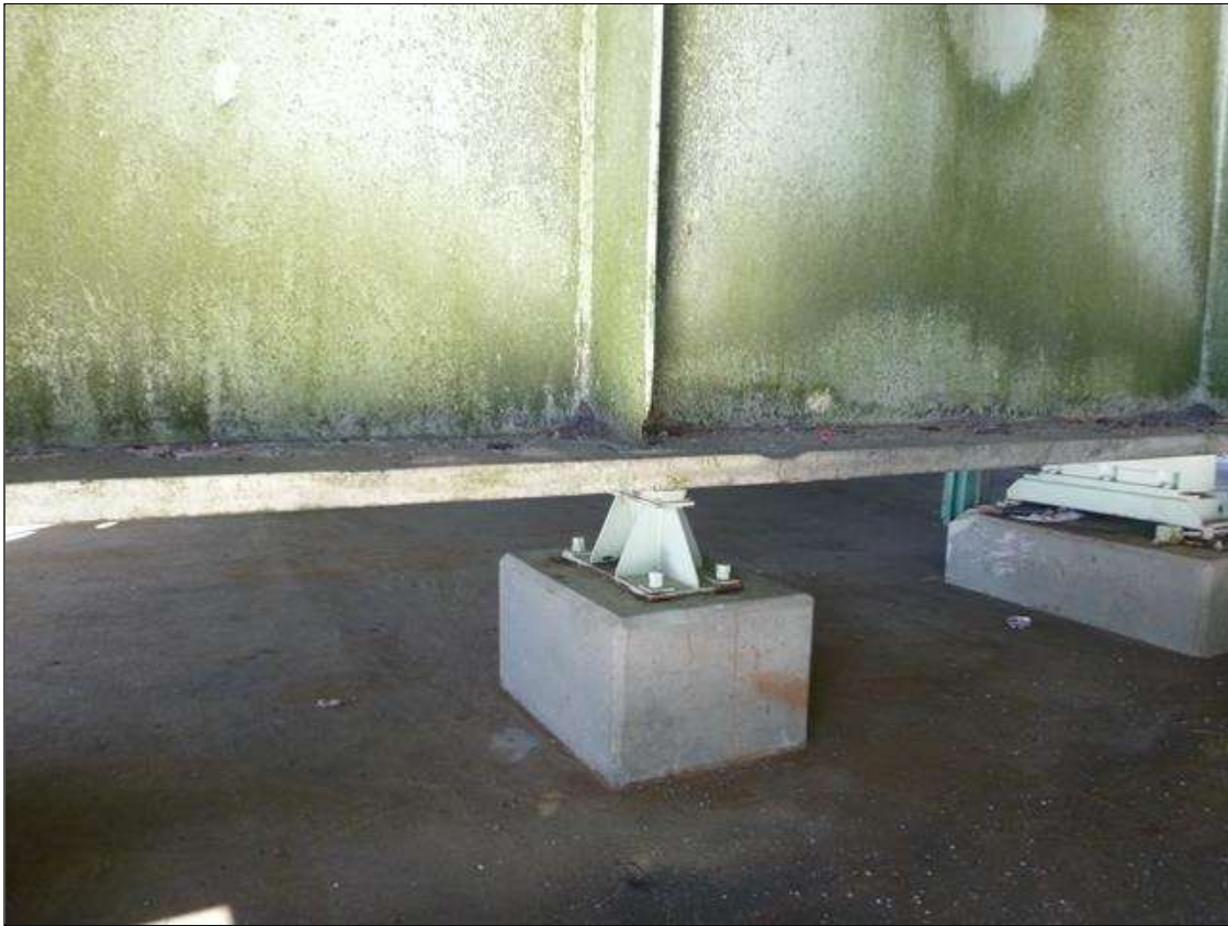
Span 18 Lift Span Floor Beam 0: PITTED AREAS UP TO 3/8" DEEP SCATTERED ALONG BOTH SIDES OF BOTTOM FLANGE AND STIFFENERS- CLEANED AND PAINTED.
