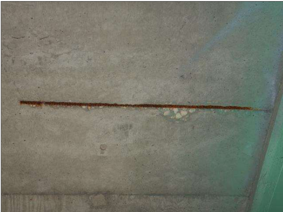
Span 14 Deck: spall with exposed rebar on the deck bottom in bay 5 at 30ft from Bent 13 (48" x 4" x 1/2")
