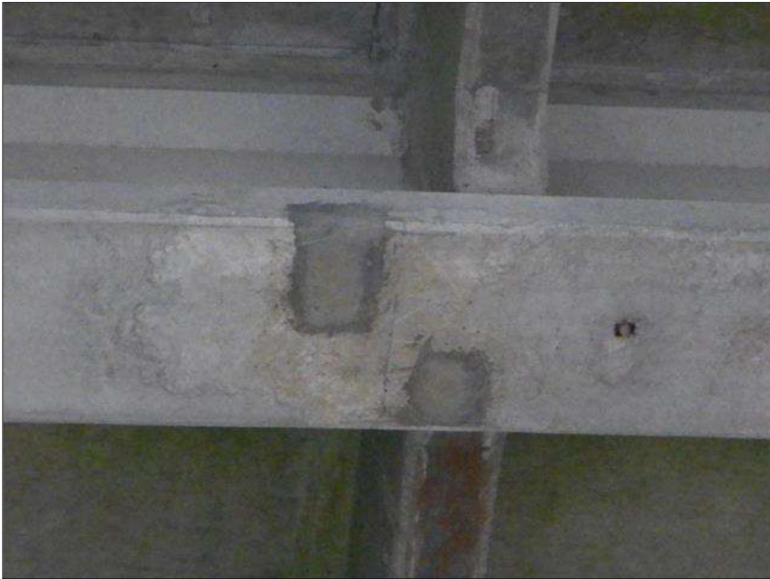
Span 10 Beam 5: [NEW REPAIR - PATCHING] FORMERLY --> (2 1/2" x 1/2") spall with exposed rebar in the bottom face at 22ft from bent 10
