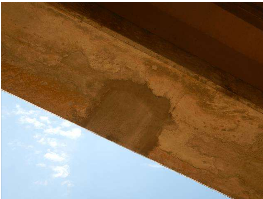
Span 30 Beam 11: [NEW REPAIR-PATCHING] FORMERLY --> DELAMINATION on the bottom face at 6ft from bent 28 (6" x 6")
