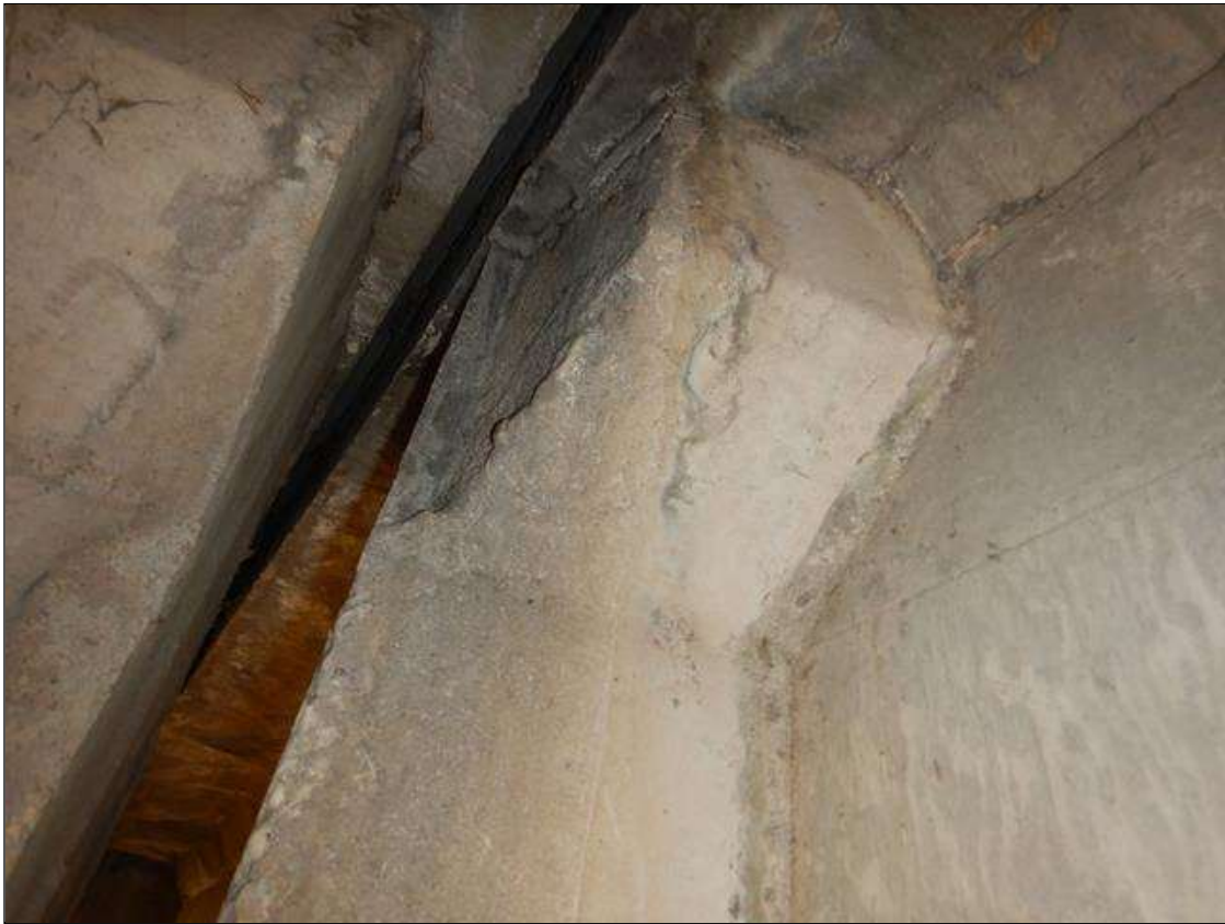
Span 31 Beam 11: [NEW REPAIR-PATCHING] FORMERLY --> spall with exposed rebar on the top of the back face at Bent 27 (6" x 5" x 1/2")
