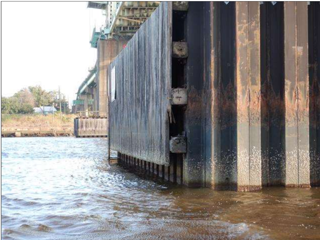
Bent 16 - Lift Span Bent Footing: BROKEN BOARD 5' HIGH NEAR CENTERLINE OF EAST FACE IN TIMBER SHEETING BUFFER.
