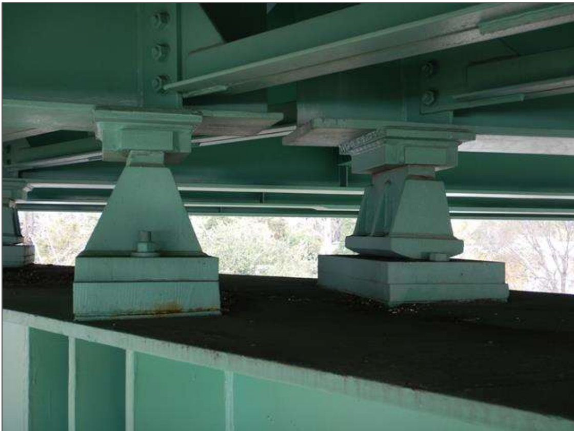
GIRDERS 4 BEARINGS AT BENT 22, TYPICAL BEARINGS AT BENT 22 [SIMILAR AT BENT 23]
