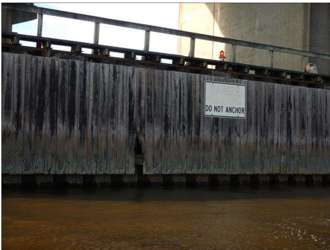
Bent 16 - Lift Span Bent Footing: broken and decayed timber at the bottom of the northwest corner (similar throughout)
