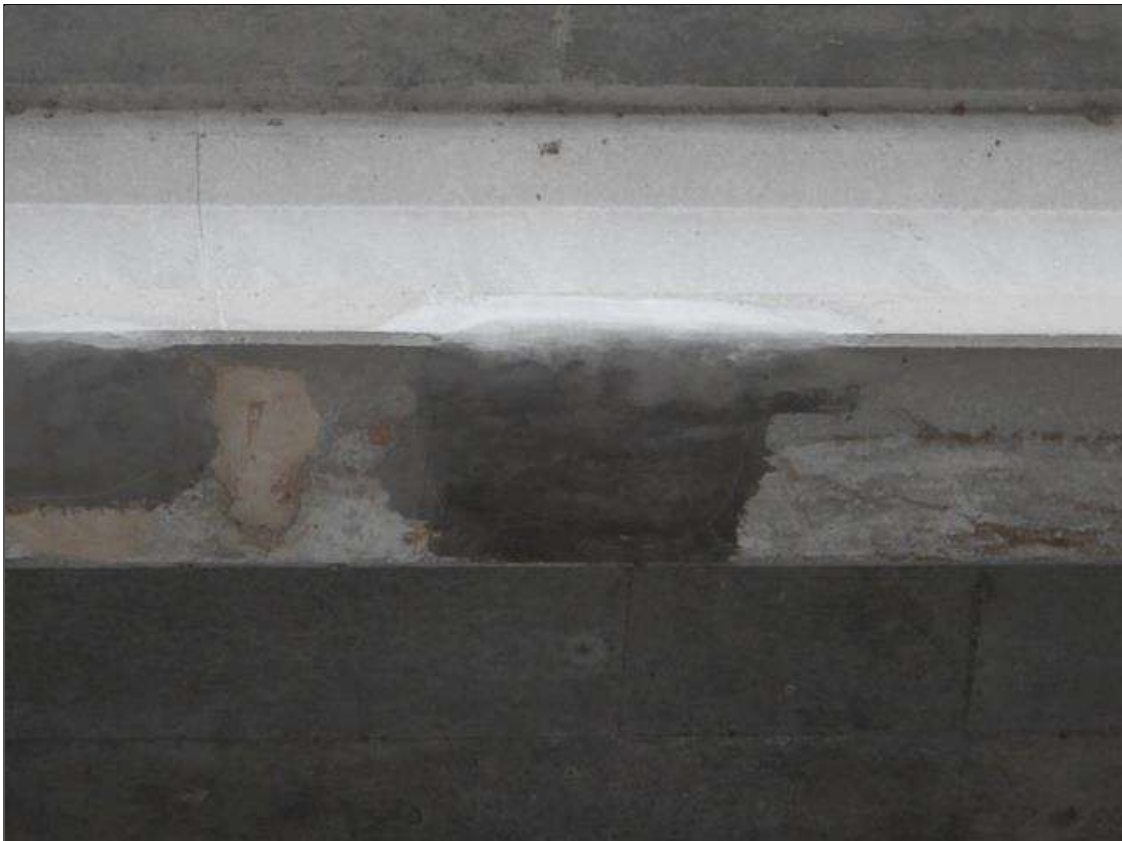
Span 9 Beam 9: [NEW REPAIR - PATCHING] FORMERLY --> PRIORITY MAINTENANCE - spall with exposed strands on the bottom face at 19ft from bent 8 (24" x 15" x 2"), (x3) strands exposed for (9") long
