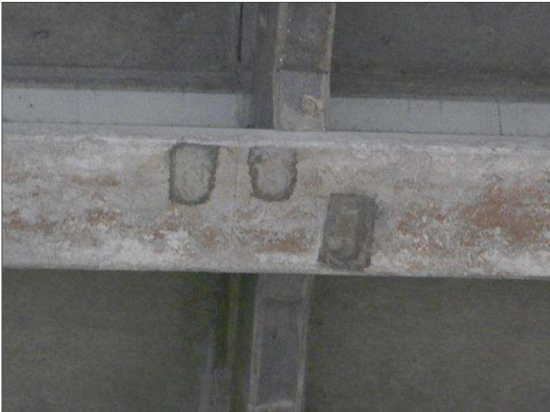
Span 10 Beam 7: [NEW REPAIR - PATCHING] FORMERLY --> (x2) spalls with exposed rebar on the bottom face at 22ft from bent 10 up to (7" x 4" x 1/2")
