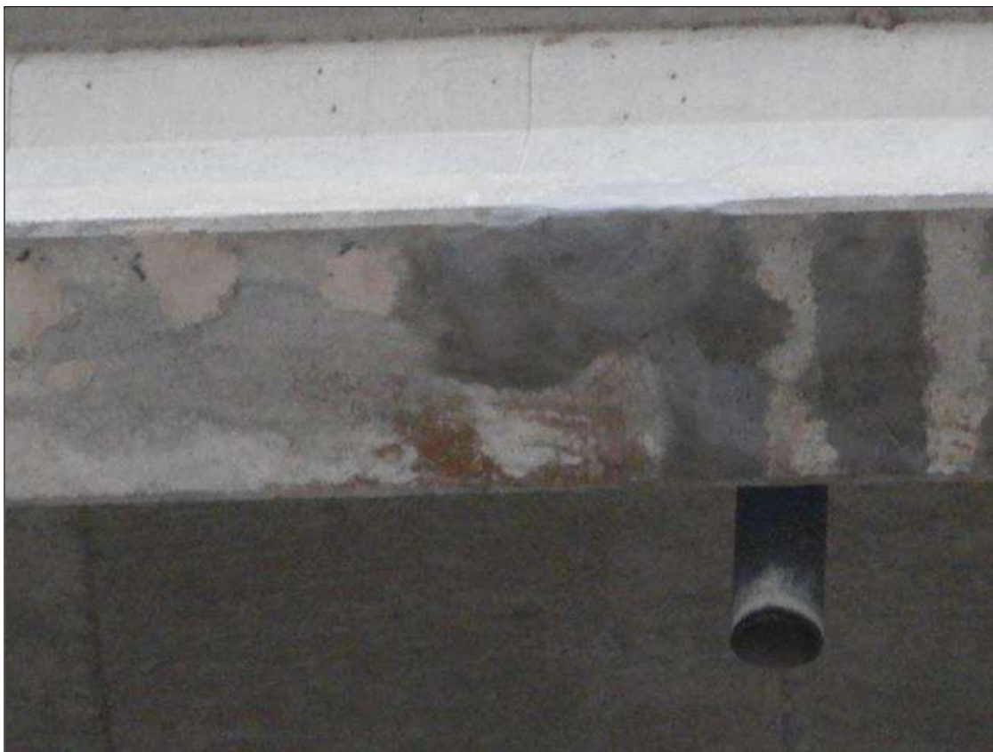
Span 10 Beam 9: [NEW REPAIR - PATCHING] FORMERLY --> PRIORITY MAINTENANCE - spall with exposed strand on the bottom face at 12ft from bent 9 (14" x 6" x 1") in a failed repair with area (18" x 9"), strand exposed for (5")
