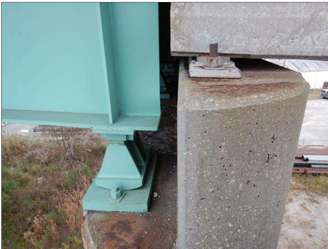
GIRDERS 1 BEARINGS AT BENT 11 [TYPICAL BEARINGS AT BENT 11]
