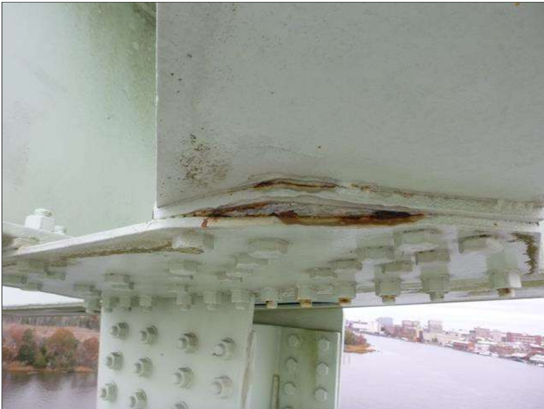
Span 18 Lift Span U2 NORTH: \frac{1}{2} " PACK RUST UNDER BOTTOM GUSSET PLATE CONNECTION TO DIAGONAL EAST SIDE OF U2, ALSO \frac{7}{32} " SECTION LOSS TO BOTTOM FLANGE OF BEAM.
