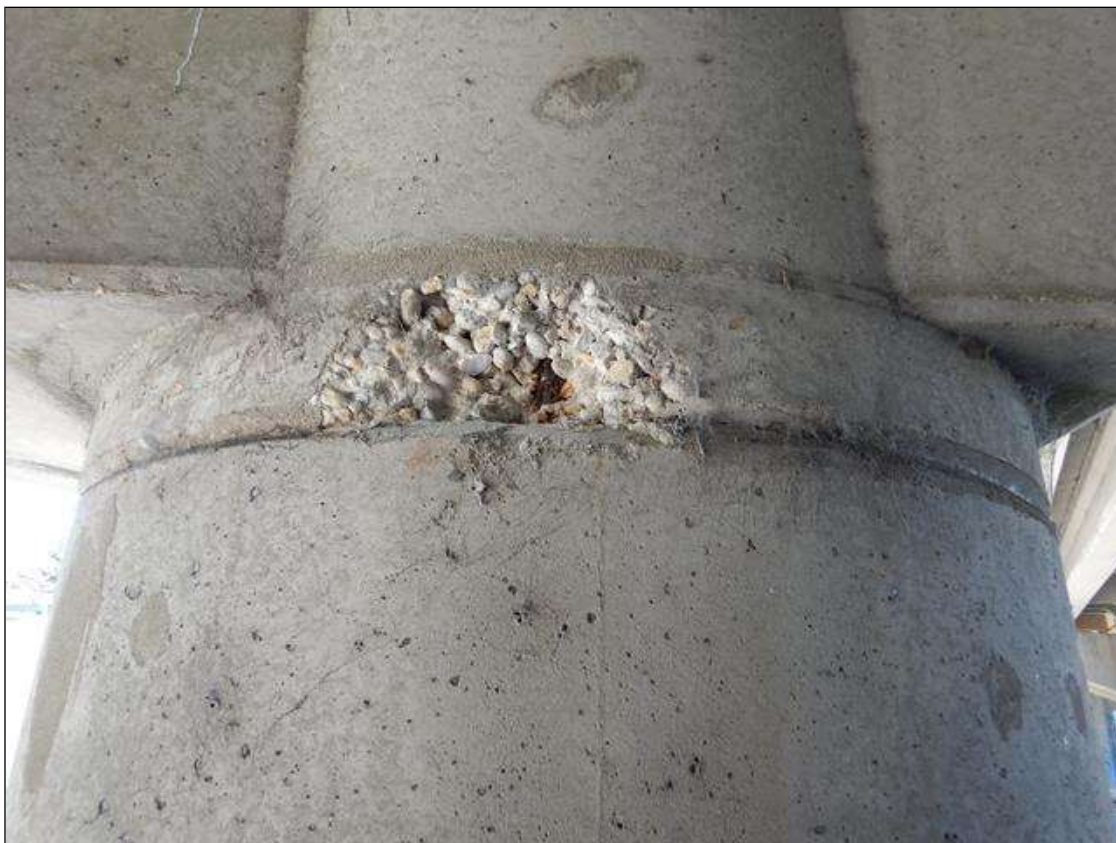
Bent 29 Pile 3: EAST FACE AT THE TOP, SPALLING WITH EXPOSED REBAR [APPROXIMATELY 1' LONG X 6" HIGH X UP TO 2" DEEP]; NO MEASURABLE SECTION LOSS
