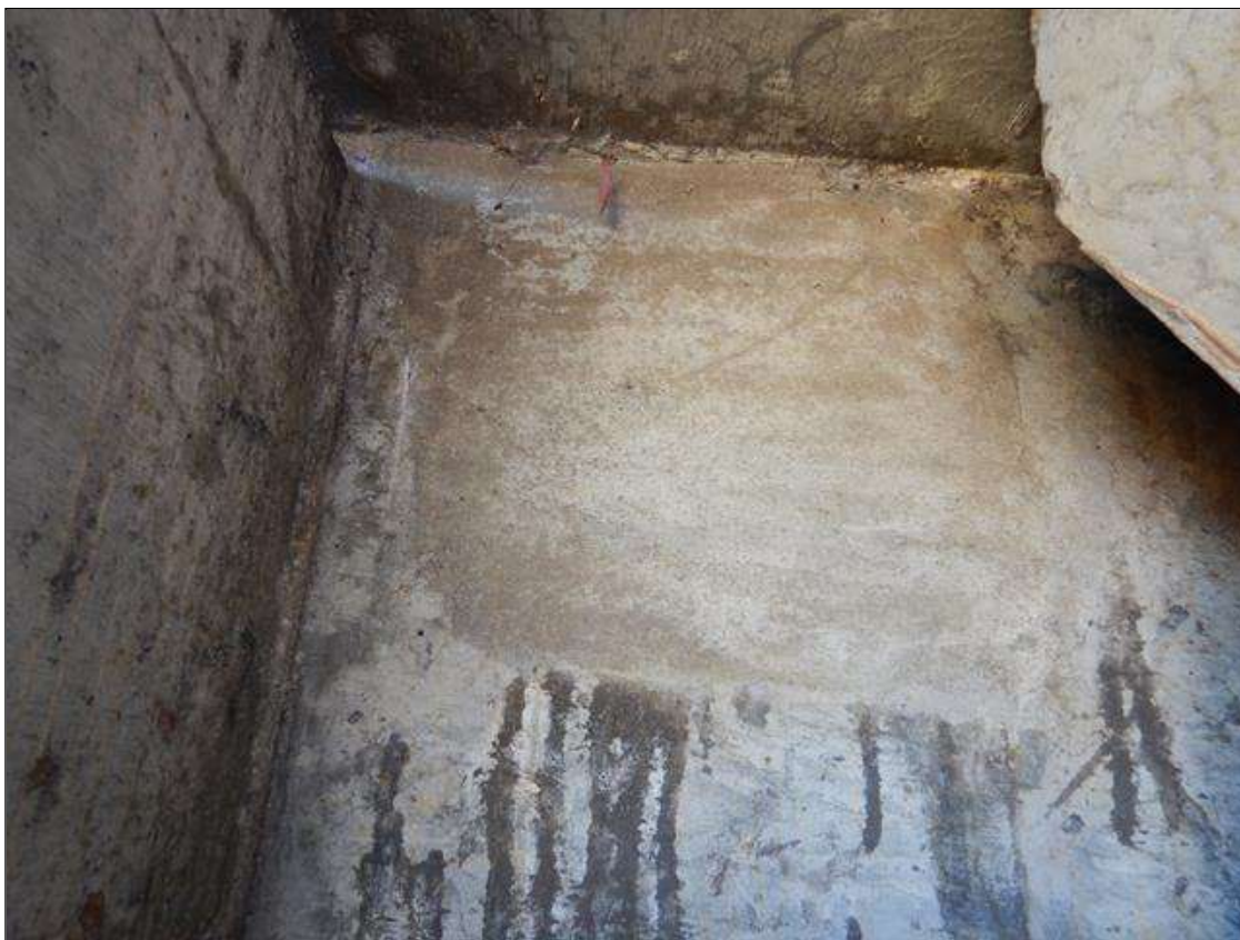
Ramp End Bent Abutment: [NEW REPAIR-PATCHING] FORMERLY --> spall with exposed rebar behind girder 1 (18" x 16" x 4")
