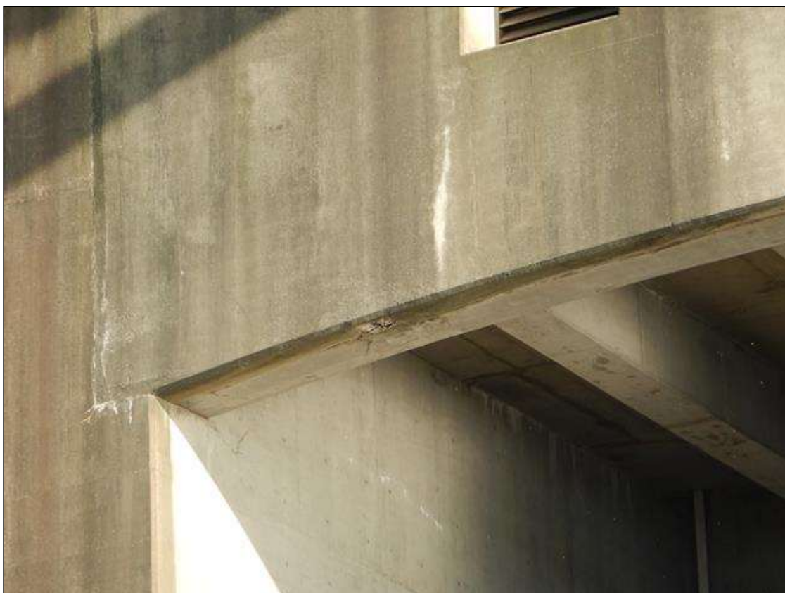
Bent 17 - Lift Span Bent Cap 1: DELAMINATION and spall with exposed rebar on the bottom face of the west arch (24" x 36" x 1 1/2")
