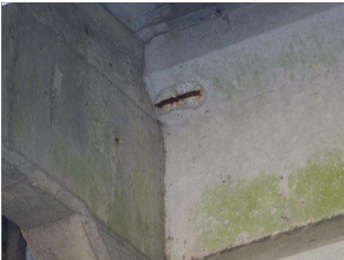
Span 28 Beam 1: [PROMPT ACTION REQUEST] spall with exposed rebar on the top right flange at bent 25 (7" x 3" x 1/2")
