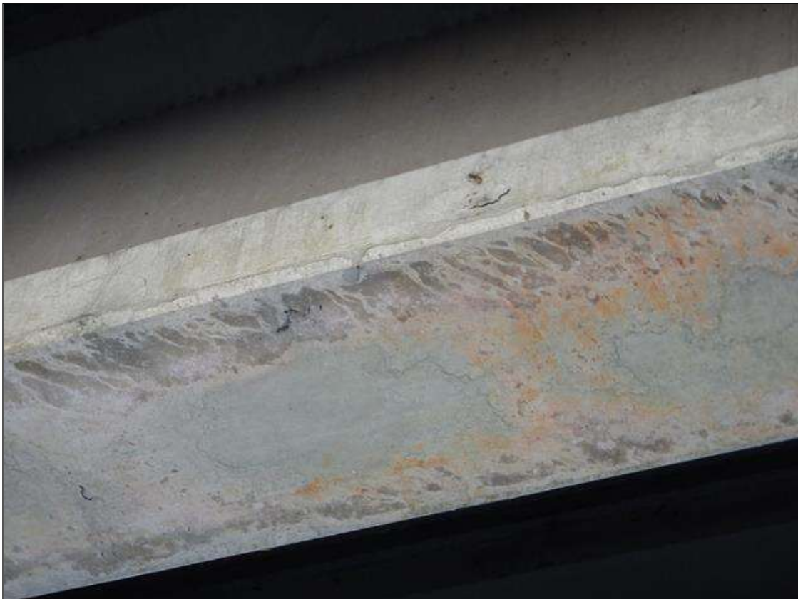
Span 31 Beam 4: [NEW REPAIR-PATCHING] FORMERLY --> (x2) DELAMINATION areas on the bottom right flange a 10ft from Bent 29 up to (6" x 3") (loose concrete over roadway)
