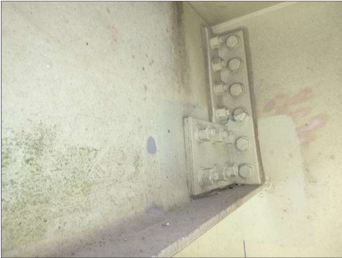
Span 18 Lift Span Stringer 12: BETWEEN FB's 7-8 - NEW REPAIR (2) 9.5" X 7" X 3/8" PLATES ON BOTH SIDES OF THE WEB AT FLOORBEAM 8, 2020 INSPECTION HAD - 5/8" HOLE IN WEB AT BOTTOM FLANGE AT FB 8 CONNECTION WIDE/ 8"HIGH x 3"WIDE PITTED AREA - CLEANED AND PAINTED - PROMPT ACTION REQUEST
