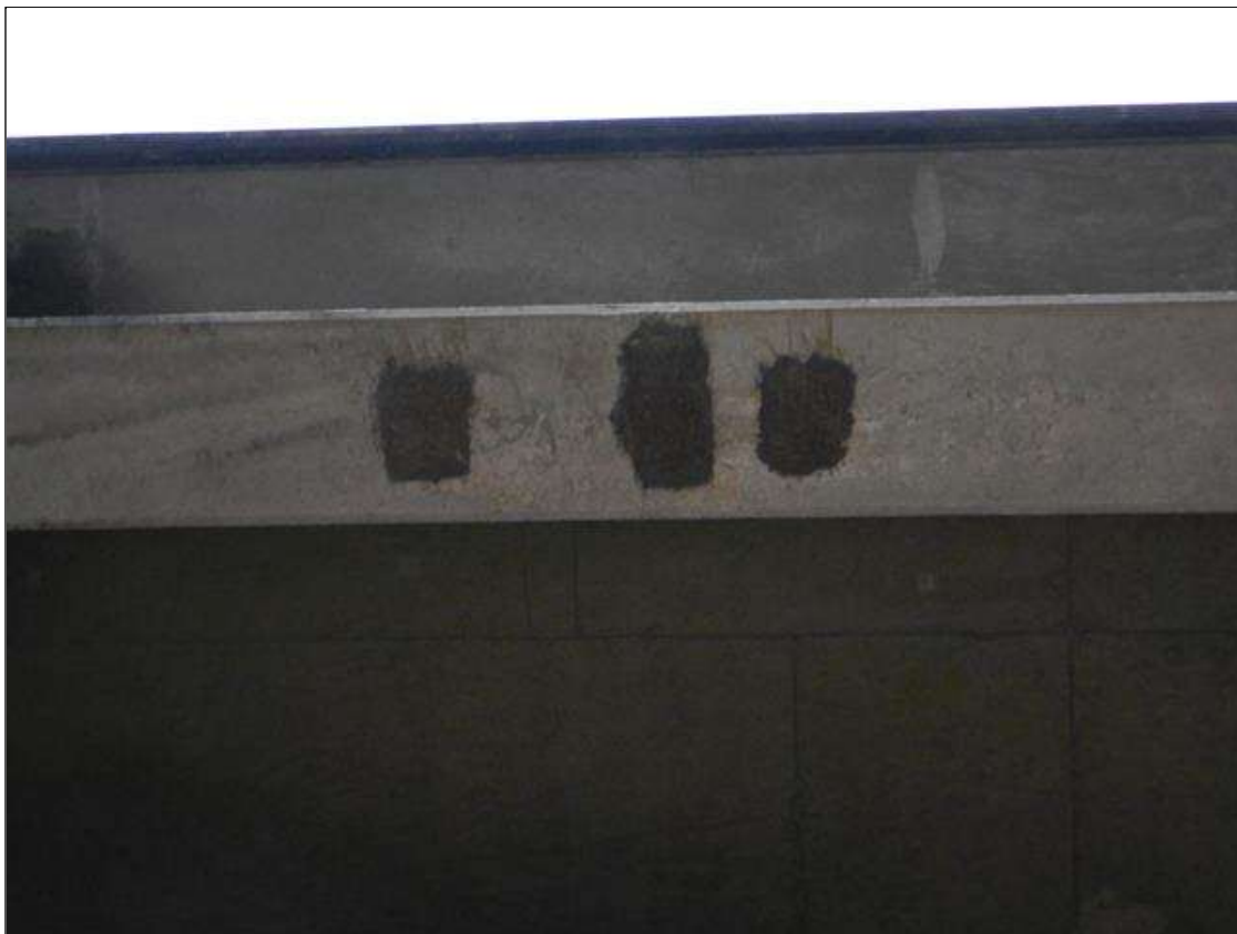
Span 9 Beam 1: [NEW REPAIR - PATCHING] FORMERLY --> (x2) spalls with exposed rebar on the bottom face at 7ft from bent 9 up to (11" x 9" x 1/2")
