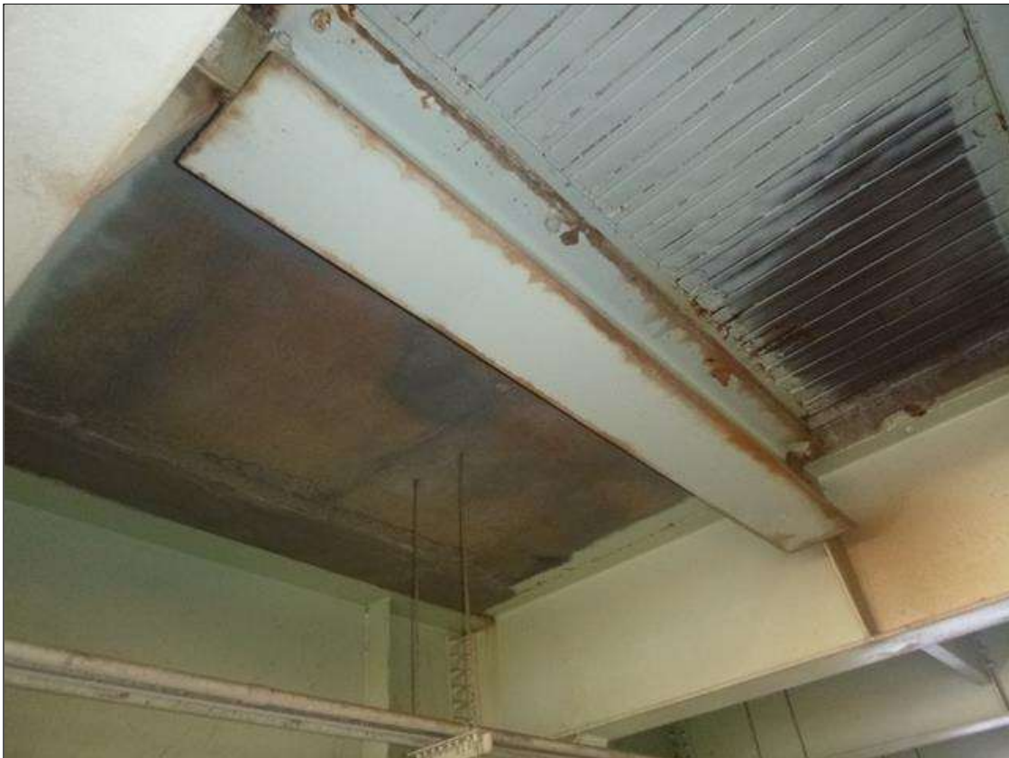
Span 19 Stringer 3: surface corrosion on the edges of the flanges between stringers which are between stringer 3 and
