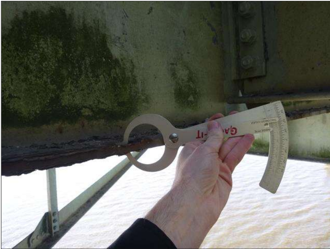
Span 18 Lift Span Stringer 2: (PAR) BETWEEN FB's 9-10 - SCATTERED ALONG THE FULL LENGTH BOTH SIDES OF BOTTOM FLANGE CORROSION WITH 1/4" AVERAGE REMAINING.
