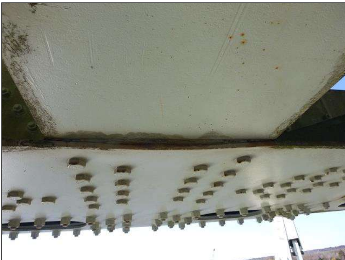
Span 18 Lift Span Floor Beam 2: BOTTOM LATERAL GUSSET AT L2 SOUTH - UP TO 1/2" PACK RUST BETWEEN GUSSET PLATE AND BOTTOM FLANGE.
