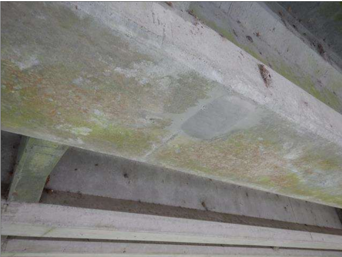
Span 3 Beam 2: [NEW REPAIR - PATCHING] FORMERLY --> area of delamination on the bottom of the girder at 1/3 point, 10" wide x 5" long with 1/8" separation.
