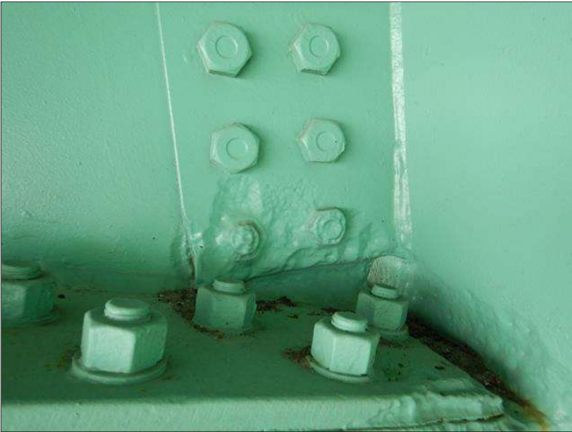
Span 16 Beam 1: PRIORITY MAINTENANCE - Bracket 2 at WB Parking Area both faces: section loss on the bottom flange/plate of the brace beam at the web (7" x 1 3/4") with (11/16") remaining; up to 75% section loss on (x1) nut on the bottom plate on the east face and up to 100% section loss on (x2) nuts on the west face; up to 100% section loss on (x2) nuts on the web plate on the west face; section loss in the web (9" x 4") by up to (1/16") into the web on both sides of the bracket (PROMPT ACTION REQUEST)
