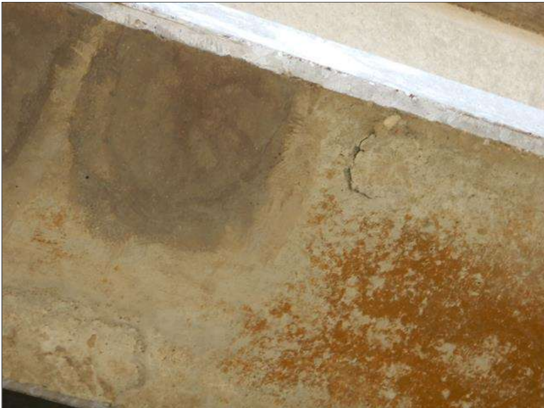
Span 34 - Ramp Span Beam 1: [NEW REPAIR-PATCHING] FORMERLY --> (x9) spalls with exposed rebar on the bottom face starting 16ft from Bent 30 up to (16" x 7" x 2")
