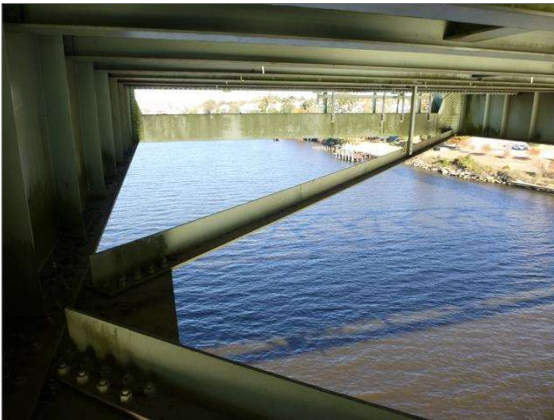
FLOOR BEAM LATERAL BRACING
