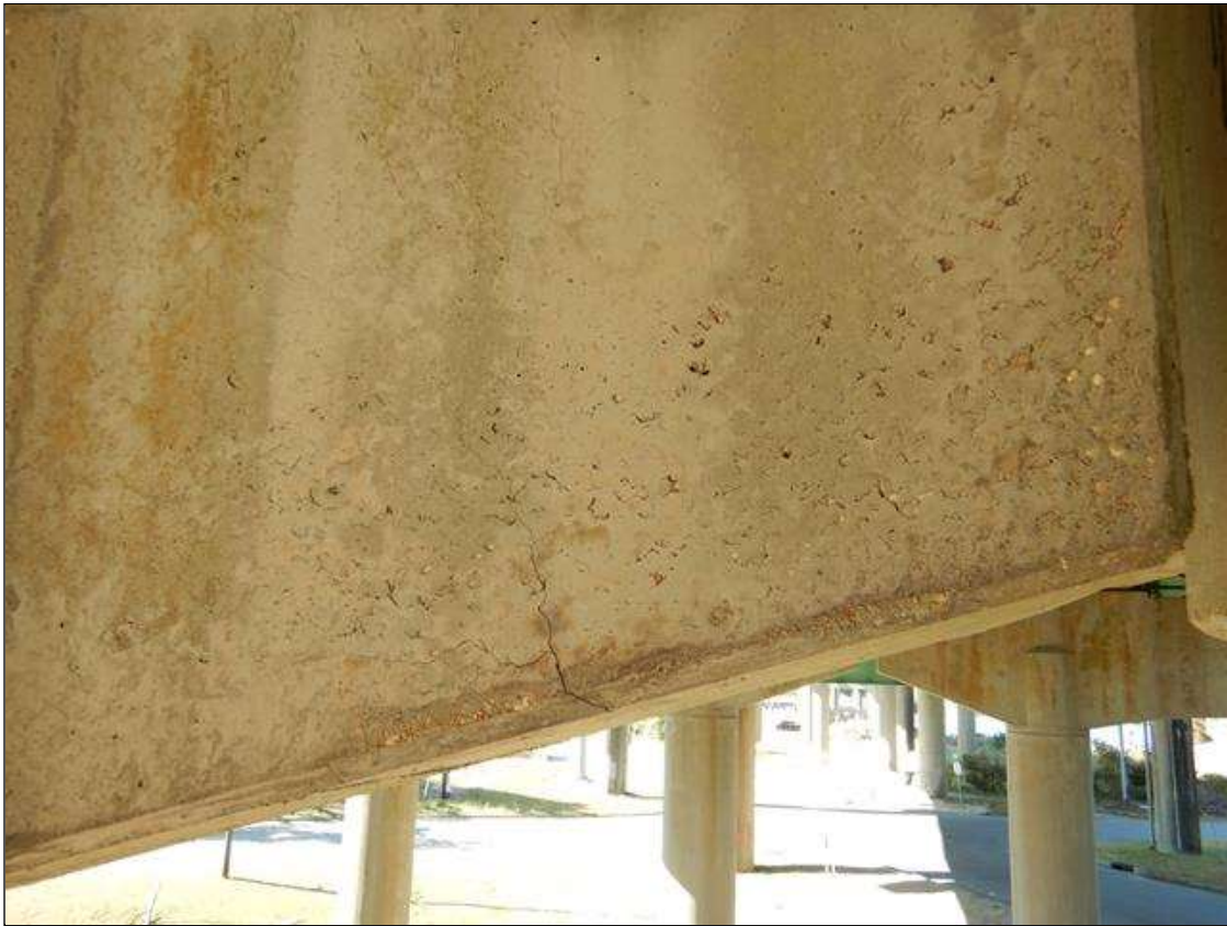
Bent 25 Cap 2: area of DELAMINATION (30" x 20") and cracking up to (1/16") wide on the west face left of column 3
