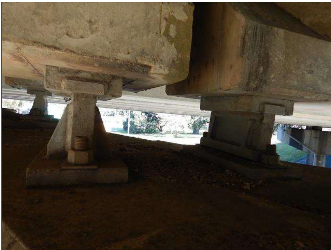
AT BENT 28, SPAN 30 GIRDER 10 FAR BEARING AND SPAN 31 GIRDER 11 NEAR BEARING [TYPICAL BEARINGS AT BENT 28, BENT 29, BENT 27, AND BENT 26 SPAN 29 SIDE]
