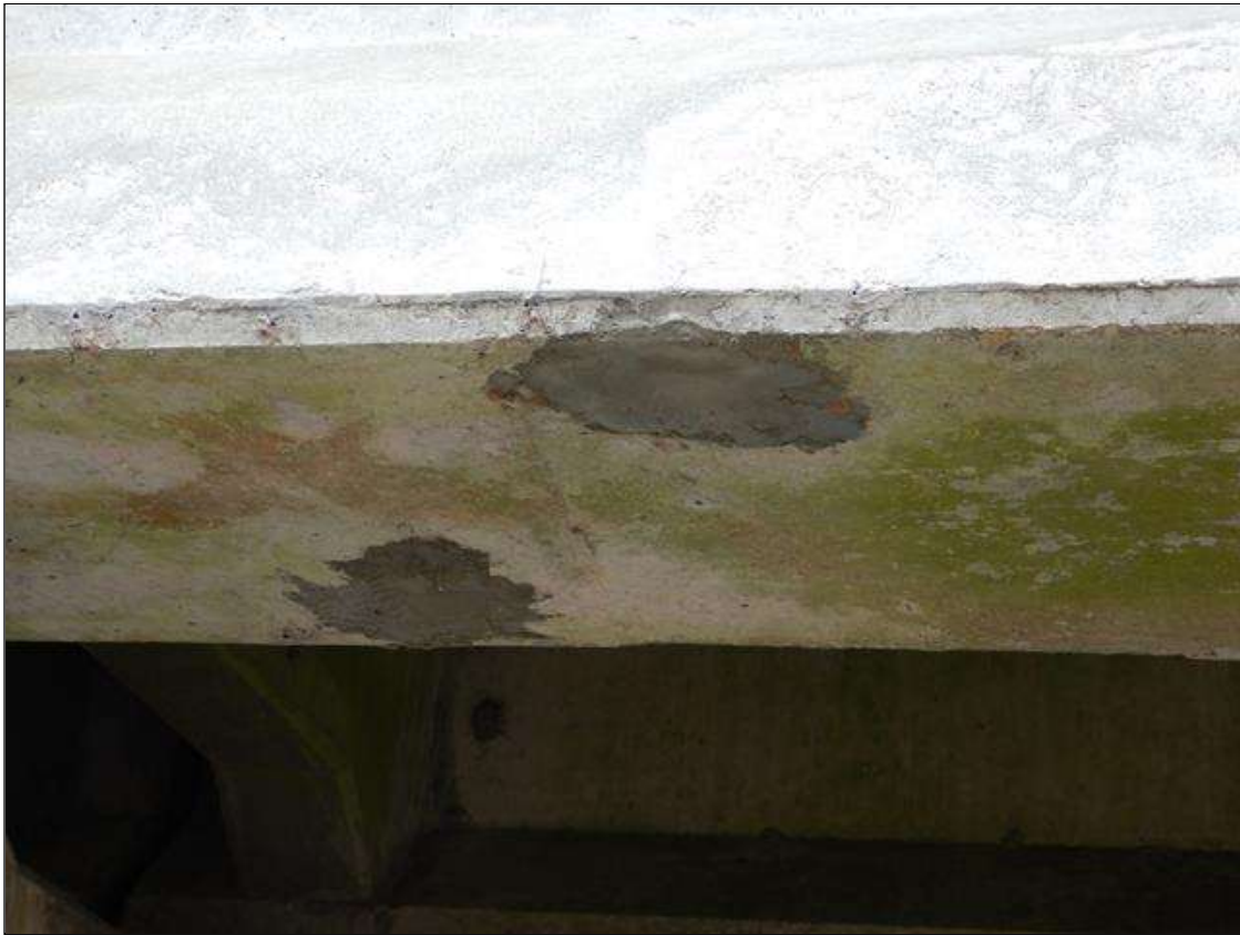
Span 2 Beam 1: [NEW REPAIR - PATCHING] FORMERLY --> PRIORITY MAINTENANCE - (x2) spalls with exposed strands at 18in and 30in from bent 2 on the bottom face (7" x 4" x 1 1/2") and (6" x 5" x 1 1/2") respectively, (x1) strand exposed at each location for (1") long (PROMPT ACTION REQUEST)
