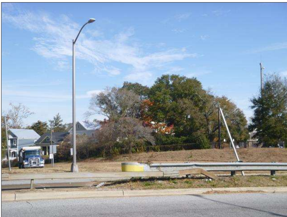
THE MEDIAN RAIL AT THE EAST APPROACH TRANSITIONS TO GUARDRAIL AT AN UNPAVED ISLAND
