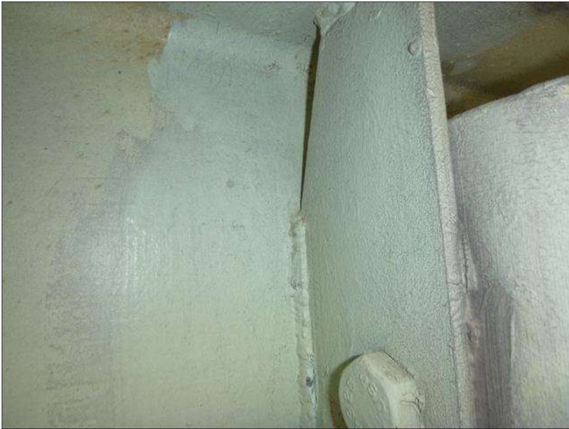
Span 18 Lift Span Stringer 10: REPAIR OBSERVED IN 2021 INSP: CRACK NOT VISIBLE AREA HAS BEEN PAINTED OVER. 2020 REPORT BETWEEN FB's 5-6 - 1" LONG CRACK IN WEB ACROSS TOP OF WELD AT DIAPHRAGM CONNECTION
