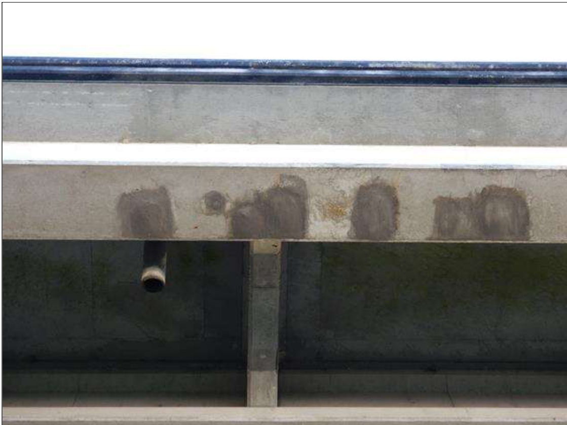
Span 28 Beam 1: [NEW REPAIR-PATCHING] FORMERLY --> (x5) spalls with with exposed rebar on the bottom face a 18.5ft from bent 26 up to (6" x 6" x 1/2")
