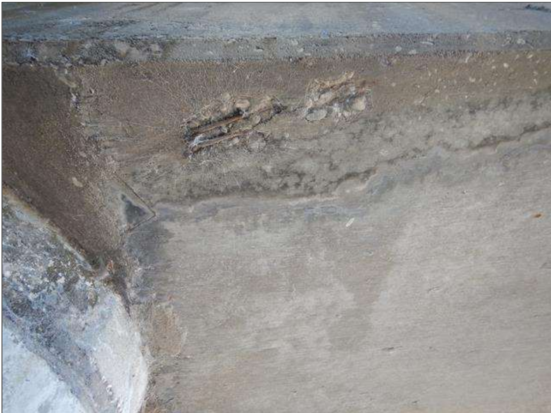
Bent 31 - Ramp Bent Cap 1: spall with no exposed rebar on the bottom face between the columns (10" x 3" x 1/4")
