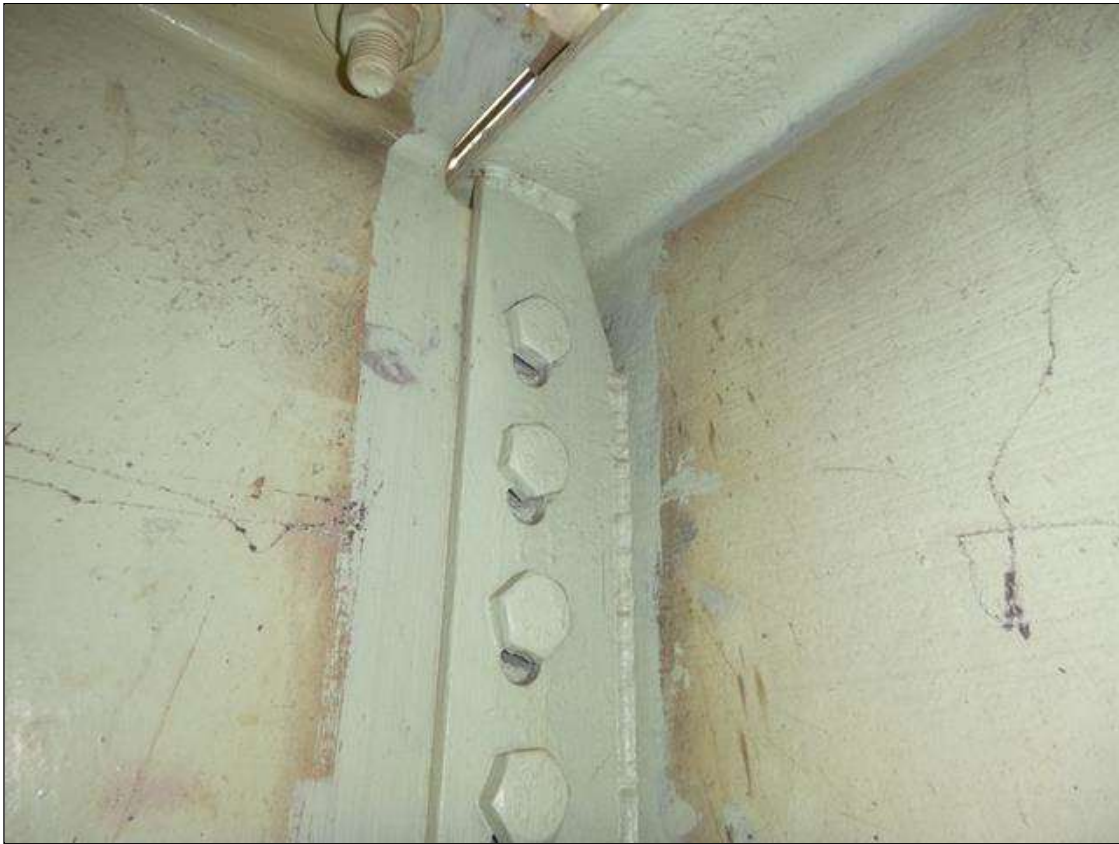
Span 18 Lift Span Stringer 8: REPAIR OBSERVED IN 2020 INSP: CRACK NOT VISIBLE, AREA HAS BEEN PAINTED OVER. 2018 REPORT HAD BETWEEN FB's 3-4 - 1/2" LONG CRACK IN WEB ACROSS TOP OF WELD AT DIAPHRAGM CONNECTION ON NORTH SIDE.
