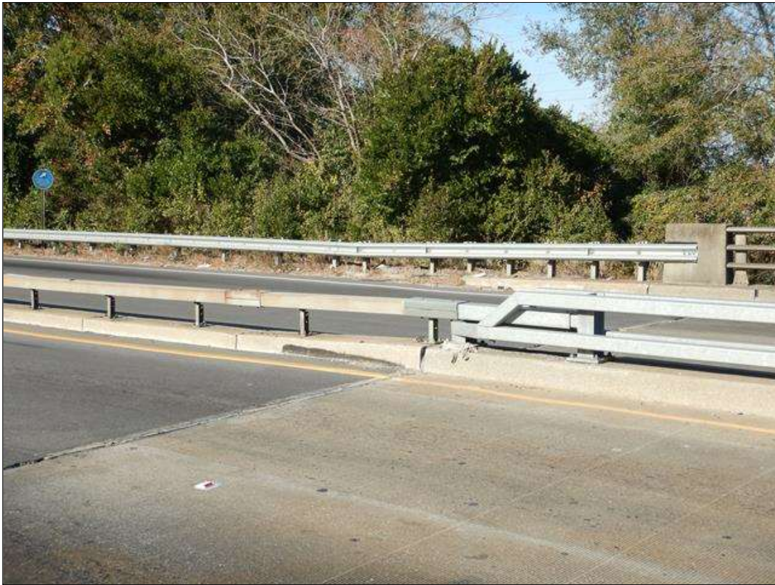
WEST APPROACH MEDIAN RAIL TRANSITION
