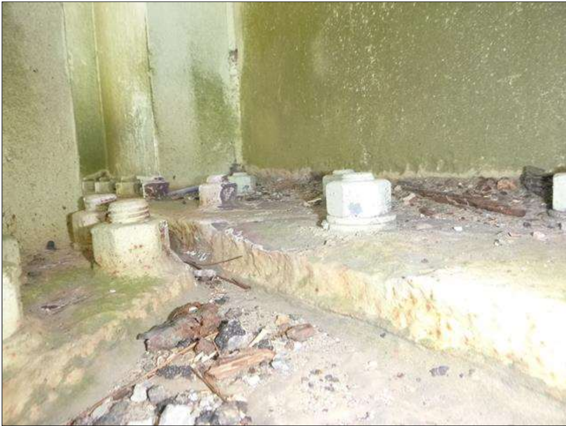
Span 18 Lift Span Floor Beam 7: SPAN 18 CENTER BOTTOM LATERAL GUSSET AT FB 7: PITTED AREA ON TOP AT THE NORTHEAST CORNER, 7" X 7" X 1/4" DEEP, CLEANED AND PAINTED.
