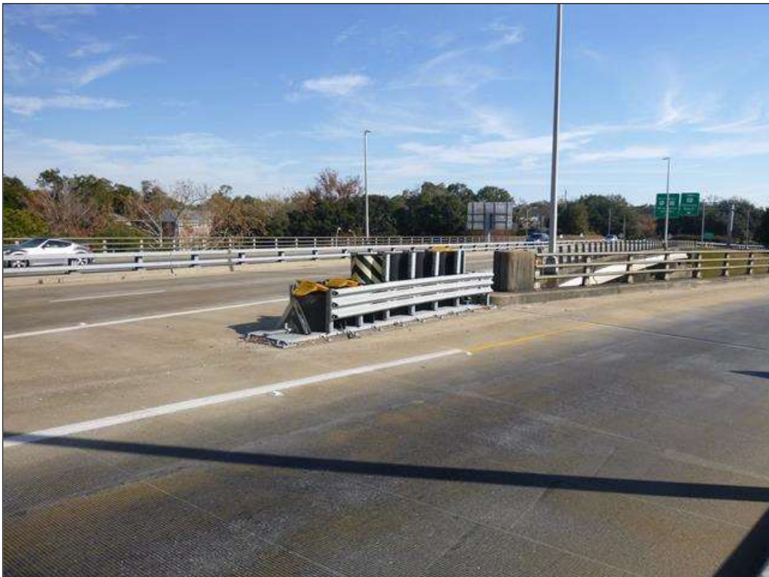
AT THE RAMP EXIT FROM THE DECK, IMPACT ATTENUATOR
