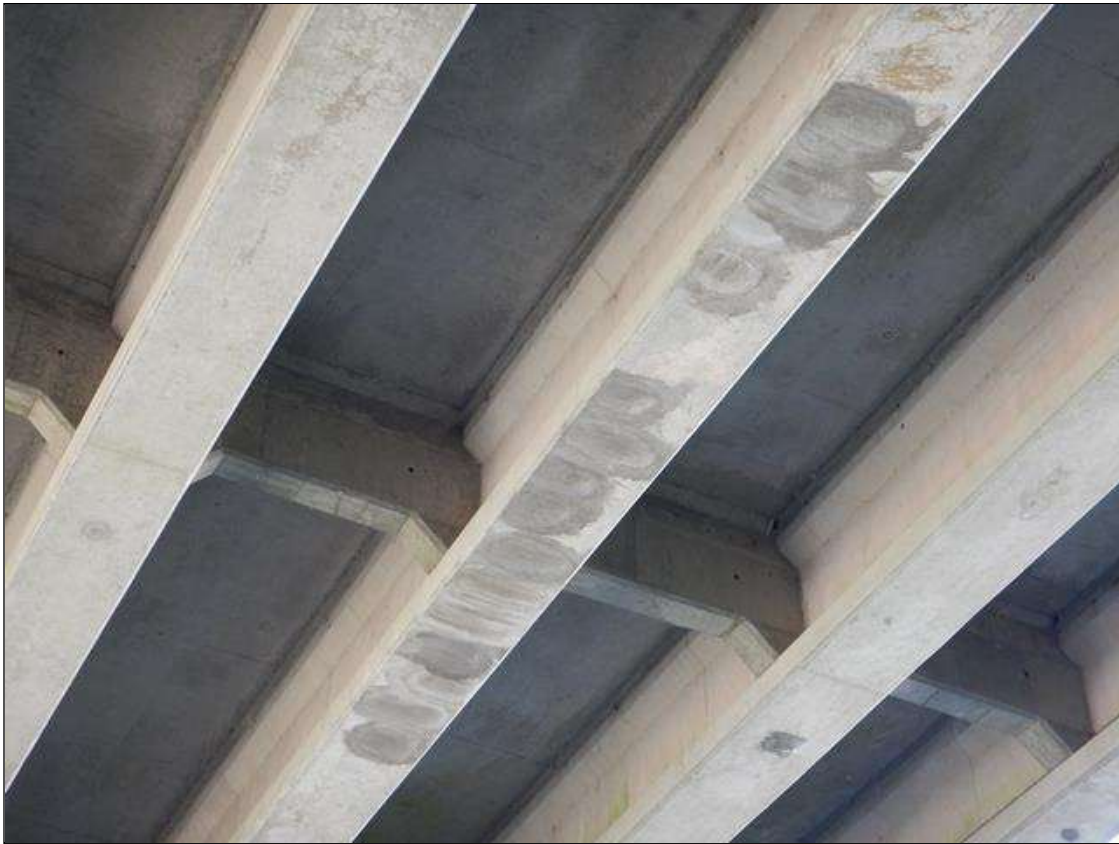
Span 28 Beam 3: REPAIR observed in 2020 insp: 15 sound patches up to 18" wide x 12" long. 2018 report had (x10) spalls with exposed rebar at mid span on the bottom face up to (14" x 6" x 1/2")
