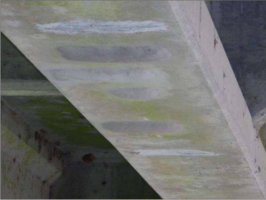
Span 3 Beam 2: [NEW REPAIR - PATCHING] FORMERLY --> (x4) spalls with exposed rebar on the bottom face starting at 24ft from bent 2 up to (8" x 3" x 1/2")
