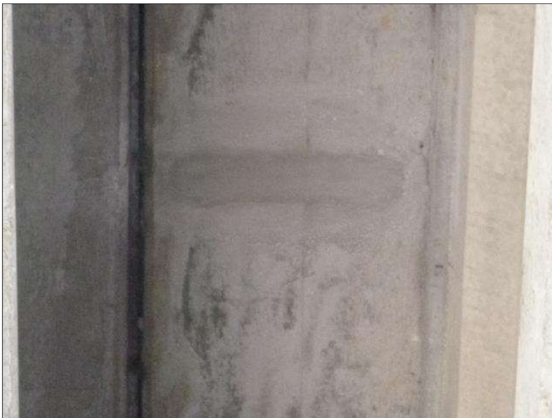
Span 31 Deck: [NEW REPAIR - PATCHING] FORMERLY --> spill with exposed rebar on the deck bottom in bay 7 at 2ft from Bent 28 (18" x 5" x 1/2")
