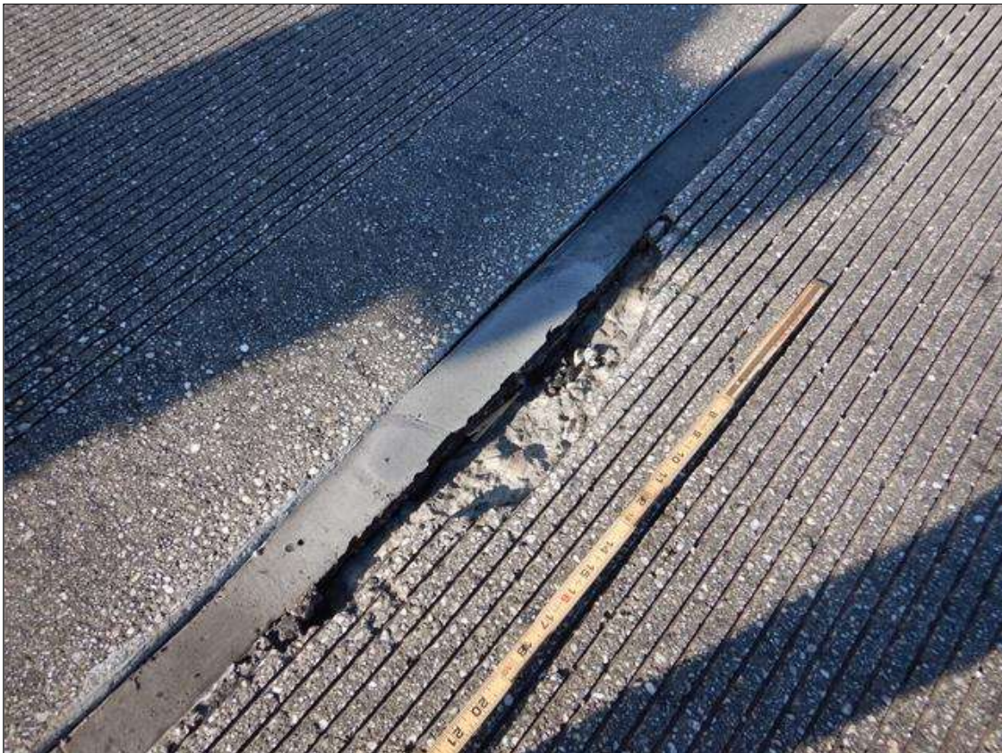
Span 7 Deck: [PROMPT ACTION REQUEST] RIGHT LANES AT BENT 6, SPALL (24" LONG x 4" WIDE x 1.5" DEEP AT 10' FROM RIGHT CURB)
