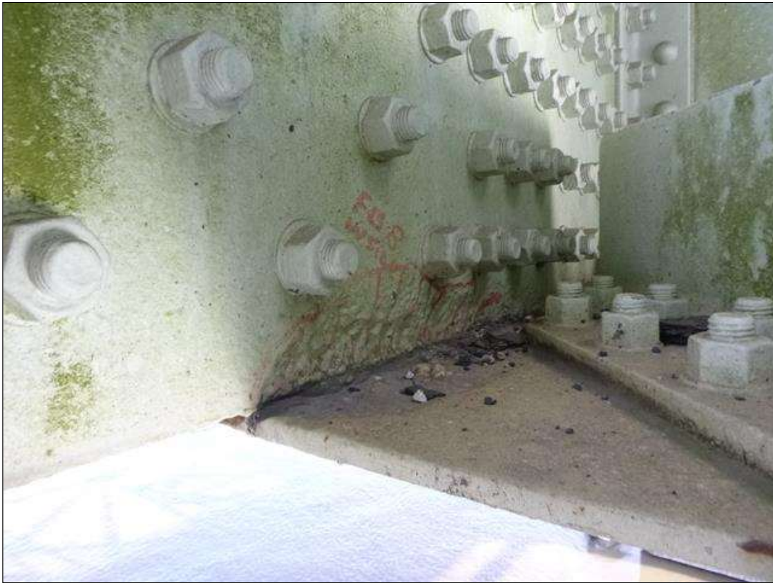
Span 18 Lift Span L8 NORTH: SOUTH PLATE, SOUTH FACE - 3" HIGH x 18" LONG PITTED AREA UP TO 1/4" DEEP ALONG BOTTOM ON WEST SIDE - CLEANED AND PAINTED
