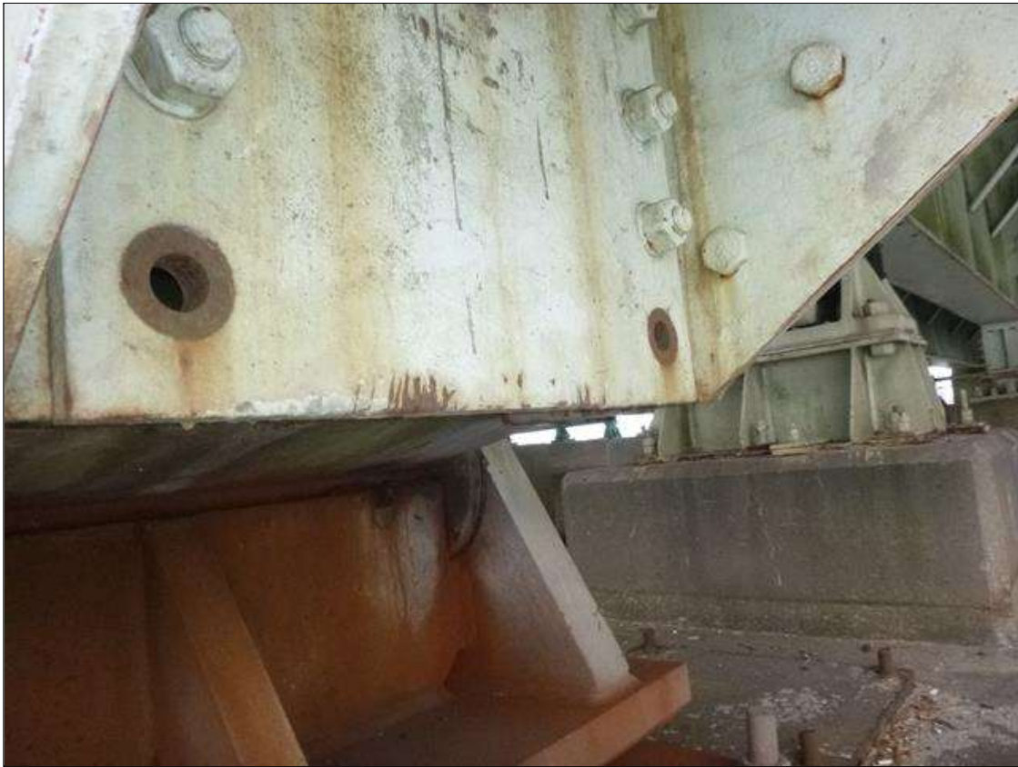
Span 18 Lift Span Truss Panel 2 - L0U0 SOUTH: (2) MISSING BOLTS AT BOTTOM OF EAST GUSSET AT BEARING (PAR)
