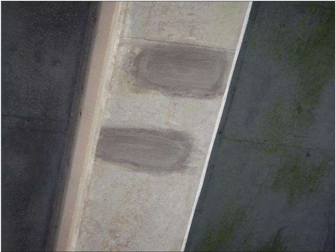
Span 29 Beam 2: [NEW REPAIR-PATCHING] FORMERLY --> spall with exposed rebar and unsound patch on the bottom face at 18ft and 20ft from Bent 27 (7" x 5" x 1/2") spall and (10" x 5") patch
