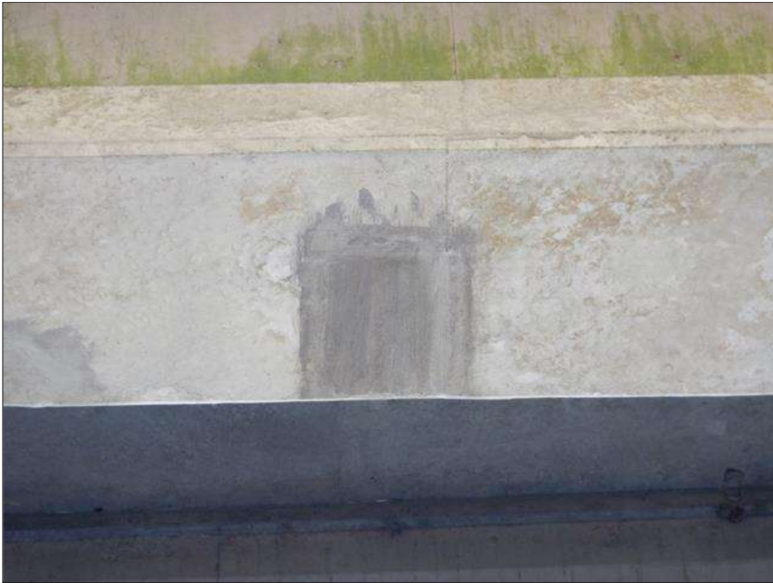
Span 30 Beam 2: [NEW REPAIR-PATCHING] FORMERLY --> spall with exposed rebar on the bottom left face at 16ft from bent 27 (7" x 2" x 1 1/2")
