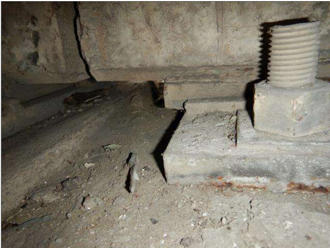
Span 1 Beam 9 - Beam 9 Far Bearing: up to (1 3/8") movement of bearing to east beyond masonry plate with 23% loss of bearing
