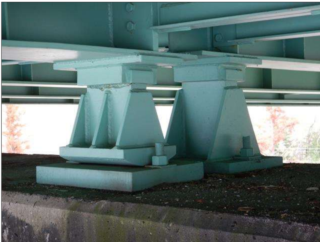
GIRDERS 5 BEARINGS AT BENT 12 [TYPICAL BEARINGS AT BENT 12]
