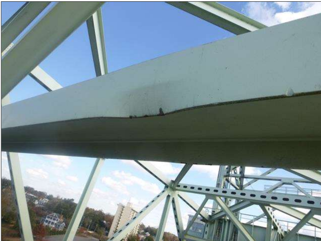
Span 18 Lift Span LB9: IMPACT DAMAGE 22" WIDE X 1-1/2" DEFORMATION ON WEST BOTTOM FLANGE OVER RIGHT EAST BOUND LANE.
