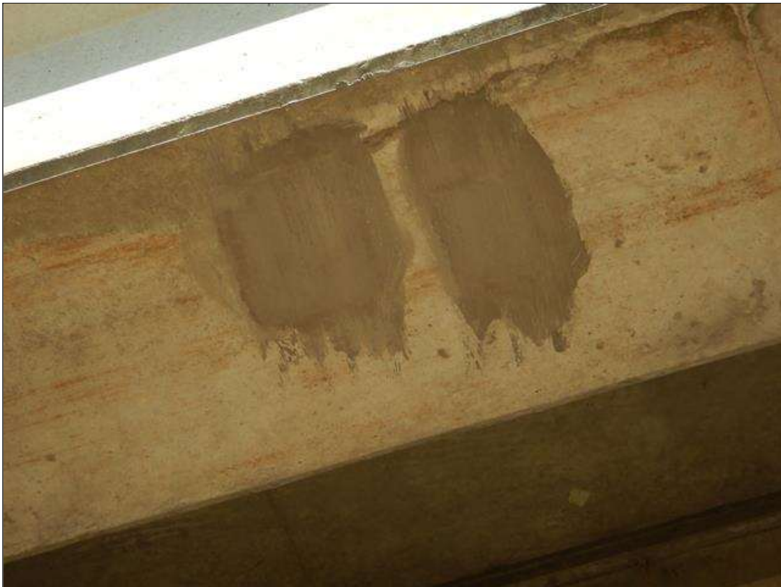
Span 31 Beam 12: [NEW REPAIR-PATCHING] FORMERLY --> spall with exposed rebar over the southbound bike lane (1 1/2" x 2" x 1/2")
