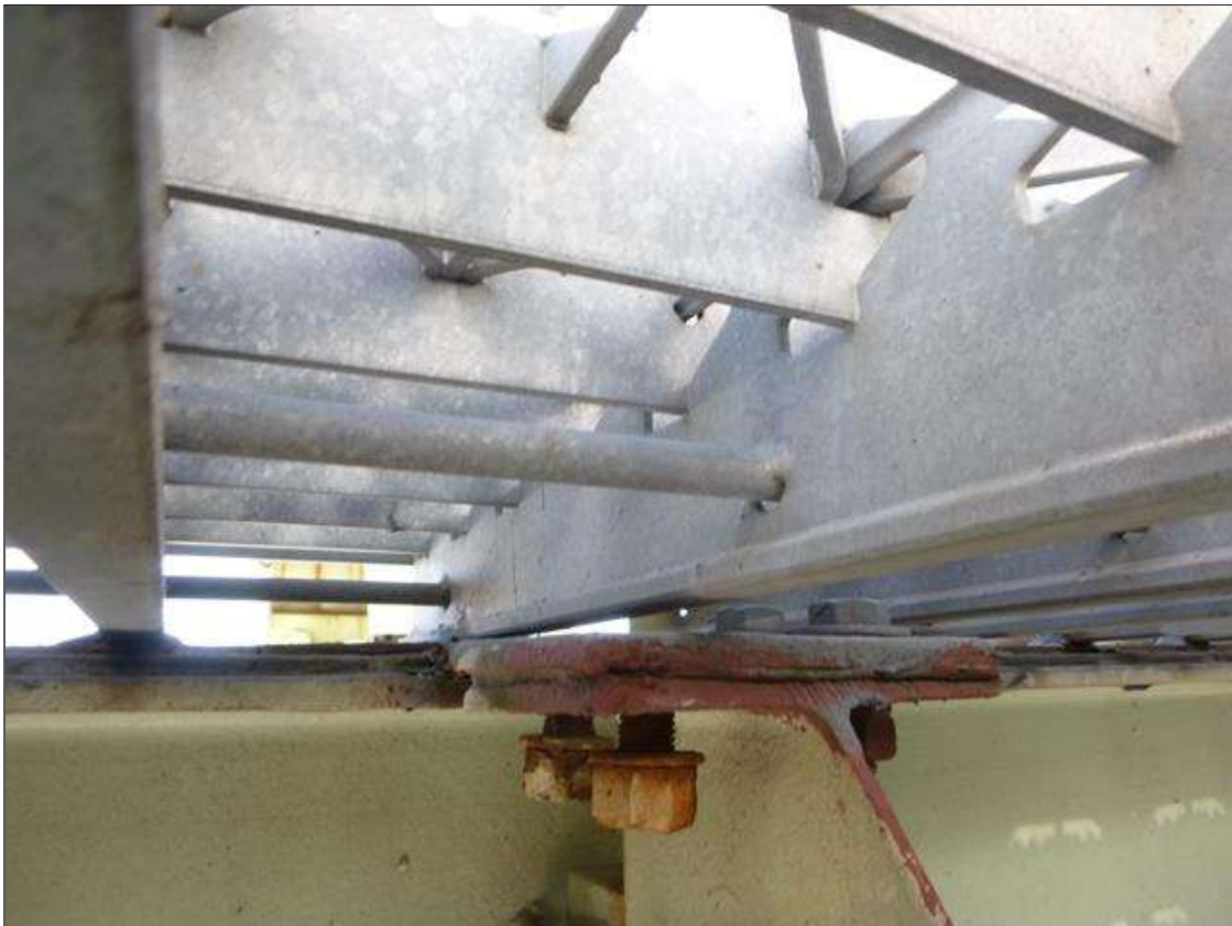
Span 18 Lift Span Stringer 14: (PAR) BETWEEN FB's 4-5 THIRD DIAPHRAGM LOOSE BOLTS WITH MISSING HEADS ON CONNECTOR PLATE.
