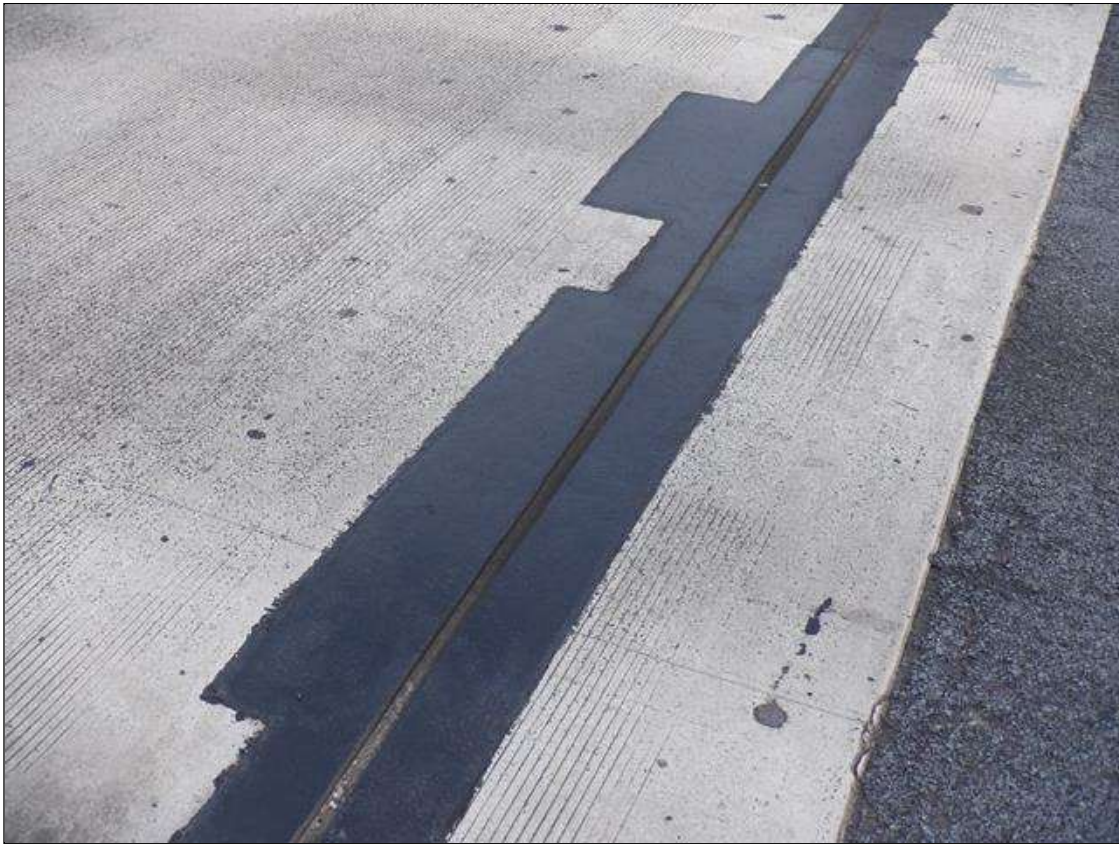
Span 4 Expansion Joint at End Bent 2: 2- UP TO 7 FEET X 18 INCHES PATCHED AREAS ALONG SOUTH EDGE IN EAST LANE.
