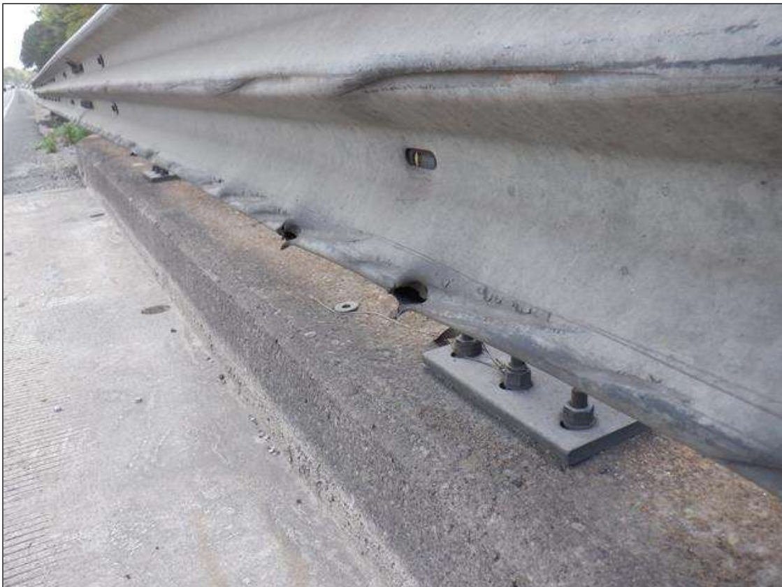
Span 4 Right Metal Rail: (PAR) 51 FEET OF IMPACT DAMAGE WITH 5- UP TO 3 INCHES X 1 INCHES GOUGES.
