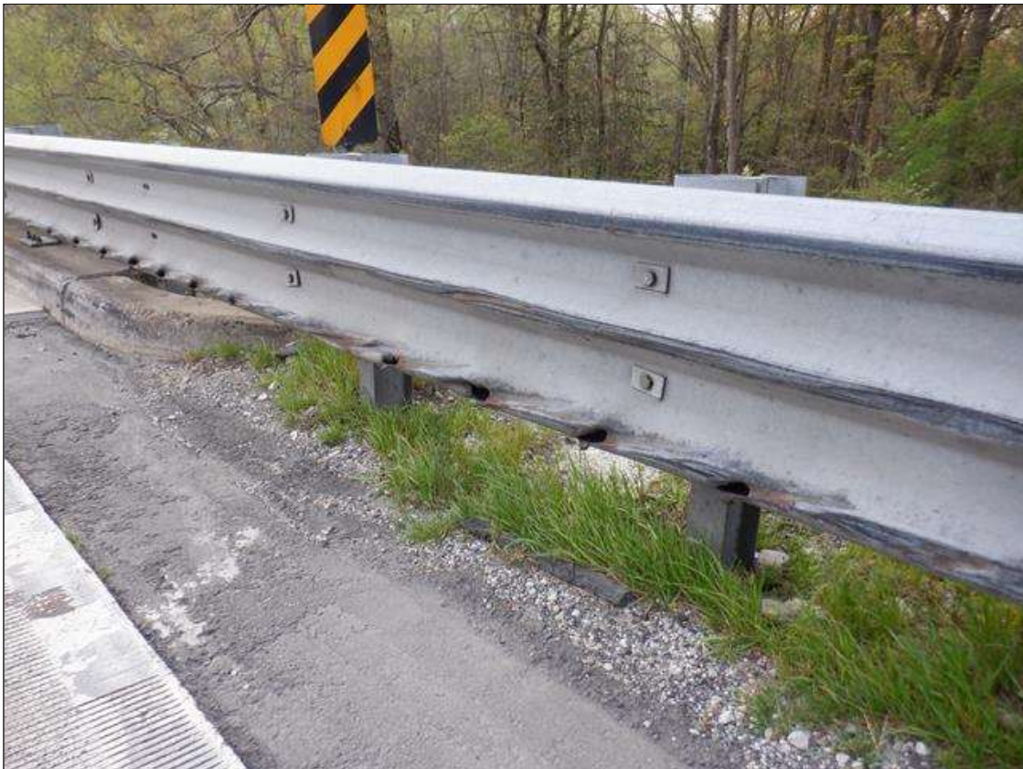
General Comments and Misc. Items: (PAR) 15 FEET OF IMPACT DAMAGE WITH 11- UP TO 4 INCHES X 2 INCHES GOUGES IN SOUTHEAST GUARDRAIL AT END BENT 1.
