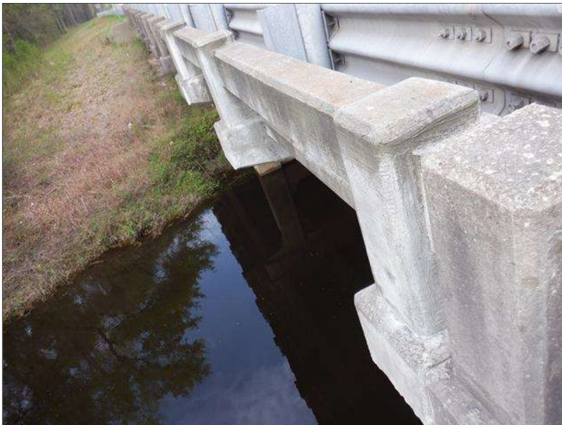
Span 2 Right Concrete Rail: 16 FEET OF REPAIRED SECTION OF CONCRETE RAIL AT BENT 2.
