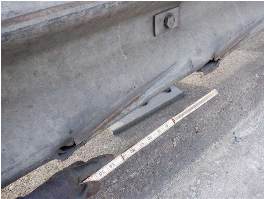
Span 3 Right Metal Rail: (PAR) 50 FEET OF IMPACT DAMAGE WITH 8- UP TO 4 INCHES X 1.5 INCHES GOUGES.
