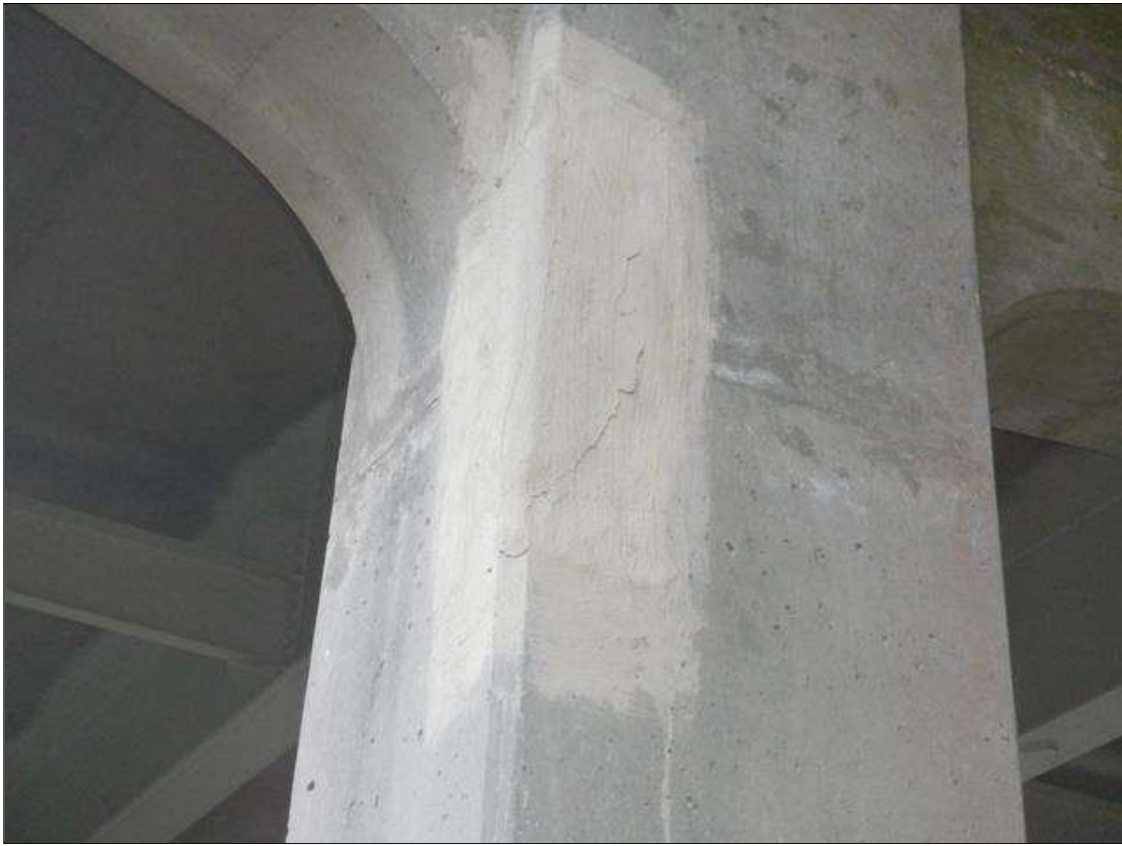
Bent 3 Pile 1: 24 INCHES X UP TO 7 INCHES X 4 INCHES CRACKED AND DELAMINATED PATCHED AREA WITH UP TO 1/16 INCHES CRACKING IN SOUTH FACE, 2 FEET FROM BOTTOM OF CAP.
