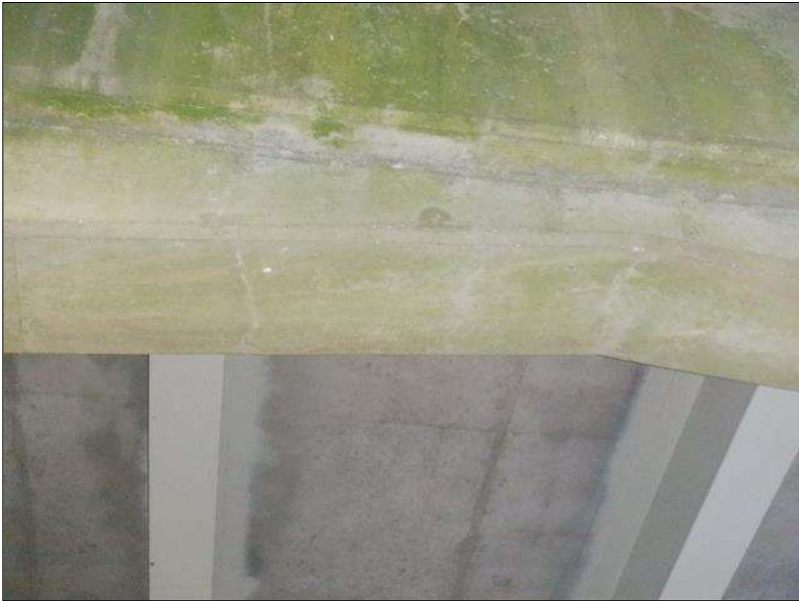
Bent 2 Cap 1: (3) UP TO 20 INCHES X 1/64 INCHES TRANSVERSE CRACKS, SOME WITH EFFLORESCENCE, ON BOTTOM OF CORBEL BETWEEN COLUMNS 1 AND 2.
