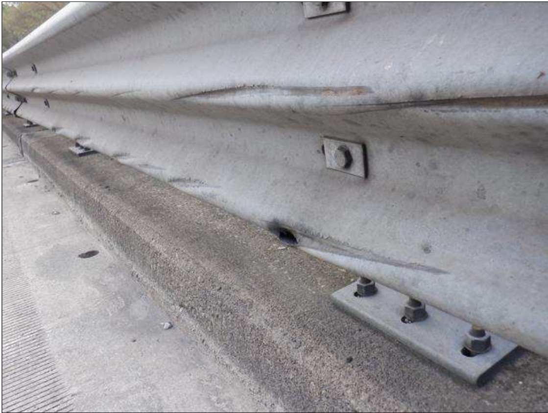
Span 1 Right Metal Rail: (PAR) 52 FEET OF IMPACT DAMAGE WITH SCRAPES AND 4- UP TO 3 INCHES X 1.5 INCHES GOUGES.
