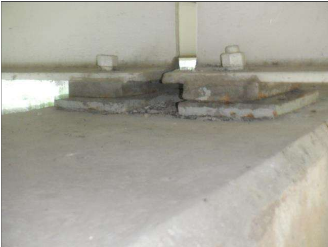
BEAM 3 BEARING ASSEMBLIES OVER BENT 3 (OTHERS SIMILAR)
