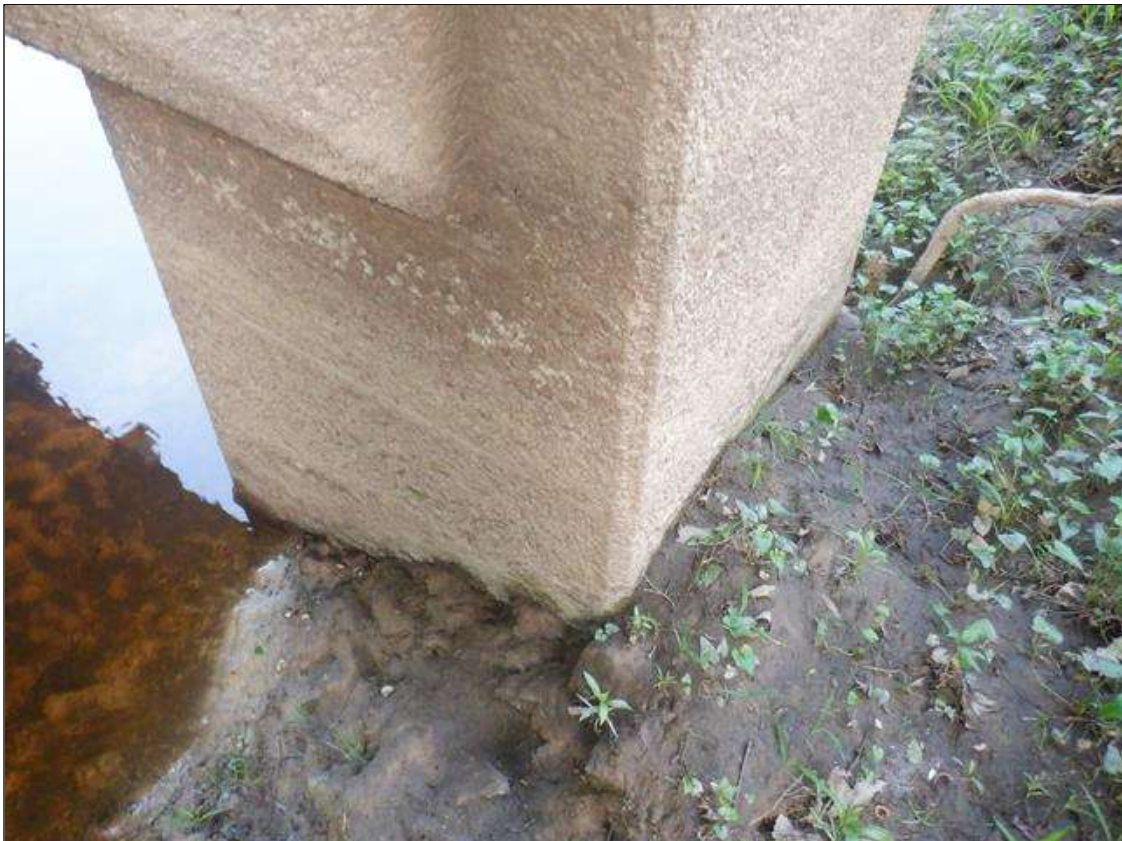
Bent 2 Pile 1: 4 FEET ABRASION/WEAR WITH EXPOSED COARSE AGGREGATE, 12 FEET FROM BOTTOM OF CAP.
