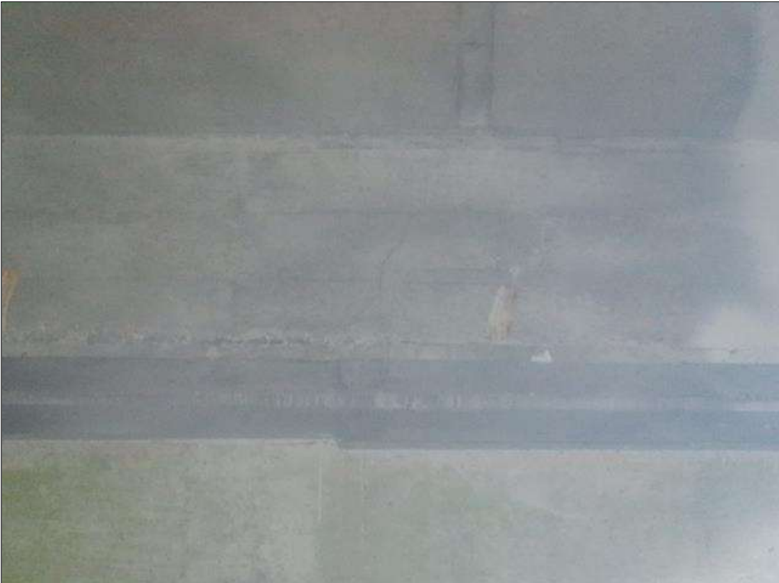
Span 4 Deck: 5- FULL HEIGHT X UP TO 1/32 INCHES VERTICAL CRACKS IN BENT 3 BAY 1 DIAPHRAGM. (BAYS 2 AND 3 SIMILAR)
