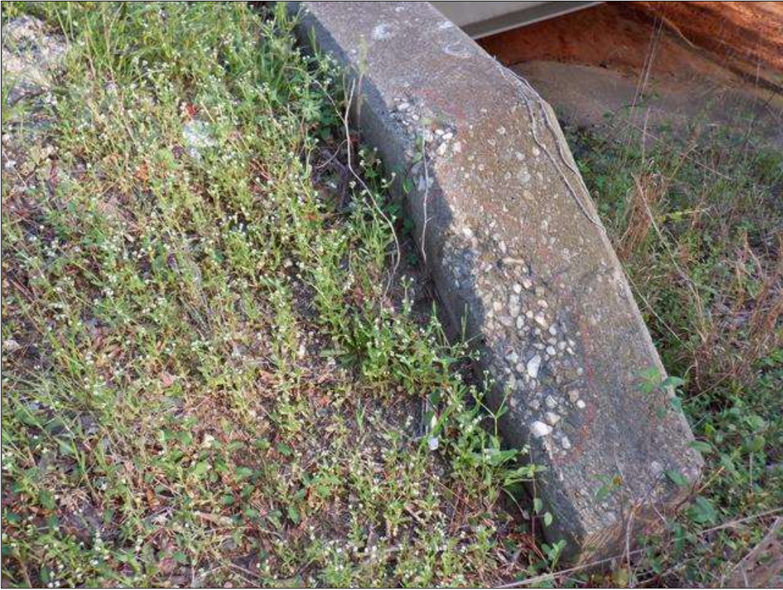
WINGWALL: 2- UP TO 18 INCHES X 5 INCHES X 3 INCHES SPALLS IN TOP OF SOUTHEAST WINGWALL.
