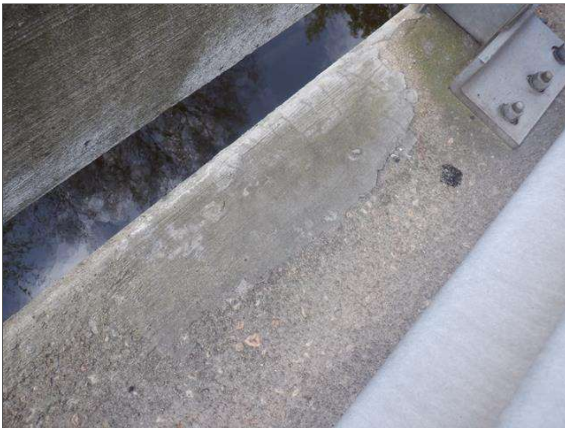
Span 2 Right Concrete Rail: 36 INCHES X UP TO 9 INCHES CRACKED PATCHED AREA WITH UP TO 1/64 INCHES CRACKING IN CURB NEAR BENT 2.
