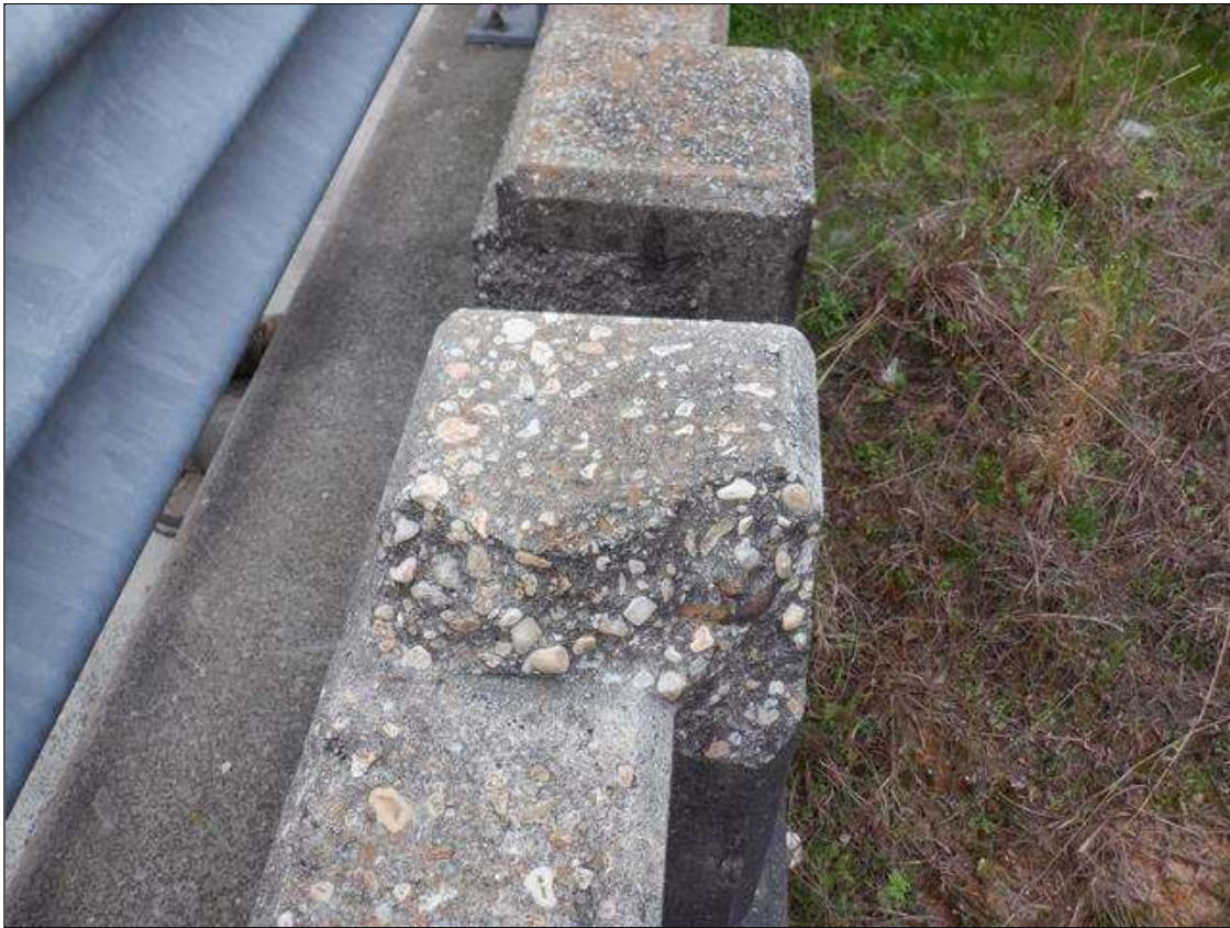
Span 1 Left Concrete Rail: 2- UP TO 4 INCHES X 10 INCHES X 7 INCHES SPALLS WITH EXPOSED REINFORCING IN TOP OF POSTS, 17 FEET FROM END BENT 1.
