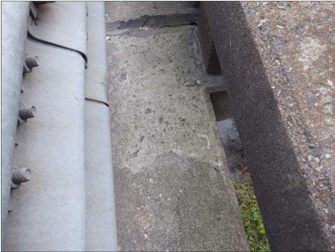
Span 1 Right Concrete Rail: 2 FEET X UP TO 2 FEET CRACKED PATCHED AREA WITH UP TO 1/32 INCHES CRACKING IN CURB AT BENT 1.
