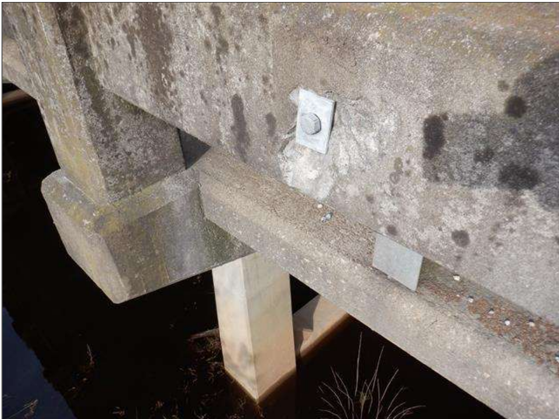
Span 4 Right Concrete Rail: 5- UP TO 7 INCHES X 6 INCHES X 1 INCHES SPALLS IN OUTSIDE FACE OF RAIL. (PHOTO TAKEN NEAR MIDSPAN)
