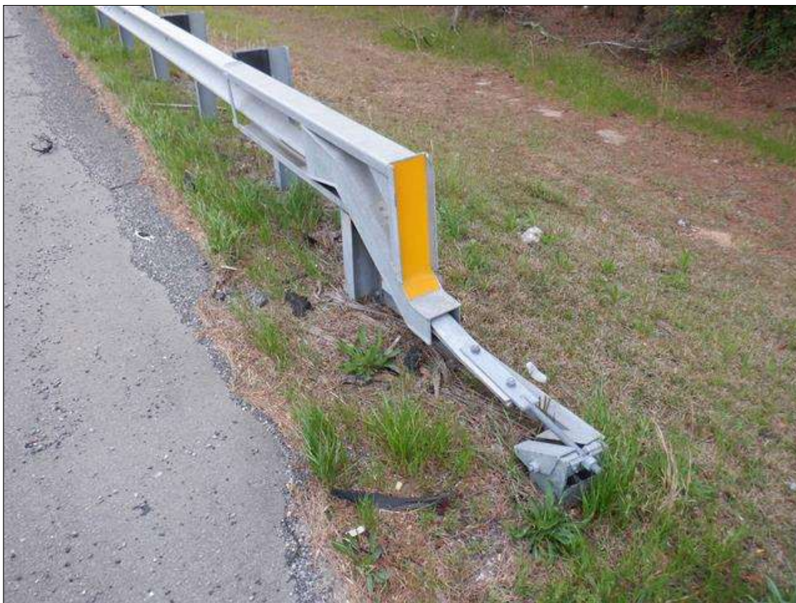
SOUTHEAST GUARDRAIL TERMINAL
