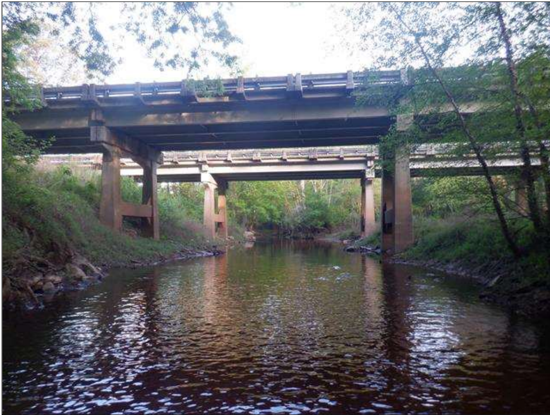
SPAN 2 WATERWAY OPENING LOOKING WEST
