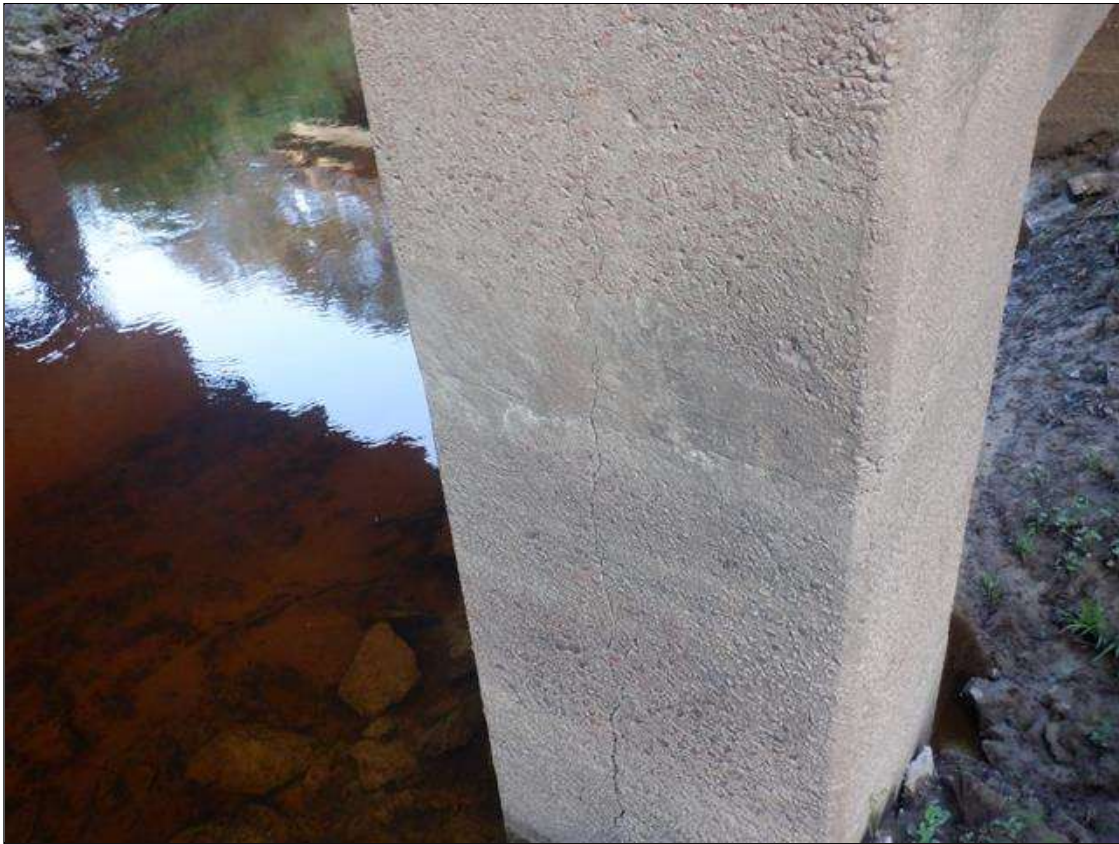
Bent 2 Pile 2: 2- UP TO 6 FEET X 1/8 INCHES VERTICAL CRACKS ON NORTH AND EAST FACE, 13 FEET FROM BOTTOM OF CAP.
