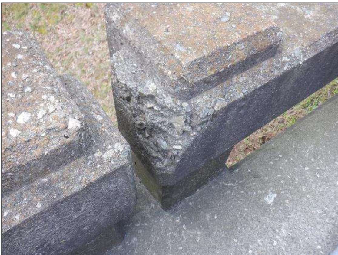
Span 1 Right Concrete Rail: 4 INCHES X 7 INCHES X UP TO 6 INCHES SPALL AT POST 2.
