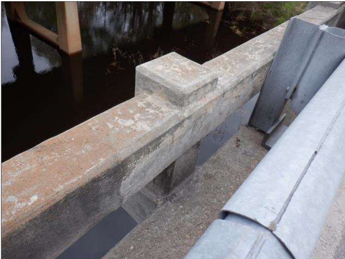
Span 2 Left Concrete Rail: 10 FEET X 1 FEET X 1 FEET CRACKED PATCHED AREA WITH UP TO 1/64 INCHES CRACKING AT MIDSPAN.
