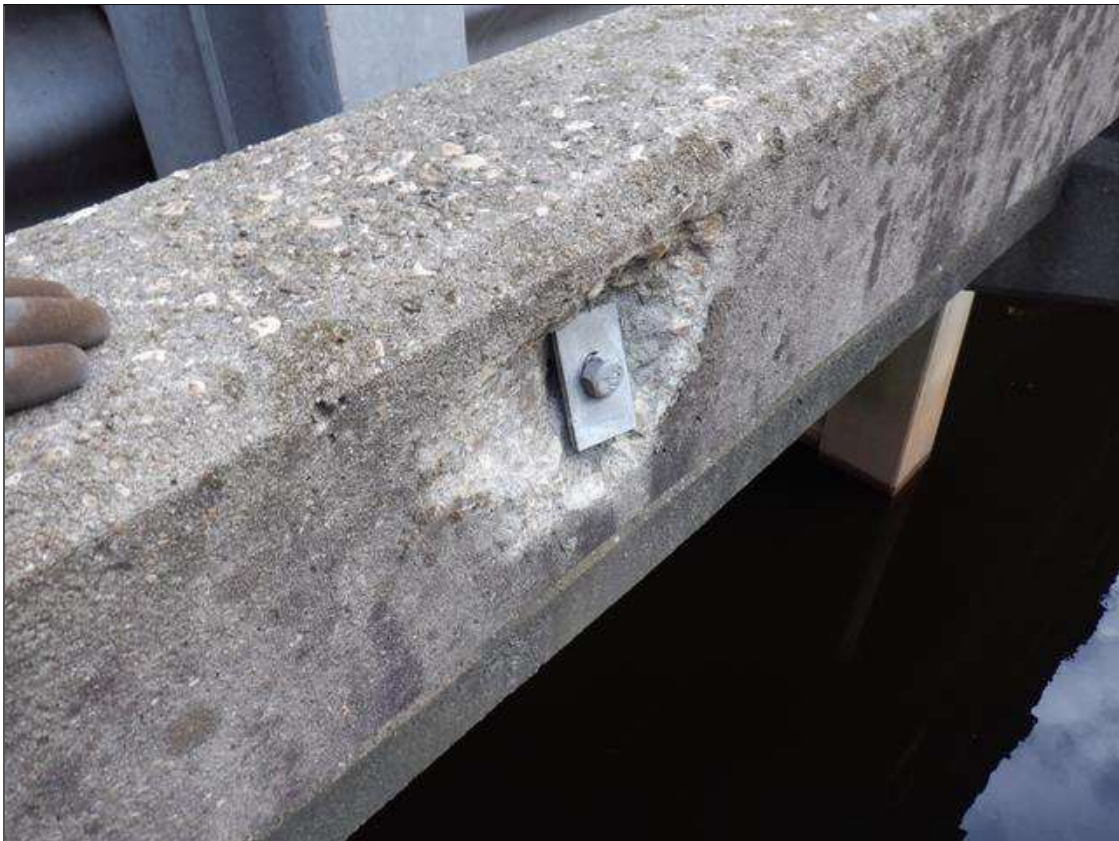
Span 2 Right Concrete Rail: 9 INCHES X UP TO 9 INCHES X 1 INCHES SPALL IN OUTSIDE FACE AT MIDSPAN.
