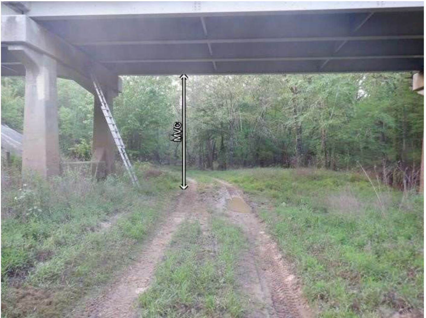
SPAN 3 CLEARANCE OPENING, GREENWAY, LOOKING EAST
