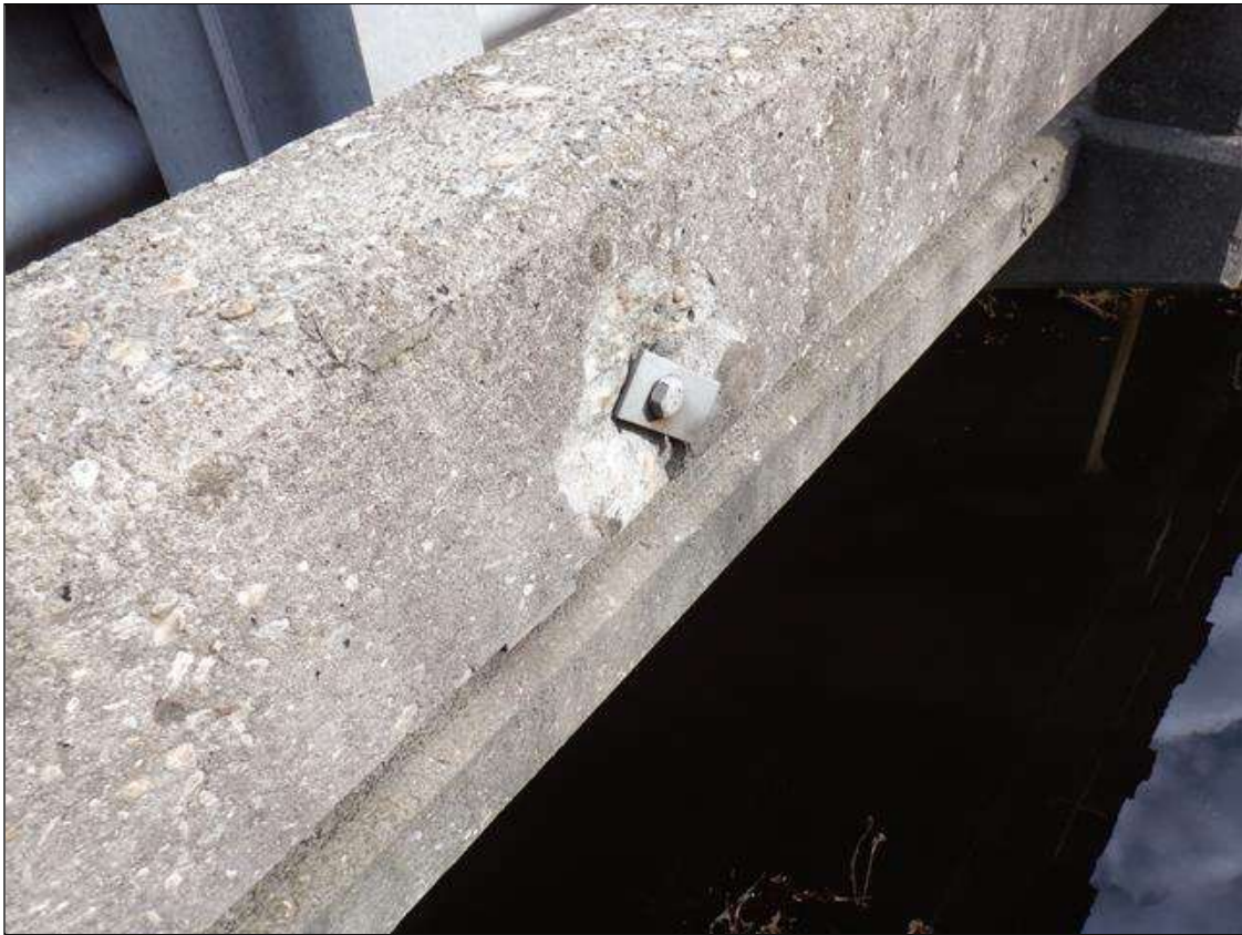
Span 3 Right Concrete Rail: (3) UP TO 9 INCHES X 9 INCHES X 1 INCHES SPALLS IN OUTSIDE FACE. (PHOTO TAKEN NEAR BENT 2)
