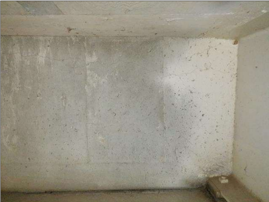
End Bent 1 Abutment: 32 FEET OF UP TO 1/32 INCHES HORIZONTAL AND VERTICAL CRACKS, SOME WITH EFFLORESCENCE. (PHOTO TAKEN IN BAY 2)
