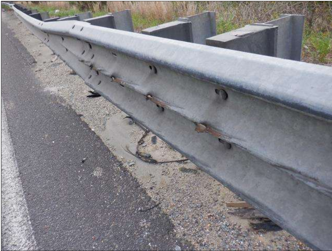
General Comments and Misc. Items: (PAR) 15 FEET OF IMPACT DAMAGE WITH 4- UP TO 3 INCHES X 1 INCHES GOUGES IN NORTHEAST GUARDRAIL, 50 FEET FROM END BENT 2.
