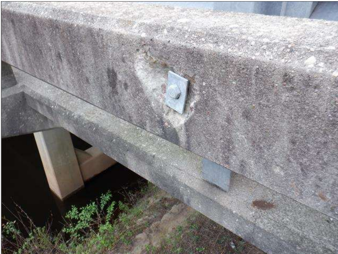
Span 1 Left Concrete Rail: (5) UP TO 7 INCHES X 9 INCHES X 1 INCHES SPALLS ON OUTSIDE FACE AT BOLT LOCATIONS.
