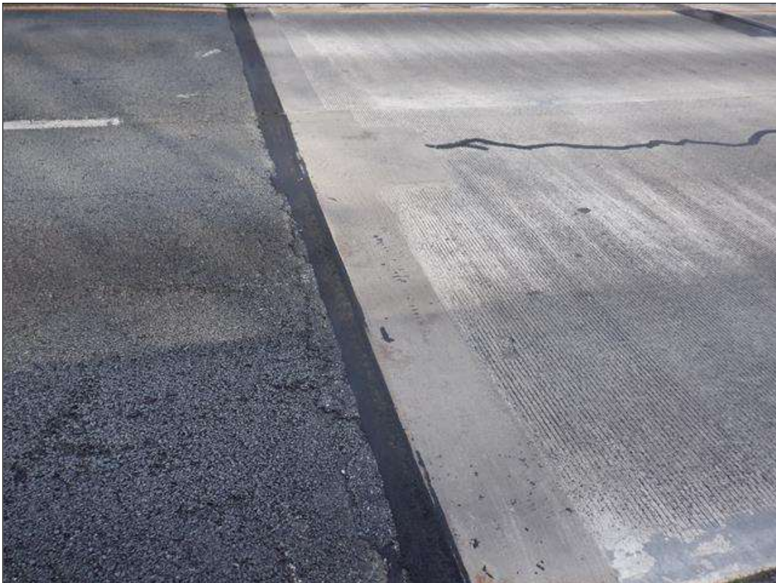
Approach 1 : FULL WIDTH X UP TO 3 FEET PATCHED AREA IN SOUTH END.
