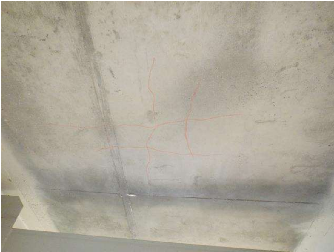
Span 1 Deck: 750 SQUARE FEET OF UP TO 1/32 INCHES MAP CRACKING AT RANDOM THROUGHOUT UNDERSIDE. (PHOTO TAKEN IN BAY 1)
