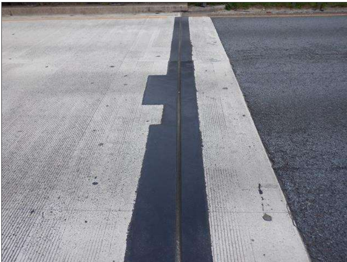
JOINT OVER END BENT 2 LOOKING WEST
