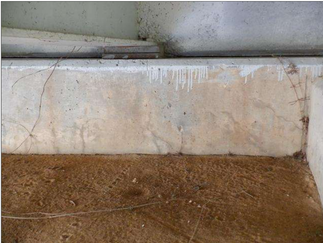
End Bent 2 Cap 1: 12 FEET X UP TO 2 FEET AREA OF UP TO 1/32 INCHES MAP CRACKING, BEGINNING AT WEST END.
