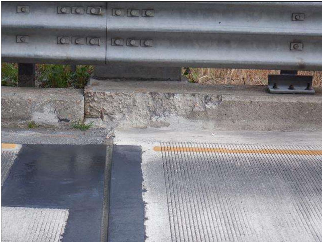
Span 1 Left Concrete Rail: 35 INCHES X UP TO 9 INCHES X 2 INCHES SPALL WITH EXPOSED REBAR IN CURB AT END BENT 1.
