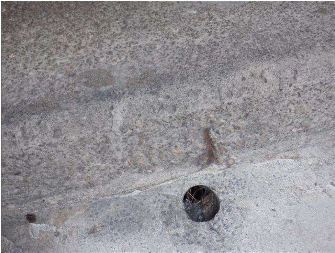
Span 4 Left Concrete Rail: 2 INCHES X 6 INCHES X UP TO 1/2 INCHES SPALL WITH EXPOSED REINFORCING IN EAST FACE OF CURB, NEAR MIDSPAN.
