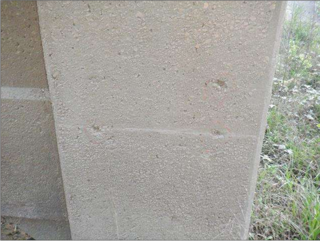
Bent 3 Pile 2: (3) UP TO 2 INCHES X 2 INCHES X 1/2 INCHES SPALLS IN SOUTH FACE, 11 FEET FROM BOTTOM OF CAP.
