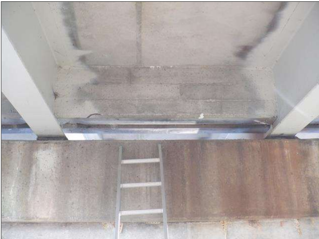
BENT 1 BAY 2 DIAPHRAGM LOOKING NORTH (OTHERS SIMILAR)
