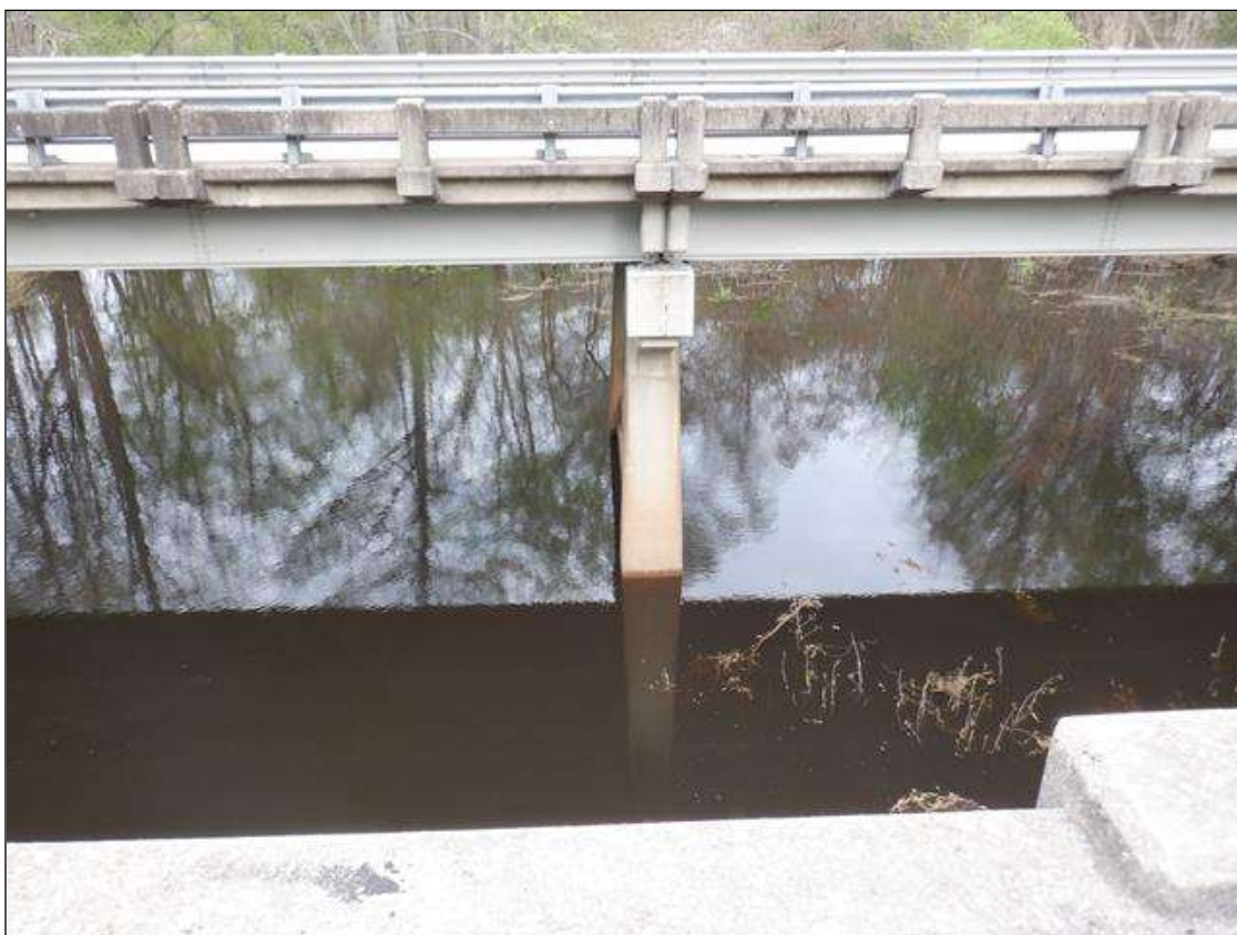
UPSTREAM VIEW FROM BRIDGE LOOKING WEST
