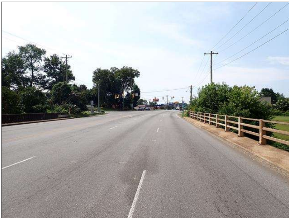
south approach looking south
