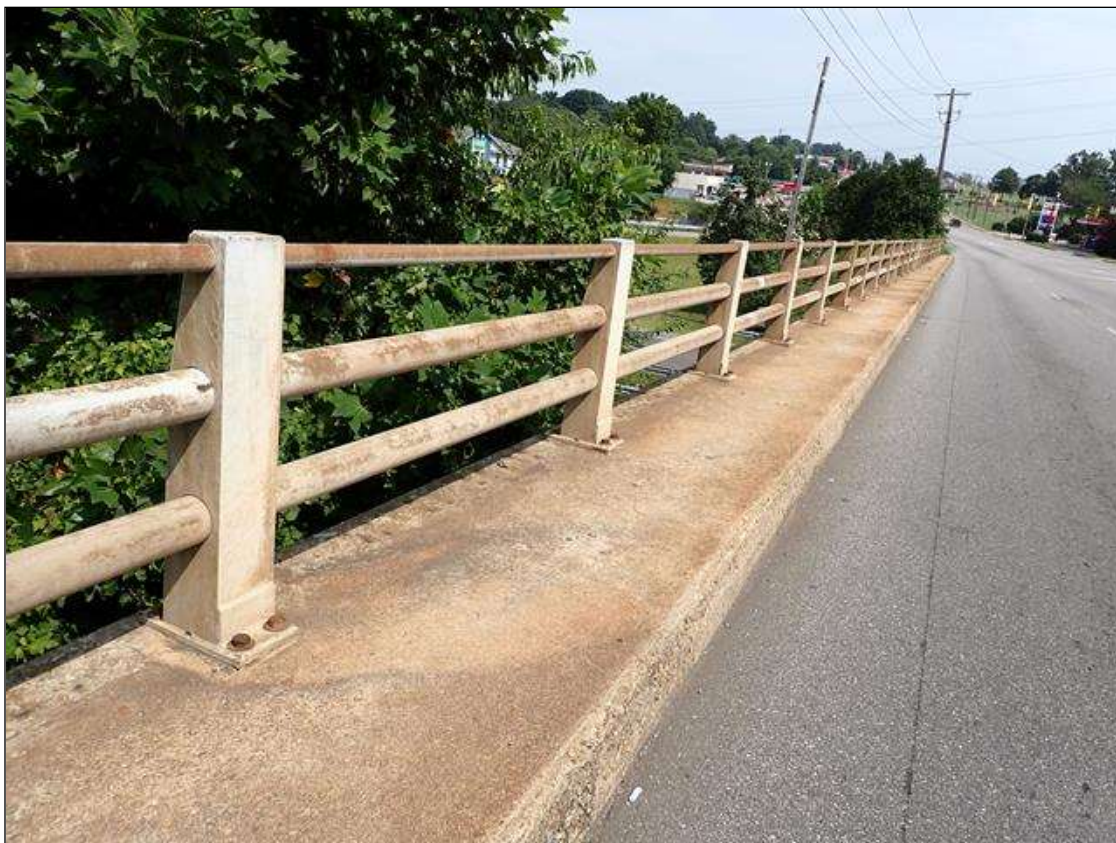
left bridge rail and sidewalk
