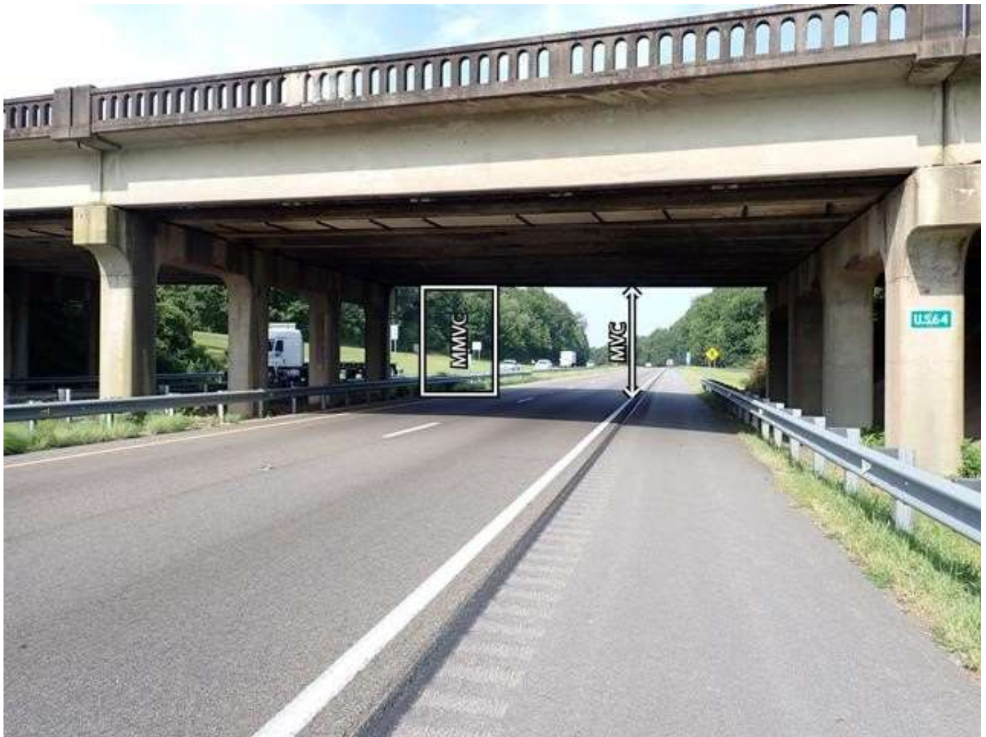
roadway under span 3, looking west
