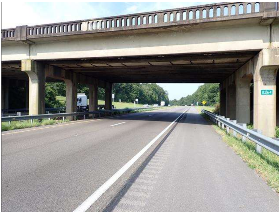
roadway under span 3, looking west (I-40 westbound)
