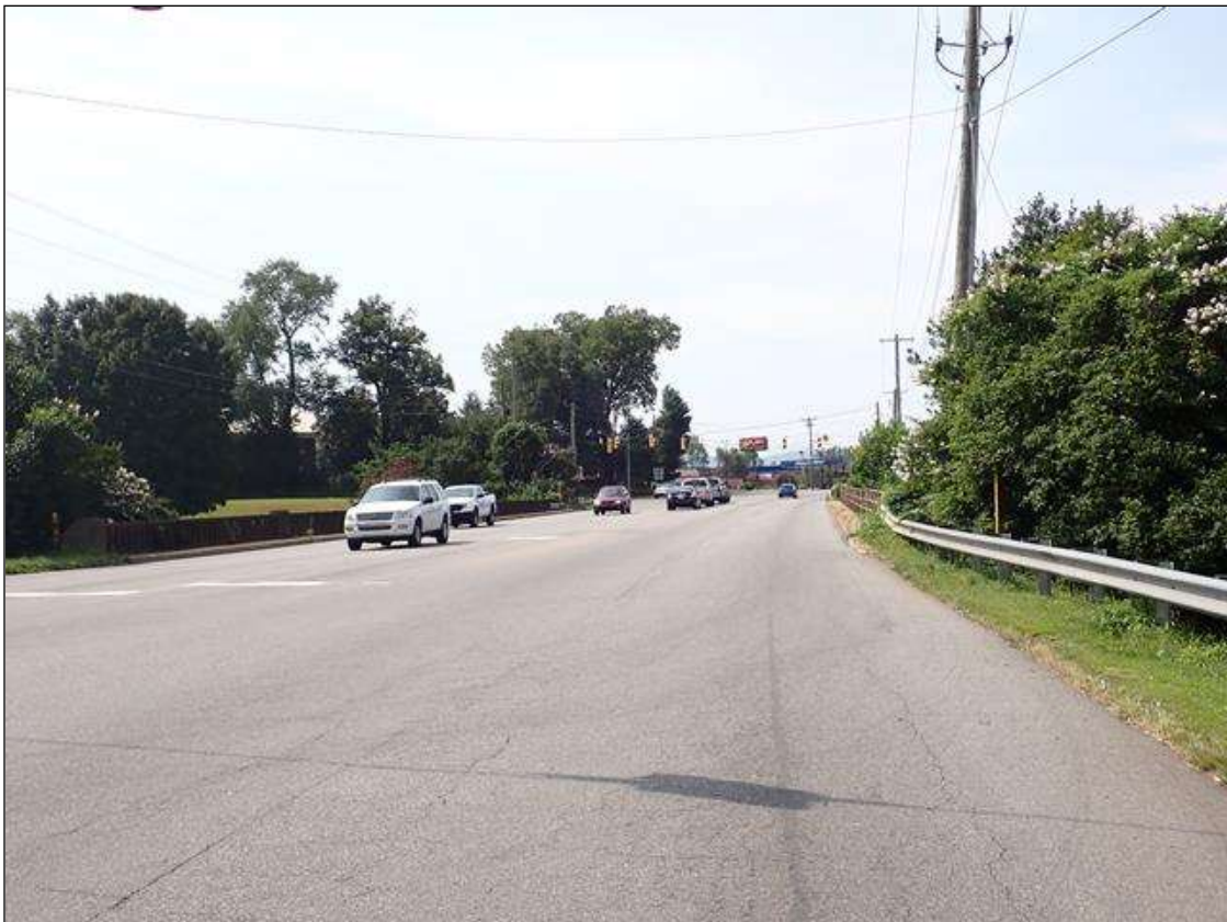
north approach looking south
