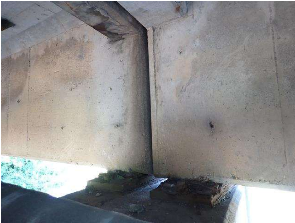
beams over bent
