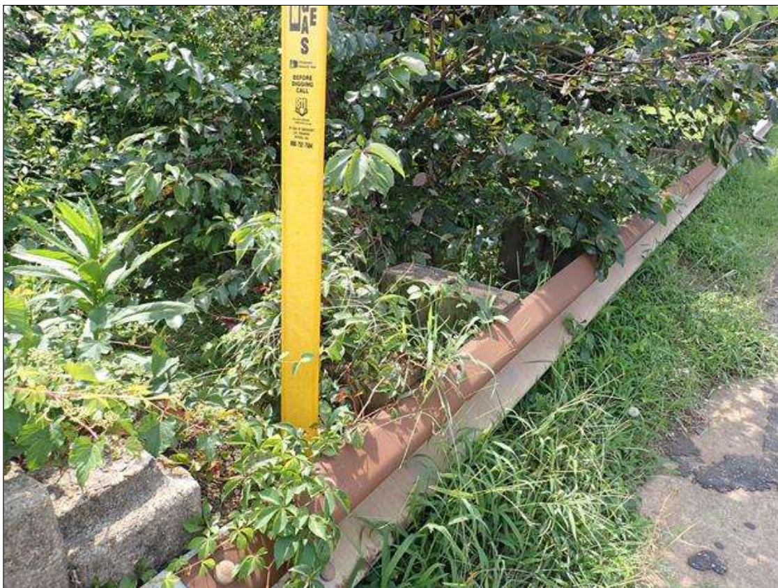
southeast guardrail transition
