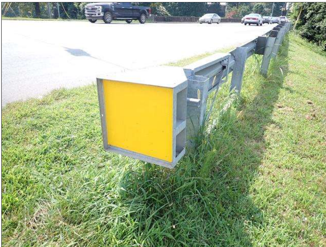
northwest guardrail termination
