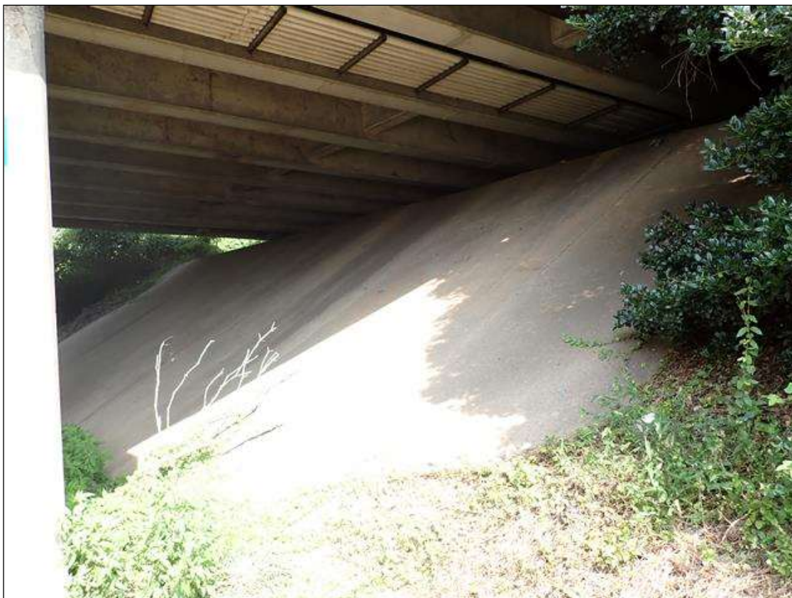
end bent 2 slope protection
