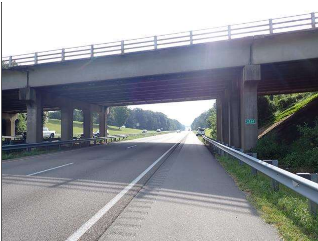
roadway under span 2, looking east (I-40 eastbound)
