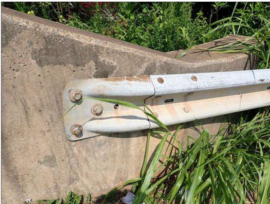
northwest guardrail attachment
