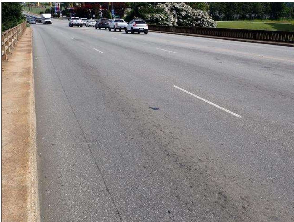
asphalt wearing surface
