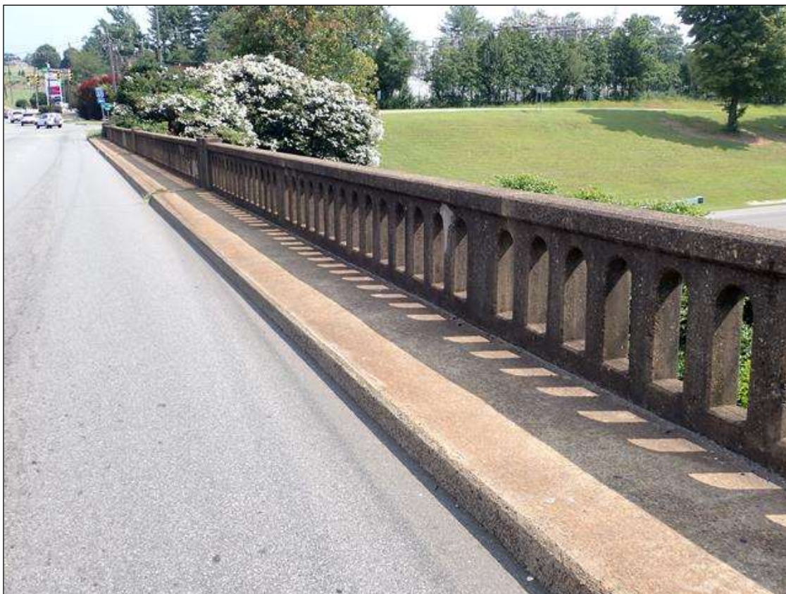
right bridge rail and sidewalk
