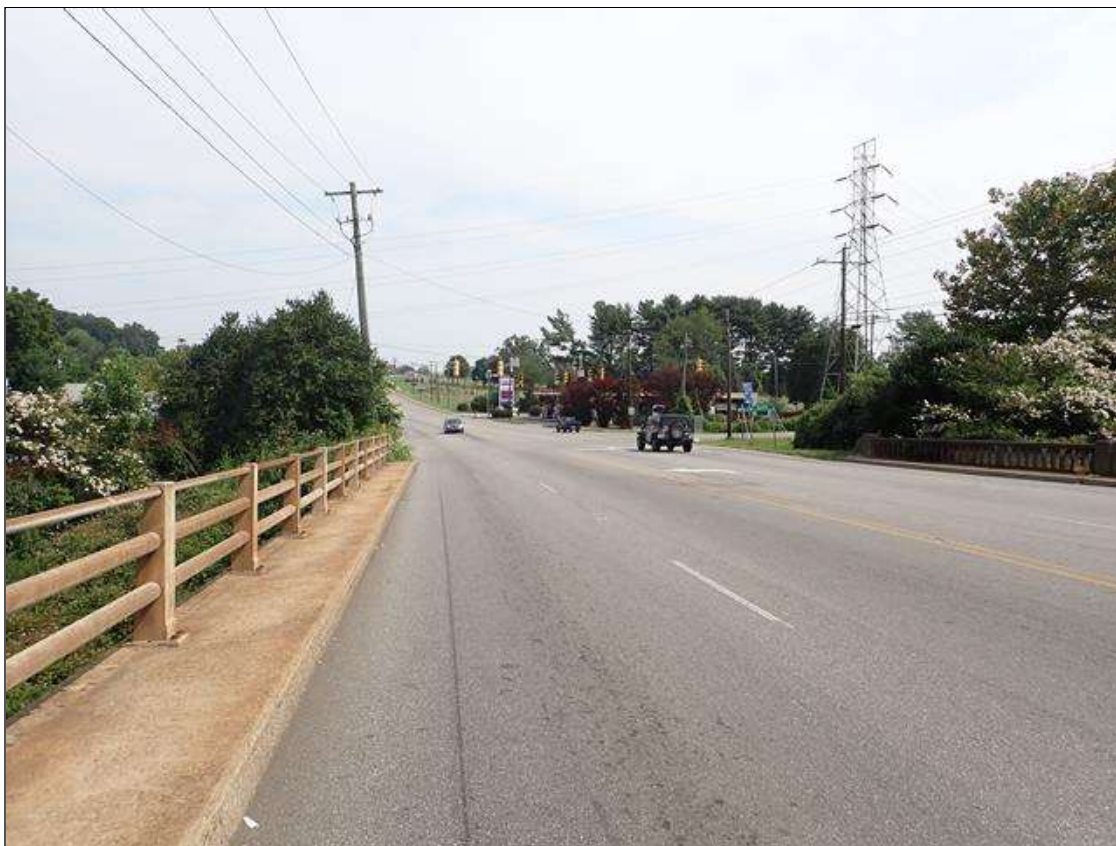
north approach looking north
