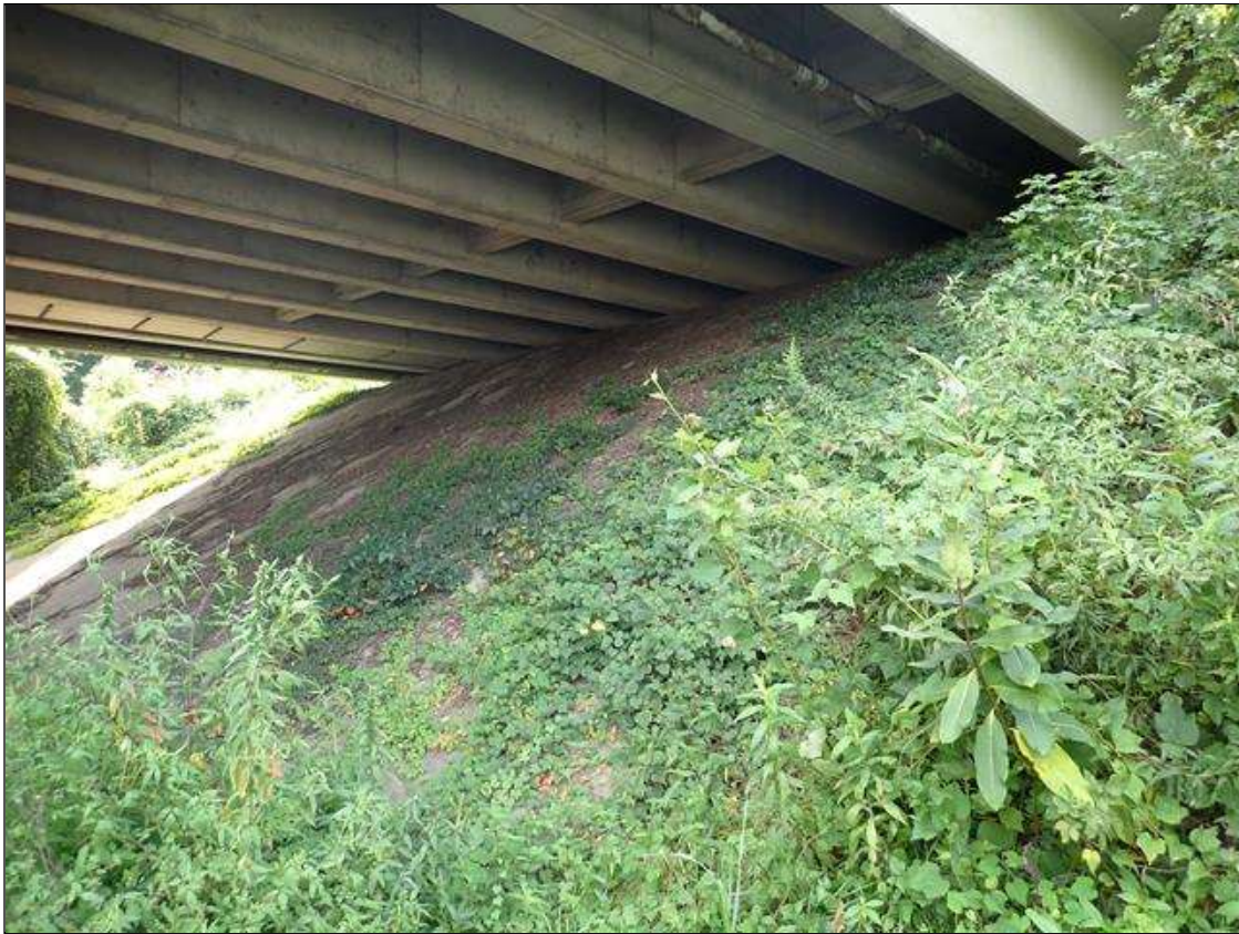
end bent 1 slope protection
