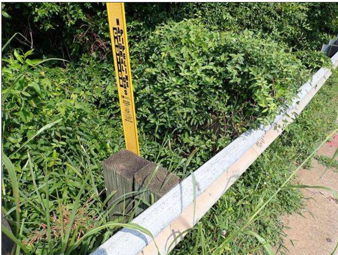
northwest guardrail transition
