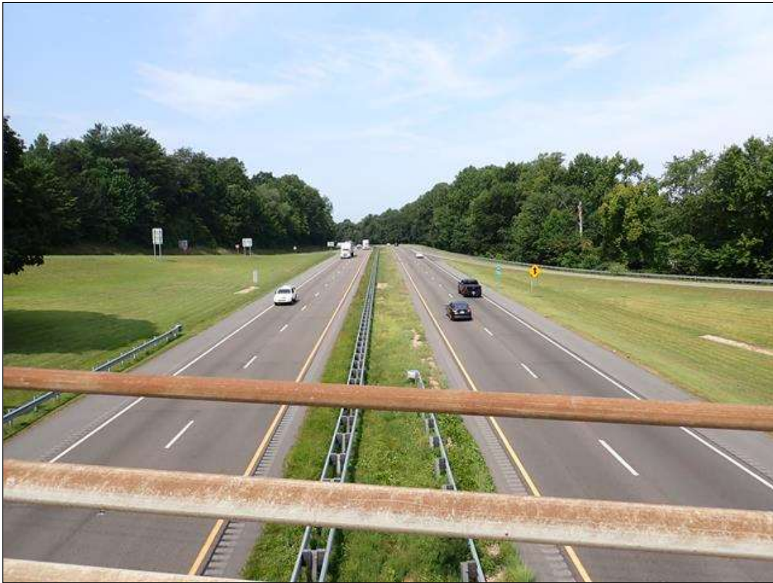
roadway looking west
