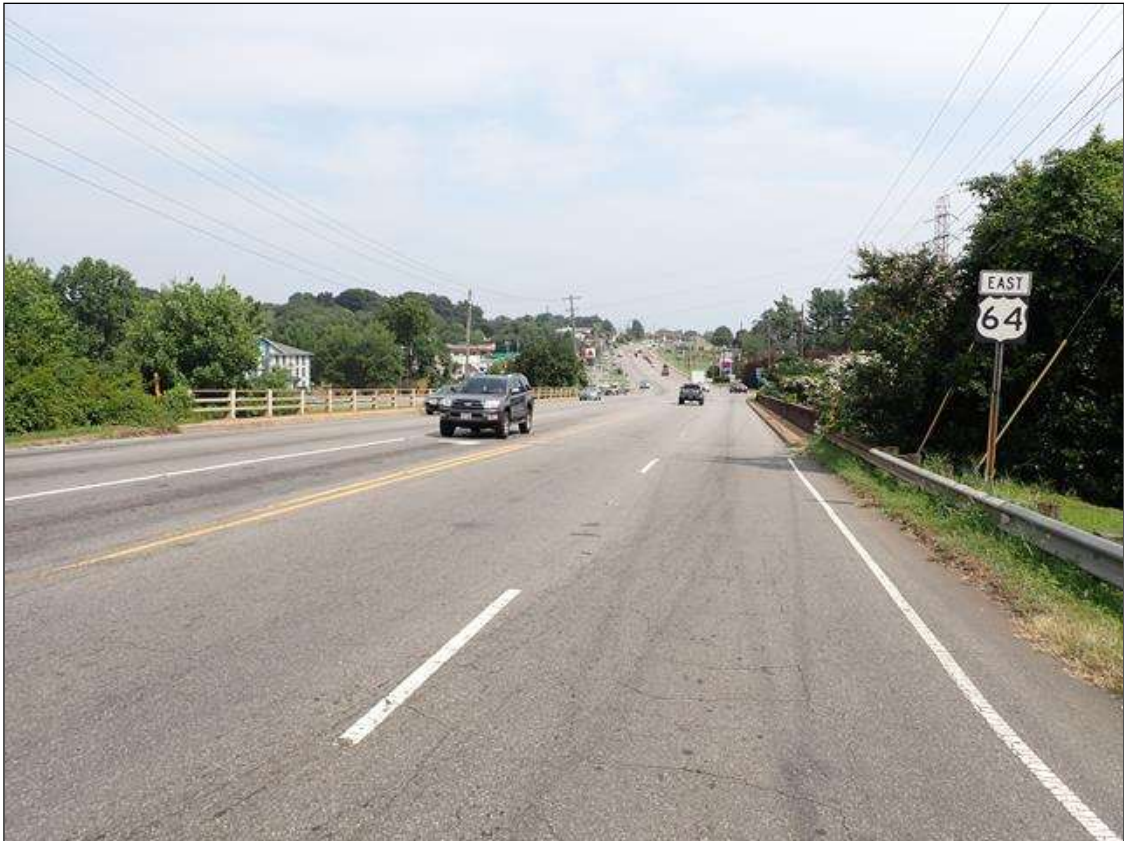
south approach looking north
