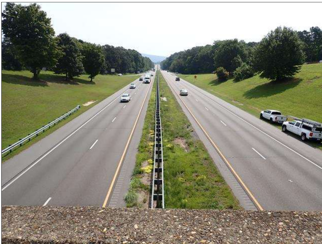
roadway looking east
