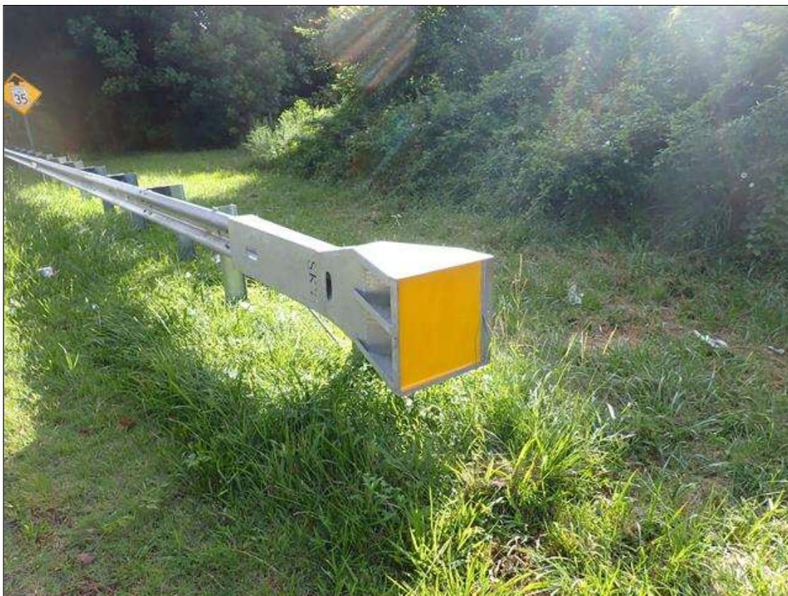
southeast guardrail termination
