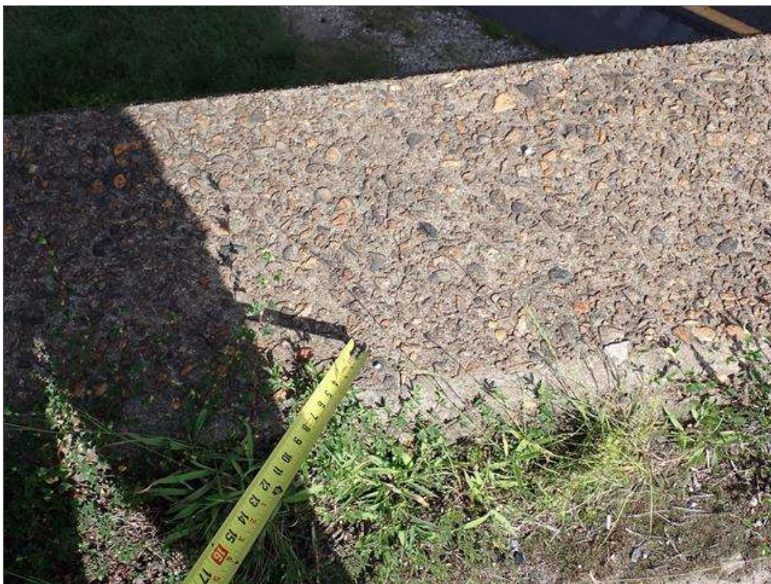
Span 2 Left Bridge Rail: WEST RAIL HAS SCATTERED CRACKS UP TO 1/32 INCH.
