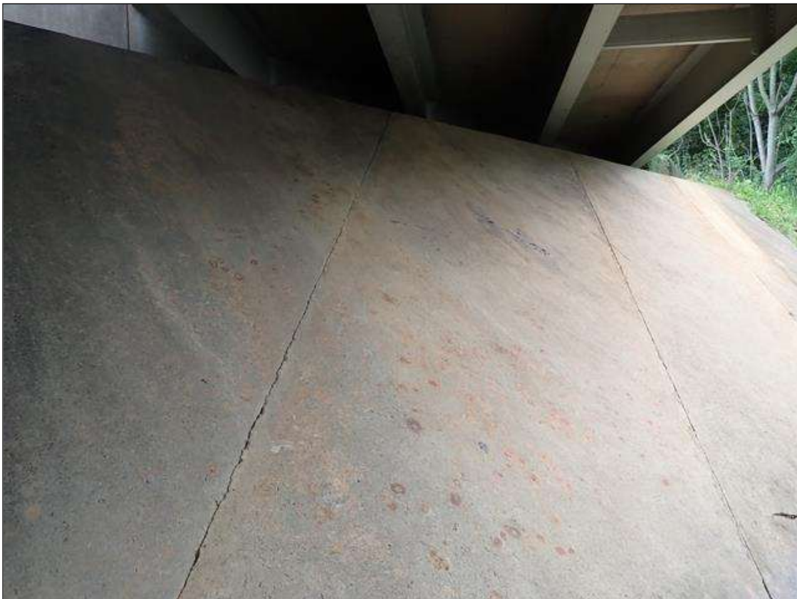
end bent 2 slope protection
