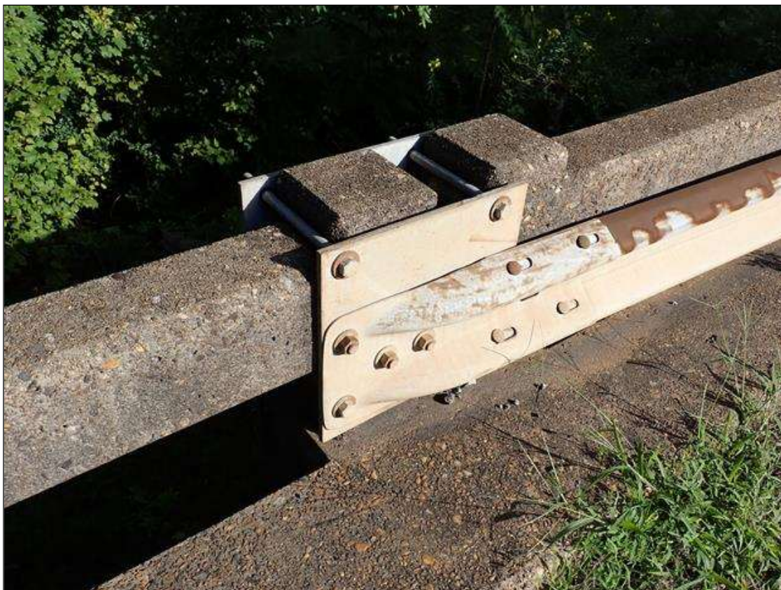
northwest guardrail attachment
