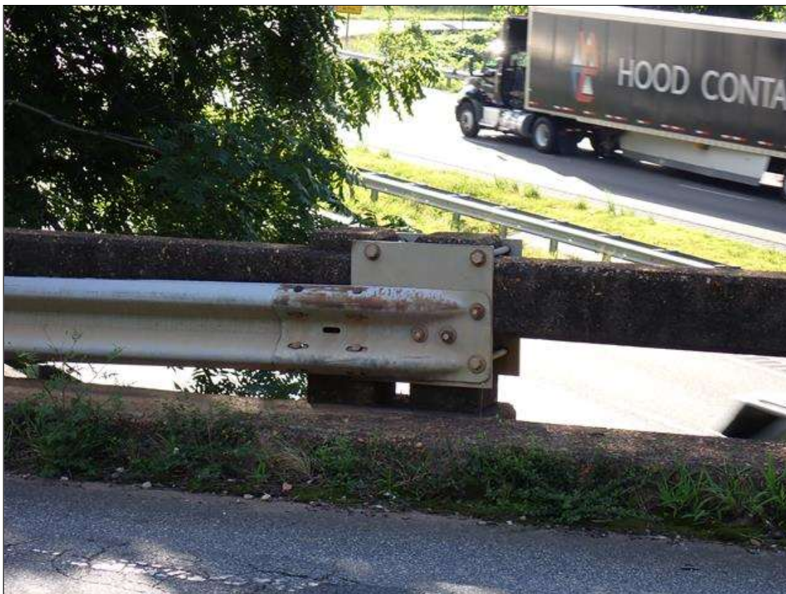
northeast guardrail attachment
