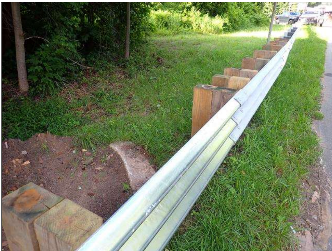
southeast guardrail transition
