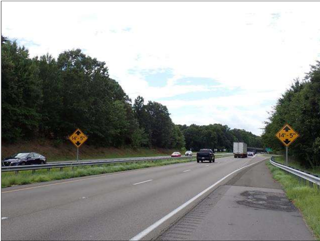
approximately 0.1 miles east of span 3, along I-40 westbound, vertical clearance signs (14 feet-5 inches)
