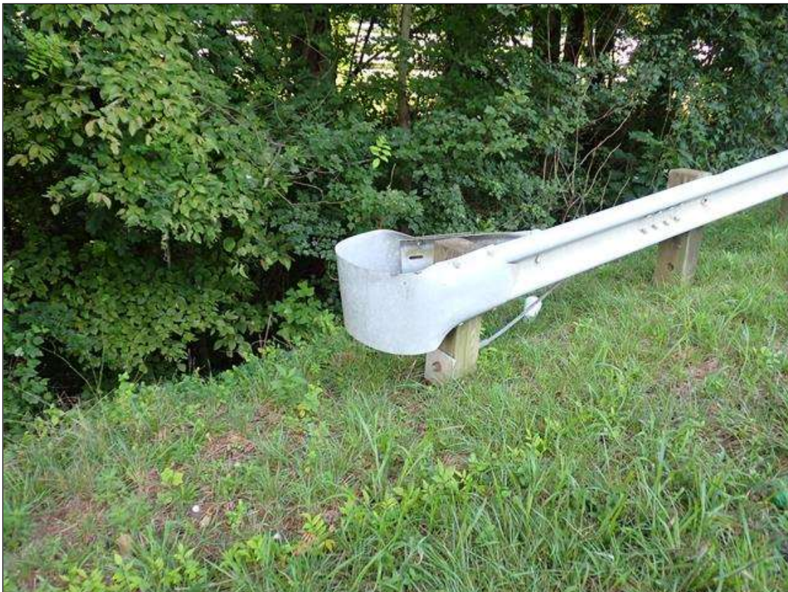
northeast guardrail termination
