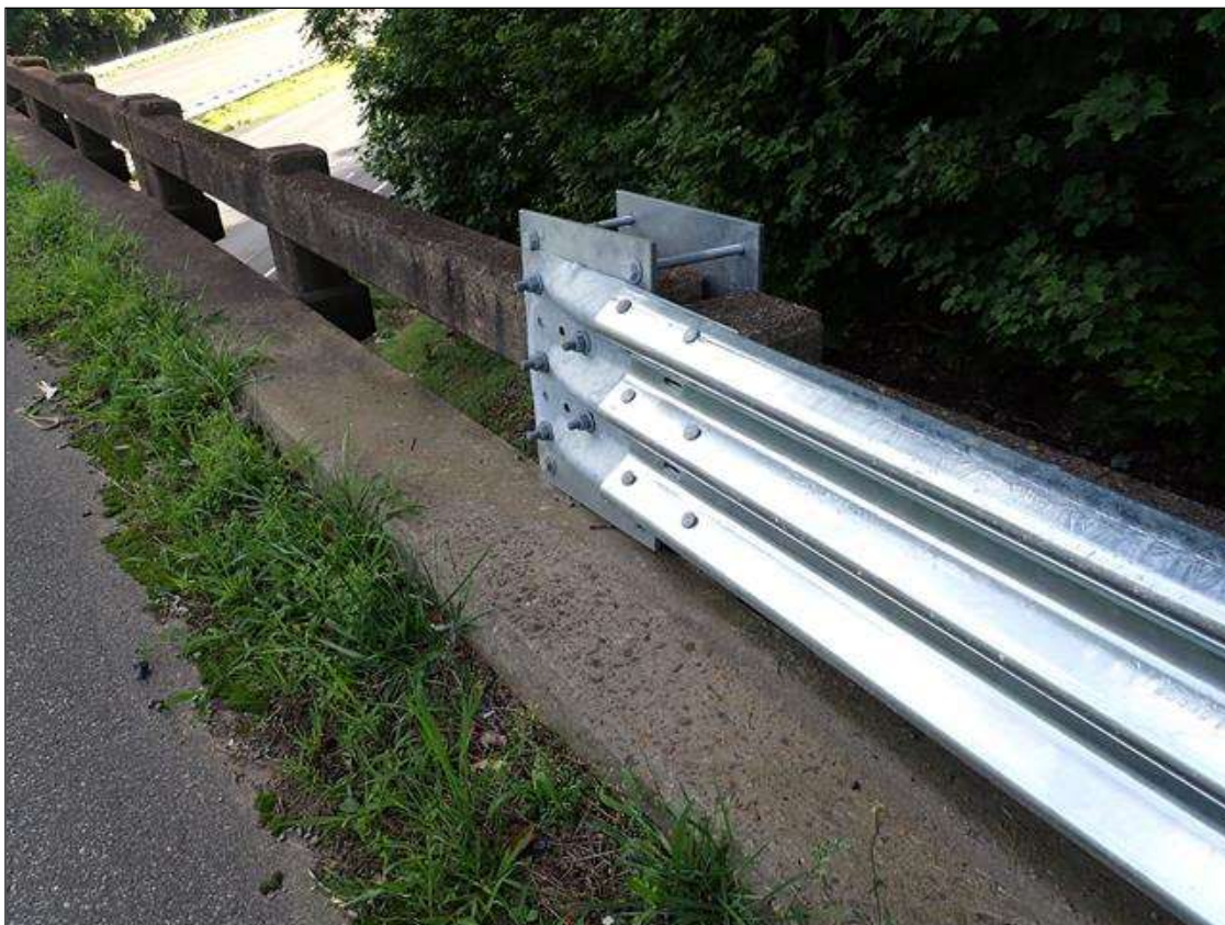
southeast guardrail attachment
