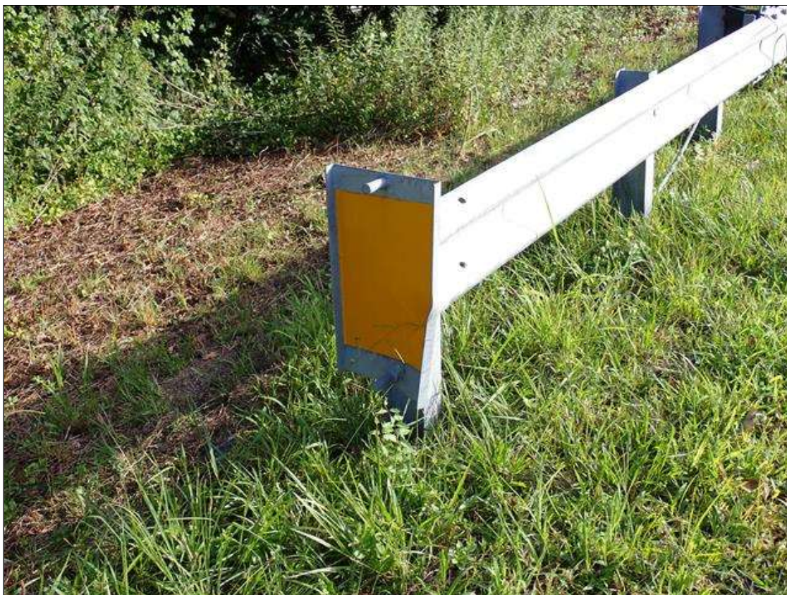
southwest guardrail termination
