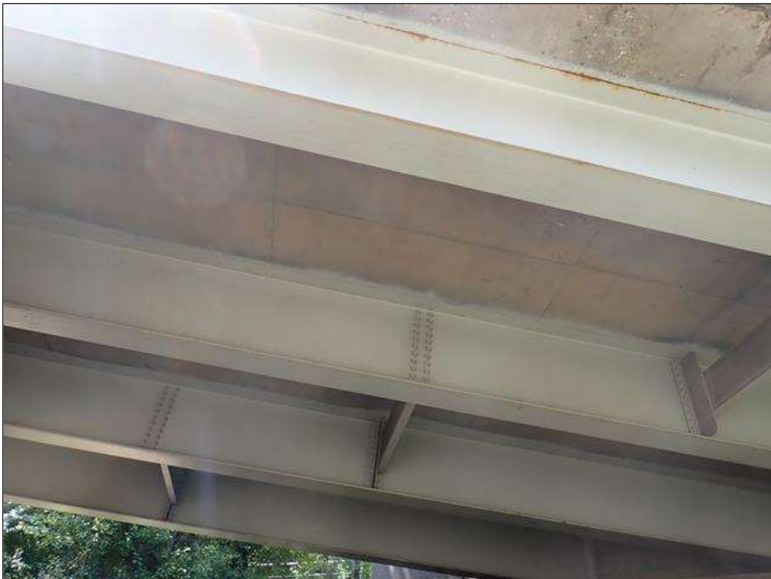
superstructure underside, span 4
