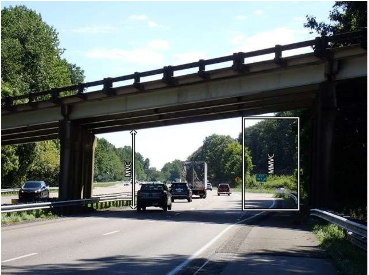
roadway under span 2, looking east (I-40 eastbound)
