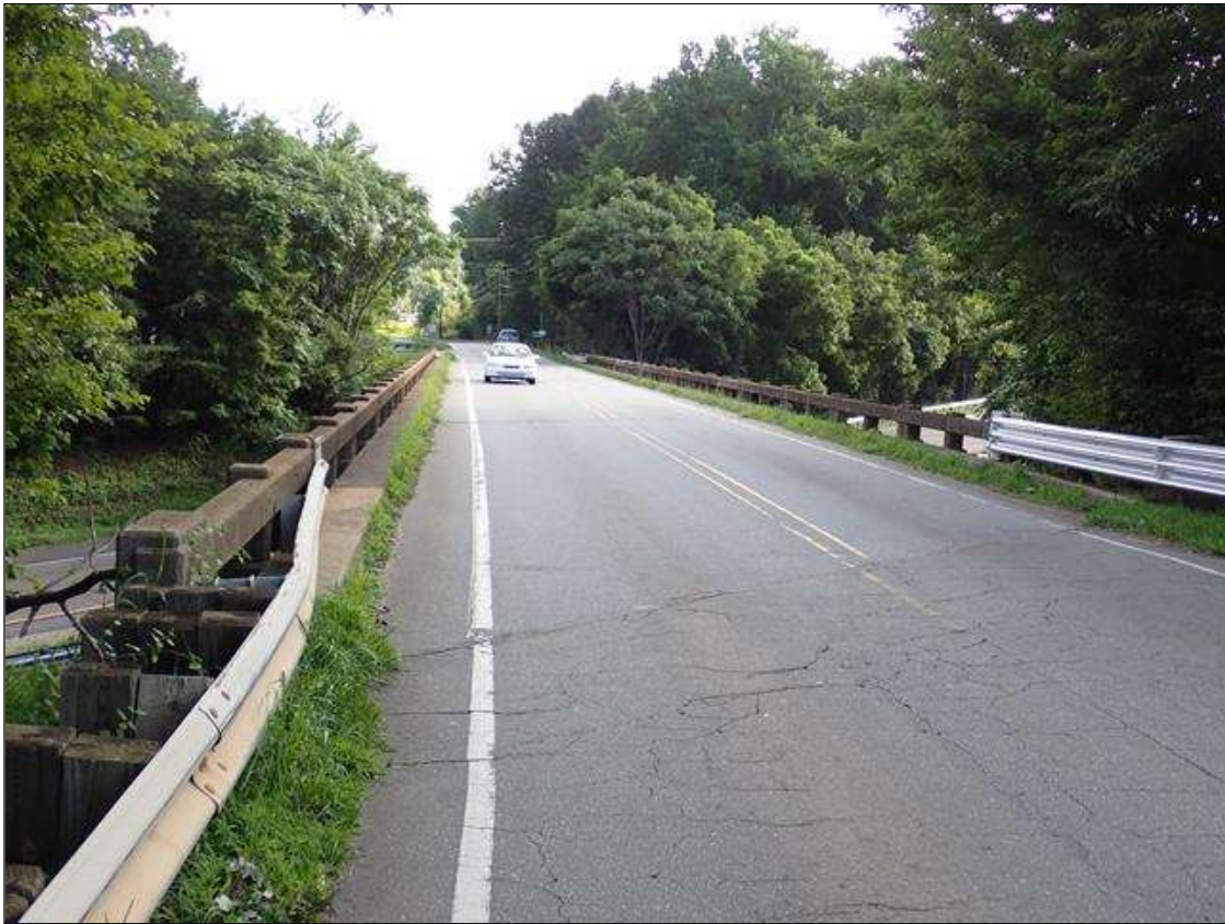
south approach looking north
