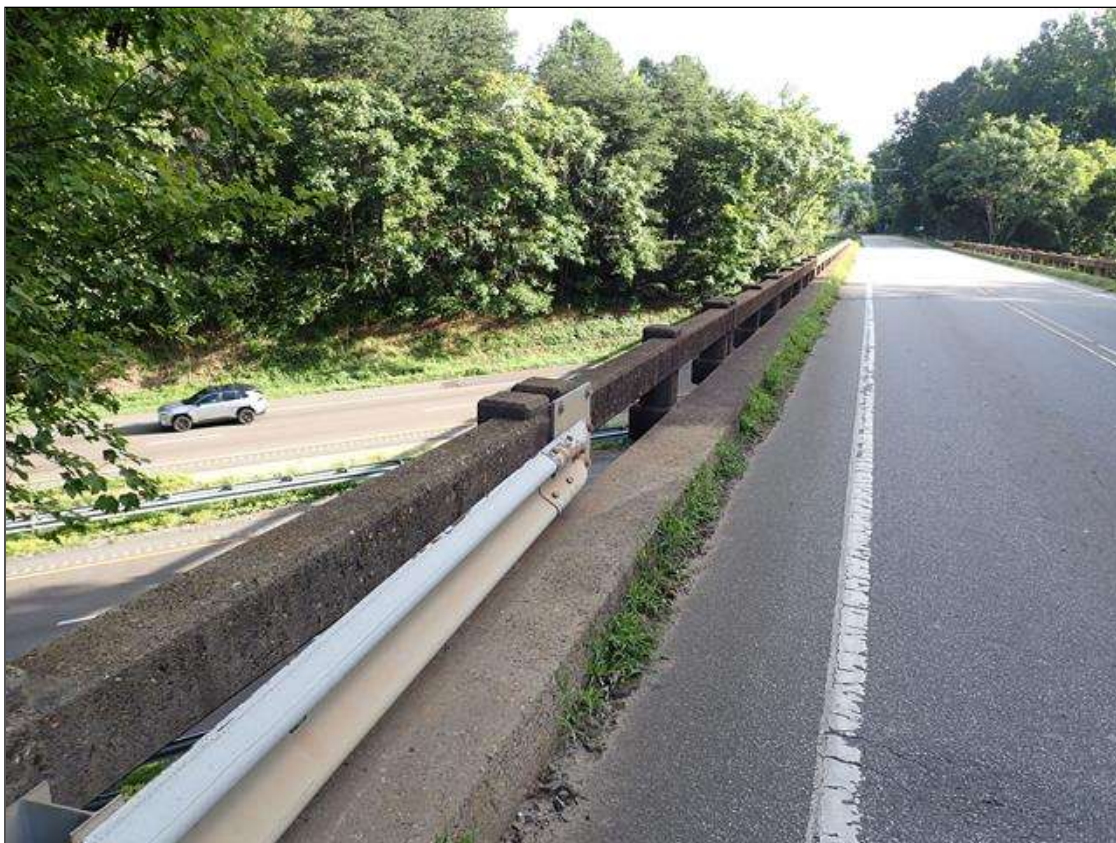
left bridge rail
