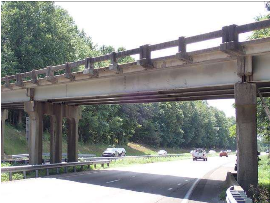
roadway under span 3, looking west (I-40 westbound)
