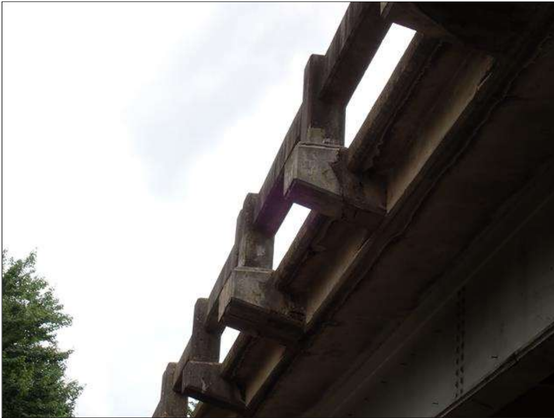
Span 3 Right Bridge Rail: (PAR) within patched area over left and right travel lanes of I-40, area of delamination with cracking (up to 1/16 inch) and rust stain, could possibly fall into traffic below
