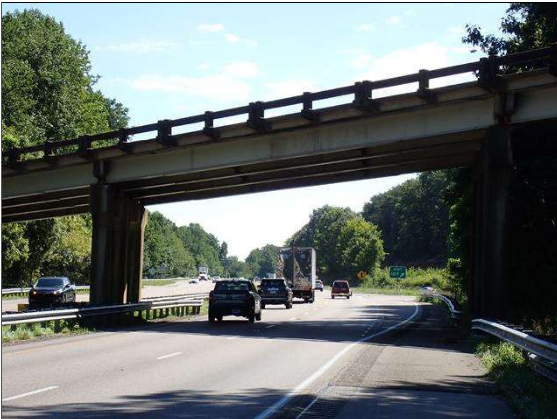
roadway under span 2, looking east (I-40 eastbound)
