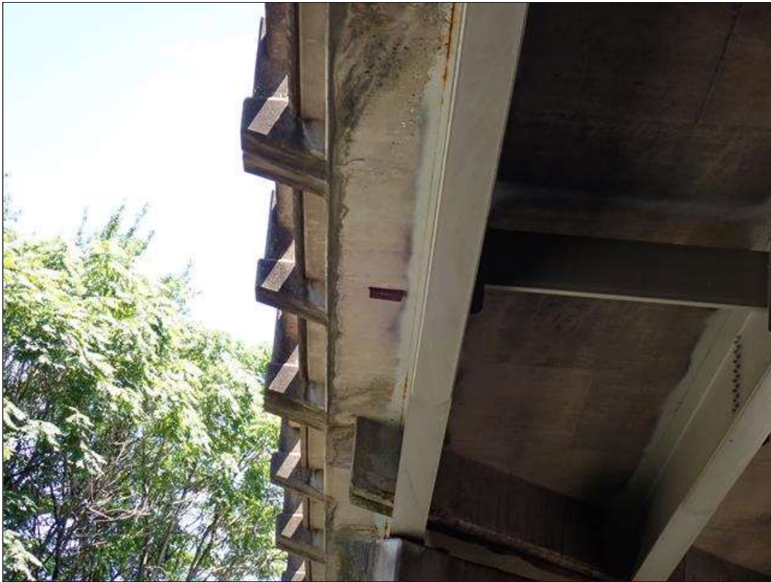
Span 2 Deck: left overhang, near bent 2, formwork left in place
