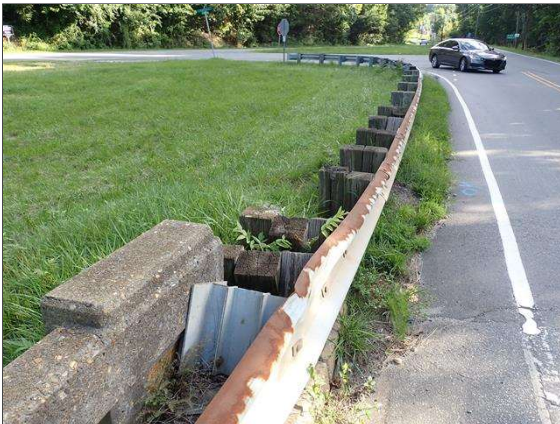
northwest guardrail transition
