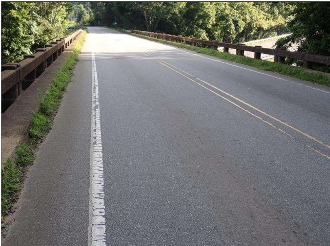
asphalt wearing surface
