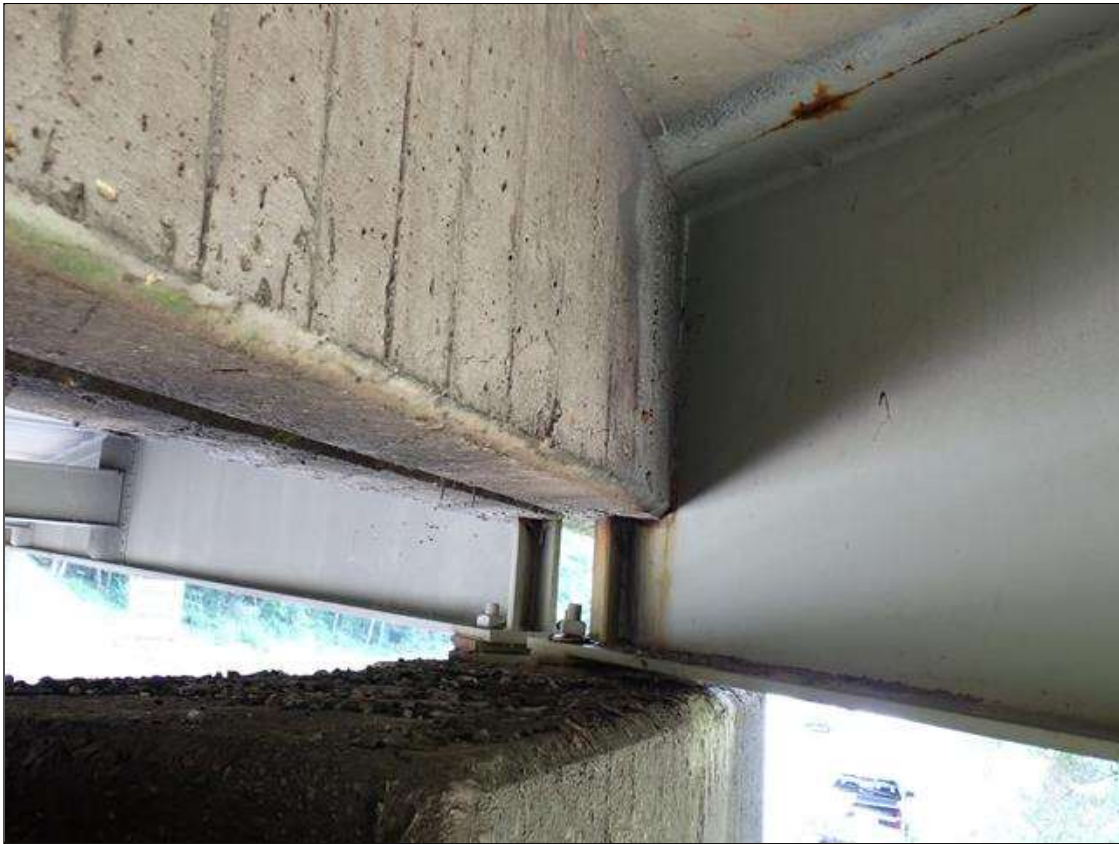
beams over bent
