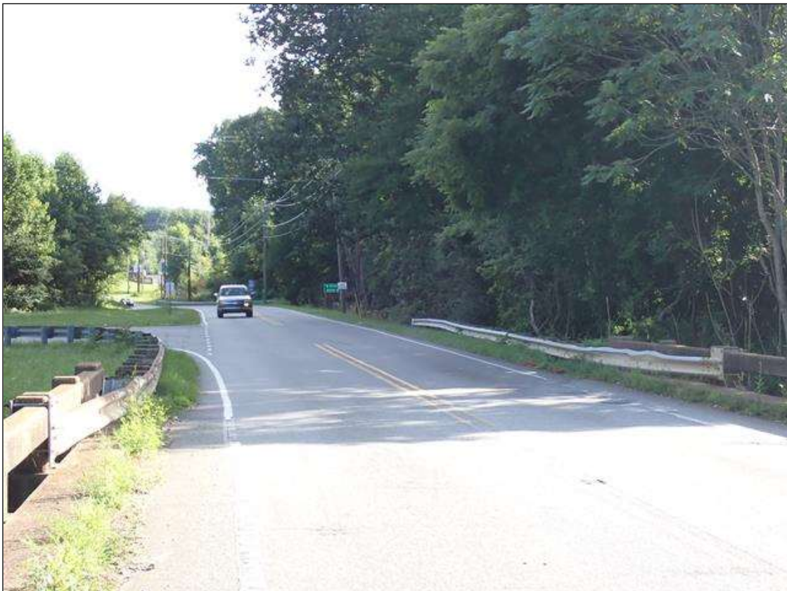
north approach looking north
