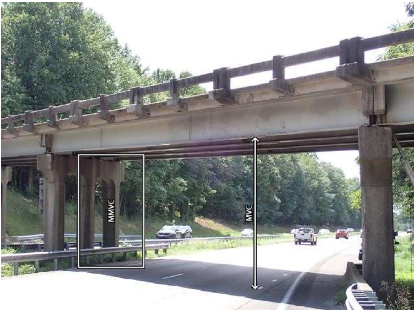
roadway under span 3, looking west (I-40 westbound)
