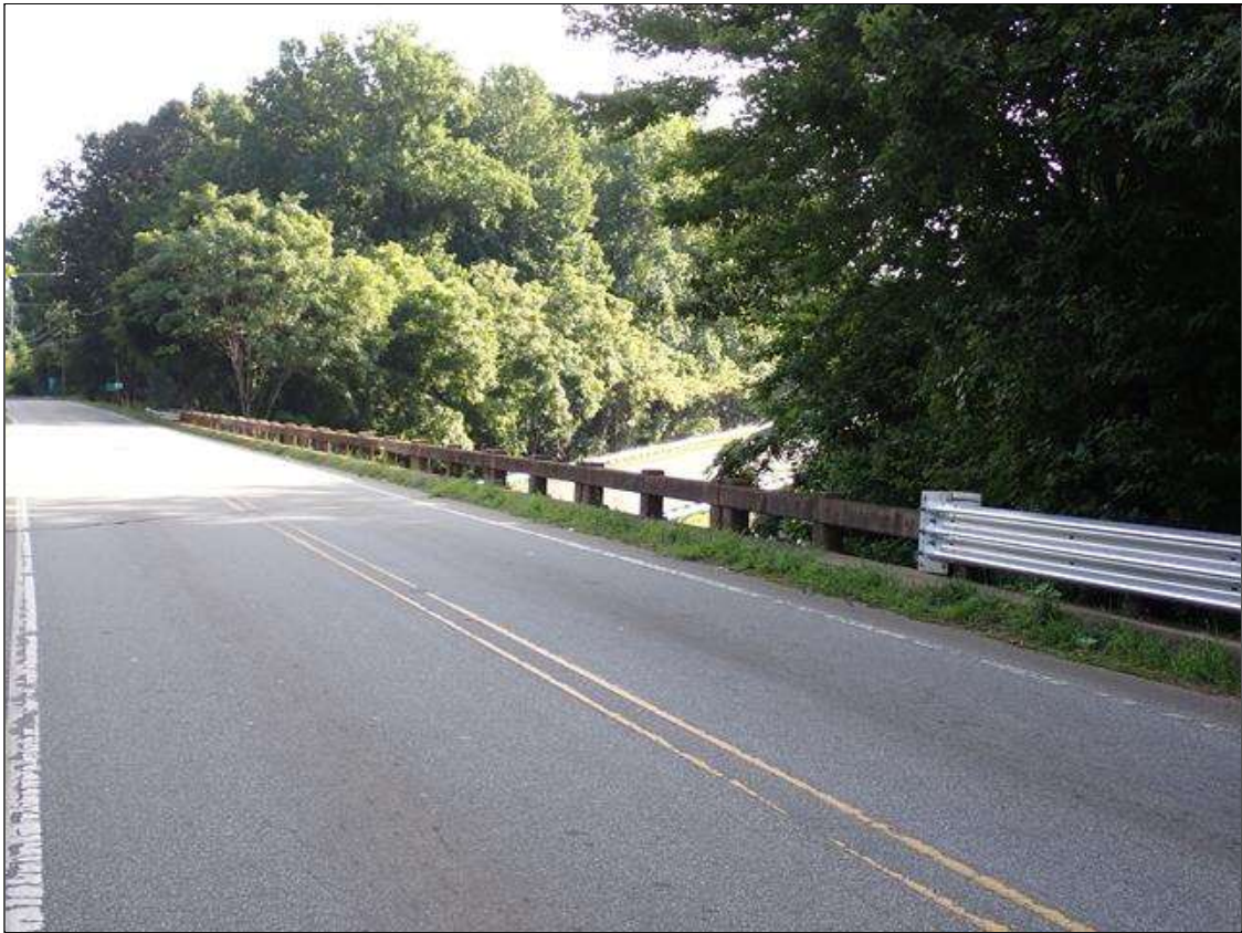
right bridge rail
