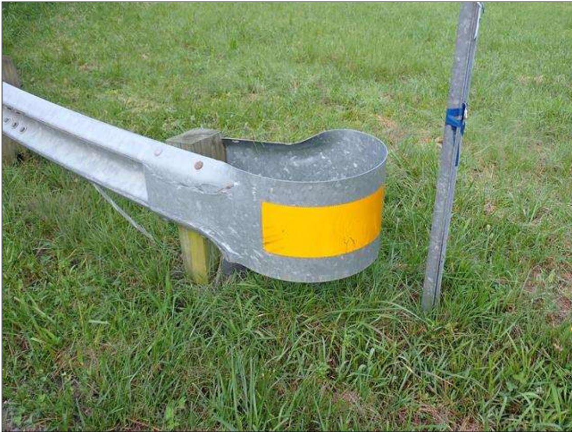
northwest guardrail termination
