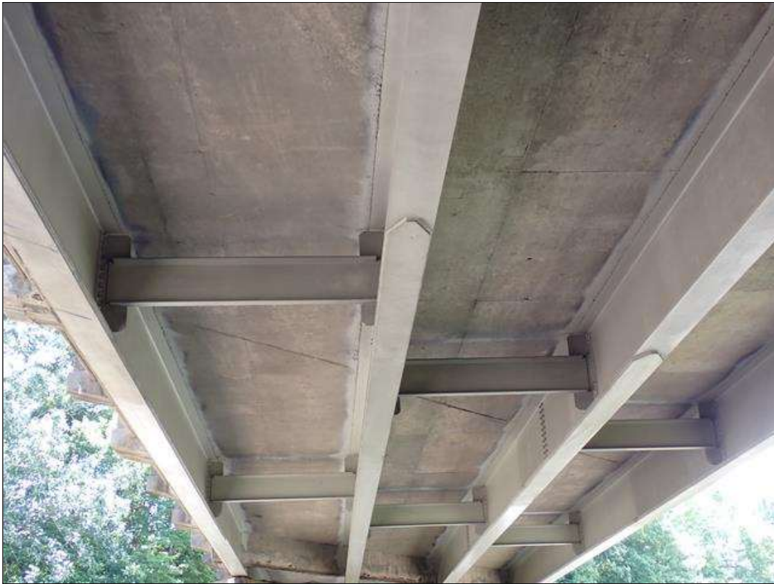
superstructure underside, span 3 (spans 1 and 2 similar)
