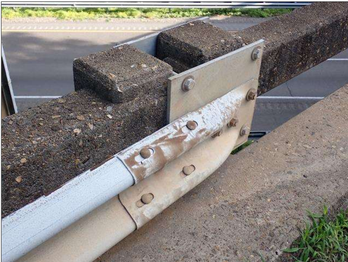
southwest guardrail attachment
