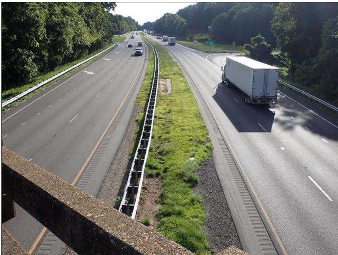
roadway looking east
