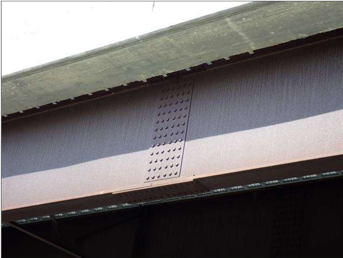
typical bolted splice connection
