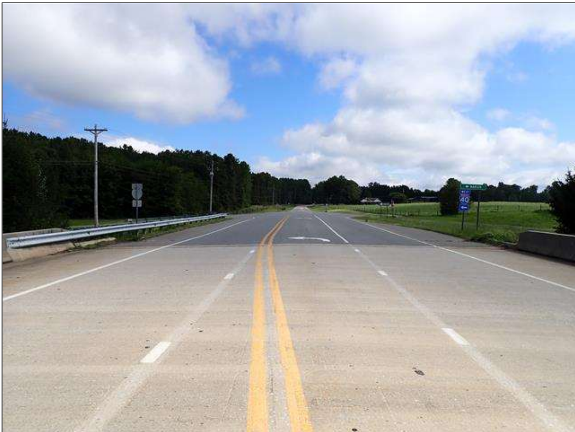
north approach looking north
