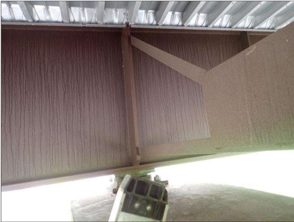
beams over bent
