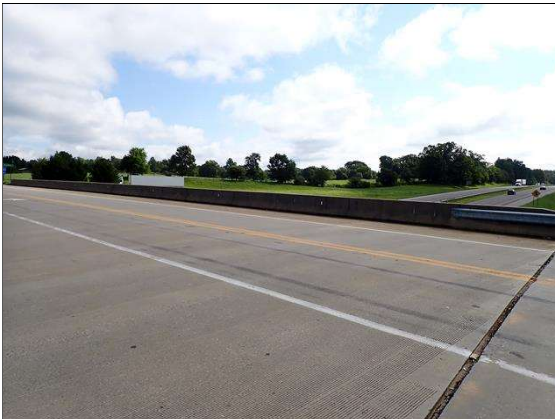
right bridge rail
