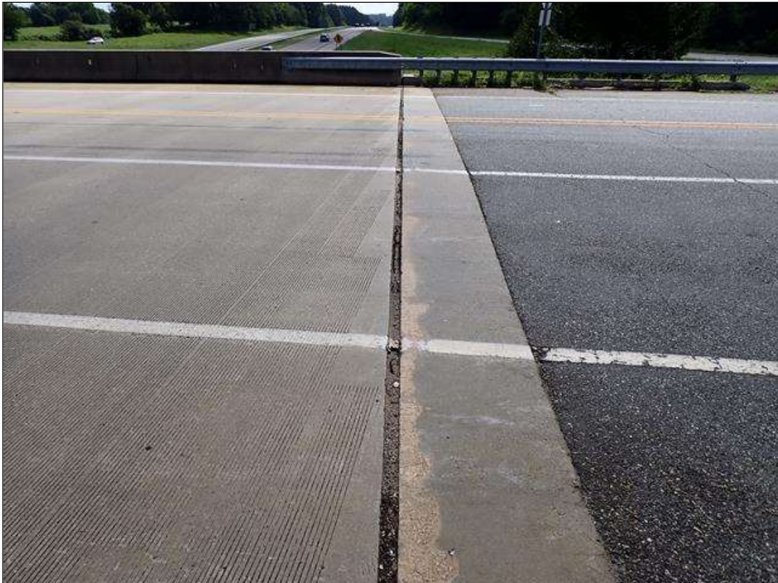
end bent 1 joint
