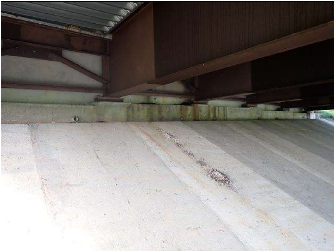
end bent 1 and slope protection
