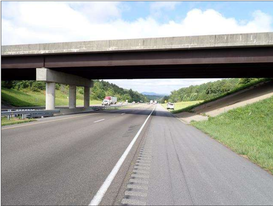
roadway under span 2, looking west
