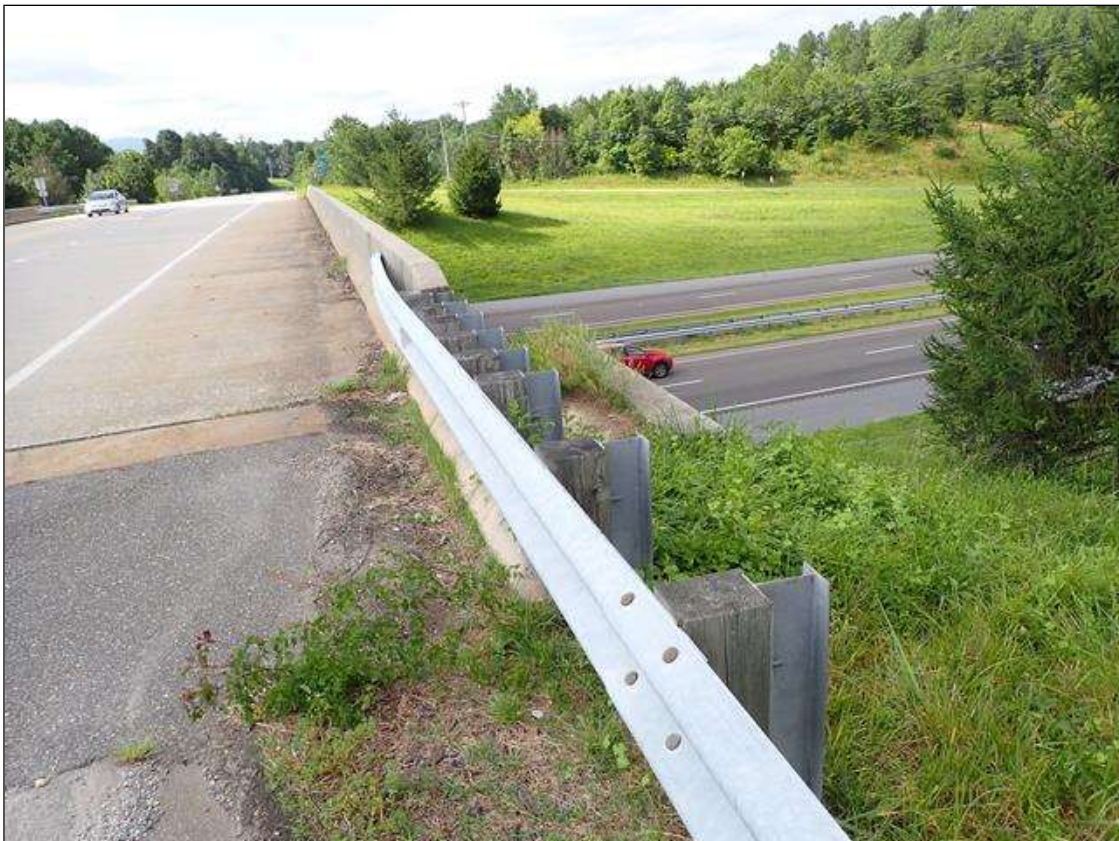
northwest guardrail transition
