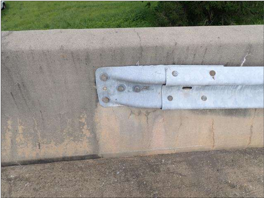
northwest guardrail attachment
