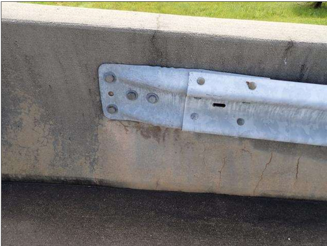
southeast guardrail attachment
