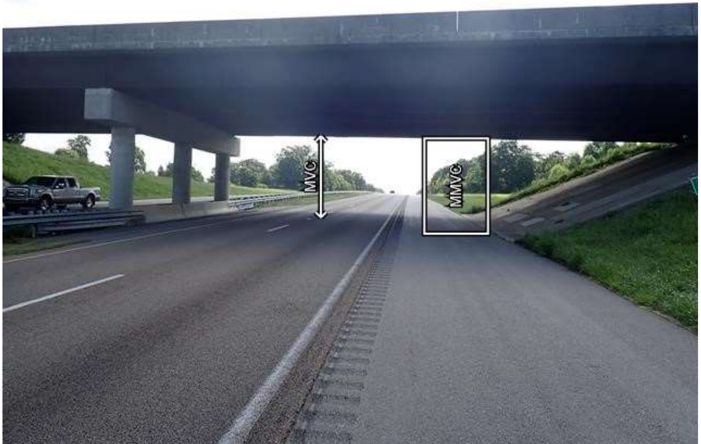
roadway under span 1, looking east
