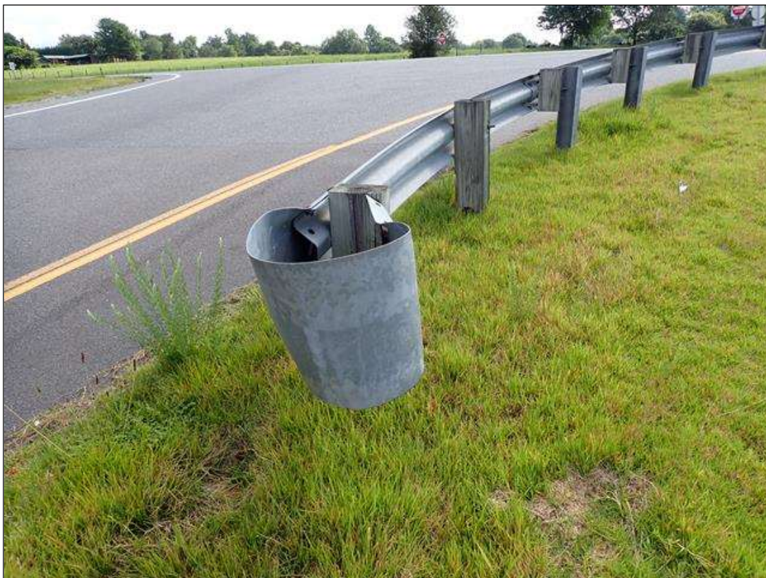
northwest guardrail termination
