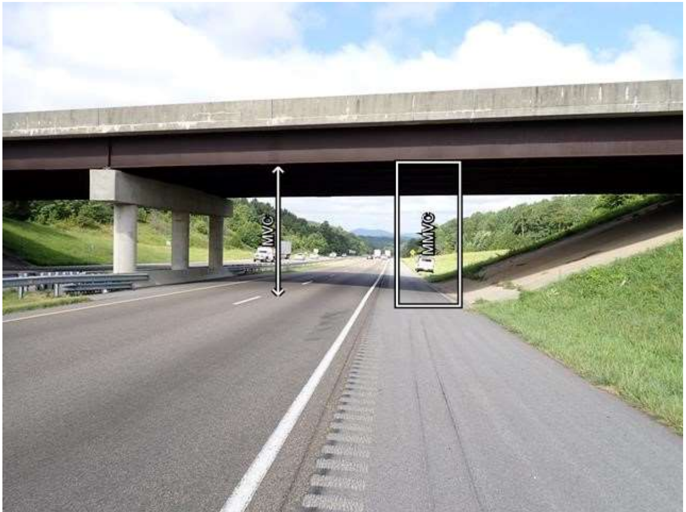
roadway under span 2, looking west
