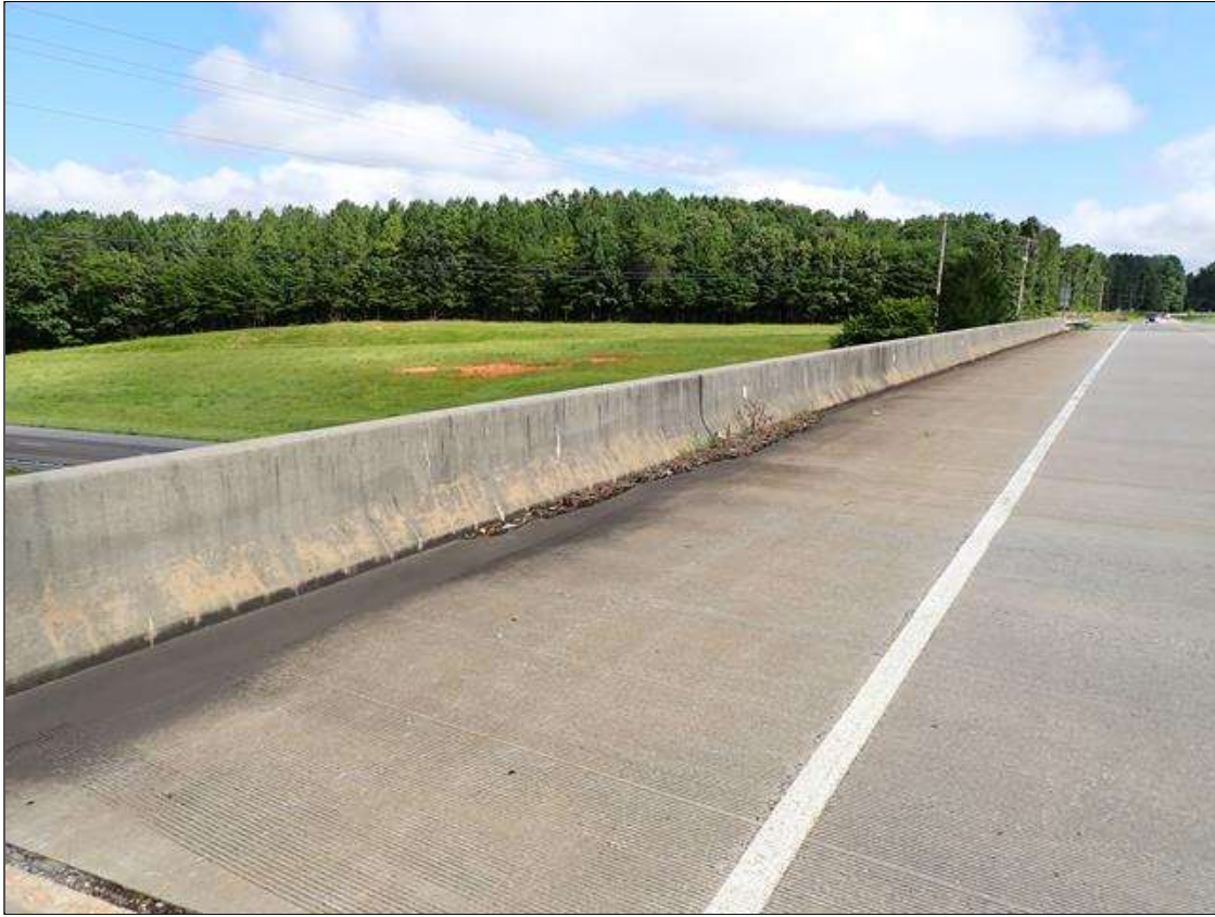
left bridge rail
