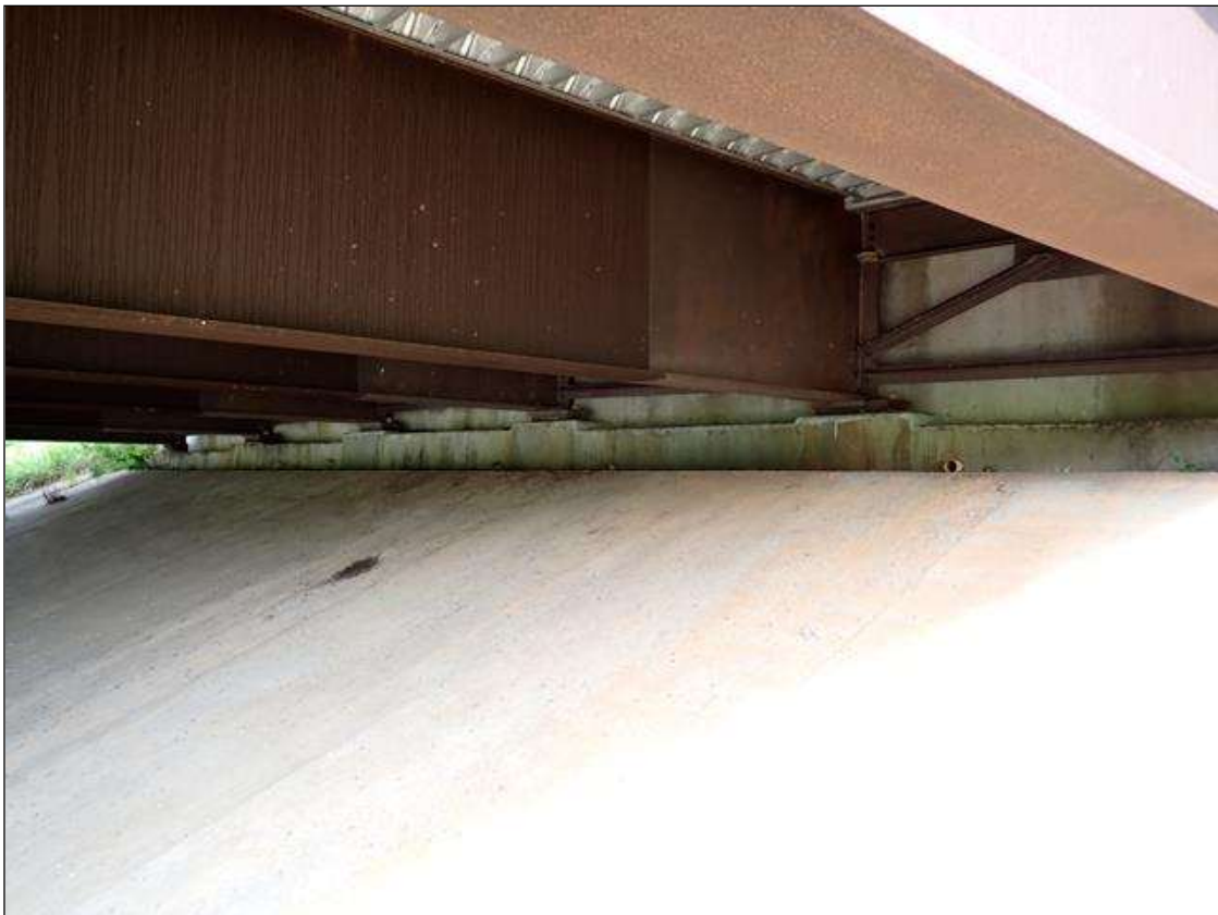
end bent 2 and slope protection
