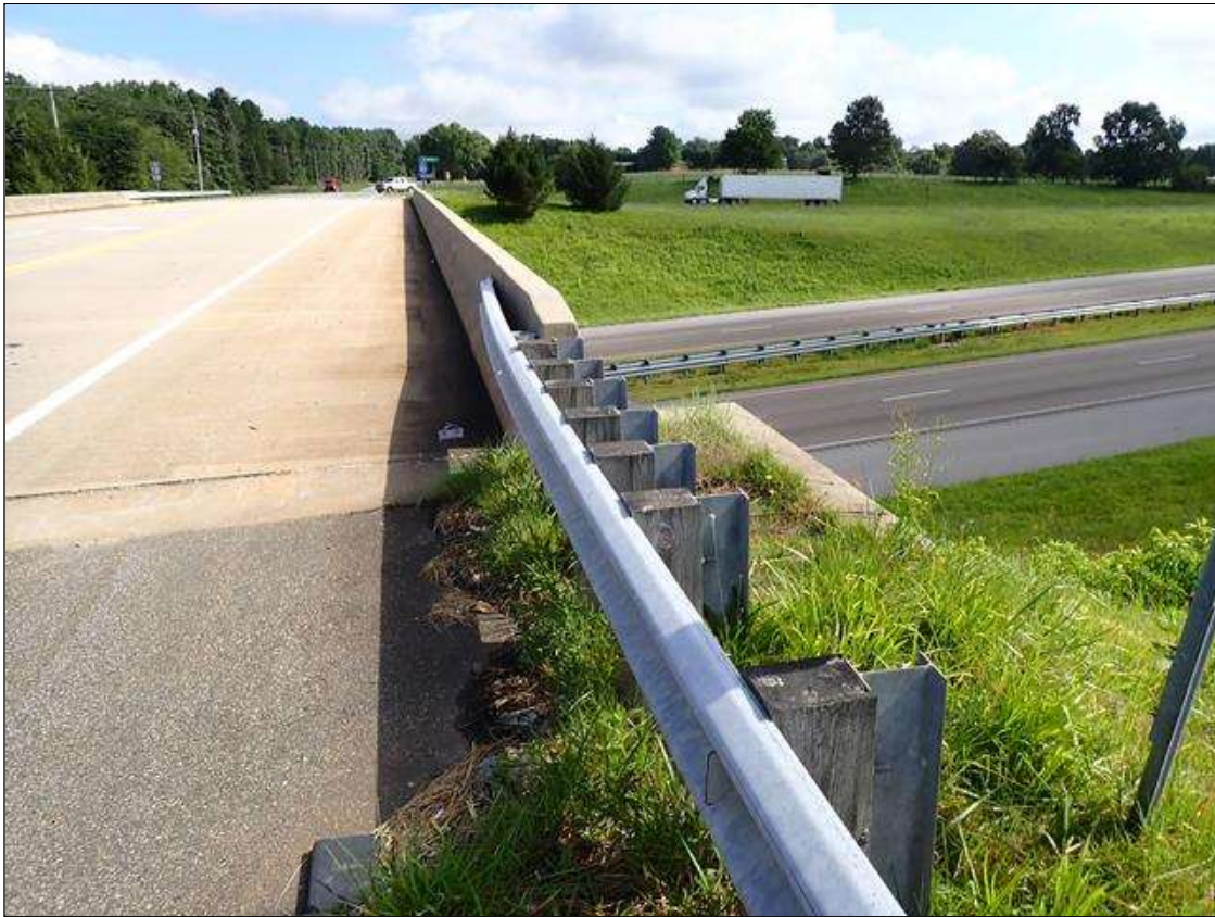
southeast guardrail transition
