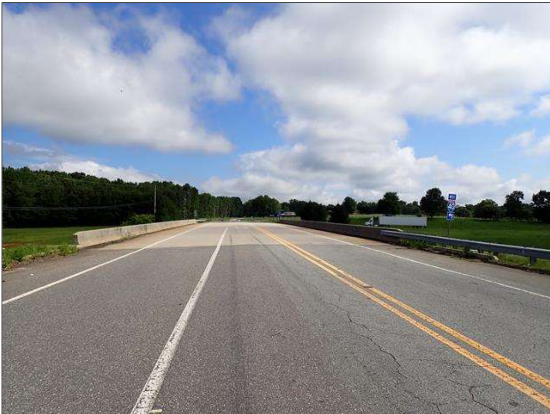
south approach looking north
