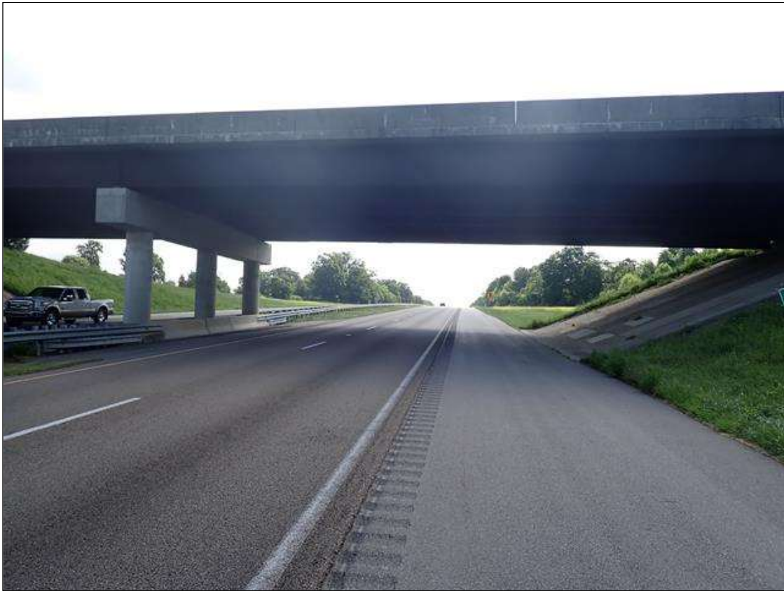
roadway under span 1, looking east
