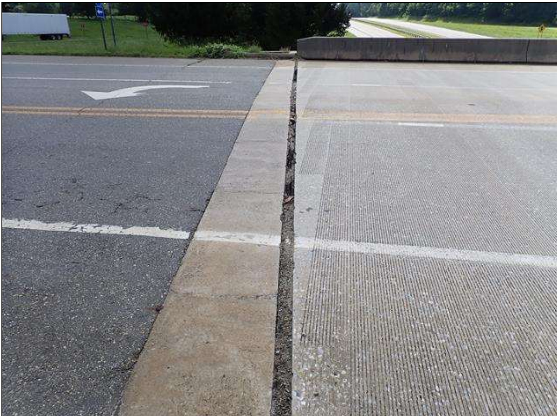
end bent 2 joint
