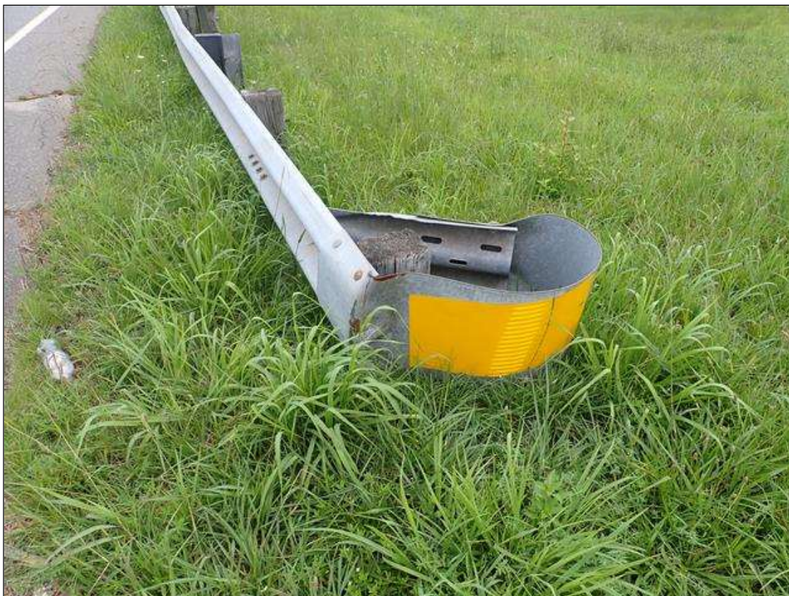
southeast guardrail termination
