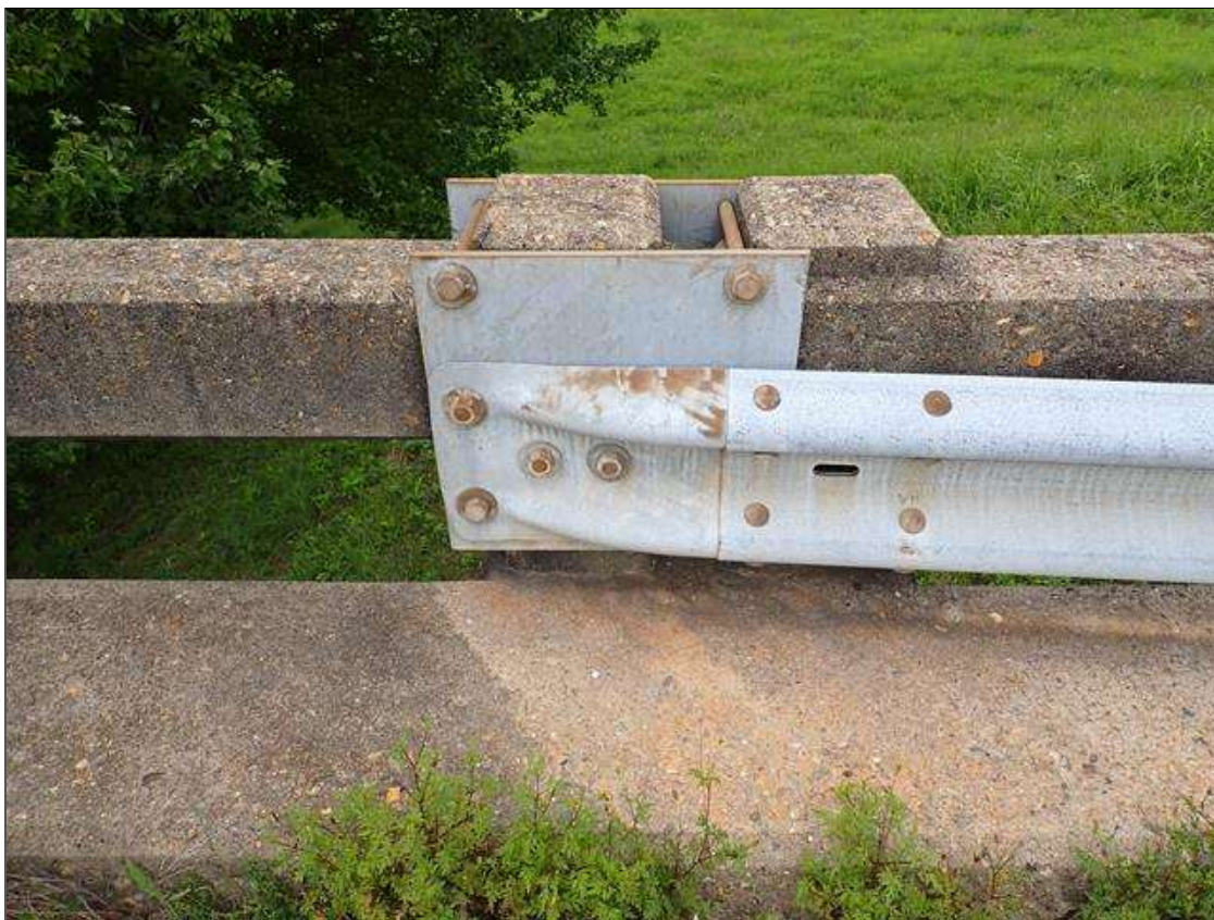
northwest guardrail attachment
