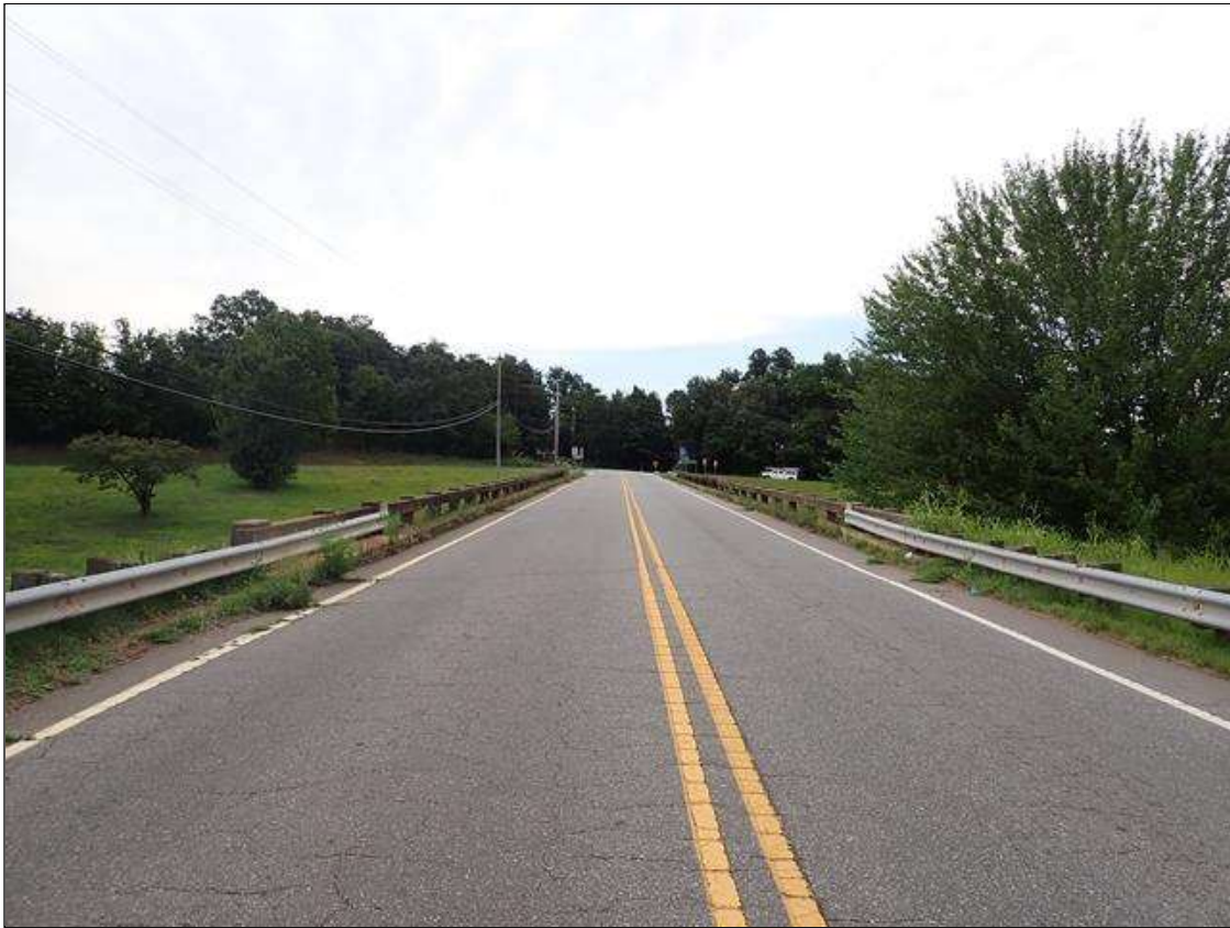
north approach looking south
