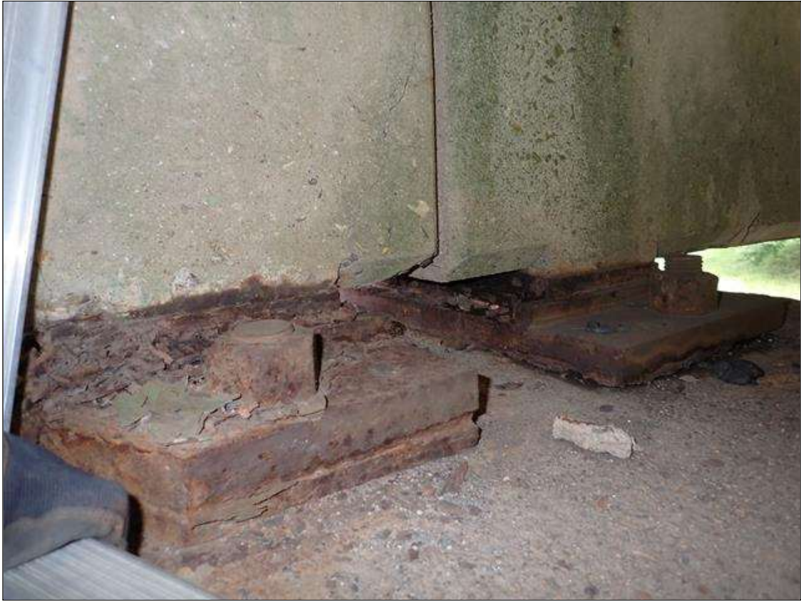
interior bearing assembly
