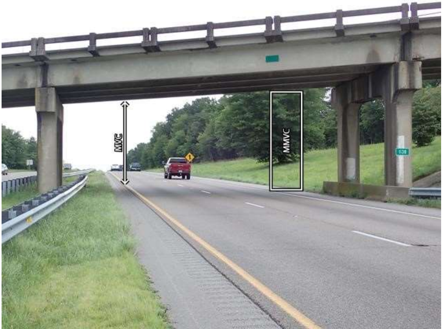
roadway under span 3, looking east
