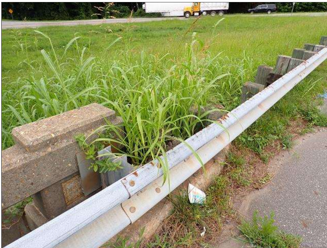
northwest guardrail transition
