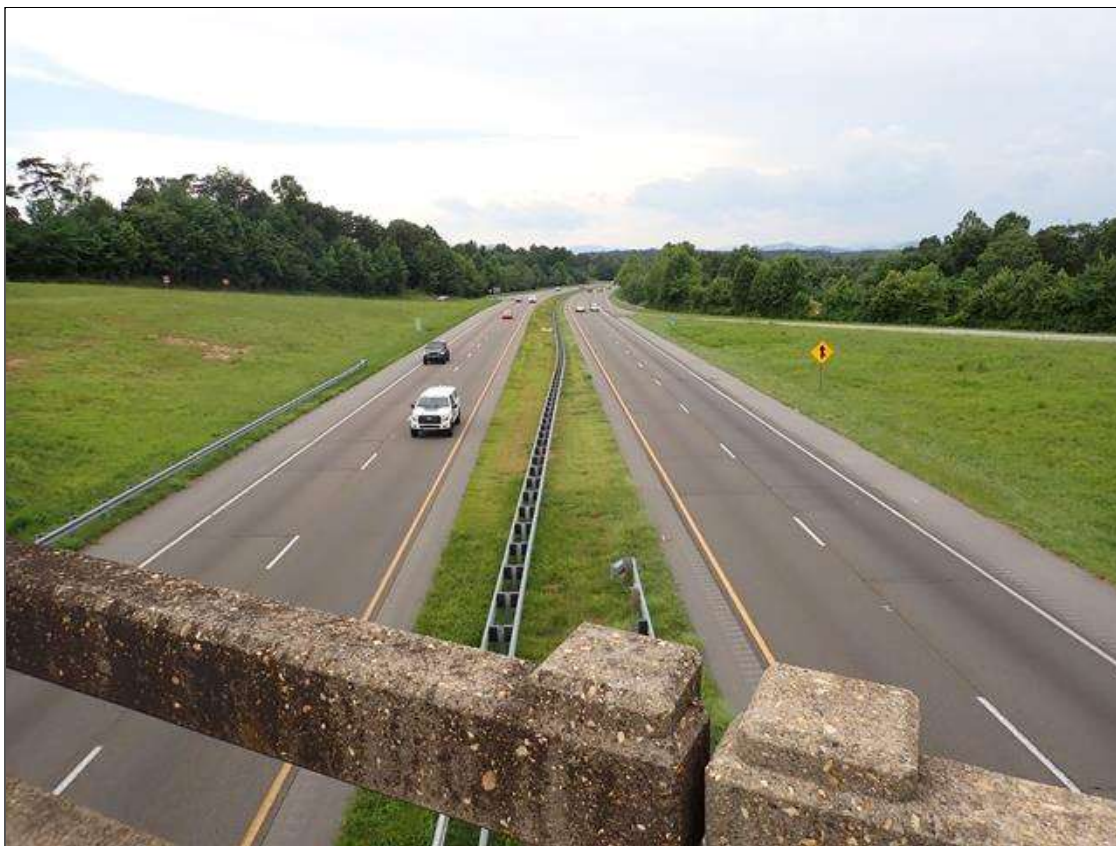
roadway looking west
