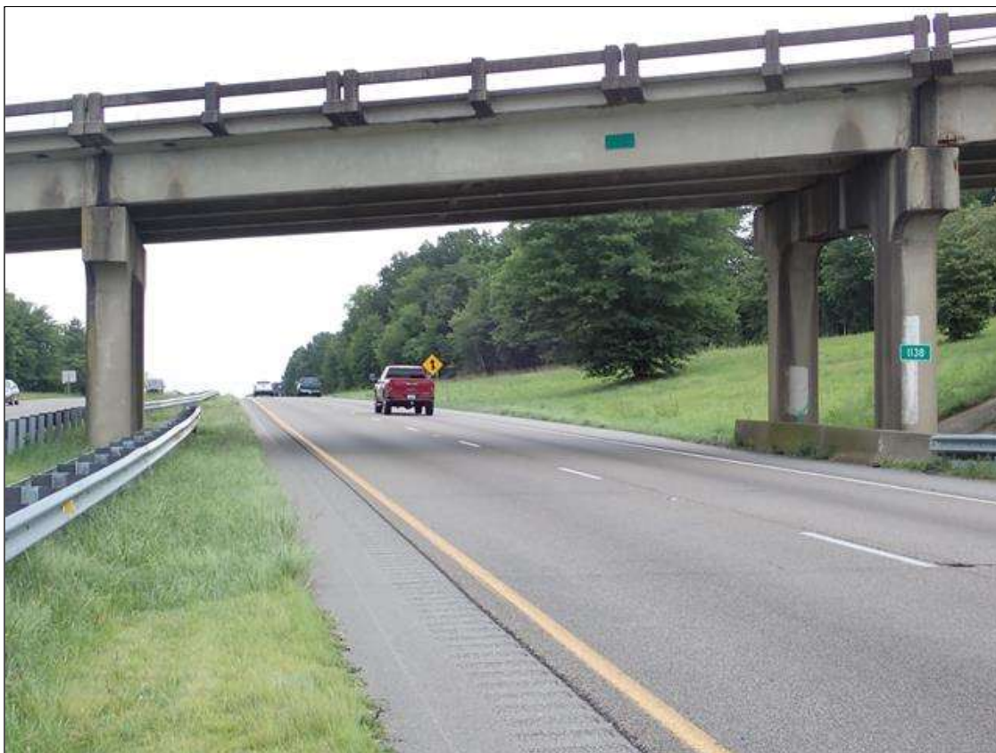
roadway under span 3, looking east (I-40 eastbound)
