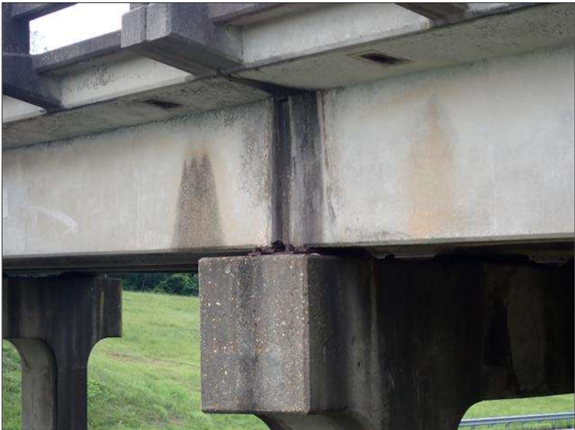
beams over bent
