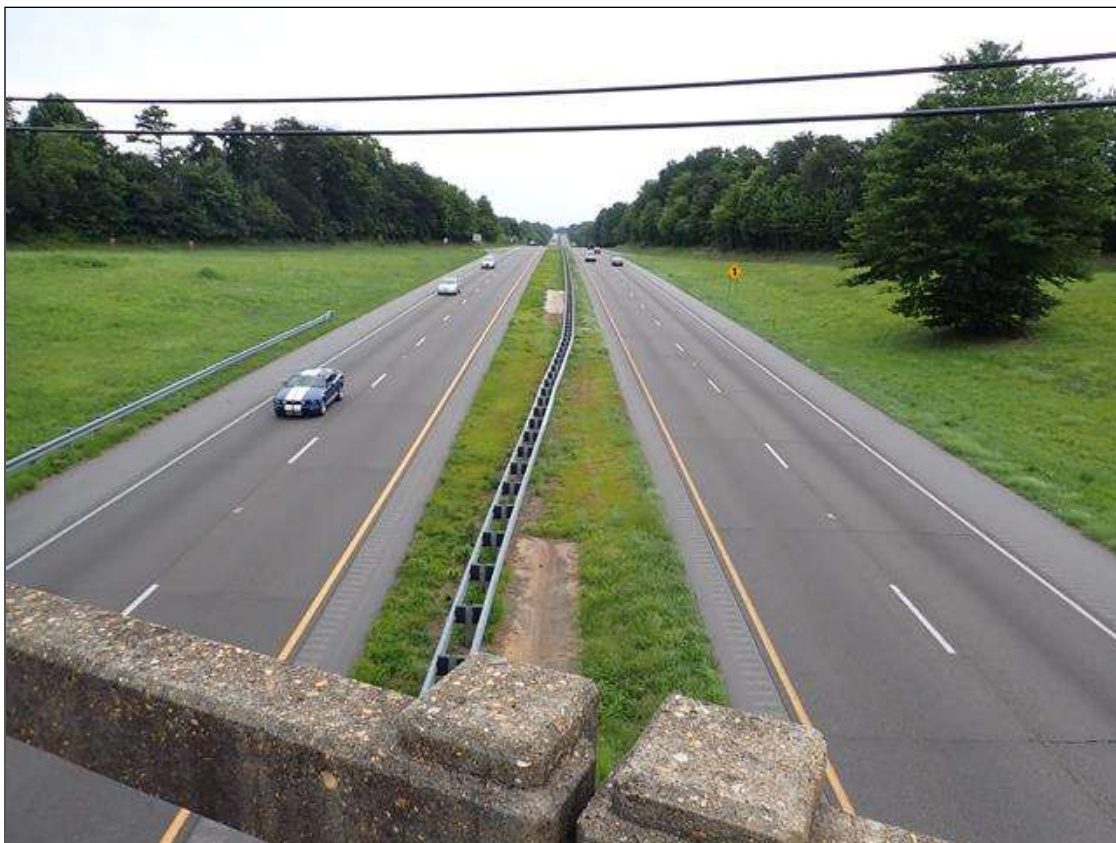
roadway looking east
