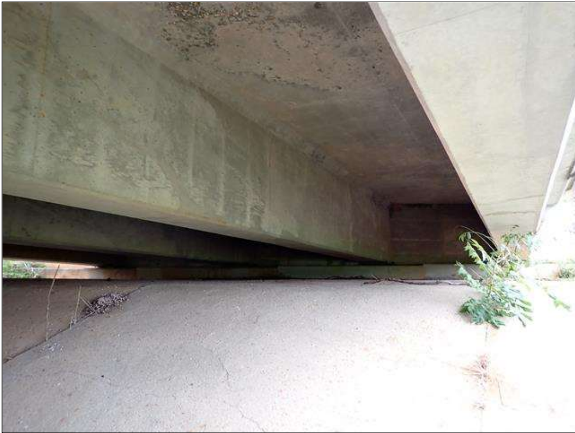
end bent 1 and slope protection
