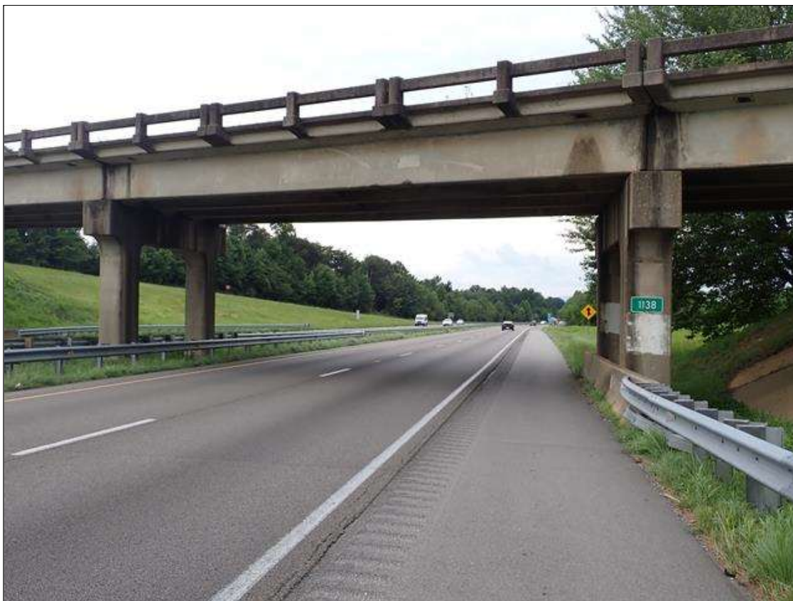
roadway under span 4, looking west (I-40 westbound)
