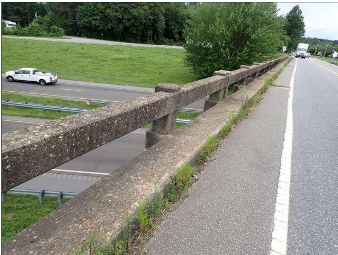
left bridge rail
