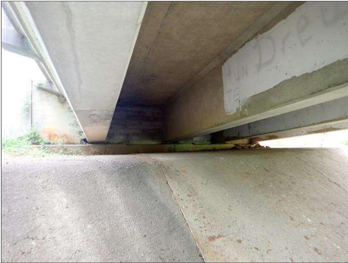
end bent 2 and slope protection
