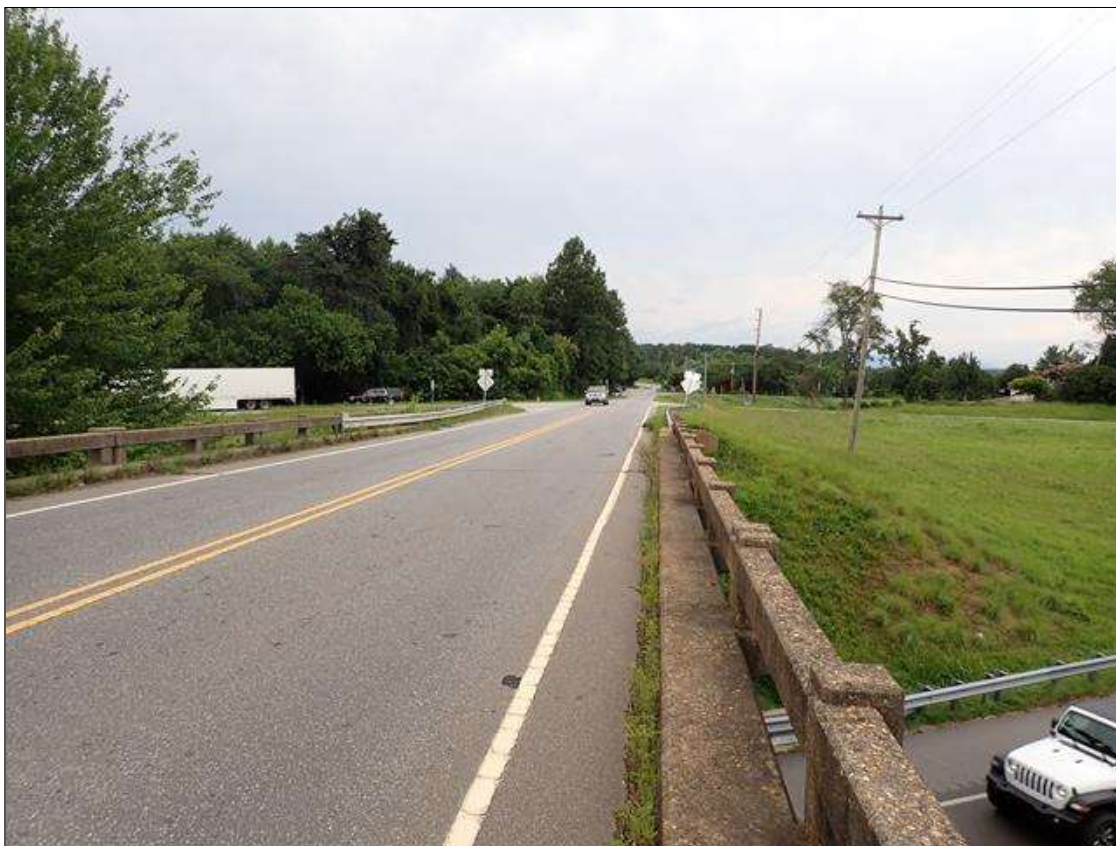
north approach looking north
