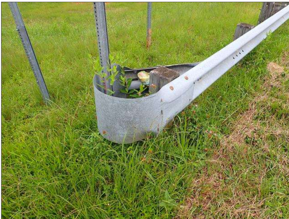
southwest guardrail termination
