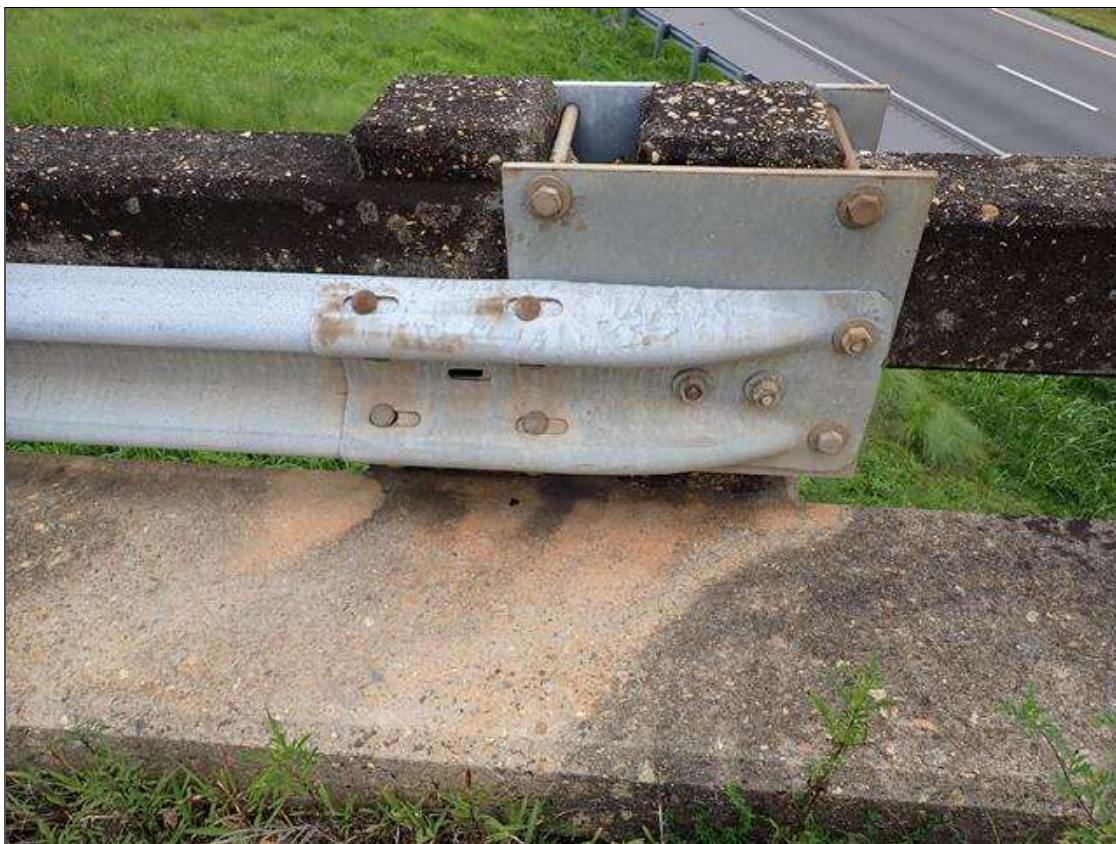
northeast guardrail attachment
