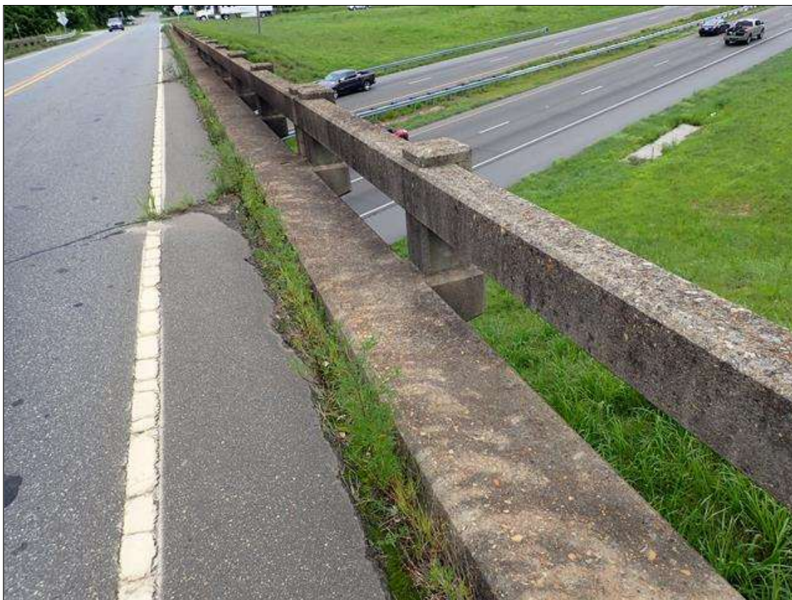
right bridge rail
