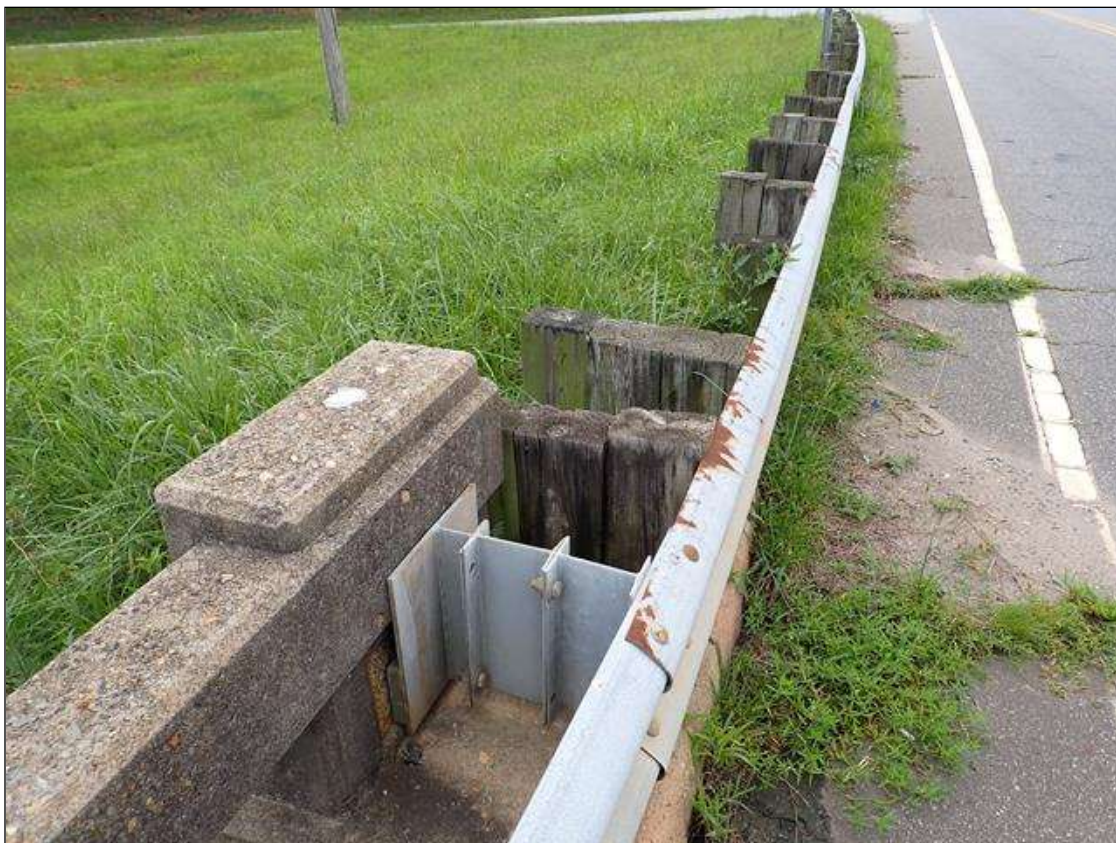
southeast guardrail transition
