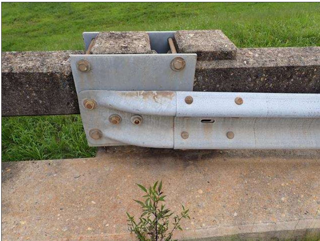
southeast guardrail attachment
