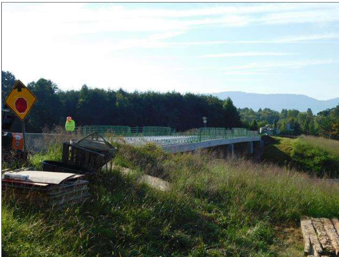
BRIDGE IS UNDER CONSTRUCTION AND CLOSED TO TRAFFIC
