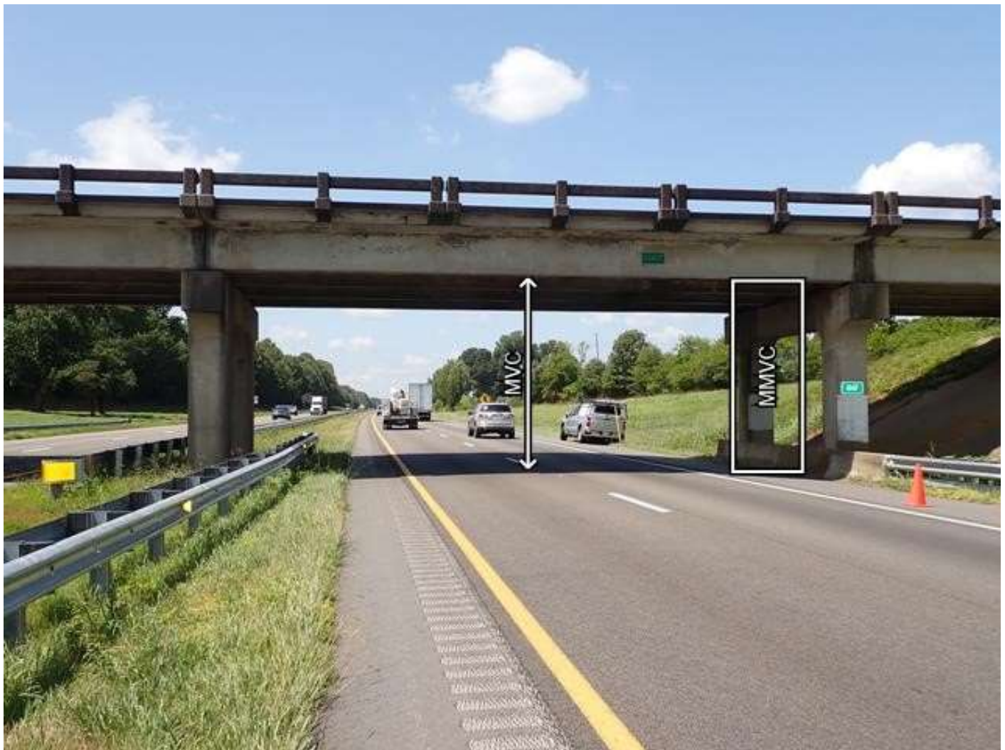
span 3 vertical clearance looking West
