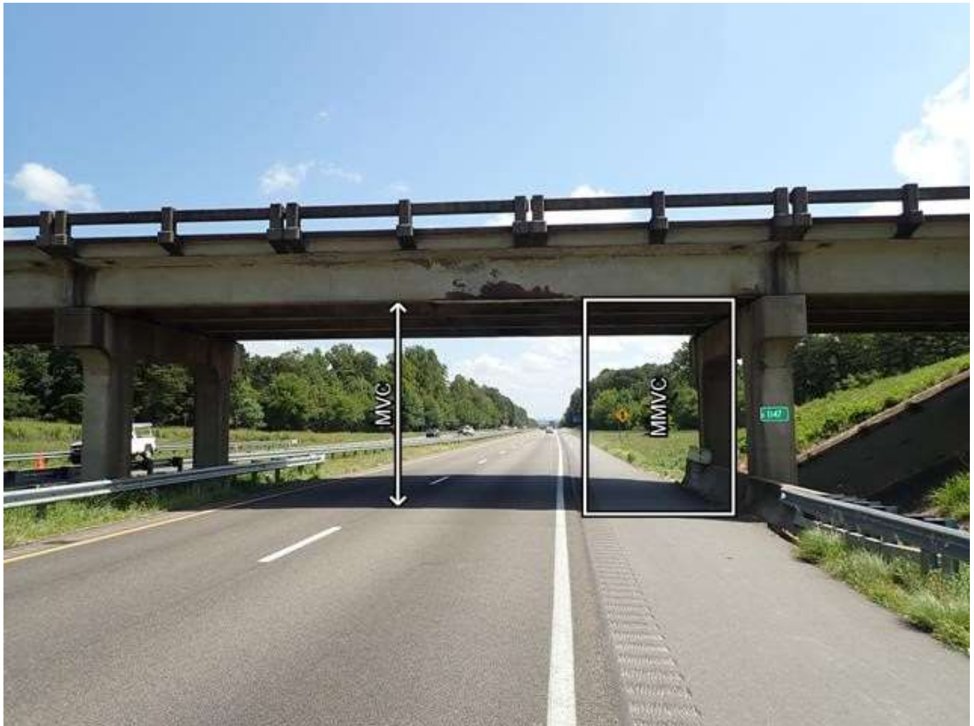
span 2 vertical clearance looking East
