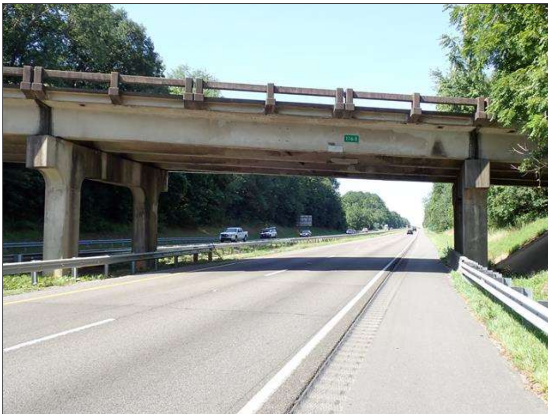
roadway under span 4, looking west
