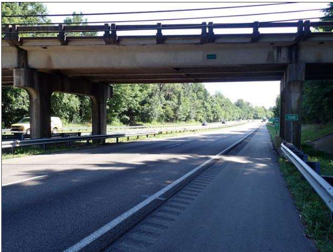
roadway under span 3, looking east
