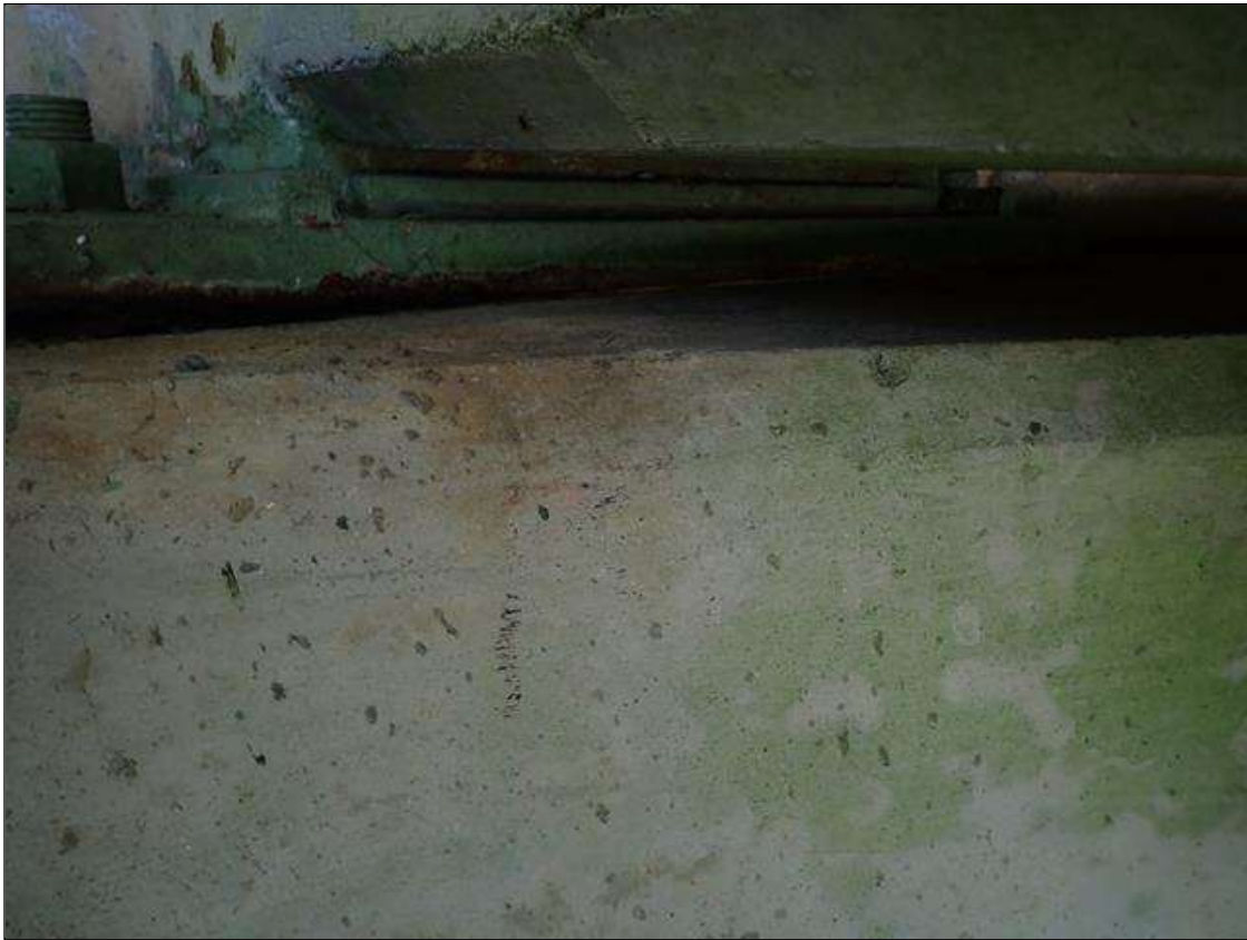
end bearing assembly
