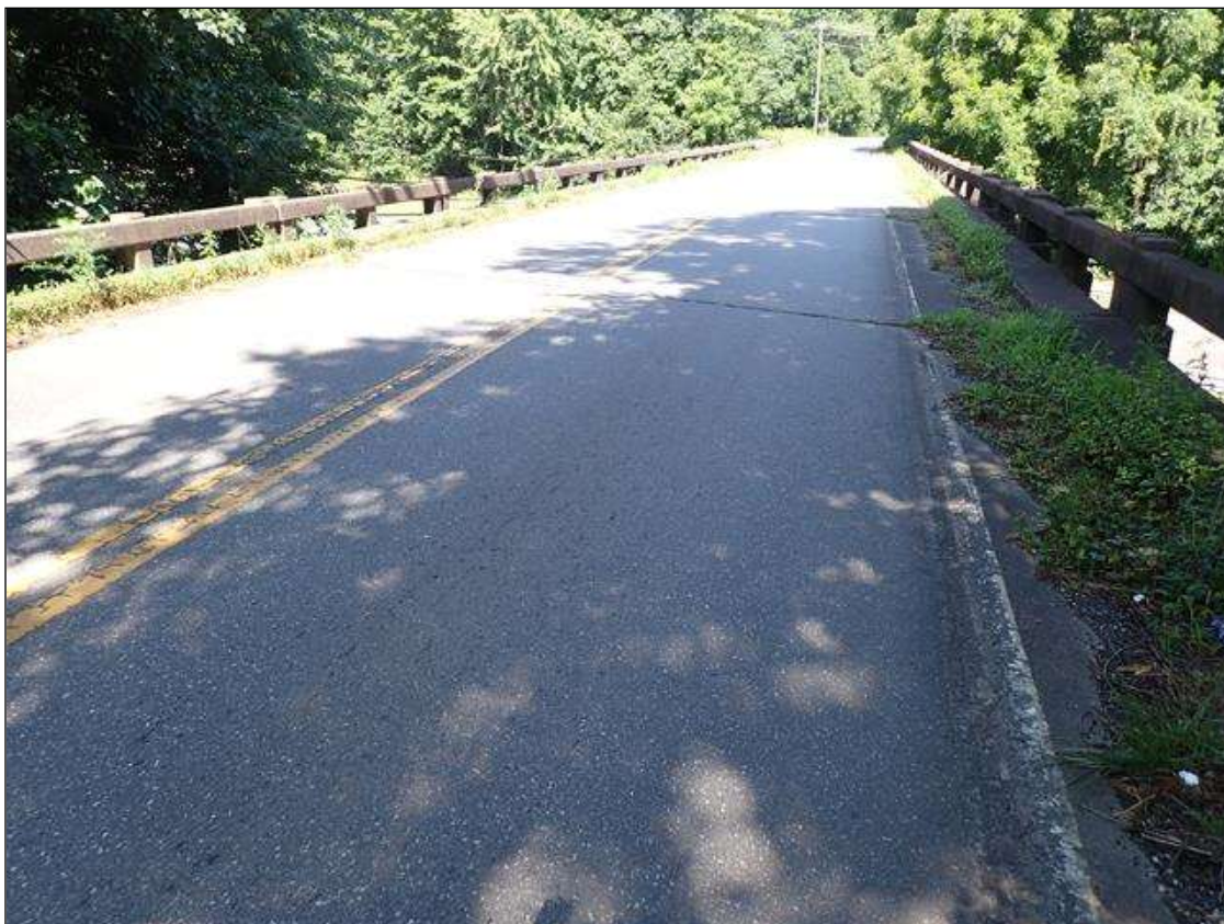
asphalt wearing surface
