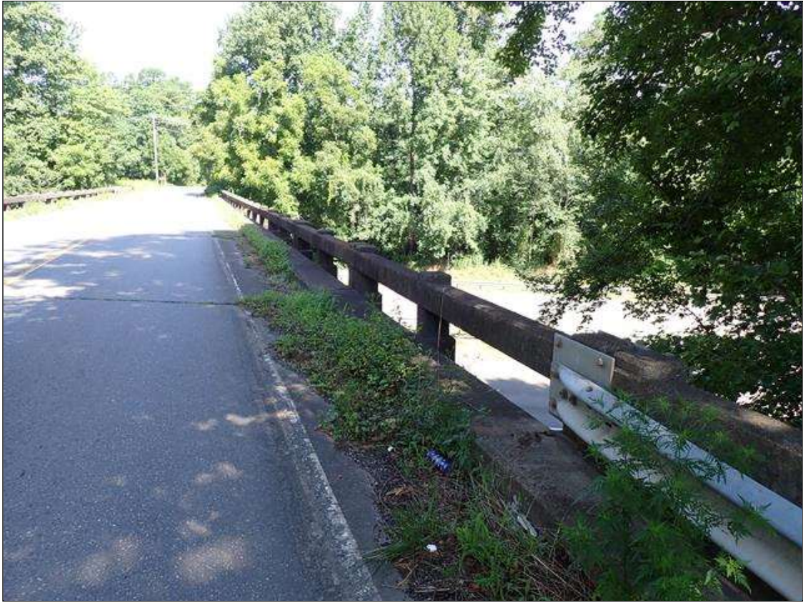
right bridge rail
