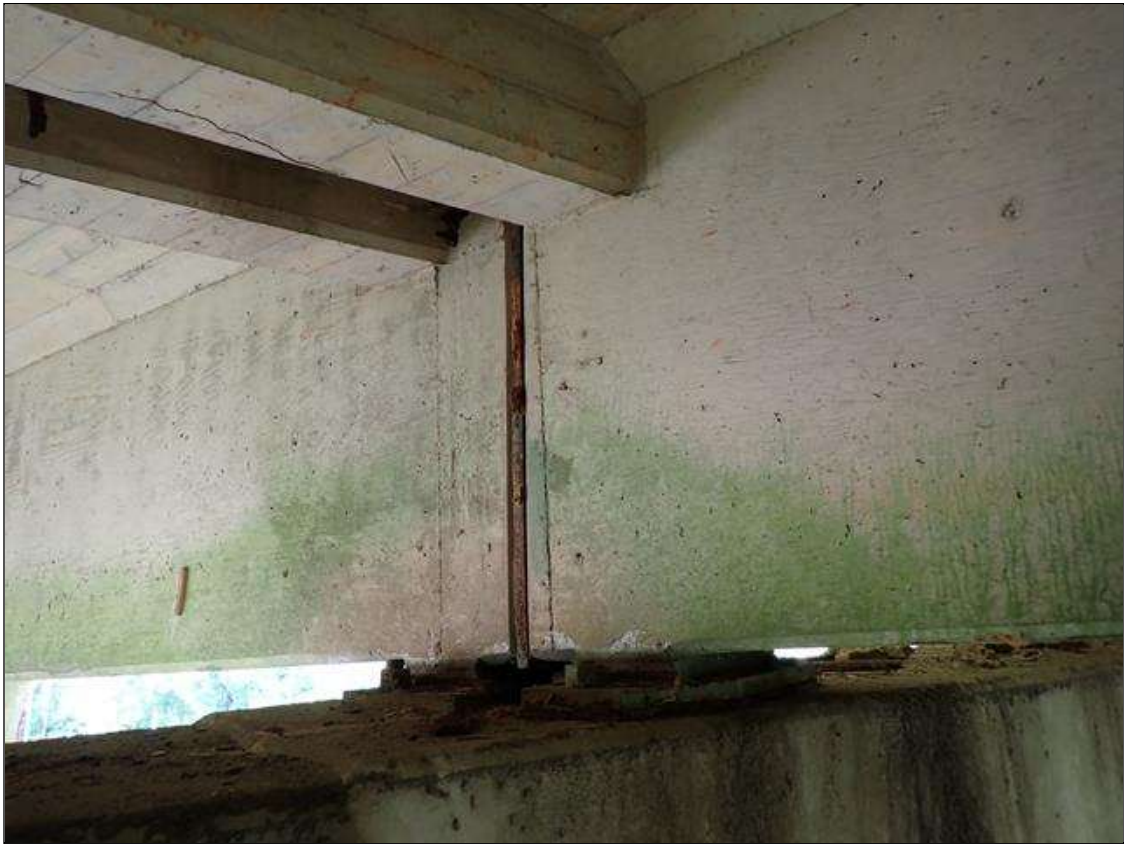
beams over bent
