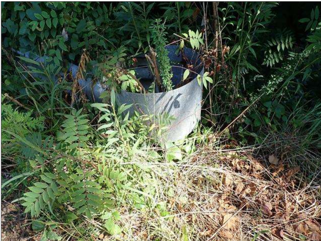
southeast guardrail termination
