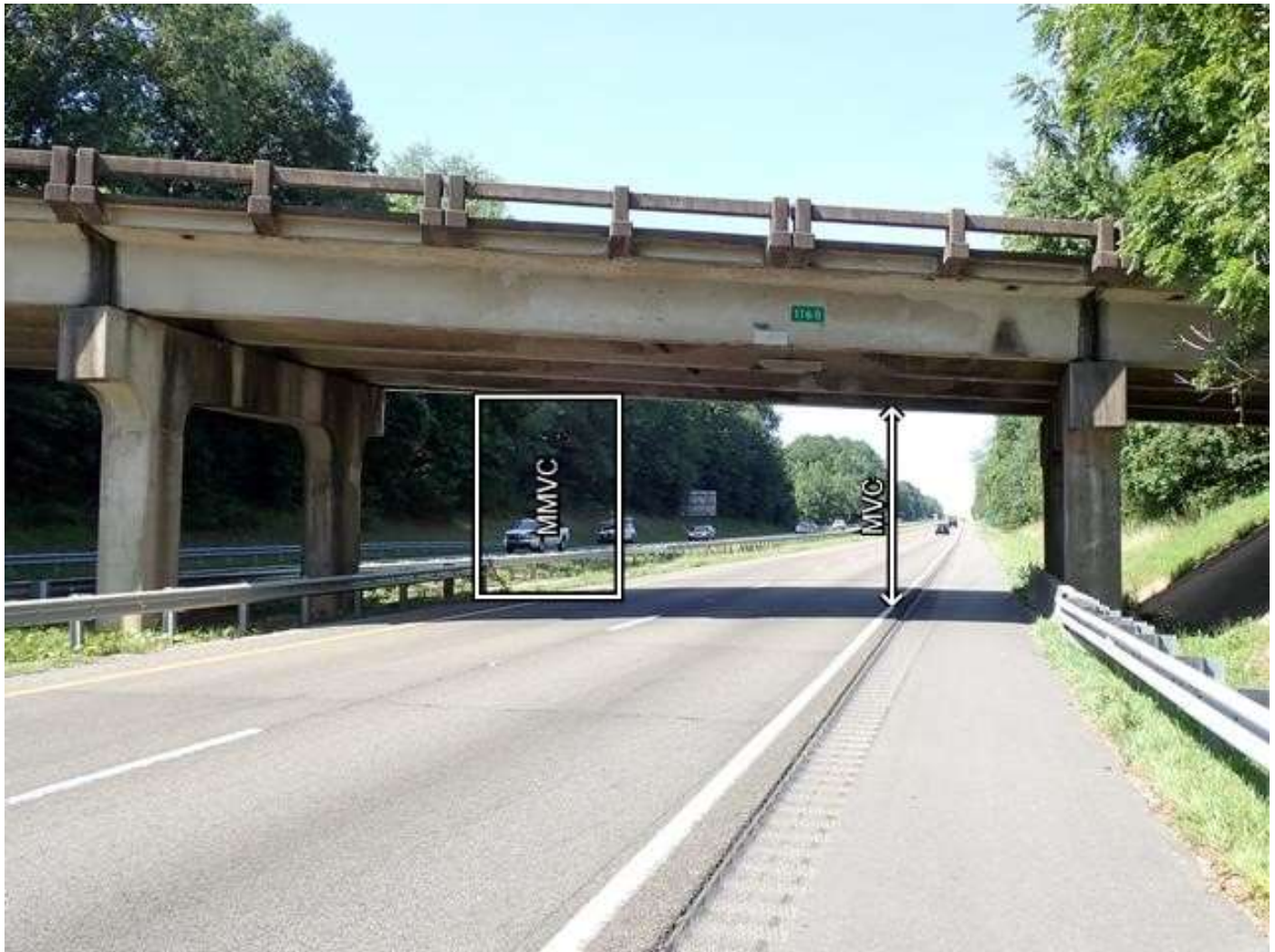
roadway under span 4, looking west
