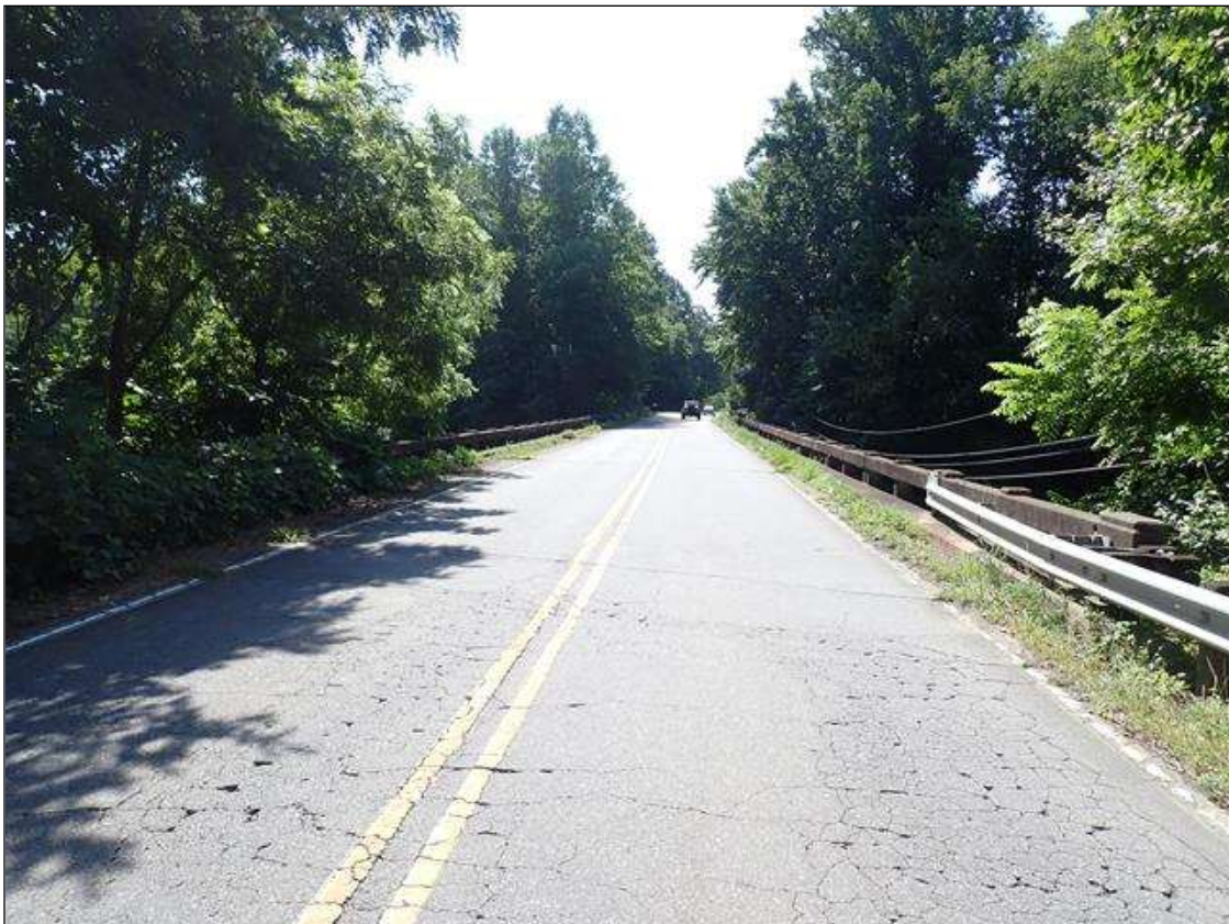
north approach looking south
