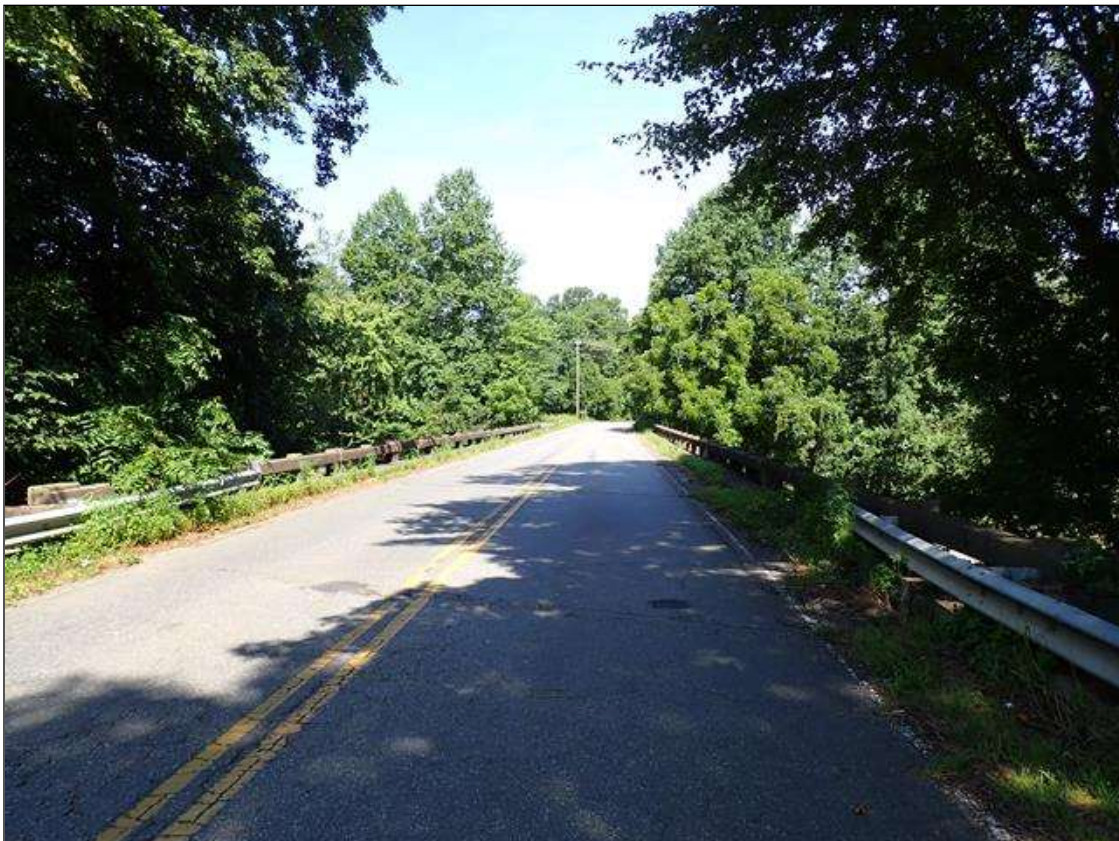
south approach looking north
