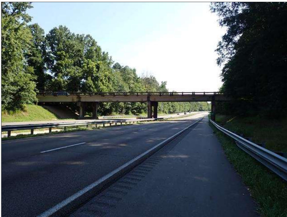
west profile looking east
