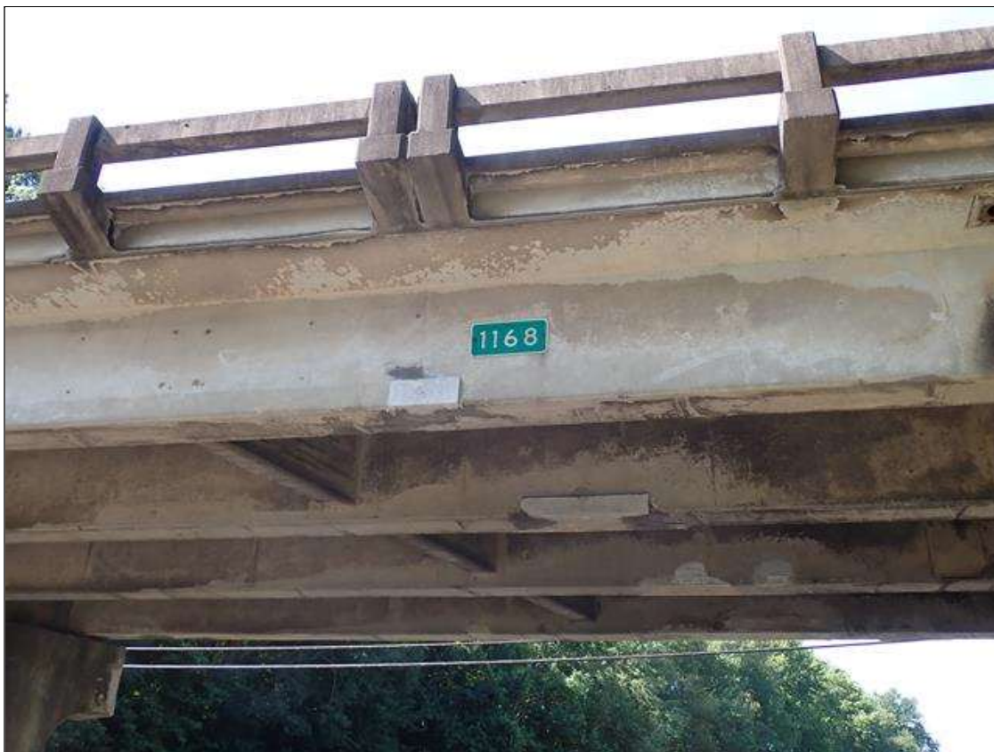
span 4 beam 4 route sign closeup
