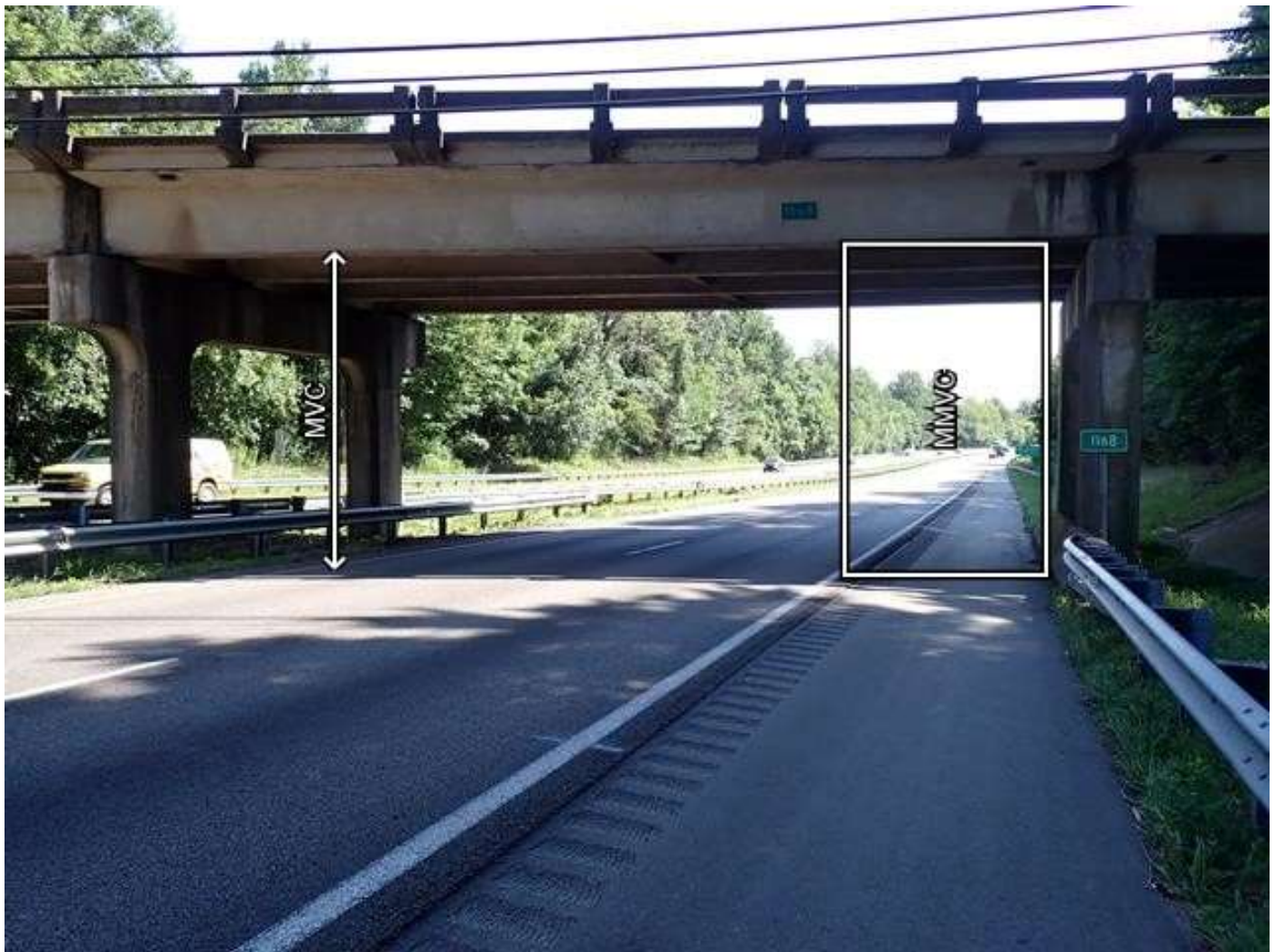
roadway under span 3, looking east
