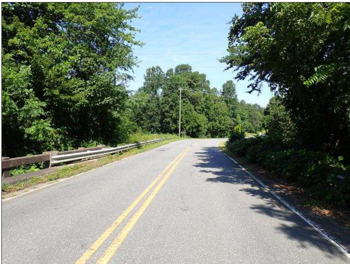
north approach looking north
