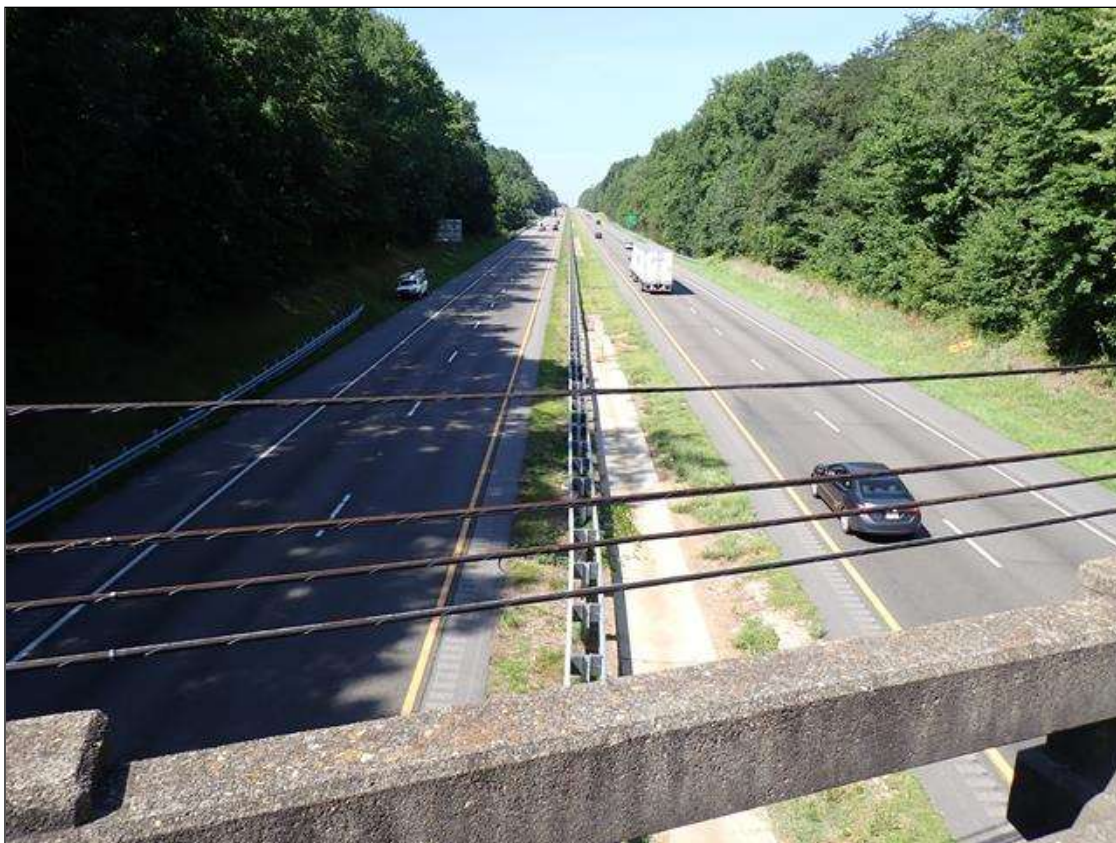
roadway looking west
