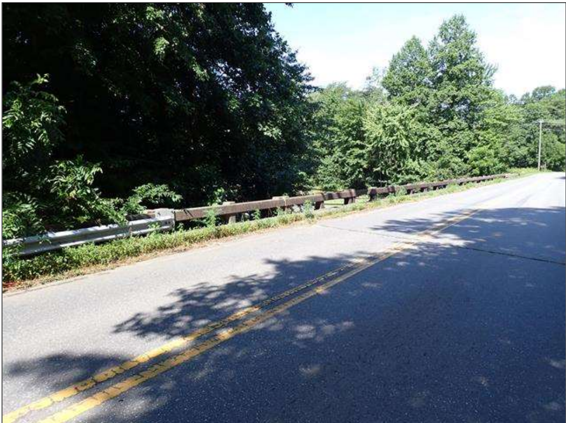
left bridge rail
