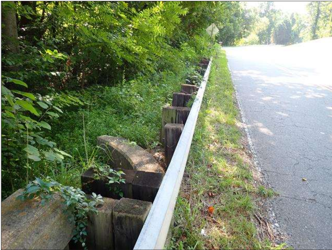
southeast guardrail transition
