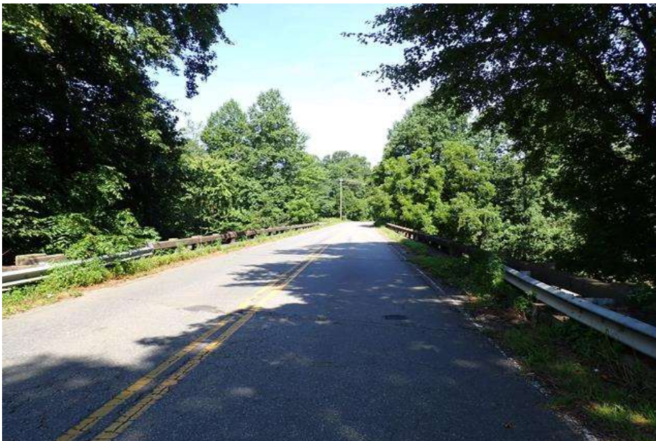
south approach looking north
