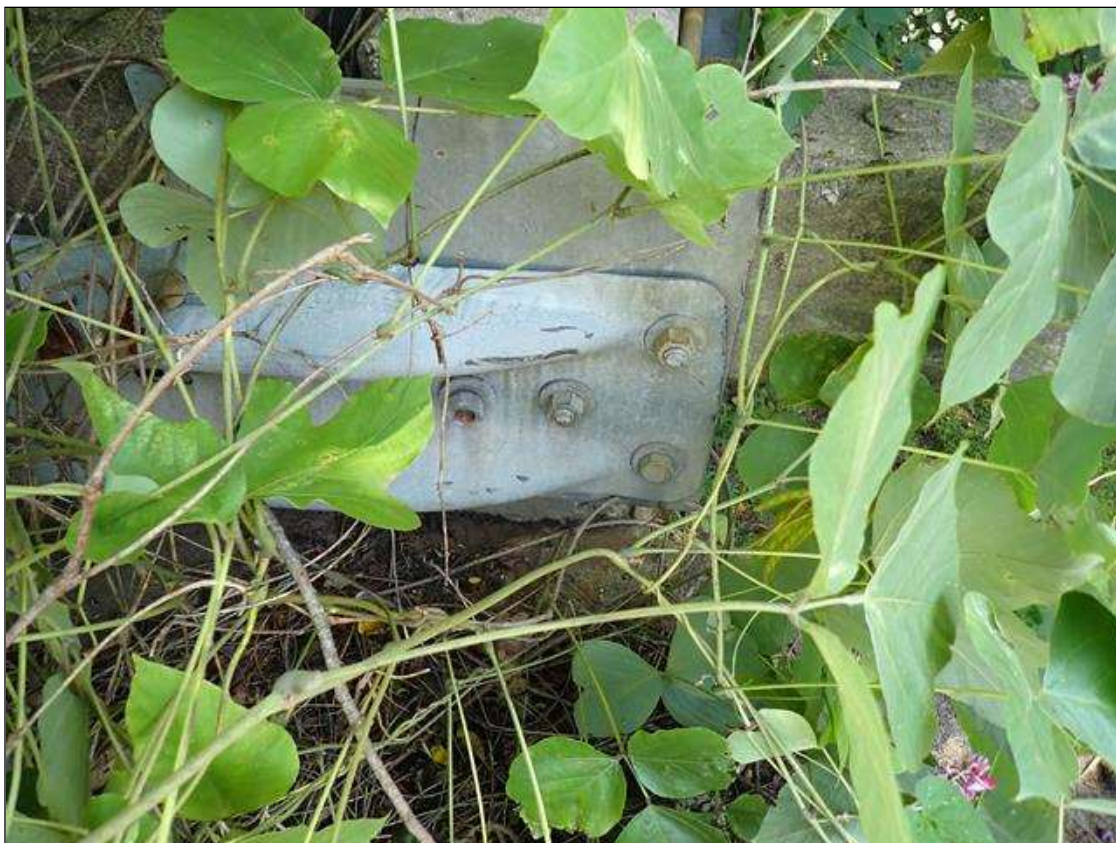
northeast guardrail attachment
