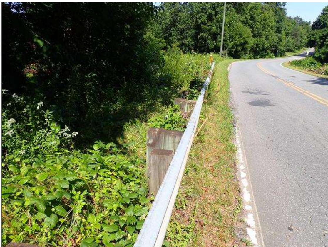
northwest guardrail transition
