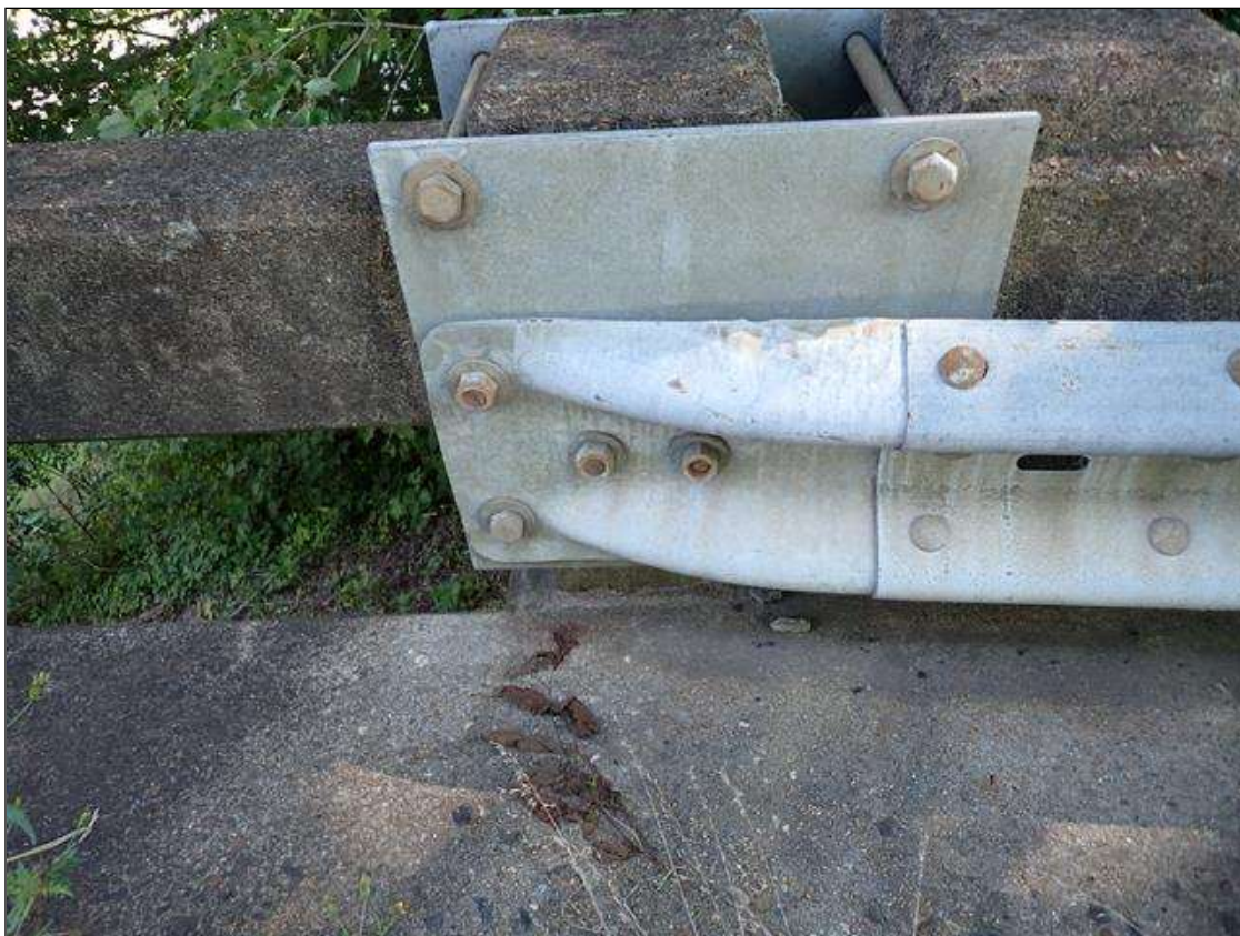
southeast guardrail attachment
