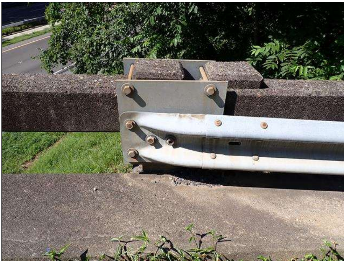
northwest guardrail attachment
