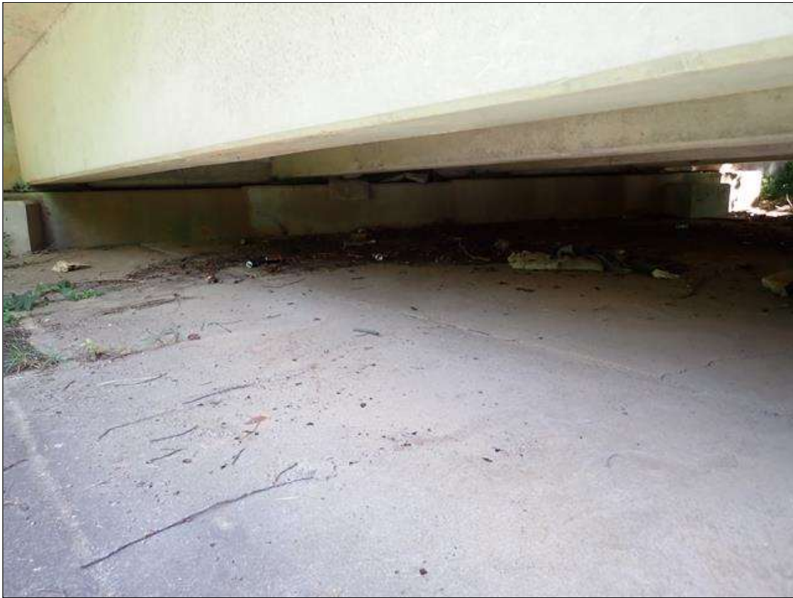
end bent 2 and slope protection
