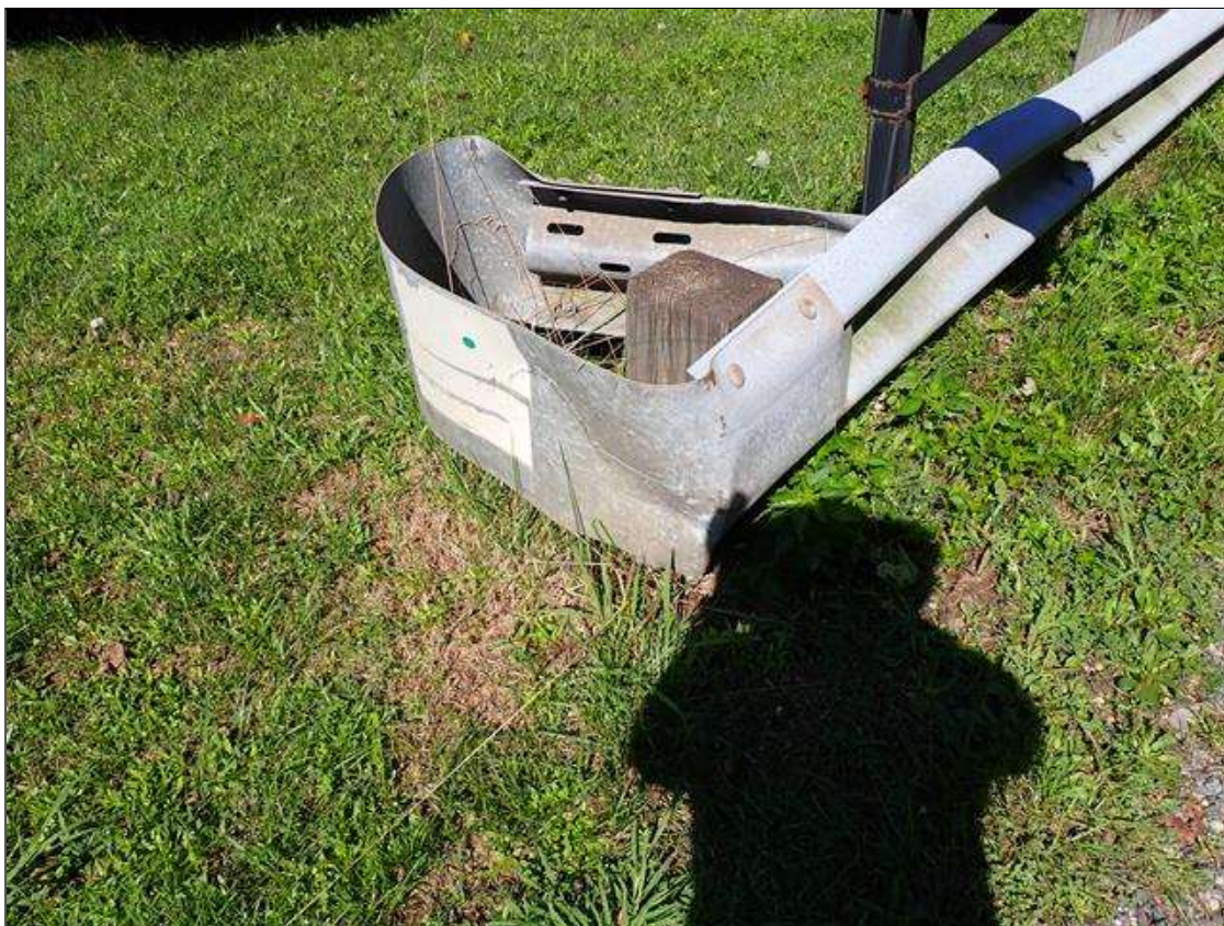
southwest guardrail termination
