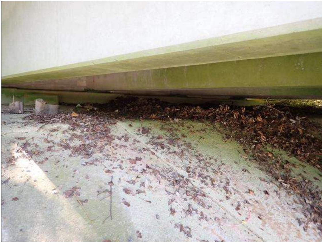
end bent 1 and slope protection
