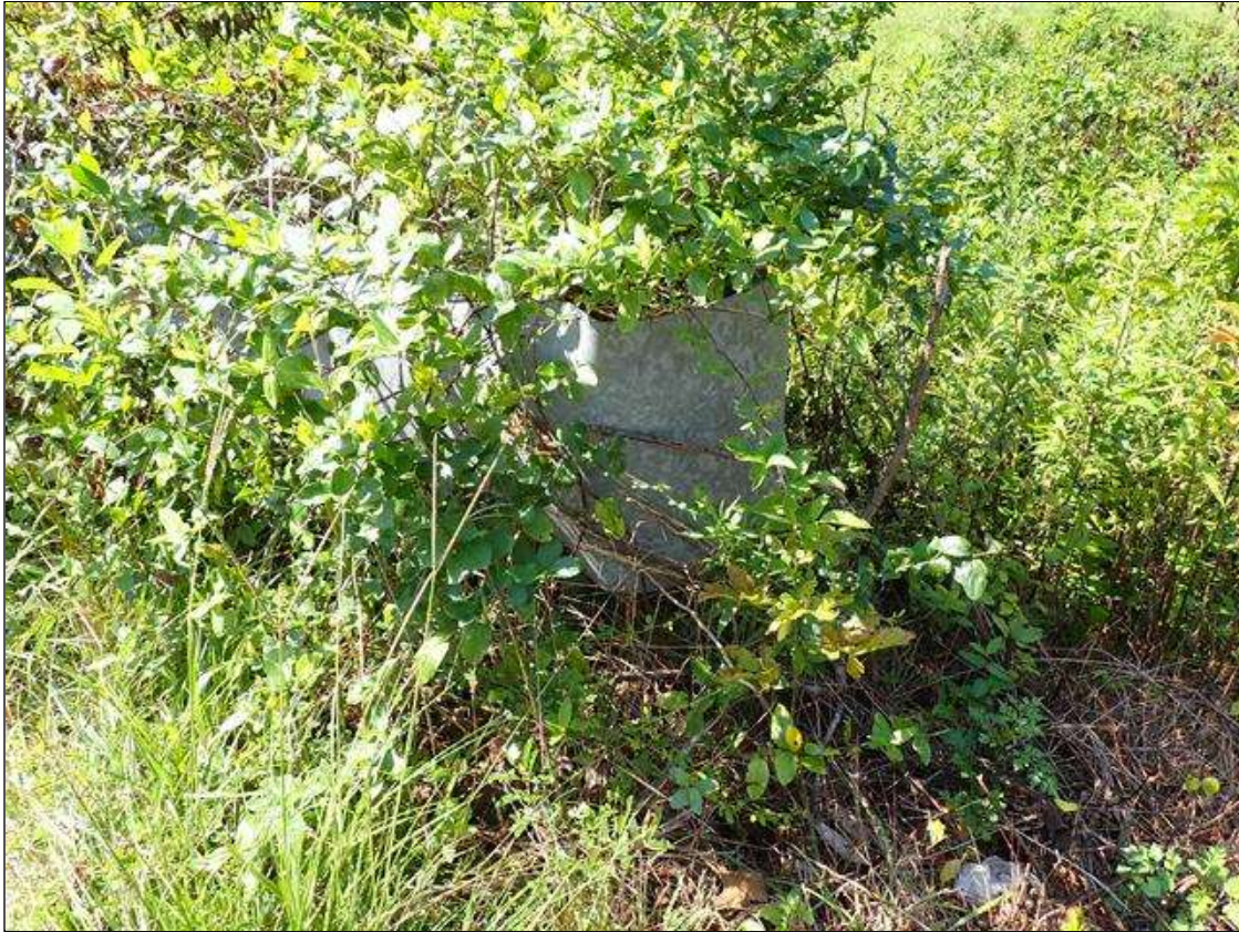
northwest guardrail termination
