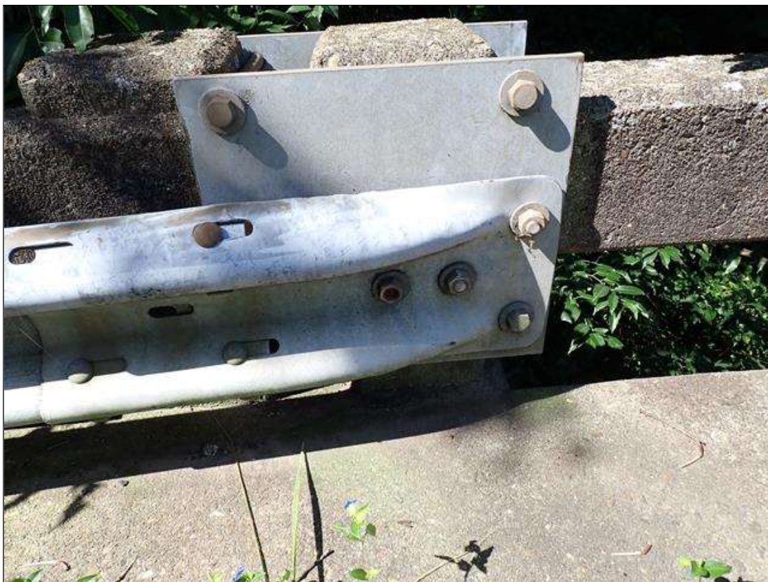
southwest guardrail attachment
