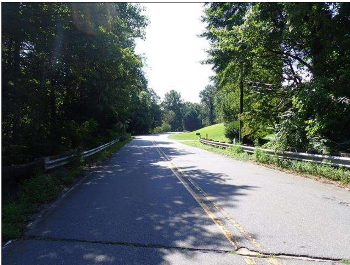
south approach looking south
