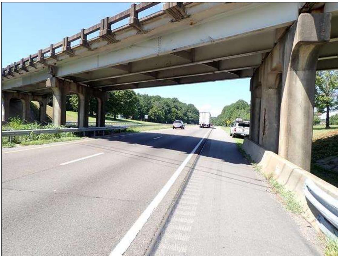
roadway under span 3, looking west (I-40 westbound)
