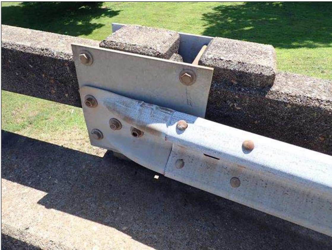
southeast guardrail attachment
