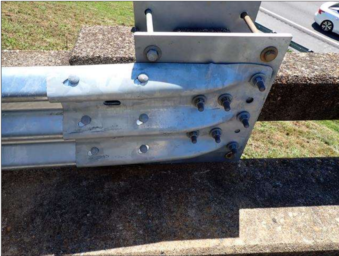
northeast guardrail attachment
