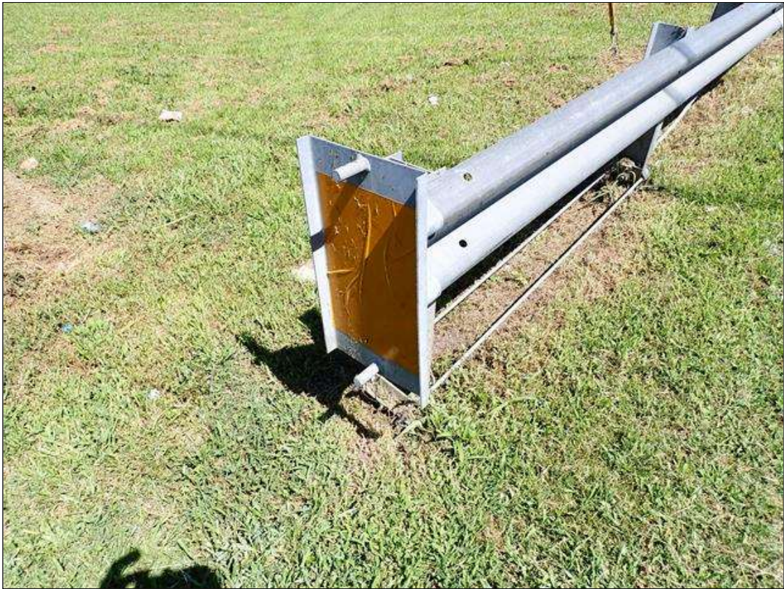
southwest guardrail termination
