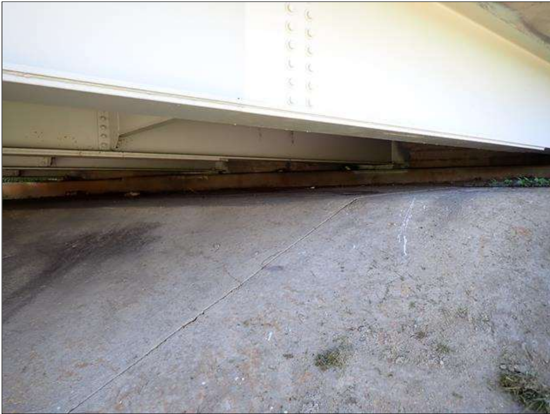
end bent 1 and slope protection
