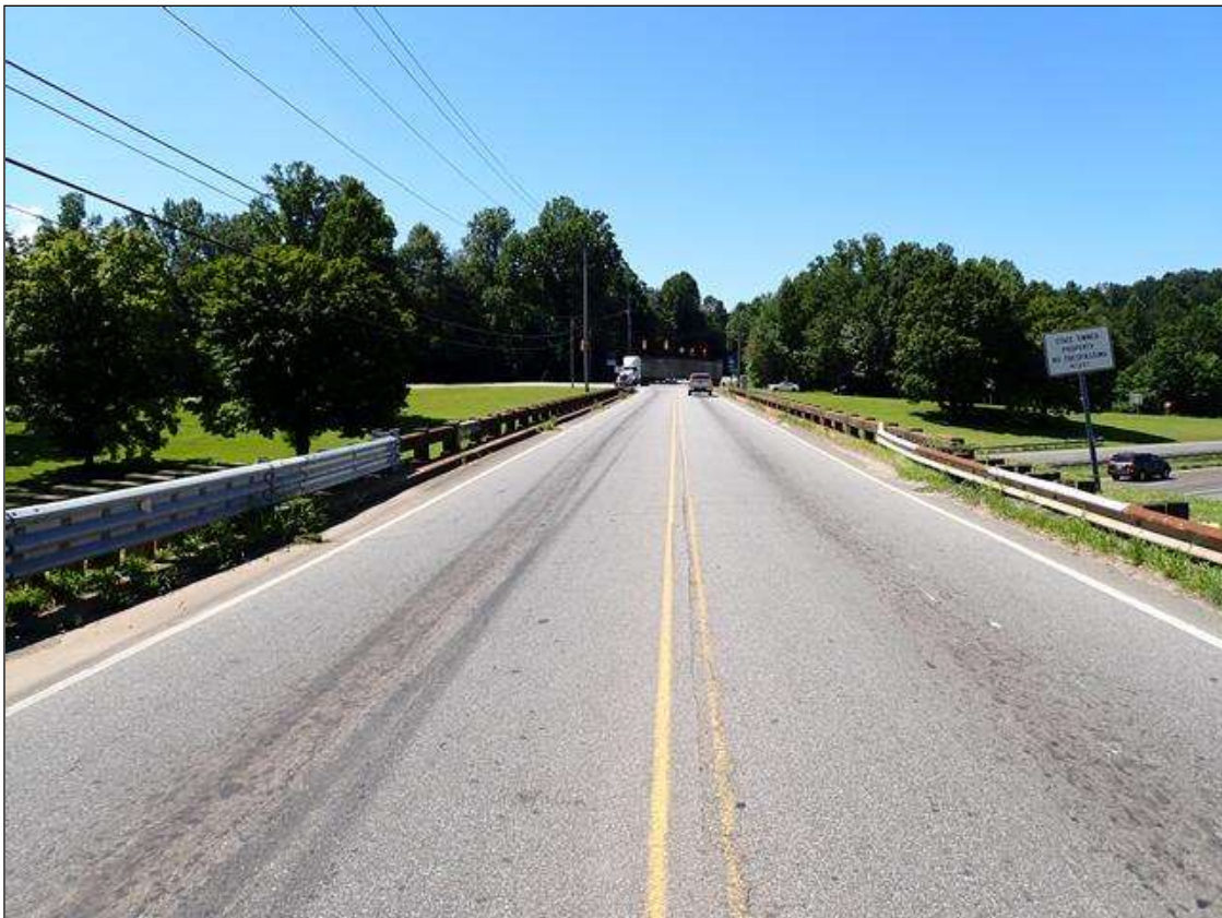
north approach looking south
