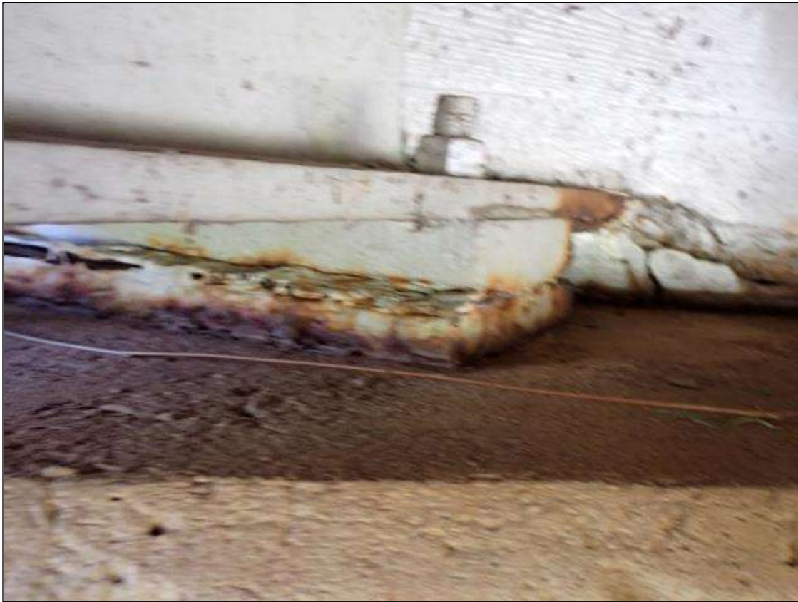
end bearing assembly
