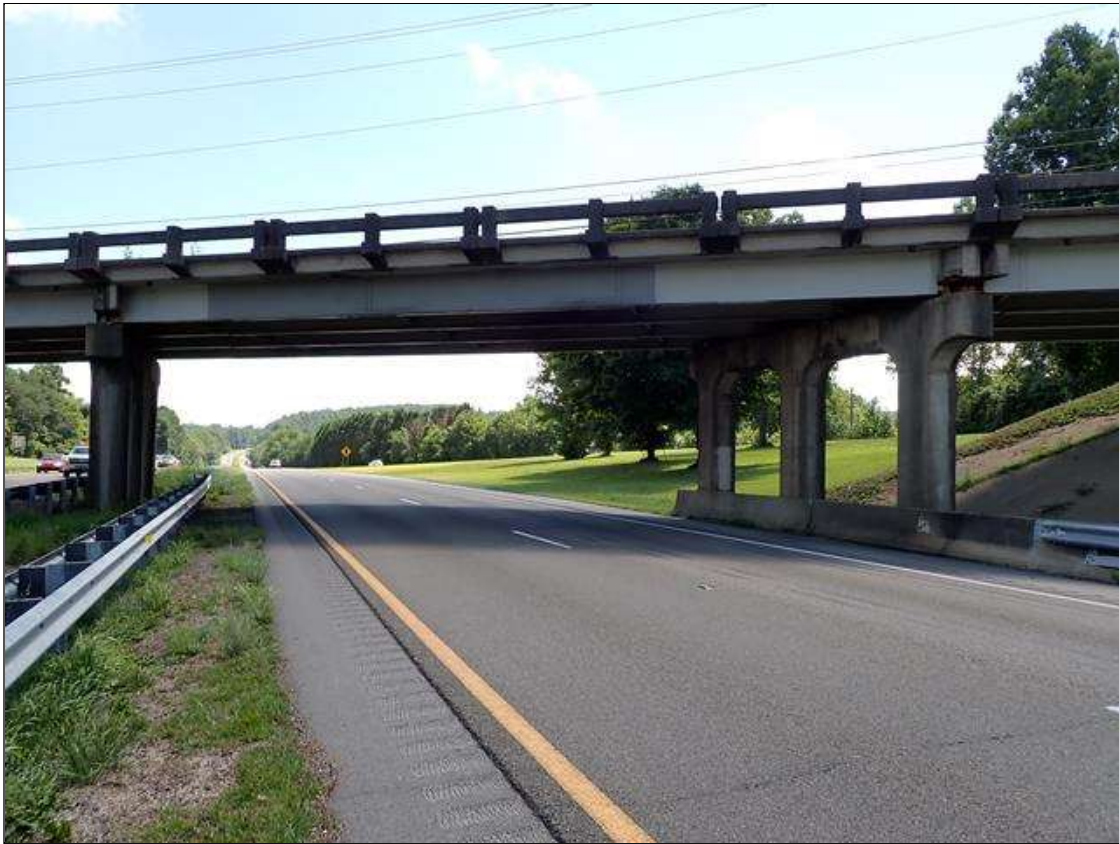
roadway under span 2, looking east (I-40 eastbound)
