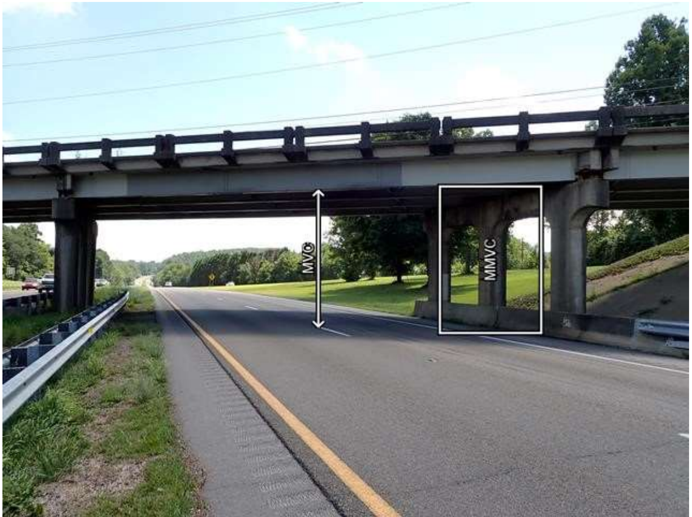
roadway under span 2, looking east
