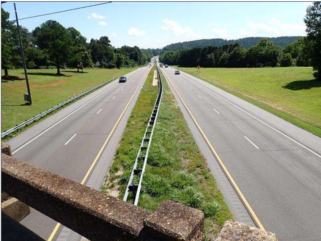
roadway looking east
