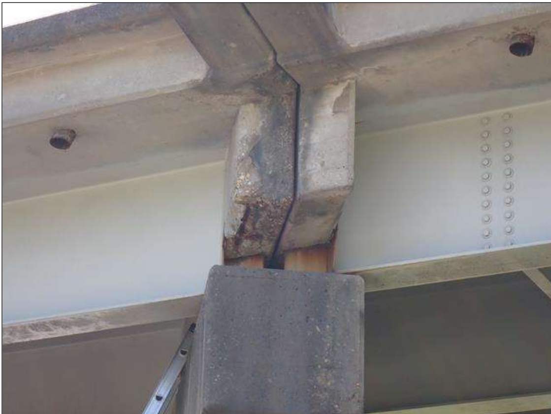
beams over bent
