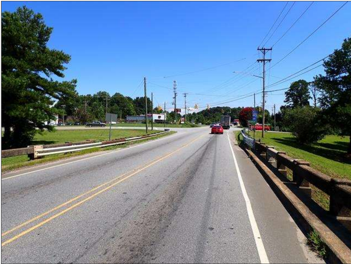
north approach looking north
