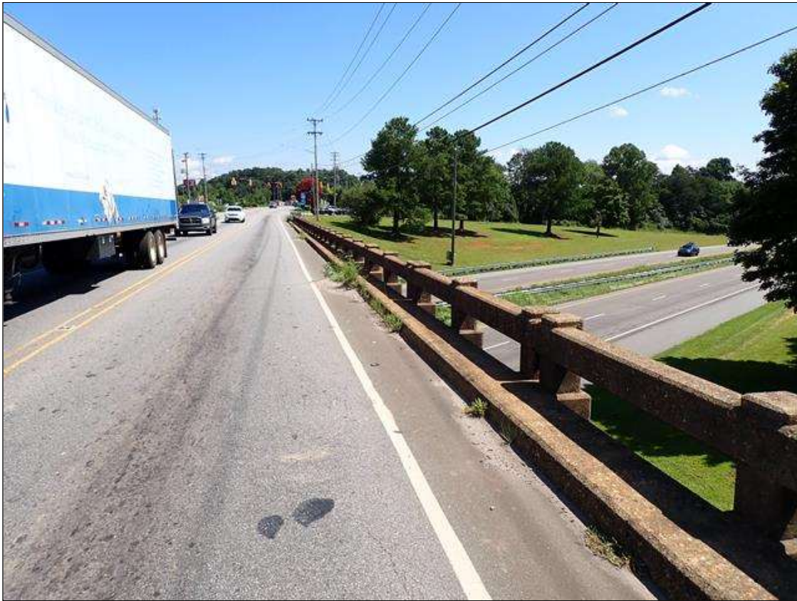
right bridge rail
