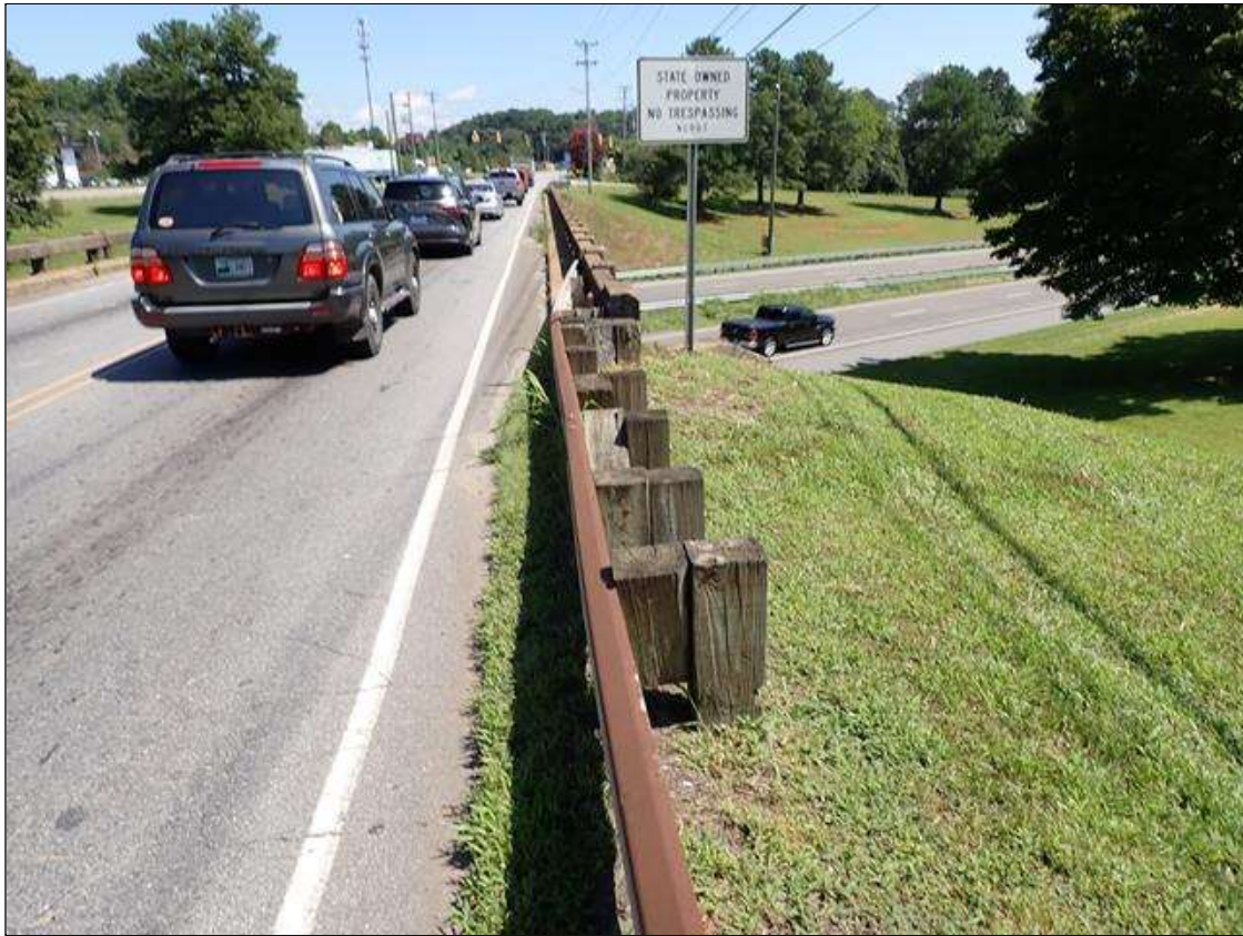
southeast guardrail transition
