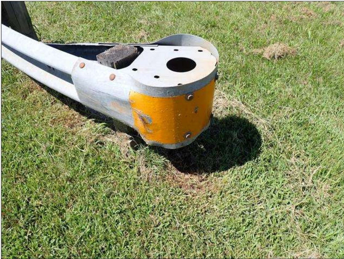
northwest guardrail termination
