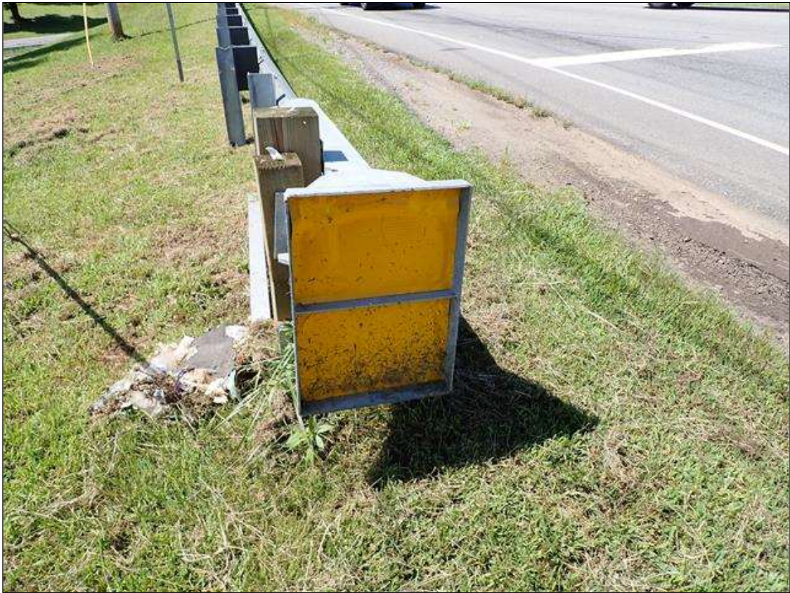
northeast guardrail termination
