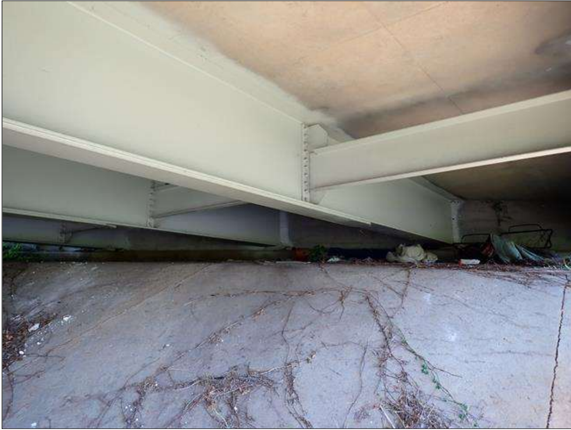
end bent 2 and slope protection
