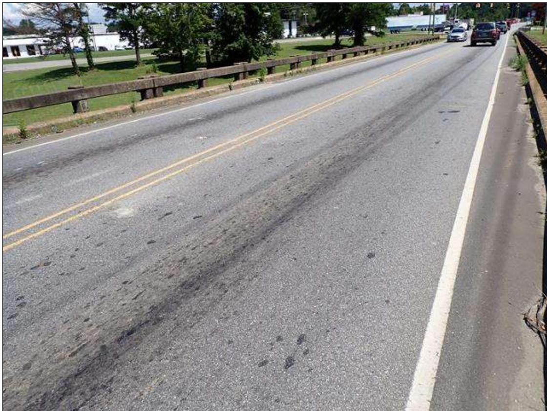
asphalt wearing surface
