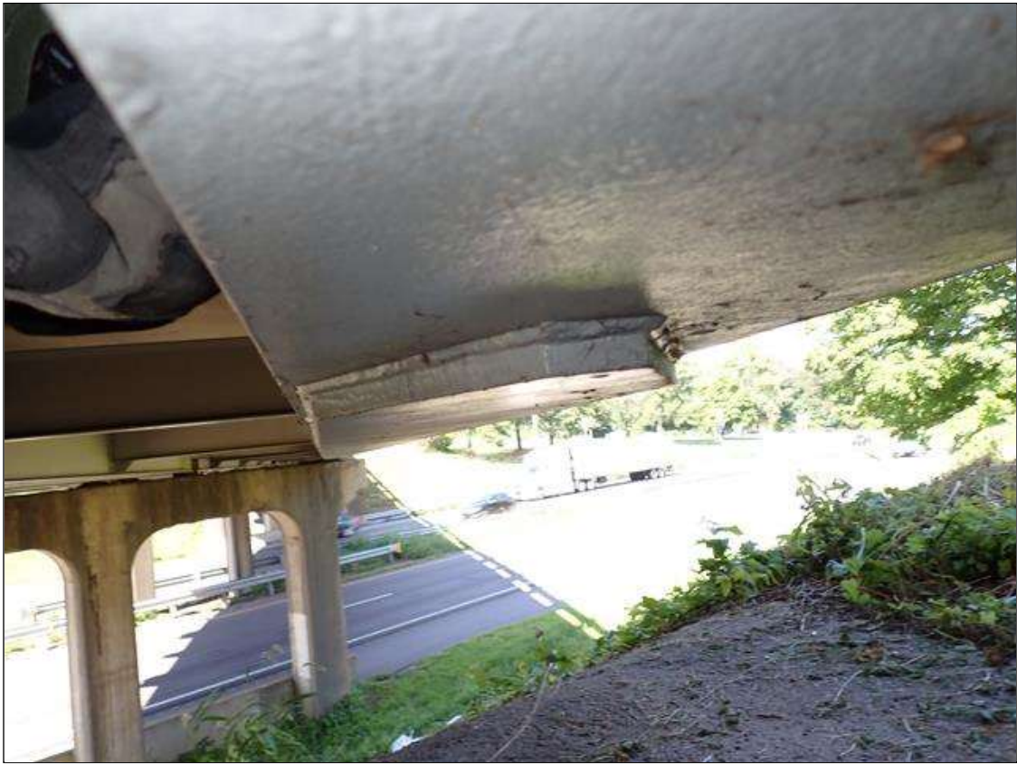
typical coverplate termination
