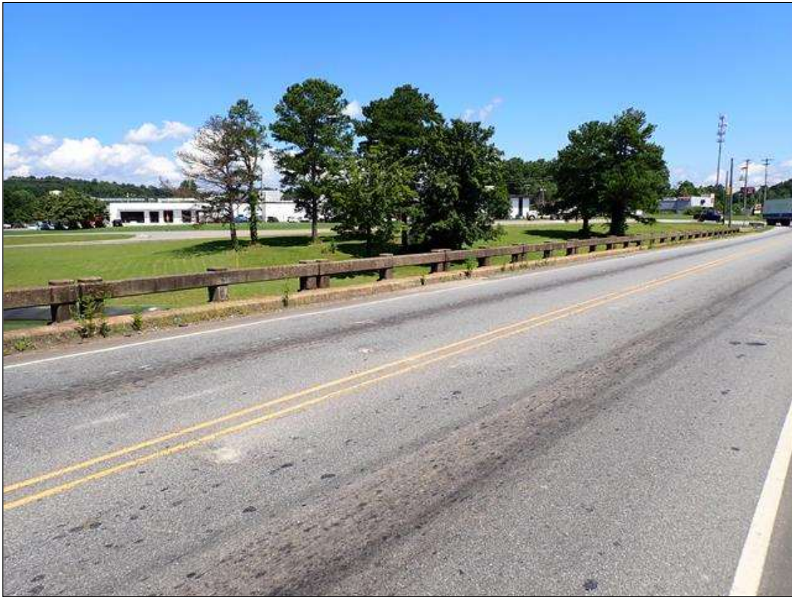
left bridge rail
