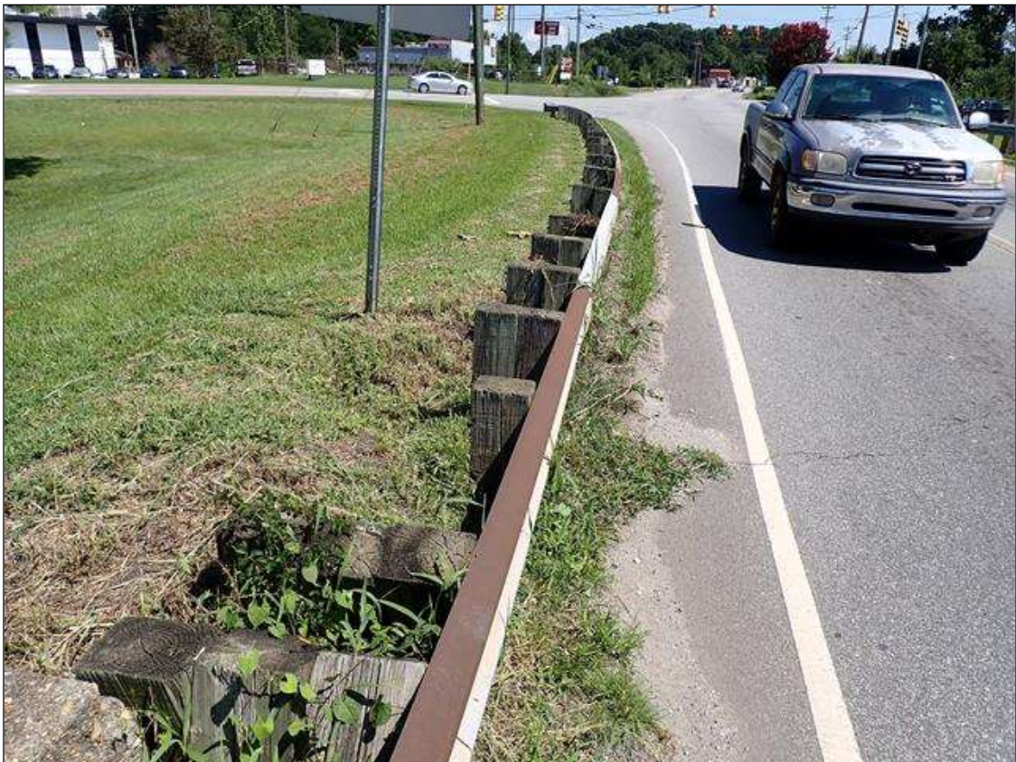
northwest guardrail transition
