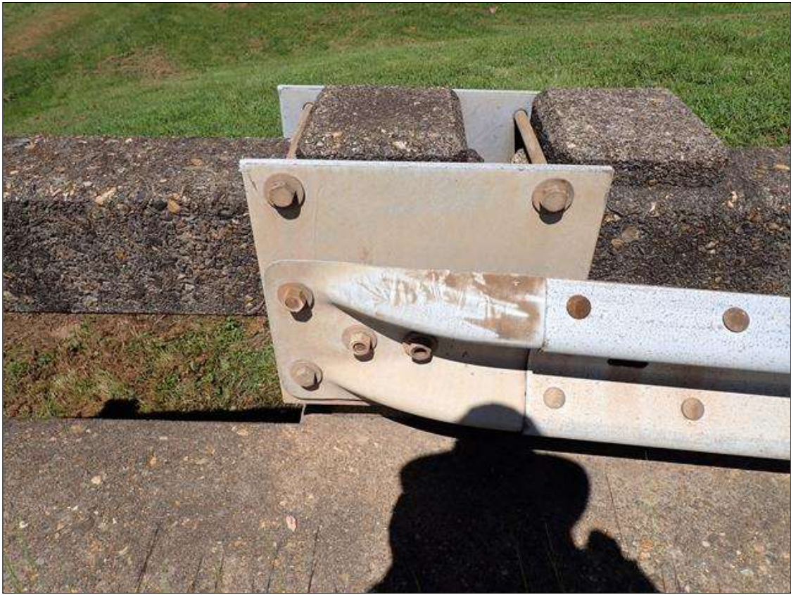
northwest guardrail attachment
