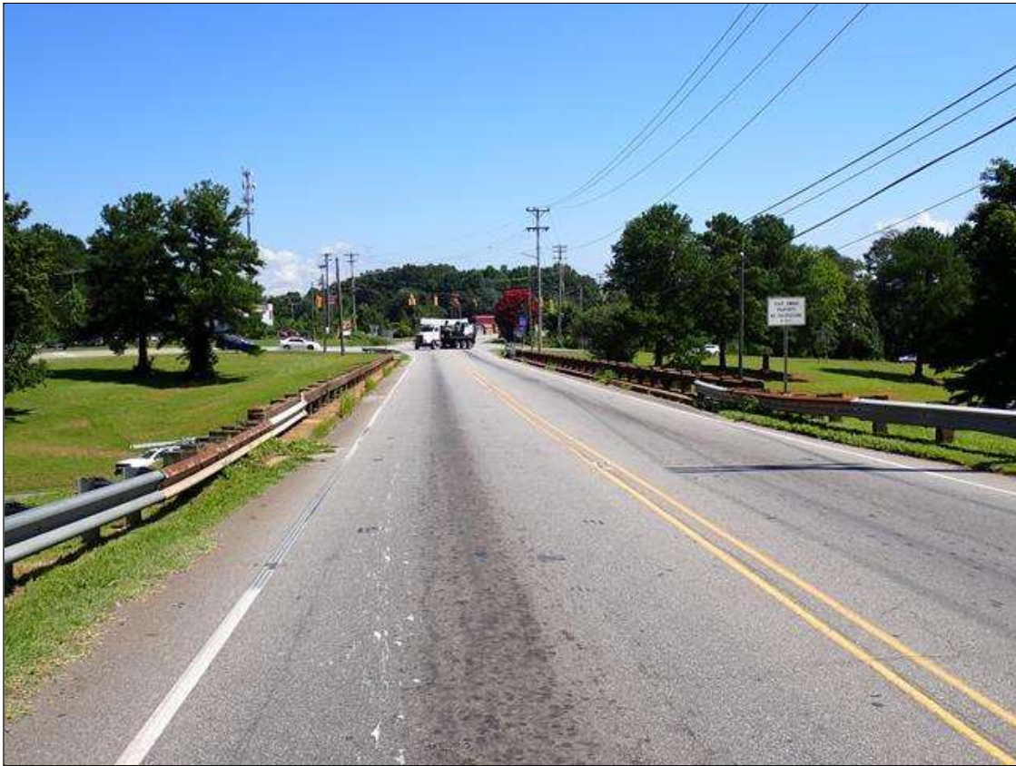
south approach looking north
