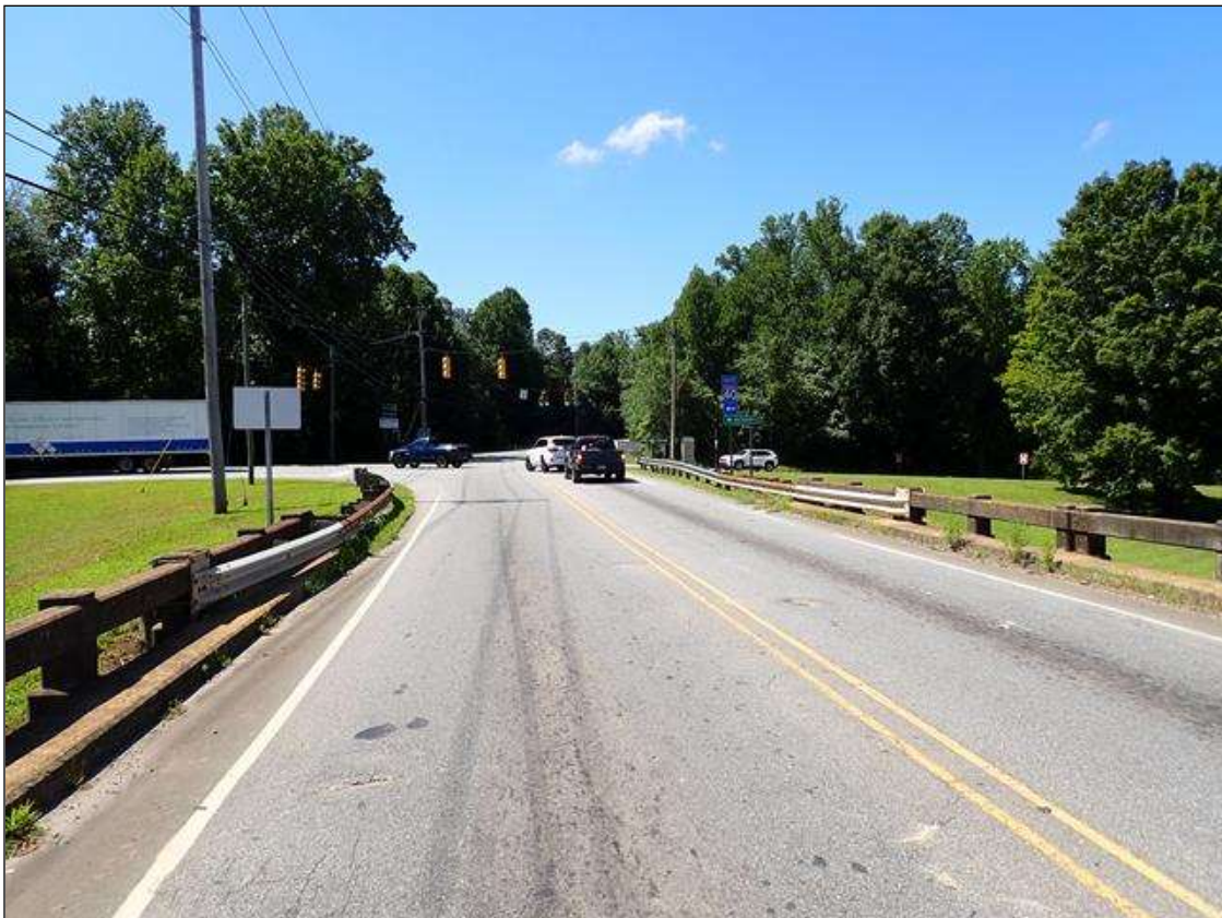
south approach looking south
