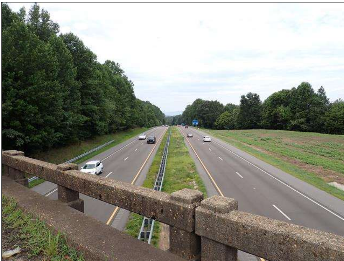
roadway looking west
