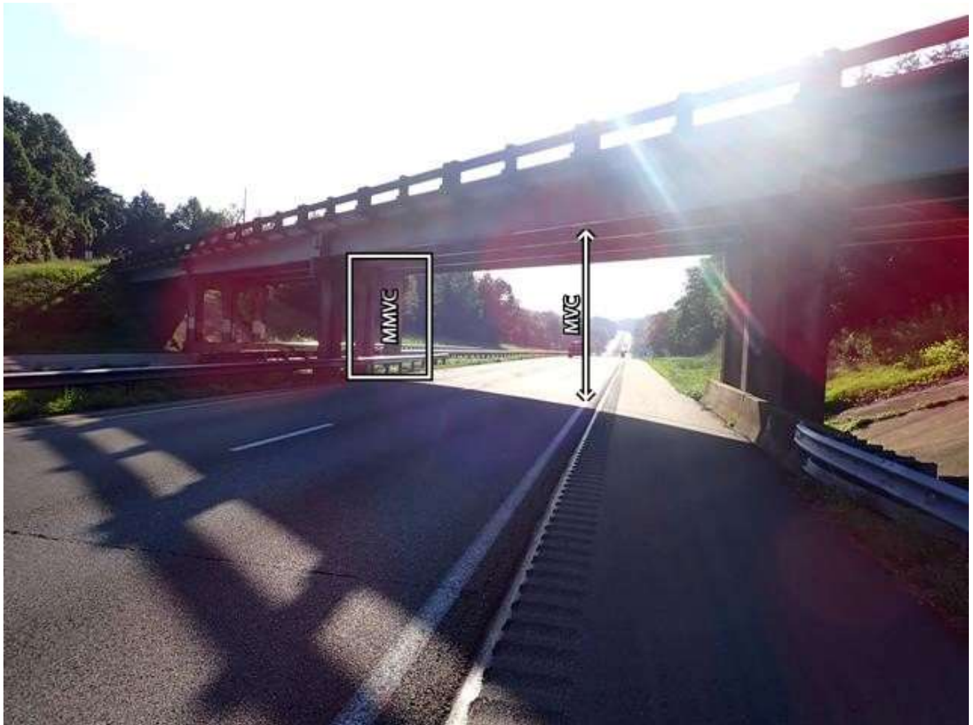
roadway under span 2, looking east
