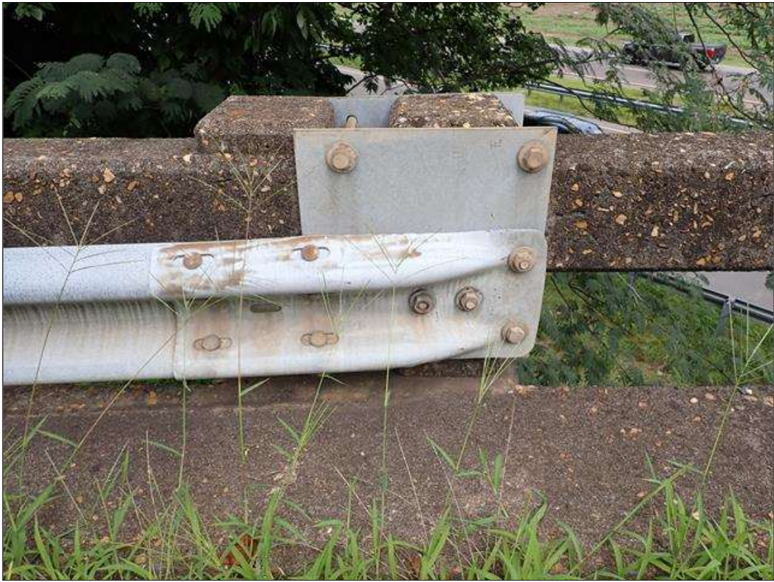
southwest guardrail attachment
