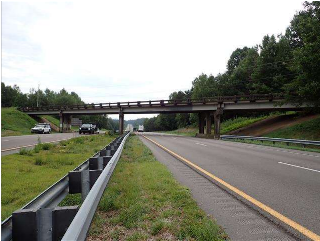
west profile looking east
