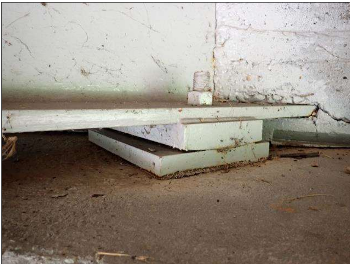
end bearing assembly
