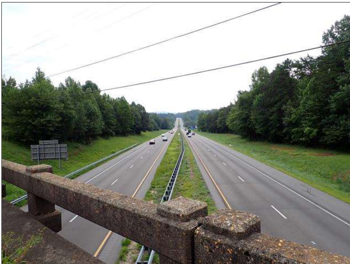
roadway looking east
