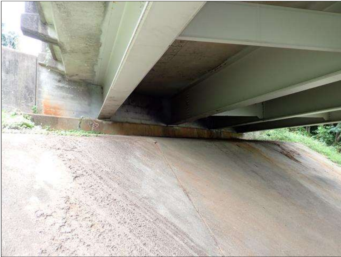
end bent 1 and slope protection
