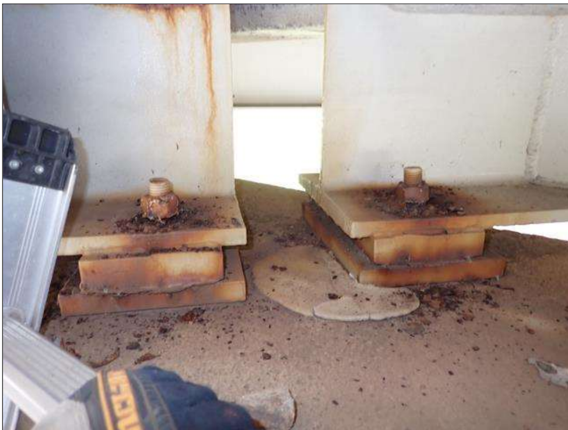
interior bearing assembly
