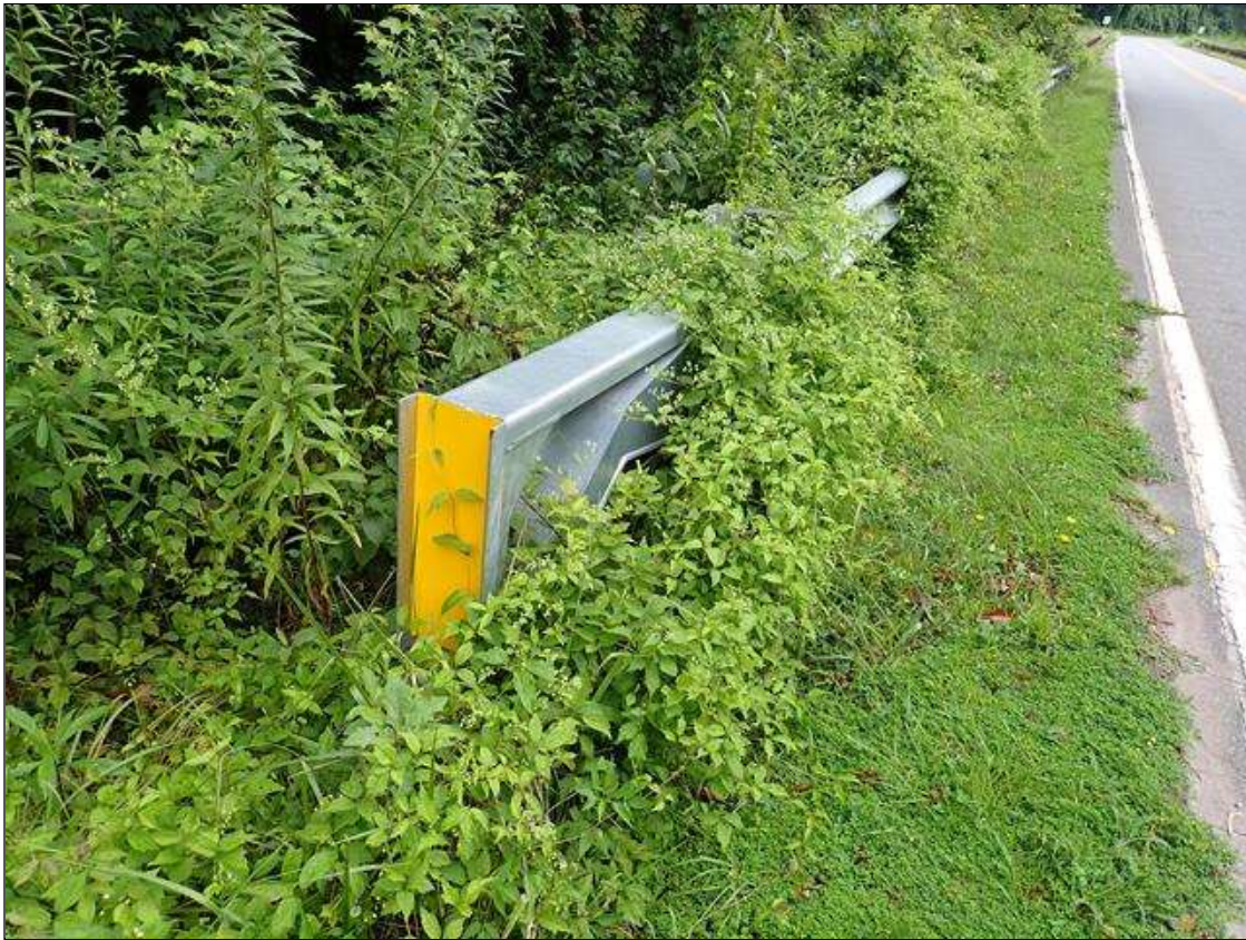
southwest guardrail termination
