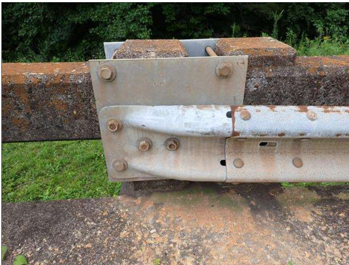
southeast guardrail attachment
