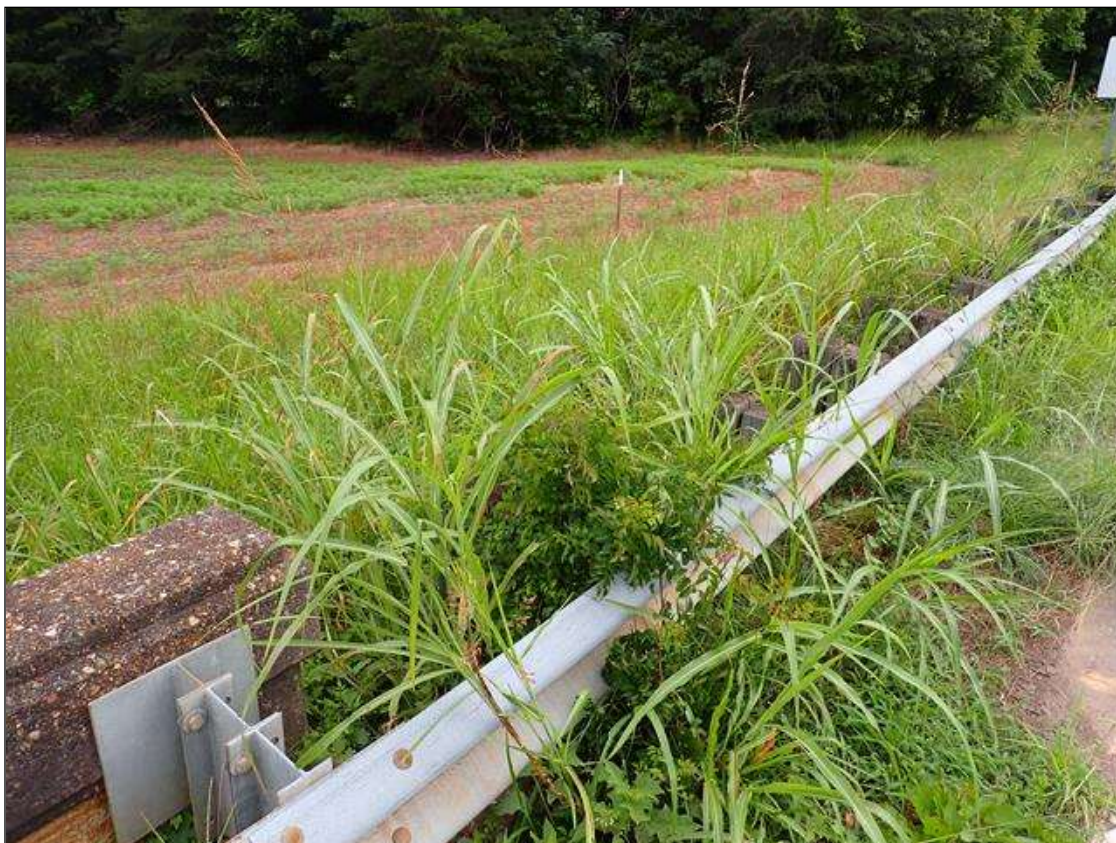
northwest guardrail transition
