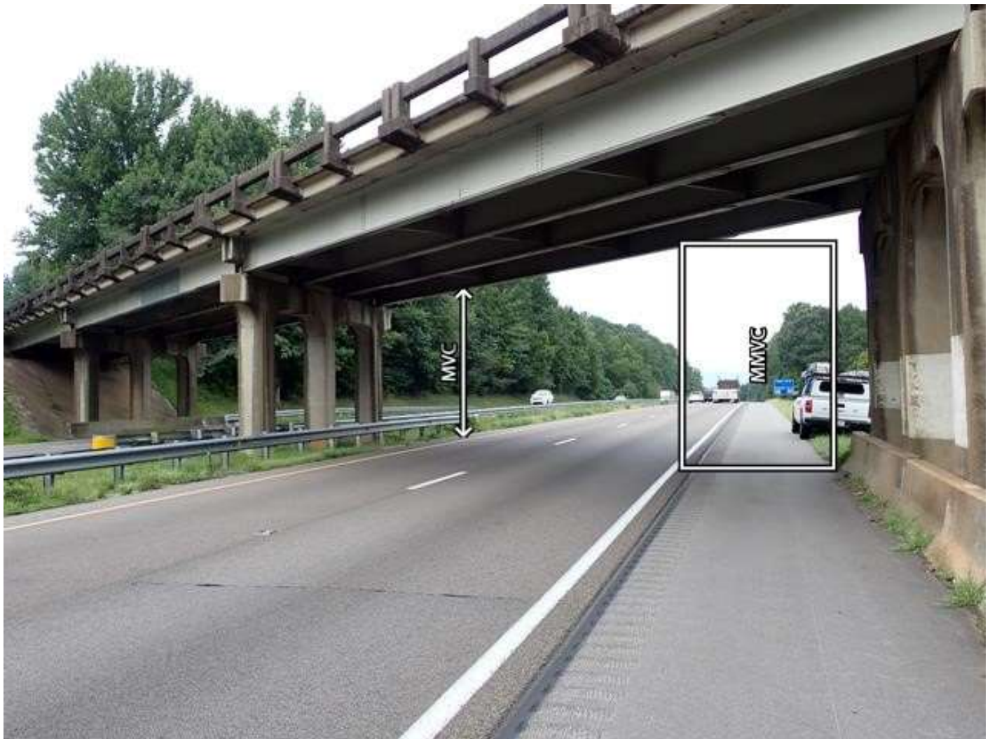
roadway under span 3, looking west
