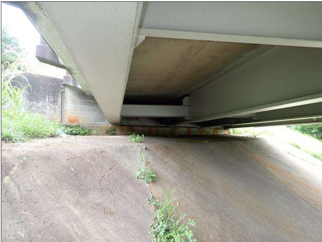
end bent 2 and slope protection
