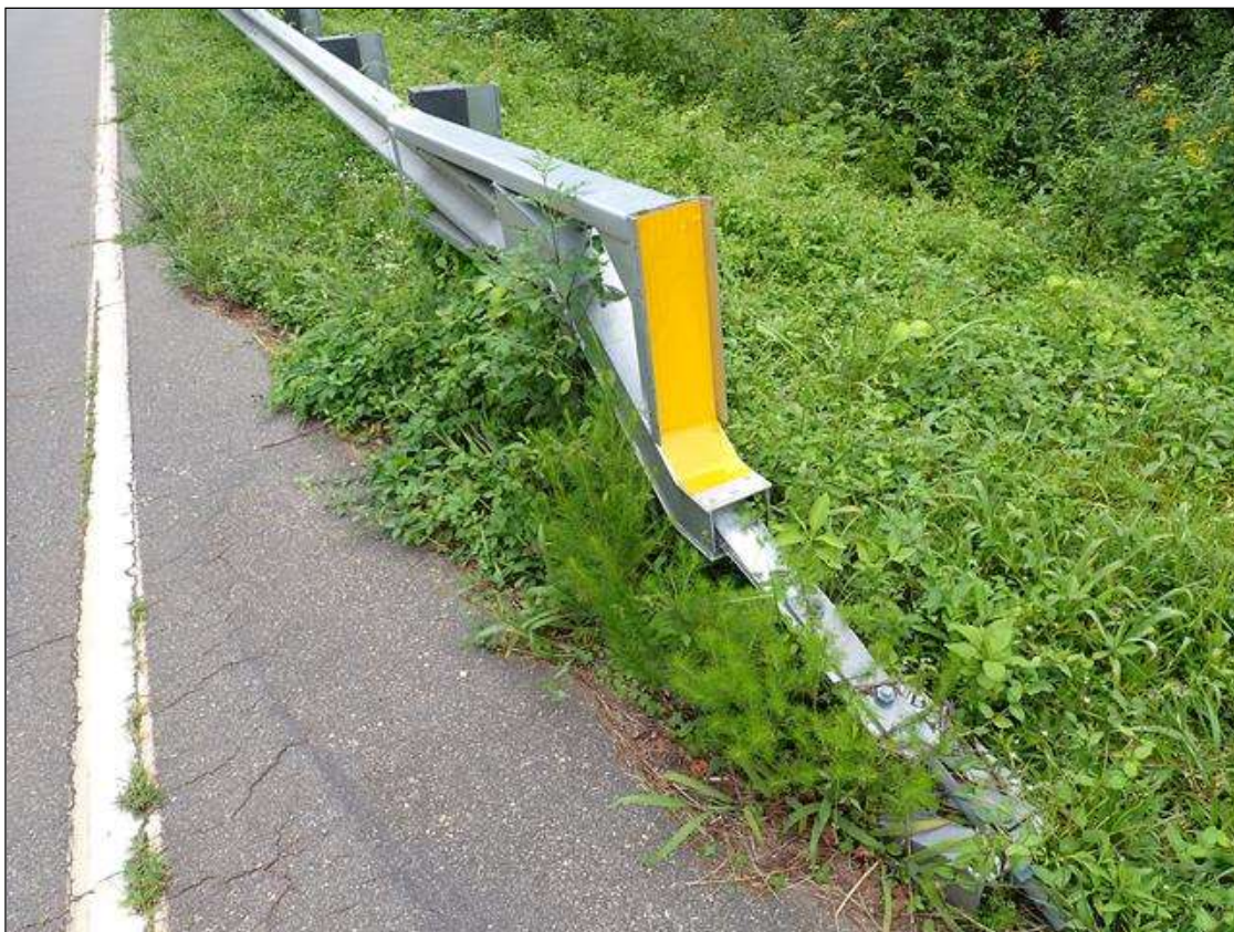
southeast guardrail termination
