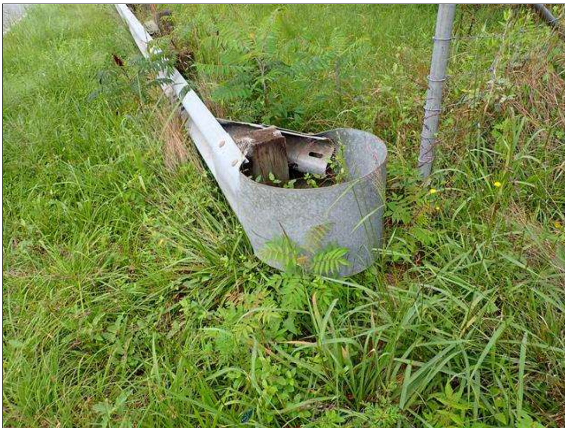
northwest guardrail termination
