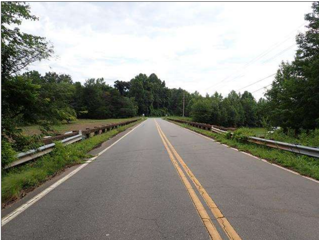
south approach looking north
