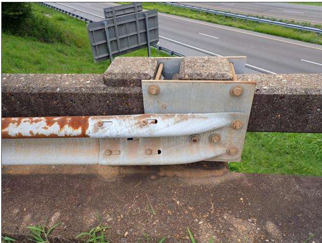
northeast guardrail attachment
