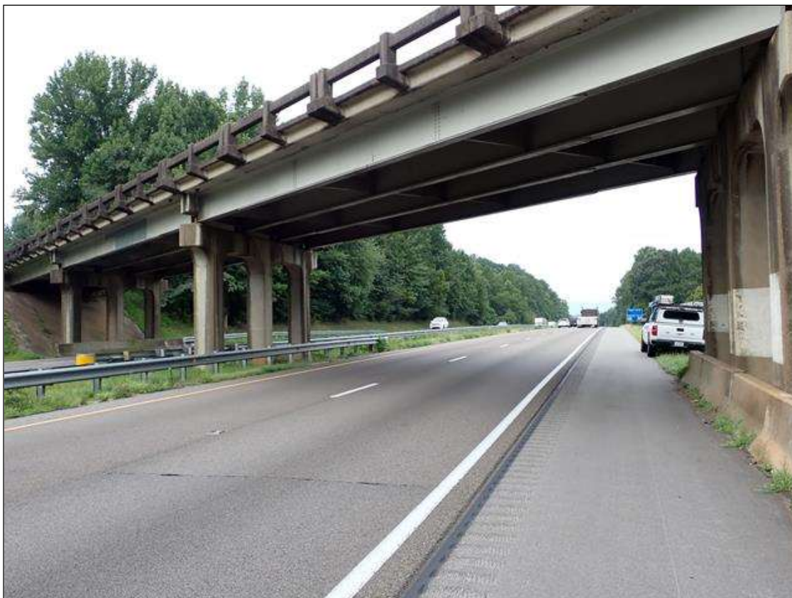
roadway under span 3, looking west (I-40 westbound)
