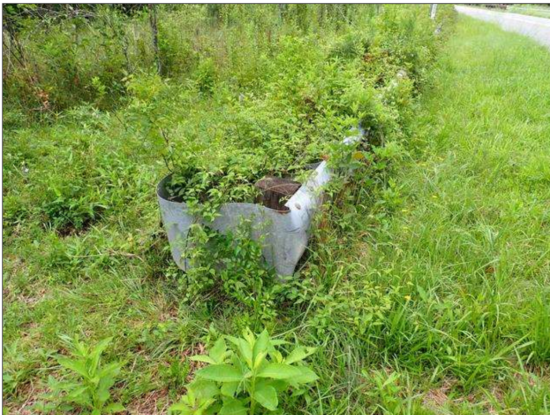
northeast guardrail termination
