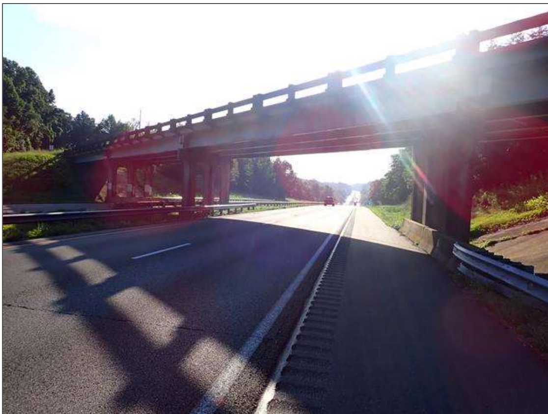
roadway under span 2, looking east (I-40 eastbound)
