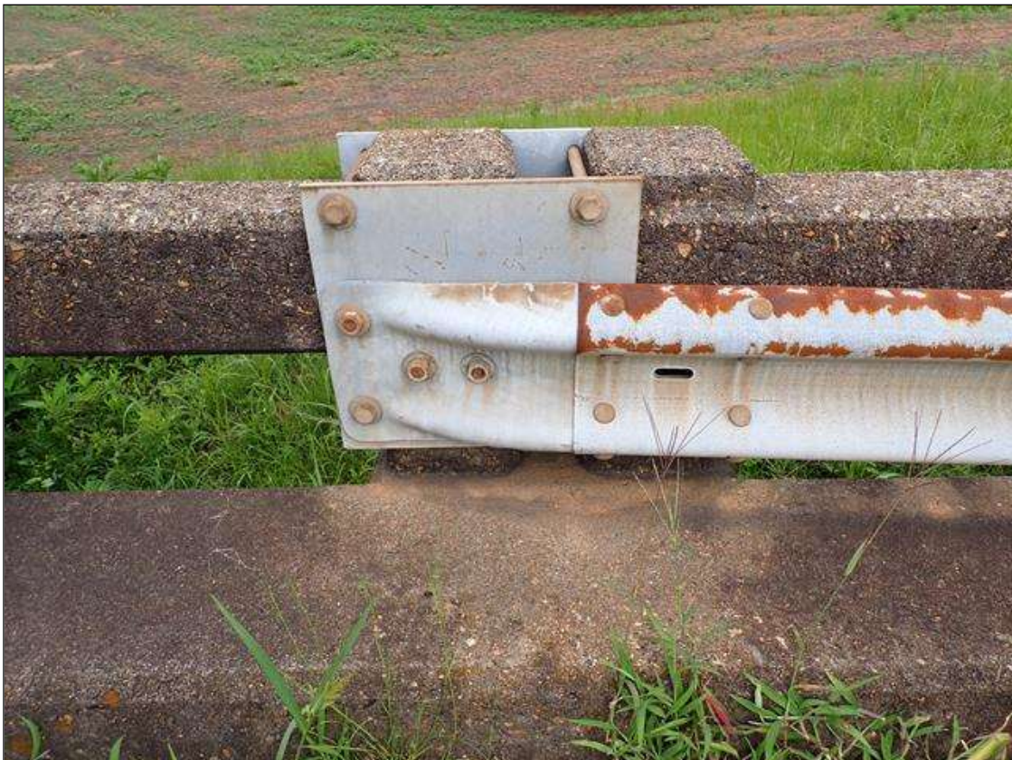
northwest guardrail attachment
