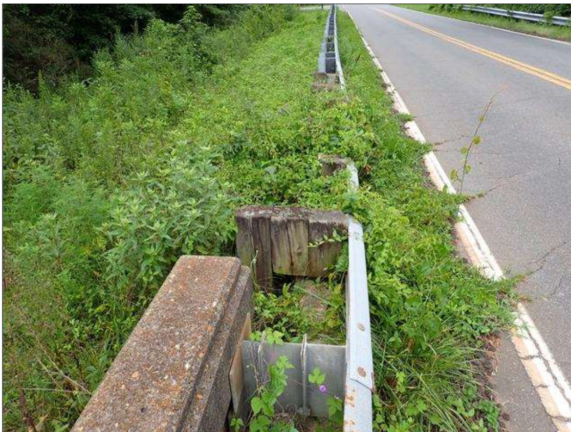
southeast guardrail transition
