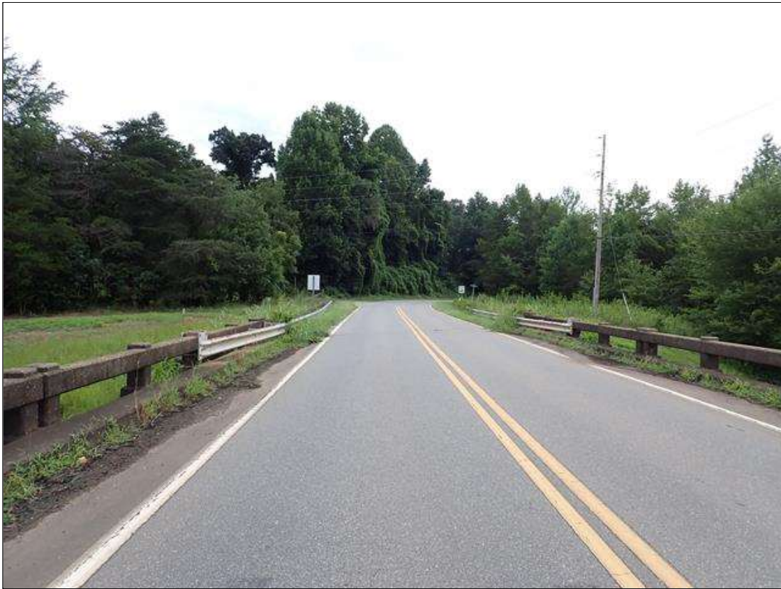
north approach looking north
