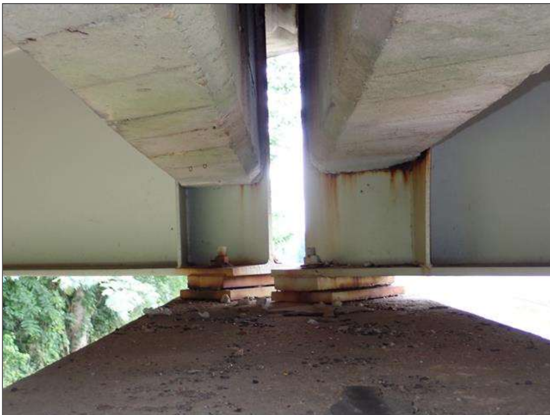
beams over bent
