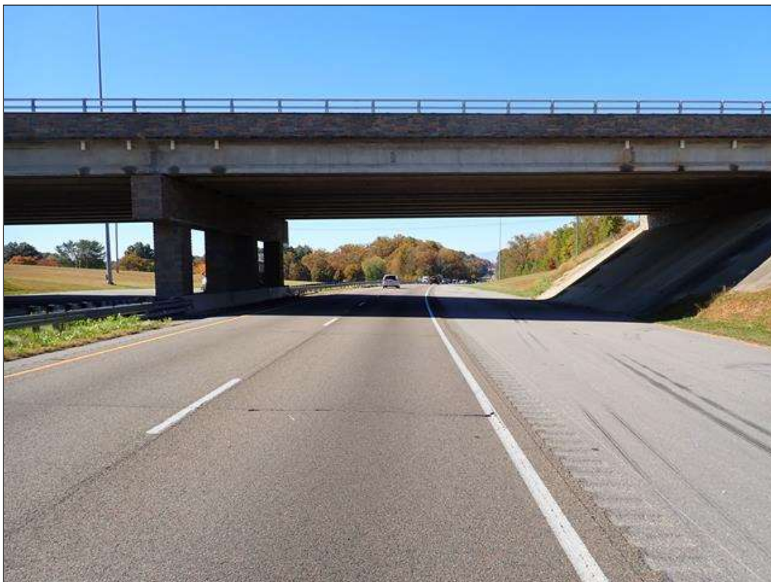
roadway under span 2, looking west (I-40 westbound)
