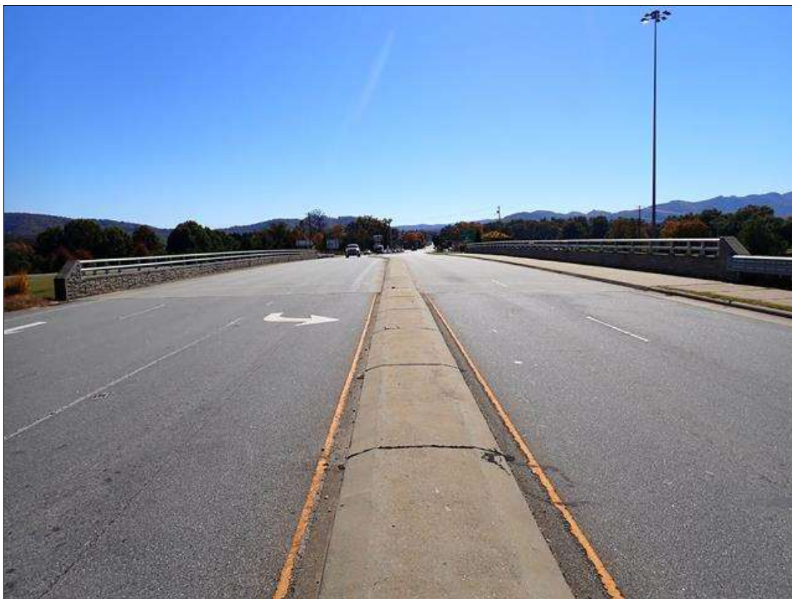
north approach looking south
