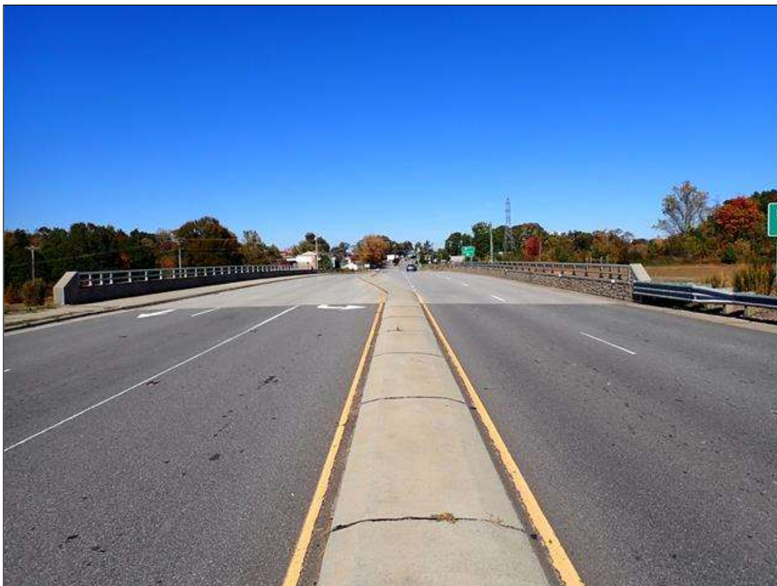
south approach looking north
