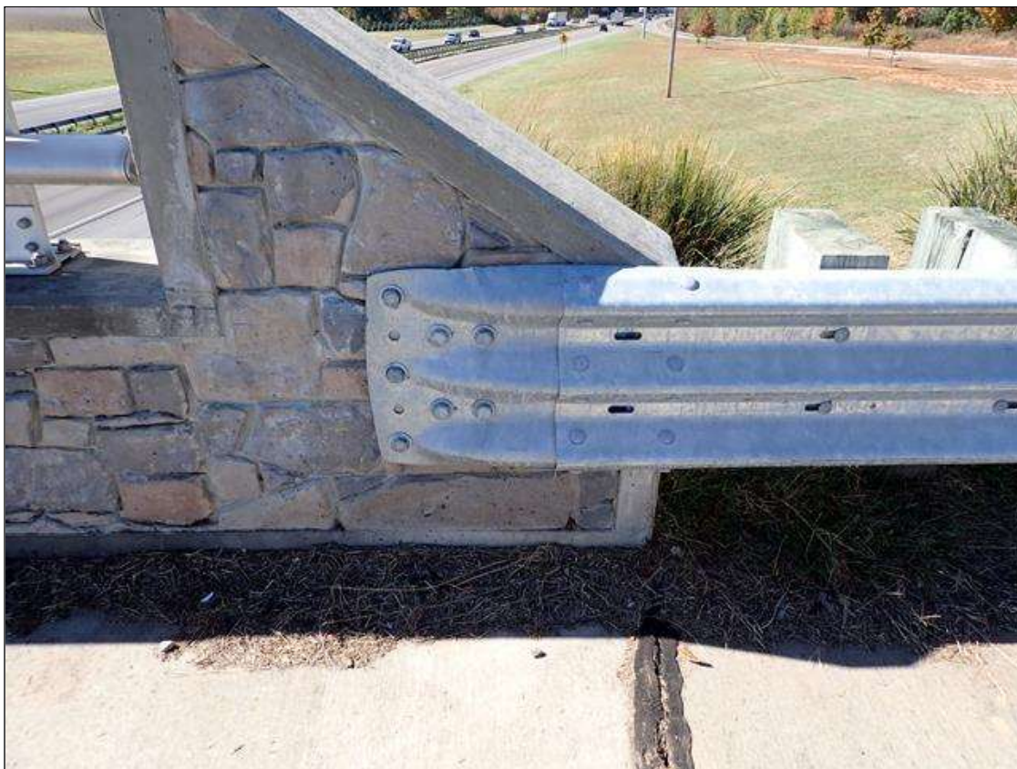
northwest guardrail attachment
