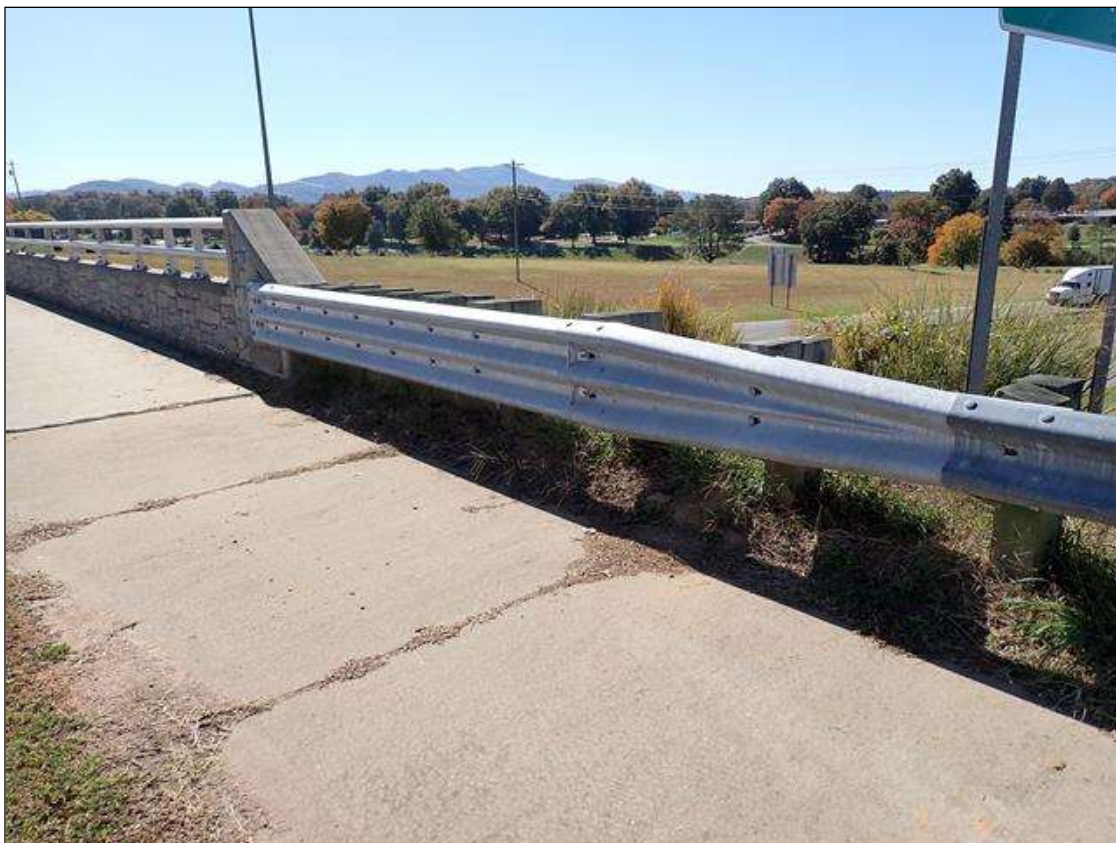
northwest guardrail transition
