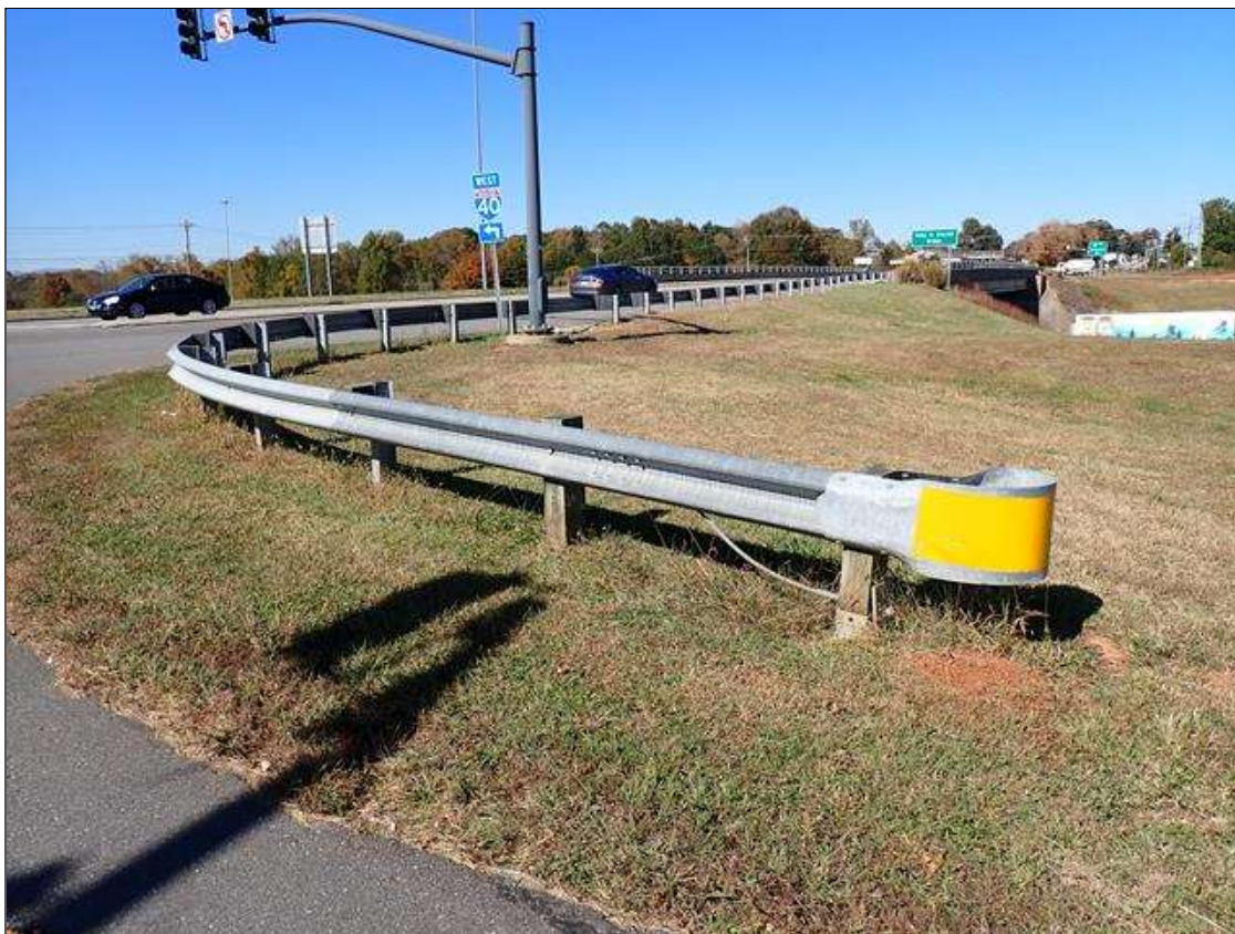
southeast guardrail and termination
