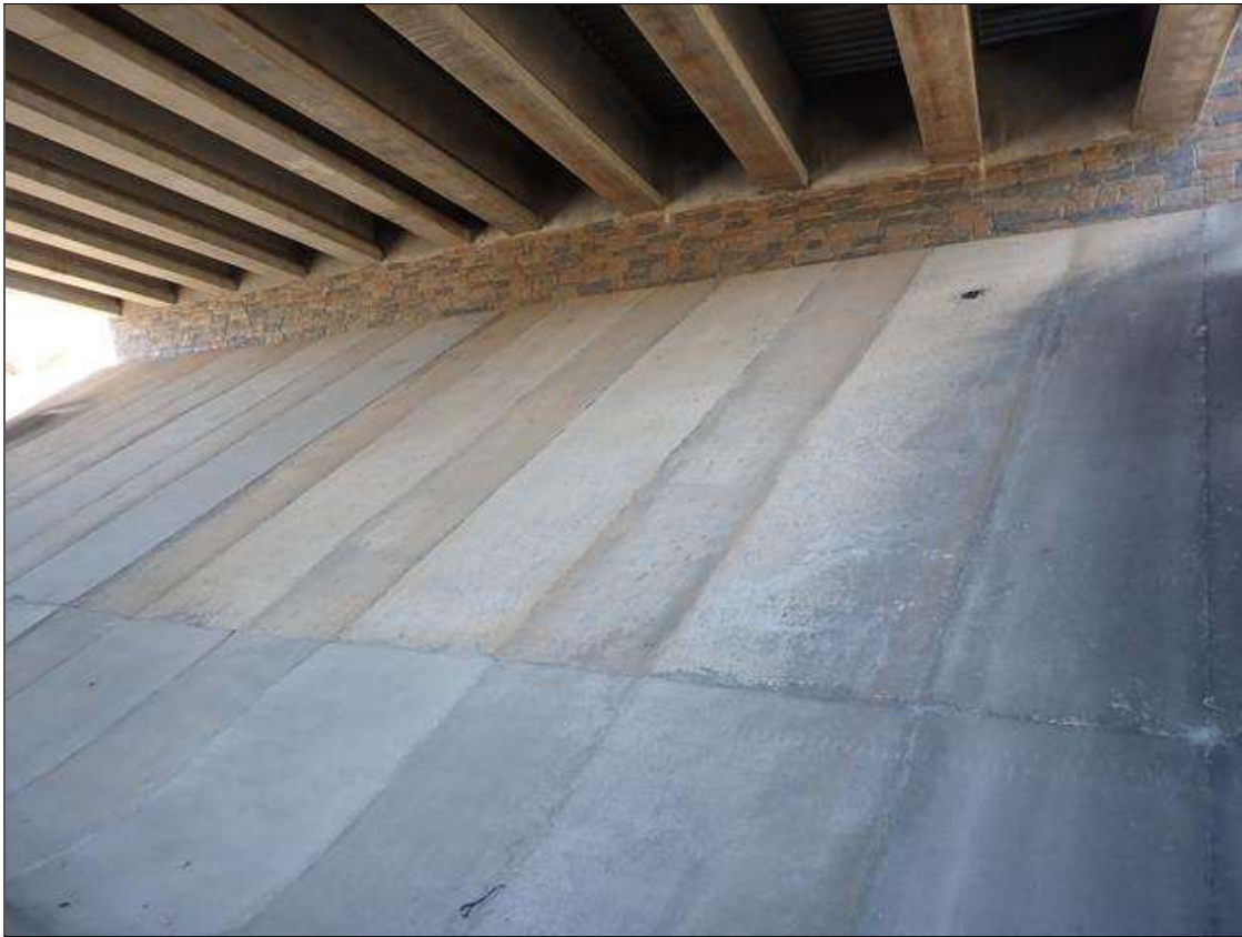
end bent 2 and slope protection
