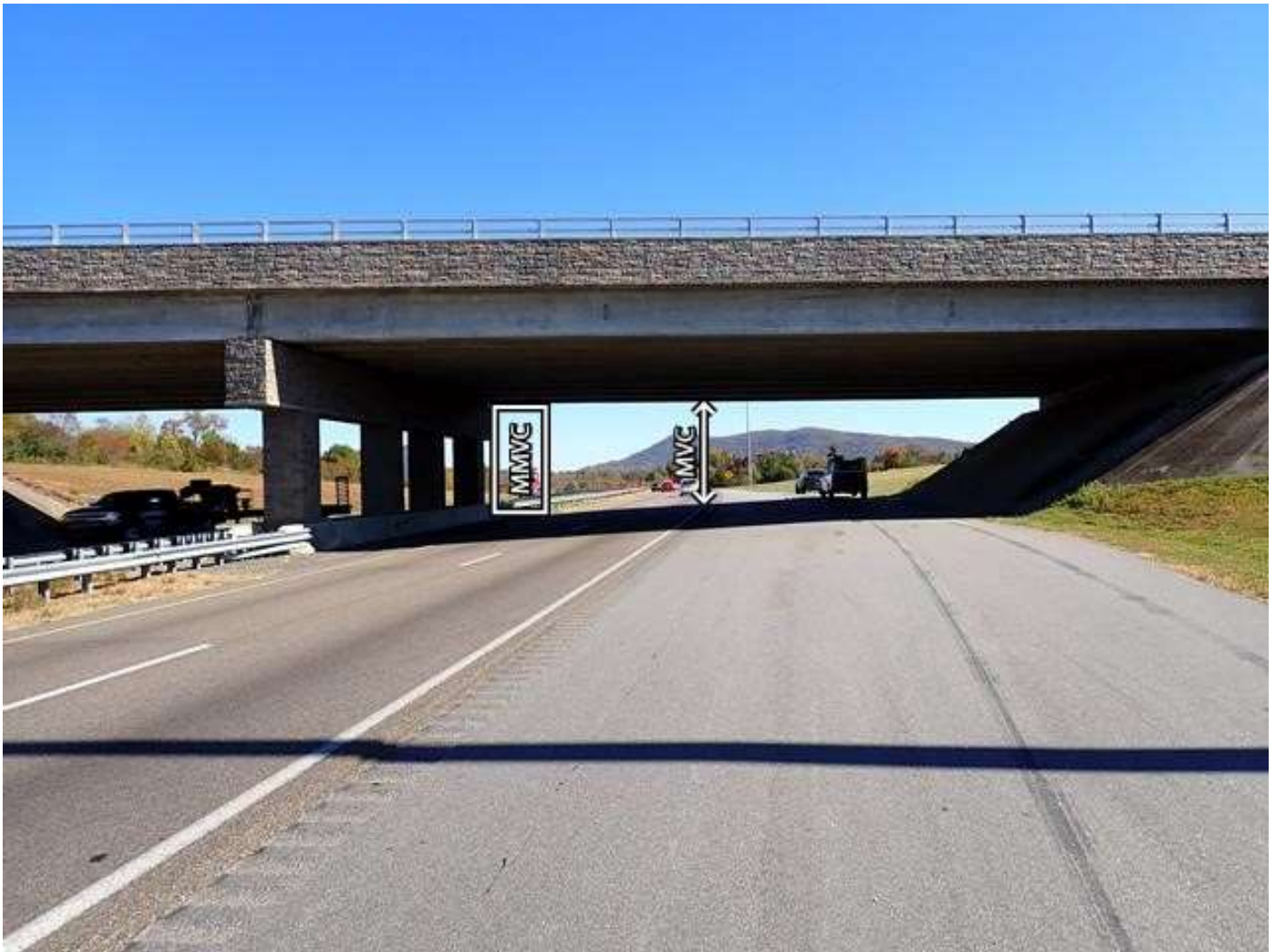
roadway under span 1, looking east (I-40 eastbound)
