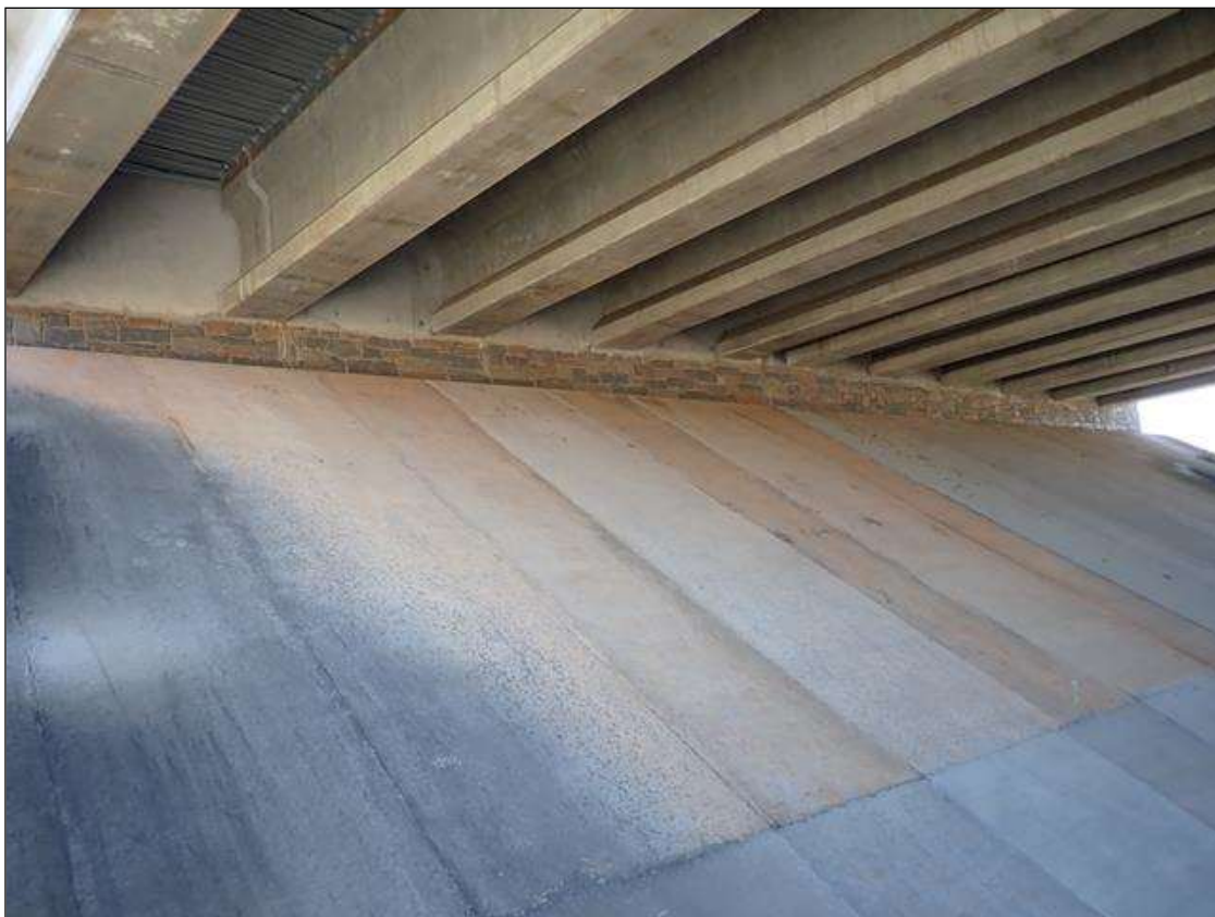
end bent 1 and slope protection
