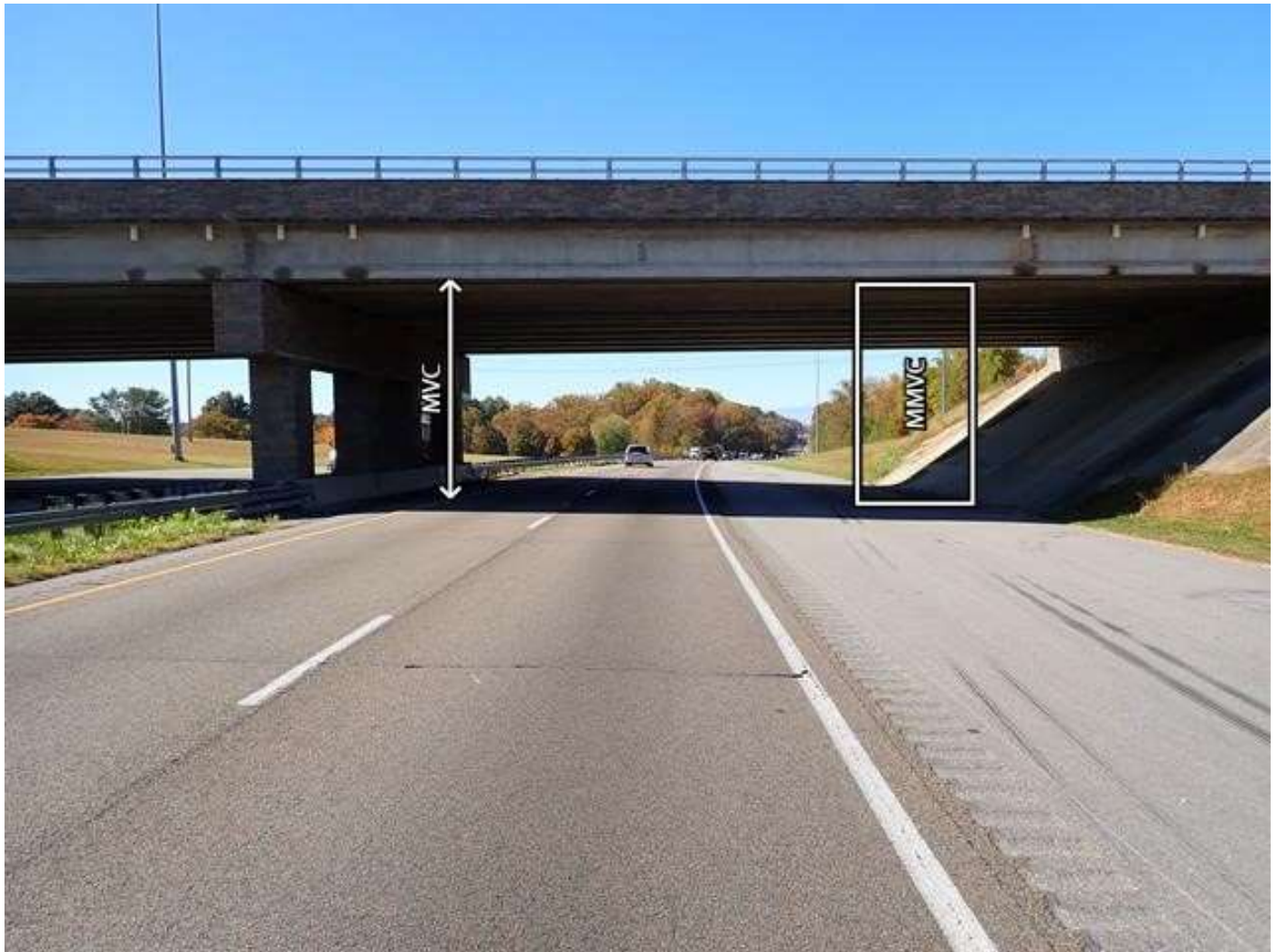
roadway under span 2, looking west (I-40 westbound)
