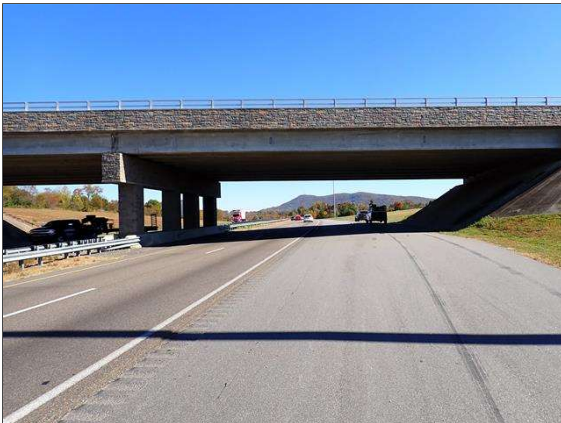
roadway under span 1, looking east (I-40 eastbound)
