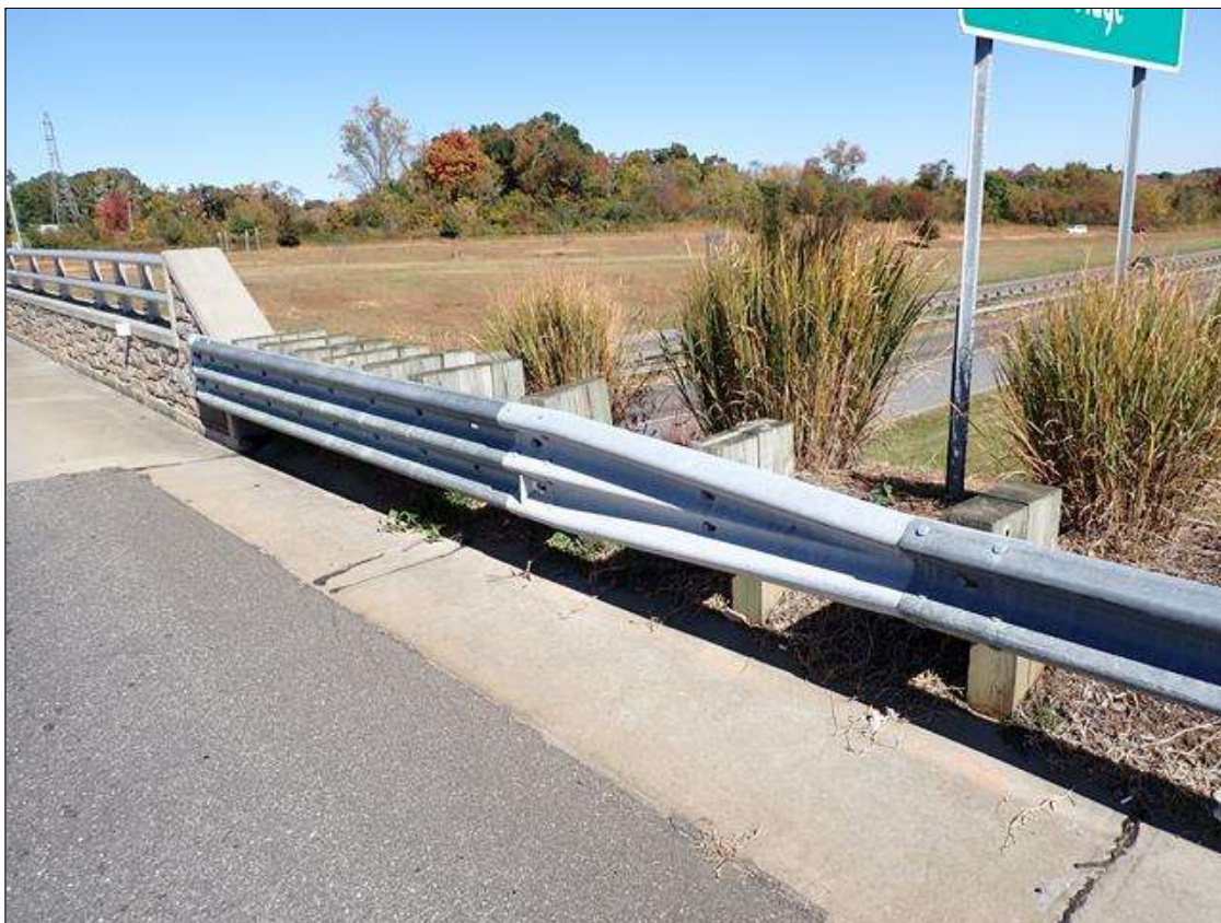
southeast guardrail transition
