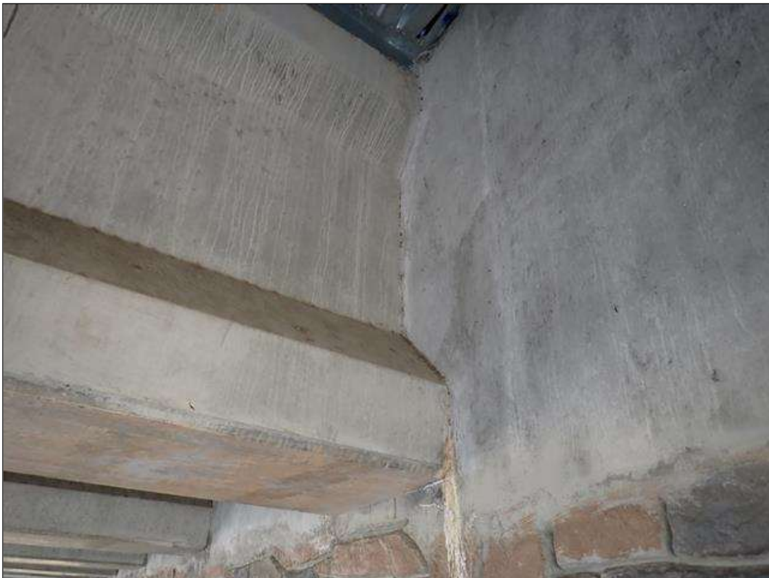
typical beams at abutment
