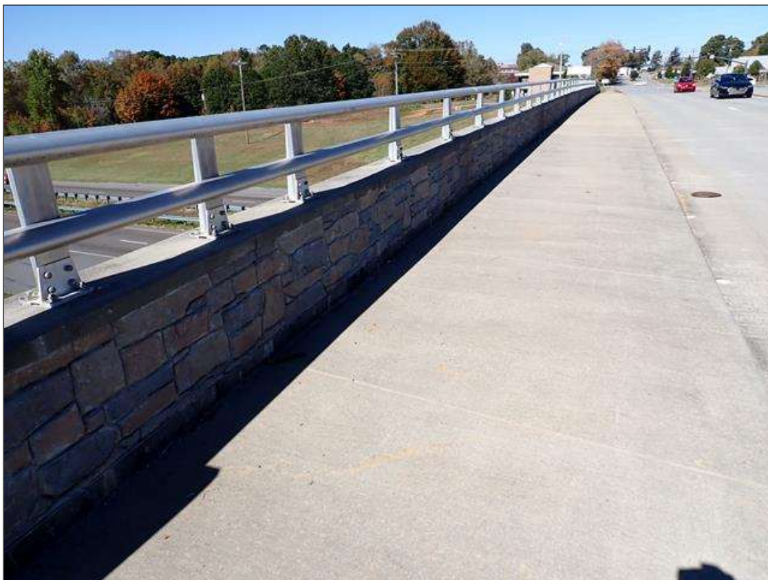
left bridge rail
