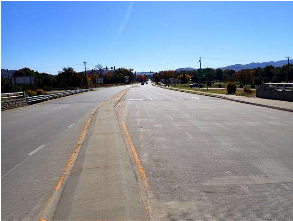
south approach looking south
