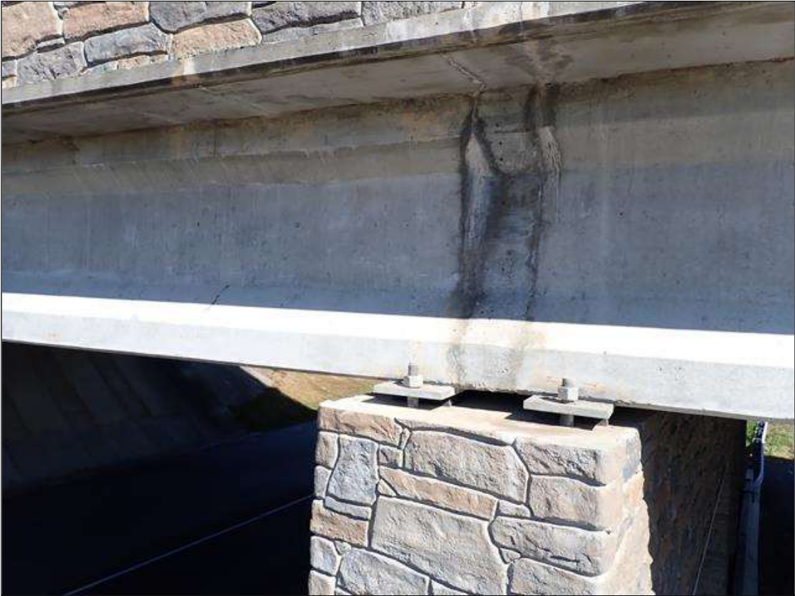
beams over bent
