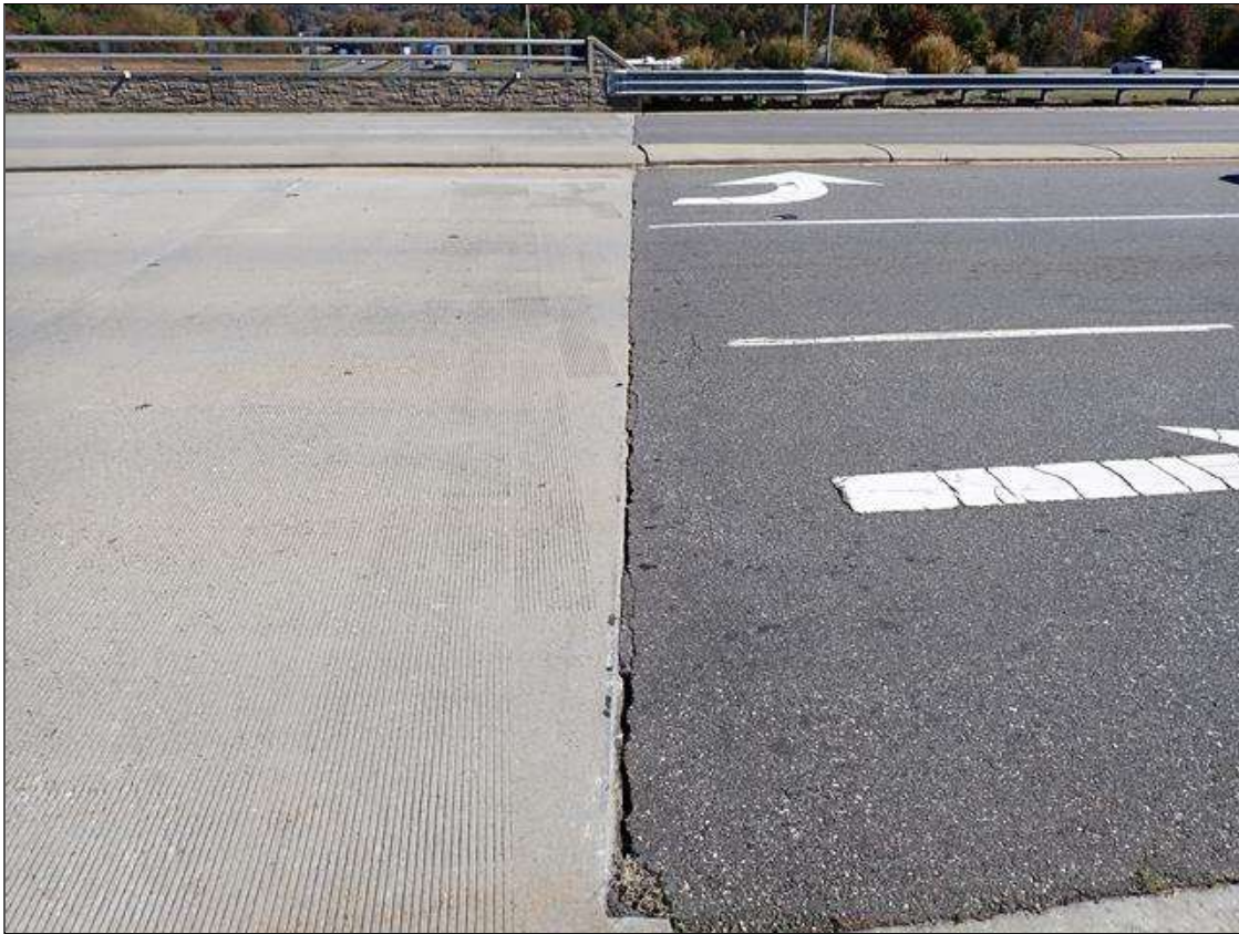
end of approach slab 1
