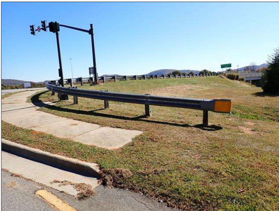
northwest guardrail and termination
