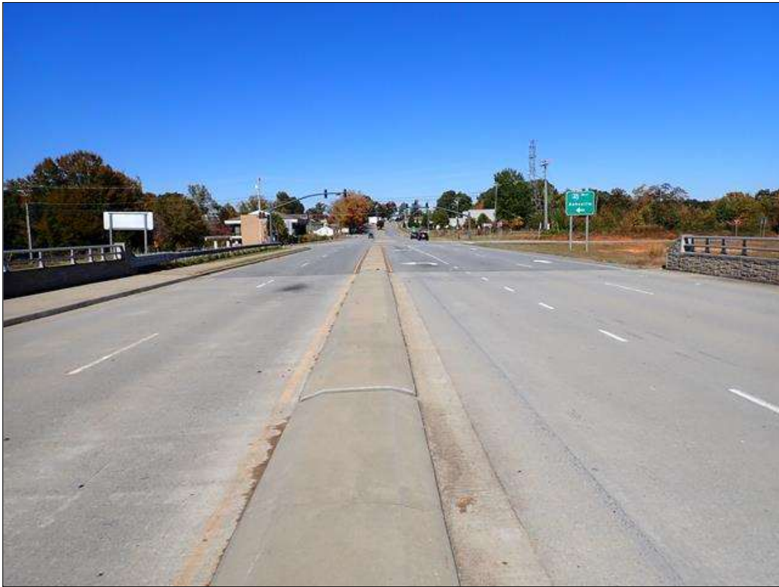
north approach looking north
