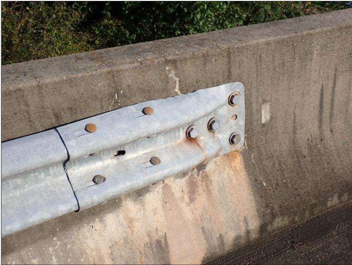
southwest guardrail attachment
