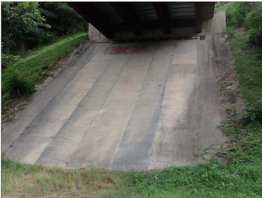
end bent 1 slope protection
