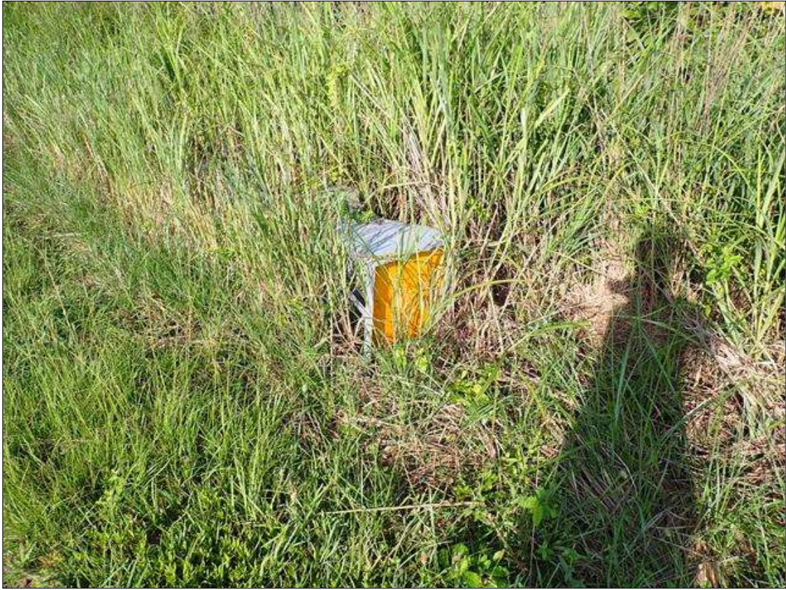
northwest guardrail termination
