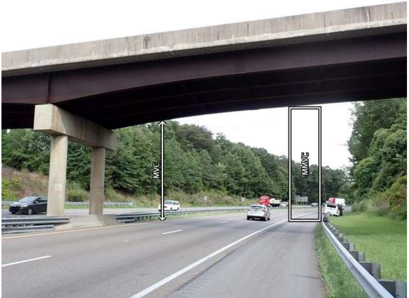
roadway under span 1, looking east (I-40 eastbound)
