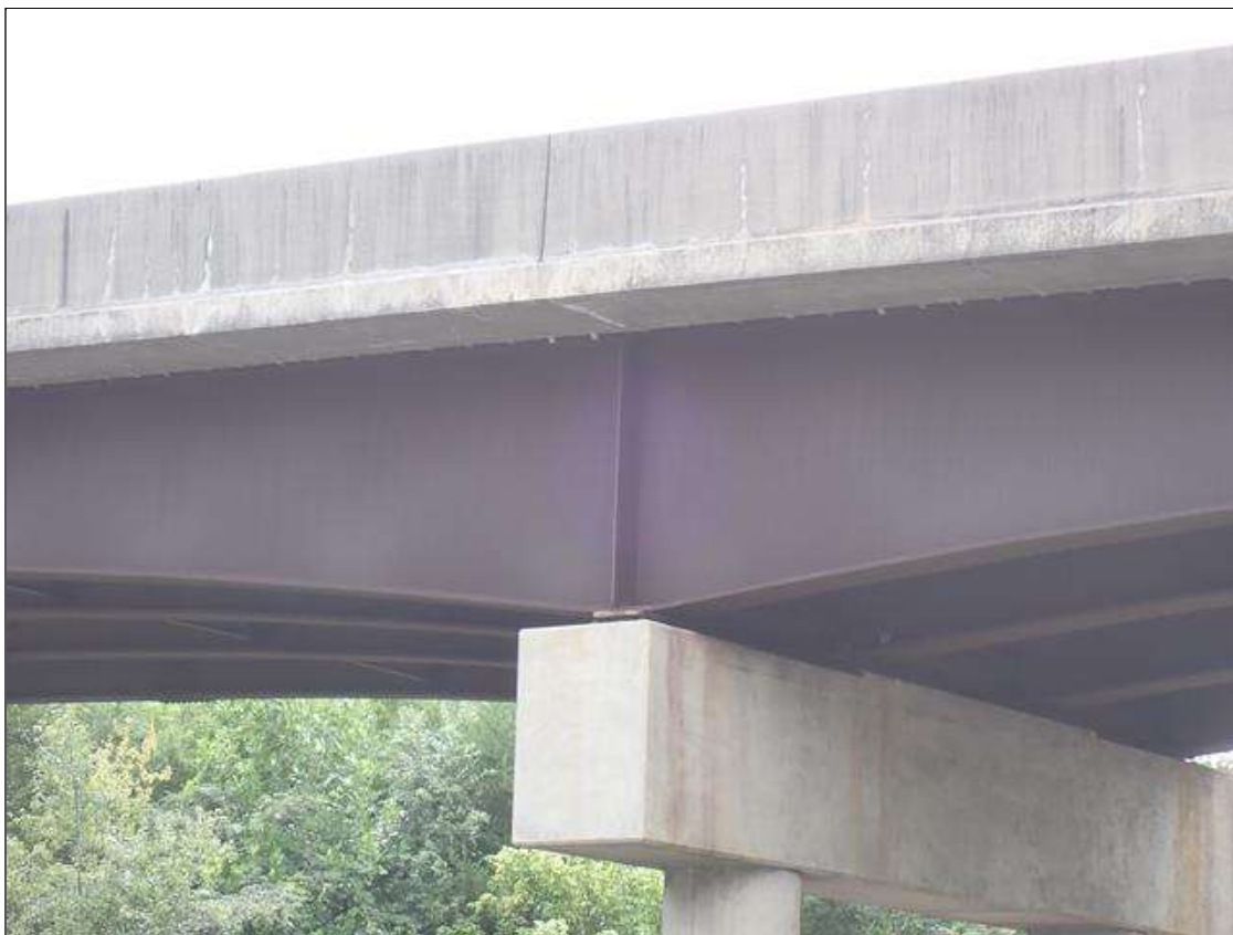
beams over bent 1
