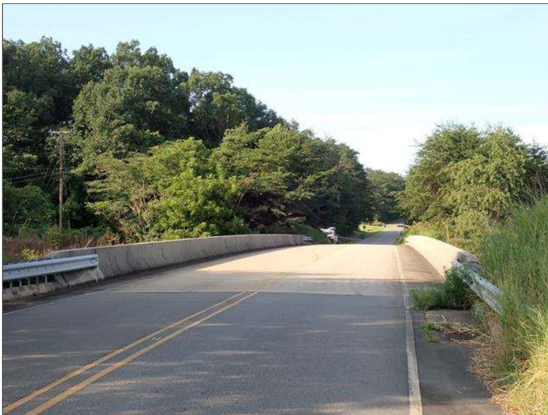
north approach looking south
