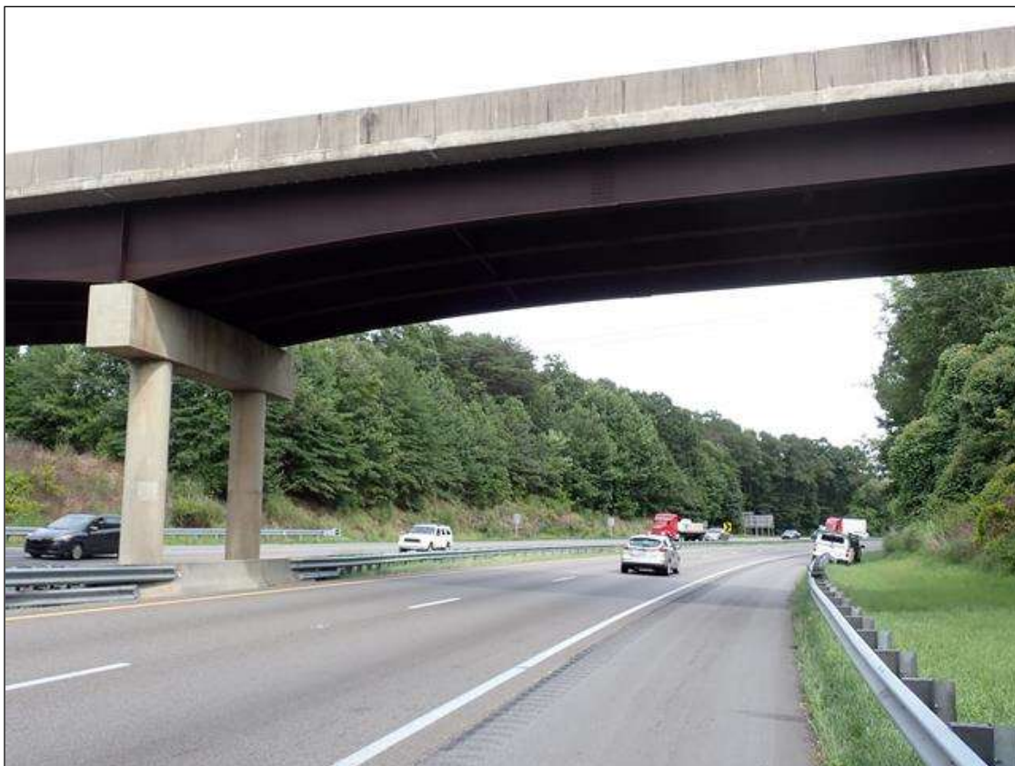
roadway under span 1, looking east (I-40 eastbound)
