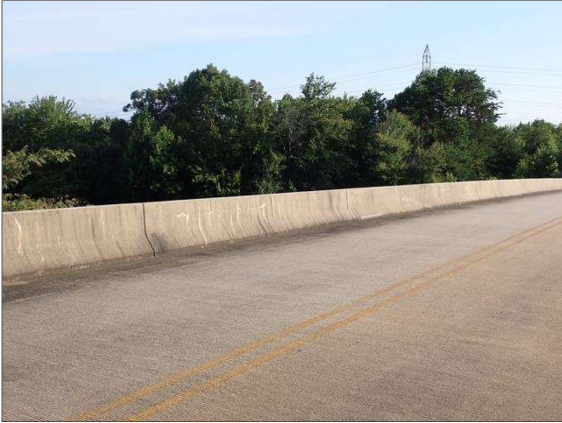
left bridge rail
