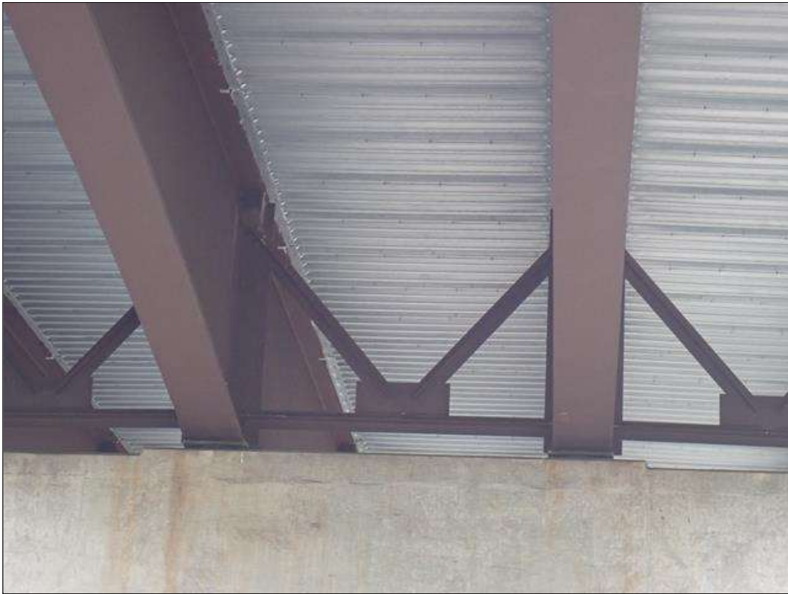
end diaphragm at bent 1
