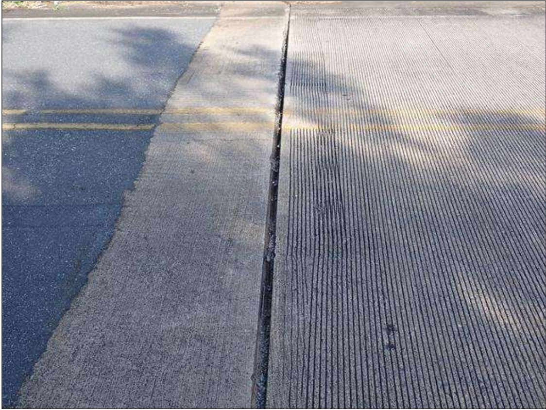
end bent 1 joint
