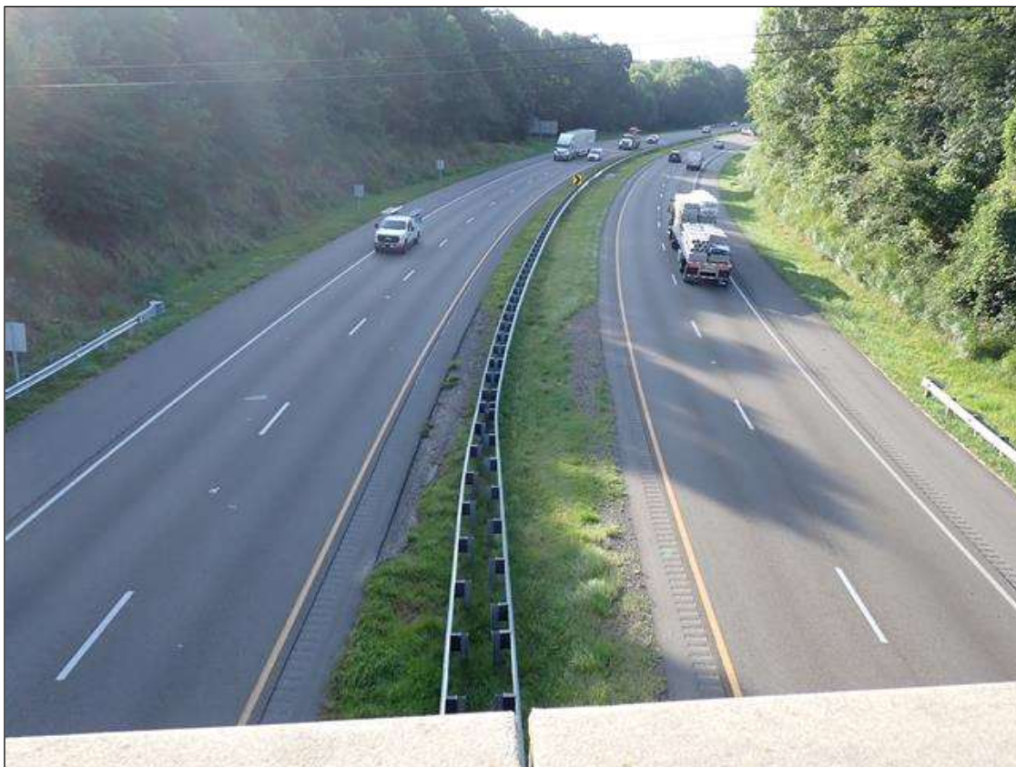
roadway looking east
