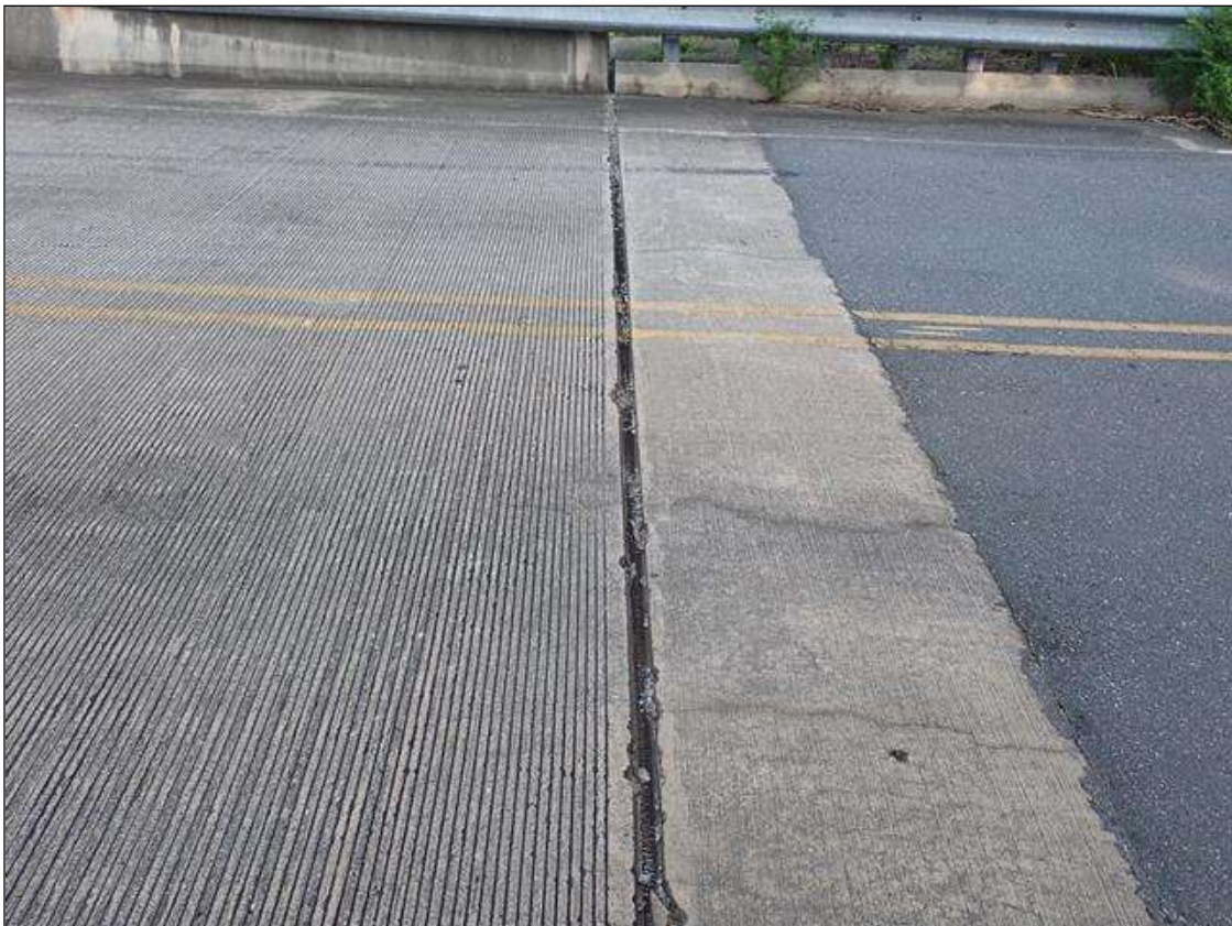
end bent 2 joint
