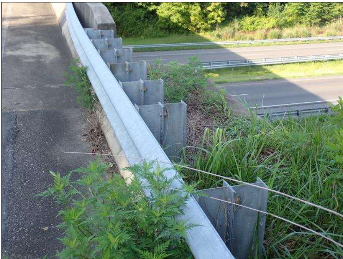
northwest guardrail transition
