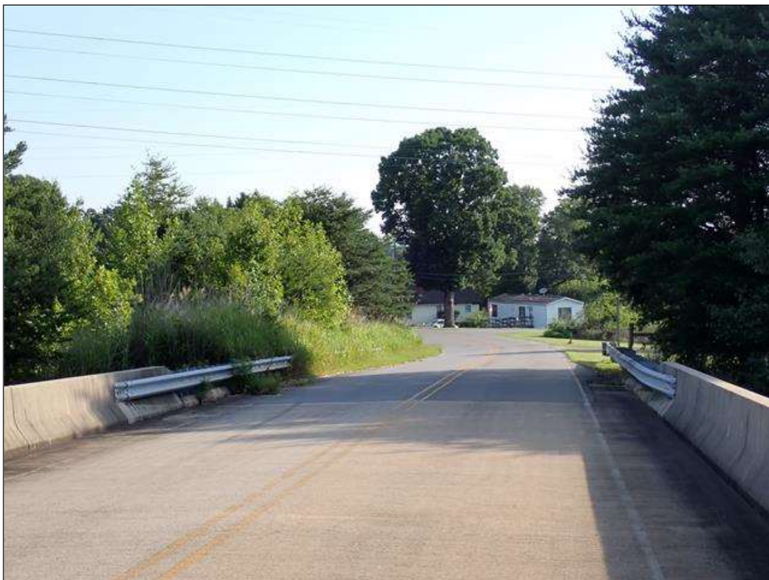
north approach looking north
