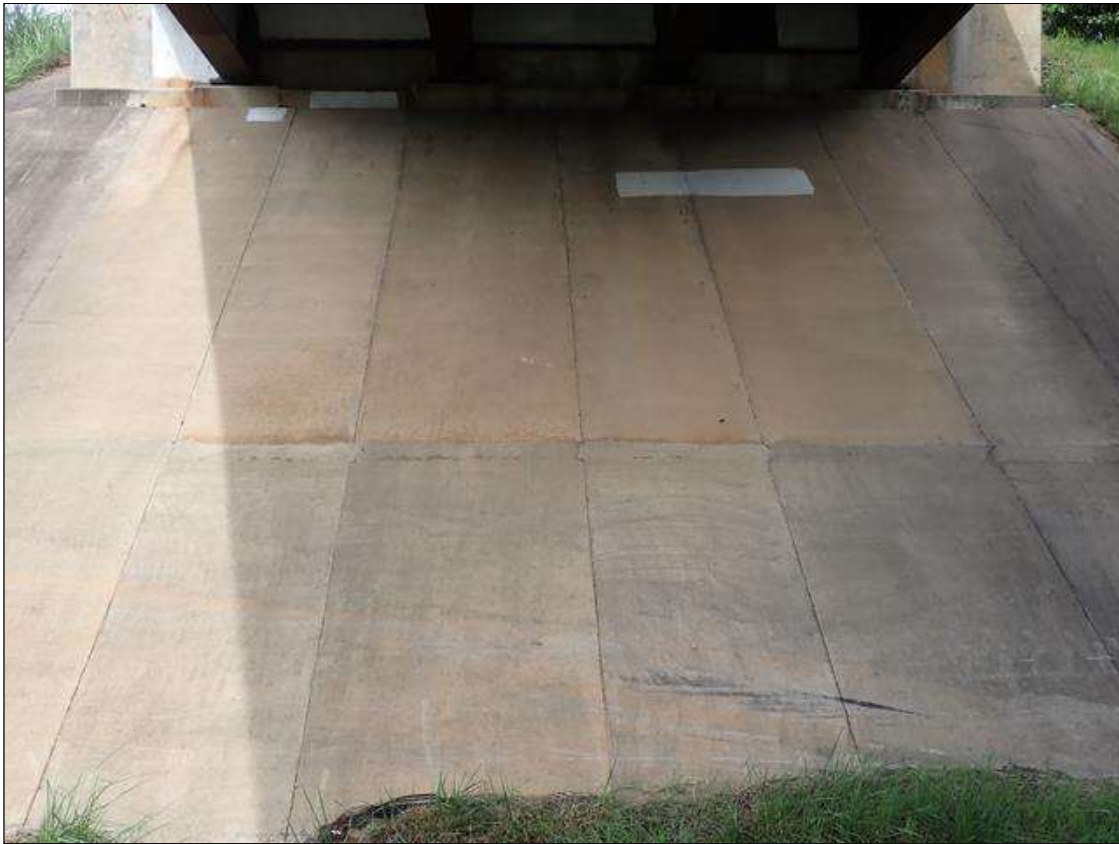
end bent 2 slope protection
