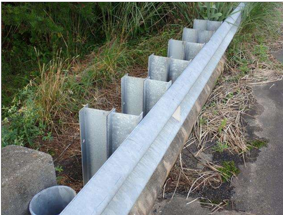
southeast guardrail transition
