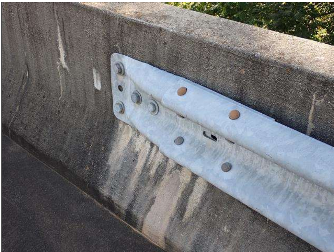
southeast guardrail attachment
