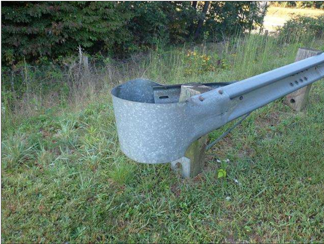
northeast guardrail termination
