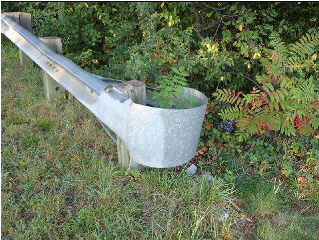
northwest guardrail termination
