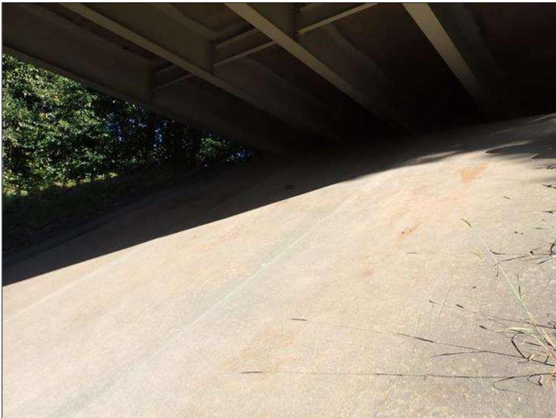
end bent 2 slope protection
