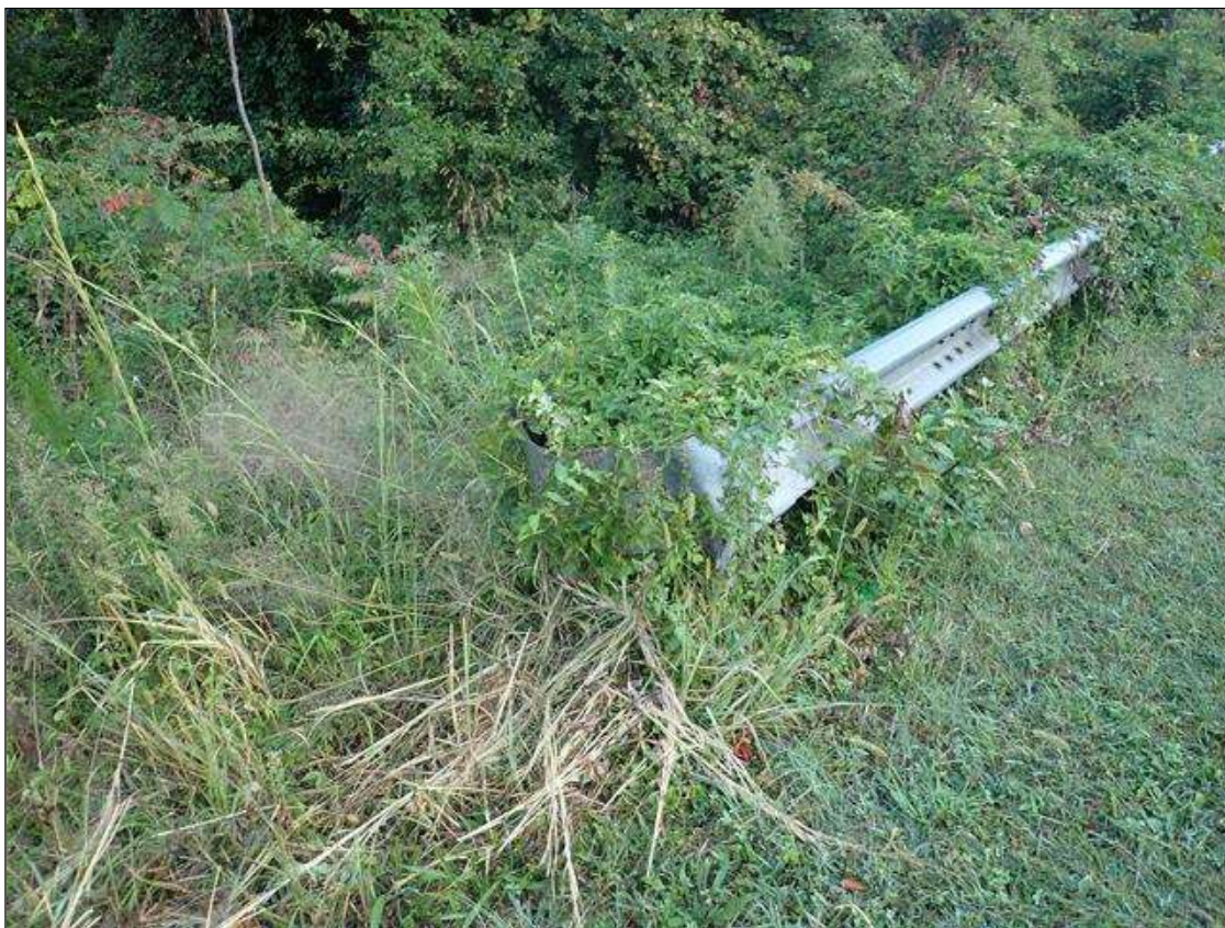
southwest guardrail termination
