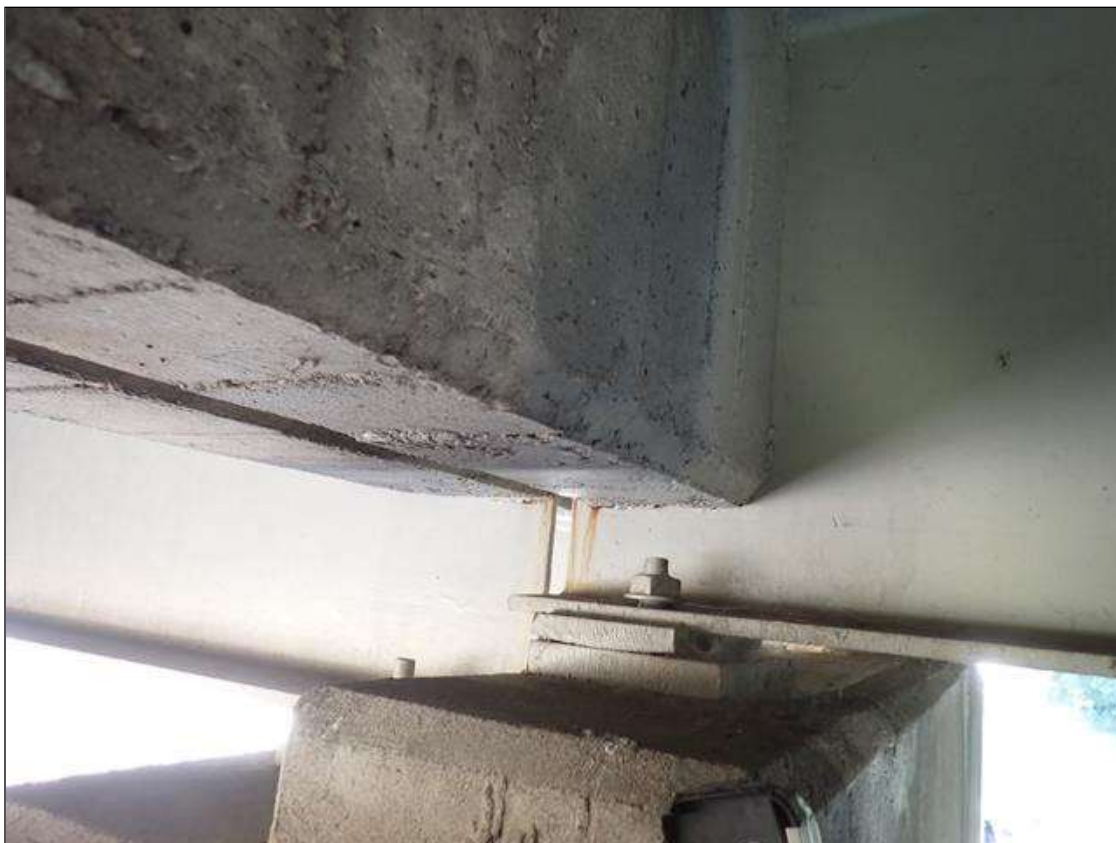
interior beams over bent 1 (bent 3 similar)
