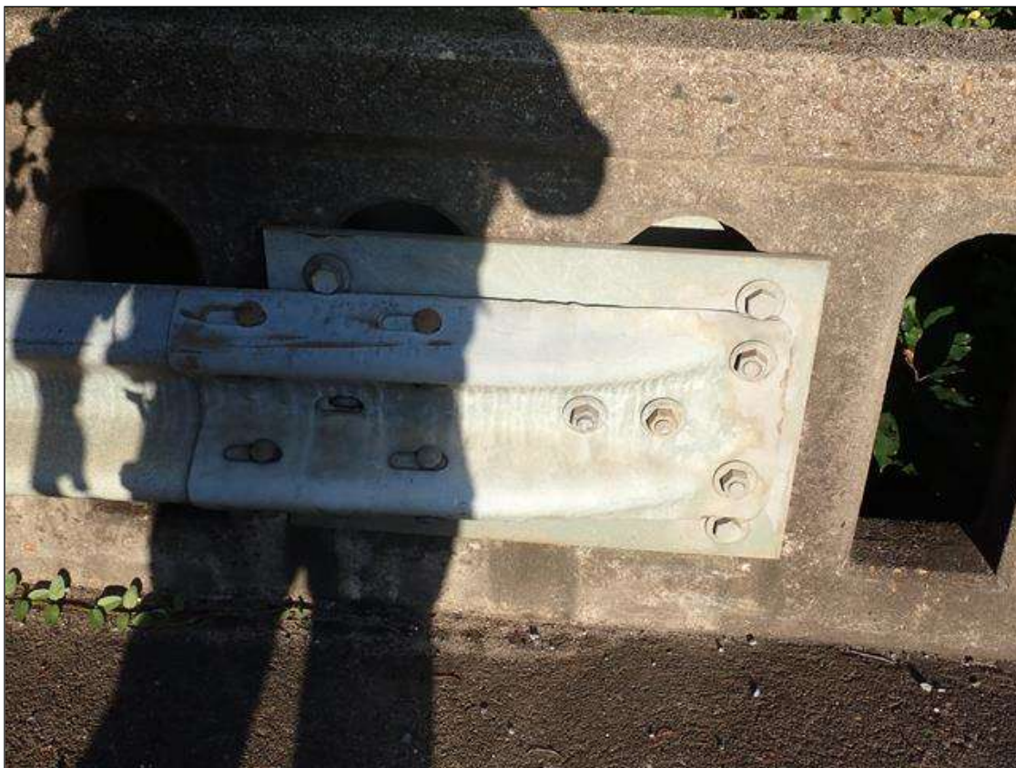
southwest guardrail attachment
