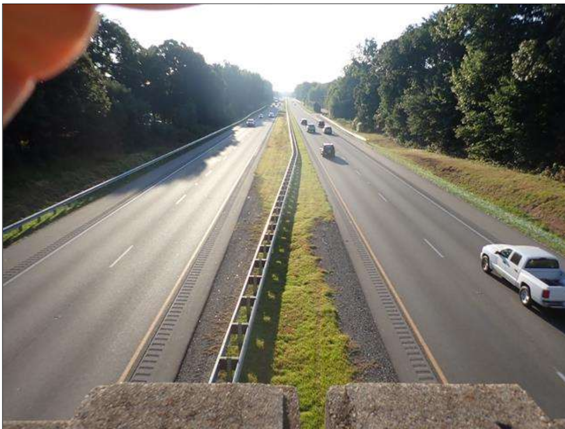
roadway looking east
