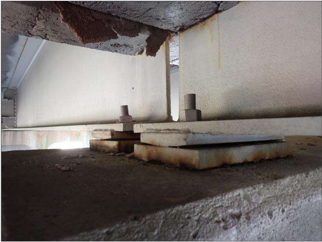
interior bearing assembly at bent 2
