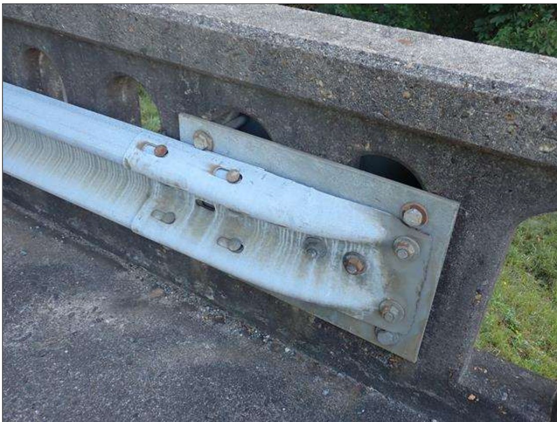
northeast guardrail attachment
