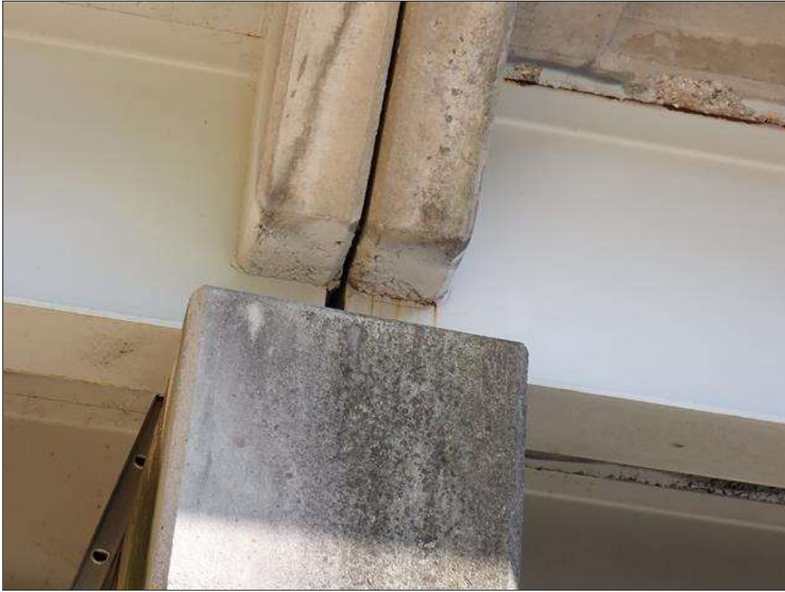
Span 3 Beam 1: (PAR) at bent 3, web adjacent to diaphragm, painted over section loss (approximately 3/8 inch average remaining x 9 inch x 1 inch) with corrosion reinitiated; no safe ladder access to exterior face
