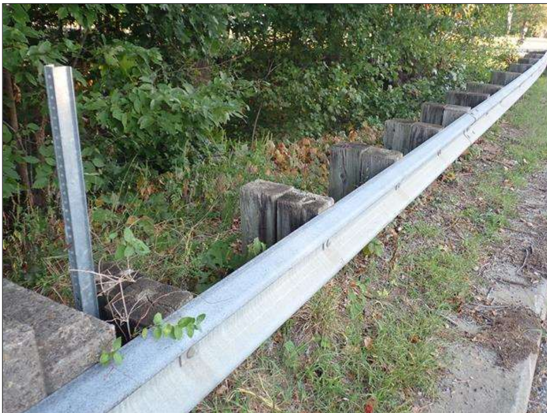
northwest guardrail transition
