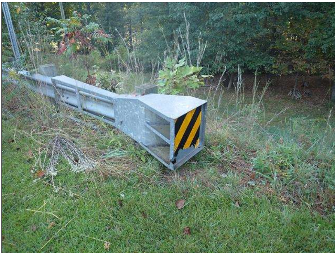
southeast guardrail termination
