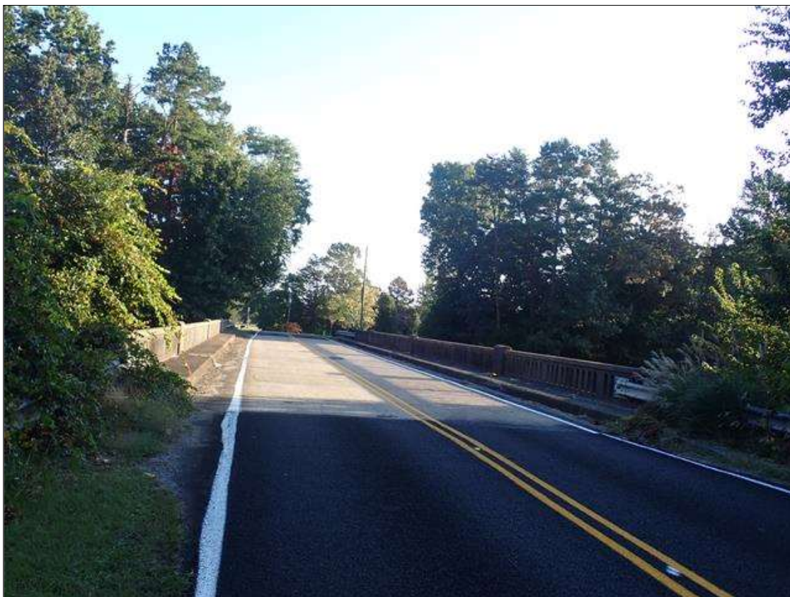
south approach looking north
