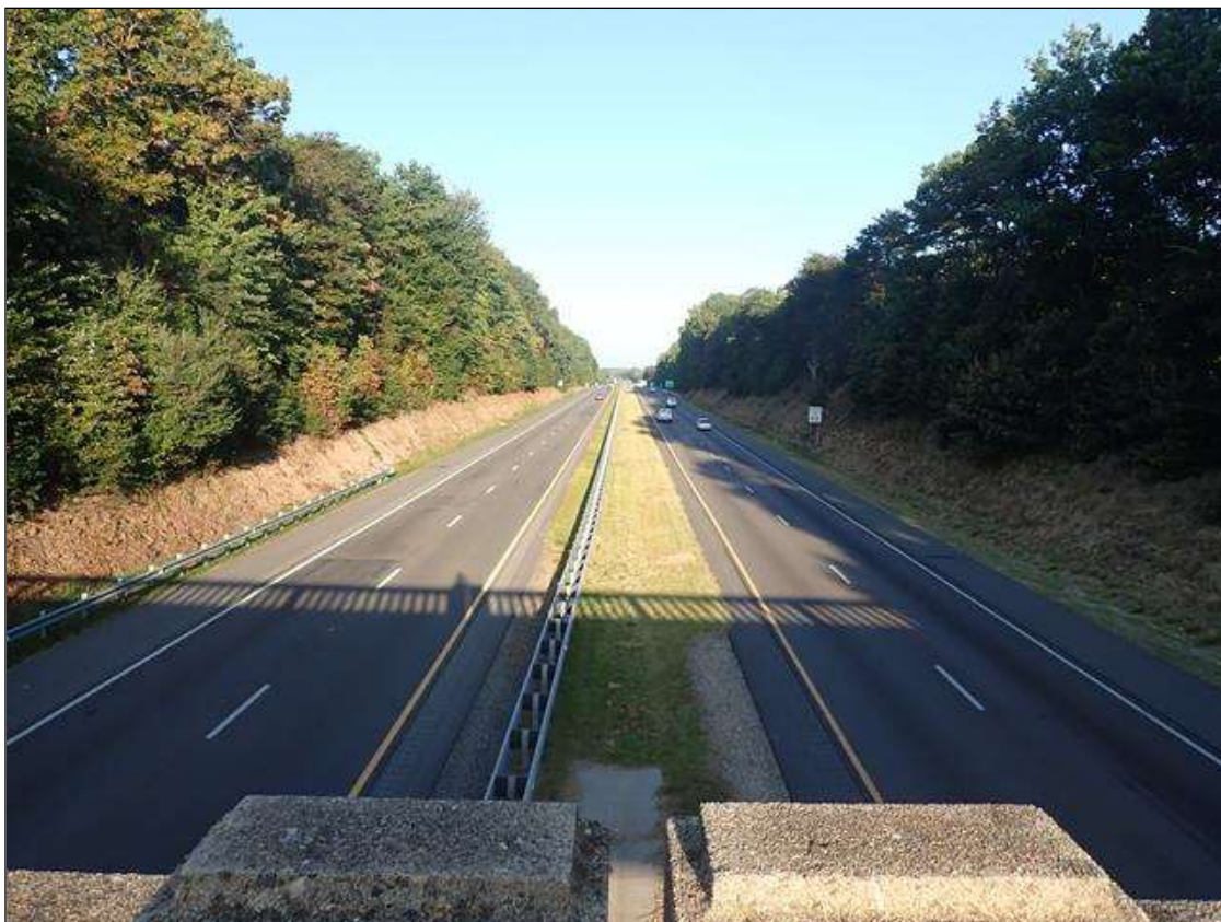
roadway looking west
