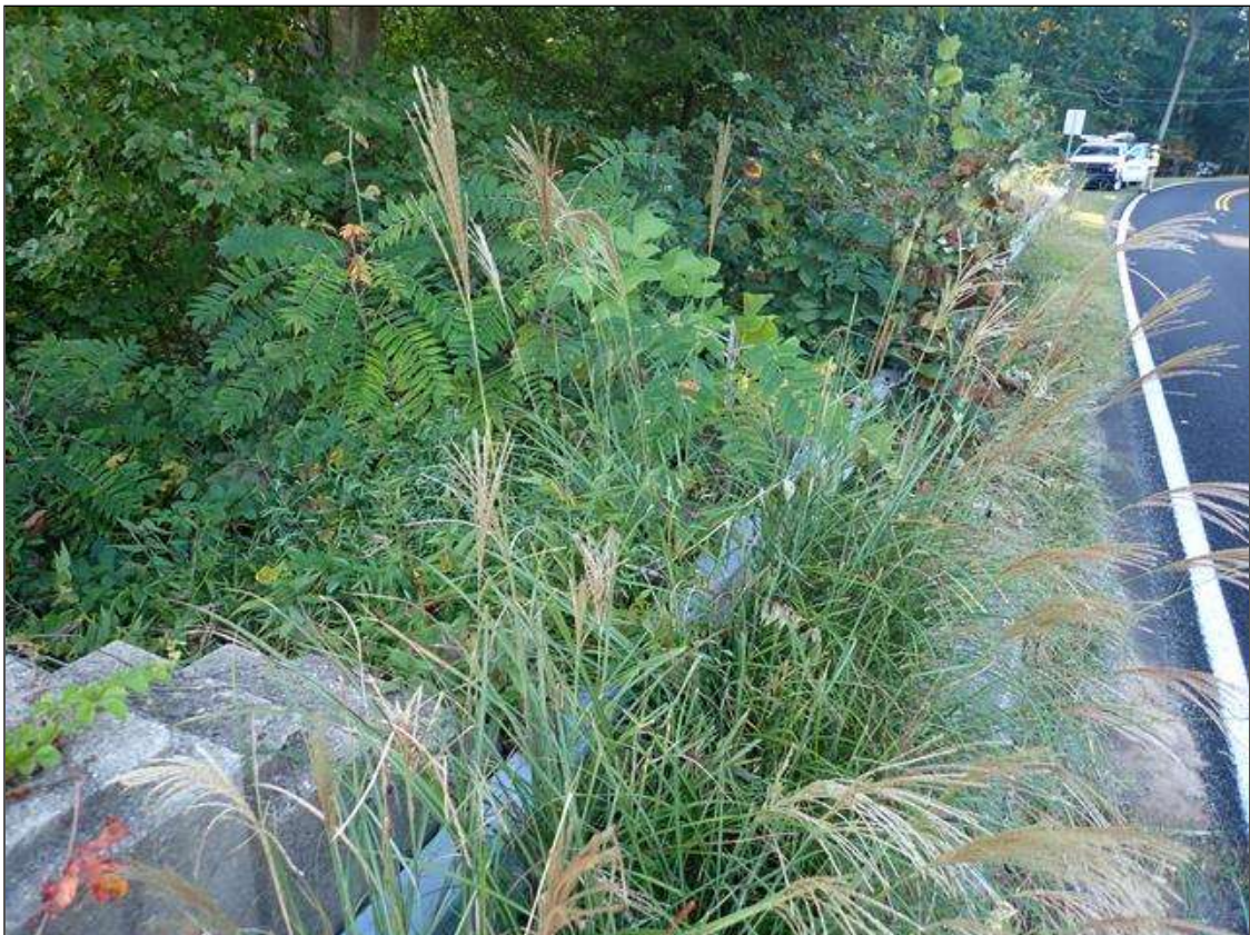
southeast guardrail transition
