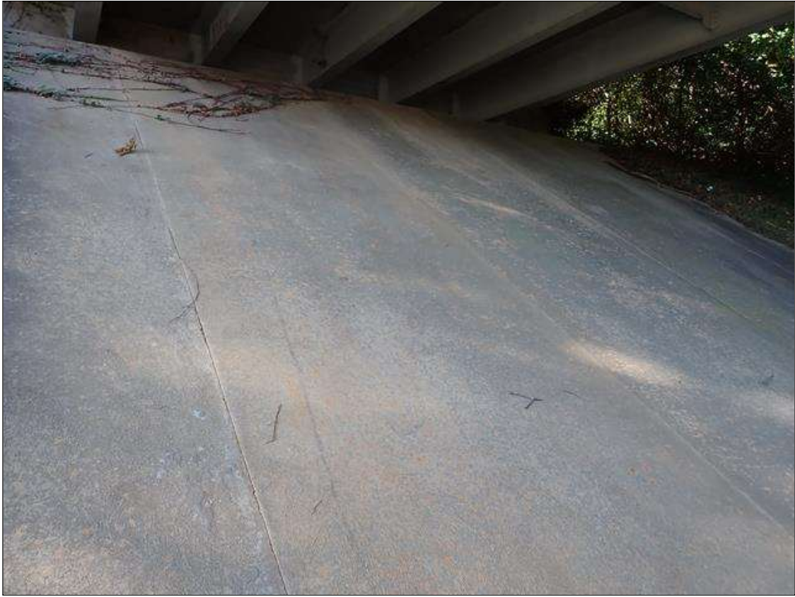
end bent 1 slope protection
