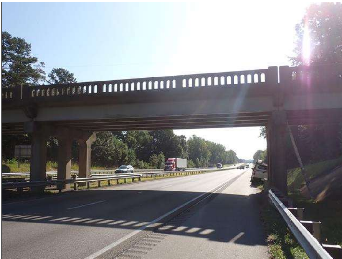
roadway under span 2, looking east (I-40 eastbound)
