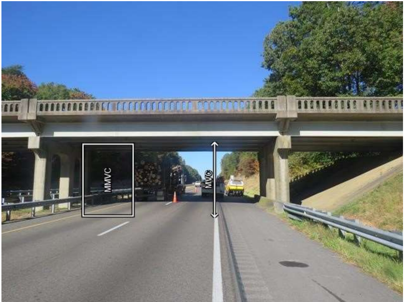
Looking West on I-40 Clearance
