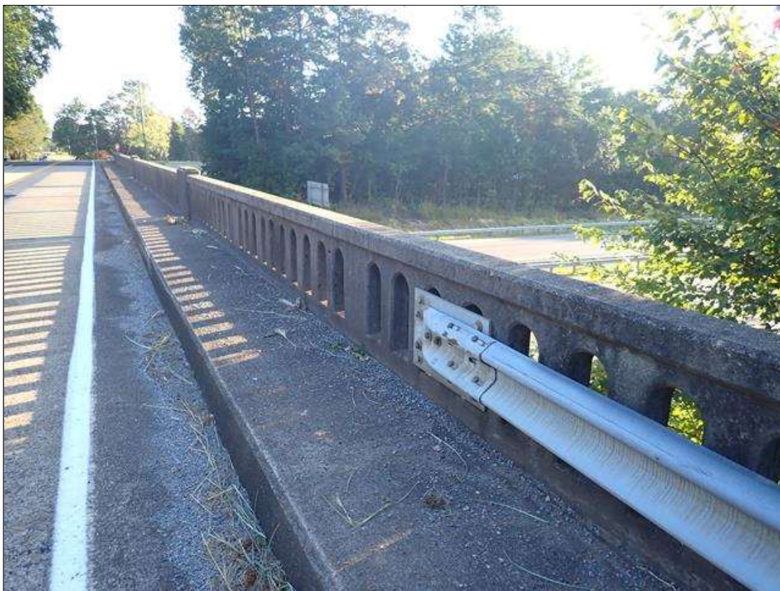
right bridge rail
