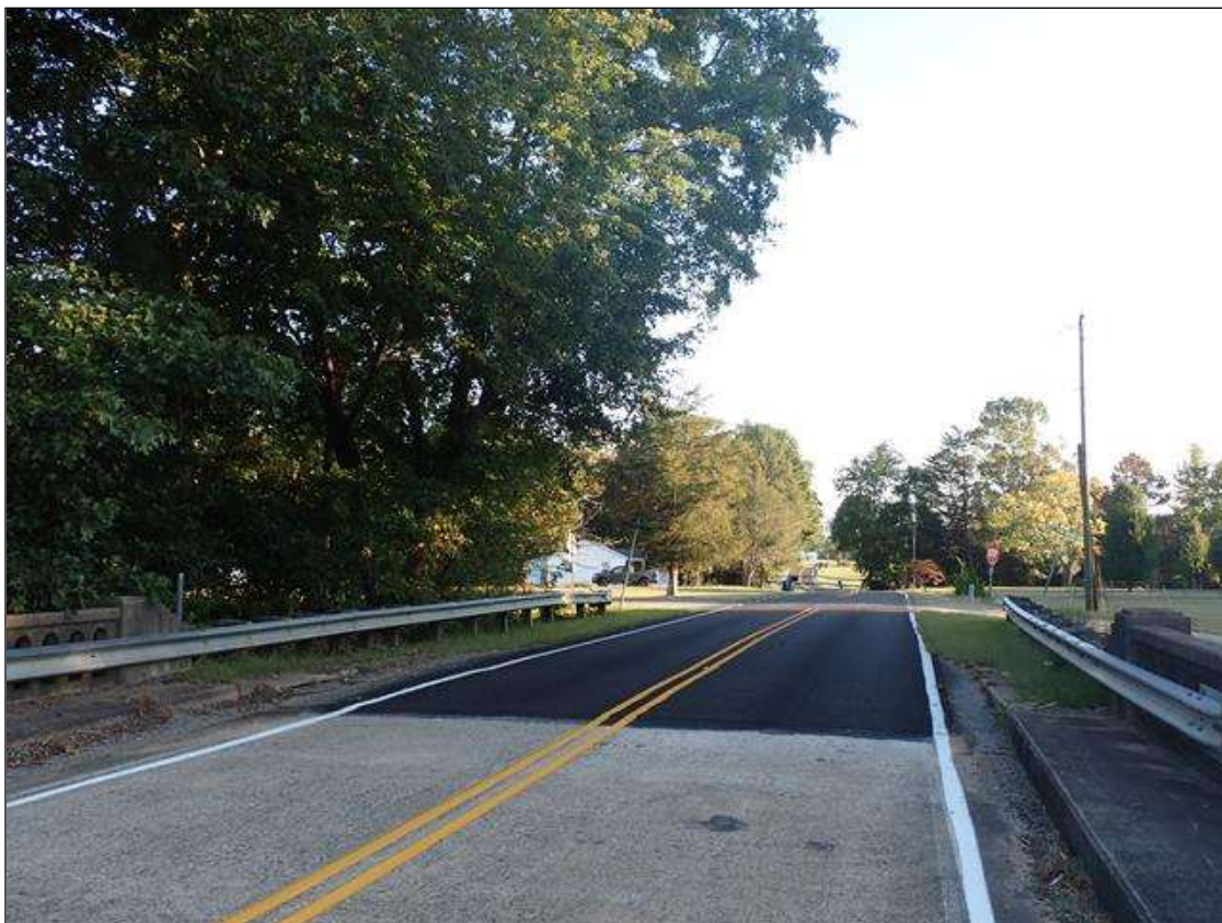
north approach looking north
