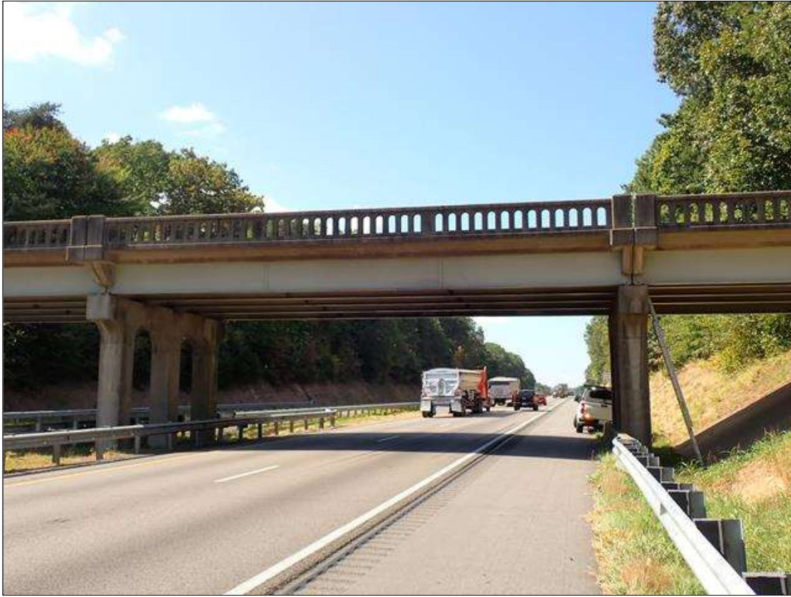
roadway under span 3, looking west (I-40 westbound)
