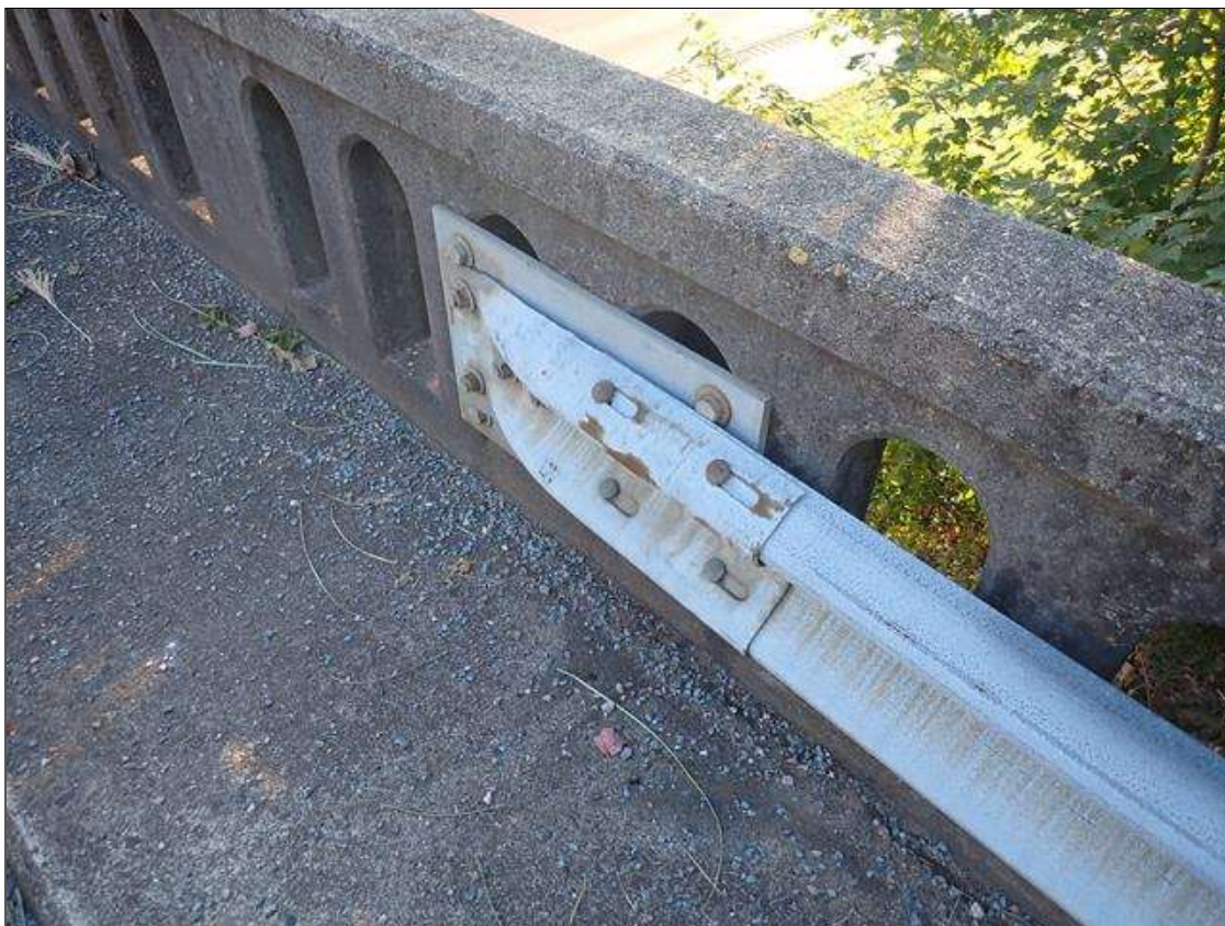
southeast guardrail attachment
