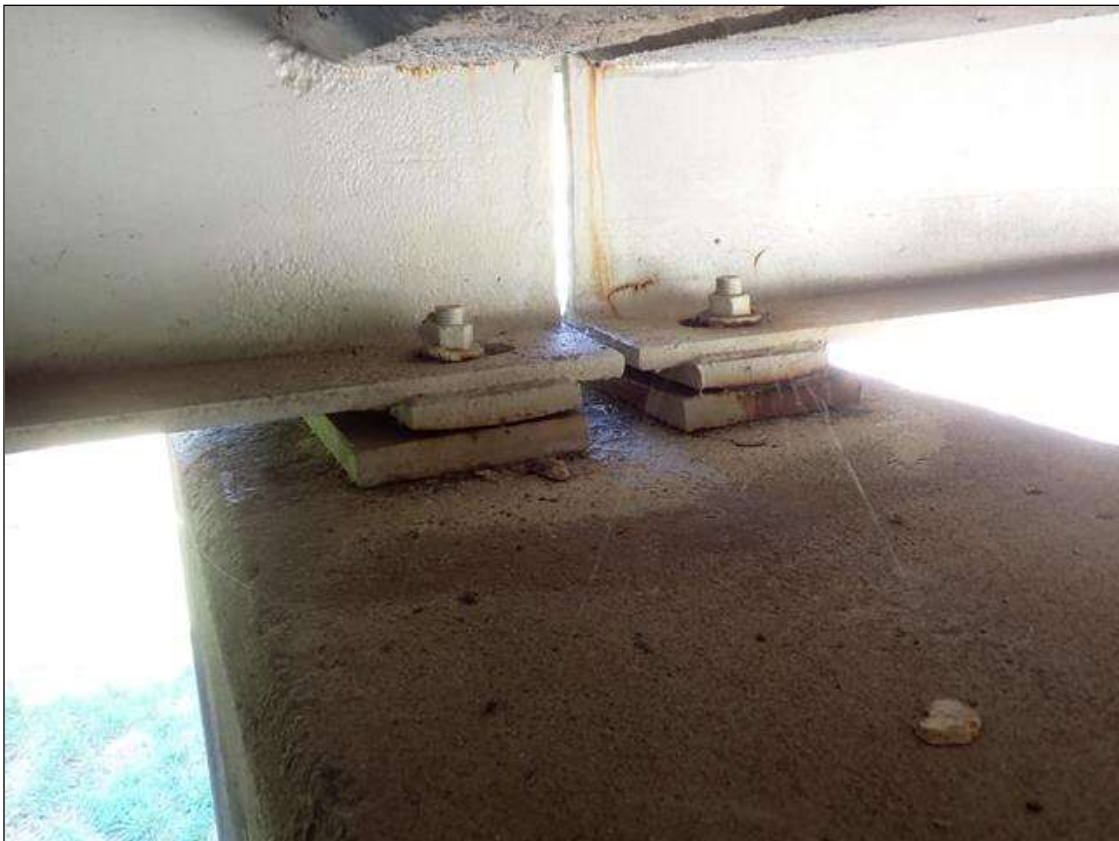
interior bearing assembly at bent 1 (bent 3 similar)
