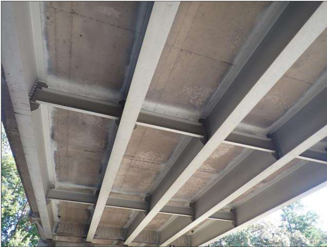
superstructure underside, span 2 (span 3 similar)
