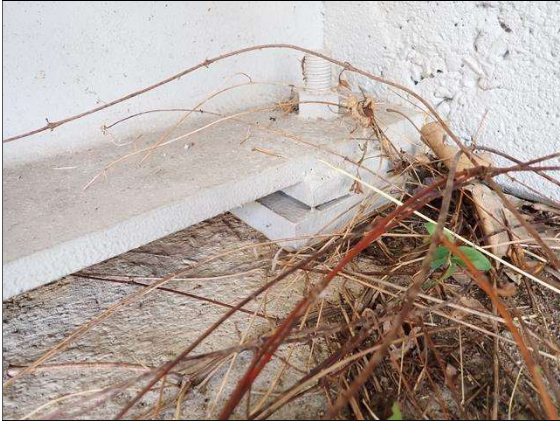
end bearing assembly
