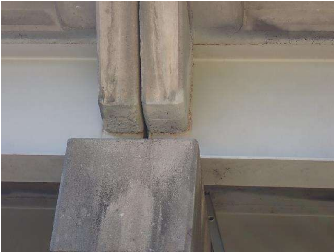
Span 4 Beam 5: (PAR) at bent 3, web adjacent to diaphragm, painted over section loss (approximately 3/8 inch average remaining x 10 inch x 1 inch) with corrosion reinitiated; underside of bottom flange, rust scale; no safe ladder access to exterior face
