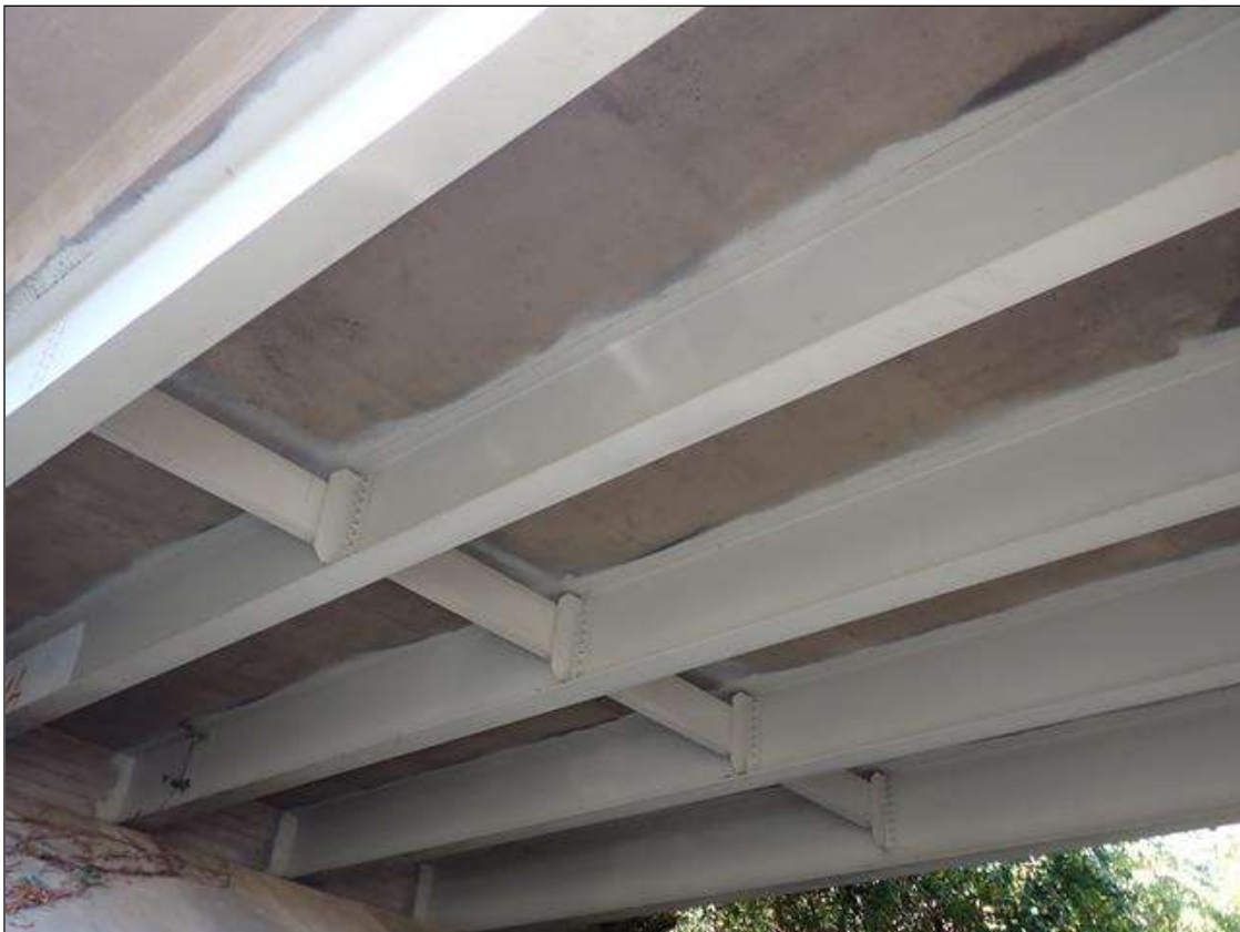
superstructure underside, span 1 (span 4 similar)
