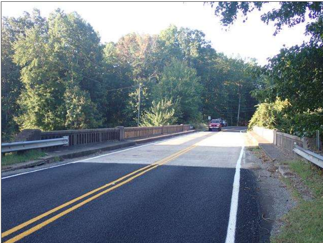
north approach looking south
