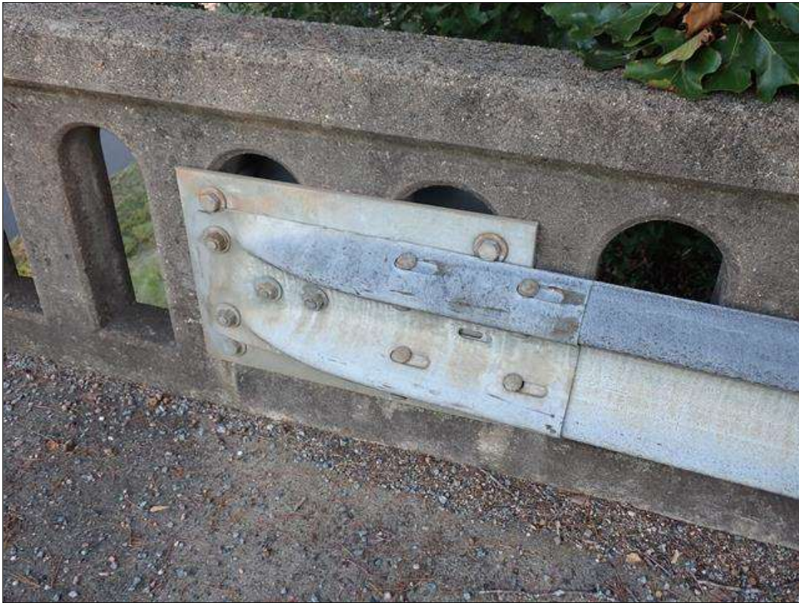
northwest guardrail attachment
