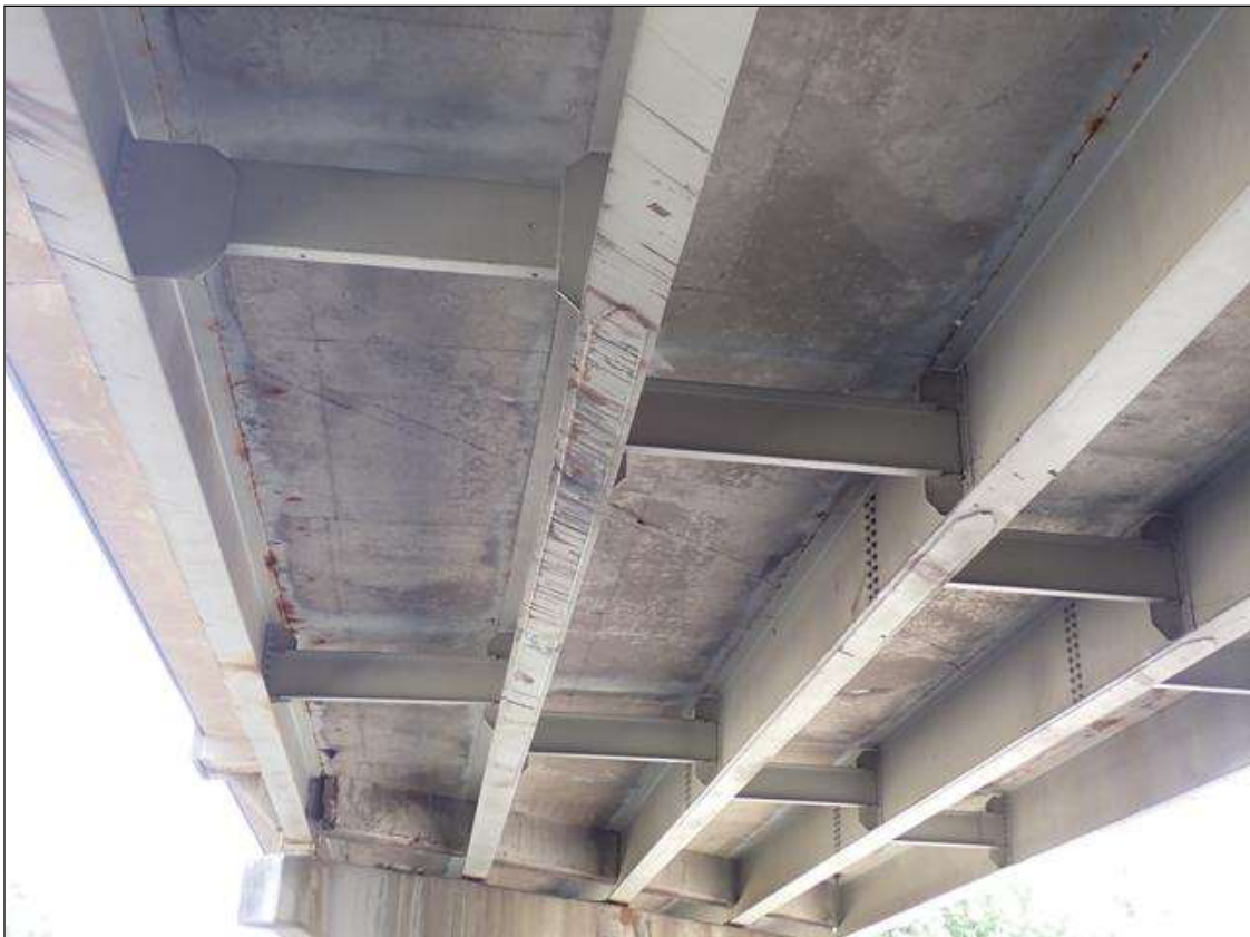
superstructure underside, span 2; note beam 1 previously replaced
