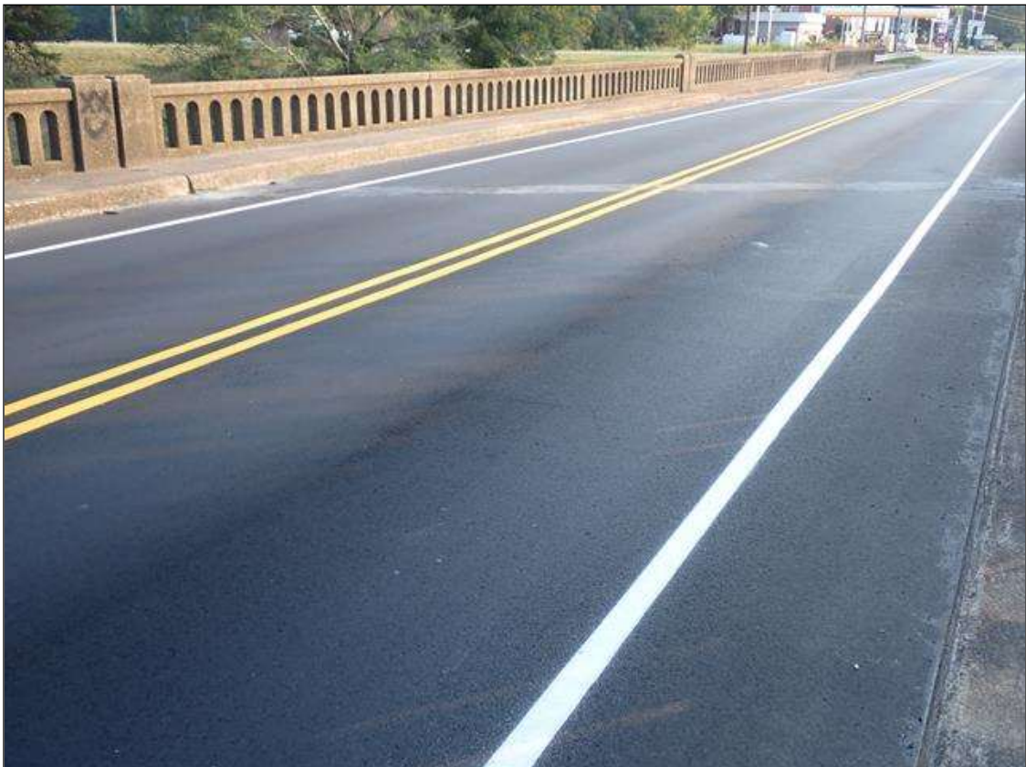
asphalt wearing surface
