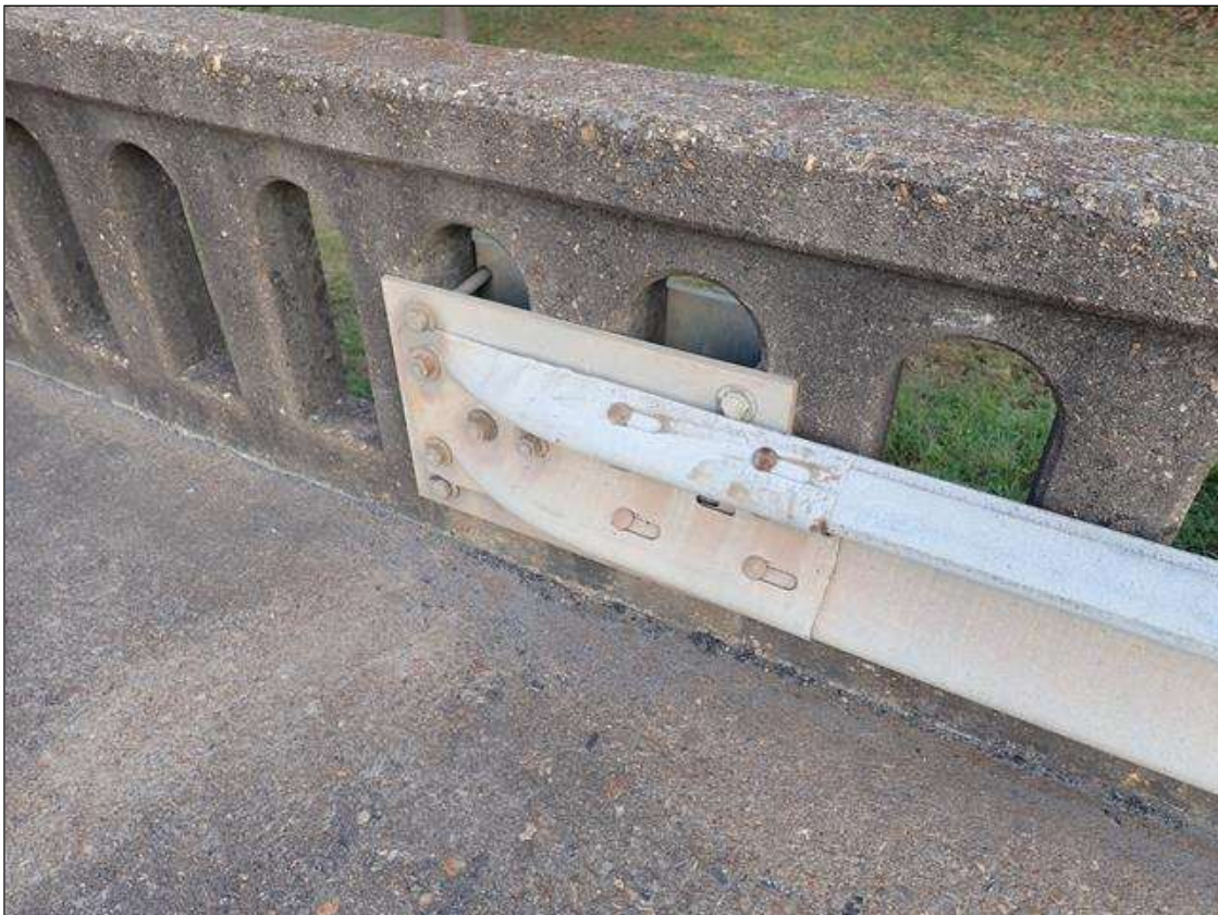
northwest guardrail attachment
