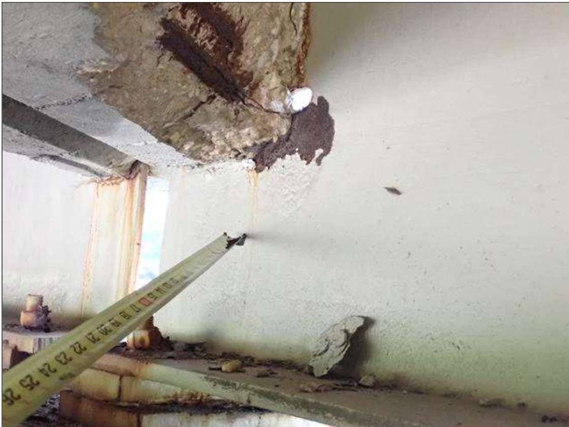
Span 4 Beam 1: (PAR) at bent 3, web adjacent to diaphragm, painted over section loss (3/8 inch average remaining x 6 inch x 4 inch); painted over pitting, lower web (up to 1/8 inch deep x 2 feet x 4 inch) with corrosion reinitiated
