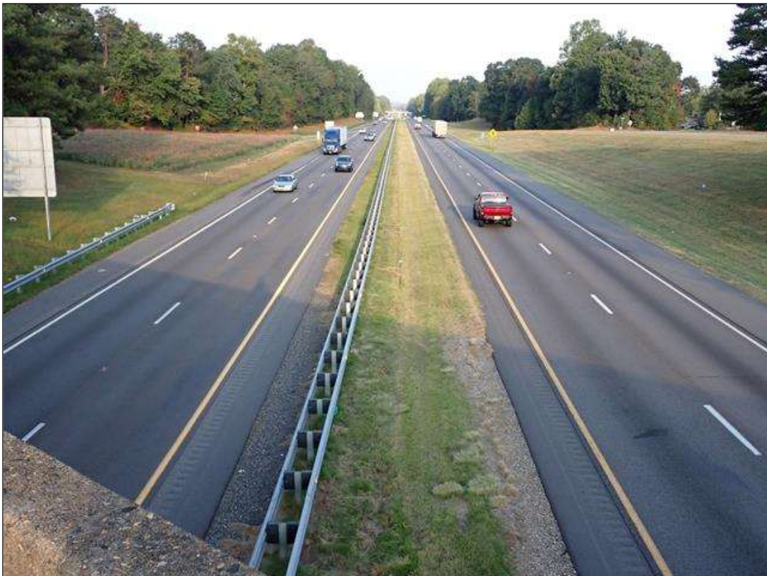
roadway looking west
