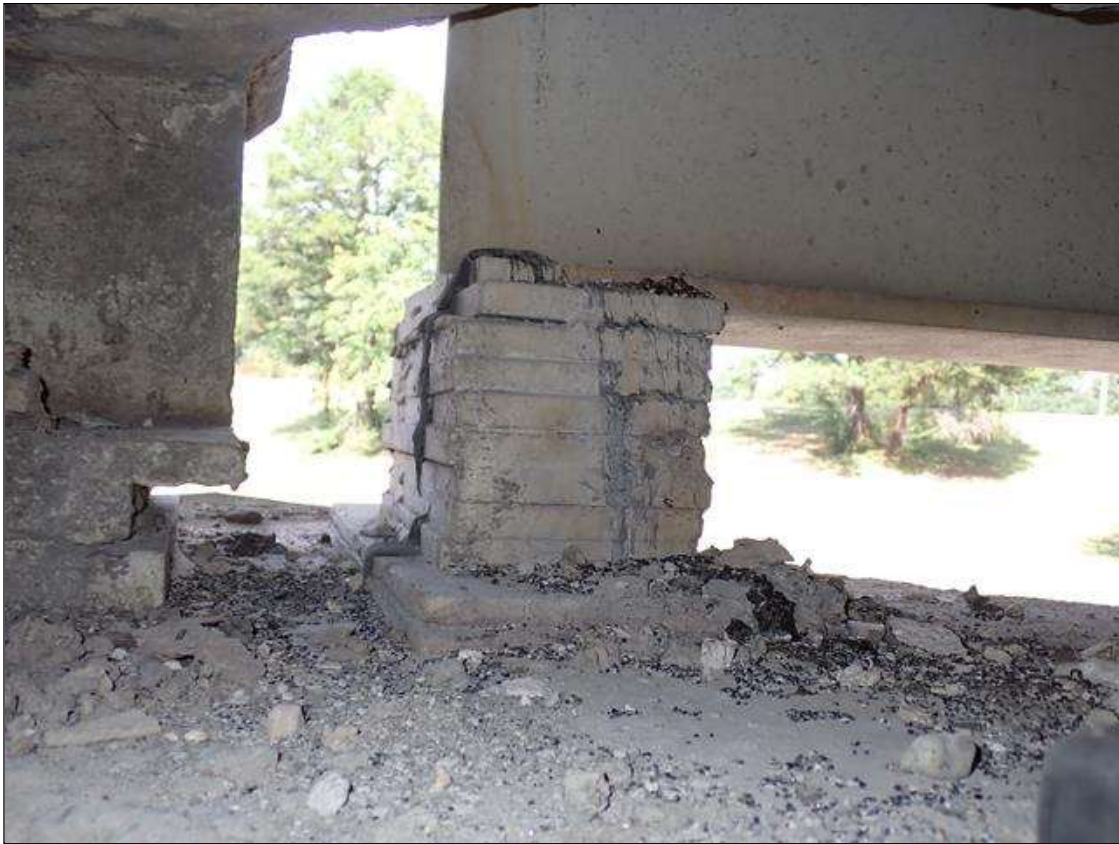
interior bearing assembly at bent 1, span 2 beam 1 (bent 2 similar)
