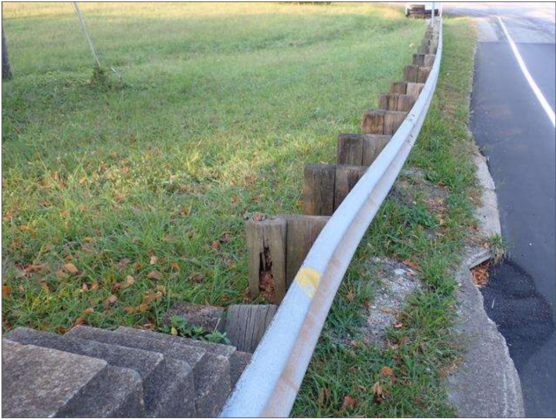
southeast guardrail transition
