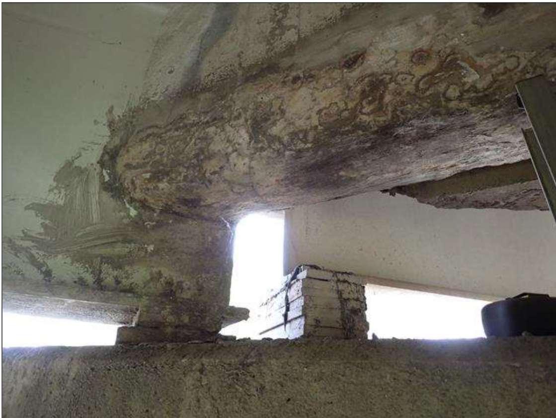
beams over bent 1 showing span 2 beam 1 (bent 2 similar)
