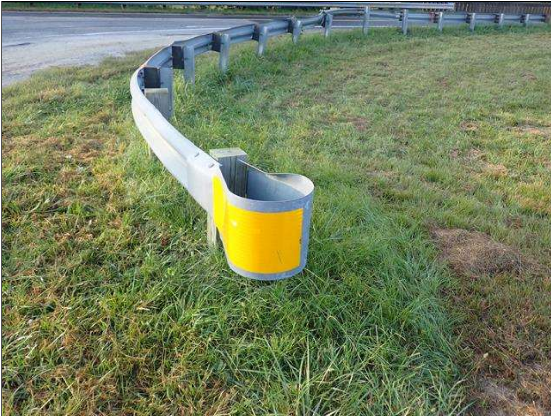
northwest guardrail termination
