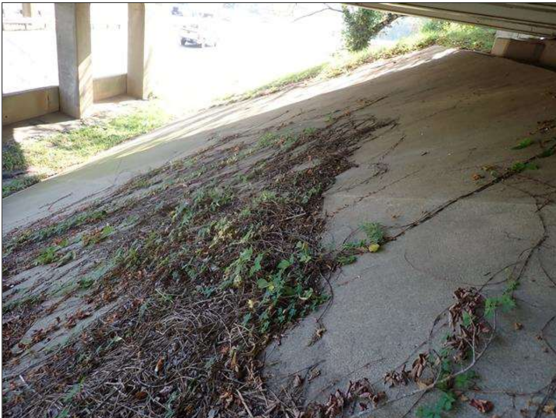
end bent 1 slope protection
