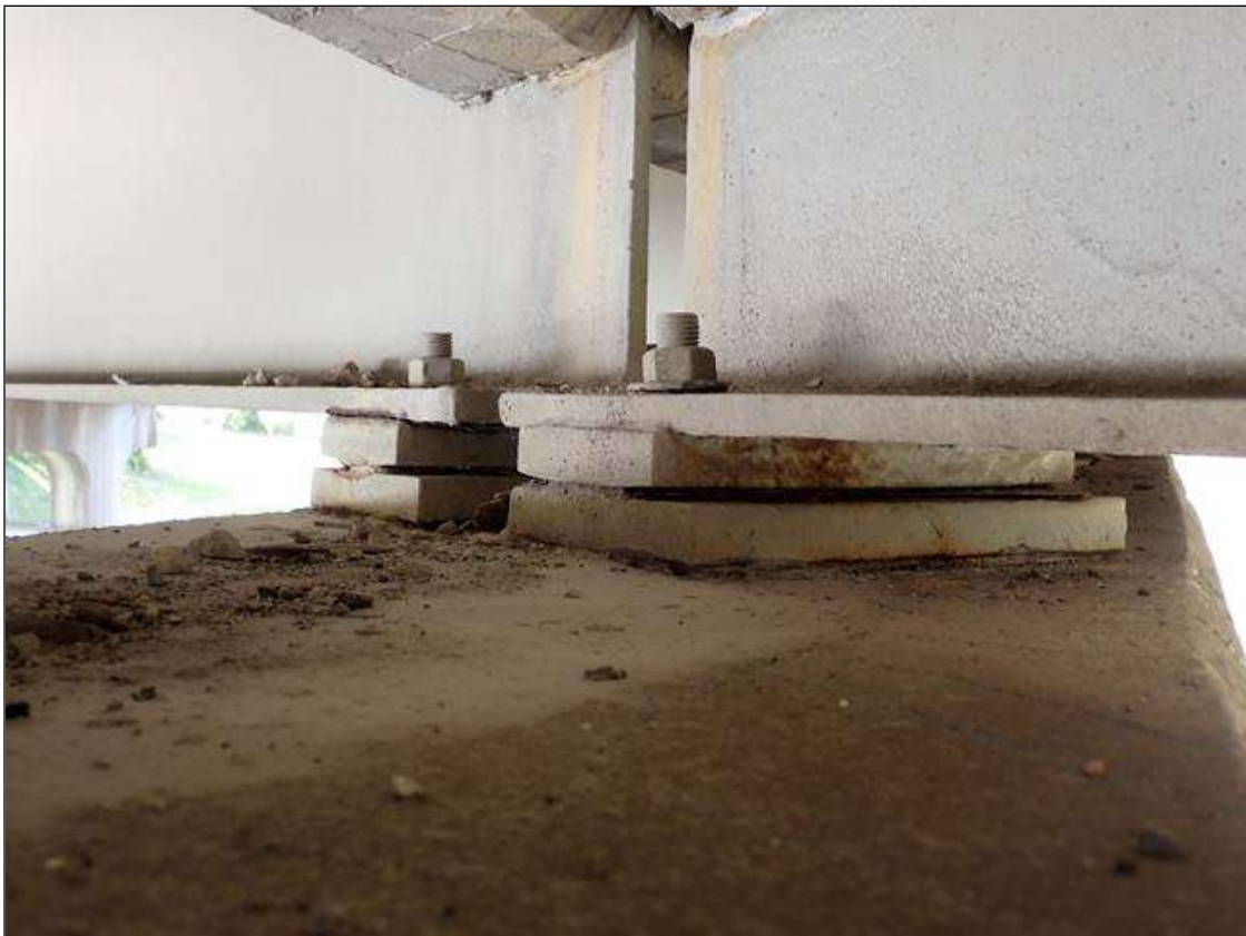
interior bearing assembly
