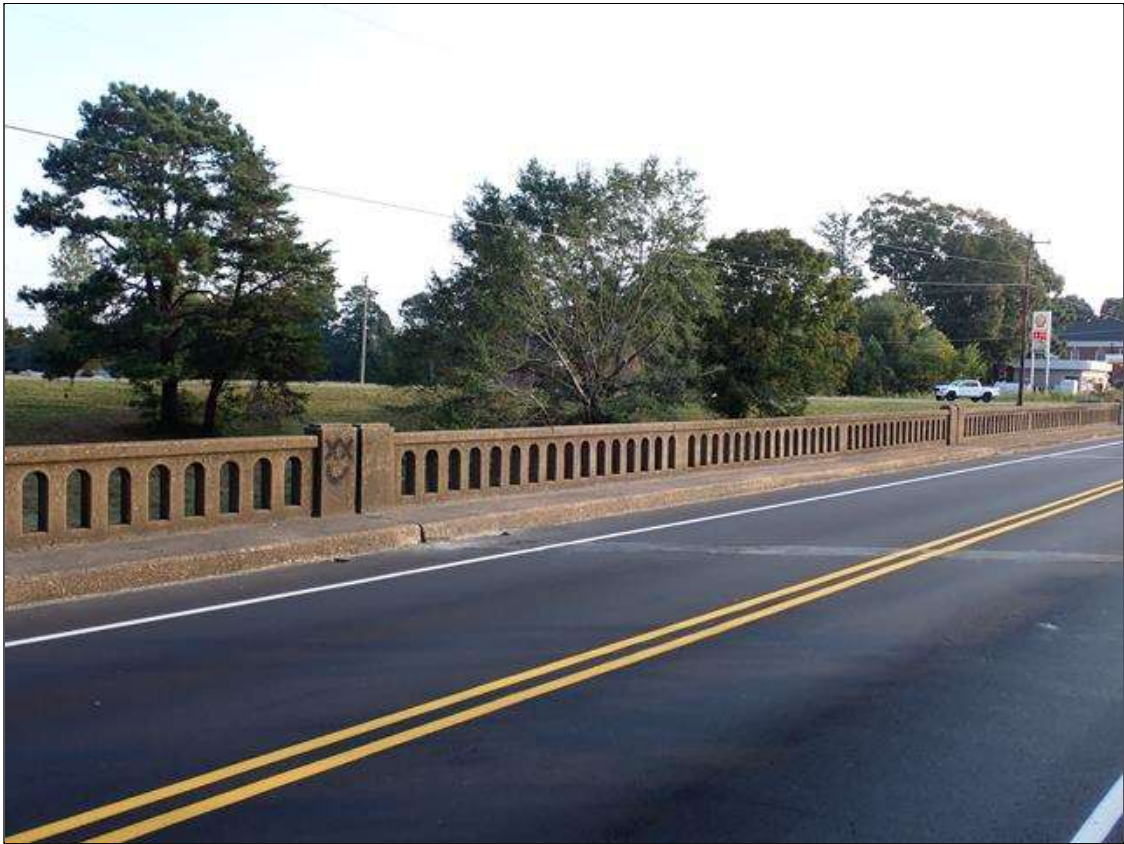
left bridge rail
