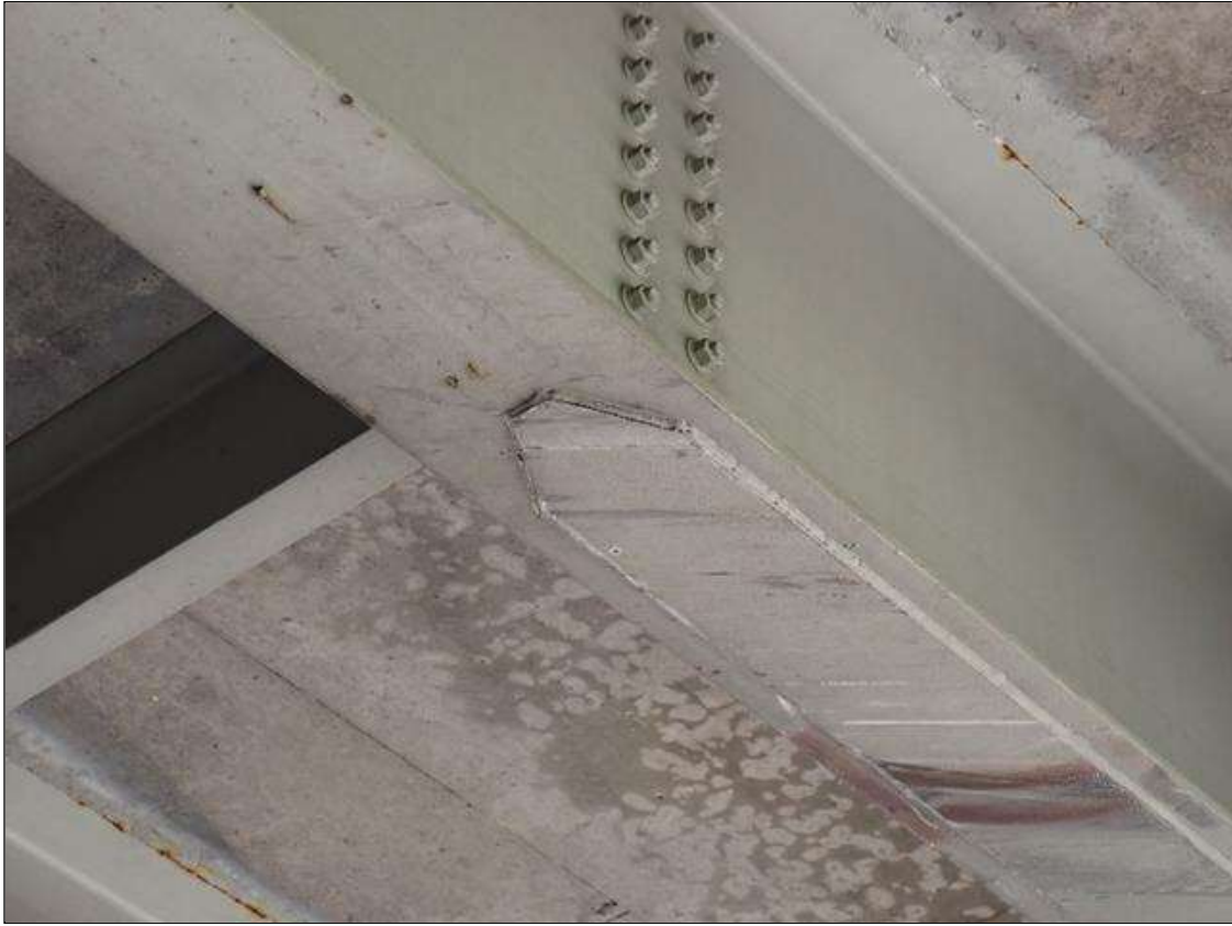
typical bottom flange cover plate end, spans 2 and 3
