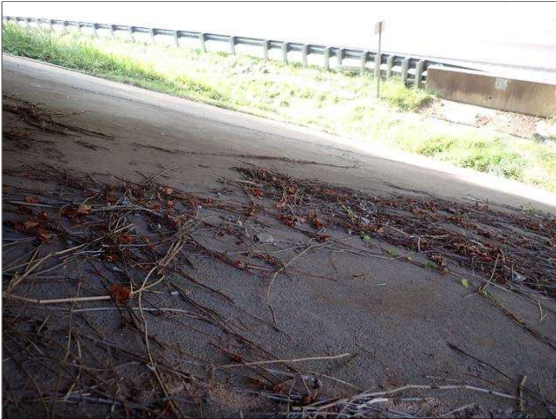
end bent 2 slope protection
