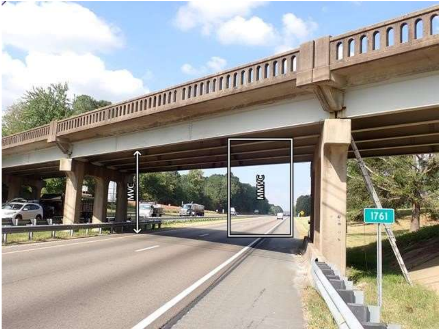
roadway under span 3, looking west (I-40 westbound)
