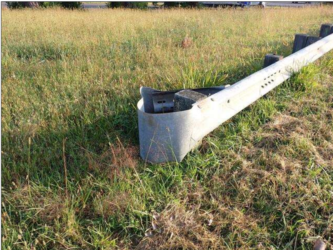
southwest guardrail termination
