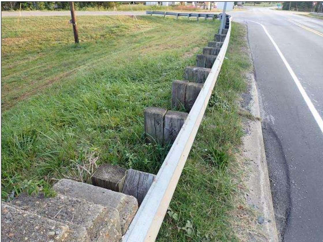
northwest guardrail transition
