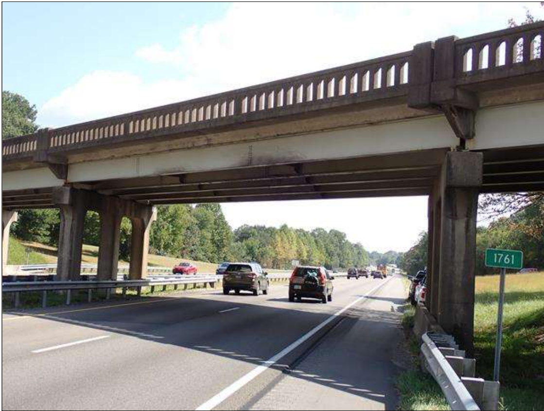
roadway under span 2, looking east (I-40 eastbound)
