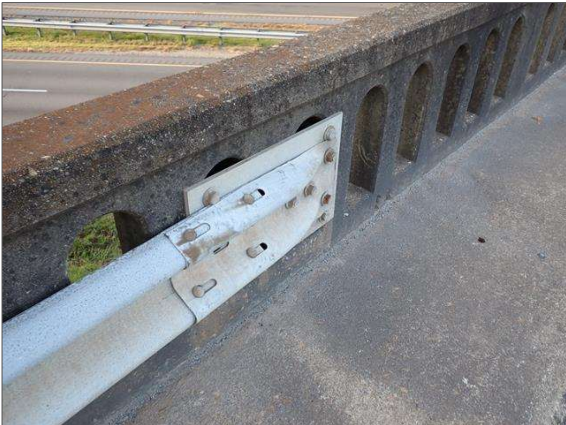
northeast guardrail attachment
