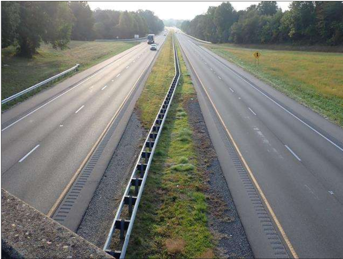
roadway looking east
