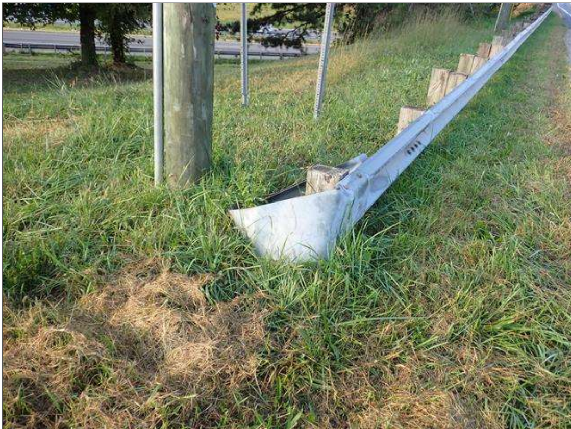
northeast guardrail termination
