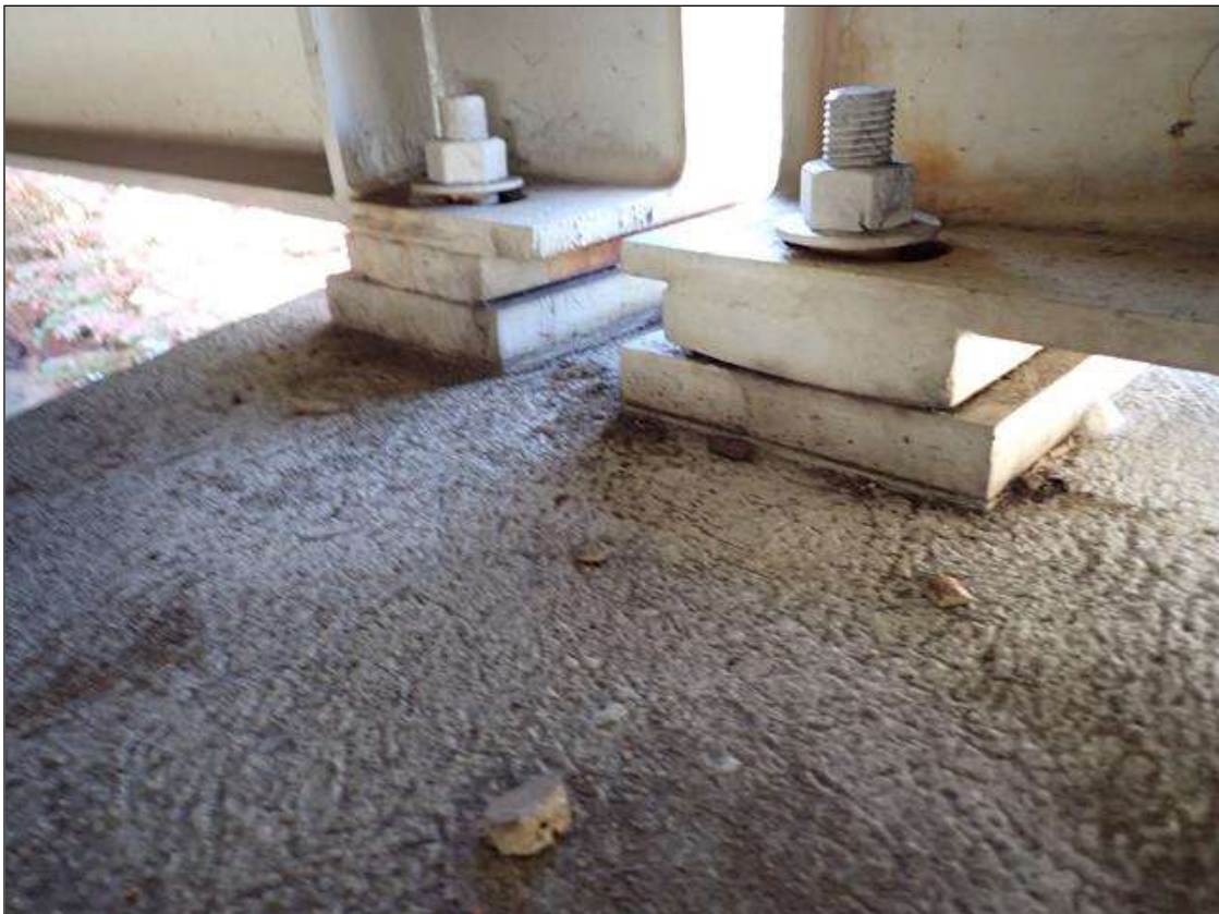
interior bearing assembly
