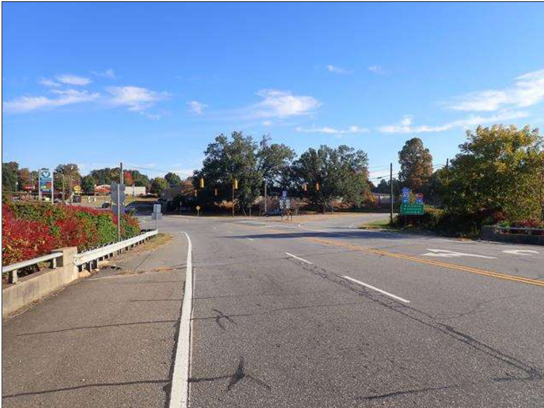
north approach looking north
