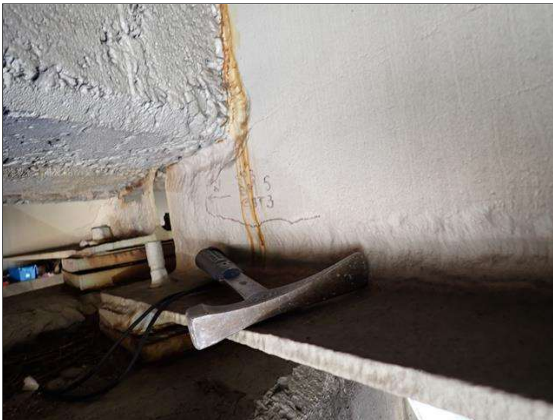
Span 3 Beam 5: (PAR) at bent 3, painted over section loss: bottom flange (0.45 inch average remaining x 1 foot); web (1/4 in average remaining x 2 foot x 9 inch) with corrosion reinitiated
