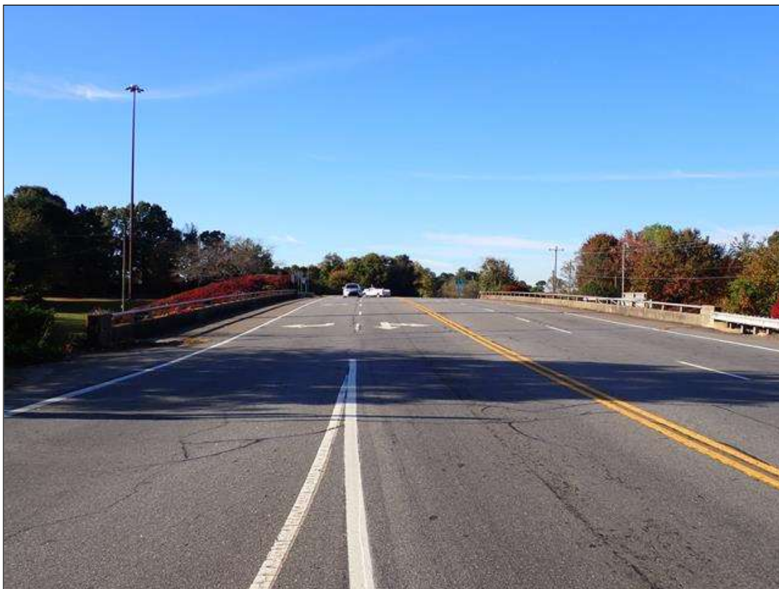
north approach looking south
