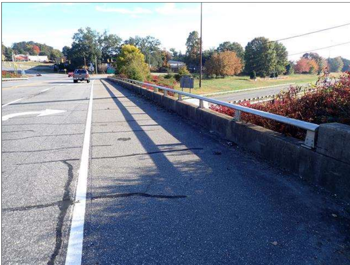
right bridge rail
