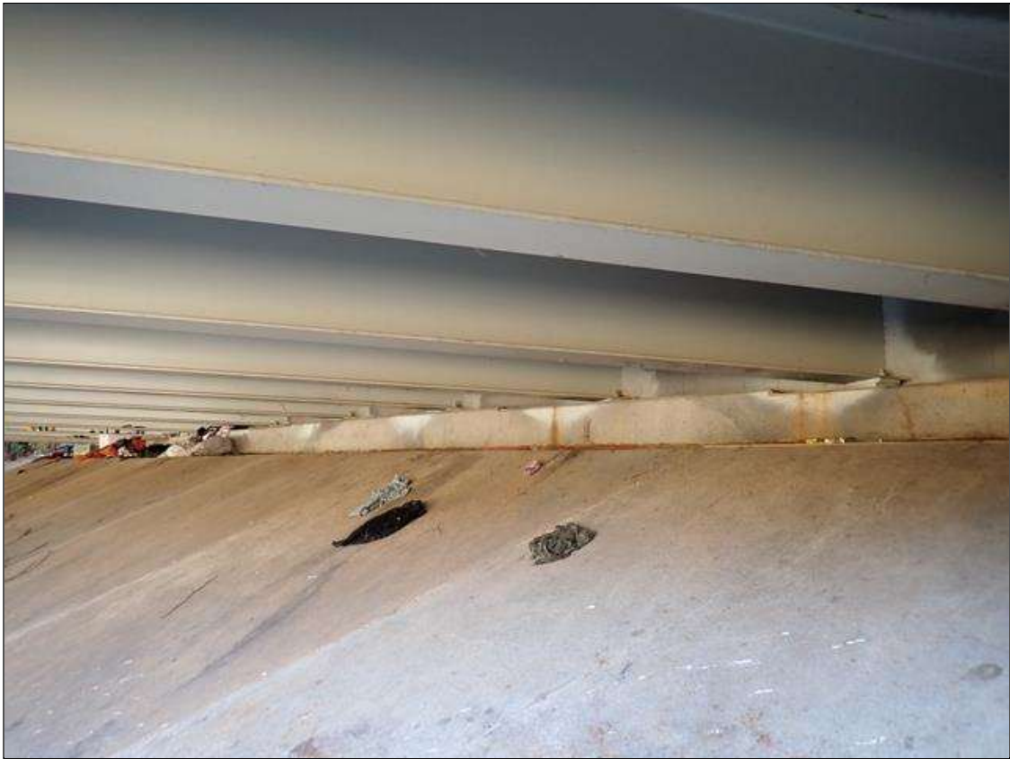
end bent 1 and slope protection
