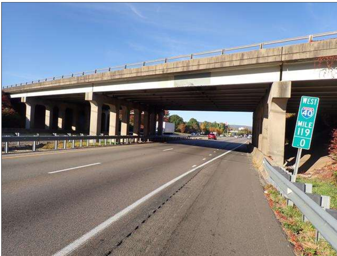
roadway under span 3, looking west (I-40 westbound)
