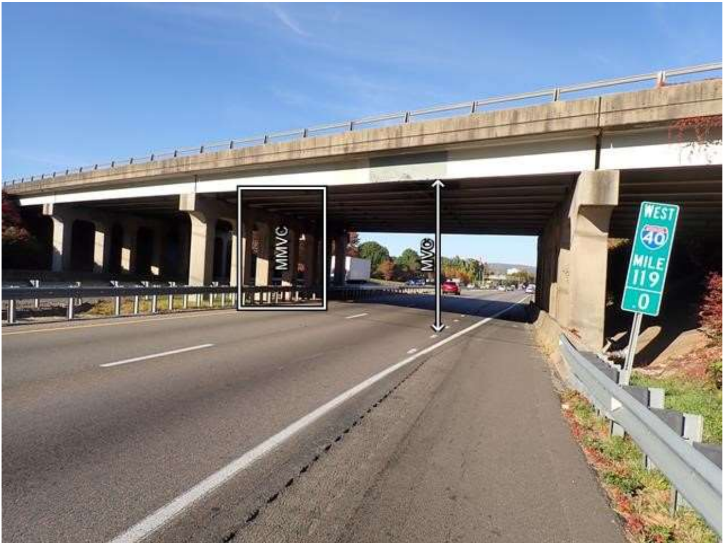
roadway under span 3, looking west
