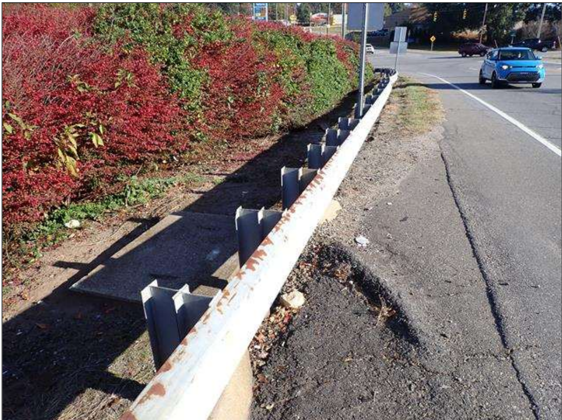
northwest guardrail transition
