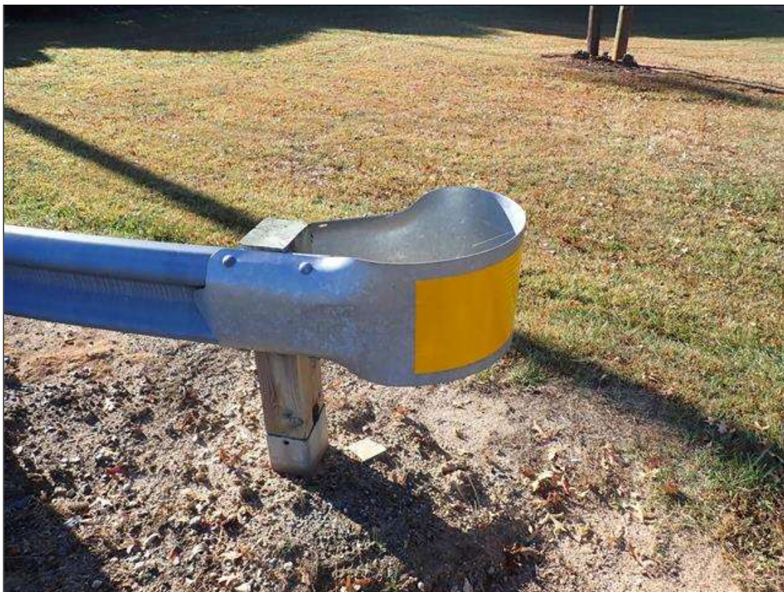
northwest guardrail termination
