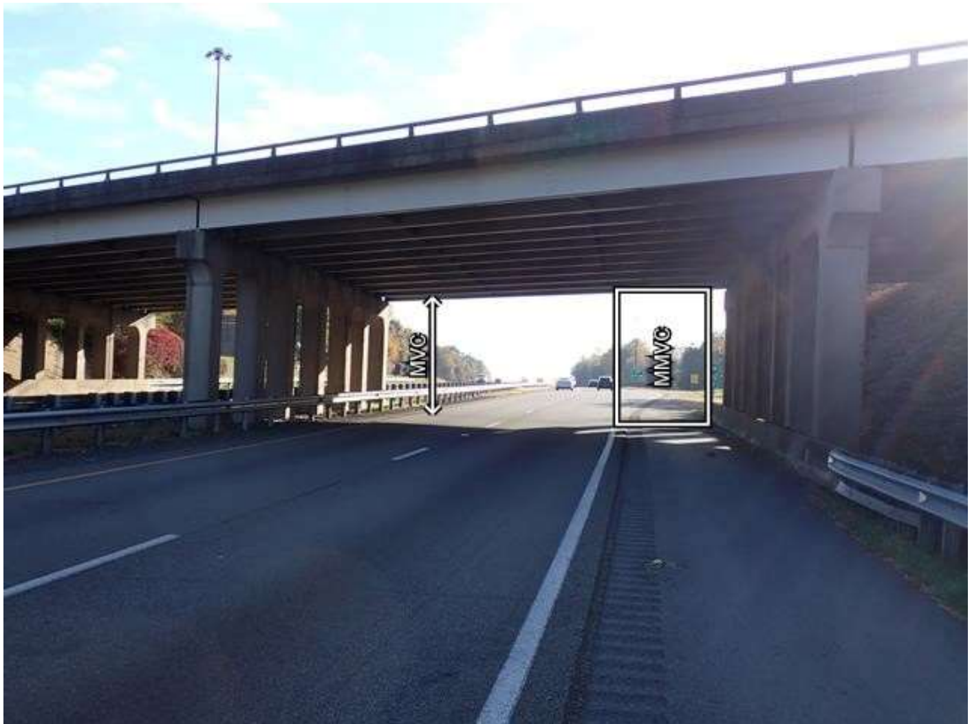
roadway under span 2, looking east
