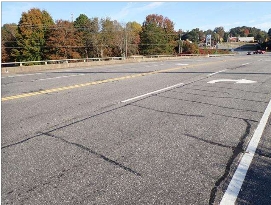
asphalt wearing surface
