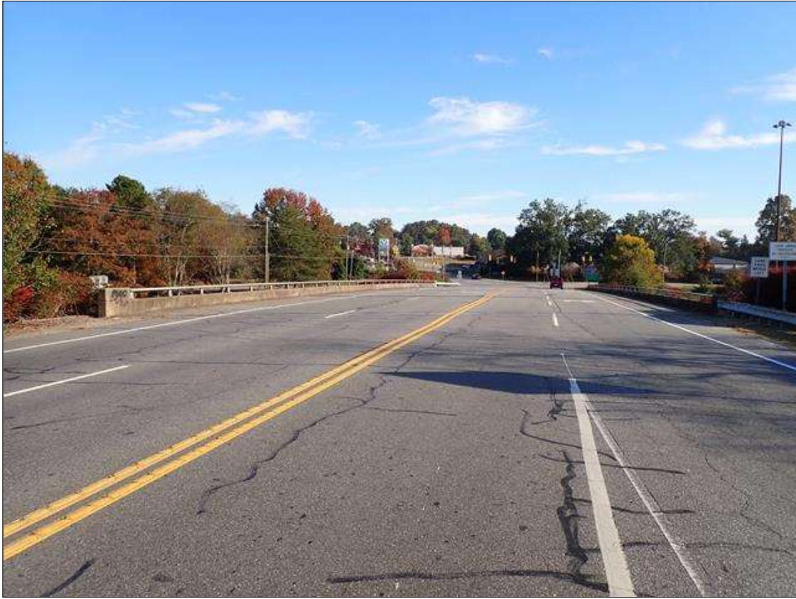
south approach looking north
