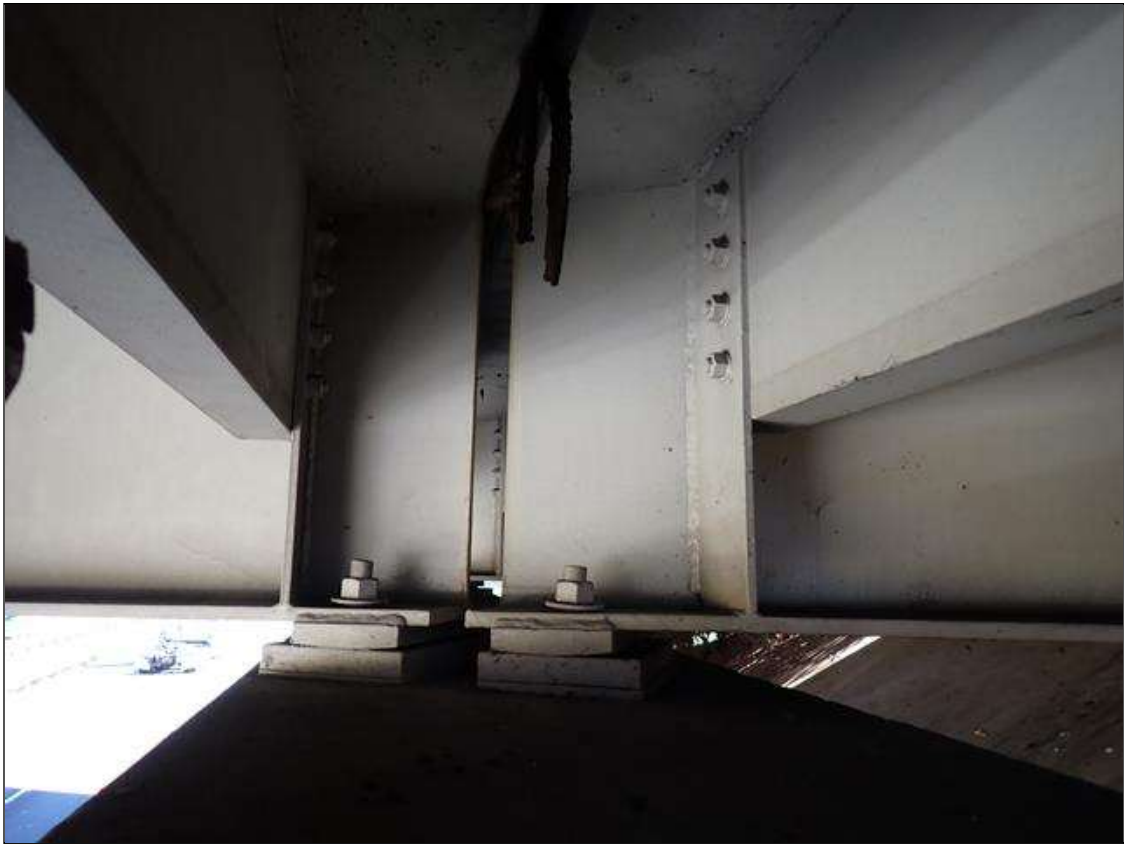
beams over bent
