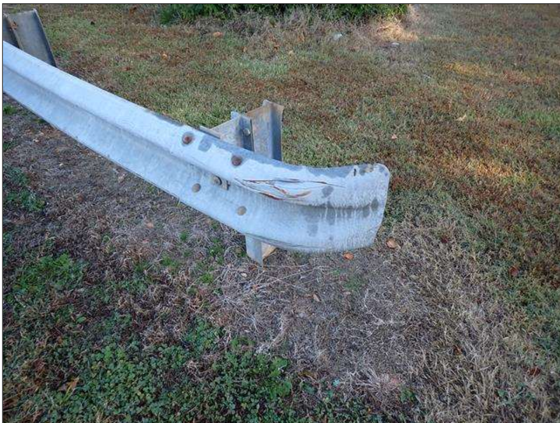
southeast guardrail termination
