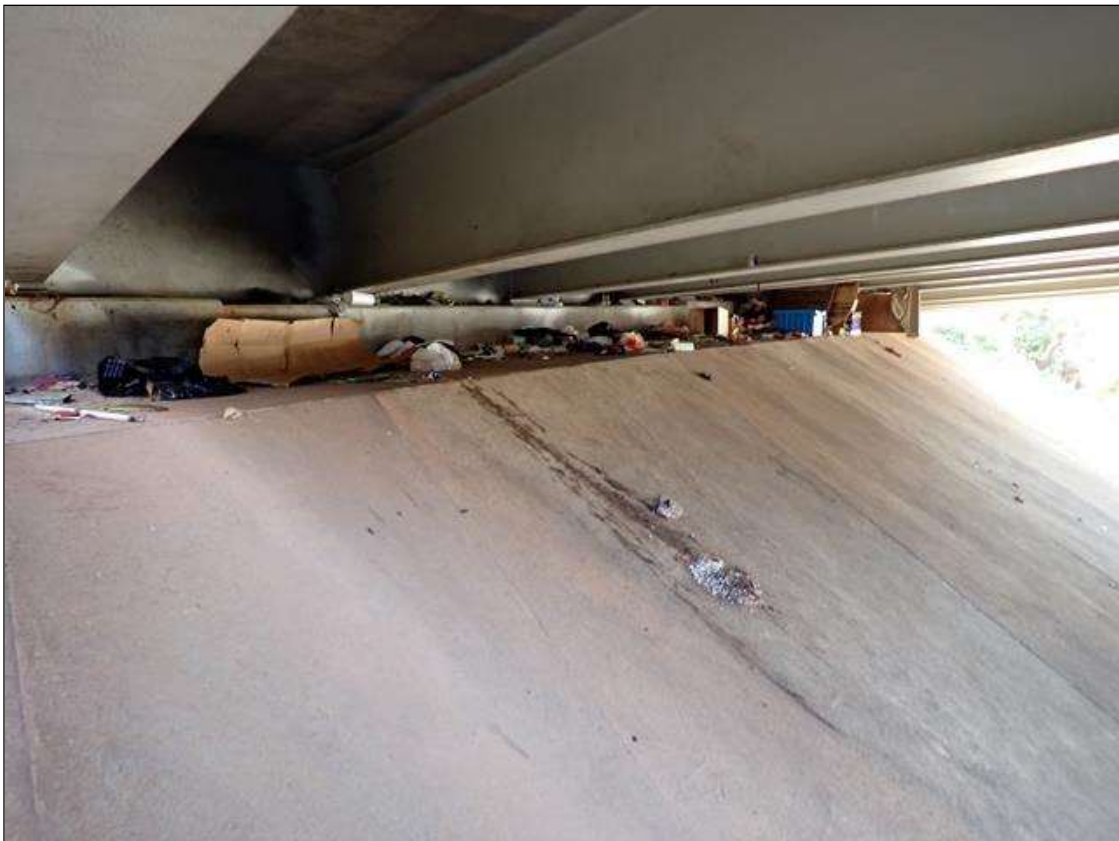
end bent 2 and slope protection
