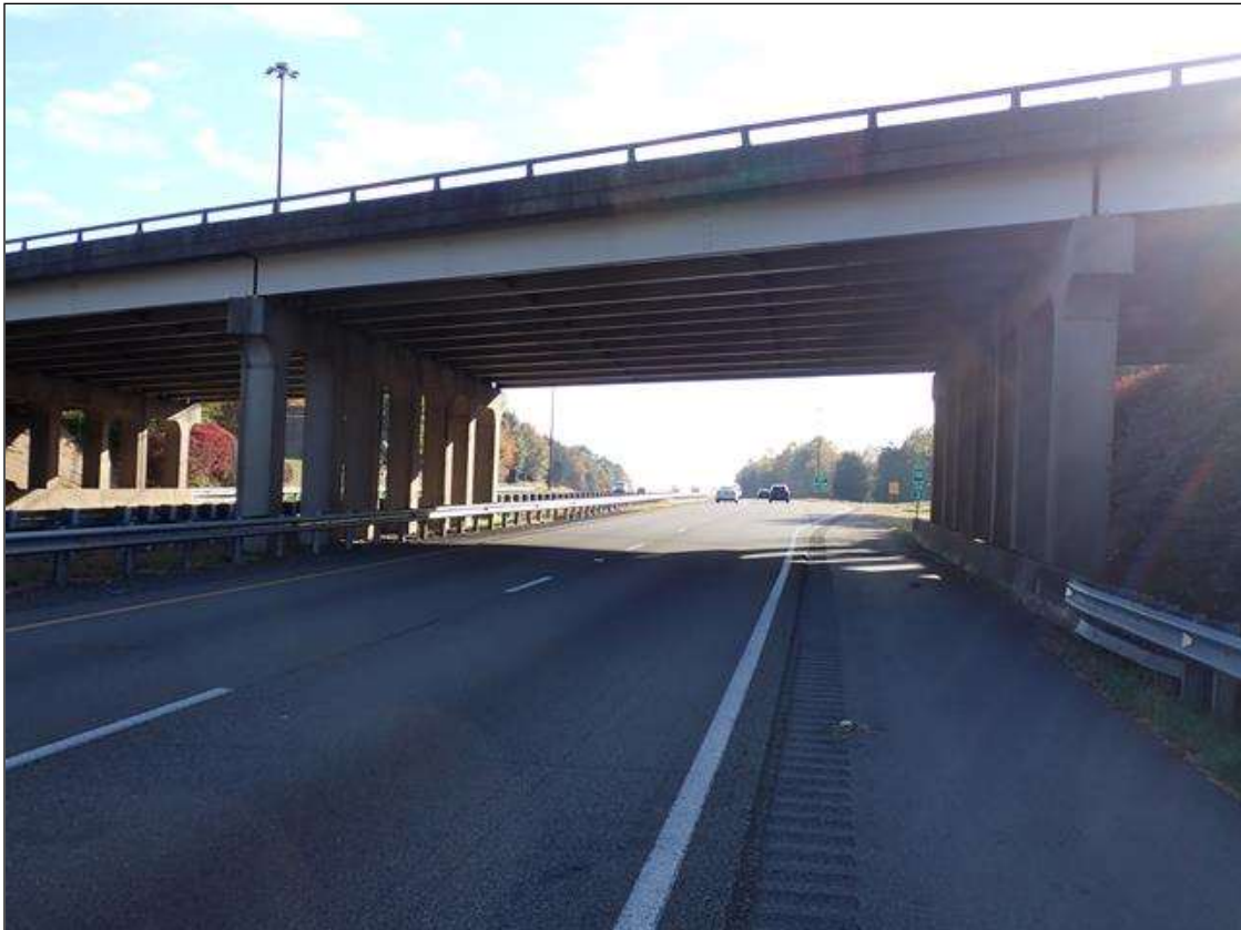
roadway under span 2, looking east (I-40 eastbound)
