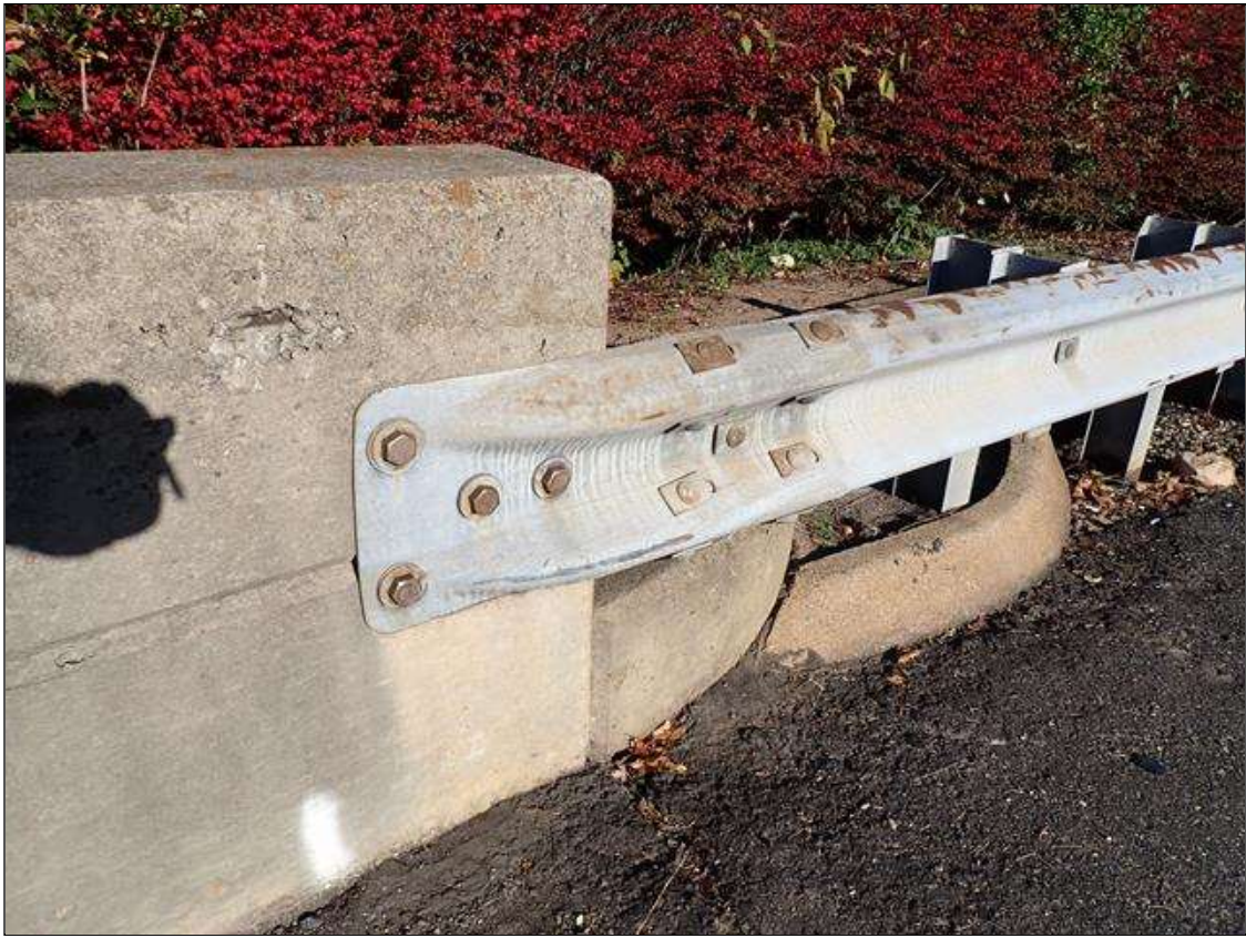
northwest guardrail attachment
