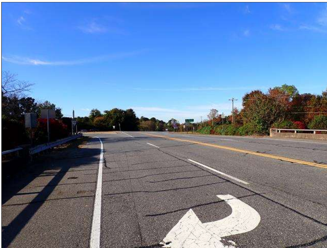
south approach looking south
