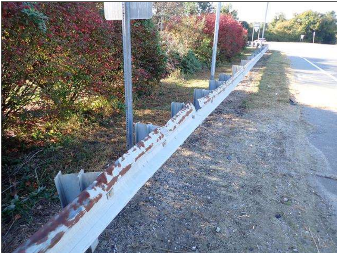
southeast guardrail transition
