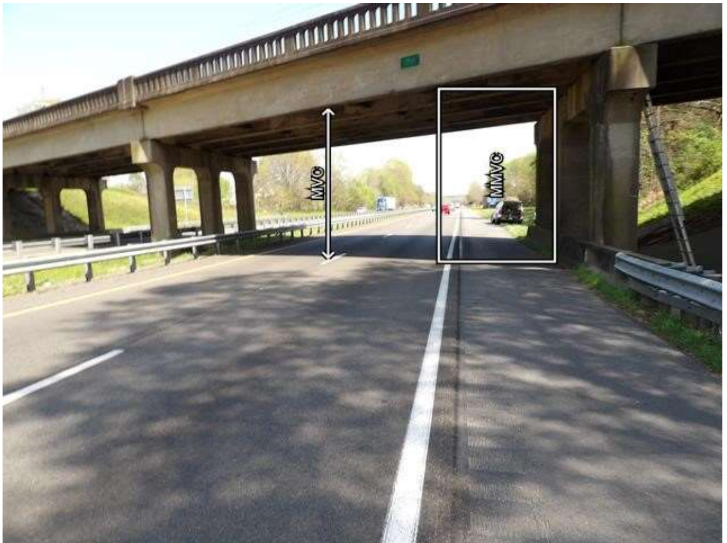
LOOKING EAST THROUGH SPAN 2
