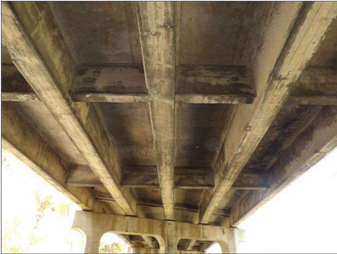
SUPERSTRUCTURE UNDERSIDE SPAN 2, ALL OTHERS SIMILAR
