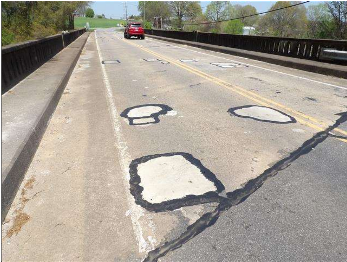
TYPICAL SOUND PATCHES IN SPAN 1 DECK
