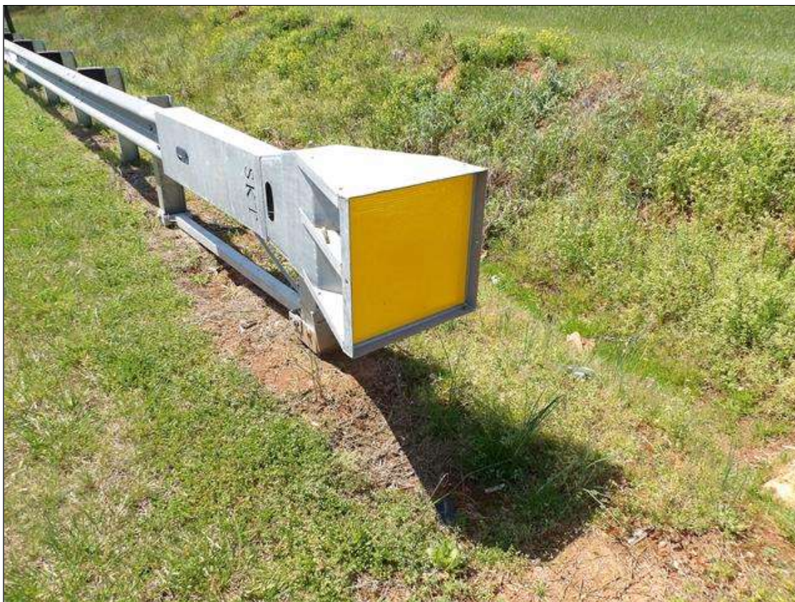
GUARDRAIL TERMINAL END NORTHWEST CORNER
