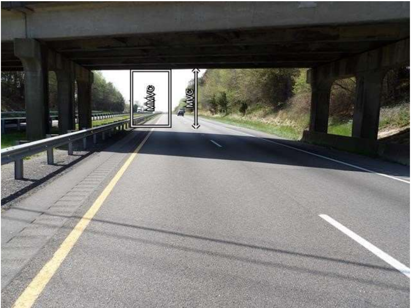
LOOKING WEST THROUGH SPAN 3
