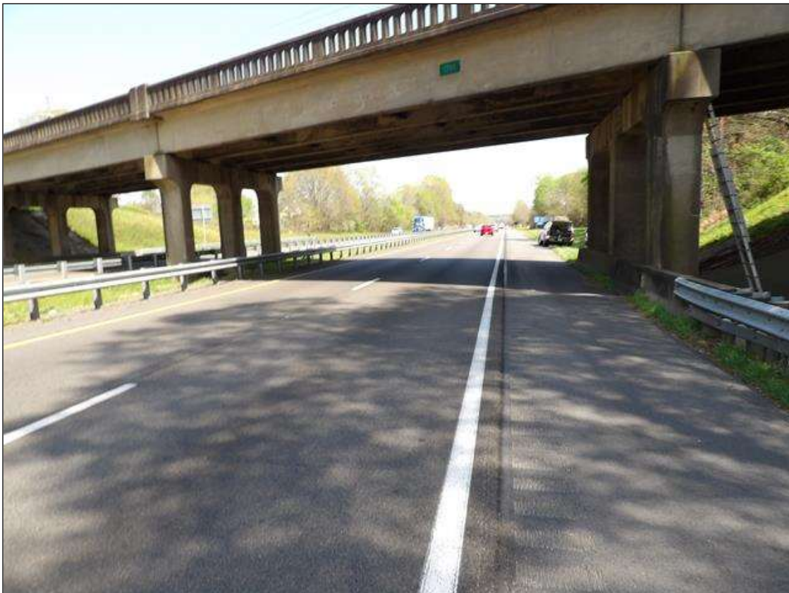
LOOKING EAST THROUGH SPAN 2
