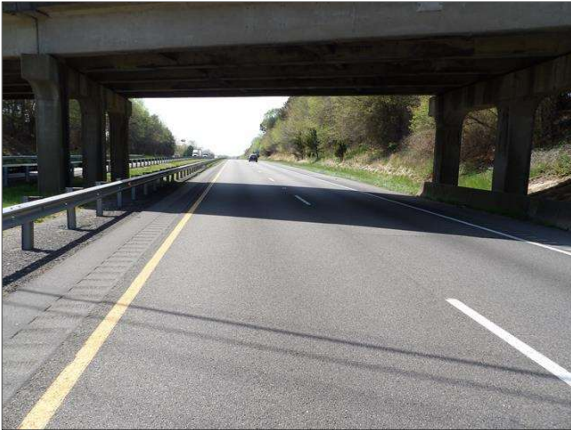
LOOKING WEST THROUGH SPAN 3
