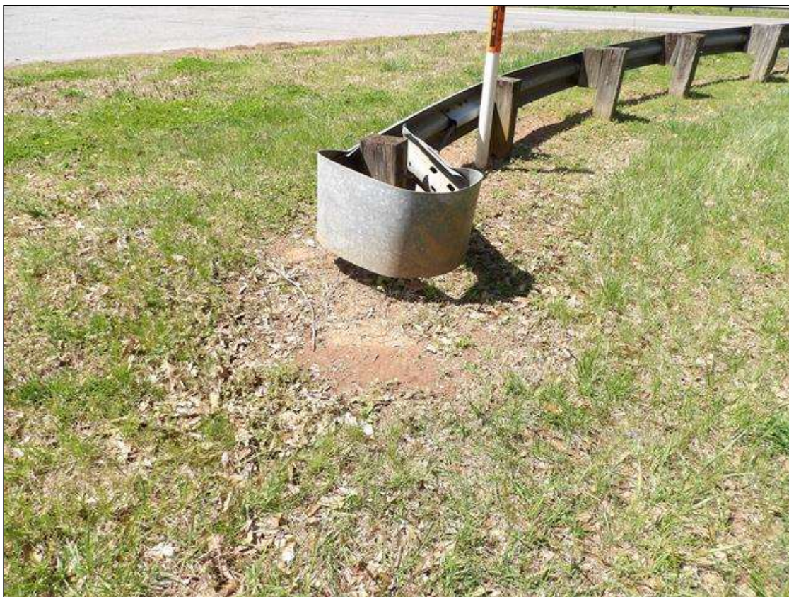
GUARDRAIL TERMINAL END SOUTHEAST CORNER, SOUTHWEST AND NORTHEAST SIMILAR
