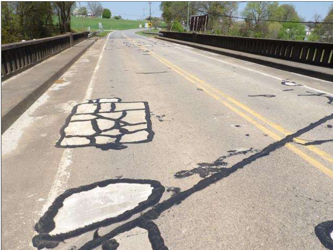
TYPICAL SOUND PATCHES IN SPAN 3 DECK
