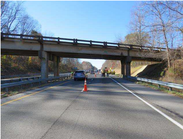
Crash at Bridge 110106 Closing I-40
