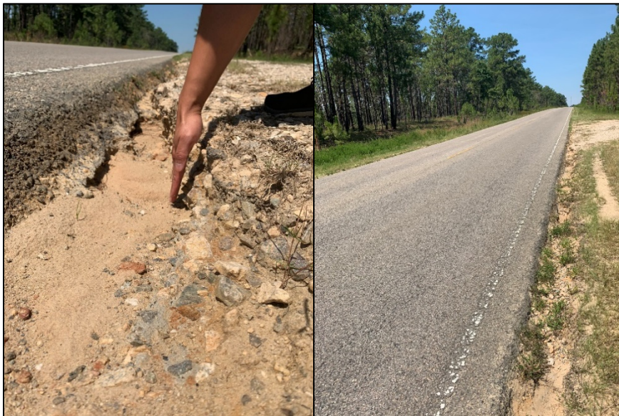
Figure 2: Examples of Road Conditions Around
