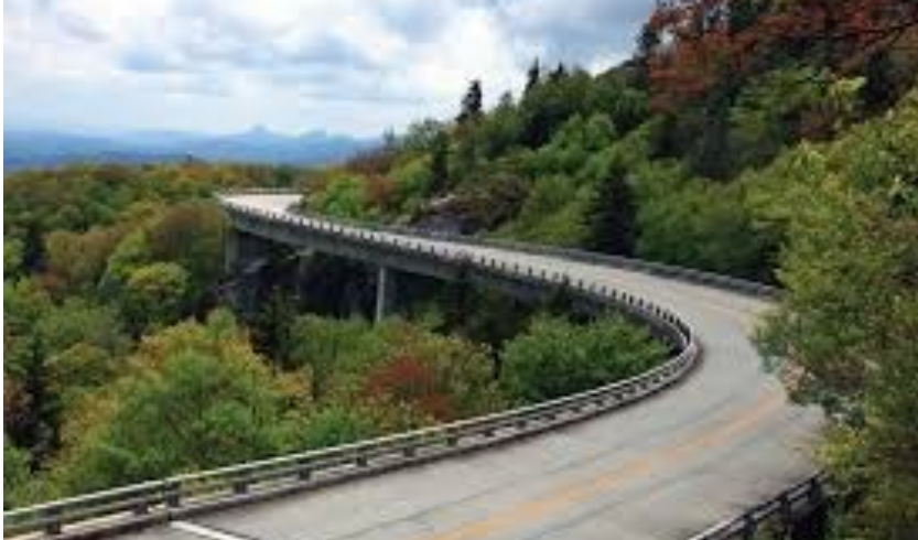
Linn Cove Viaduct
