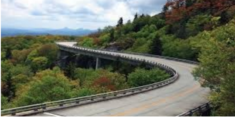
Linn Cove Viaduct
