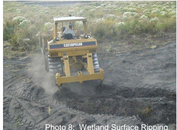
Photo 8: Wetland Surface Ripping
