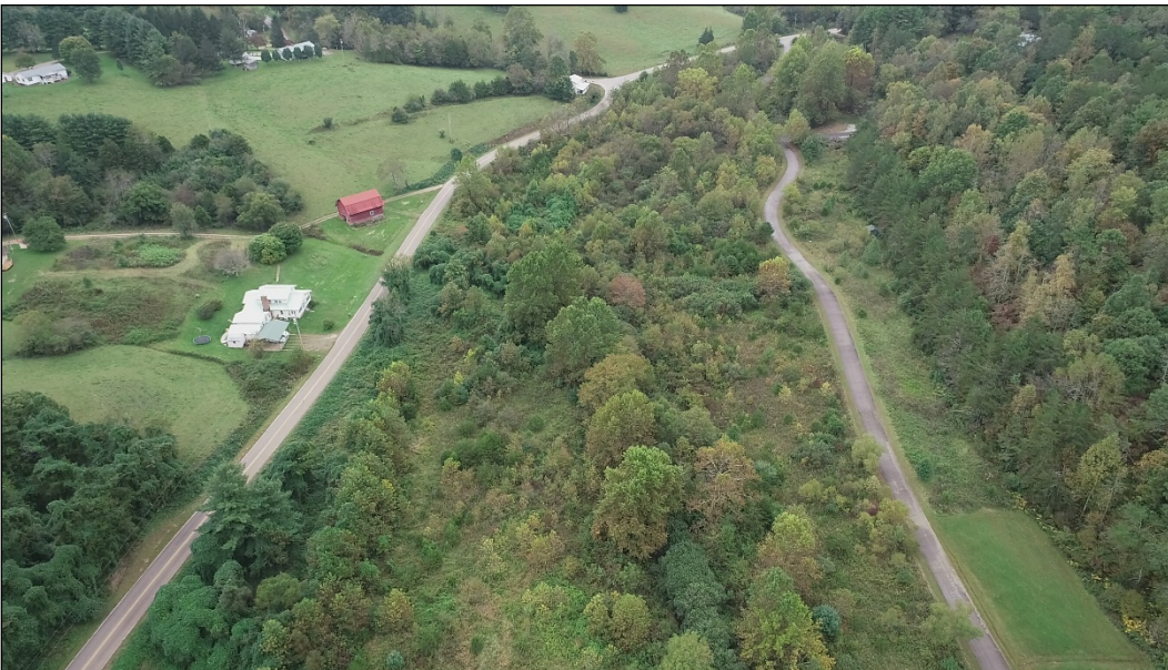
Photo 4 – Aerial view of the northeastern end of the site.
