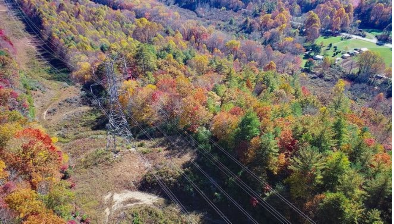
Image #4: Powerline easement through the site
