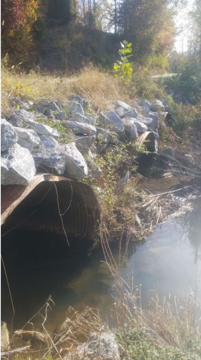
Image #1: Culvert on site
