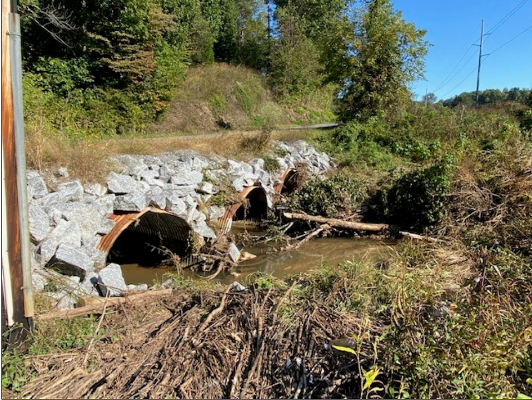
Photo 3 – Culvert repaired on south side of Propst Road.
