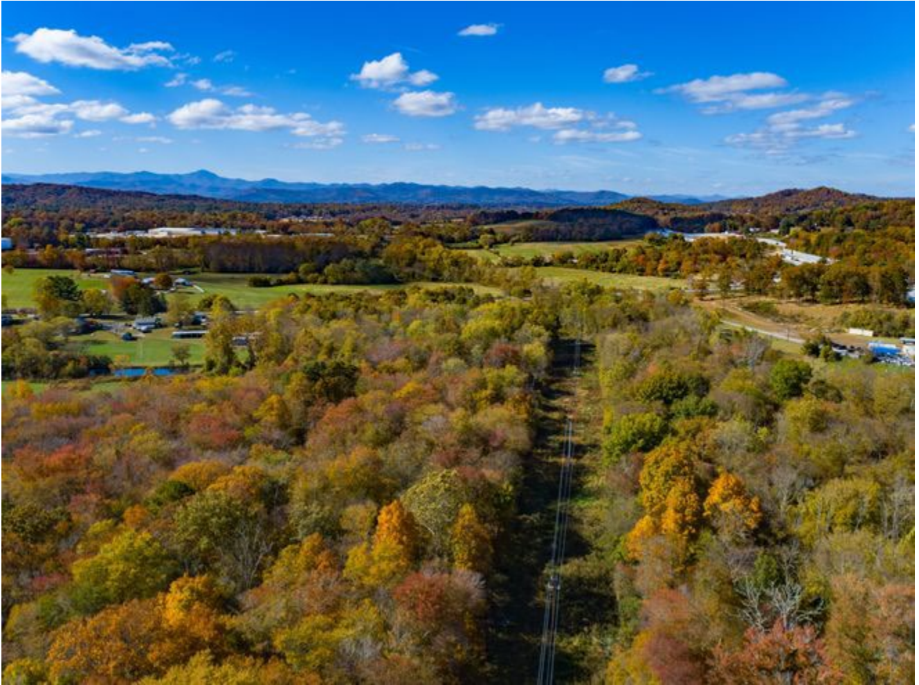
Image #4: Aerial view of the site
