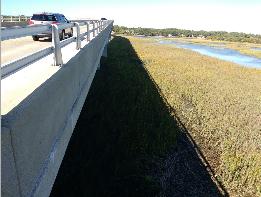
Photo 1 – View of eastern side of site.
