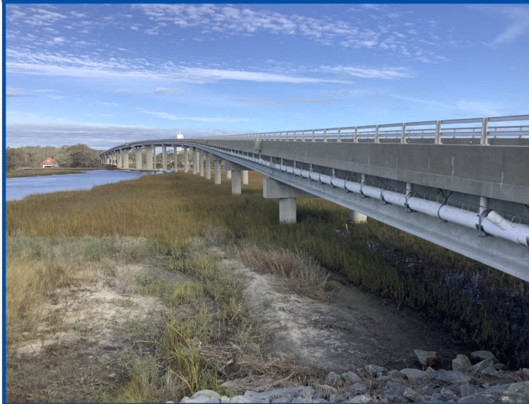
2 - UAS Site View
