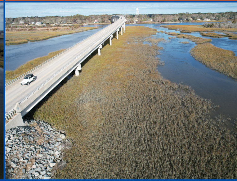
5 - UAS Site View
