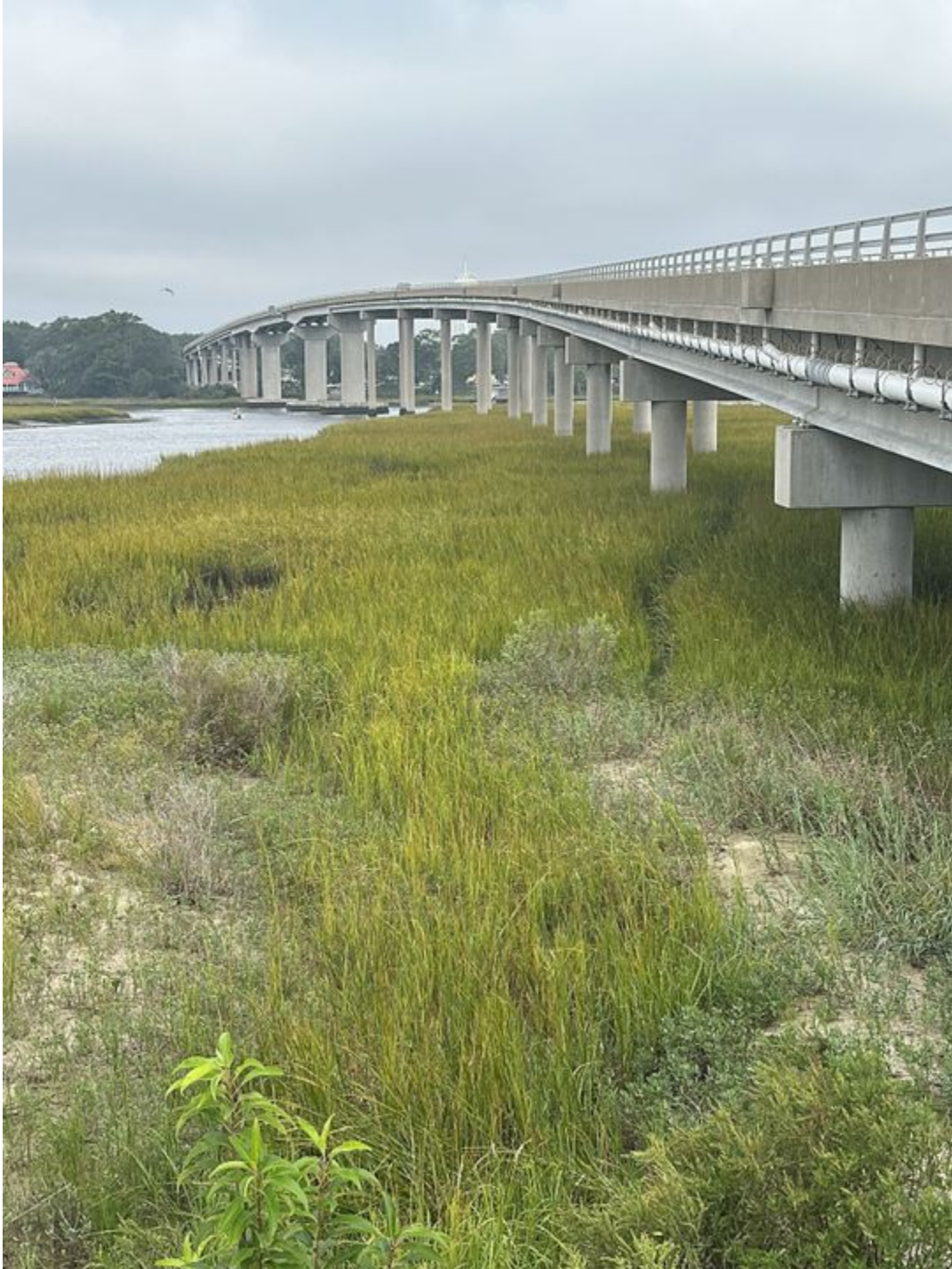
Image #1: View of interior of site along bridge.
