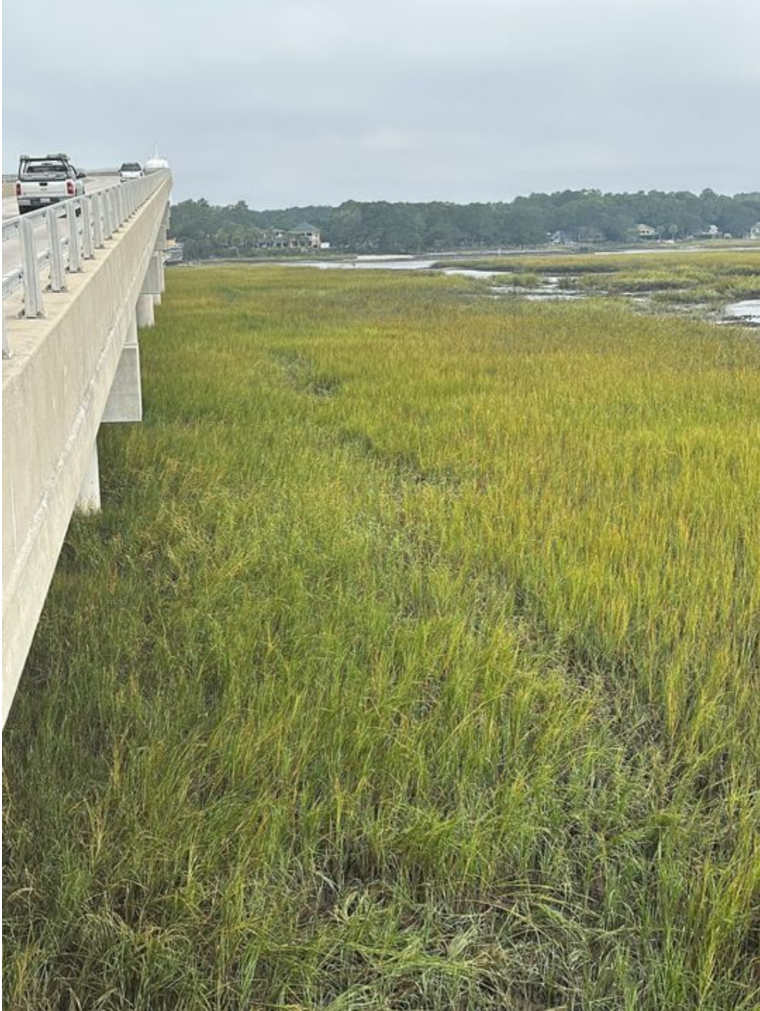
Image #2: View of interior of site on opposite side of bridge.
