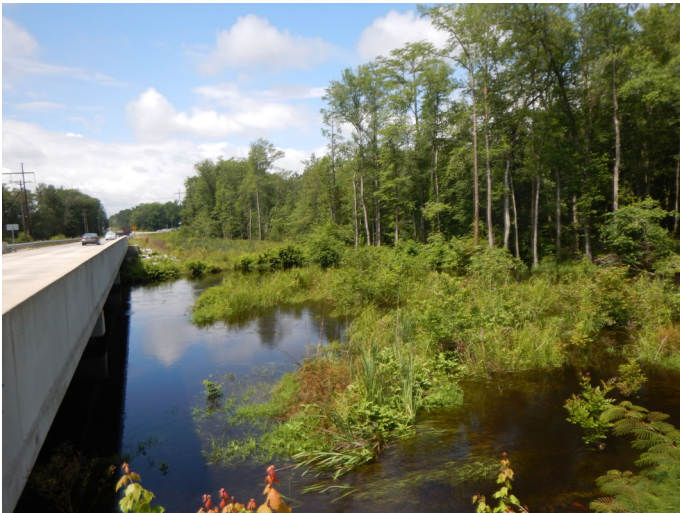
Overview photo looking southwest from US 15
