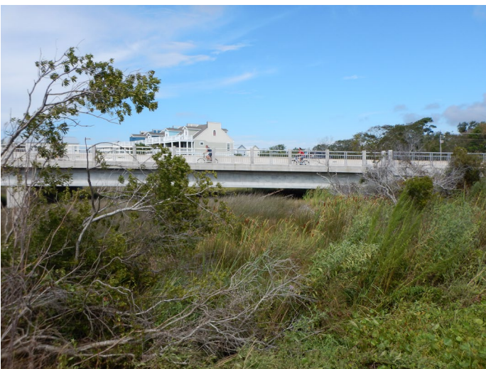
PP#5 Site 3CAMA (utility temp. impact)
