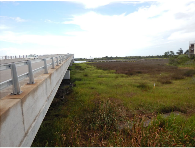
PP# 1 Site 4 (temporary work bridge)
