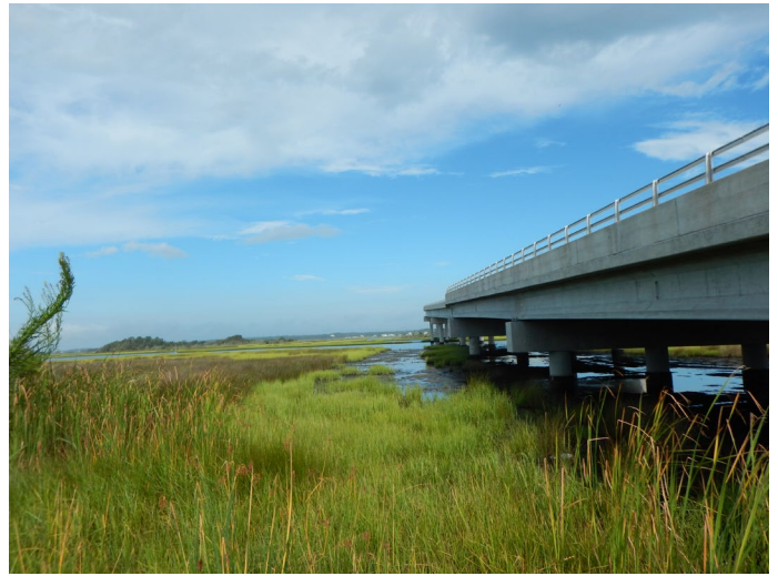
PP#2 Site 4 (temporary work bridge)
