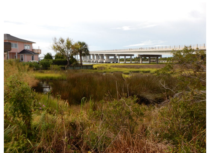
PP#6 Site 3CAMA (utility temp. impact)
